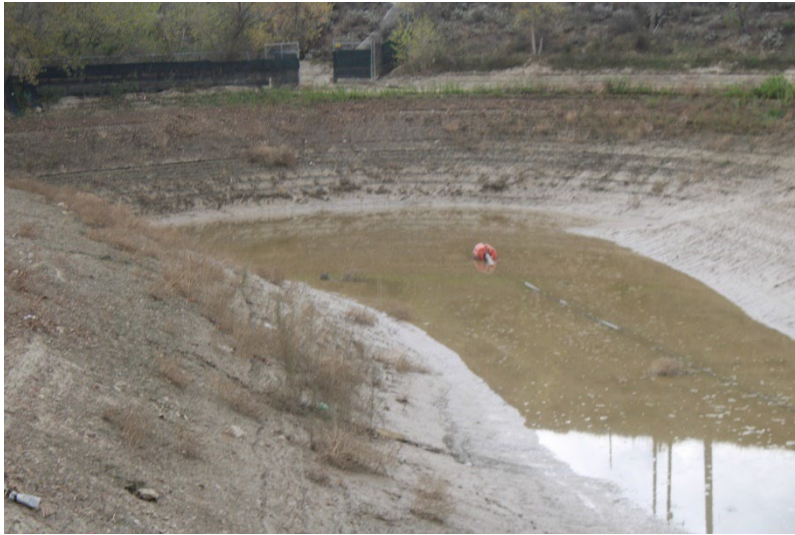
Photo 53: South Terminal and Catch Basins: November 13, 2025
