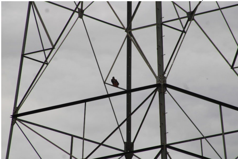
Photo 95: Northeast Sediment Basin: November 13, 2025
