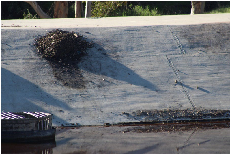
Photo 69: South Terminal and Catch Basins: December 10, 2025
