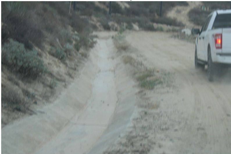
Photo 119: Landfill Perimeter Drainage Channel: November 13, 2025
