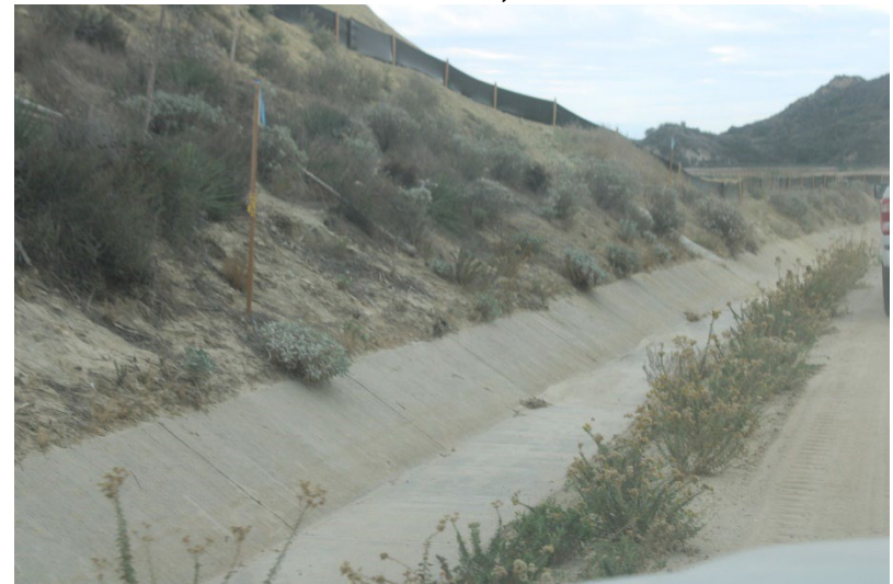
Photo 120: Landfill Perimeter Drainage Channel: November 13, 2025
