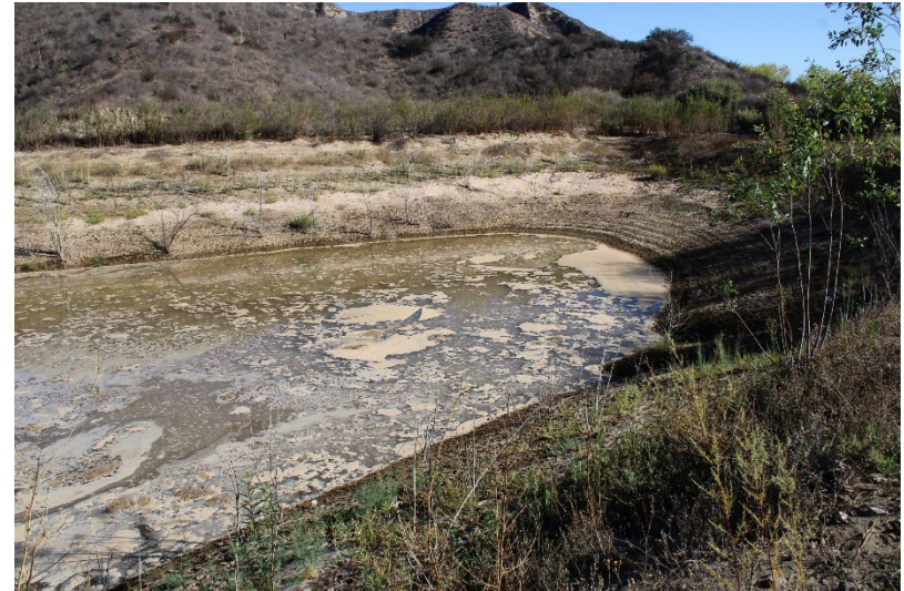
Photo 86: Northeast Sediment Basin: October 16, 2025
