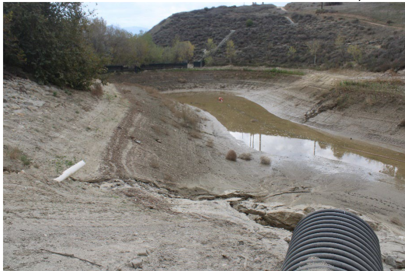
Photo 51: South Terminal and Catch Basins: November 13, 2025
