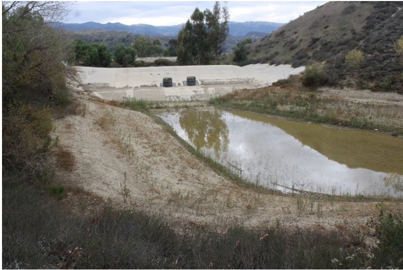
Photo 57: South Terminal and Catch Basins: November 13, 2025
