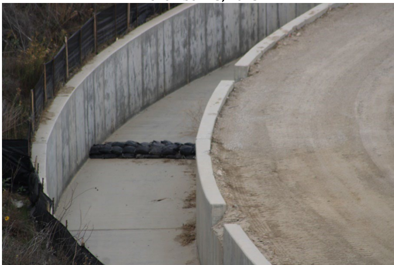
Photo 111: Landfill Perimeter Drainage Channel: November 13, 2025
