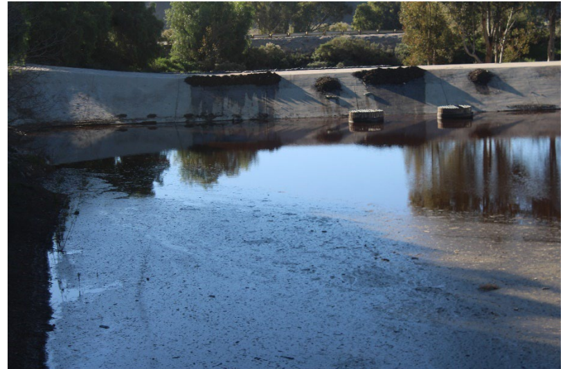
Photo 64: South Terminal and Catch Basins: December 10, 2025
