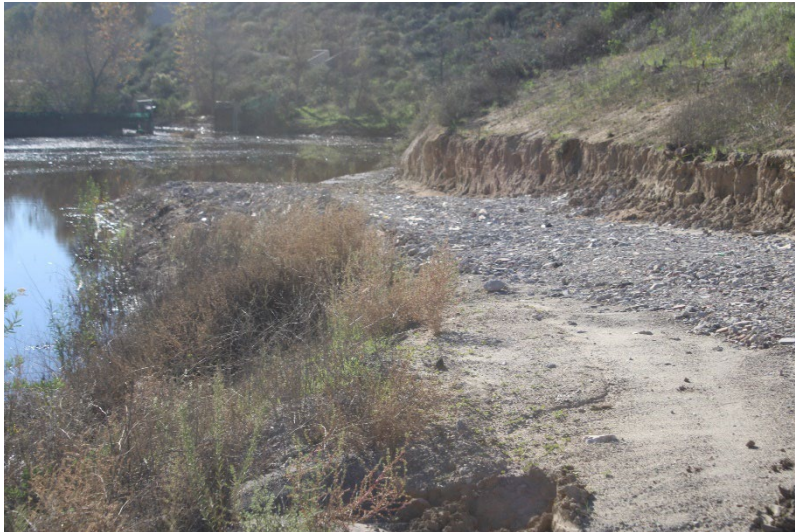
Photo 83: South Terminal and Catch Basins: December 10, 2025
