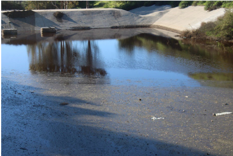
Photo 65: South Terminal and Catch Basins: December 10, 2025
