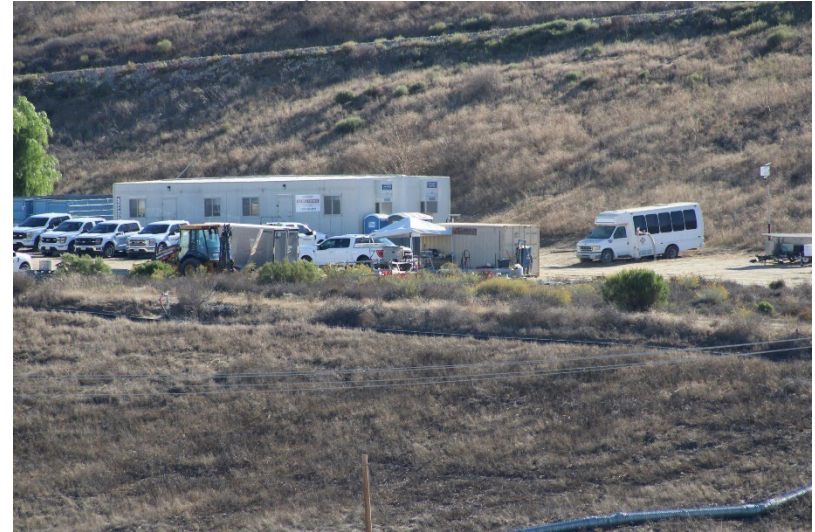
Photo 156: Maintenance and Admin Buildings: October 16, 2025
