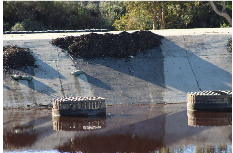
Photo 68: South Terminal and Catch Basins: December 10, 2025
