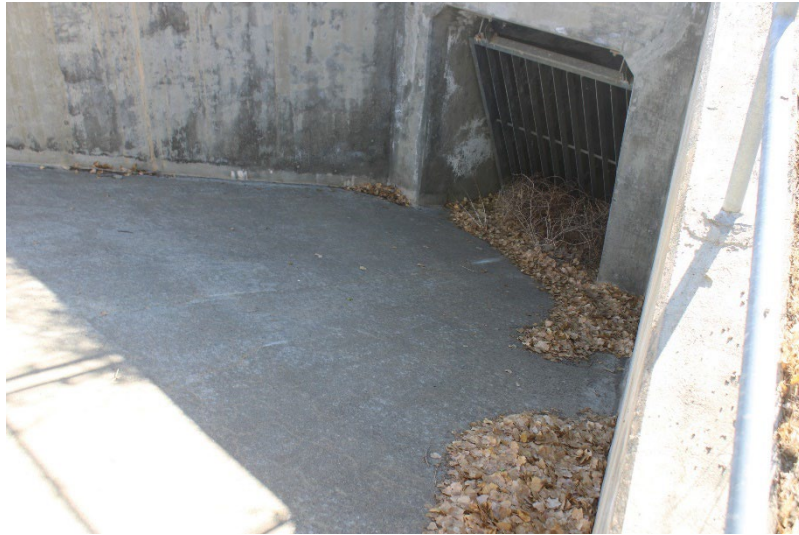
Photo 89: Northeast Sediment Basin: October 16, 2025
