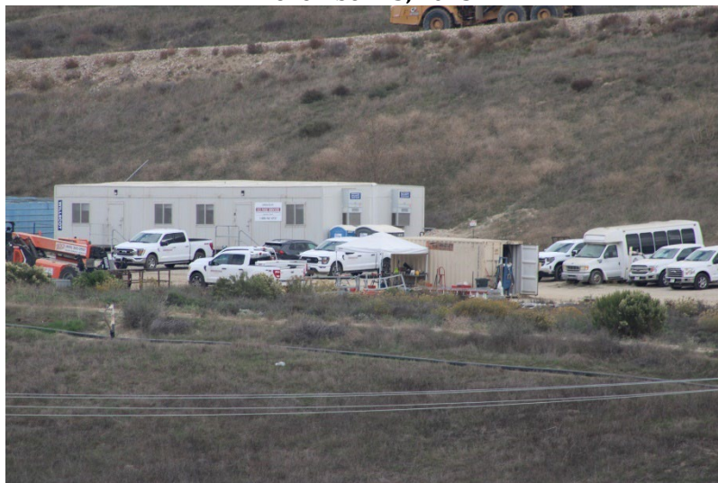
Photo 159: Maintenance and Admin Buildings: November 13, 2025
