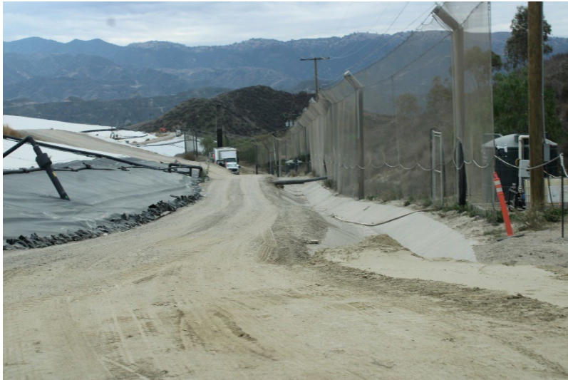
Photo 113: Landfill Perimeter Drainage Channel: November 13, 2025
