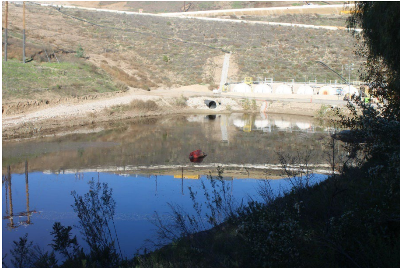
Photo 73: South Terminal and Catch Basins: December 10, 2025
