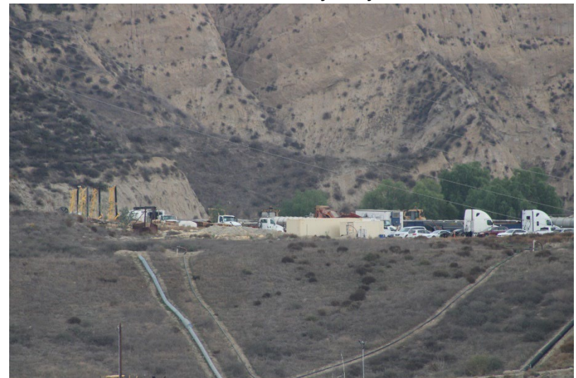
Photo 12: Closed Landfill - Primary Canyon: November 13, 2025
