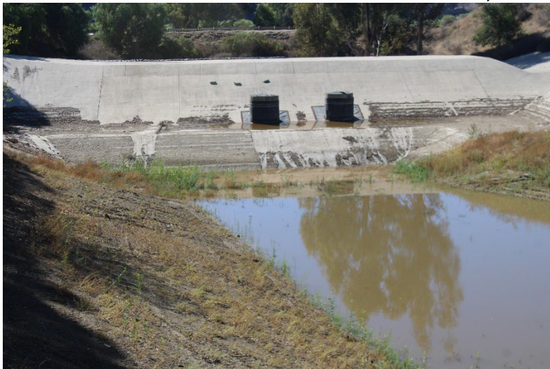
Photo 47: South Terminal and Catch Basins: October 16, 2025
