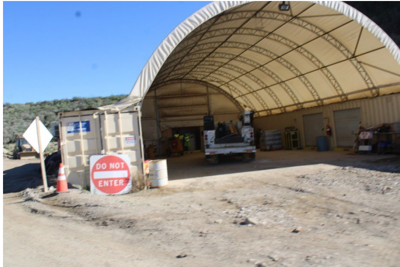
Photo 161: Maintenance and Admin Buildings: December 10, 2025
