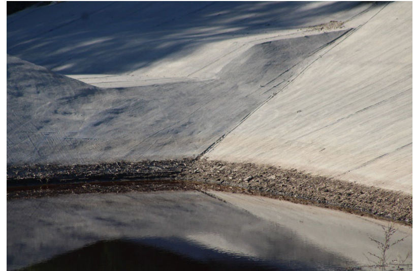
Photo 70: South Terminal and Catch Basins: December 10, 2025
