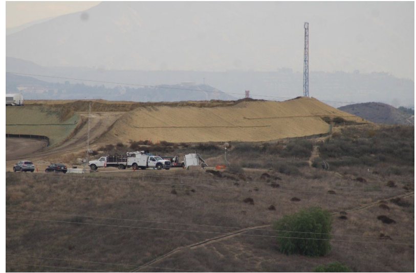
Photo 14: Closed Landfill - Primary Canyon: November 13, 2025
