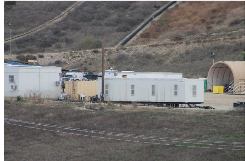
Photo 158: Maintenance and Admin Buildings: November 13, 2025
