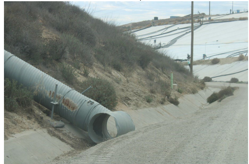
Photo 116: Landfill Perimeter Drainage Channel: November 13, 2025
