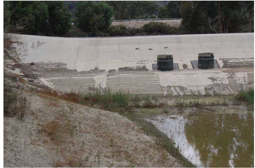
Photo 58: South Terminal and Catch Basins: November 13, 2025
