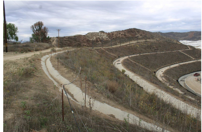
Photo 106: Landfill Perimeter Drainage Channel: November 13, 2025
