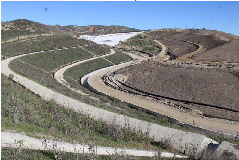
Photo 123: Landfill Perimeter Drainage Channel: December 10, 2025
