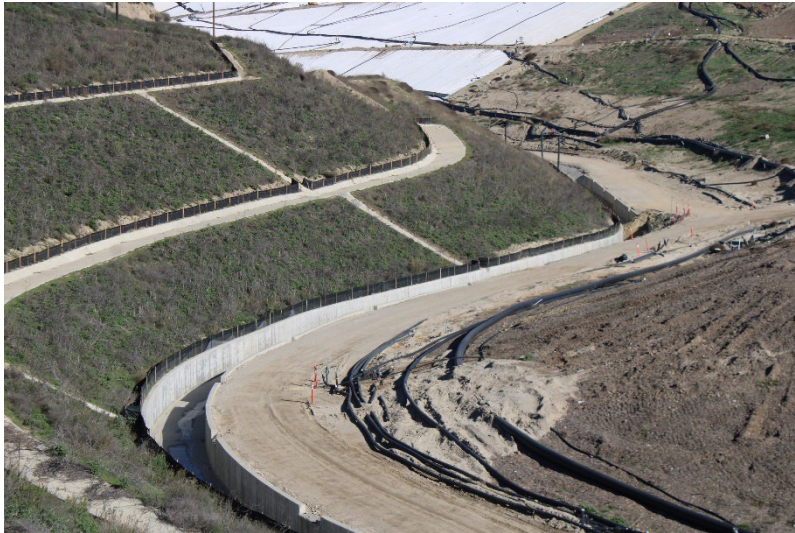
Photo 125: Landfill Perimeter Drainage Channel: December 10, 2025
