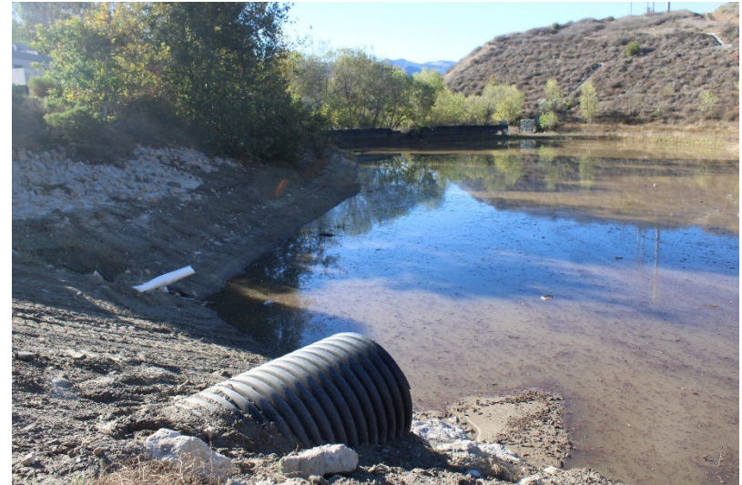
Photo 42: South Terminal and Catch Basins: October 16, 2025
