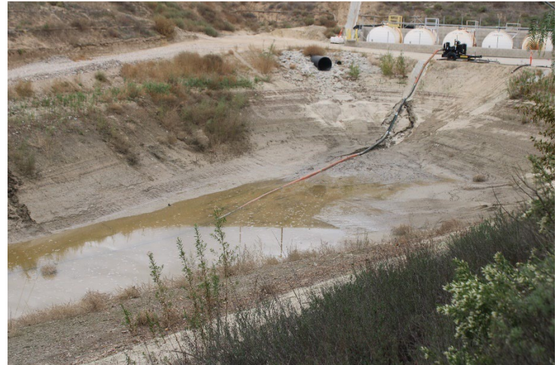
Photo 62: South Terminal and Catch Basins: November 13, 2025
