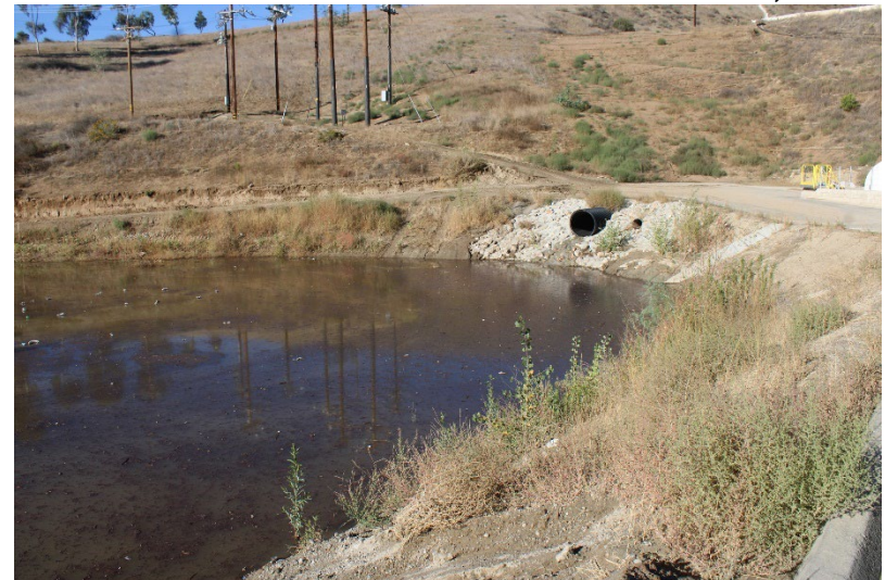
Photo 44: South Terminal and Catch Basins: October 16, 2025
