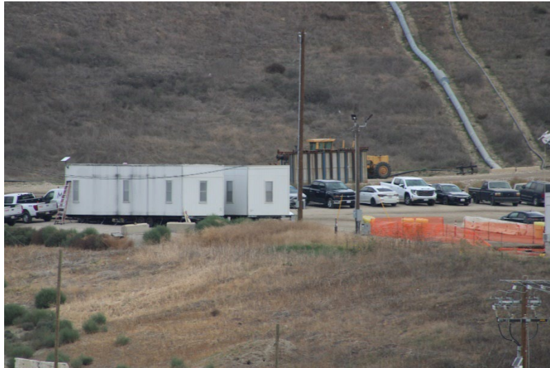
Photo 157: Maintenance and Admin Buildings: November 13, 2025
