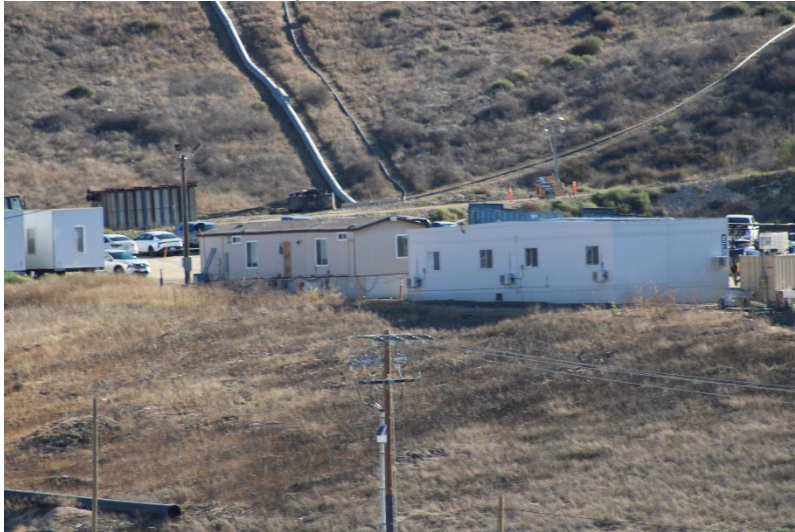
Photo 155: Maintenance and Admin Buildings: October 16, 2025
