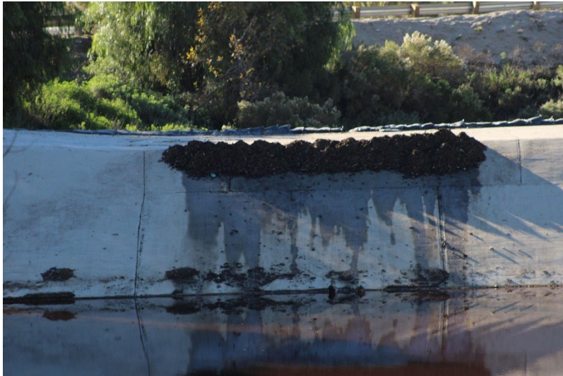
Photo 67: South Terminal and Catch Basins: December 10, 2025
