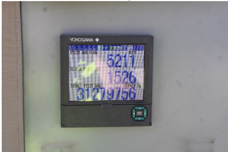
Photo 151: Flare 100, Flare 150 and Flare 250: December 10, 2025
