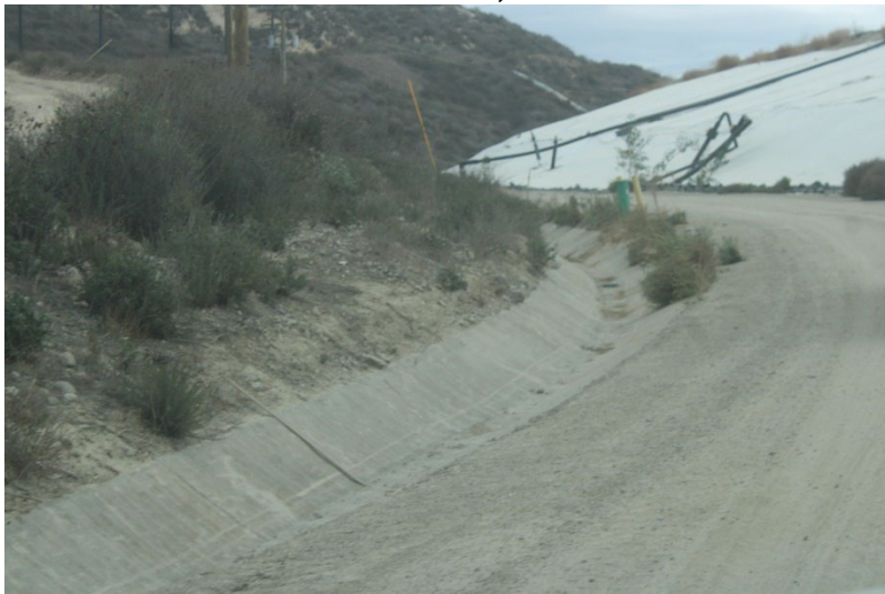
Photo 115: Landfill Perimeter Drainage Channel: November 13, 2025
