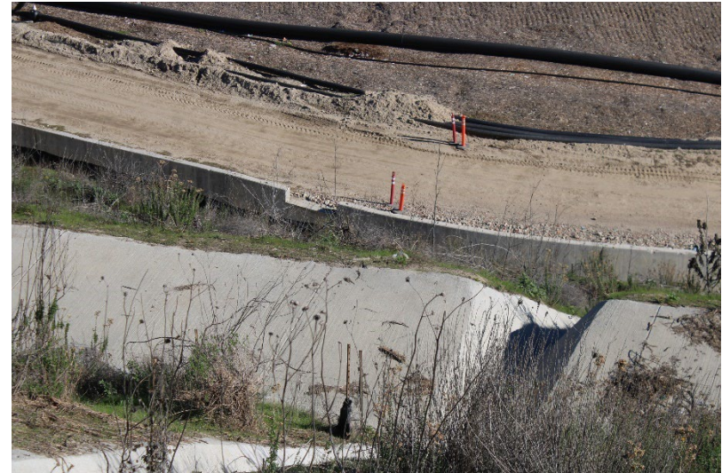
Photo 126: Landfill Perimeter Drainage Channel: December 10, 2025
