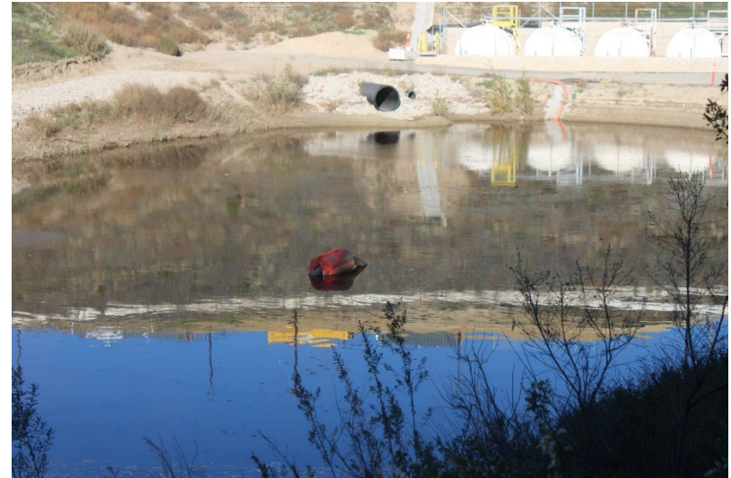
Photo 74: South Terminal and Catch Basins: December 10, 2025
