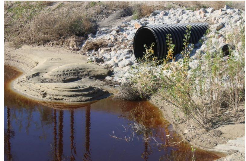
Photo 82: South Terminal and Catch Basins: December 10, 2025
