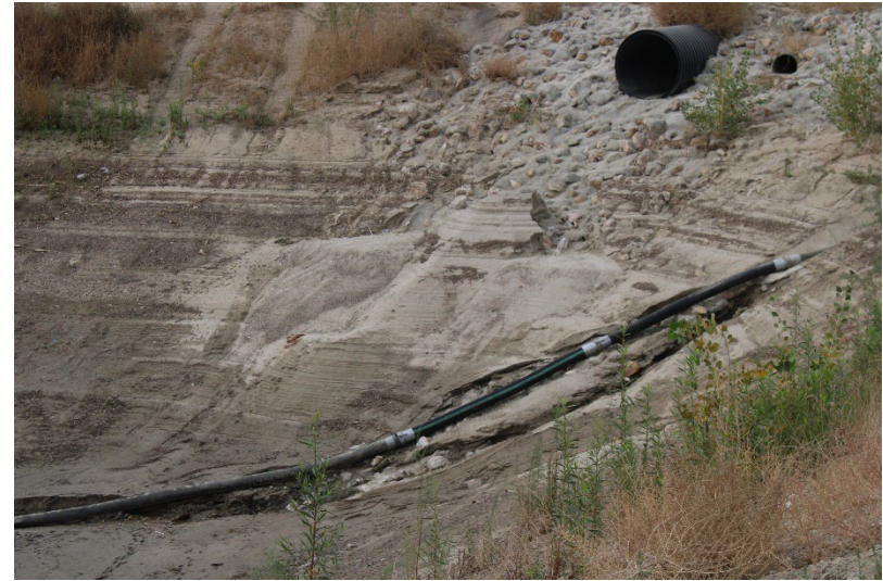
Photo 54: South Terminal and Catch Basins: November 13, 2025
