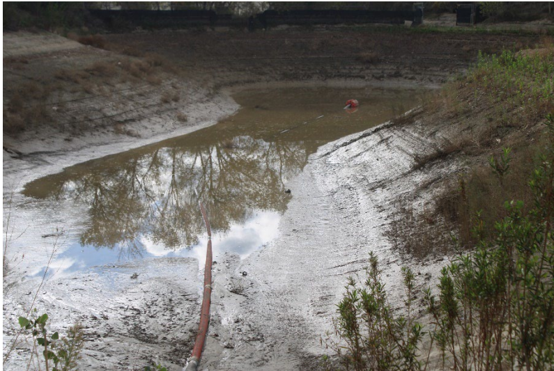
Photo 55: South Terminal and Catch Basins: November 13, 2025
