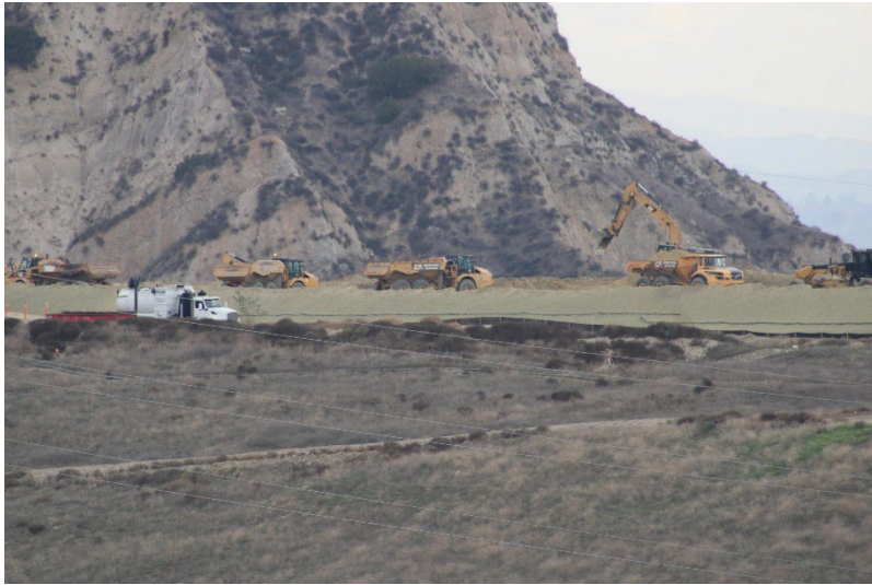
Photo 13: Closed Landfill - Primary Canyon: November 13, 2025
