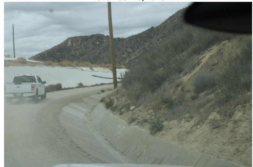
Photo 112: Landfill Perimeter Drainage Channel: November 13, 2025
