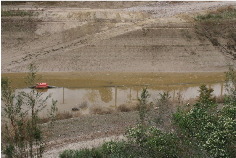
Photo 61: South Terminal and Catch Basins: November 13, 2025
