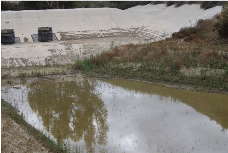
Photo 59: South Terminal and Catch Basins: November 13, 2025
