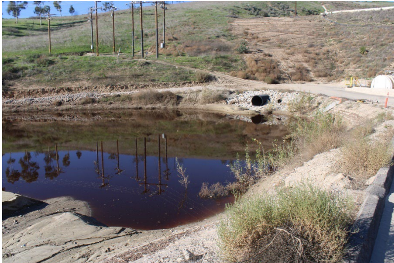
Photo 77: South Terminal and Catch Basins: December 10, 2025
