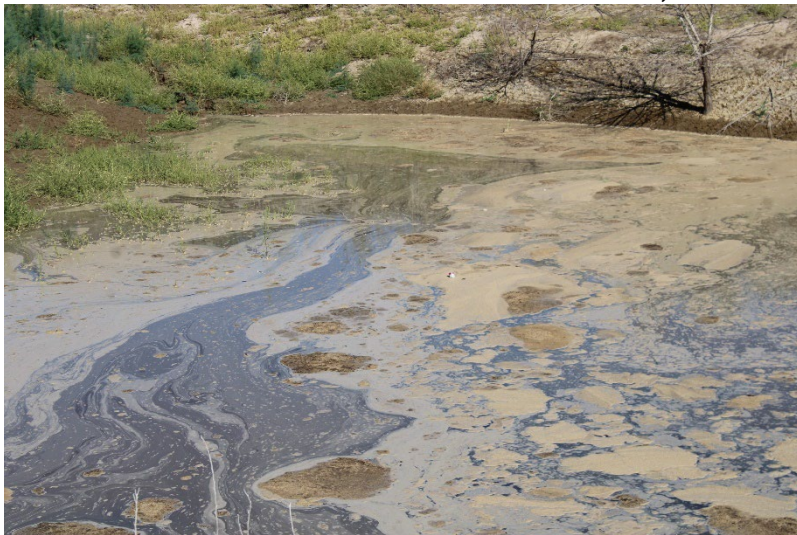
Photo 87: Northeast Sediment Basin: October 16, 2025
