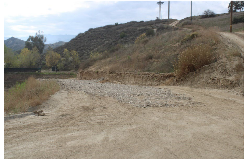
Photo 56: South Terminal and Catch Basins: November 13, 2025
