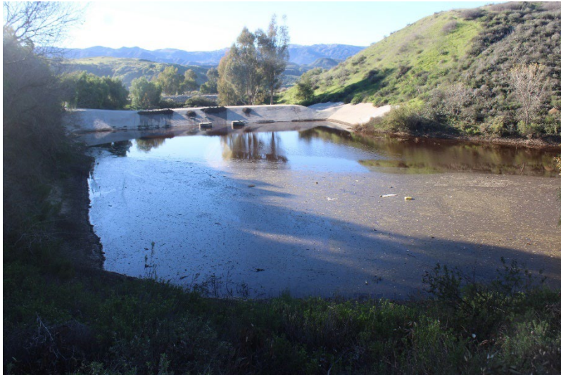
Photo 63: South Terminal and Catch Basins: December 10, 2025
