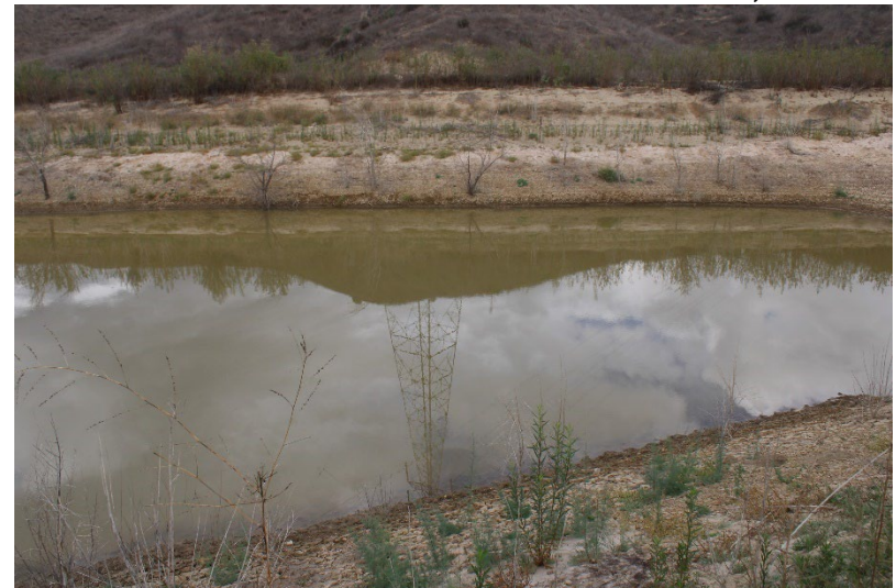
Photo 92: Northeast Sediment Basin: November 13, 2025
