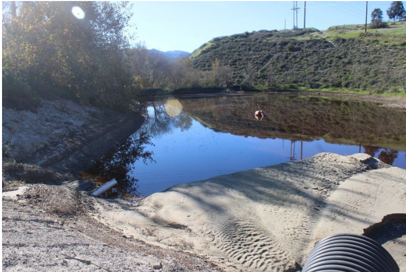
Photo 75: South Terminal and Catch Basins: December 10, 2025
