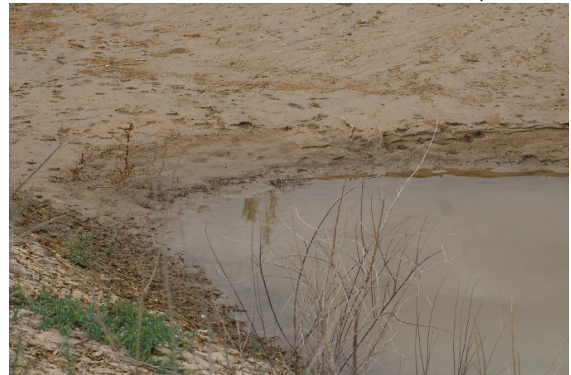
Photo 96: Northeast Sediment Basin: November 13, 2025
