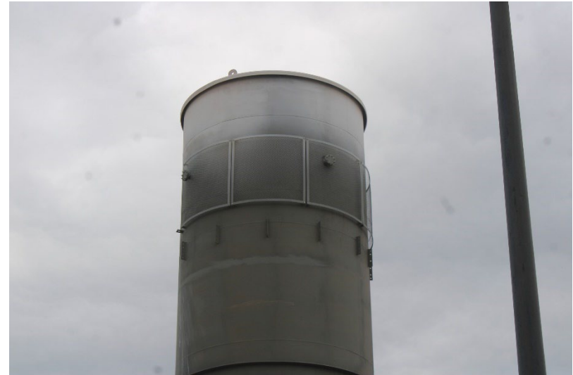
Photo 146: Flare 100, Flare 150 and Flare 250: November 13, 2025
