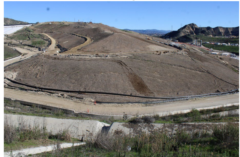
Photo 4: Cell 6 and Cell 8 Working Area: December 10, 2025
