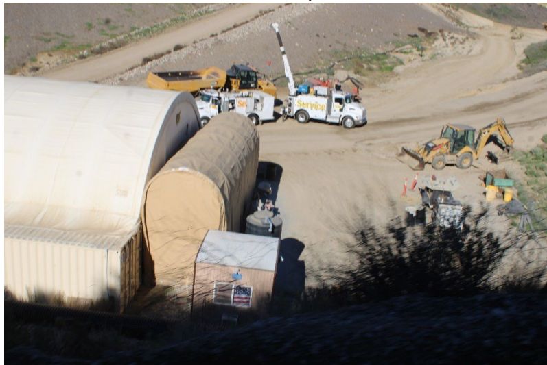
Photo 163: Maintenance and Admin Buildings: December 10, 2025
