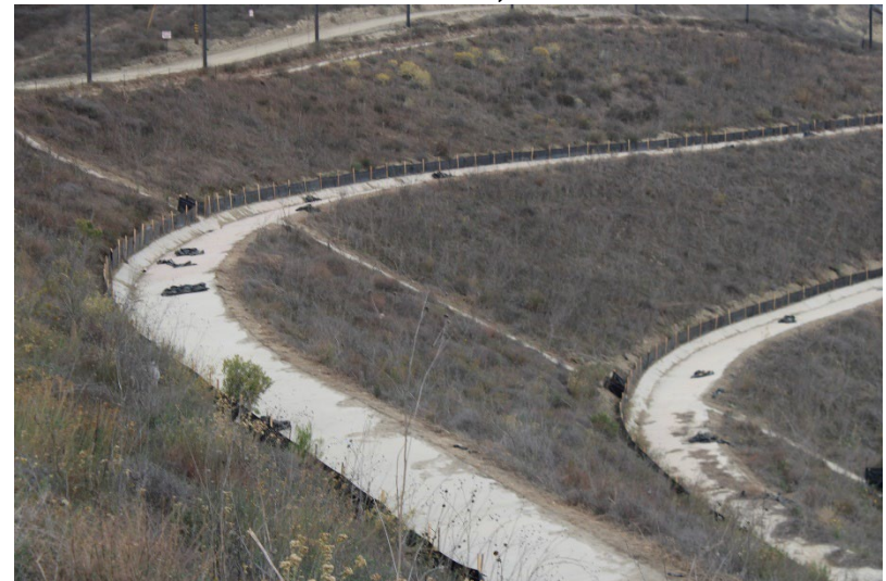
Photo 108: Landfill Perimeter Drainage Channel: November 13, 2025
