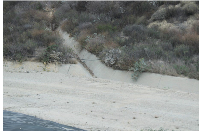
Photo 118: Landfill Perimeter Drainage Channel: November 13, 2025
