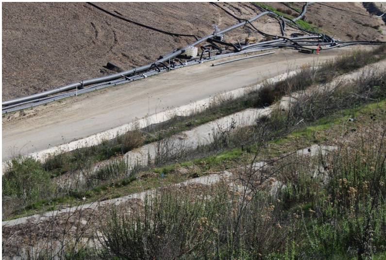
Photo 127: Landfill Perimeter Drainage Channel: December 10, 2025
