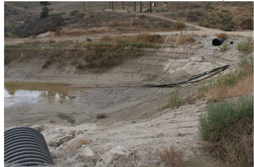
Photo 52: South Terminal and Catch Basins: November 13, 2025
