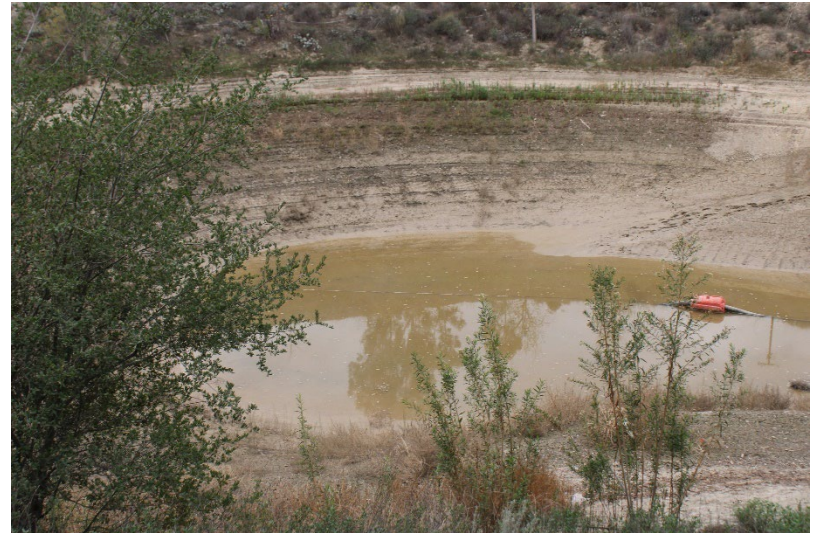
Photo 60: South Terminal and Catch Basins: November 13, 2025
