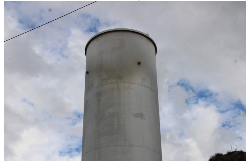
Photo 148: Flare 100, Flare 150 and Flare 250: November 13, 2025
