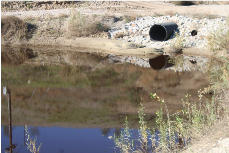
Photo 81: South Terminal and Catch Basins: December 10, 2025
