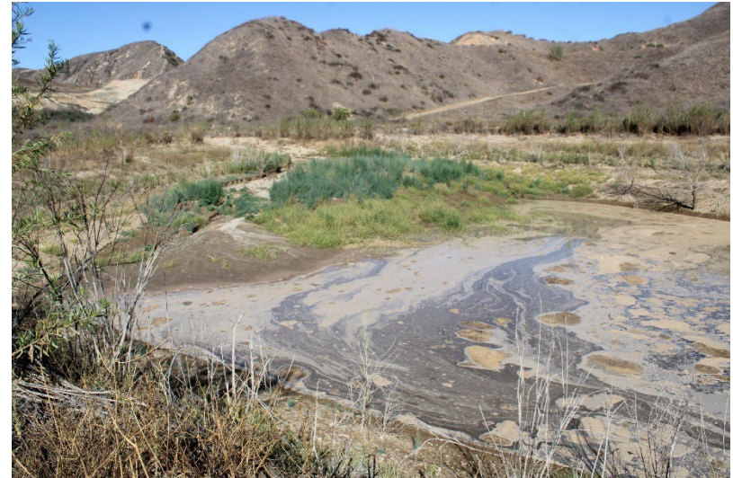
Photo 84: Northeast Sediment Basin: October 16, 2025
