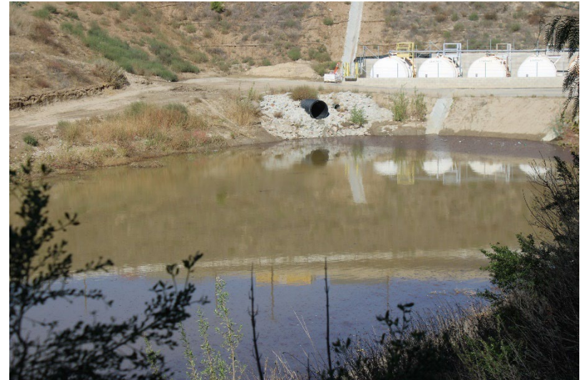
Photo 50: South Terminal and Catch Basins: October 16, 2025
