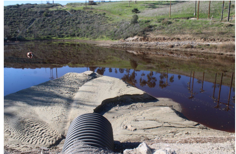
Photo 76: South Terminal and Catch Basins: December 10, 2025
