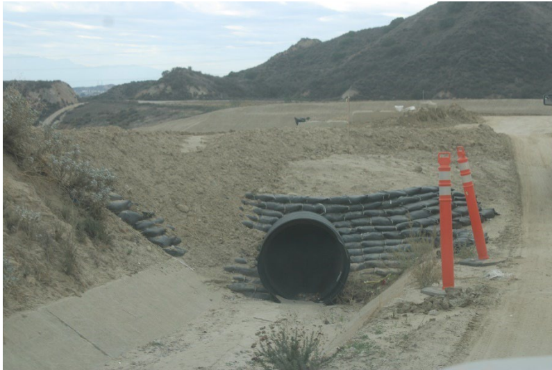
Photo 121: Landfill Perimeter Drainage Channel: November 13, 2025
