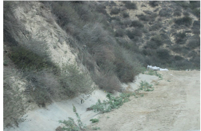
Photo 114: Landfill Perimeter Drainage Channel: November 13, 2025
