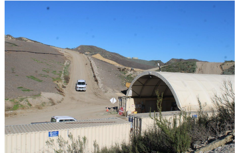
Photo 162: Maintenance and Admin Buildings: December 10, 2025
