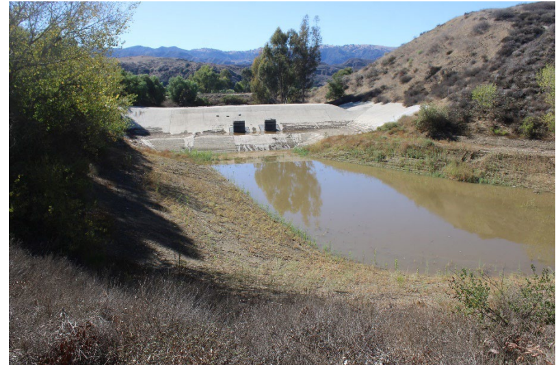
Photo 46: South Terminal and Catch Basins: October 16, 2025
