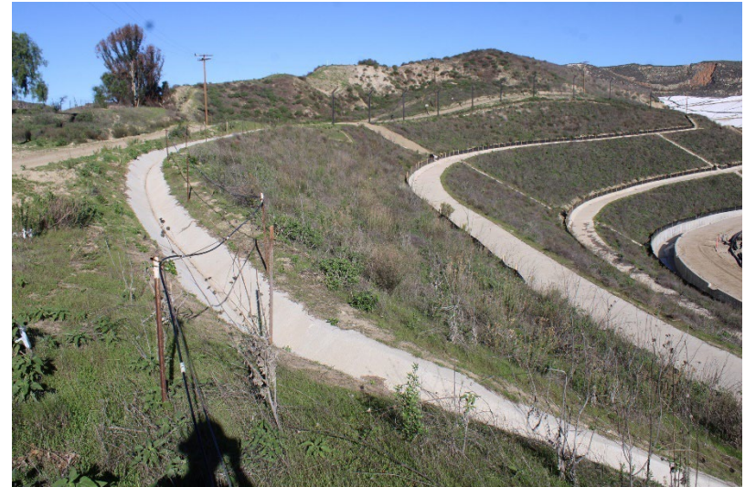
Photo 122: Landfill Perimeter Drainage Channel: December 10, 2025
