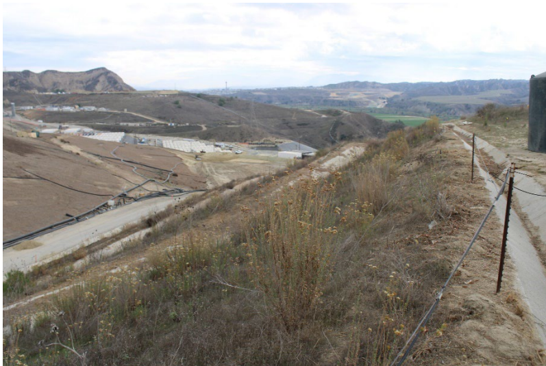
Photo 107: Landfill Perimeter Drainage Channel: November 13, 2025
