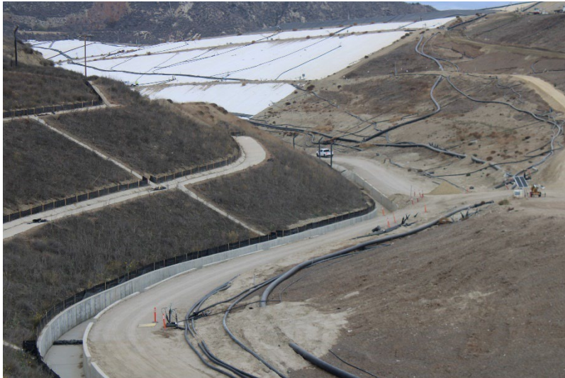
Photo 109: Landfill Perimeter Drainage Channel: November 13, 2025
