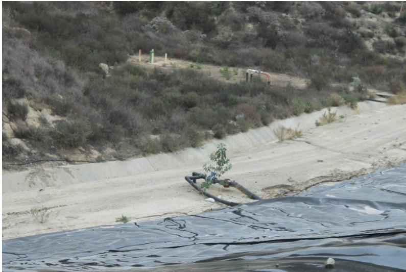
Photo 117: Landfill Perimeter Drainage Channel: November 13, 2025
