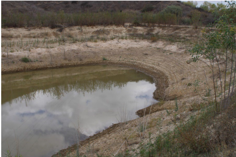
Photo 93: Northeast Sediment Basin: November 13, 2025
