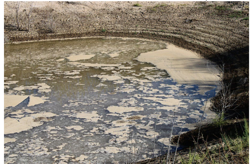
Photo 88: Northeast Sediment Basin: October 16, 2025
