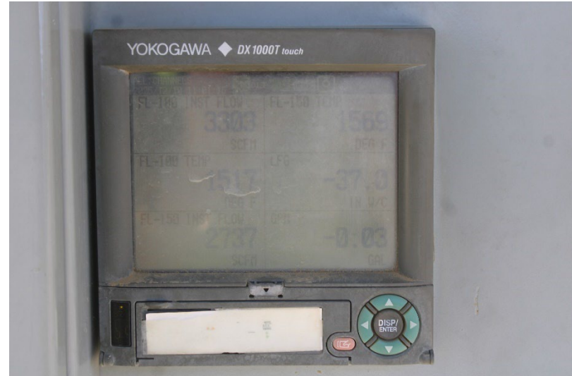
Photo 150: Flare 100, Flare 150 and Flare 250: December 10, 2025
