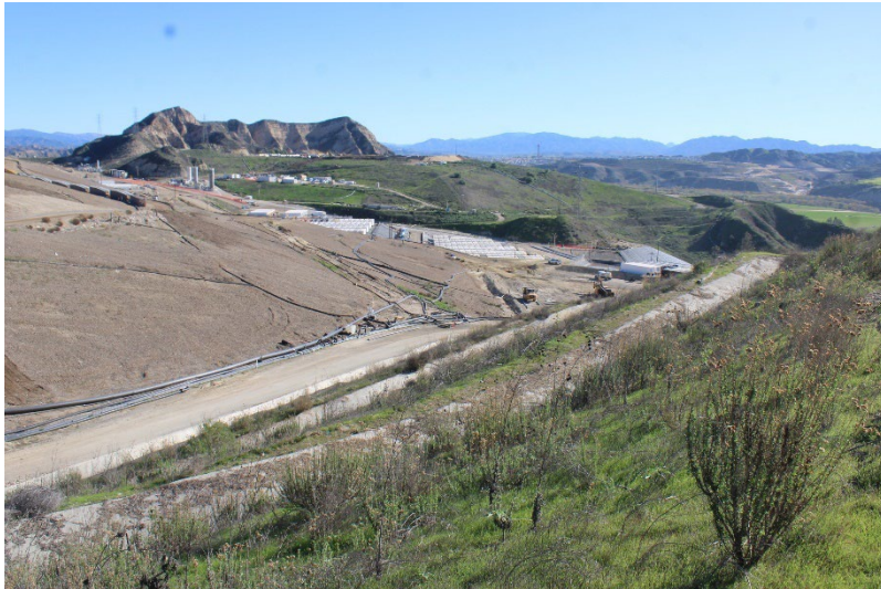
Photo 5: Cell 6 and Cell 8 Working Area: December 10, 2025
