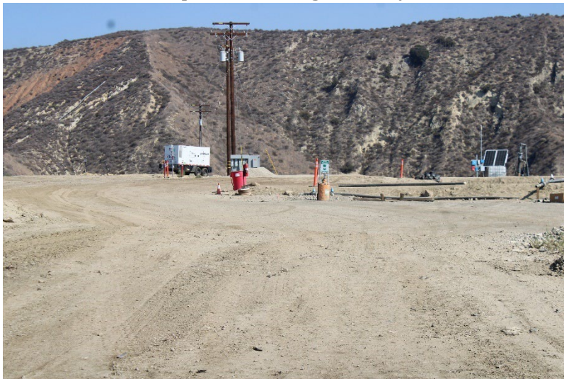
Photo 3: Top Deck Working Area: August 14, 2025
