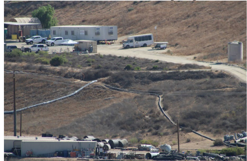
Photo 148: Maintenance and Admin Buildings: September 16, 2025
