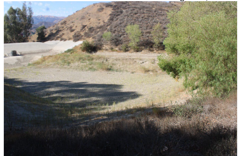
Photo 76: South Terminal and Catch Basins: September 16, 2025
