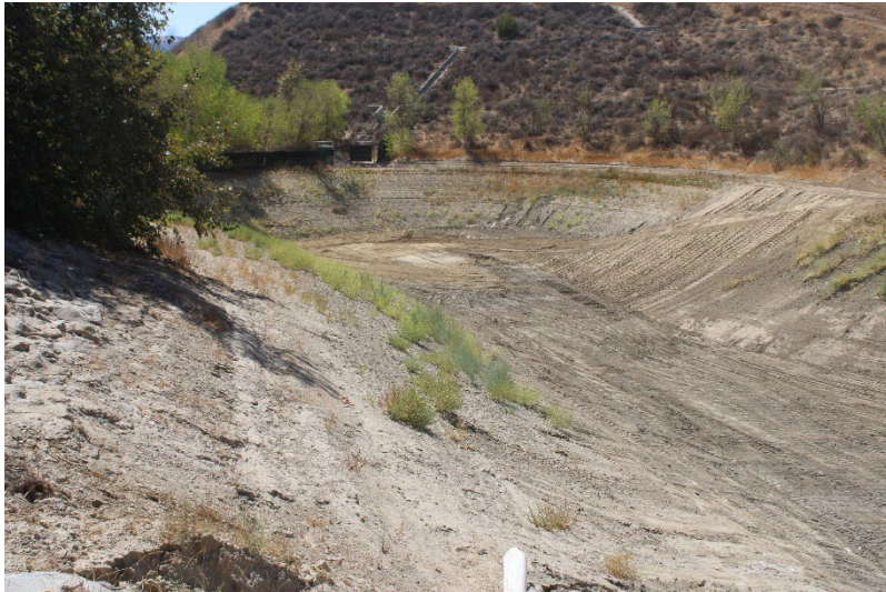
Photo 81: South Terminal and Catch Basins: September 16, 2025
