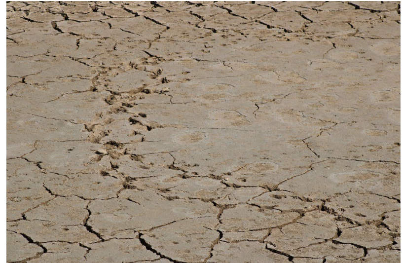
Photo 106: Northeast Sediment Basin: September 16, 2025
