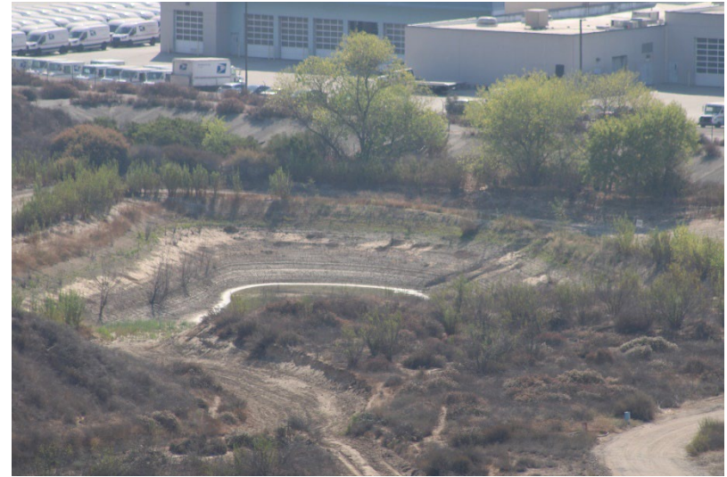
Photo 90: Northeast Sediment Basin: August 14, 2025
