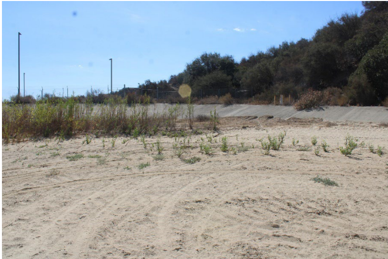
Photo 109: Northeast Sediment Basin: September 16, 2025
