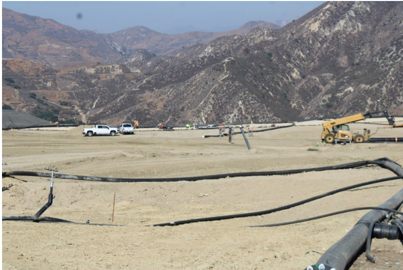
Photo 5: Top Deck Working Area: August 14, 2025
