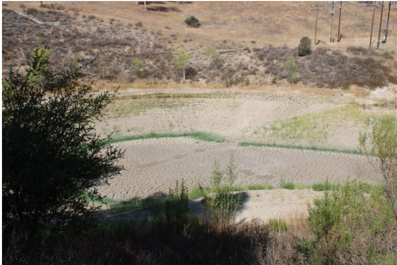
Photo 73: South Terminal and Catch Basins: August 14, 2025
