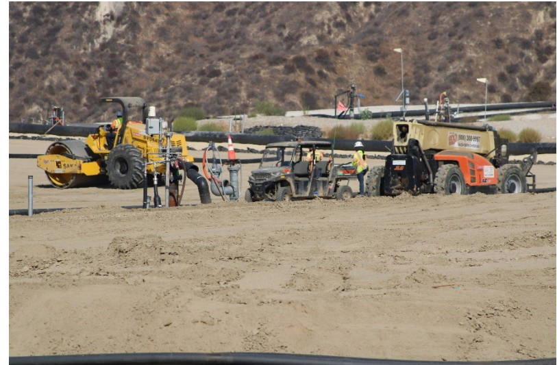
Photo 10: Top Deck Working Area: August 14, 2025
