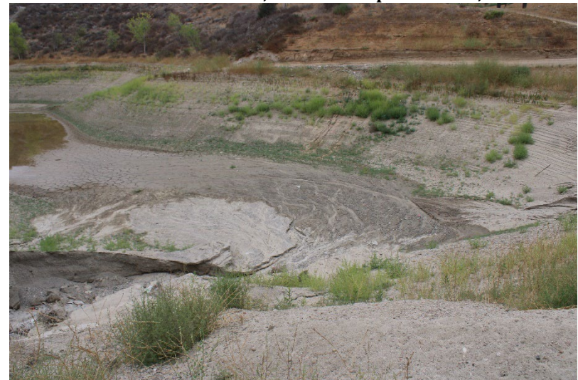
Photo 56: South Terminal and Catch Basins: July 22, 2025
