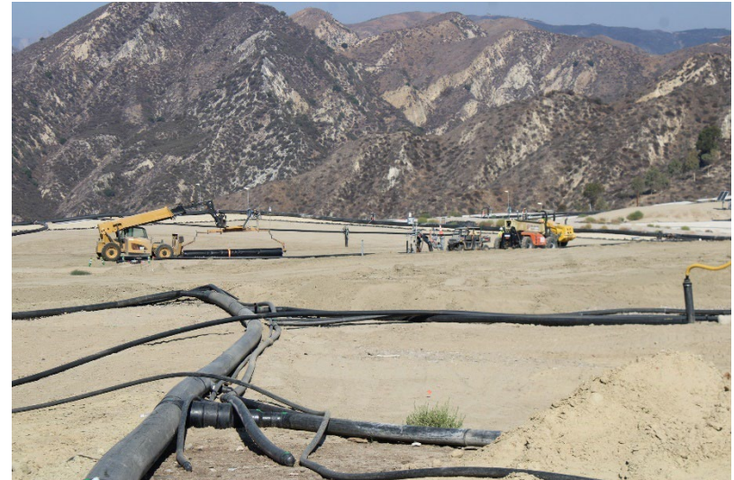
Photo 6: Top Deck Working Area: August 14, 2025
