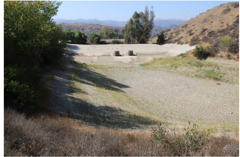
Photo 70: South Terminal and Catch Basins: August 14, 2025
