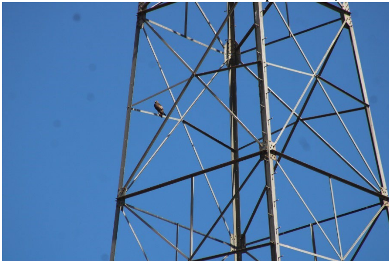
Photo 107: Northeast Sediment Basin: September 16, 2025
