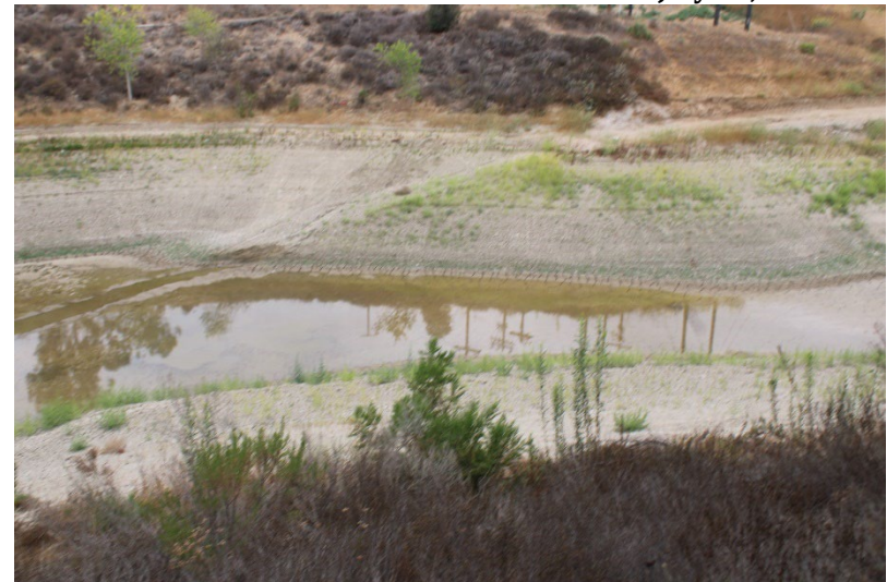
Photo 64: South Terminal and Catch Basins: July 22, 2025
