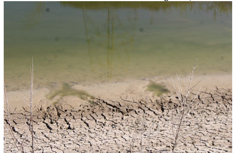
Photo 96: Northeast Sediment Basin: August 14, 2025
