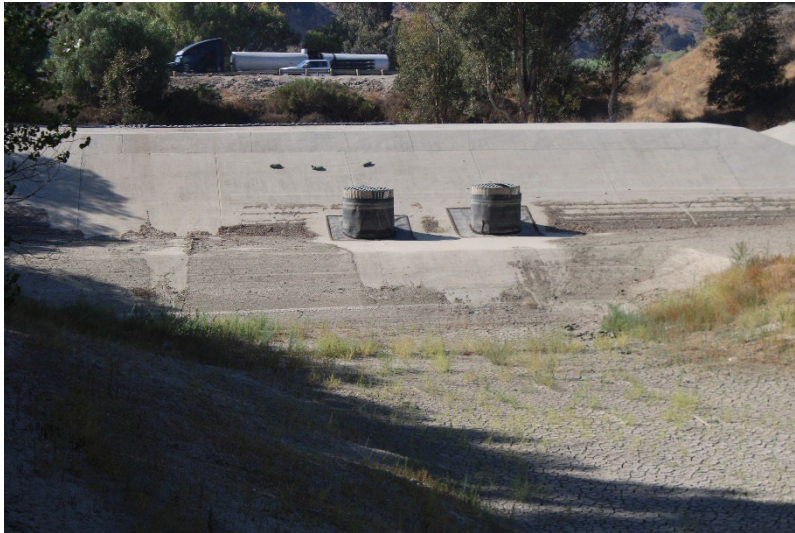
Photo 77: South Terminal and Catch Basins: September 16, 2025
