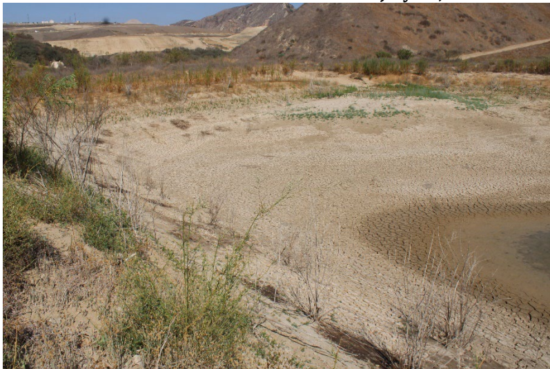
Photo 91: Northeast Sediment Basin: August 14, 2025
