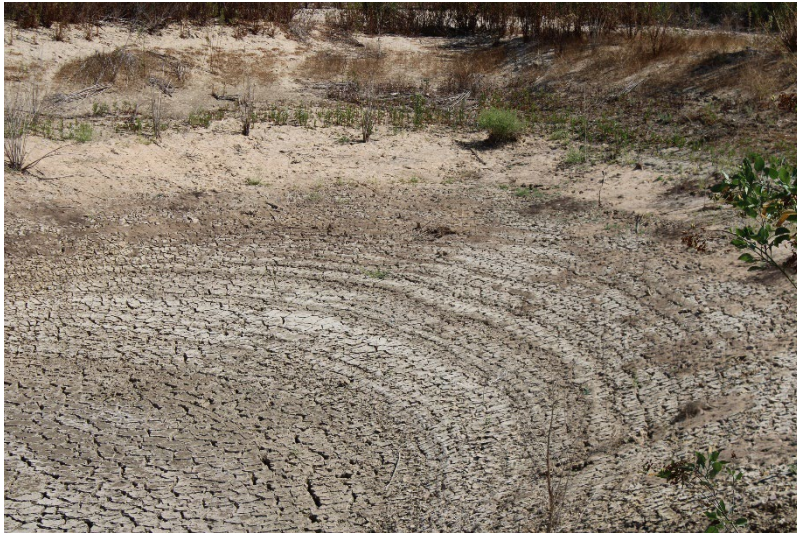
Photo 105: Northeast Sediment Basin: September 16, 2025
