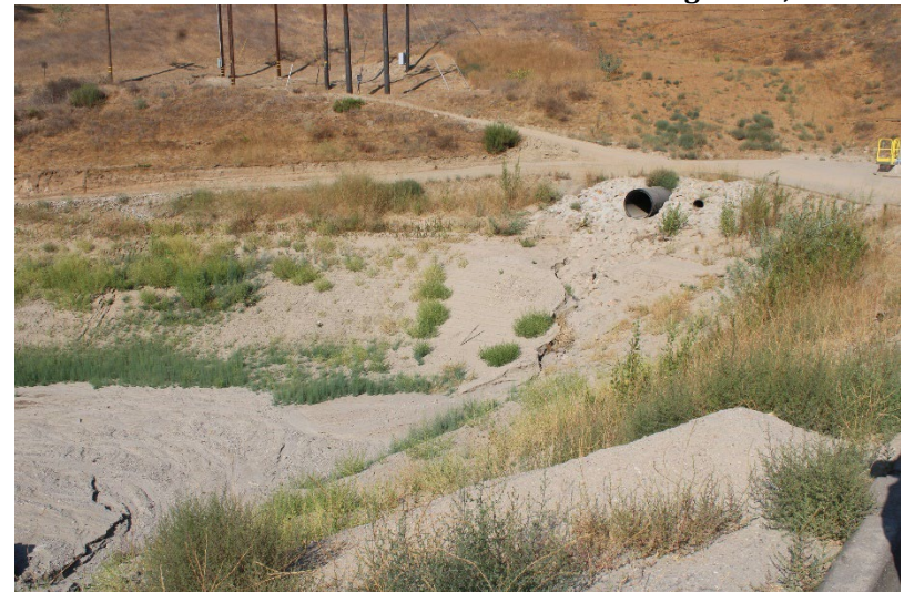
Photo 68: South Terminal and Catch Basins: August 14, 2025
