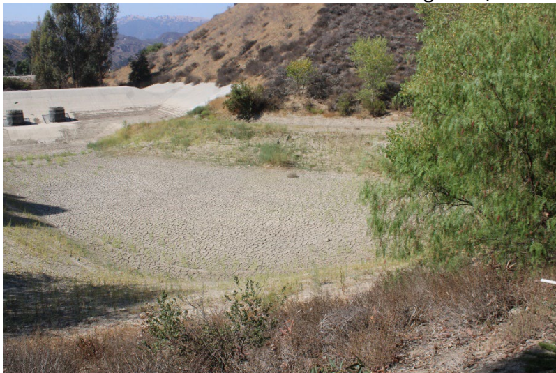
Photo 71: South Terminal and Catch Basins: August 14, 2025
