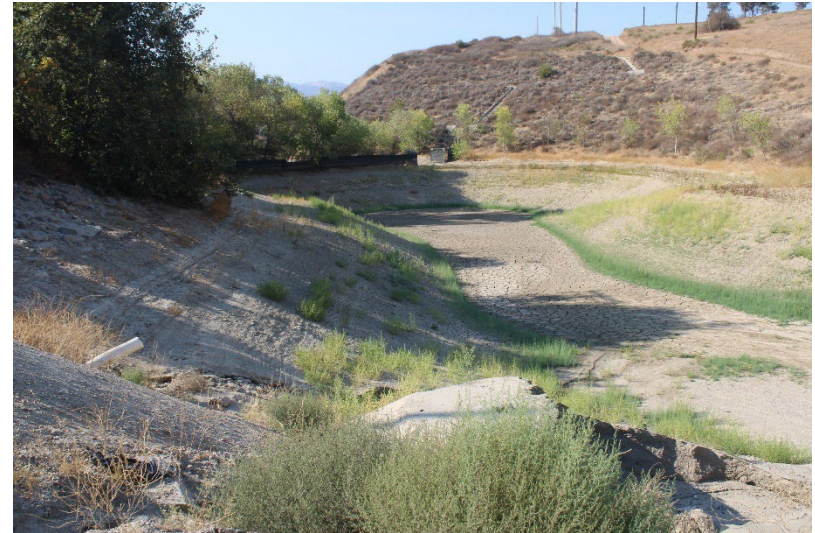
Photo 66: South Terminal and Catch Basins: August 14, 2025
