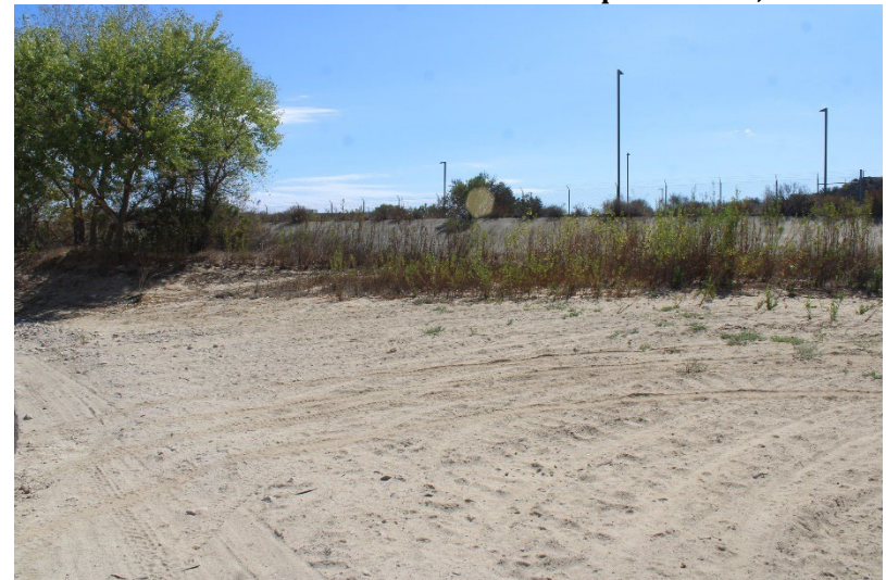
Photo 108: Northeast Sediment Basin: September 16, 2025
