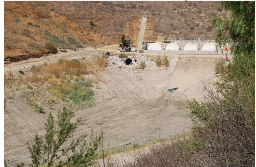
Photo 80: South Terminal and Catch Basins: September 16, 2025
