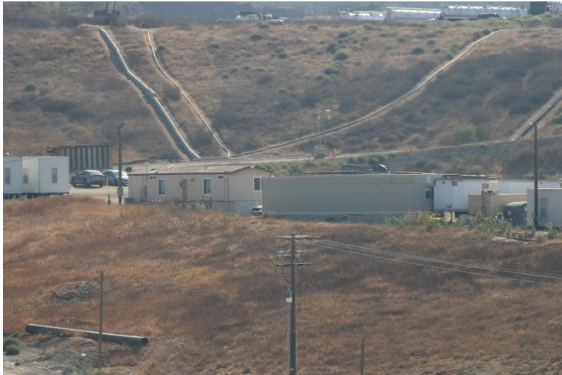
Photo 145: Maintenance and Admin Buildings: August 14, 2025
