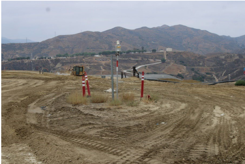
Photo 1: Top Deck Working Area: July 22, 2025
