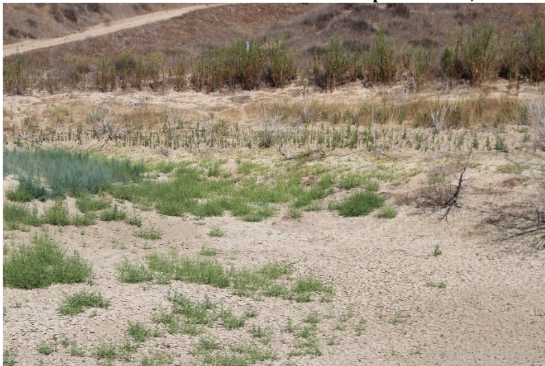
Photo 103: Northeast Sediment Basin: September 16, 2025
