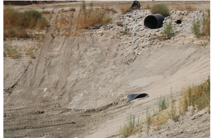
Photo 84: South Terminal and Catch Basins: September 16, 2025
