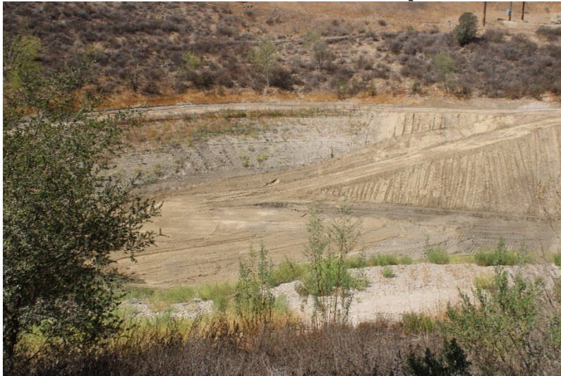
Photo 79: South Terminal and Catch Basins: September 16, 2025
