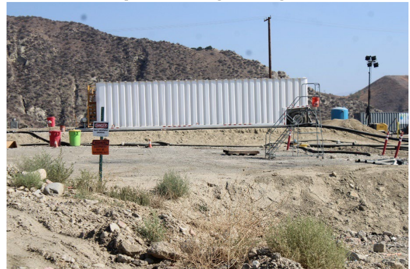
Photo 4: Top Deck Working Area: August 14, 2025
