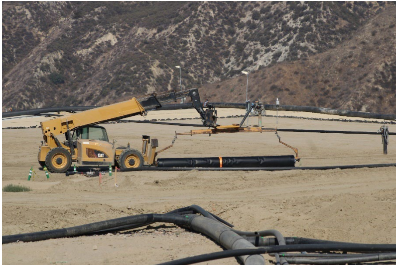
Photo 9: Top Deck Working Area: August 14, 2025
