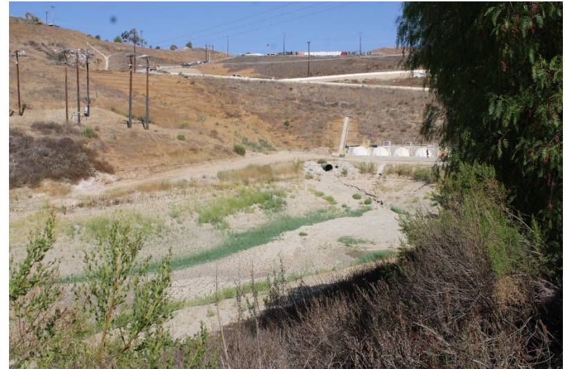
Photo 74: South Terminal and Catch Basins: August 14, 2025
