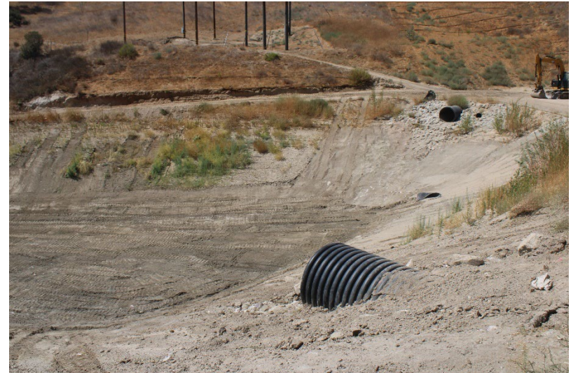
Photo 82: South Terminal and Catch Basins: September 16, 2025
