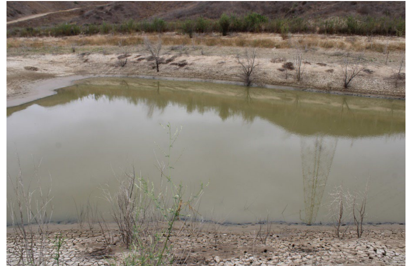
Photo 86: Northeast Sediment Basin: July 22, 2025
