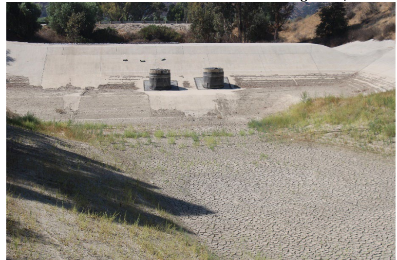
Photo 72: South Terminal and Catch Basins: August 14, 2025
