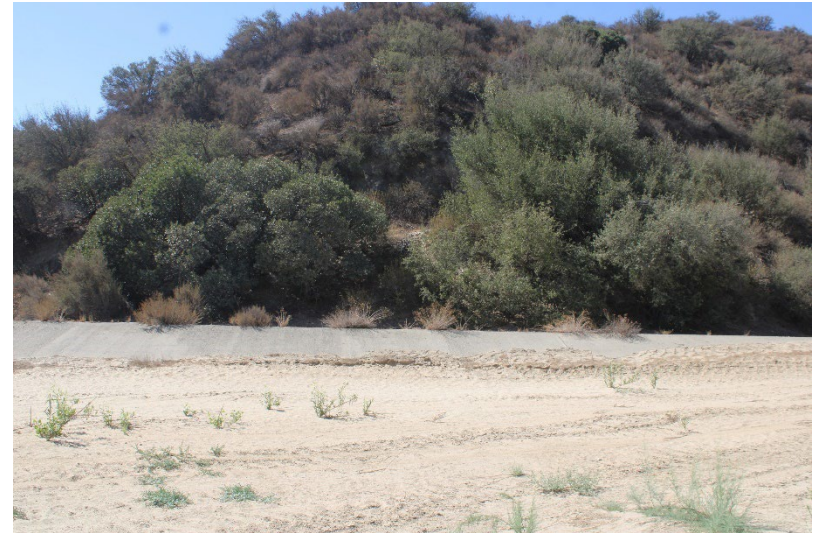
Photo 110: Northeast Sediment Basin: September 16, 2025
