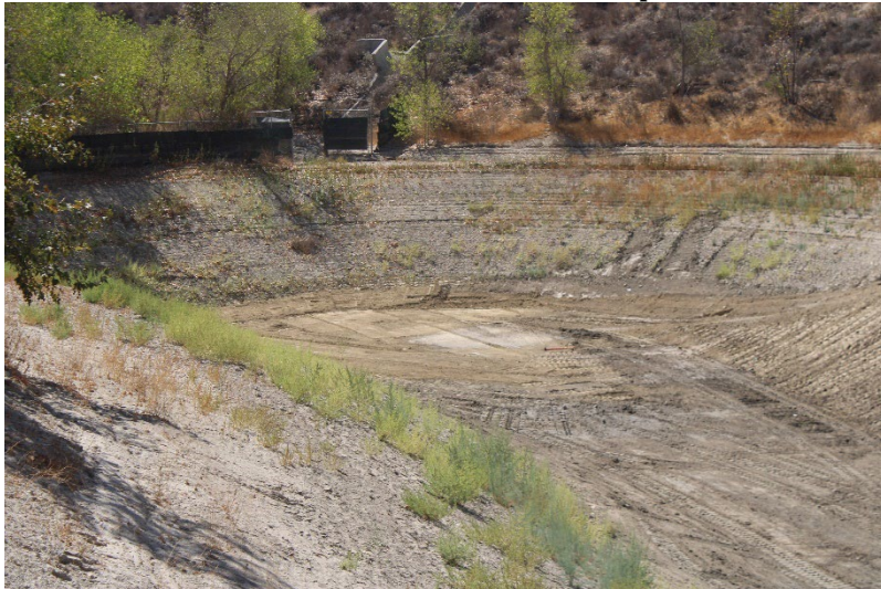
Photo 83: South Terminal and Catch Basins: September 16, 2025
