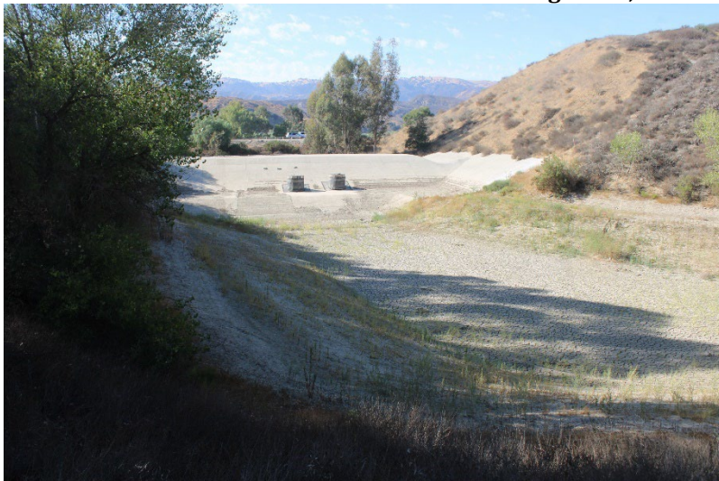
Photo 75: South Terminal and Catch Basins: September 16, 2025
