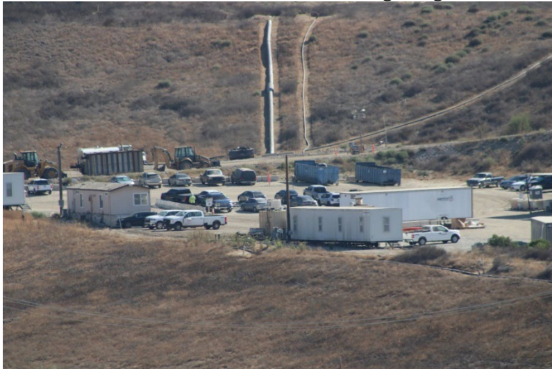
Photo 147: Maintenance and Admin Buildings: September 16, 2025
