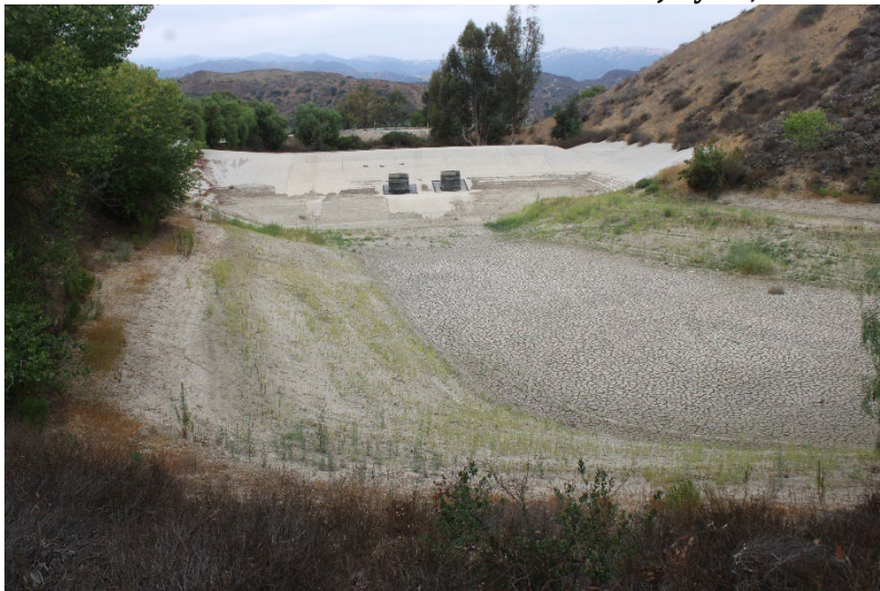
Photo 59: South Terminal and Catch Basins: July 22, 2025
