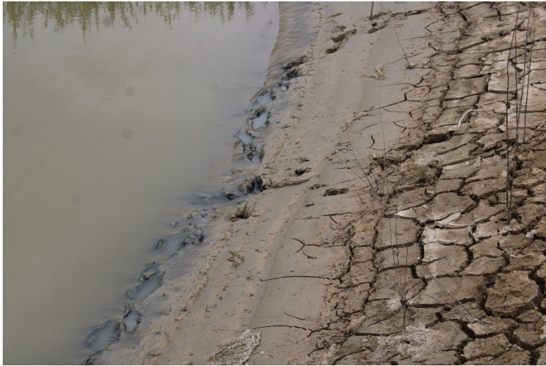
Photo 89: Northeast Sediment Basin: July 22, 2025
