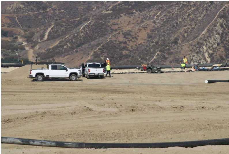
Photo 7: Top Deck Working Area: August 14, 2025
