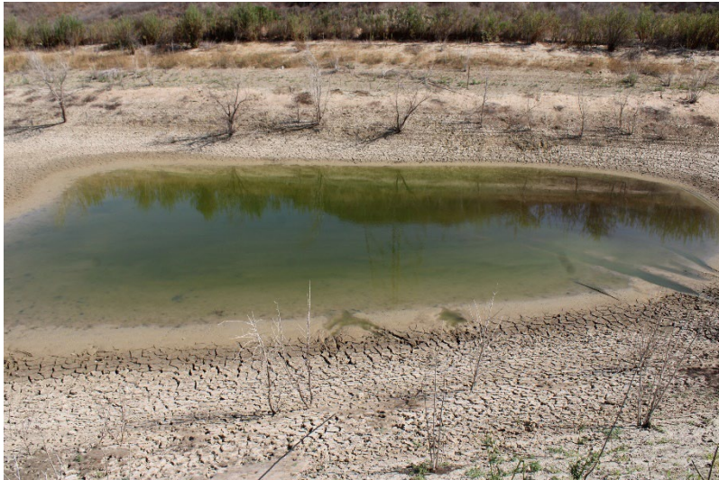
Photo 93: Northeast Sediment Basin: August 14, 2025
