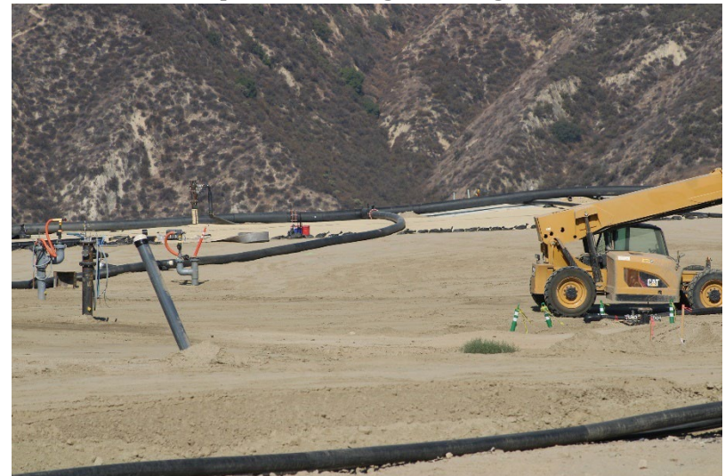
Photo 8: Top Deck Working Area: August 14, 2025
