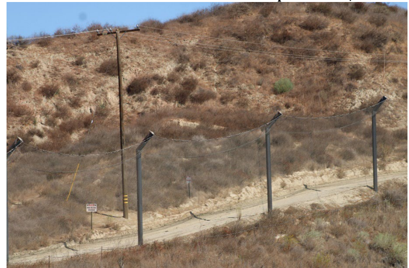
Photo 112: Westside Perimeter Ridge: September 16, 2025
