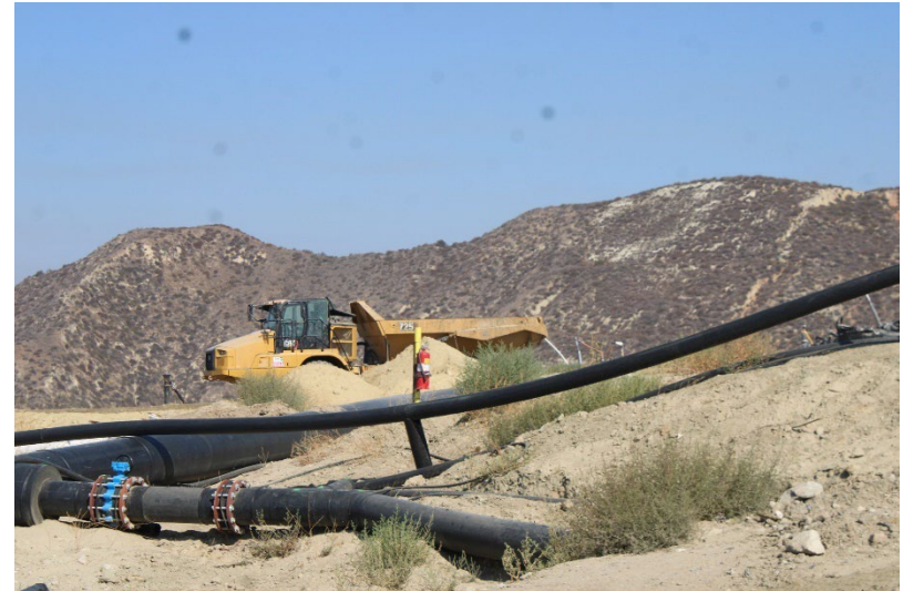
Photo 2: Top Deck Working Area: August 14, 2025
