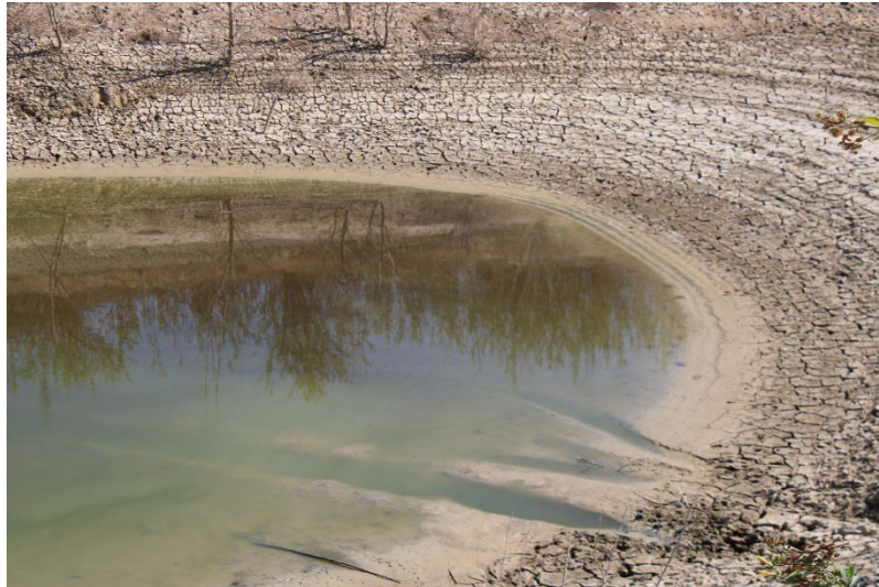
Photo 97: Northeast Sediment Basin: August 14, 2025
