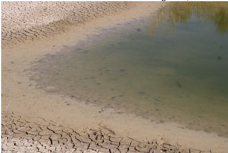
Photo 95: Northeast Sediment Basin: August 14, 2025
