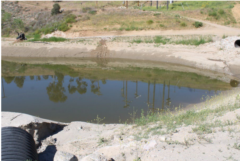
Photo 45: South Terminal and Catch Basins: May 15, 2025
