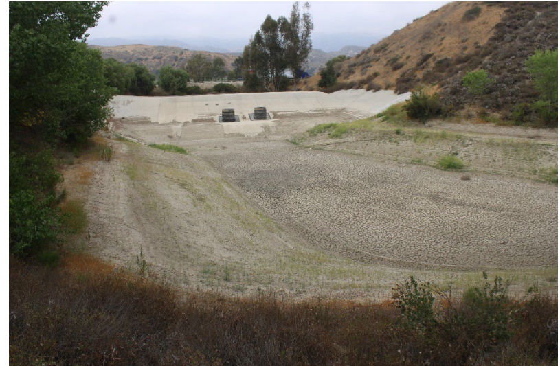
Photo 58: South Terminal and Catch Basins: June 24, 2025
