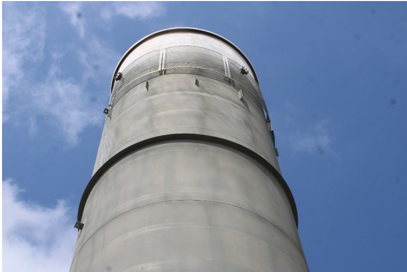
Photo 105: Flare 100, Flare 150 and Flare 250: June 24, 2025
