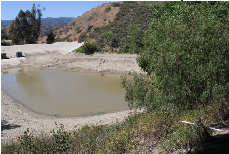
Photo 47: South Terminal and Catch Basins: May 15, 2025
