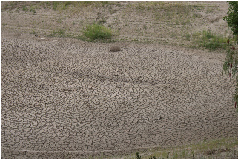
Photo 61: South Terminal and Catch Basins: June 24, 2025
