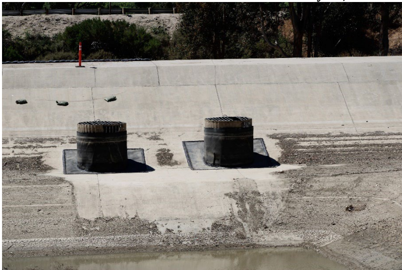
Photo 51: South Terminal and Catch Basins: May 15, 2025
