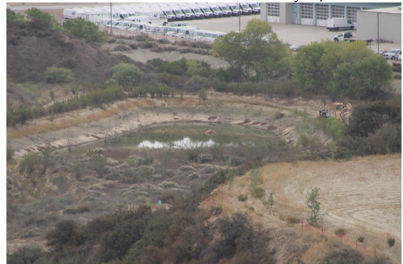
Photo 72: Northeast Sediment Basin: June 24, 2025
