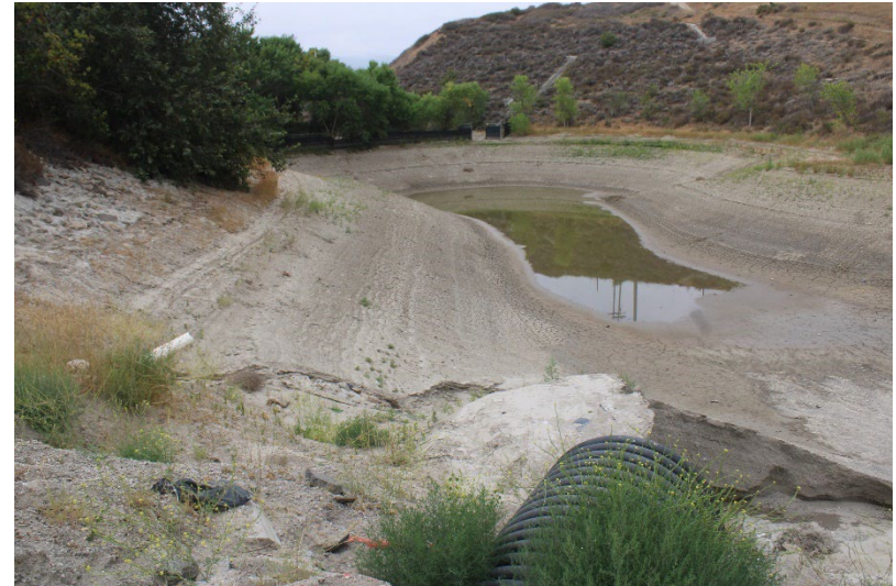
Photo 66: South Terminal and Catch Basins: June 24, 2025
