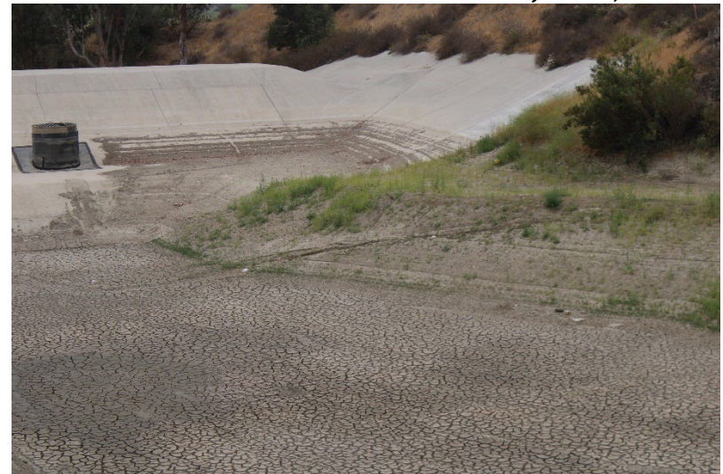
Photo 60: South Terminal and Catch Basins: June 24, 2025
