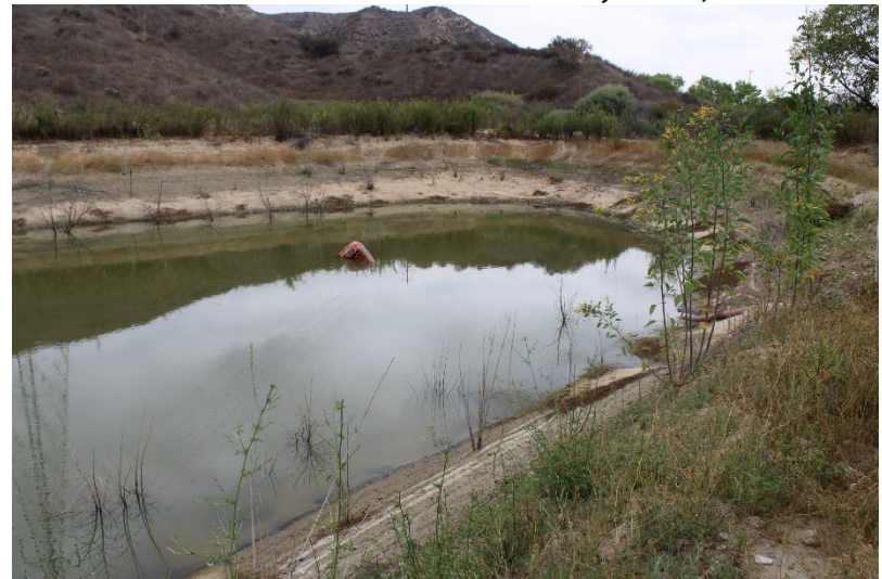
Photo 76: Northeast Sediment Basin: June 24, 2025
