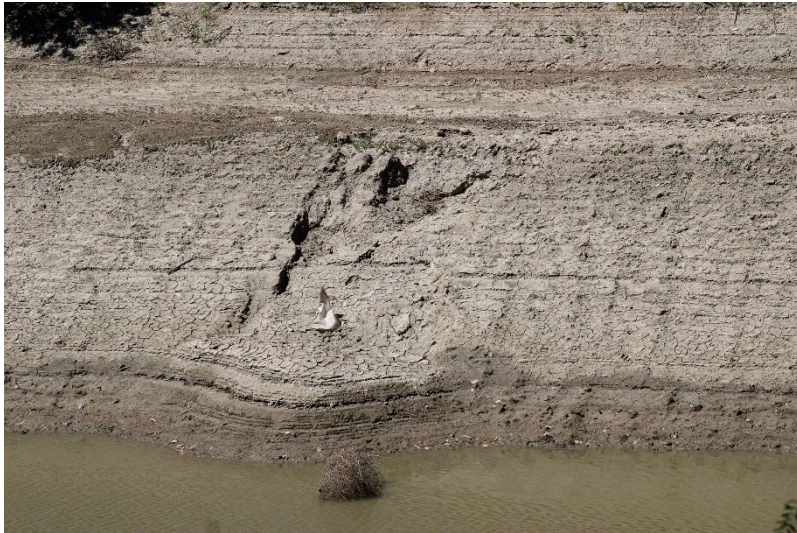
Photo 53: South Terminal and Catch Basins: May 15, 2025
