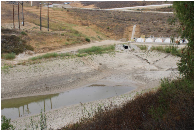
Photo 63: South Terminal and Catch Basins: June 24, 2025
