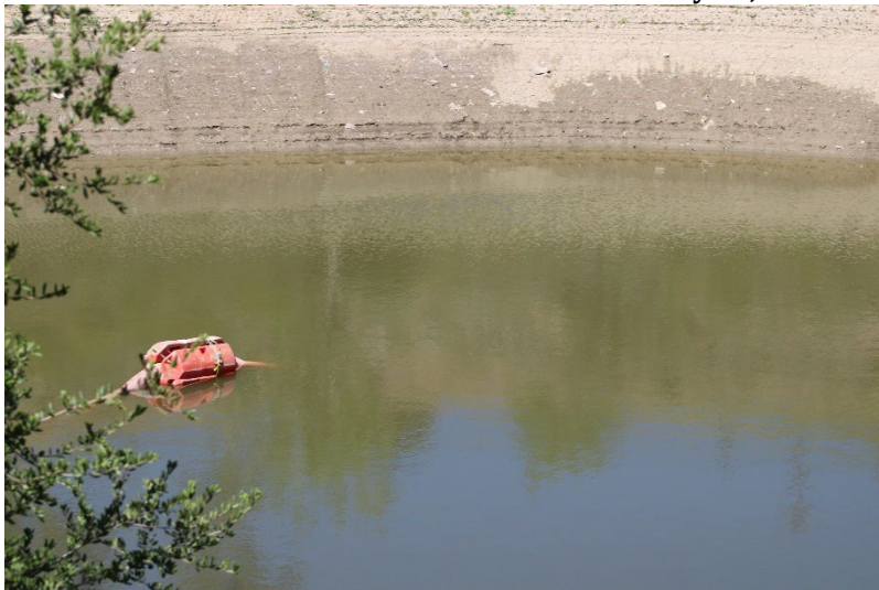
Photo 55: South Terminal and Catch Basins: May 15, 2025
