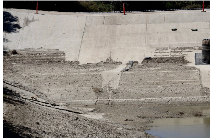
Photo 50: South Terminal and Catch Basins: May 15, 2025
