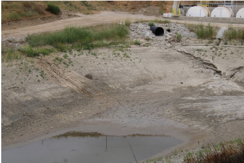
Photo 65: South Terminal and Catch Basins: June 24, 2025
