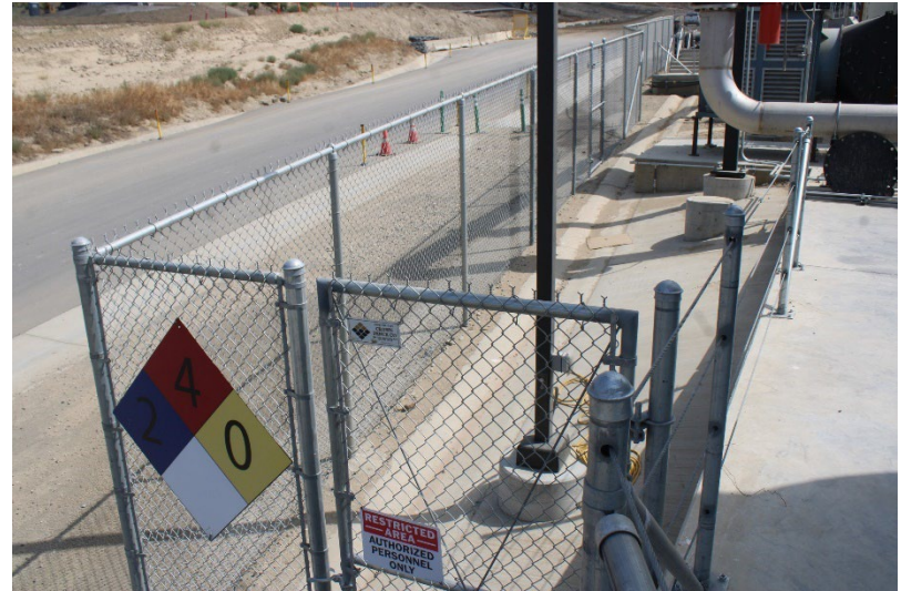
Photo 106: Flare 100, Flare 150 and Flare 250: June 24, 2025
