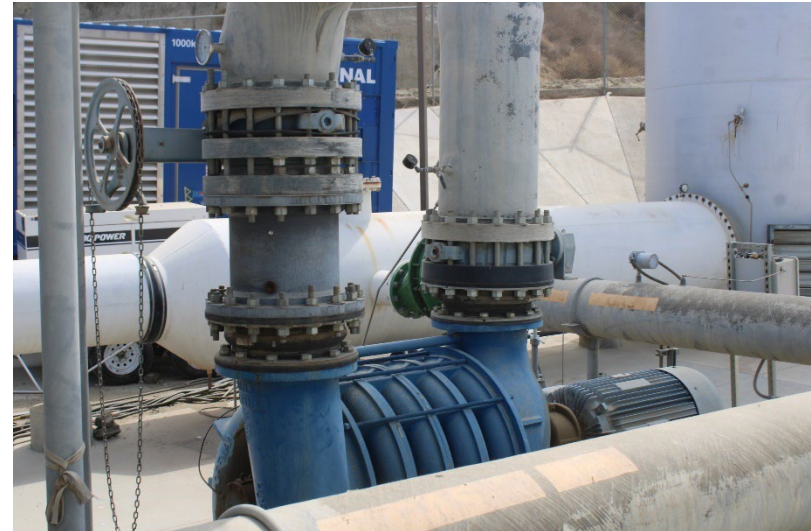
Photo 102: Flare 100, Flare 150 and Flare 250: June 24, 2025
