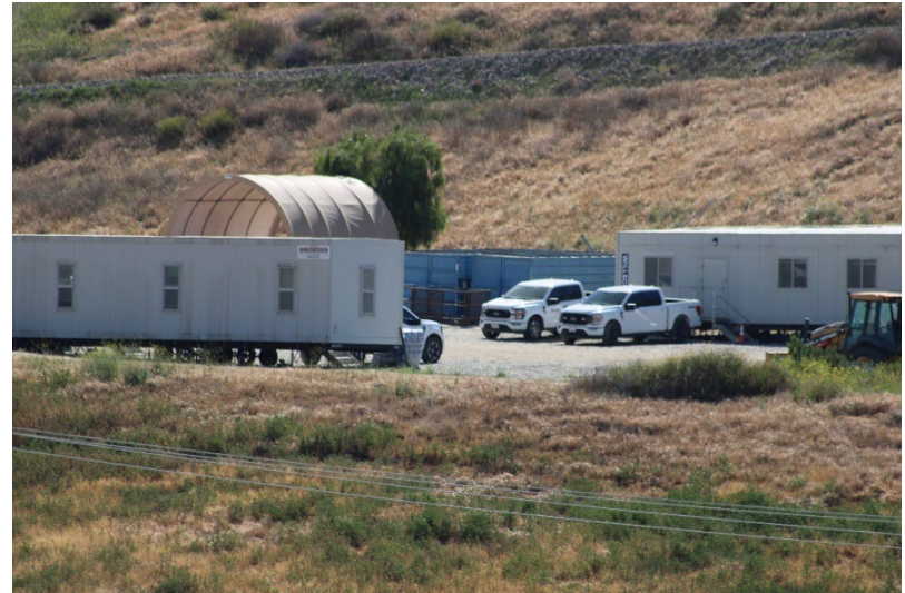
Photo 110: Maintenance and Admin Buildings: May 15, 2025
