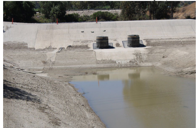
Photo 48: South Terminal and Catch Basins: May 15, 2025
