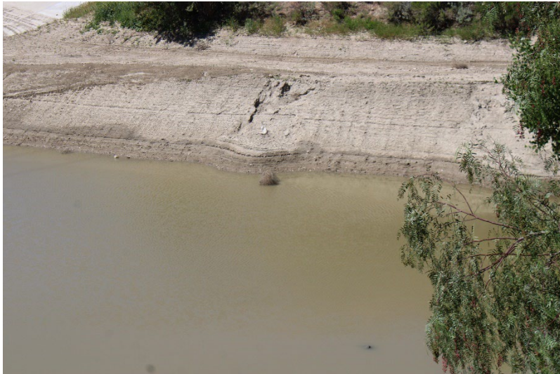
Photo 49: South Terminal and Catch Basins: May 15, 2025
