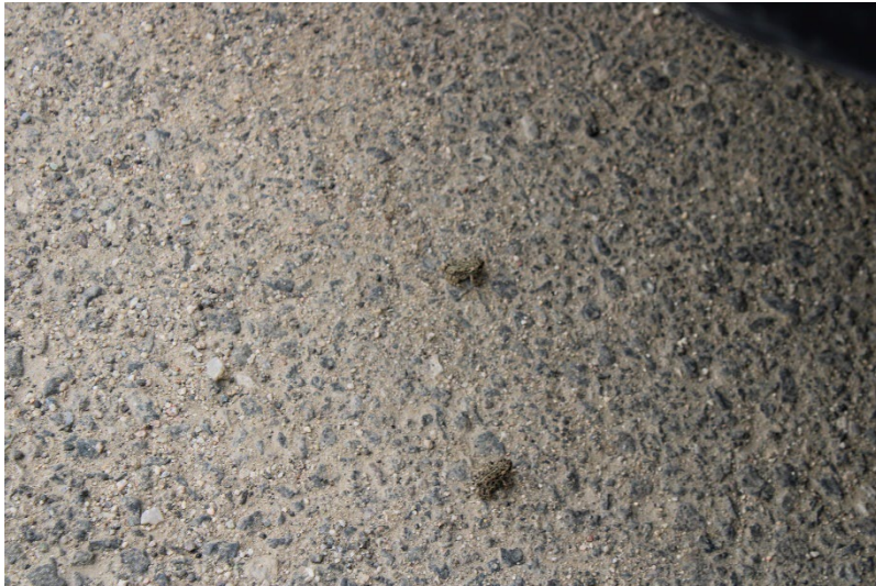
Photo 73: Northeast Sediment Basin: June 24, 2025
