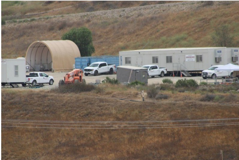
Photo 113: Maintenance and Admin Buildings: June 24, 2025
