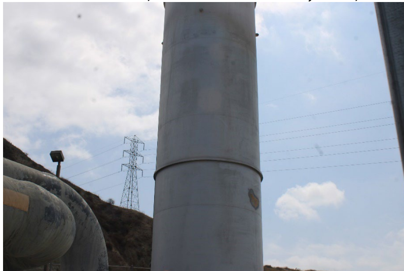
Photo 103: Flare 100, Flare 150 and Flare 250: June 24, 2025
