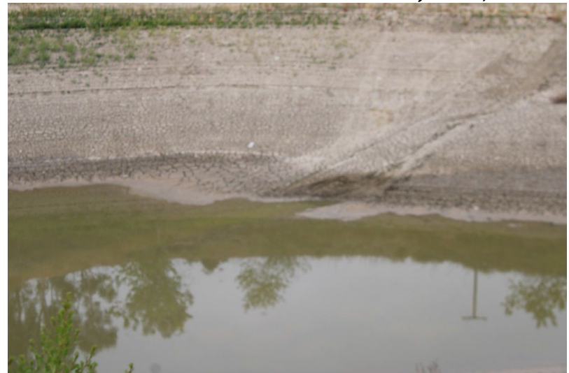
Photo 64: South Terminal and Catch Basins: June 24, 2025
