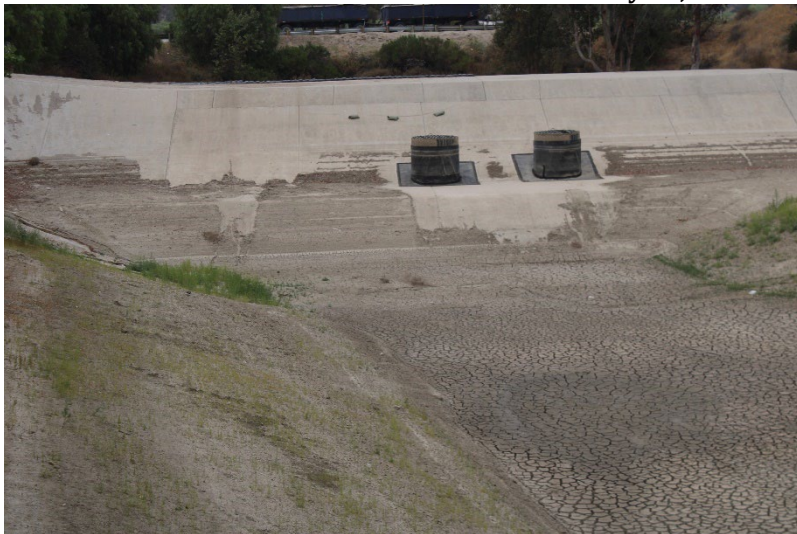
Photo 59: South Terminal and Catch Basins: June 24, 2025
