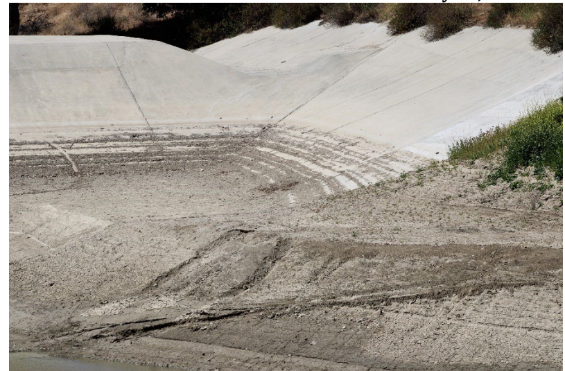
Photo 52: South Terminal and Catch Basins: May 15, 2025
