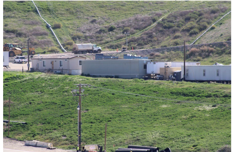
Photo 108: Maintenance and Admin Buildings: April 10, 2025
