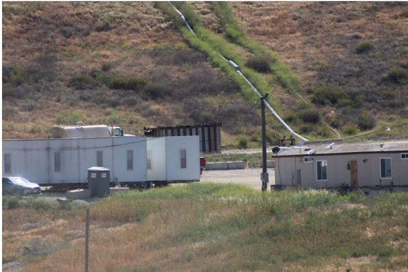
Photo 109: Maintenance and Admin Buildings: May 15, 2025
