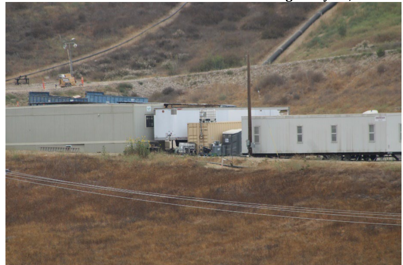
Photo 112: Maintenance and Admin Buildings: June 24, 2025
