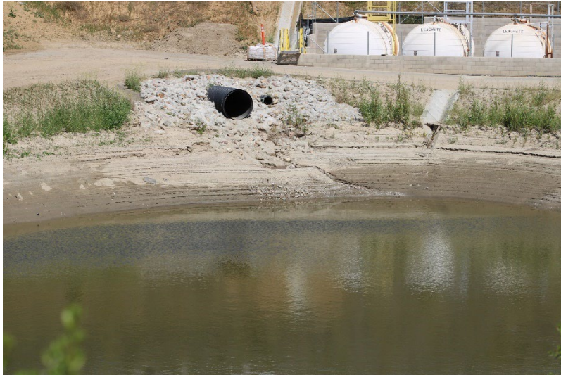
Photo 57: South Terminal and Catch Basins: May 15, 2025
