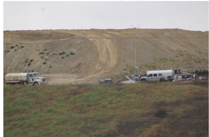
Photo 4: Closed Landfill – Primary Canyon: June 24, 2025
