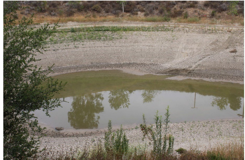
Photo 62: South Terminal and Catch Basins: June 24, 2025
