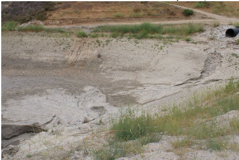
Photo 67: South Terminal and Catch Basins: June 24, 2025
