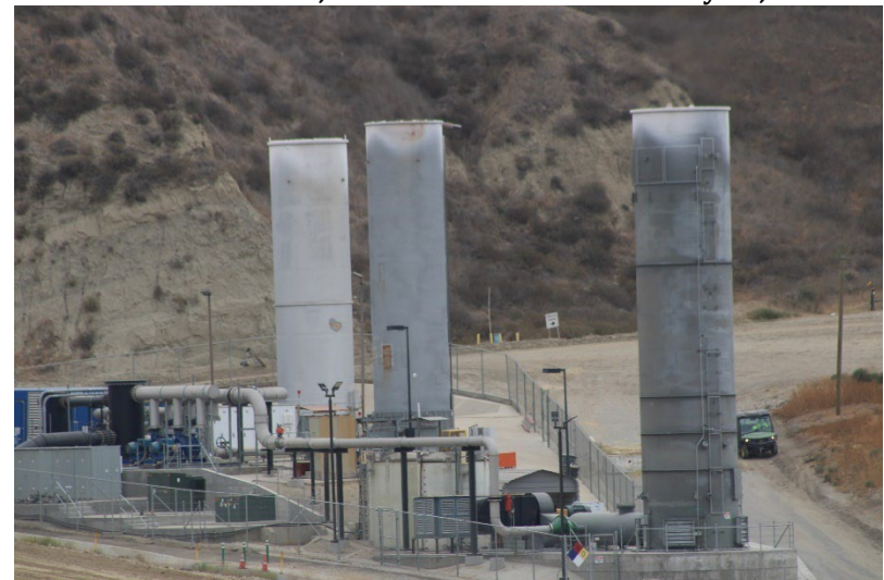
Photo 100: Flare 100, Flare 150 and Flare 250: June 24, 2025
