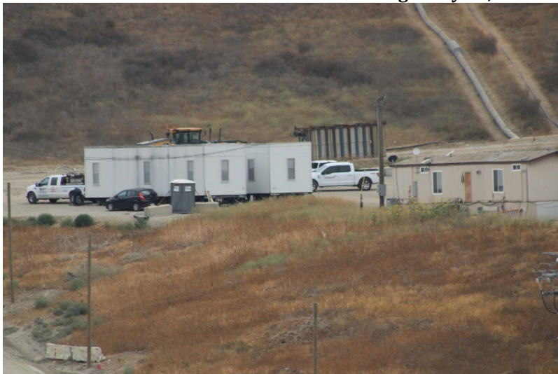
Photo 111: Maintenance and Admin Buildings: June 24, 2025
