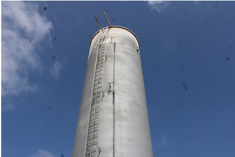
Photo 107: Flare 100, Flare 150 and Flare 250: June 24, 2025
