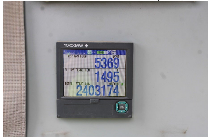
Photo 104: Flare 100, Flare 150 and Flare 250: June 24, 2025
