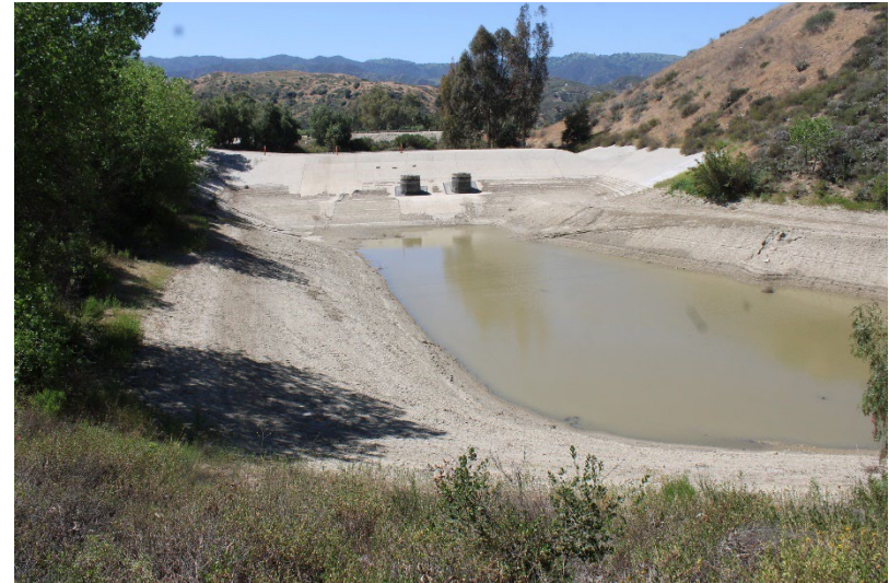
Photo 46: South Terminal and Catch Basins: May 15, 2025
