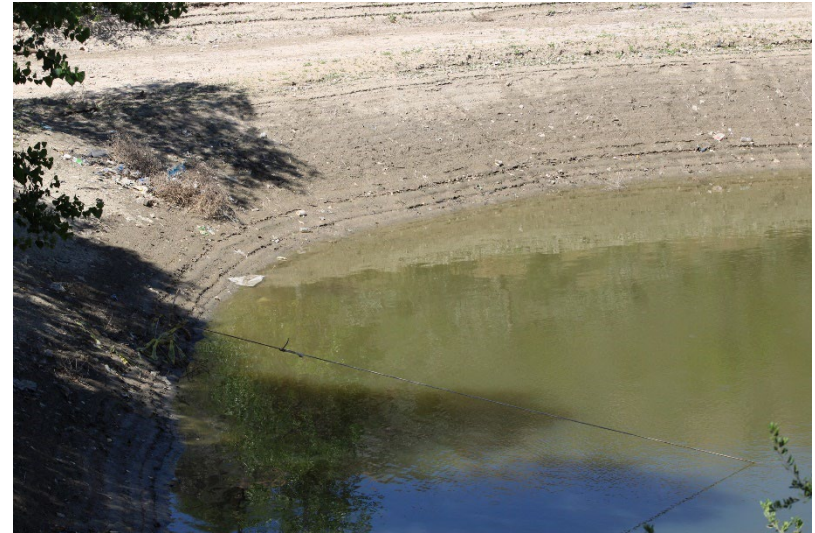
Photo 54: South Terminal and Catch Basins: May 15, 2025
