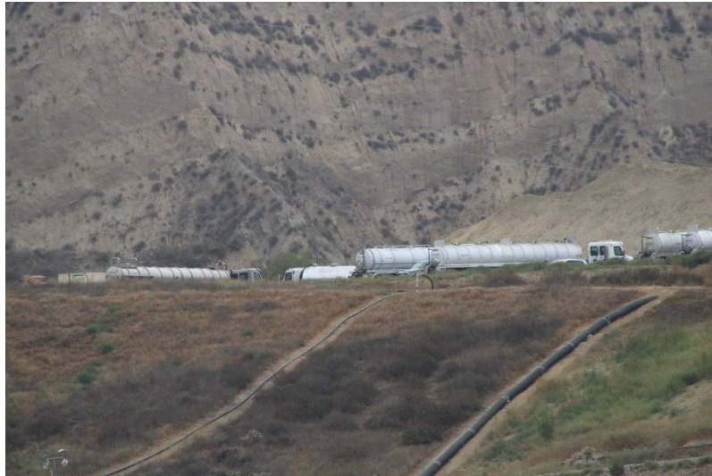
Photo 1: Closed Landfill – Primary Canyon: June 24, 2025
