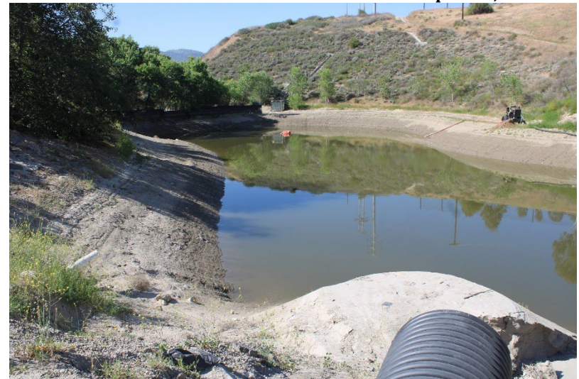
Photo 44: South Terminal and Catch Basins: May 15, 2025
