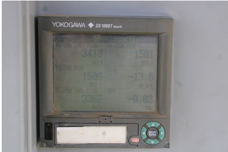
Photo 101: Flare 100, Flare 150 and Flare 250: June 24, 2025
