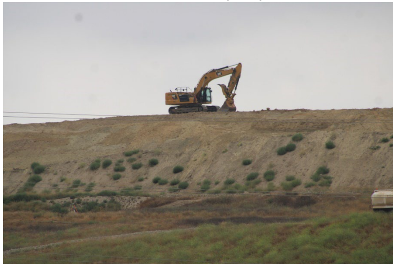
Photo 3: Closed Landfill – Primary Canyon: June 24, 2025
