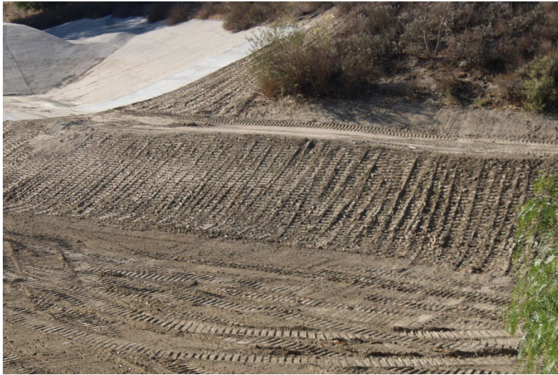
Photo 57: South Terminal and Catch Basins: January 16, 2025
