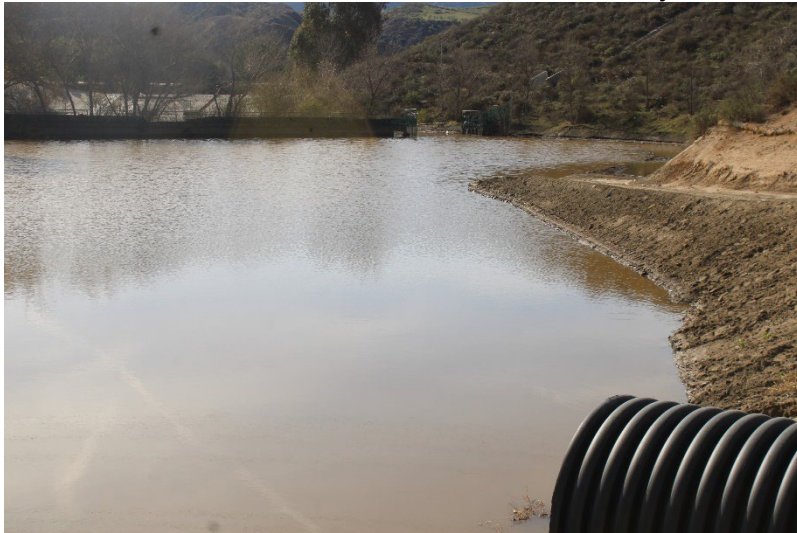
Photo 63: South Terminal and Catch Basins: February 18, 2025
