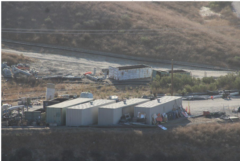
Photo 7: Closed Landfill – Primary Canyon: January 16, 2025
