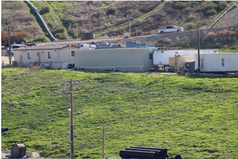
Photo 135: Maintenance and Admin Buildings: March 20, 2025
