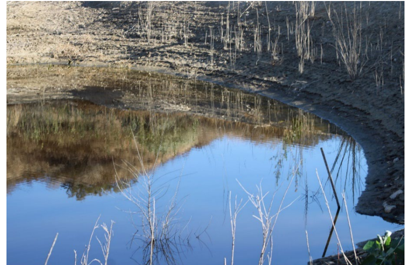
Photo 90: Northeast Sediment Basin: January 16, 2025
