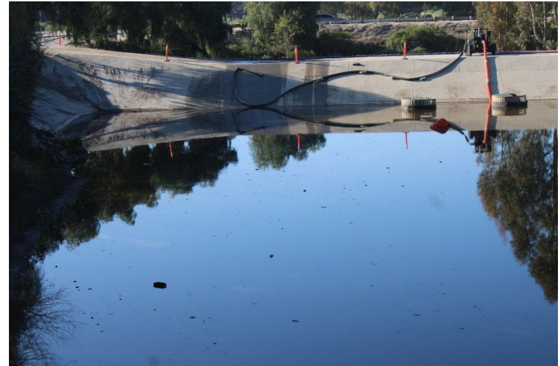
Photo 74: South Terminal and Catch Basins: March 20, 2025
