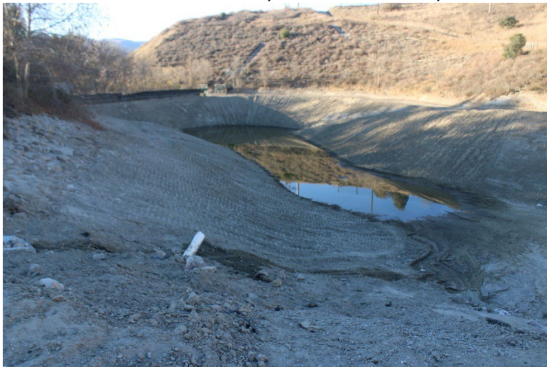
Photo 51: South Terminal and Catch Basins: January 16, 2025
