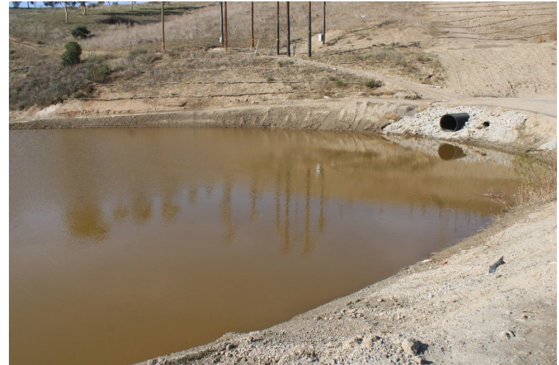
Photo 62: South Terminal and Catch Basins: February 18, 2025
