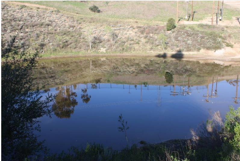
Photo 81: South Terminal and Catch Basins: March 20, 2025
