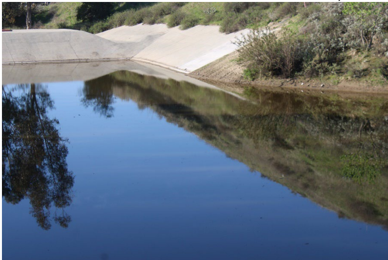
Photo 75: South Terminal and Catch Basins: March 20, 2025
