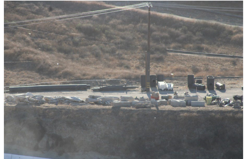
Photo 6: Closed Landfill – Primary Canyon: January 16, 2025
