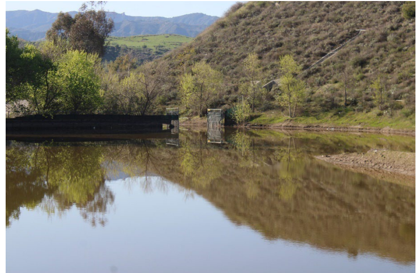
Photo 86: South Terminal and Catch Basins: March 20, 2025
