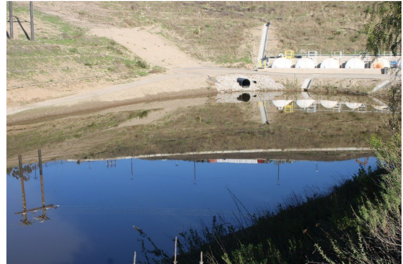
Photo 82: South Terminal and Catch Basins: March 20, 2025
