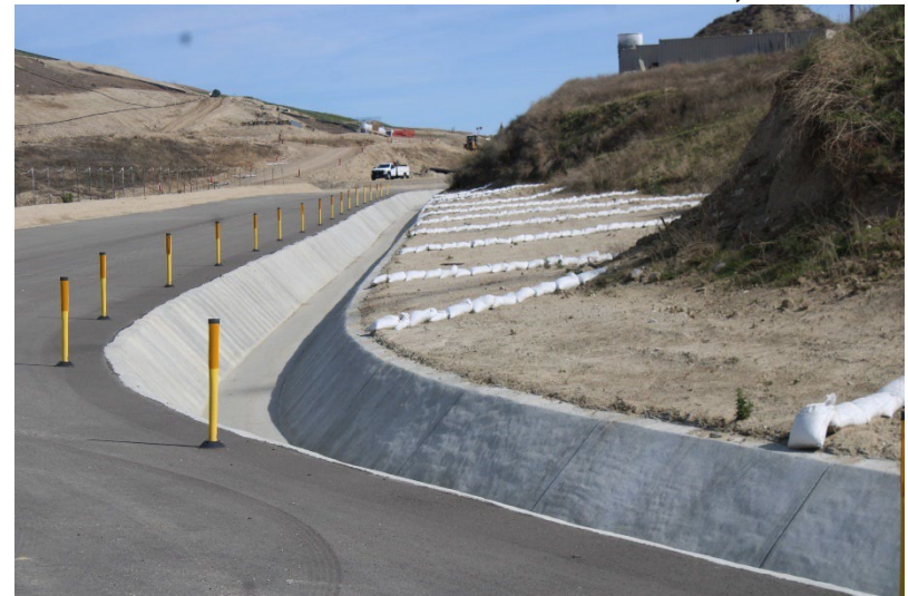
Photo 96: Landfill Perimeter Drainage Channel: February 18, 2025
