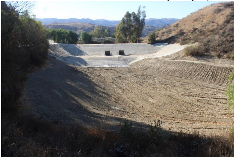
Photo 55: South Terminal and Catch Basins: January 16, 2025
