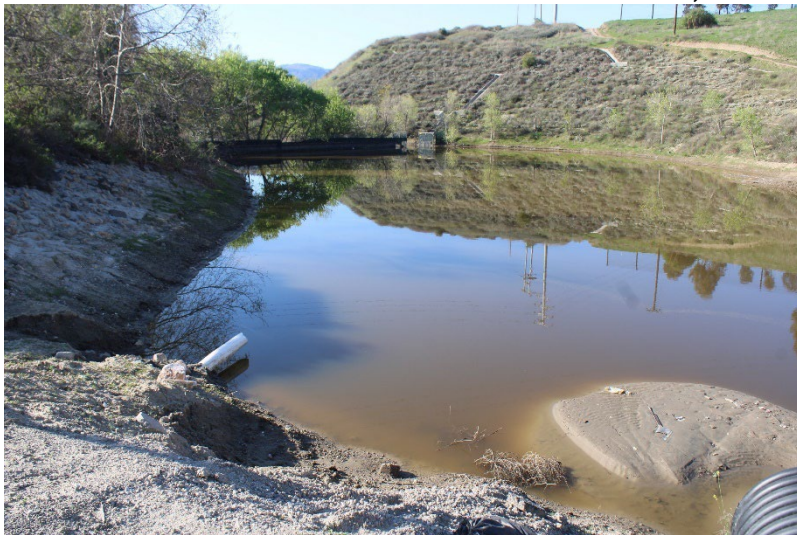
Photo 83: South Terminal and Catch Basins: March 20, 2025
