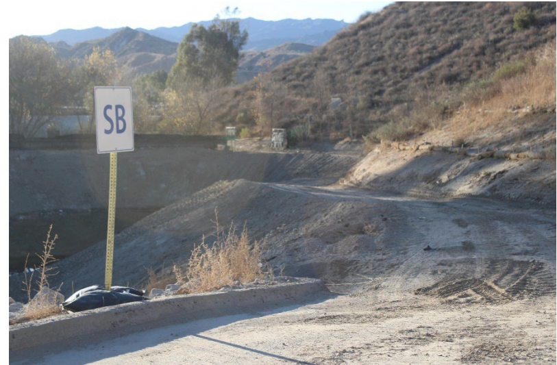
Photo 54: South Terminal and Catch Basins: January 16, 2025
