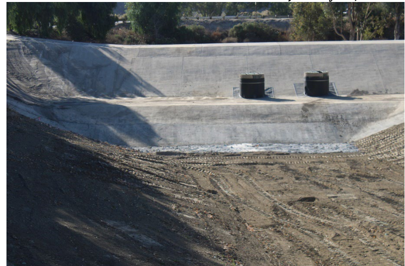
Photo 56: South Terminal and Catch Basins: January 16, 2025
