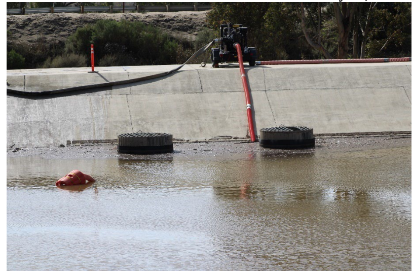
Photo 68: South Terminal and Catch Basins: February 18, 2025
