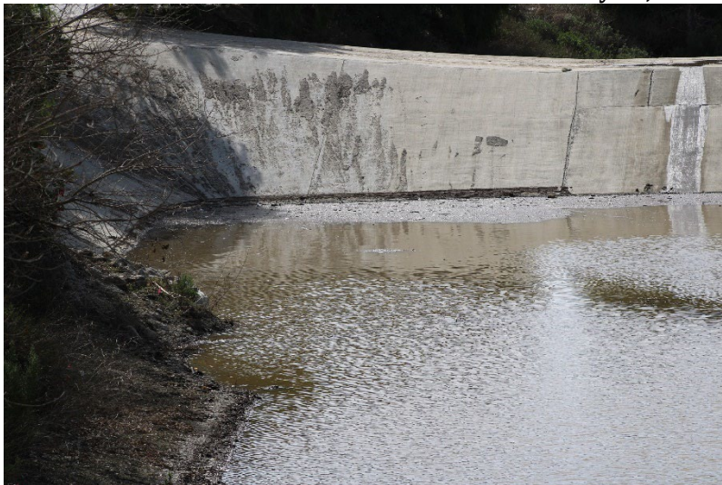
Photo 67: South Terminal and Catch Basins: February 18, 2025
