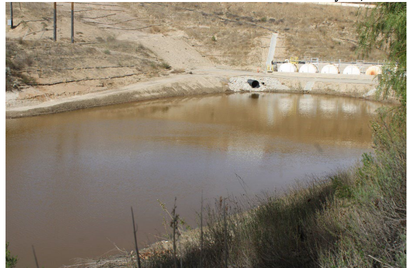
Photo 72: South Terminal and Catch Basins: February 18, 2025
