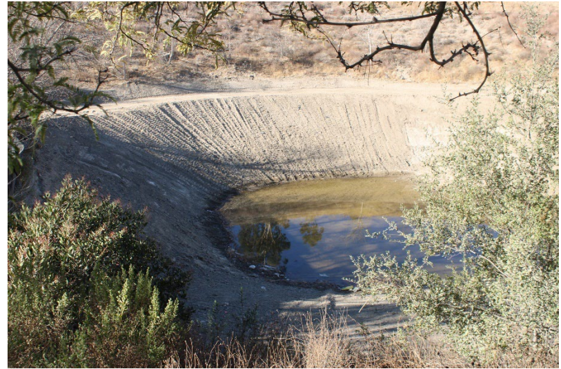
Photo 58: South Terminal and Catch Basins: January 16, 2025
