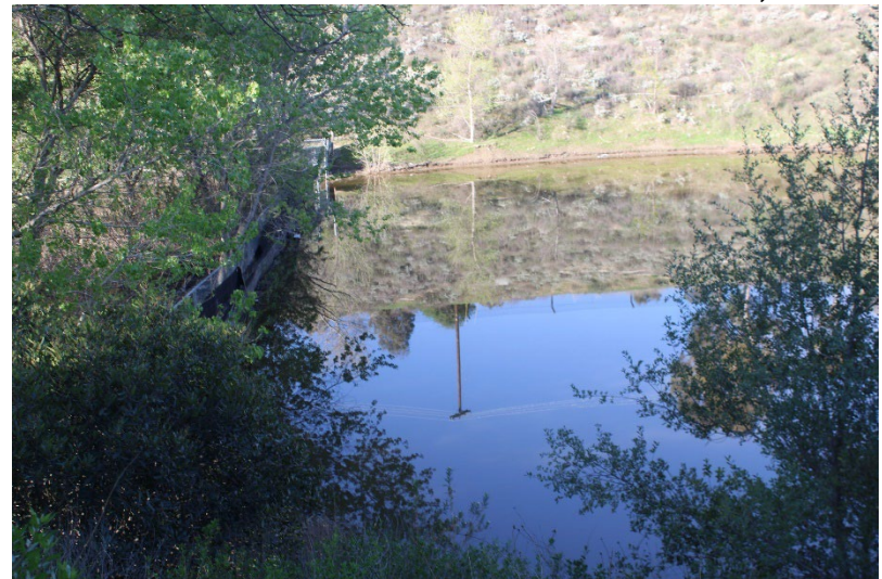
Photo 80: South Terminal and Catch Basins: March 20, 2025
