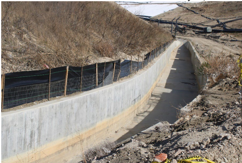
Photo 95: Landfill Perimeter Drainage Channel: February 18, 2025
