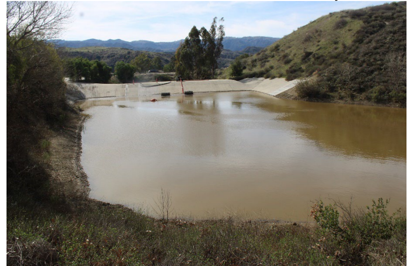
Photo 64: South Terminal and Catch Basins: February 18, 2025
