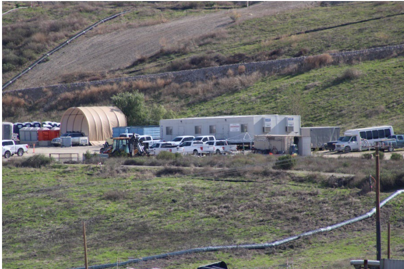
Photo 133: Maintenance and Admin Buildings: February 18, 2025
