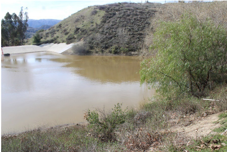
Photo 65: South Terminal and Catch Basins: February 18, 2025
