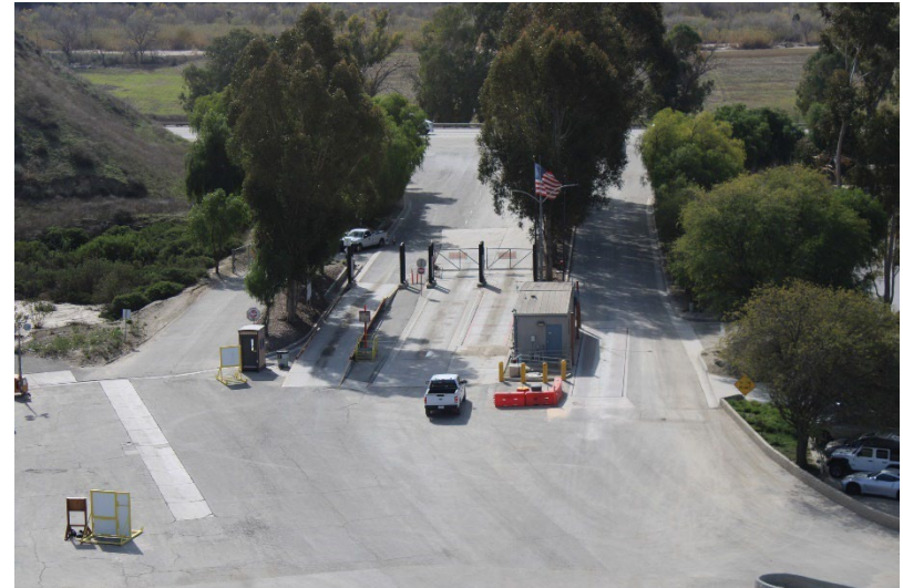
Photo 134: Maintenance and Admin Buildings: February 18, 2025
