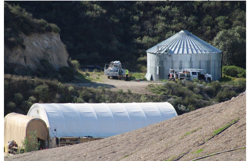
Photo 136: Maintenance and Admin Buildings: March 20, 2025
