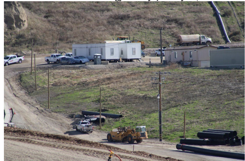
Photo 132: Maintenance and Admin Buildings: February 18, 2025
