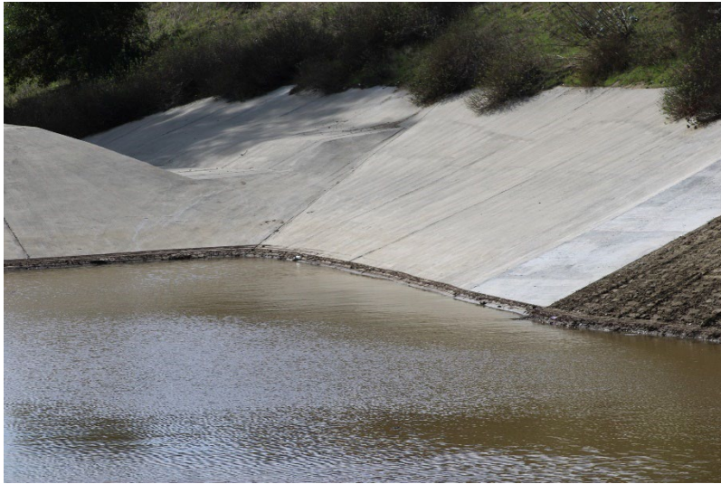
Photo 69: South Terminal and Catch Basins: February 18, 2025
