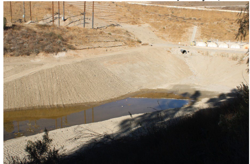
Photo 60: South Terminal and Catch Basins: January 16, 2025
