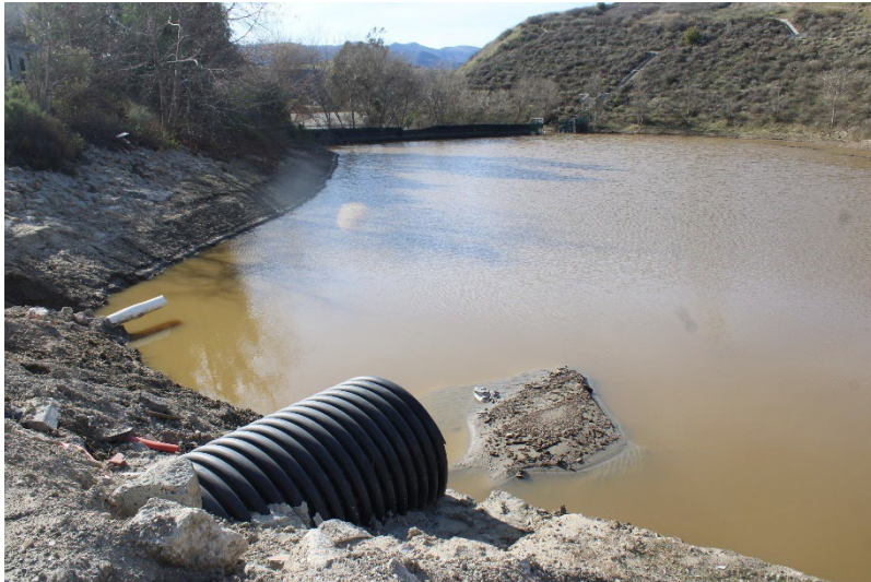
Photo 61: South Terminal and Catch Basins: February 18, 2025
