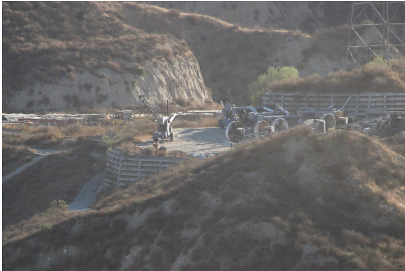
Photo 1: Closed Landfill - Primary Canyon: January 16, 2025
