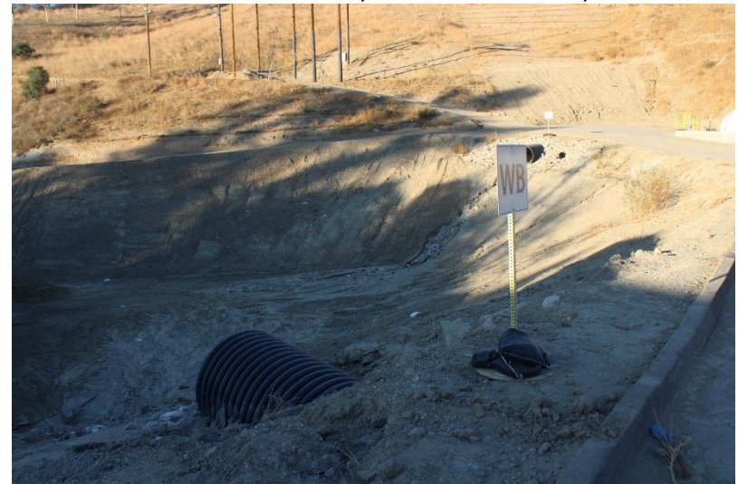
Photo 52: South Terminal and Catch Basins: January 16, 2025
