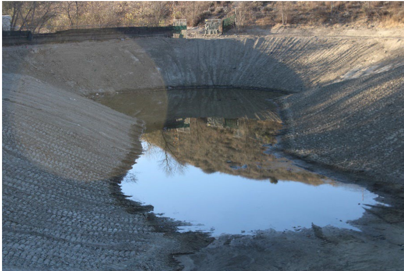
Photo 53: South Terminal and Catch Basins: January 16, 2025
