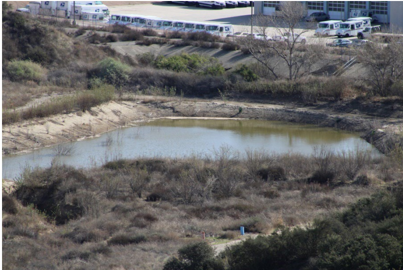
Photo 93: Northeast Sediment Basin: February 18, 2025
