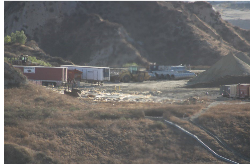
Photo 2: Closed Landfill - Primary Canyon: January 16, 2025
