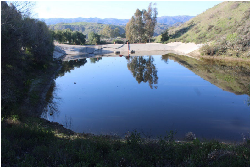
Photo 73: South Terminal and Catch Basins: March 20, 2025
