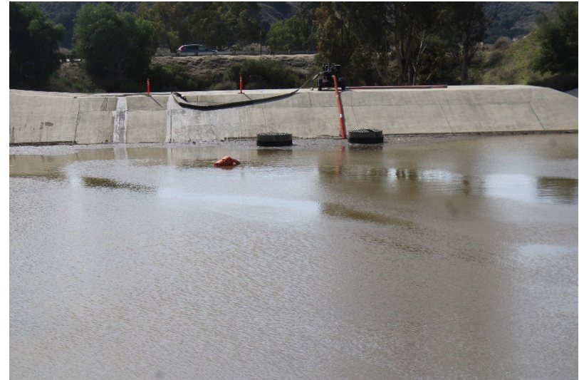
Photo 66: South Terminal and Catch Basins: February 18, 2025
