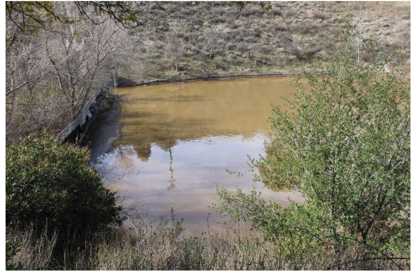
Photo 70: South Terminal and Catch Basins: February 18, 2025
