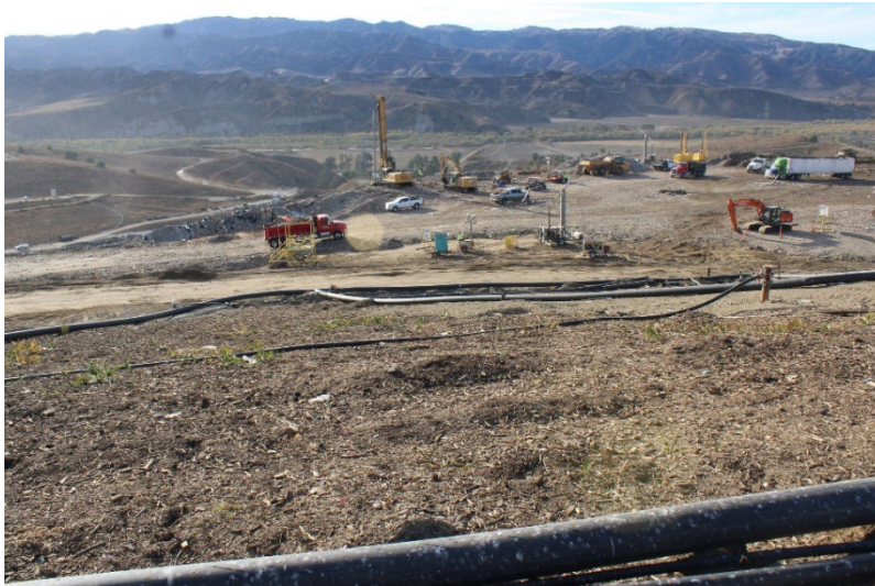
Photo 17: Cell 6 and Cell 8 Working Area: December 3, 2024
