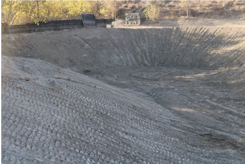
Photo 103: South Terminal and Catch Basins: December 3, 2024
