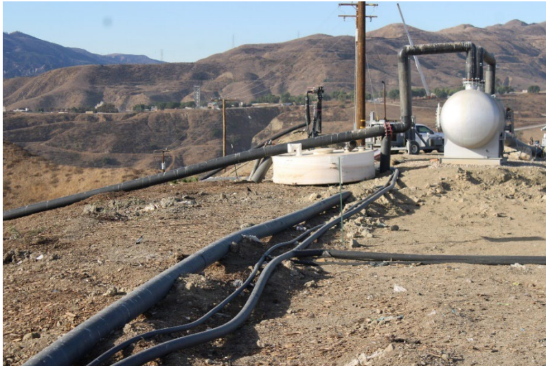
Photo 25: Cell 6 and Cell 8 Working Area: December 3, 2024
