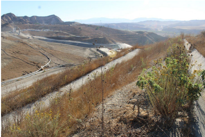
Photo 145: Landfill Perimeter Drainage Channel: October 23, 2024
