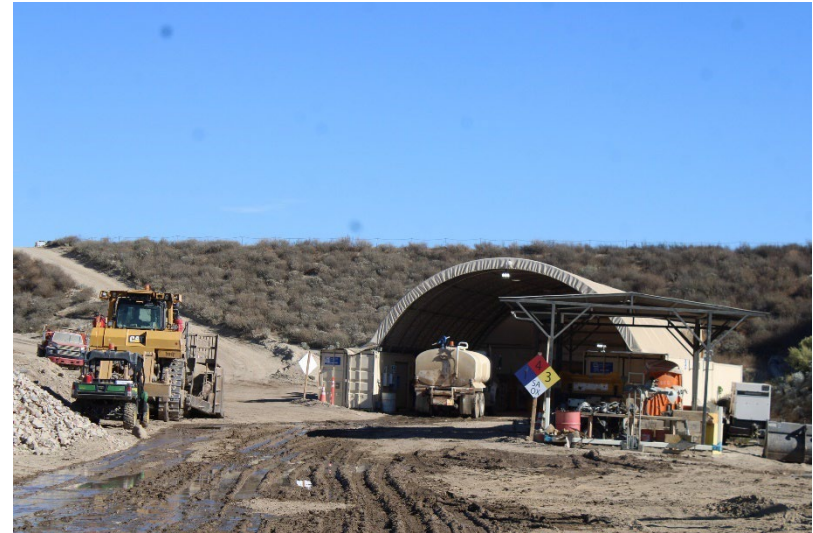
Photo 198: Maintenance and Admin Buildings: November 18, 2024
