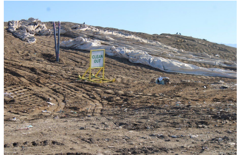
Photo 10: Top Deck Working Area: November 18, 2024
