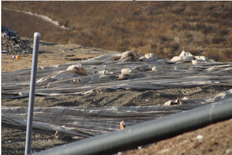
Photo 35: Cell 6 and Cell 8 Working Area: December 3, 2024
