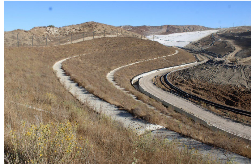
Photo 142: Landfill Perimeter Drainage Channel: October 23, 2024
