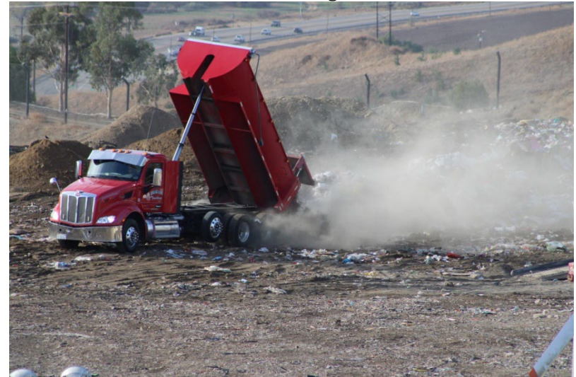
Photo 36: Cell 6 and Cell 8 Working Area: December 3, 2024
