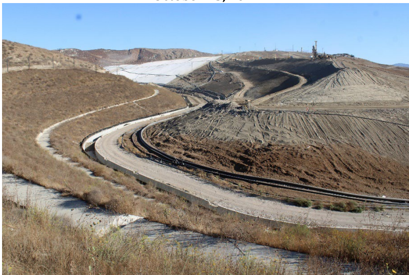
Photo 143: Landfill Perimeter Drainage Channel: October 23, 2024
