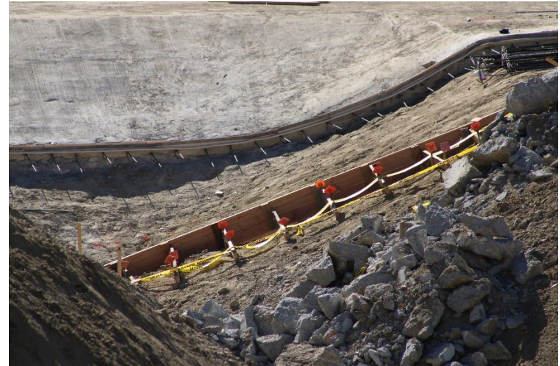
Photo 94: South Terminal and Catch Basins: November 18, 2024
