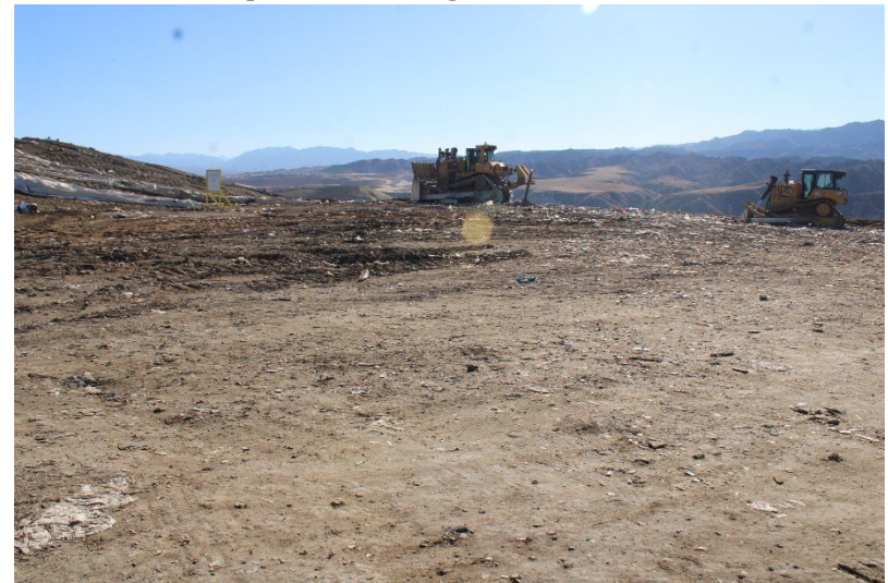
Photo 4: Top Deck Working Area: November 18, 2024
