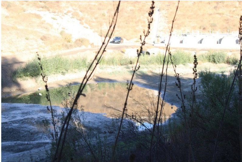
Photo 77: South Terminal and Catch Basins: October 23, 2024
