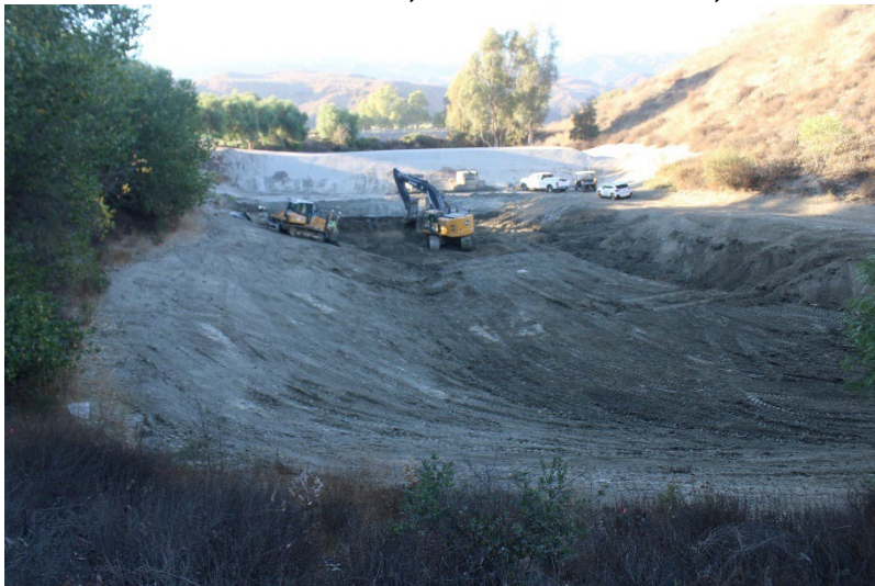
Photo 67: South Terminal and Catch Basins: October 23, 2024
