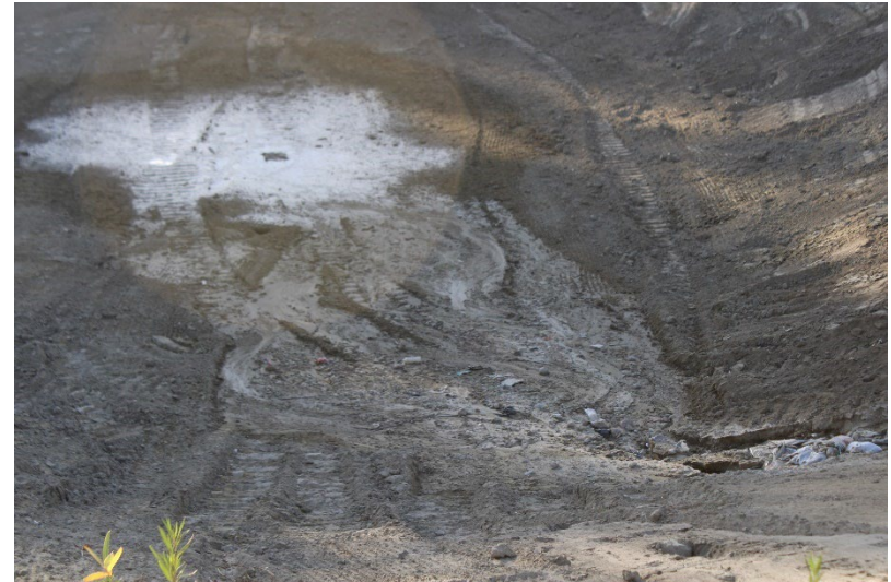
Photo 106: South Terminal and Catch Basins: December 3, 2024
