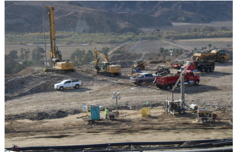
Photo 22: Cell 6 and Cell 8 Working Area: December 3, 2024
