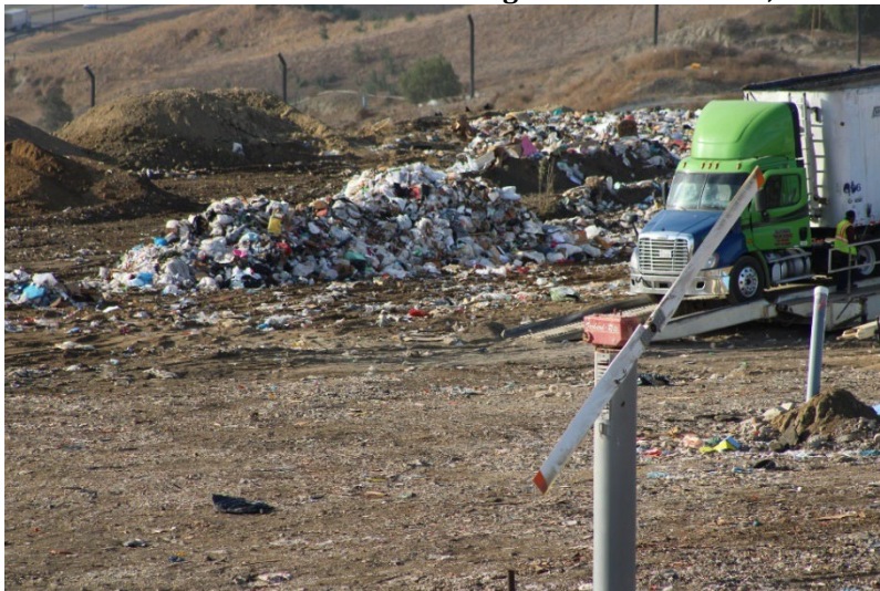
Photo 31: Cell 6 and Cell 8 Working Area: December 3, 2024
