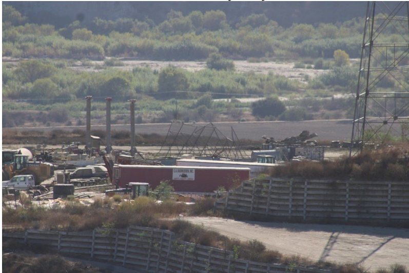
Photo 43: Closed Landfill – Primary Canyon: October 23, 2024
