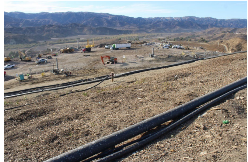
Photo 18: Cell 6 and Cell 8 Working Area: December 3, 2024
