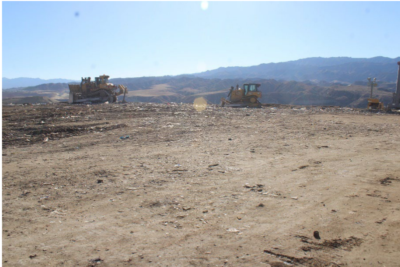
Photo 5: Top Deck Working Area: November 18, 2024
