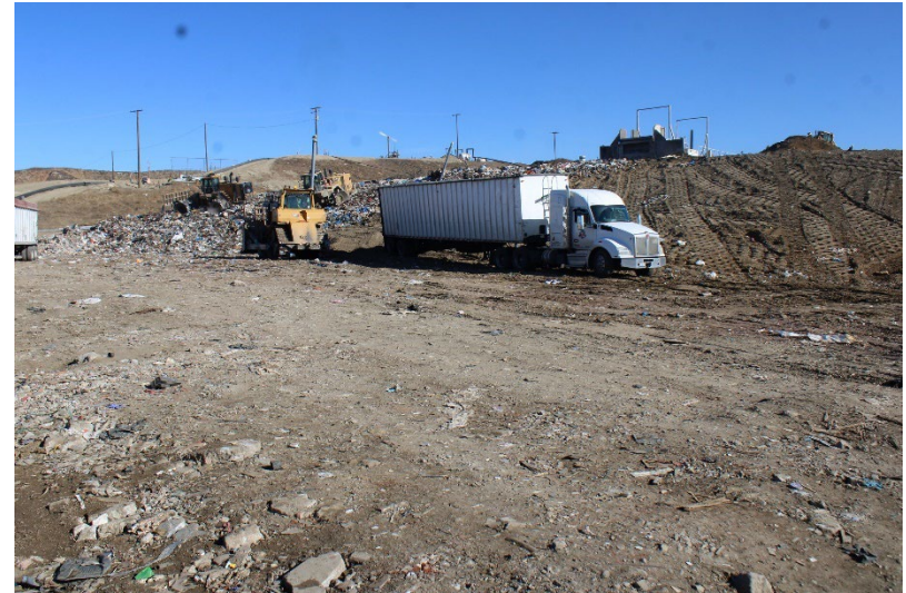
Photo 2: Top Deck Working Area: November 18, 2024
