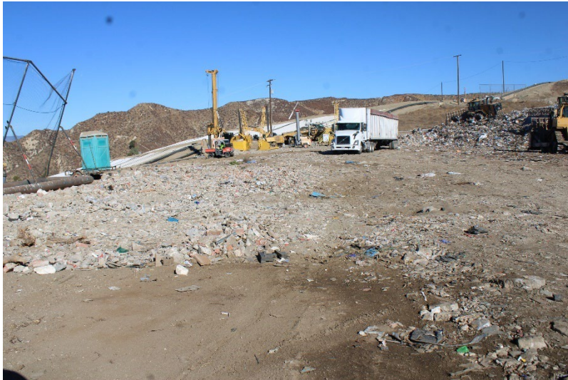
Photo 1: Top Deck Working Area: November 18, 2024
