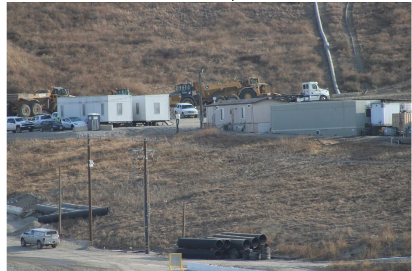
Photo 200: Maintenance and Admin Buildings: December 3, 2024
