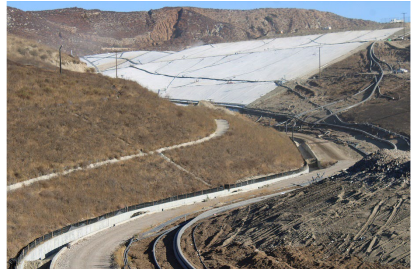
Photo 146: Landfill Perimeter Drainage Channel: October 23, 2024
