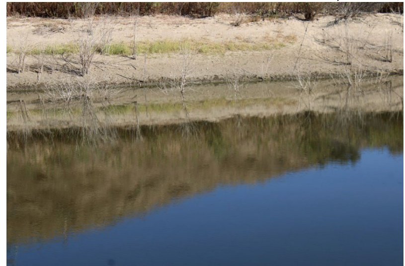
Photo 124: Northeast Sediment Basin: October 23, 2024
