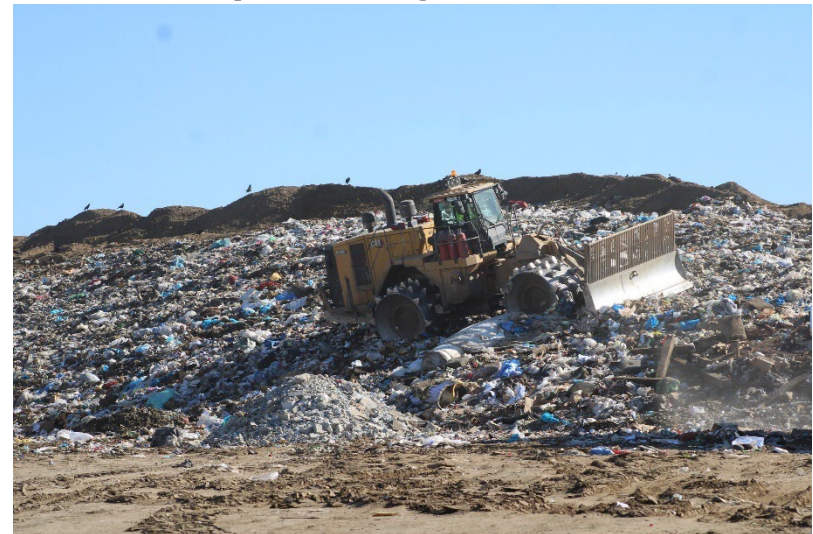
Photo 16: Cell 6 and Cell 8 Working Area: October 23, 2024
