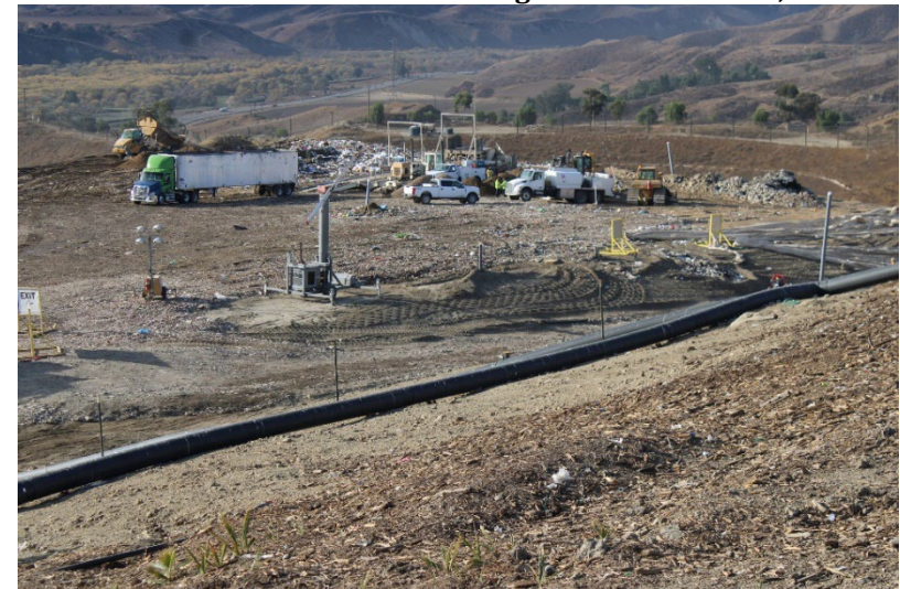
Photo 24: Cell 6 and Cell 8 Working Area: December 3, 2024
