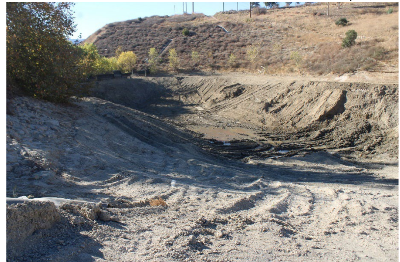
Photo 84: South Terminal and Catch Basins: November 18, 2024
