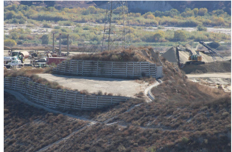
Photo 50: Closed Landfill – Primary Canyon: November 18, 2024
