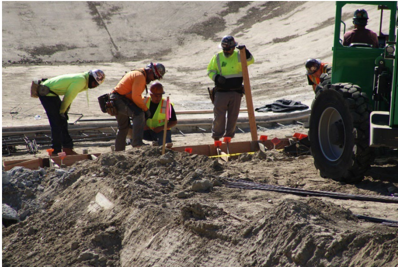
Photo 95: South Terminal and Catch Basins: November 18, 2024
