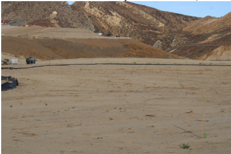
Photo 59: Closed Landfill – Canyon B: December 3, 2024
