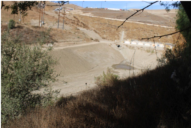
Photo 119: South Terminal and Catch Basins: December 3, 2024
