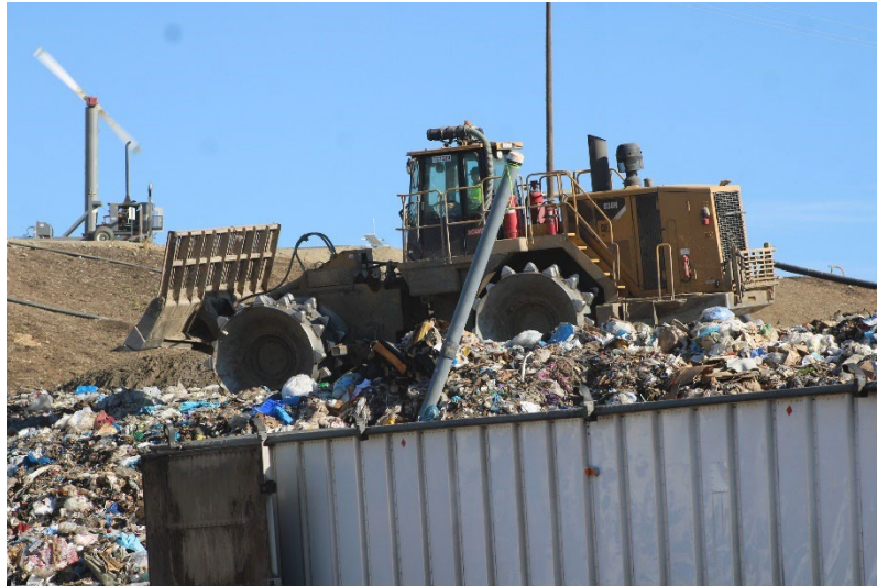
Photo 13: Top Deck Working Area: November 18, 2024
