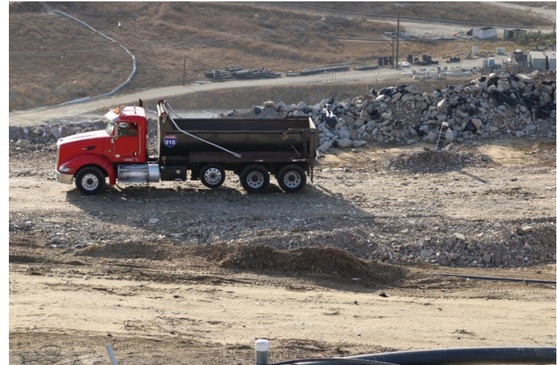
Photo 26: Cell 6 and Cell 8 Working Area: December 3, 2024
