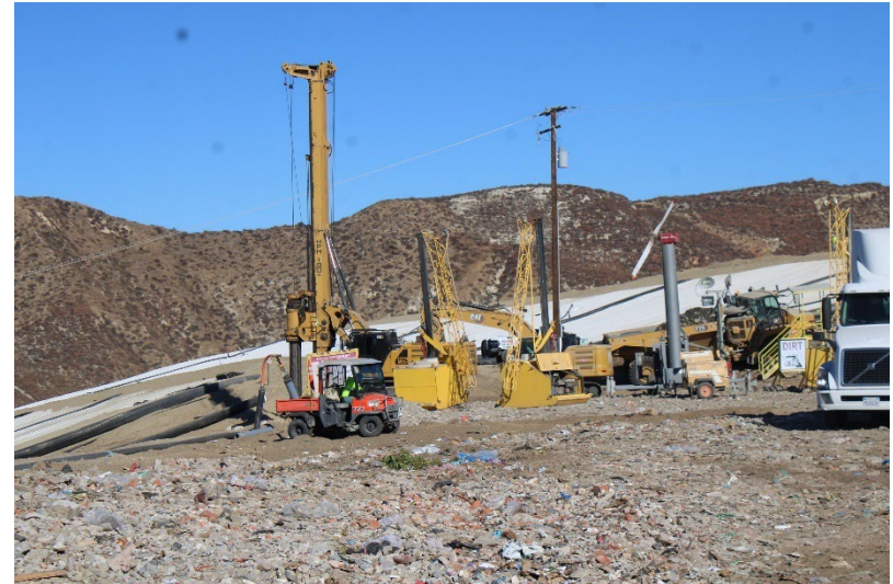
Photo 6: Top Deck Working Area: November 18, 2024
