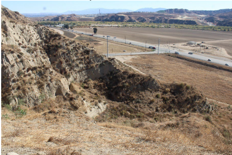
Photo 191: Wolcott Way Entrance Facilities: November 18, 2024
