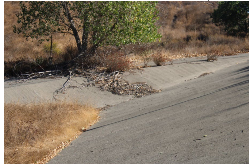
Photo 128: Northeast Sediment Basin: October 23, 2024
