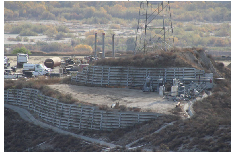
Photo 56: Closed Landfill – Primary Canyon: December 3, 2024
