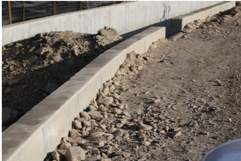
Photo 151: Landfill Perimeter Drainage Channel: December 3, 2024
