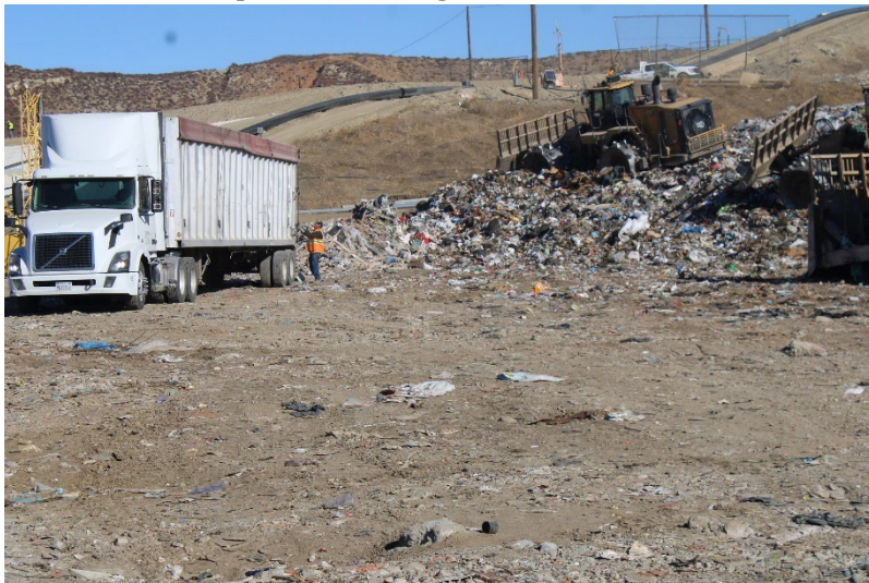
Photo 7: Top Deck Working Area: November 18, 2024
