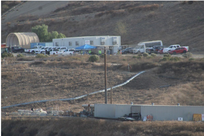
Photo 201: Maintenance and Admin Buildings: December 3, 2024
