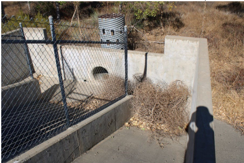
Photo 127: Northeast Sediment Basin: October 23, 2024
