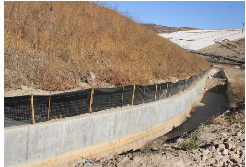
Photo 150: Landfill Perimeter Drainage Channel: November 18, 2024
