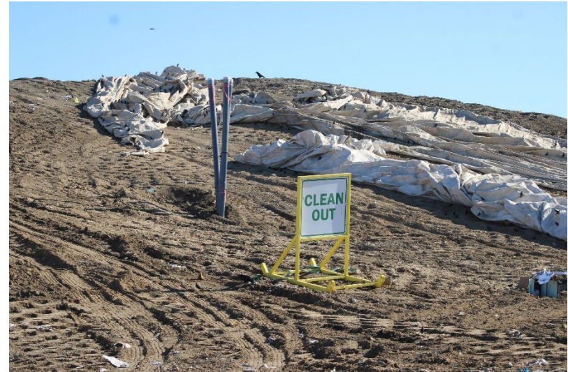
Photo 14: Top Deck Working Area: November 18, 2024
