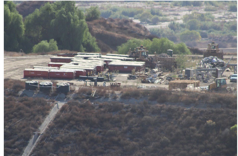
Photo 42: Closed Landfill – Primary Canyon: October 23, 2024
