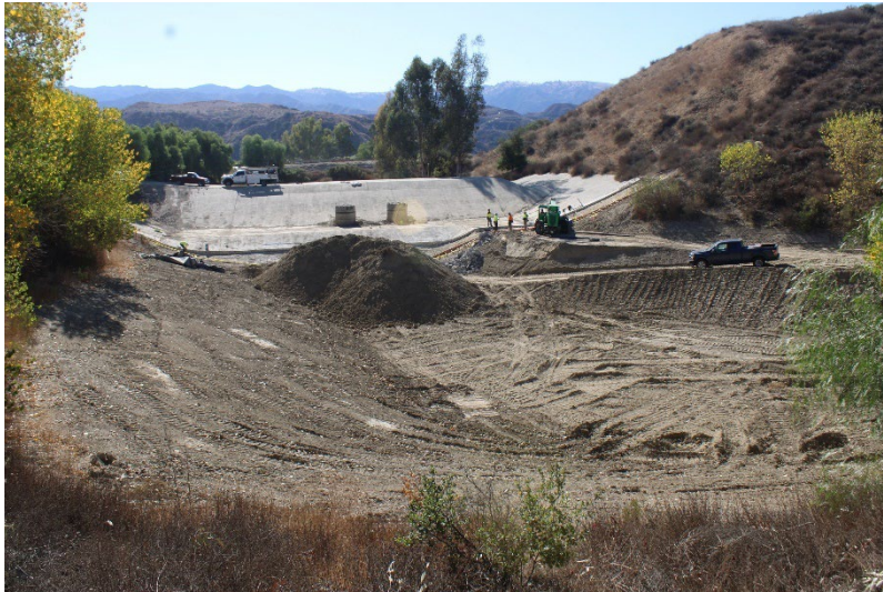
Photo 89: South Terminal and Catch Basins: November 18, 2024
