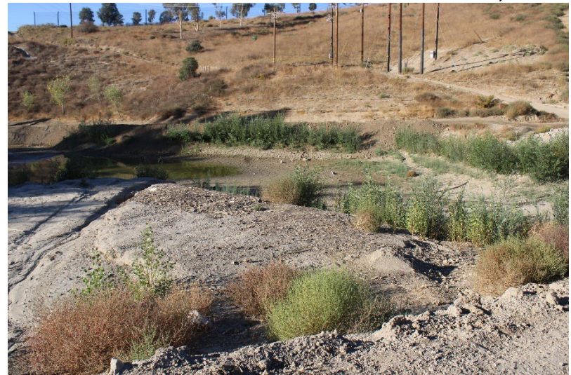
Photo 80: South Terminal and Catch Basins: October 23, 2024
