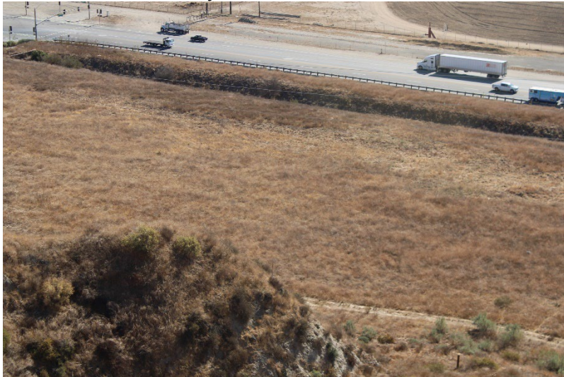
Photo 195: Wolcott Way Entrance Facilities: November 18, 2024
