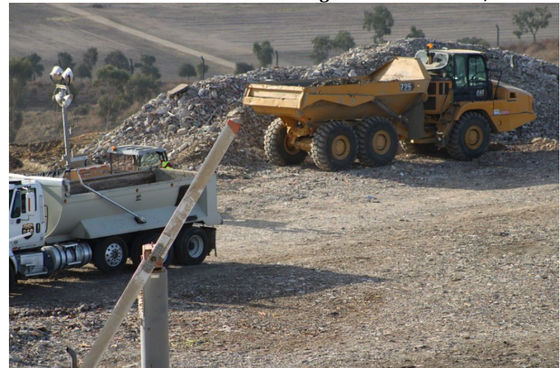
Photo 28: Cell 6 and Cell 8 Working Area: December 3, 2024
