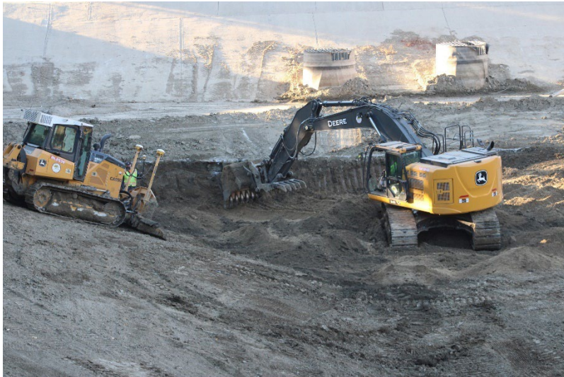
Photo 71: South Terminal and Catch Basins: October 23, 2024
