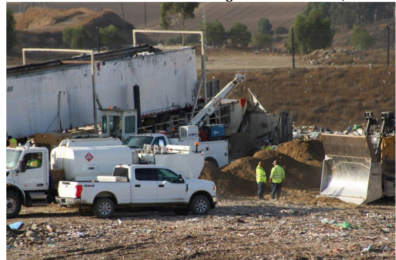
Photo 32: Cell 6 and Cell 8 Working Area: December 3, 2024
