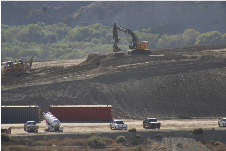
Photo 45: Closed Landfill – Primary Canyon: October 23, 2024
