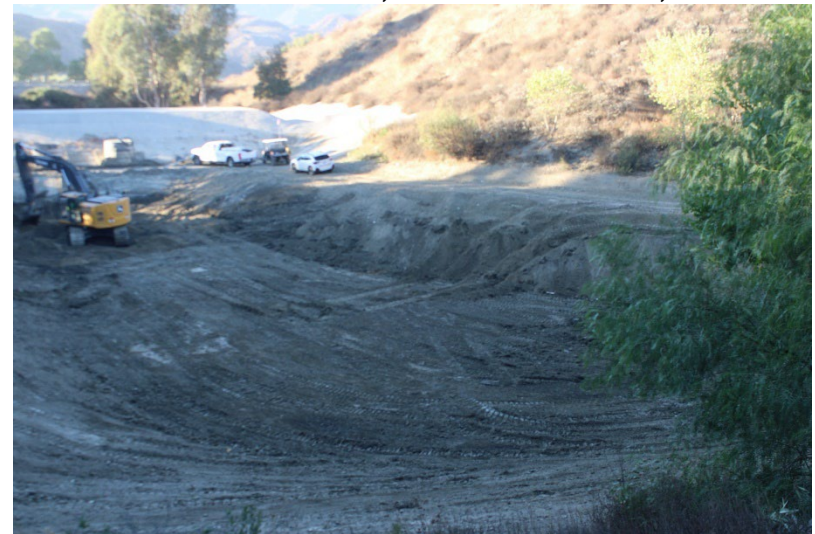
Photo 68: South Terminal and Catch Basins: October 23, 2024
