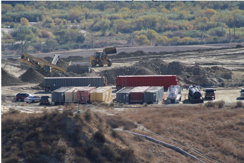
Photo 51: Closed Landfill – Primary Canyon: November 18, 2024
