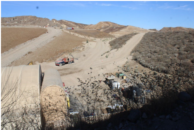
Photo 199: Maintenance and Admin Buildings: November 18, 2024
