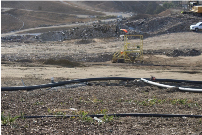
Photo 21: Cell 6 and Cell 8 Working Area: December 3, 2024
