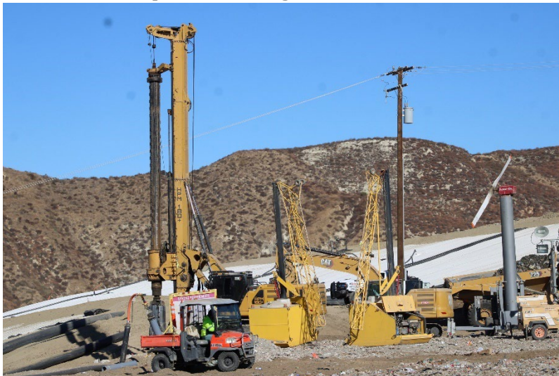
Photo 11: Top Deck Working Area: November 18, 2024
