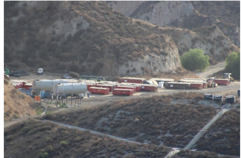
Photo 54: Closed Landfill – Primary Canyon: December 3, 2024
