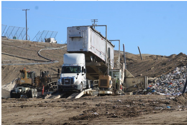
Photo 15: Cell 6 and Cell 8 Working Area: October 23, 2024
