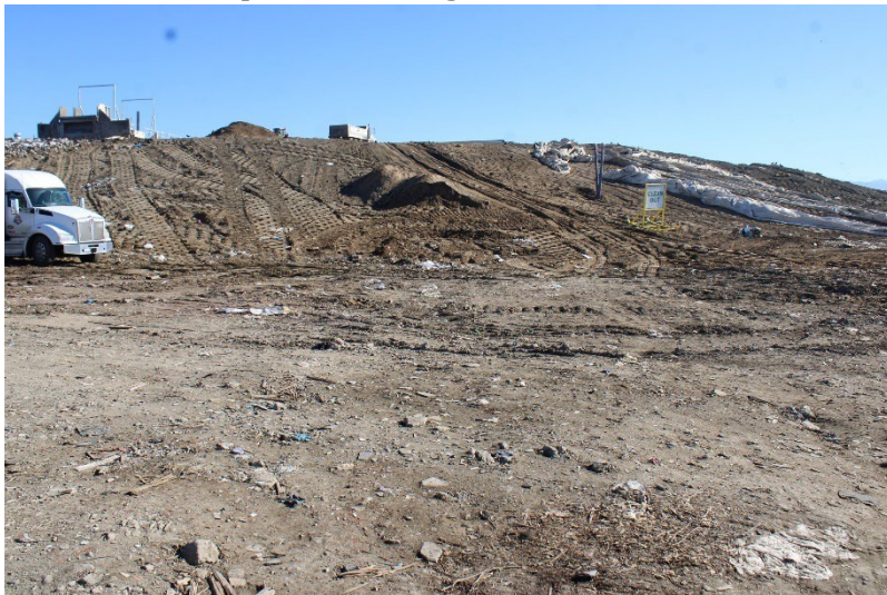
Photo 3: Top Deck Working Area: November 18, 2024
