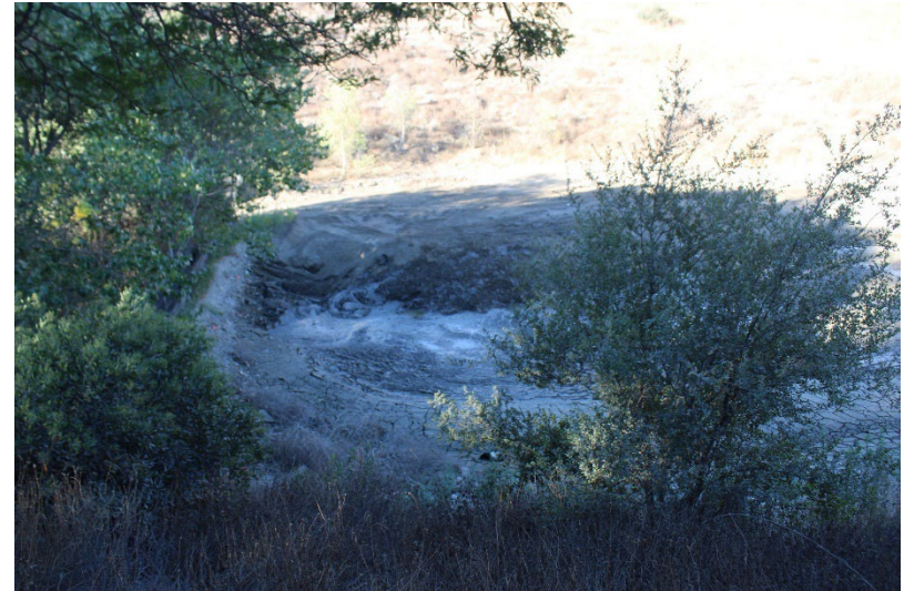
Photo 72: South Terminal and Catch Basins: October 23, 2024
