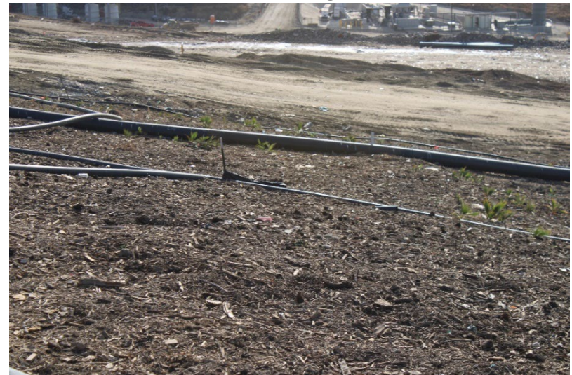
Photo 20: Cell 6 and Cell 8 Working Area: December 3, 2024
