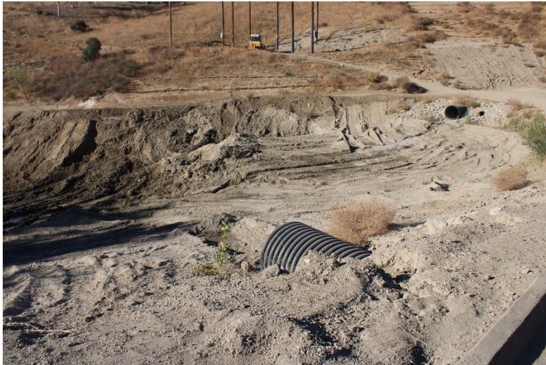
Photo 85: South Terminal and Catch Basins: November 18, 2024
