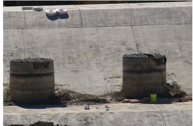
Photo 96: South Terminal and Catch Basins: November 18, 2024
