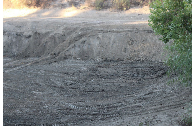
Photo 70: South Terminal and Catch Basins: October 23, 2024
