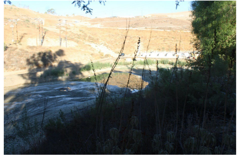
Photo 74: South Terminal and Catch Basins: October 23, 2024
