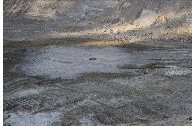
Photo 104: South Terminal and Catch Basins: December 3, 2024
