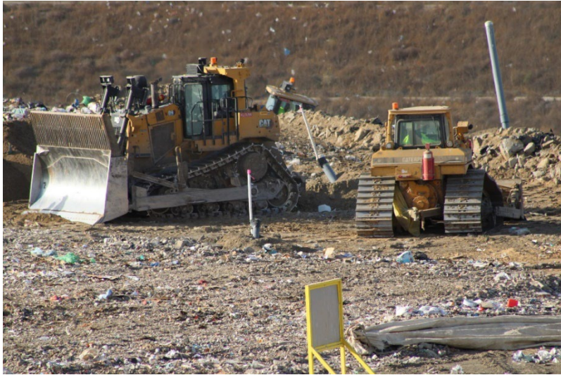
Photo 33: Cell 6 and Cell 8 Working Area: December 3, 2024
