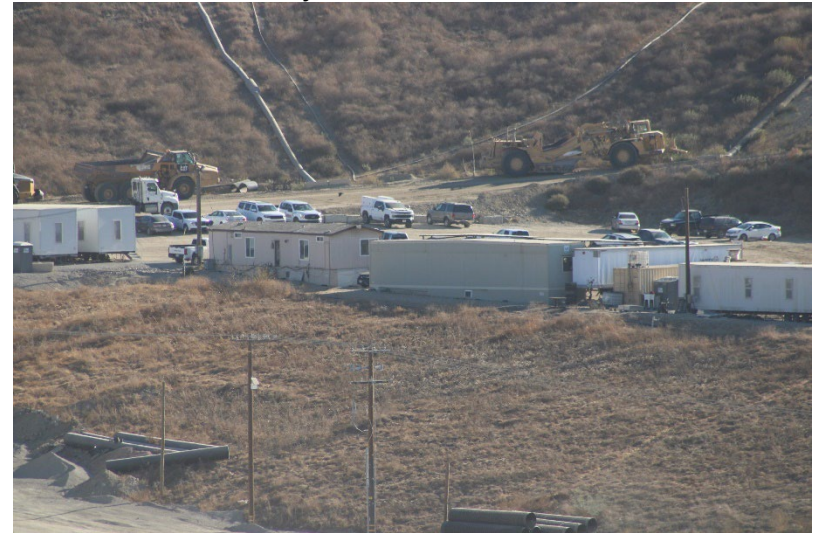
Photo 196: Maintenance and Admin Buildings: October 23, 2024
