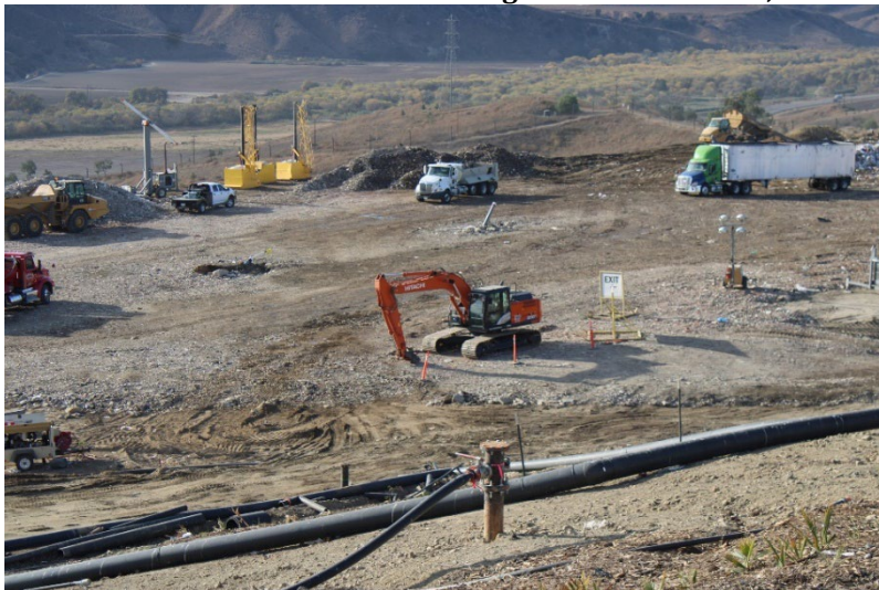
Photo 23: Cell 6 and Cell 8 Working Area: December 3, 2024
