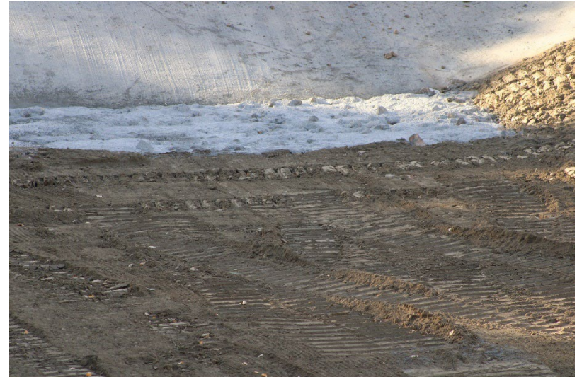
Photo 116: South Terminal and Catch Basins: December 3, 2024
