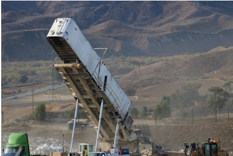
Photo 37: Cell 6 and Cell 8 Working Area: December 3, 2024
