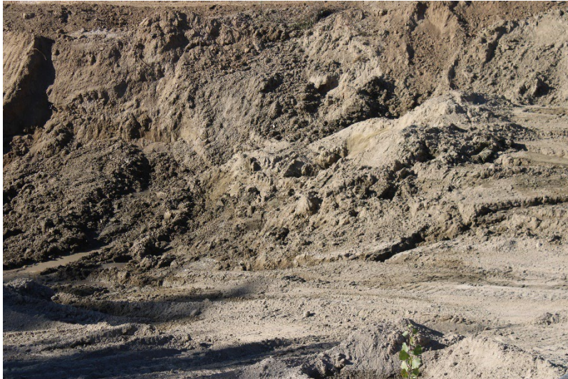
Photo 87: South Terminal and Catch Basins: November 18, 2024
