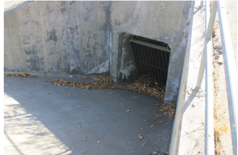
Photo 126: Northeast Sediment Basin: October 23, 2024
