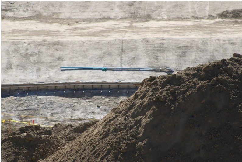
Photo 93: South Terminal and Catch Basins: November 18, 2024
