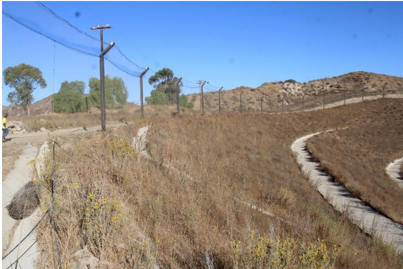
Photo 141: Landfill Perimeter Drainage Channel: October 23, 2024
