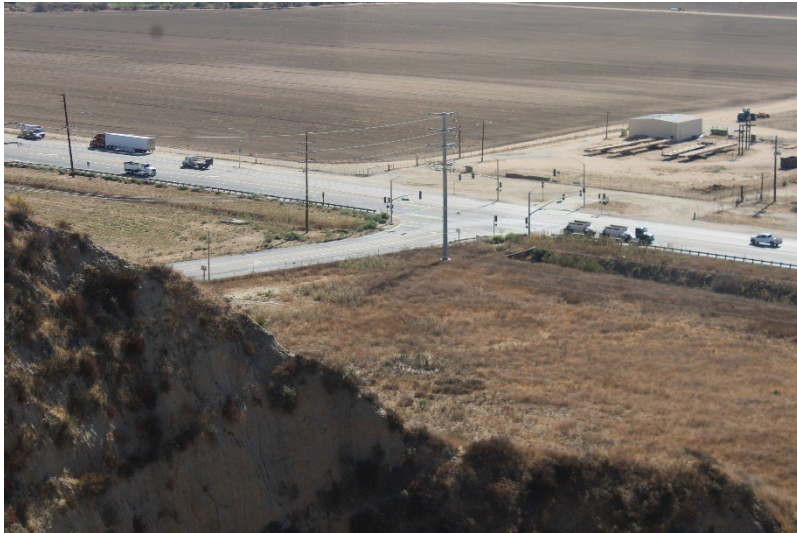
Photo 189: Wolcott Way Entrance Facilities: October 23, 2024
