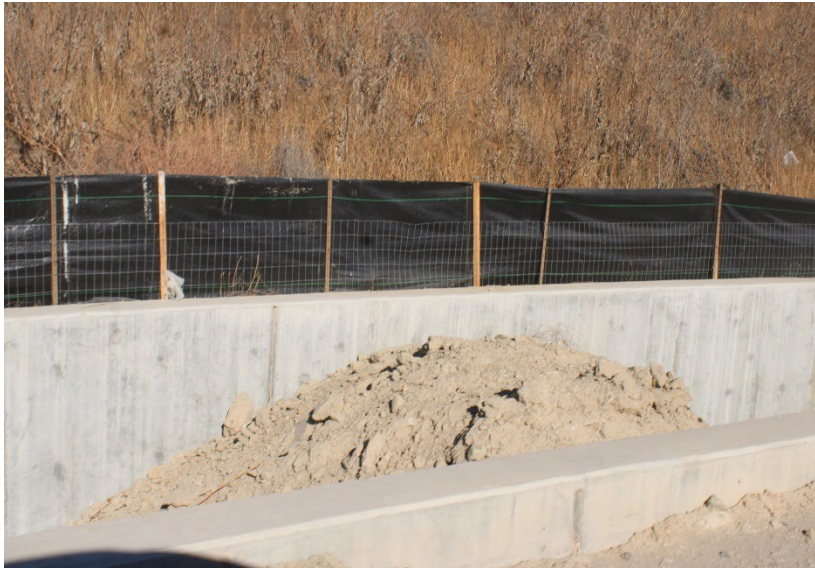
Photo 149: Landfill Perimeter Drainage Channel: November 18, 2024
