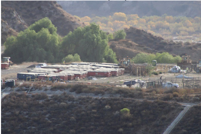
Photo 55: Closed Landfill – Primary Canyon: December 3, 2024
