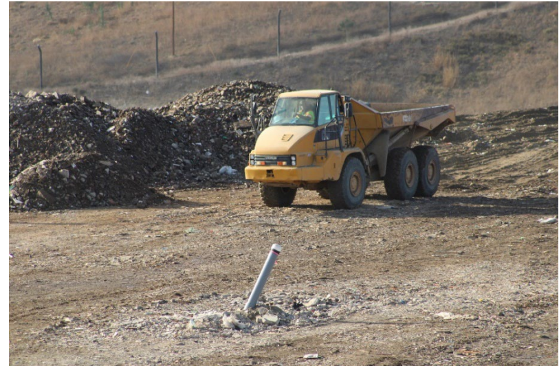
Photo 30: Cell 6 and Cell 8 Working Area: December 3, 2024
