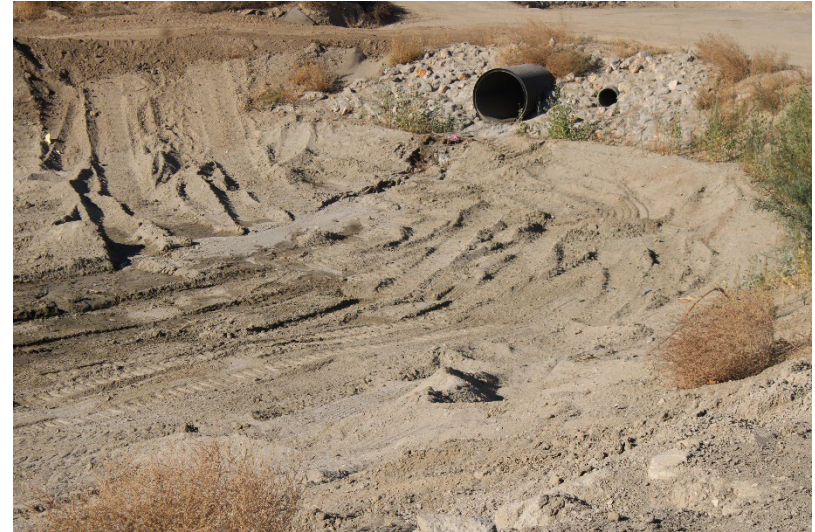
Photo 88: South Terminal and Catch Basins: November 18, 2024
