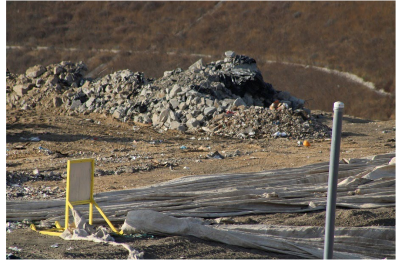
Photo 34: Cell 6 and Cell 8 Working Area: December 3, 2024
