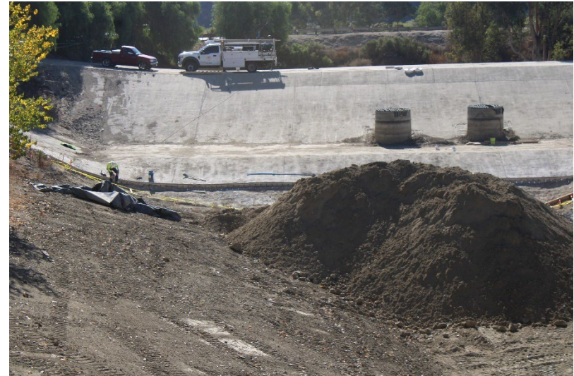
Photo 90: South Terminal and Catch Basins: November 18, 2024
