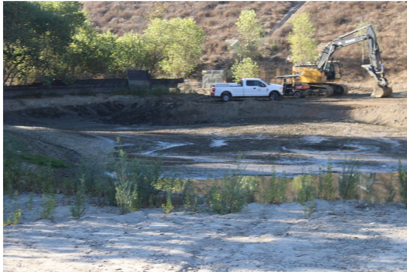
Photo 81: South Terminal and Catch Basins: October 23, 2024
