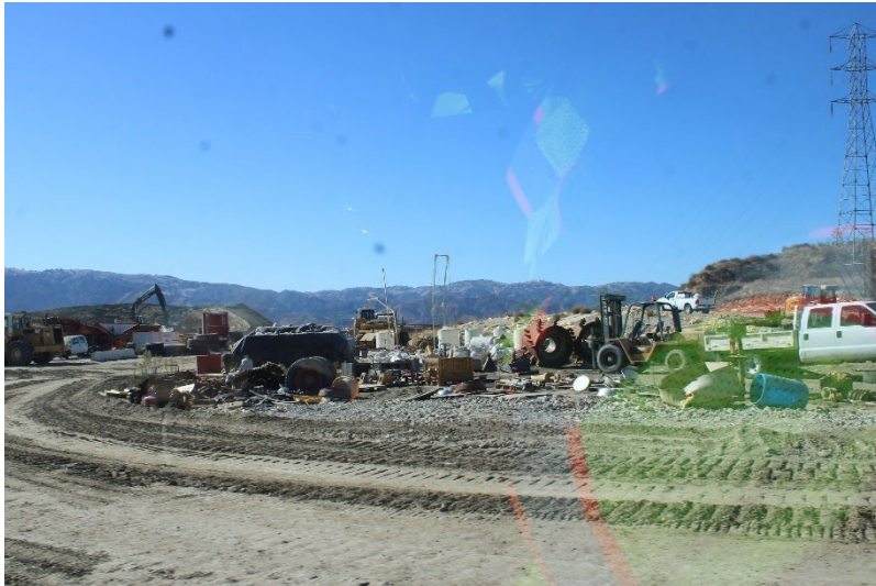
Photo 53: Closed Landfill – Primary Canyon: November 18, 2024
