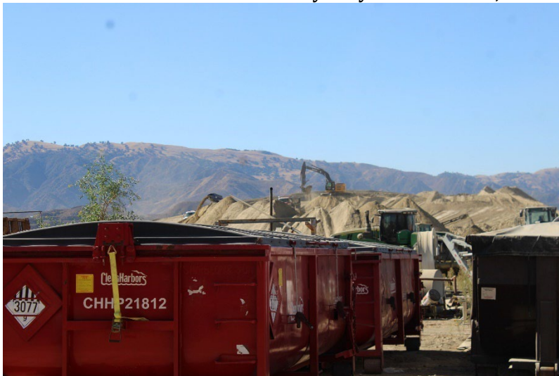
Photo 47: Closed Landfill – Primary Canyon: October 23, 2024
