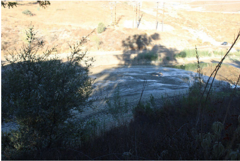
Photo 73: South Terminal and Catch Basins: October 23, 2024
