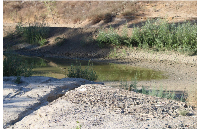
Photo 82: South Terminal and Catch Basins: October 23, 2024
