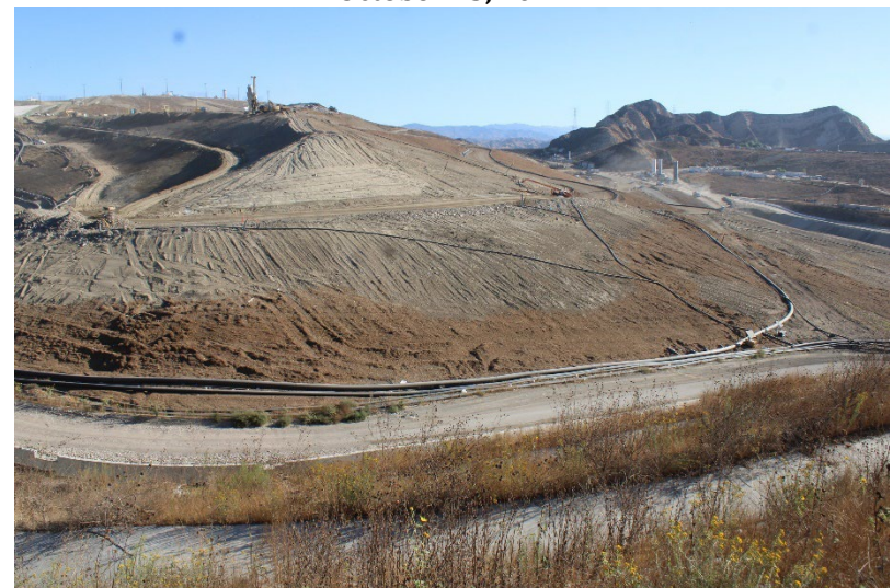
Photo 144: Landfill Perimeter Drainage Channel: October 23, 2024
