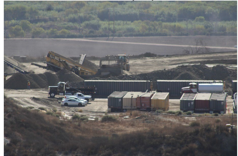
Photo 44: Closed Landfill – Primary Canyon: October 23, 2024
