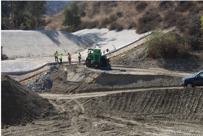
Photo 91: South Terminal and Catch Basins: November 18, 2024
