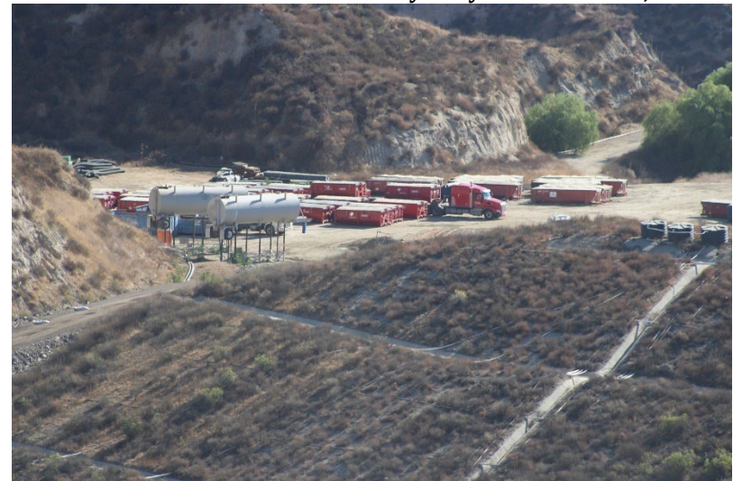
Photo 48: Closed Landfill – Primary Canyon: November 18, 2024
