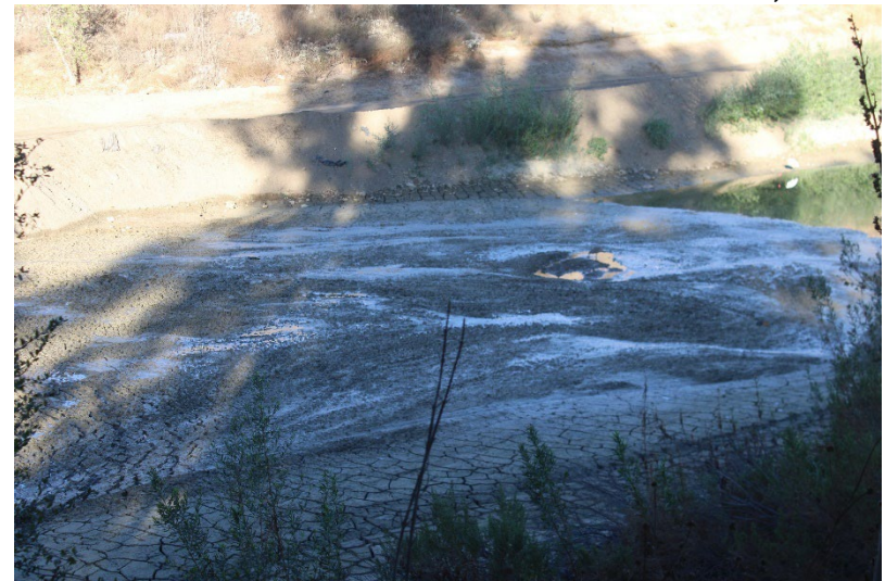
Photo 76: South Terminal and Catch Basins: October 23, 2024
