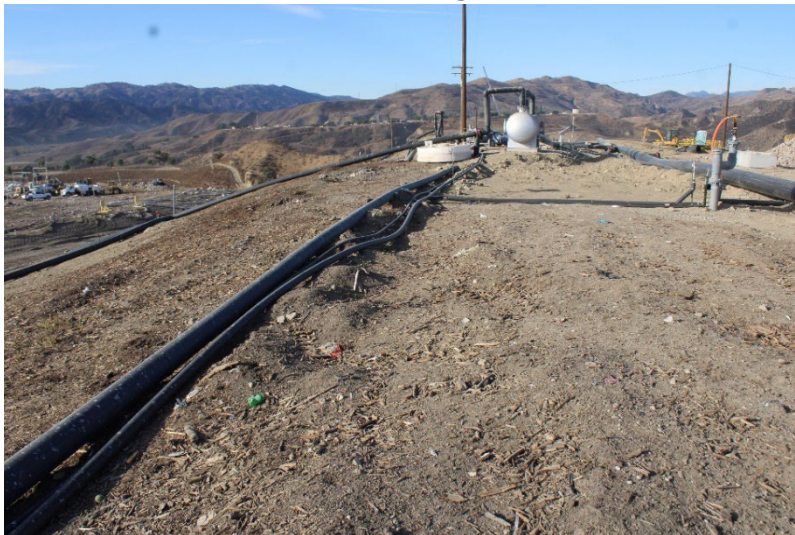
Photo 19: Cell 6 and Cell 8 Working Area: December 3, 2024
