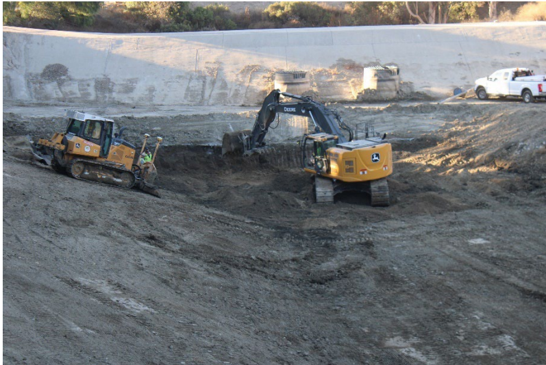
Photo 69: South Terminal and Catch Basins: October 23, 2024
