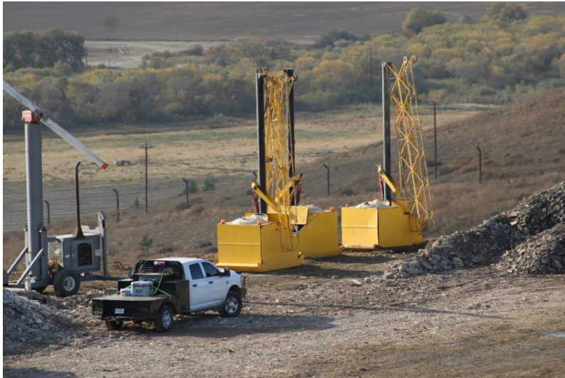
Photo 29: Cell 6 and Cell 8 Working Area: December 3, 2024
