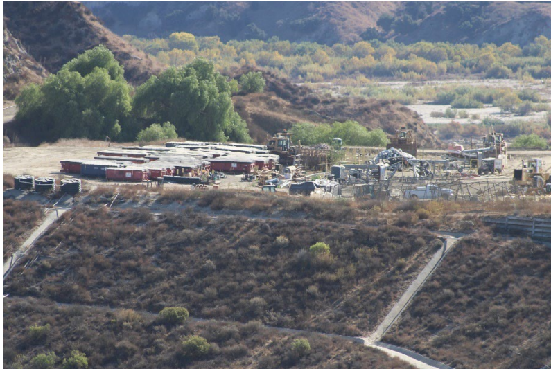
Photo 49: Closed Landfill – Primary Canyon: November 18, 2024
