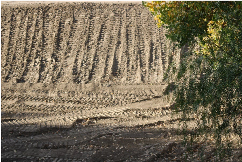
Photo 117: South Terminal and Catch Basins: December 3, 2024
