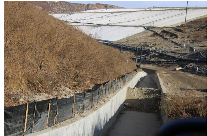
Photo 152: Landfill Perimeter Drainage Channel: December 3, 2024
