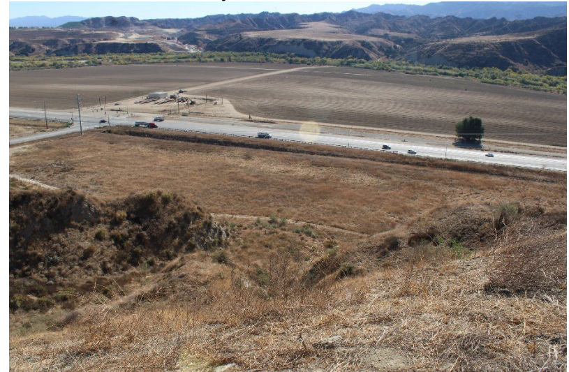
Photo 192: Wolcott Way Entrance Facilities: November 18, 2024
