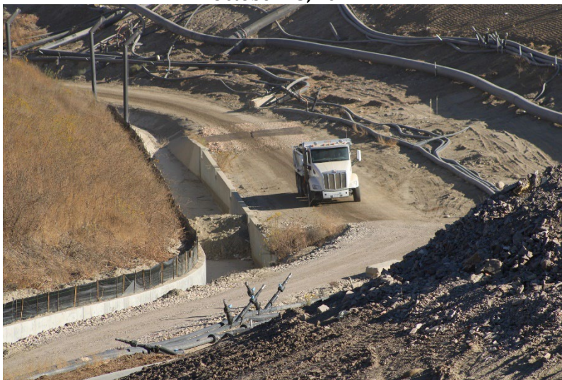
Photo 147: Landfill Perimeter Drainage Channel: October 23, 2024
