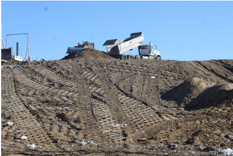
Photo 9: Top Deck Working Area: November 18, 2024
