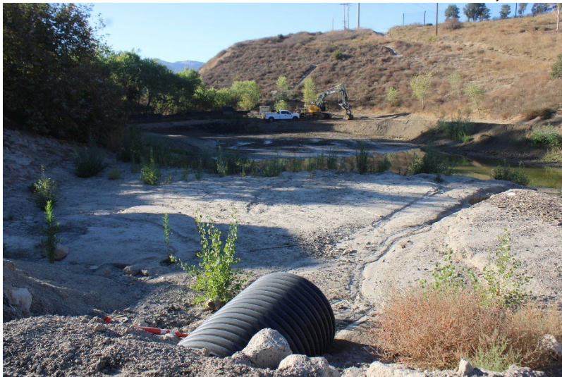
Photo 79: South Terminal and Catch Basins: October 23, 2024
