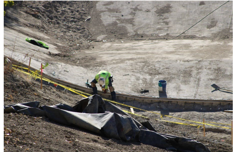
Photo 92: South Terminal and Catch Basins: November 18, 2024
