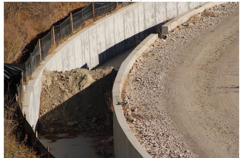
Photo 148: Landfill Perimeter Drainage Channel: October 23, 2024
