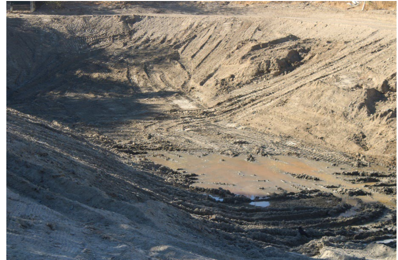
Photo 86: South Terminal and Catch Basins: November 18, 2024
