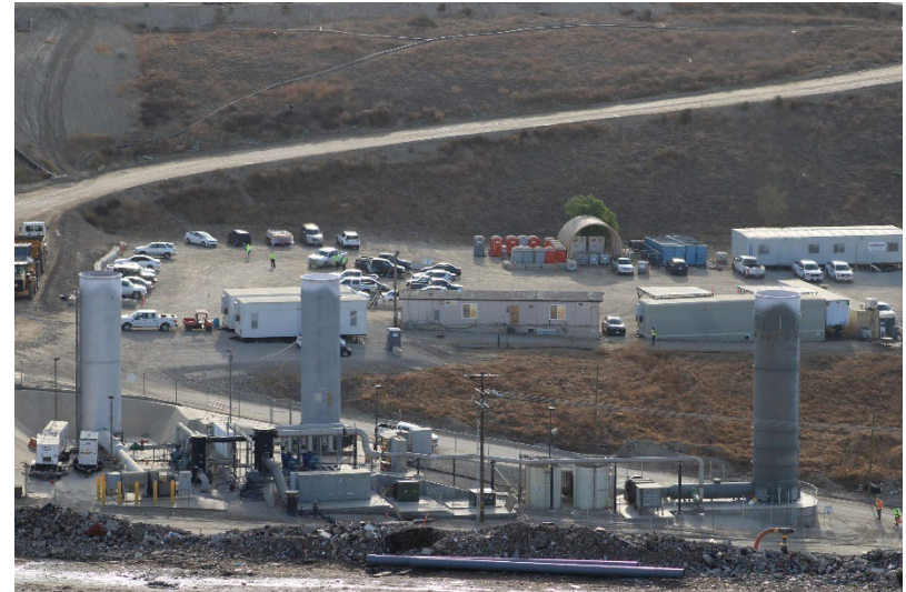
Photo 202: Maintenance and Admin Buildings: December 3, 2024
