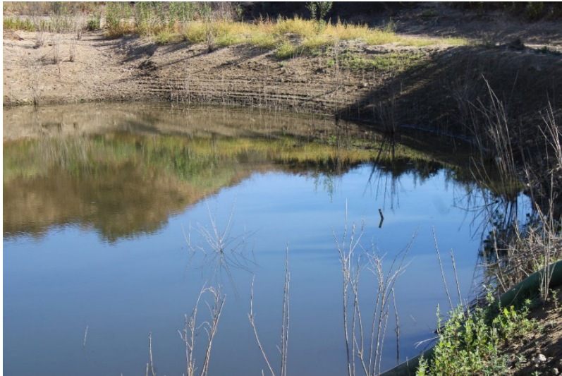
Photo 125: Northeast Sediment Basin: October 23, 2024
