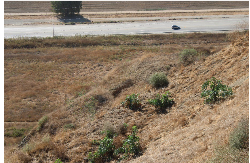
Photo 190: Wolcott Way Entrance Facilities: October 23, 2024
