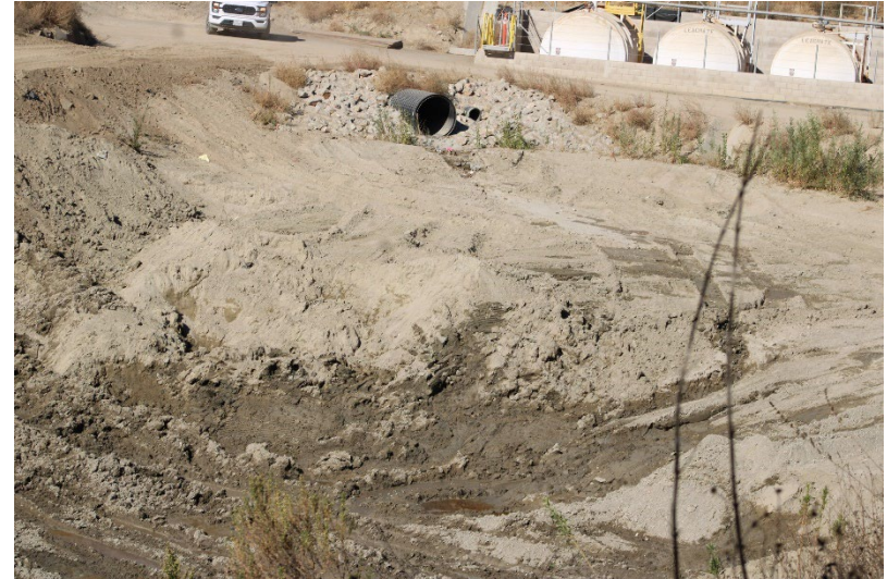
Photo 100: South Terminal and Catch Basins: November 18, 2024
