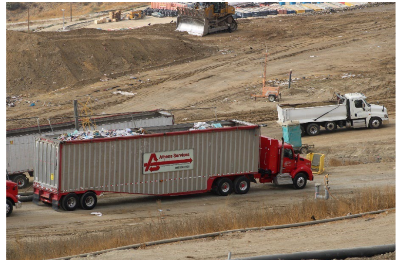
Photo 20: Cell 6 and Cell 8 Working Area: September 19, 2024
