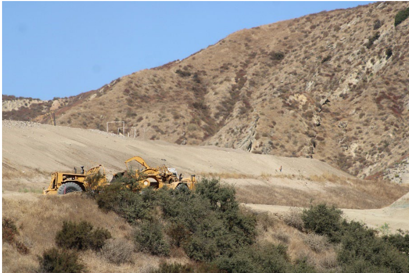
Photo 33: Closed Landfill - Canyon B: August 21, 2024
