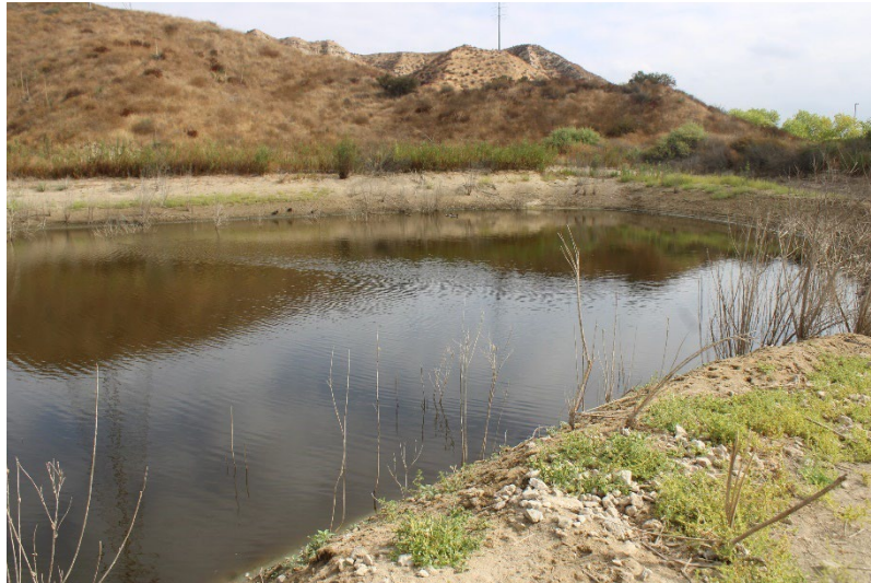
Photo 105: Northeast Sediment Basin: September 19, 2024
