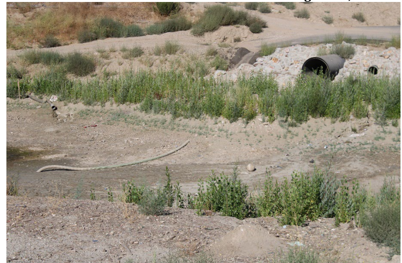
Photo 76: South Terminal and Catch Basins: August 21, 2024
