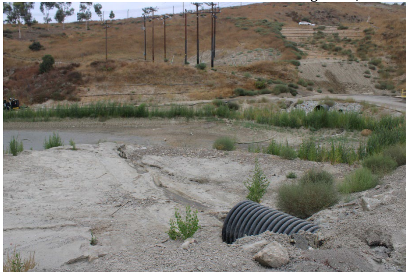
Photo 83: South Terminal and Catch Basins: September 19, 2024
