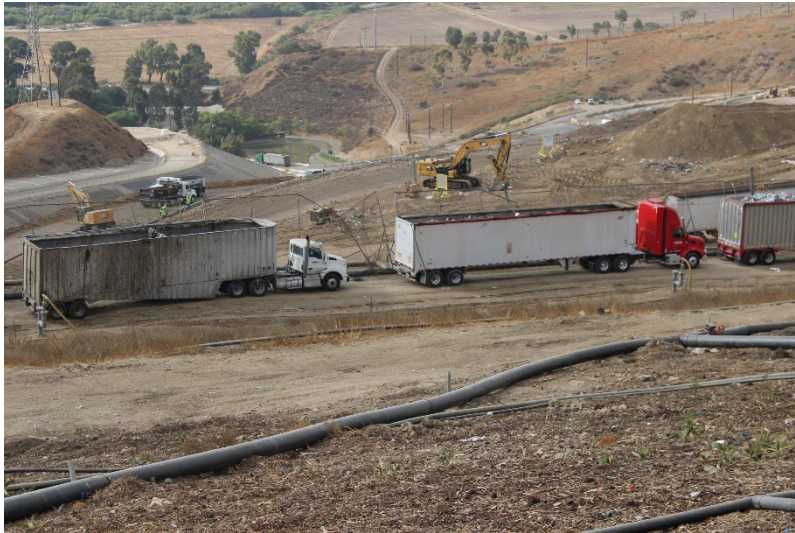
Photo 17: Cell 6 and Cell 8 Working Area: September 19, 2024
