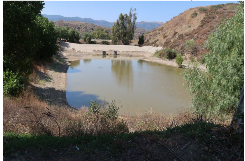
Photo 68: South Terminal and Catch Basins: July 24, 2024
