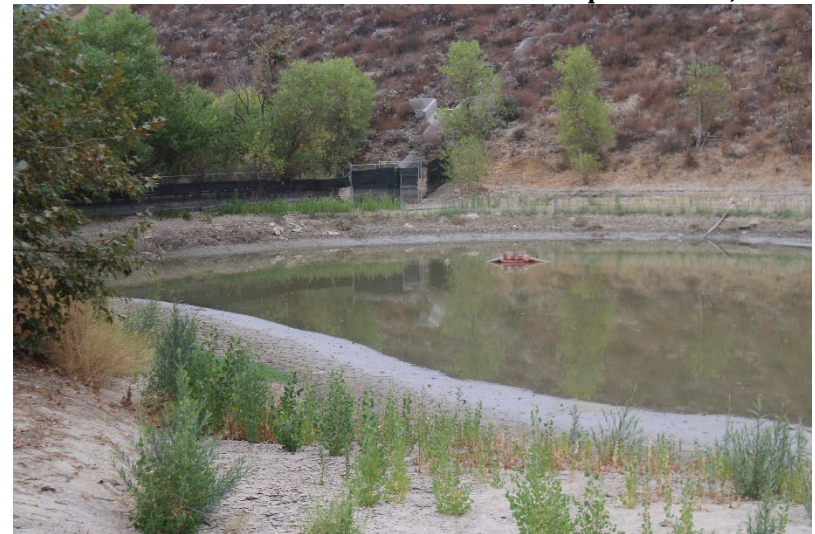
Photo 84: South Terminal and Catch Basins: September 19, 2024
