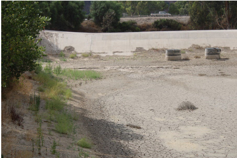
Photo 89: South Terminal and Catch Basins: September 19, 2024
