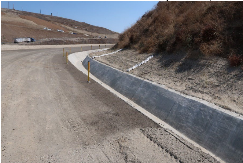
Photo 111: Landfill Perimeter Drainage Channel: July 24, 2024
