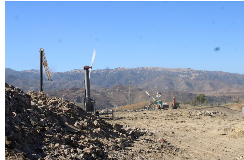
Photo 8: Top Deck Working Area: August 21, 2024
