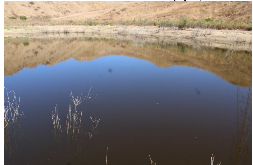
Photo 100: Northeast Sediment Basin: August 21, 2024
