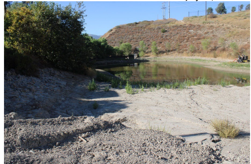
Photo 72: South Terminal and Catch Basins: August 21, 2024
