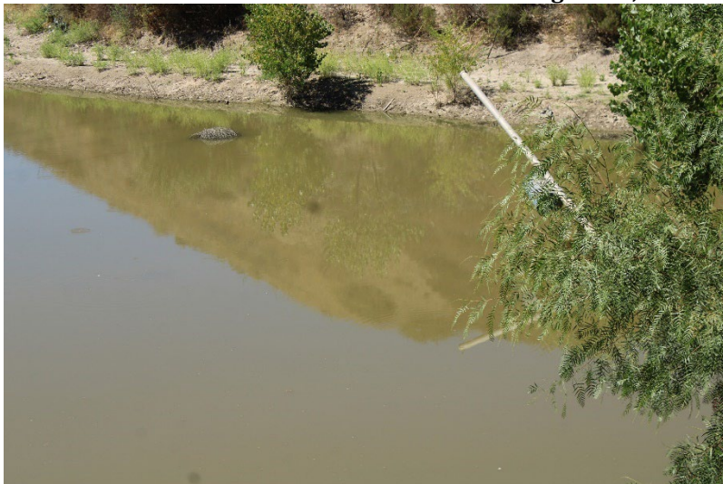
Photo 79: South Terminal and Catch Basins: August 21, 2024
