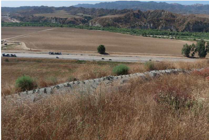
Photo 137: Wolcott Way Entrance Facilities: July 24, 2024
