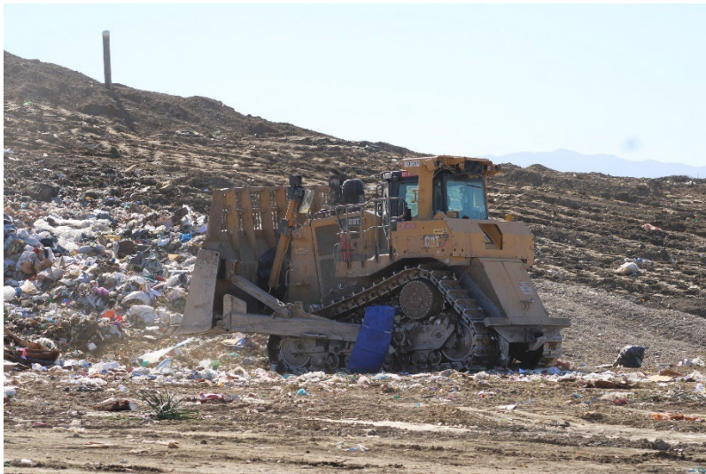
Photo 13: Top Deck Working Area: August 21, 2024
