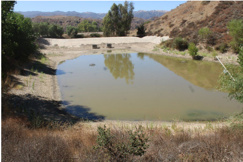
Photo 77: South Terminal and Catch Basins: August 21, 2024
