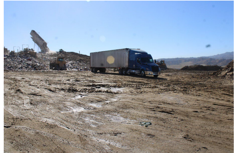
Photo 2: Top Deck Working Area: August 21, 2024
