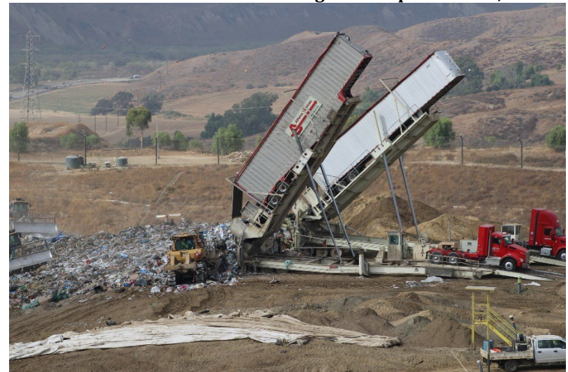
Photo 28: Cell 6 and Cell 8 Working Area: September 19, 2024
