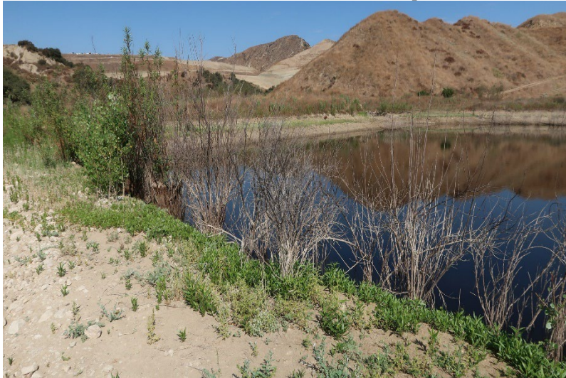
Photo 95: Northeast Sediment Basin: July 24, 2024
