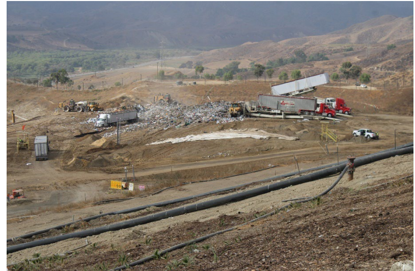
Photo 18: Cell 6 and Cell 8 Working Area: September 19, 2024
