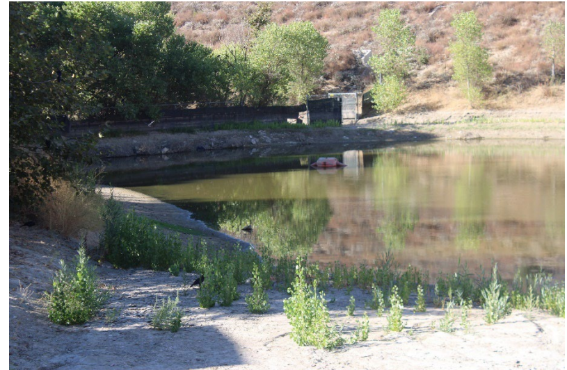
Photo 74: South Terminal and Catch Basins: August 21, 2024
