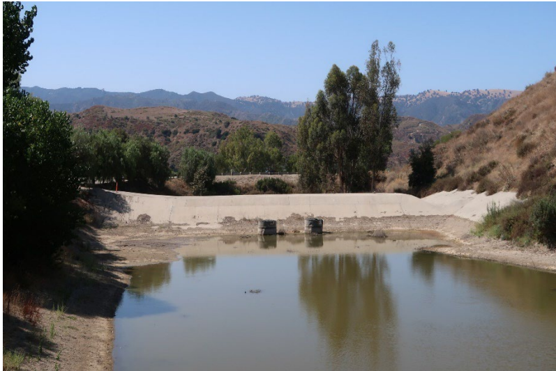
Photo 69: South Terminal and Catch Basins: July 24, 2024
