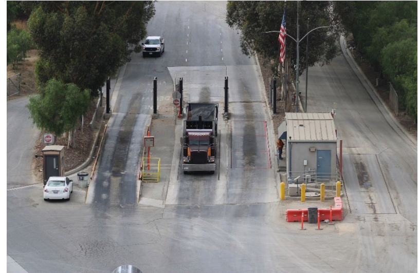
Photo 148: Maintenance and Admin Buildings: September 19, 2024
