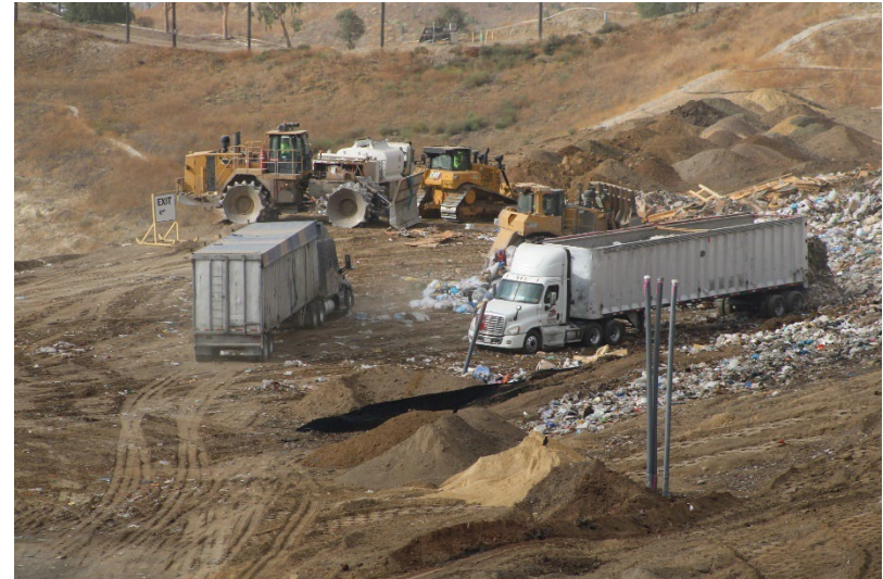
Photo 22: Cell 6 and Cell 8 Working Area: September 19, 2024
