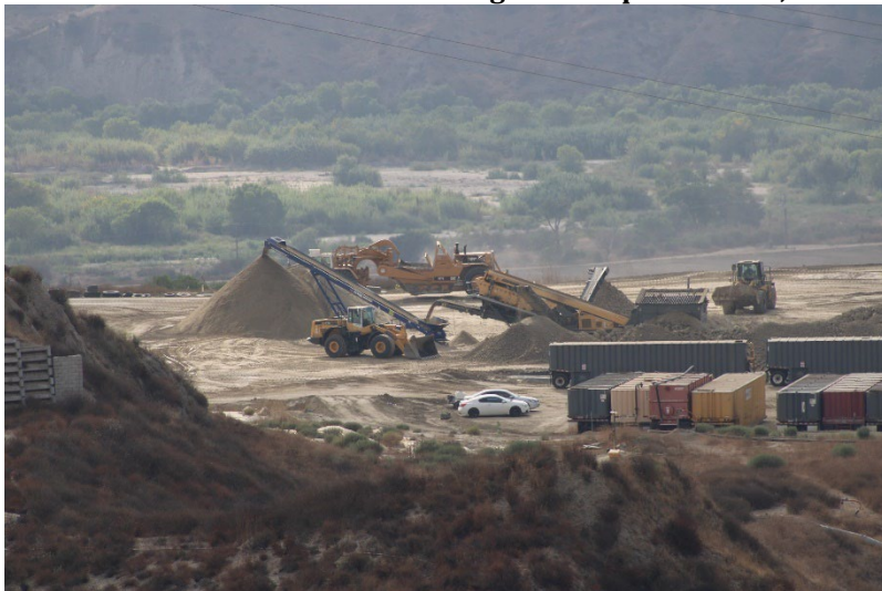
Photo 27: Cell 6 and Cell 8 Working Area: September 19, 2024
