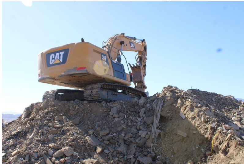
Photo 7: Top Deck Working Area: August 21, 2024
