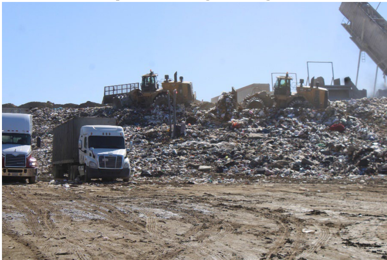
Photo 3: Top Deck Working Area: August 21, 2024
