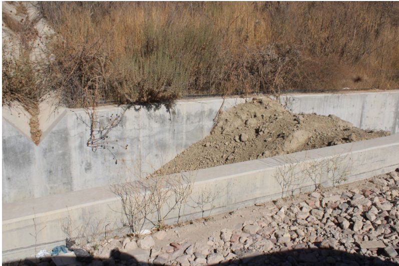
Photo 113: Landfill Perimeter Drainage Channel: August 21, 2024
