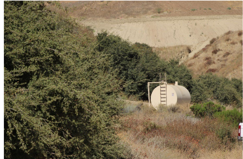
Photo 30: Closed Landfill – Canyon B: August 21, 2024
