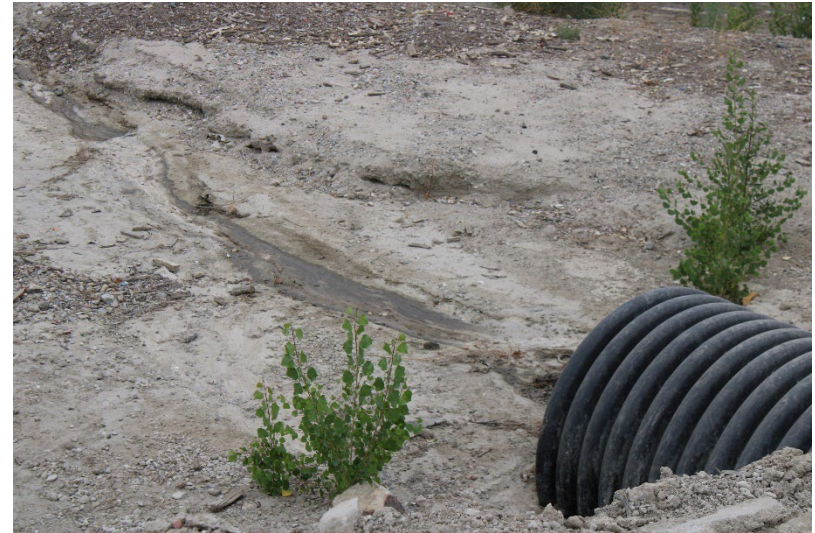
Photo 86: South Terminal and Catch Basins: September 19, 2024
