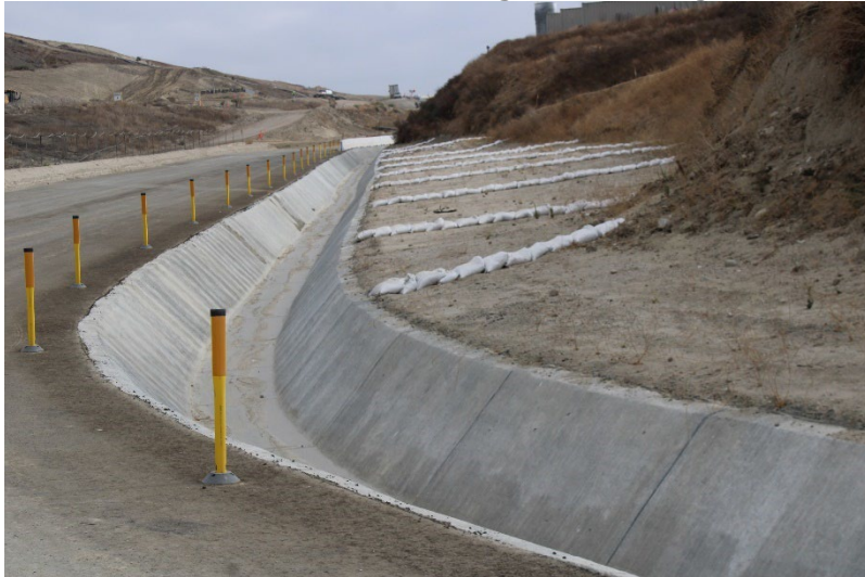
Photo 115: Landfill Perimeter Drainage Channel: September 19, 2024
