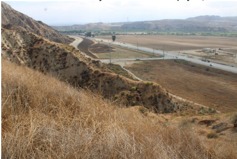
Photo 139: Wolcott Way Entrance Facilities: September 19, 2024
