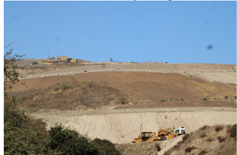
Photo 32: Closed Landfill – Canyon B: August 21, 2024
