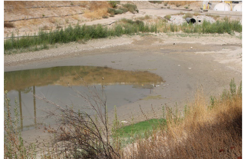
Photo 94: South Terminal and Catch Basins: September 19, 2024
