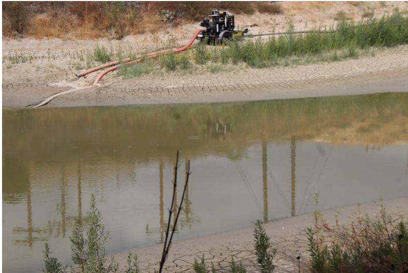
Photo 93: South Terminal and Catch Basins: September 19, 2024
