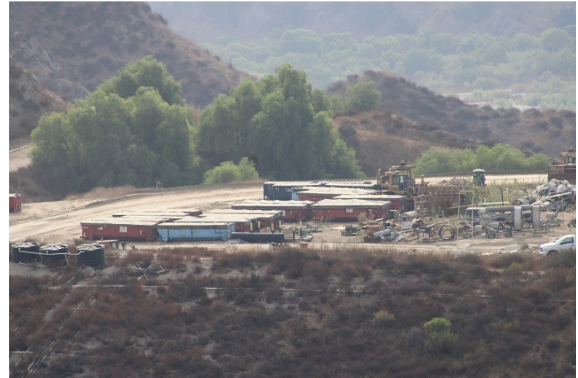
Photo 26: Cell 6 and Cell 8 Working Area: September 19, 2024
