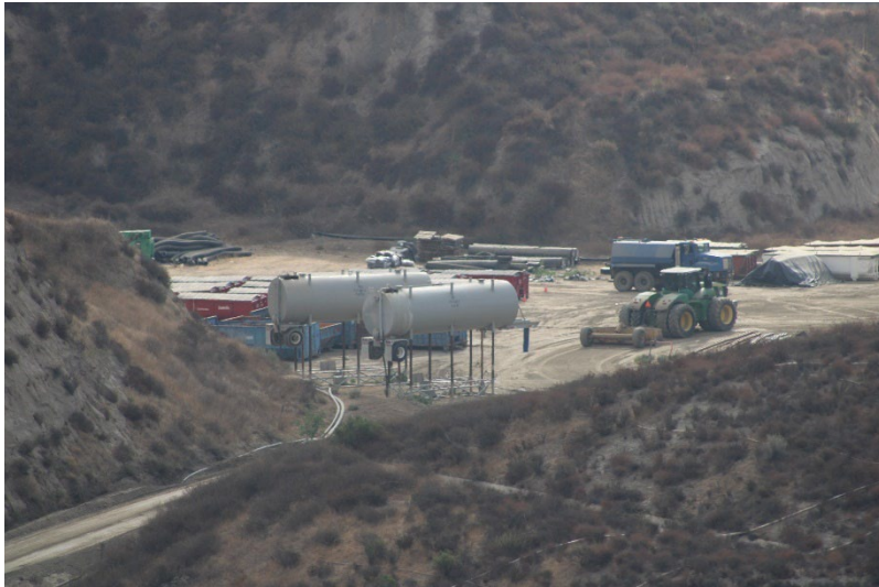
Photo 25: Cell 6 and Cell 8 Working Area: September 19, 2024
