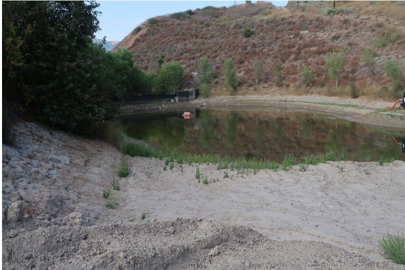
Photo 65: South Terminal and Catch Basins: July 24, 2024
