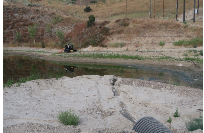
Photo 66: South Terminal and Catch Basins: July 24, 2024
