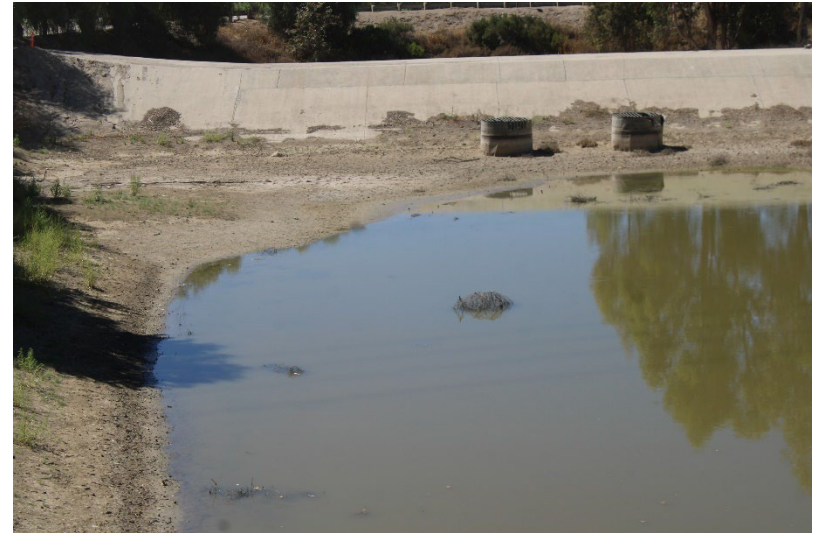
Photo 78: South Terminal and Catch Basins: August 21, 2024
