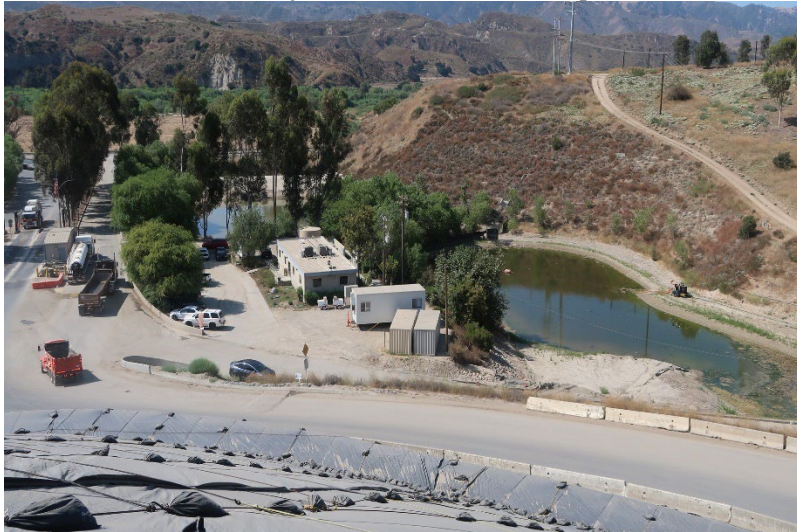
Photo 147: Maintenance and Admin Buildings: July 24, 2024
