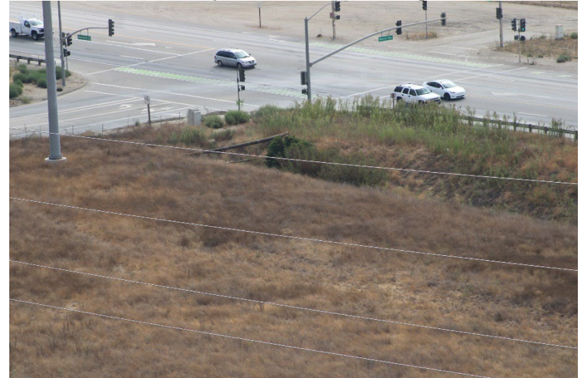
Photo 144: Wolcott Way Entrance Facilities: September 19, 2024
