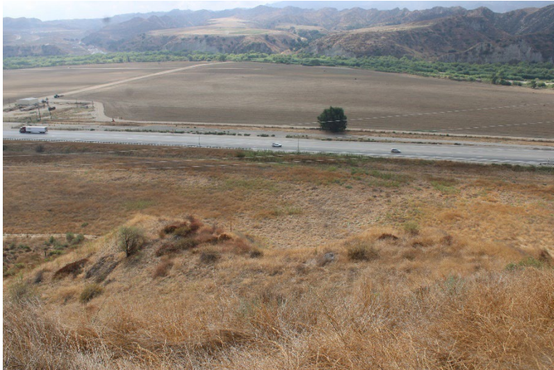
Photo 141: Wolcott Way Entrance Facilities: September 19, 2024
