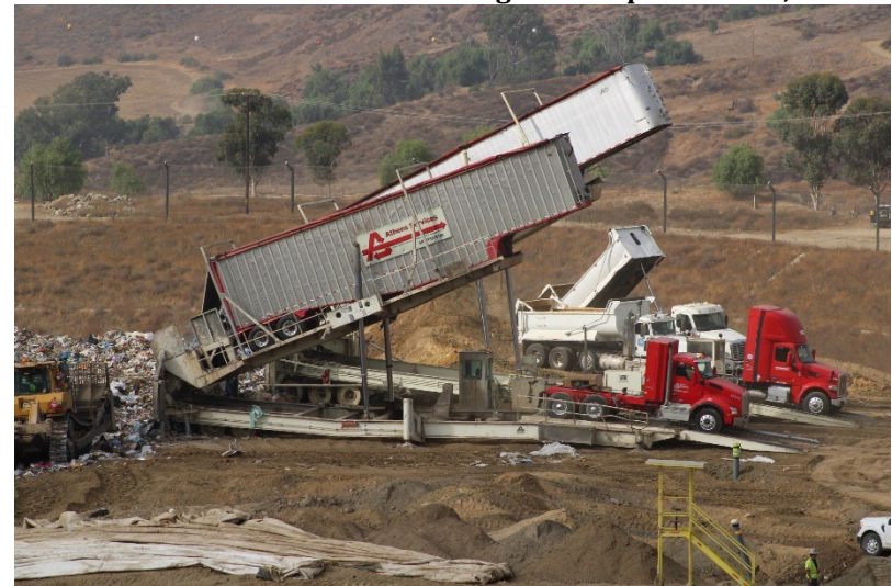
Photo 24: Cell 6 and Cell 8 Working Area: September 19, 2024
