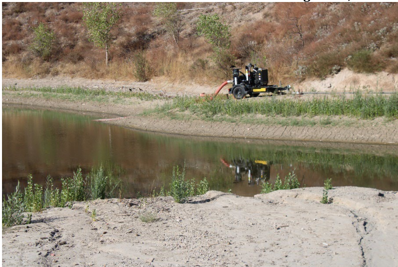
Photo 75: South Terminal and Catch Basins: August 21, 2024
