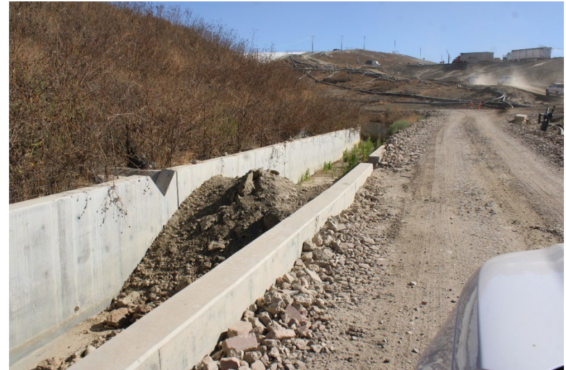
Photo 114: Landfill Perimeter Drainage Channel: August 21, 2024
