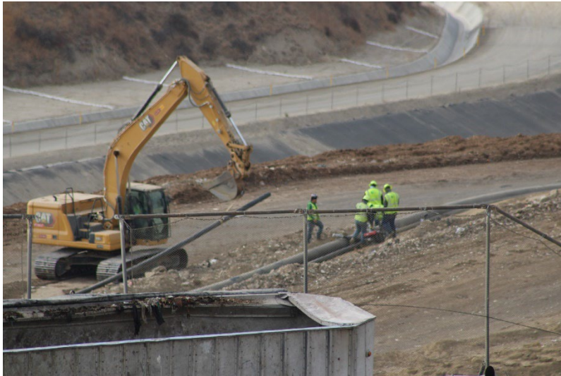
Photo 29: Cell 6 and Cell 8 Working Area: September 19, 2024
