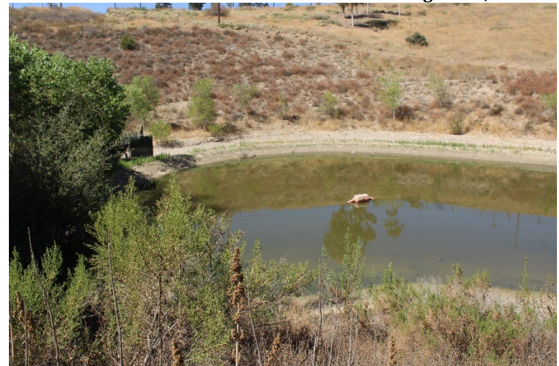
Photo 80: South Terminal and Catch Basins: August 21, 2024
