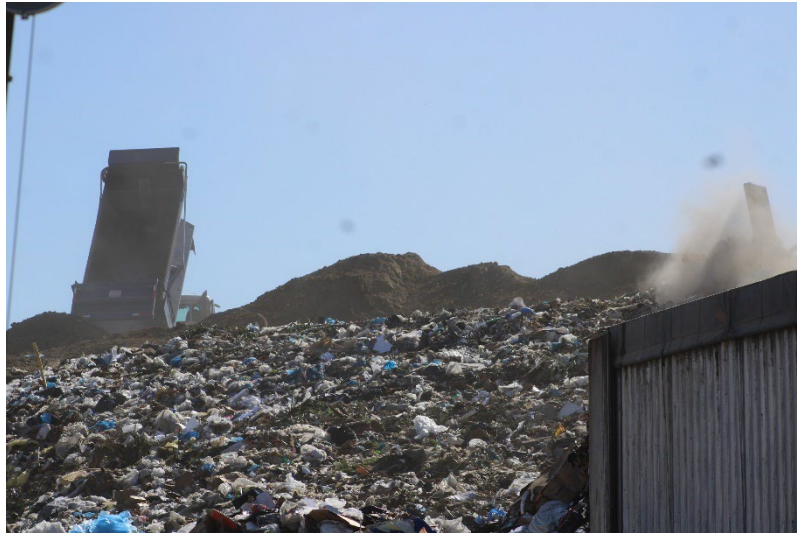
Photo 9: Top Deck Working Area: August 21, 2024
