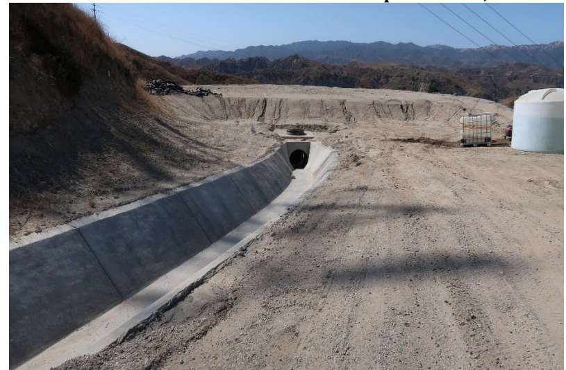
Photo 112: Landfill Perimeter Drainage Channel: July 24, 2024
