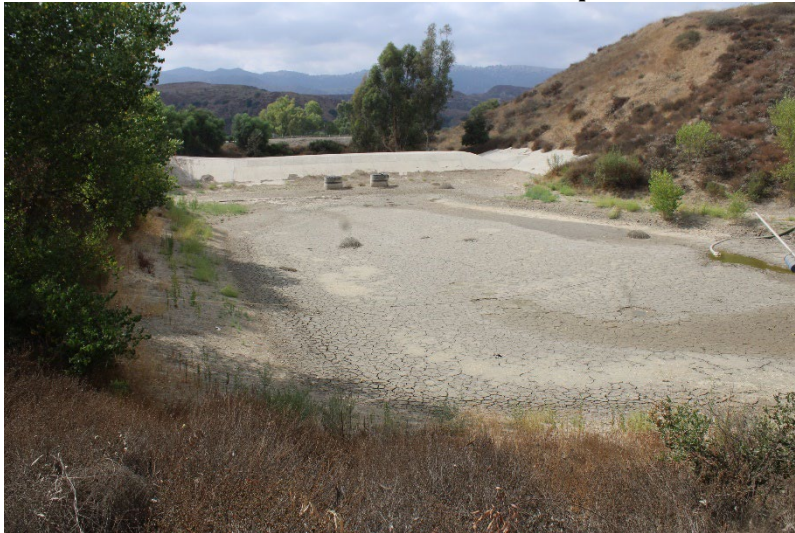
Photo 87: South Terminal and Catch Basins: September 19, 2024
