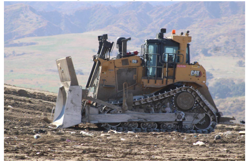
Photo 12: Top Deck Working Area: August 21, 2024
