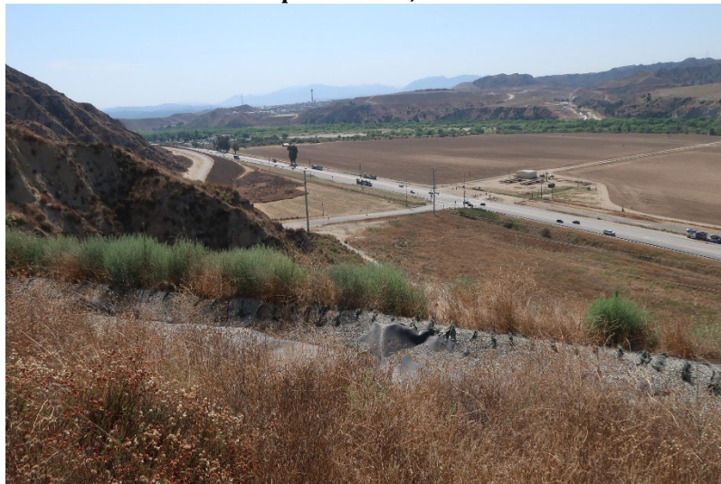
Photo 135: Wolcott Way Entrance Facilities: July 24, 2024
