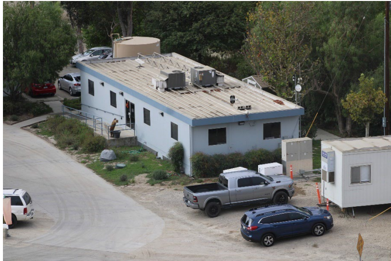
Photo 149: Maintenance and Admin Buildings: September 19, 2024
