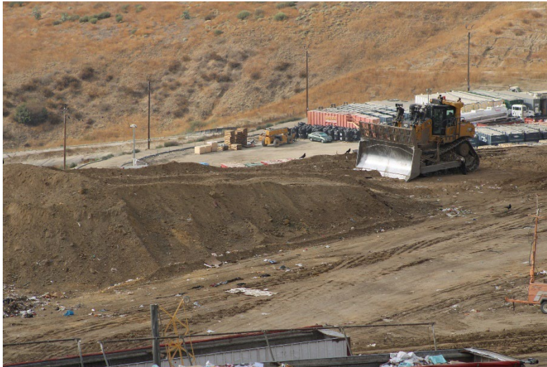
Photo 21: Cell 6 and Cell 8 Working Area: September 19, 2024
