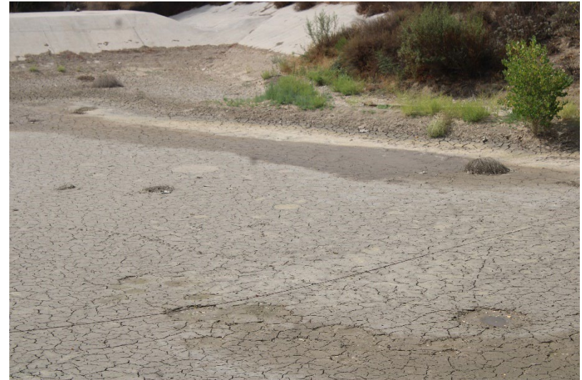
Photo 90: South Terminal and Catch Basins: September 19, 2024
