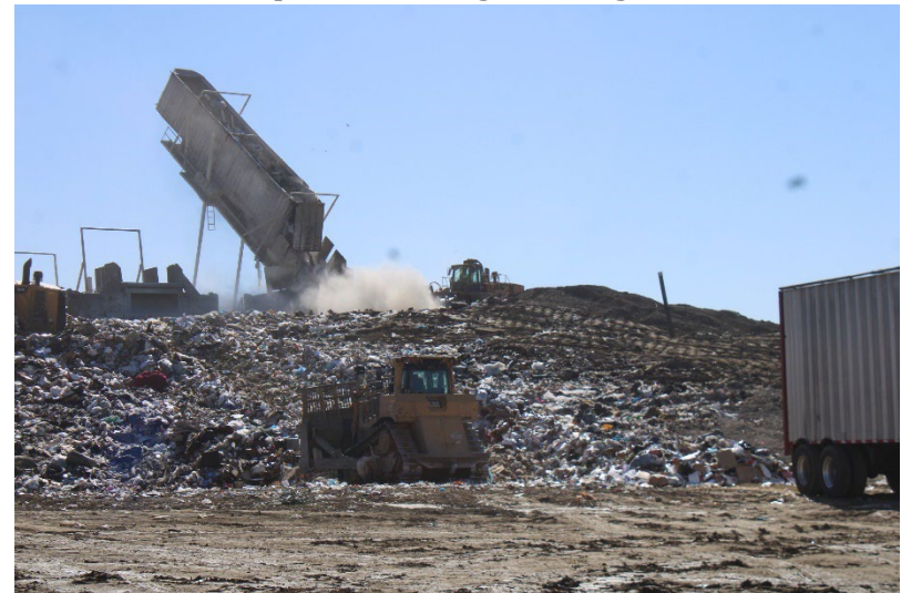
Photo 4: Top Deck Working Area: August 21, 2024
