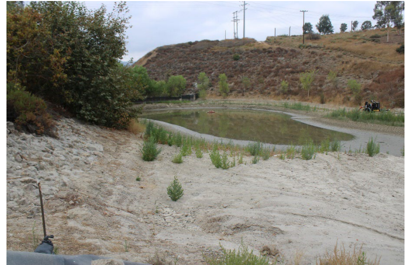
Photo 82: South Terminal and Catch Basins: September 19, 2024
