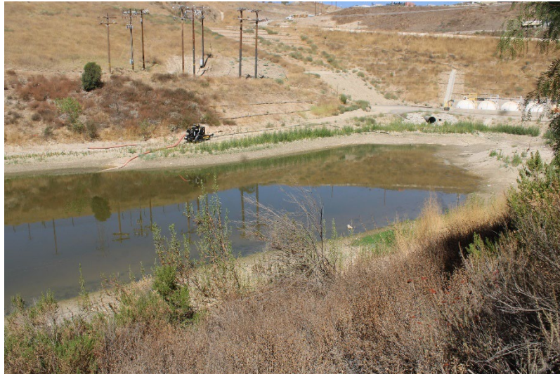
Photo 81: South Terminal and Catch Basins: August 21, 2024
