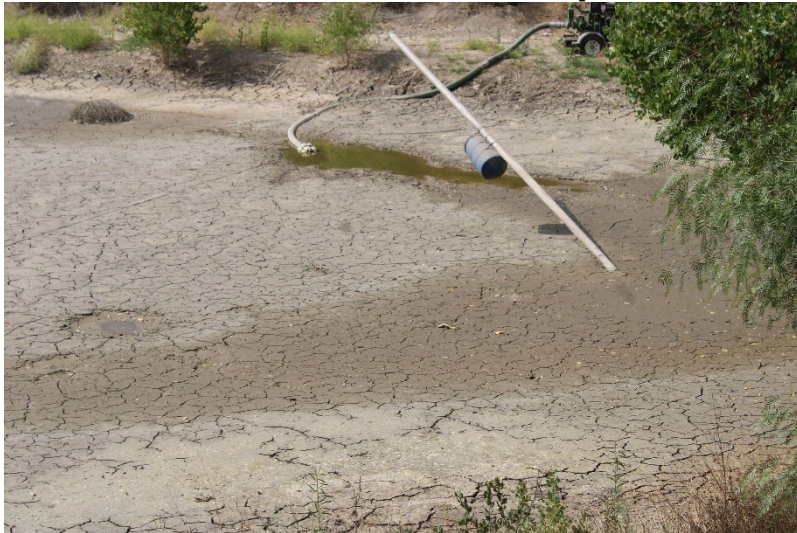
Photo 91: South Terminal and Catch Basins: September 19, 2024
