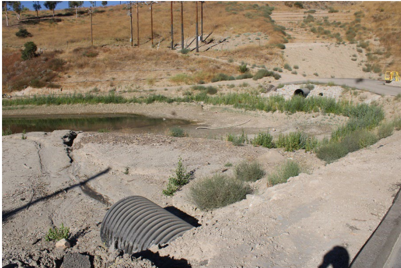
Photo 73: South Terminal and Catch Basins: August 21, 2024
