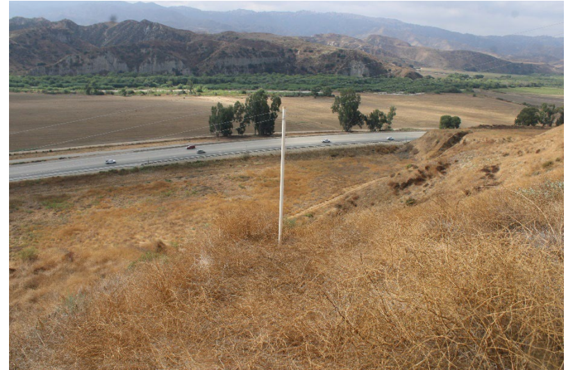
Photo 142: Wolcott Way Entrance Facilities: September 19, 2024
