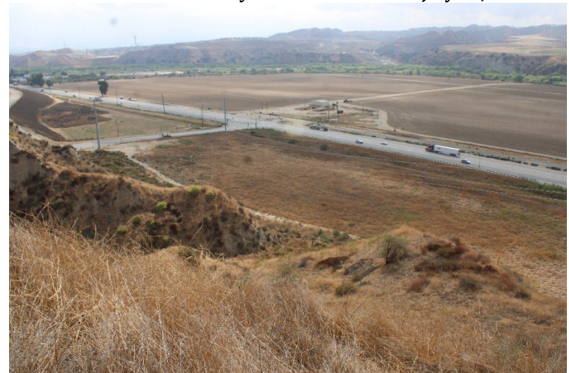
Photo 140: Wolcott Way Entrance Facilities: September 19, 2024
