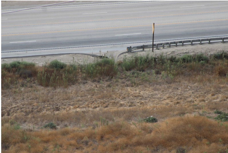
Photo 145: Wolcott Way Entrance Facilities: September 19, 2024
