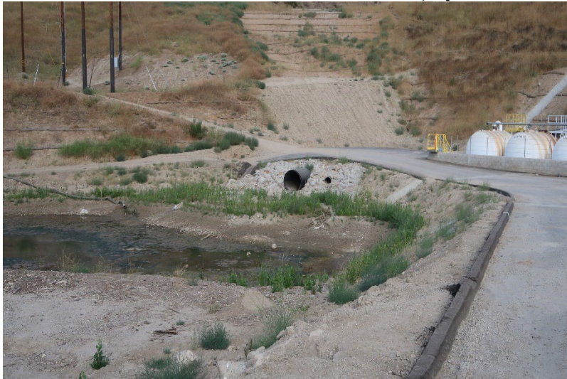
Photo 67: South Terminal and Catch Basins: July 24, 2024
