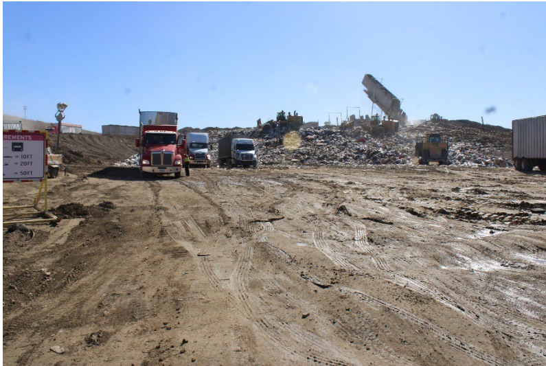
Photo 1: Top Deck Working Area: August 21, 2024
