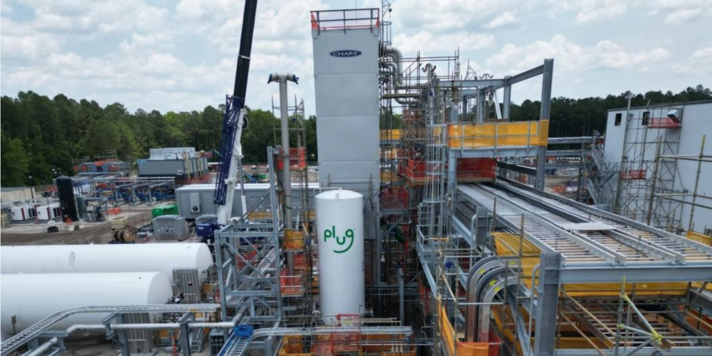
Photo of a green hydrogen production facility in Woodbine, Georgia (15,000 kg/day of liquid hydrogen)
