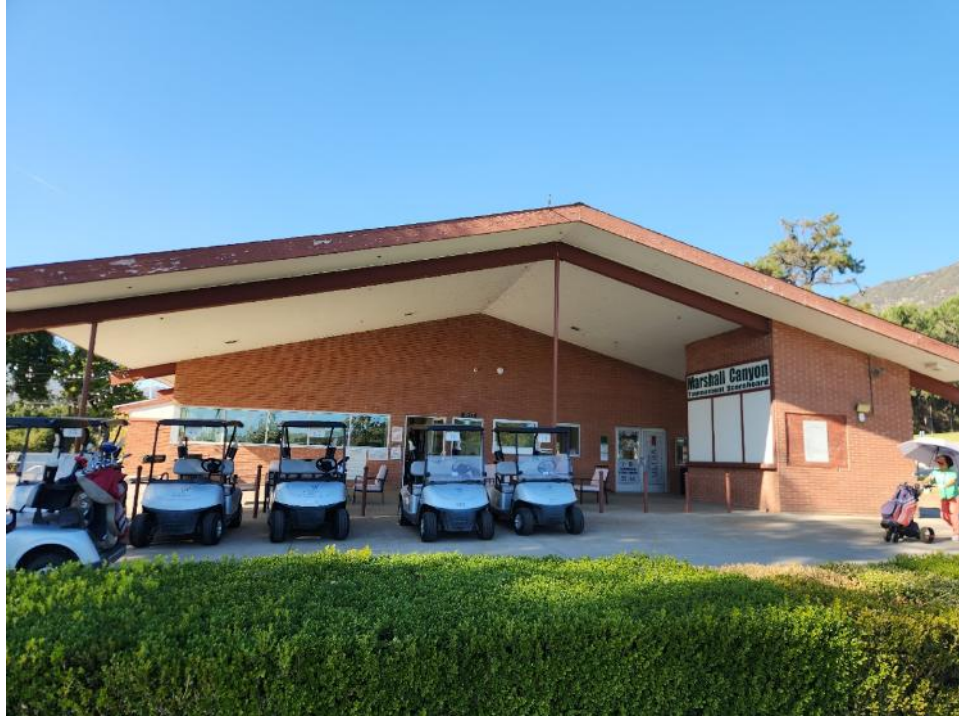
Figure 4.5.8-5. Marshall Canyon Golf Clubhouse (southeast elevation)
