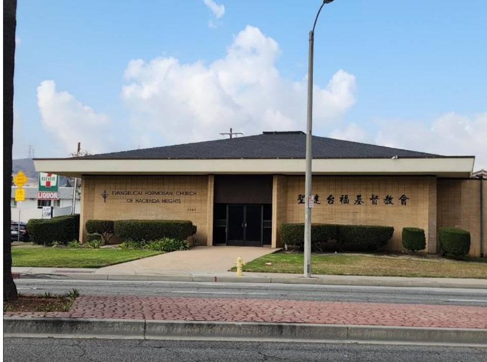
Figure 4.5.7-4. Evangelical Formosan Church of Hacienda Heights (built 1969)
