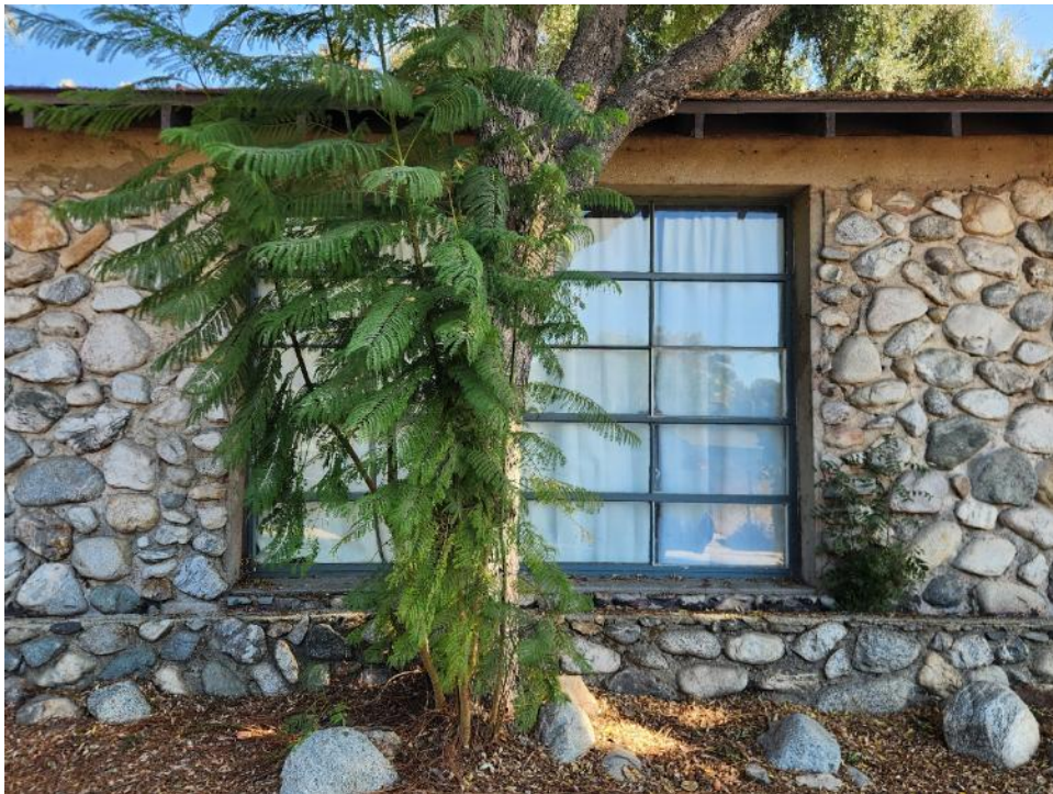
Figure 4.5.1-9. 4436 N Towne Avenue (built 1910)
