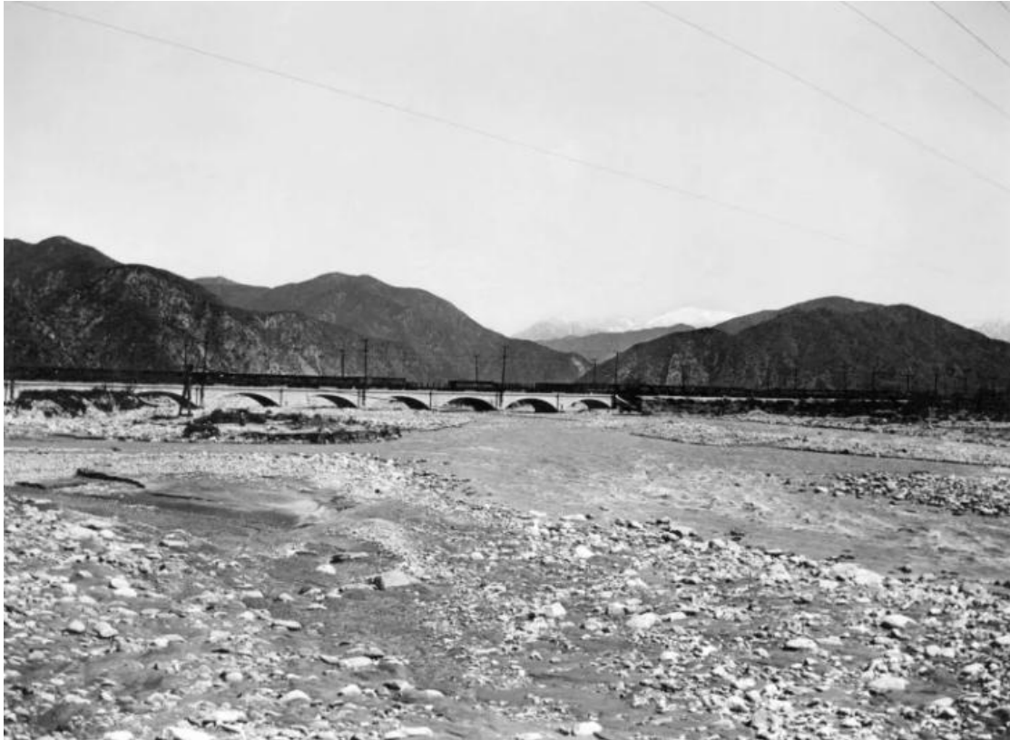
Figure 4.5.4-3. Atchison, Topeka, and Santa Fe Railroad Bridge Crossing the San Gabriel River (early 1990s) 125
