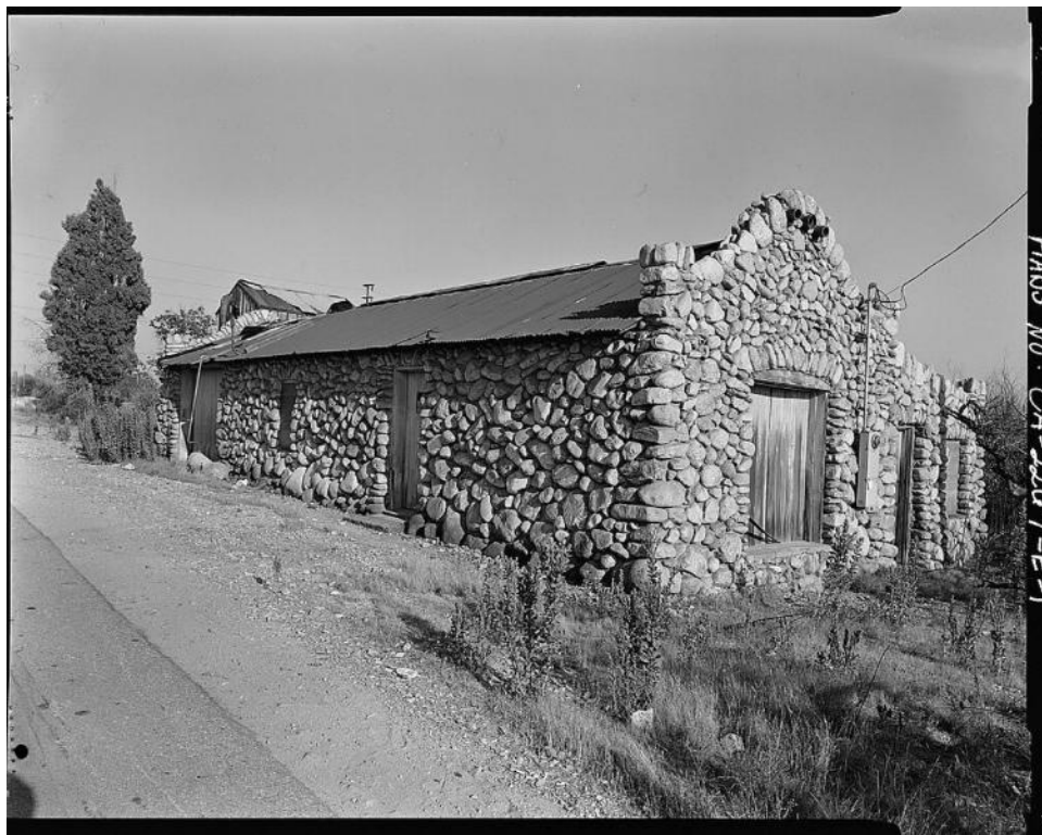
Figure 4.5.1-7. Pitzer Ranch, Pumphouse (c. 1933) 38
