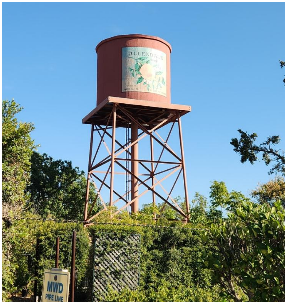
Figure 4.5.1-10. Water Tower at Foothill Blvd.
