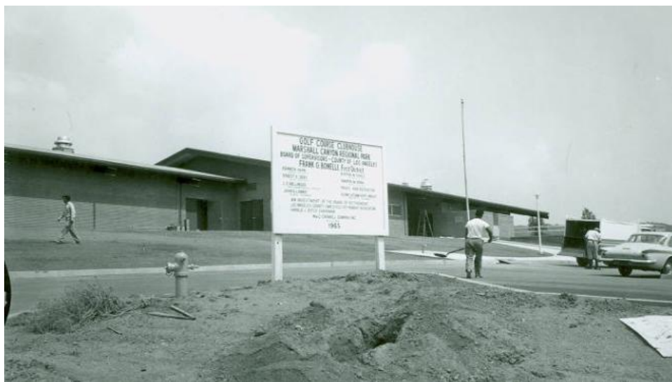
Figure 4.5.8-4. View of Construction of Marshall Canyon Golf Course (1966) 220
