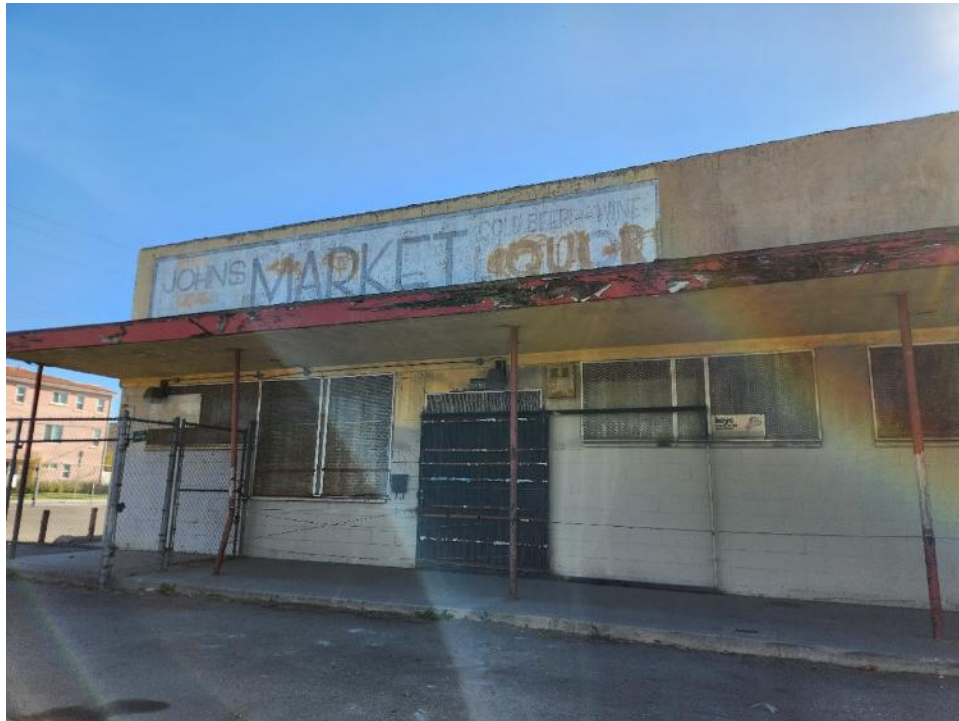
Figure 4.5.6-6. 15978 Francisquito Avenue, Valinda (built 1952)
