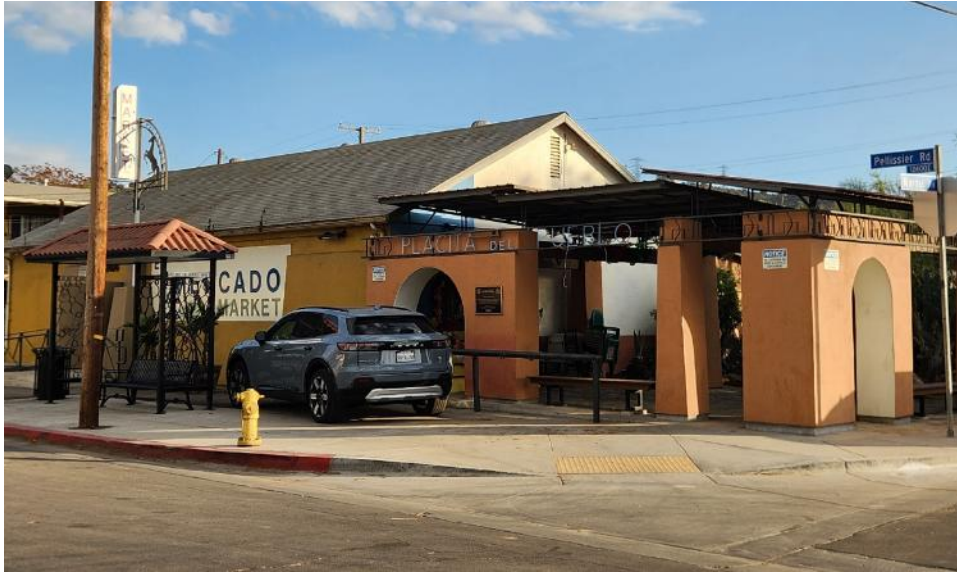
Figure 4.5.6-4. 12404 Pellissier Road, Pellissier Village (built 1956)
