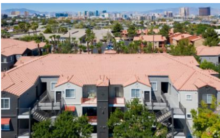
This multifamily development has a hipped roof with cross gables along the primary façade.
