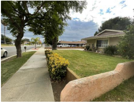
This single-family home in Charter Oak incorporates landscaping along the property line to further separate the sidewalk from the front yard setback
