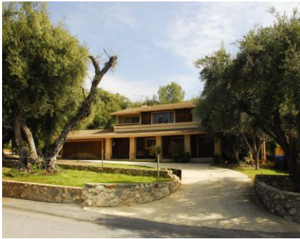
Two-story single-family residential home in North Claremont
