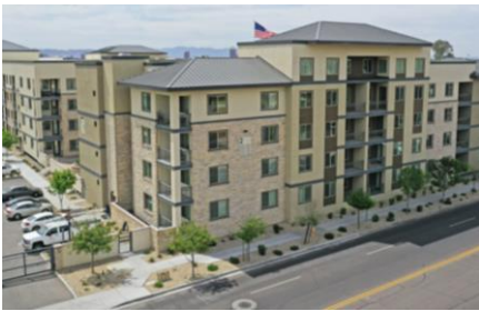
The above multifamily residential development alternates between flat and hipped roofs, as well as changes in roof height, to add scale to the overall building mass.
