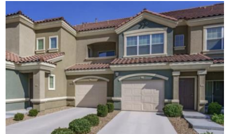
The townhomes above recess and project the entrances and garages to create a modulated front façade.
