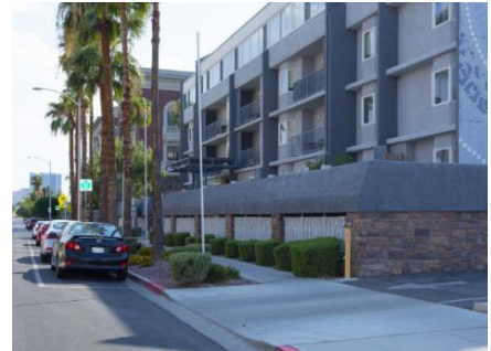
Decorative metal grills along the ground-level, sidewalk-facing façade help mask the podium parking.
