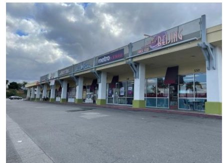
Commercial strip malls like the one shown above in Avocado Heights are common throughout the ESGV
