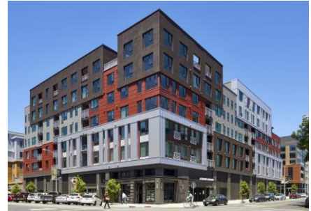
This multifamily residential development uses color to distinguish the base, middle, and top of the structure and incorporates an overhang over the building entrance.
