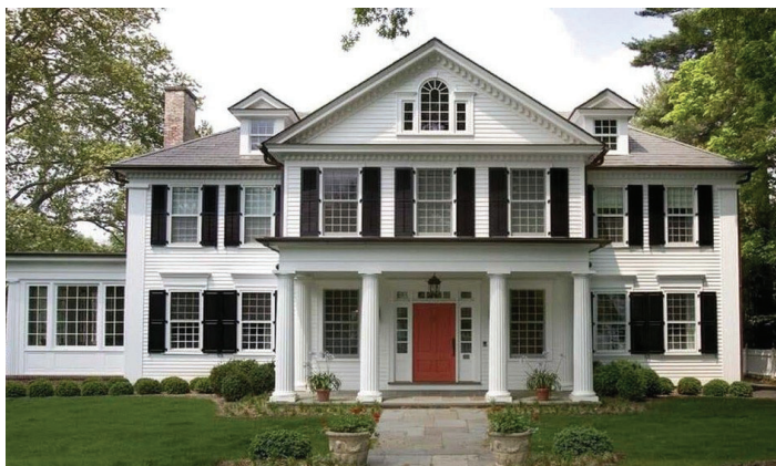
Front facade with "Doric" scalloped columns.
