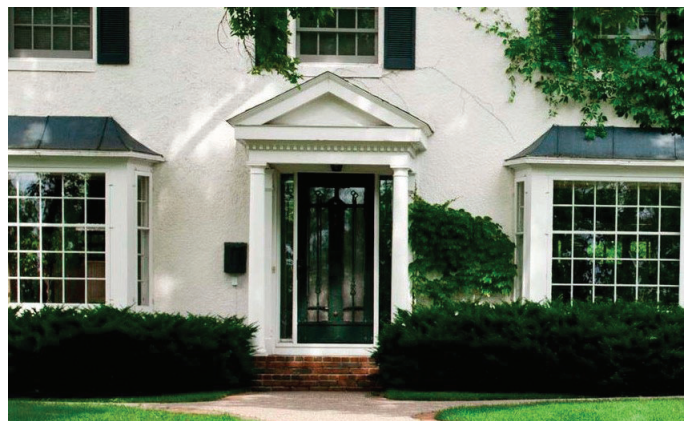
Centralized front door with "pediment" above.
