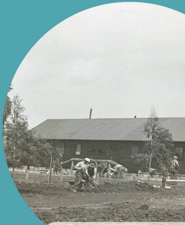
Alondra Park under construction, 1935
