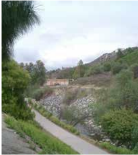
Example photo of multi-use path in a drainage channel.
