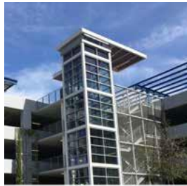
Example of photo illustrating a parking structure with architectural and screening features.
