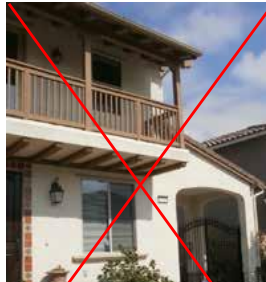
Example photo illustrating a balcony on the upper story to provide "eyes on the street."
