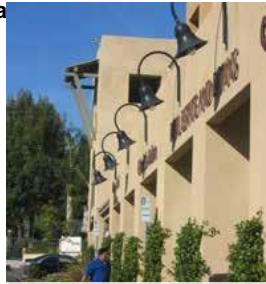
Example of photo illustrating outdoor lighting located at all building entryways
