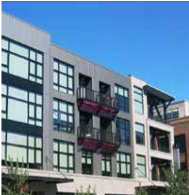
Example of a building façade with a distinct base and varying treatment to breakup building mass.
