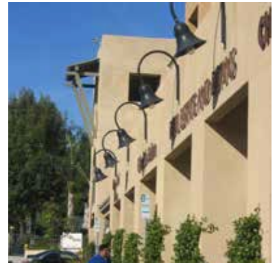
Example of a clearly defined and distinct building entrances.
