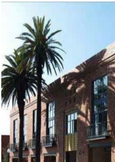
Example of a building aligned with the right-of-way.
