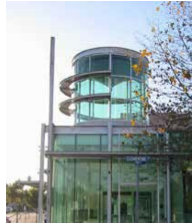
Example of a corner architectural treatment.
