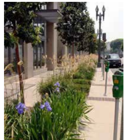
Example of a pervious surfaces used to manage stormwater.
