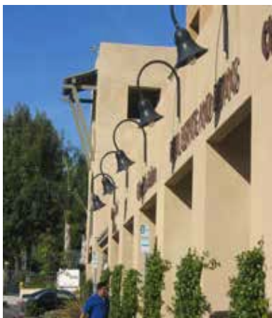
Example of outdoor lighting located at all building entryways.
