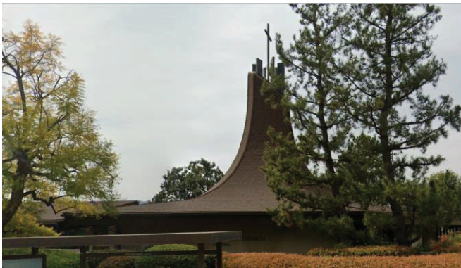
First Presbyterian Church 2775 Lincoln Avenue AIN: 5828009013 Date of Construction: 1967
