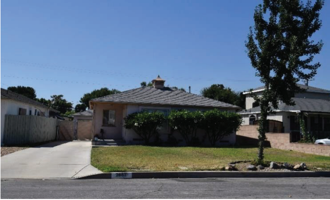
2881 Ashmont Avenue, Arcadia AIN: 8511023064
