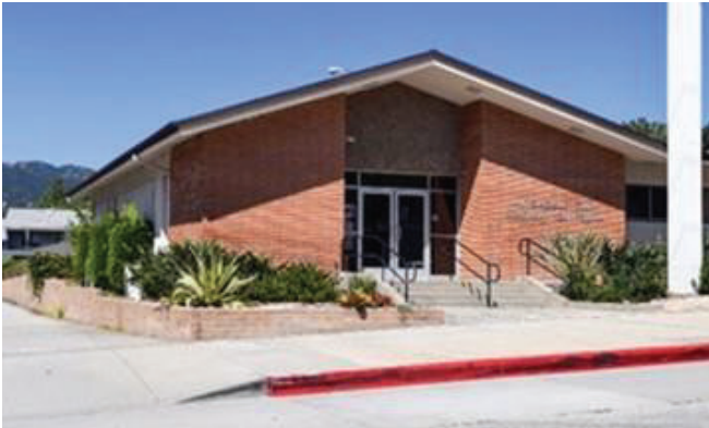
2112 Montrose Avenue, La Crescenta-Montrose AIN: 5807008031 Date of Construction: 1964
