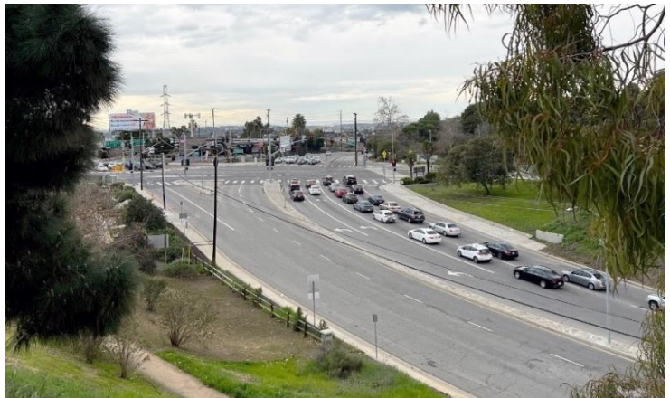
Photo of five-way intersection at La Brea Ave., Stocker St. and Overhill Dr. (LA County Planning)
