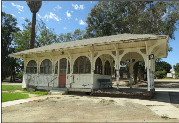
West Los Angeles VA Building 66, Row 10 (Historic Preservation Solutions LLC)
