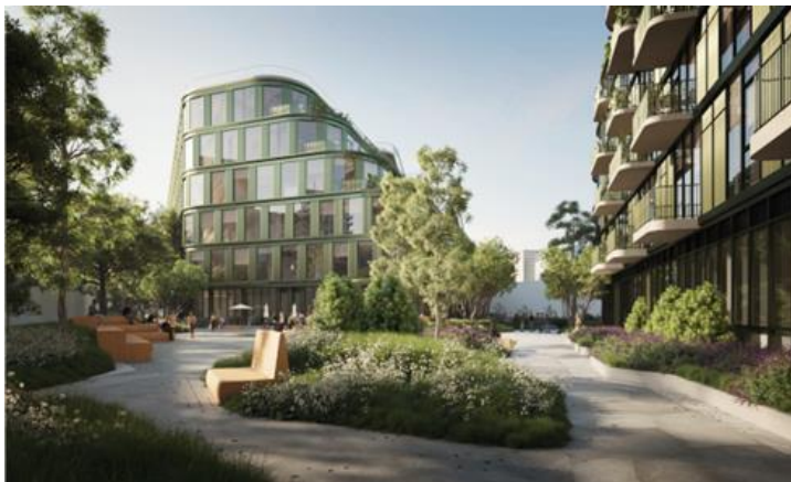
An example of housing currently under construction near the E-line. (SHoP Architects)
