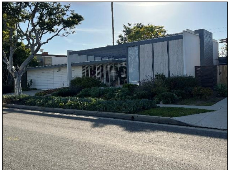
Linnell Residence, 6443 S. Halm Avenue (Historic Resources Group)
