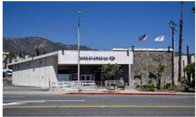
3141 Foothill Blvd, La Crescenta-Montrose AIN: 5802010002 Date of Construction: 1962
