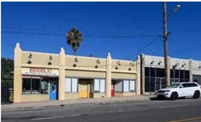
2591 Fair Oaks Ave, Altadena AIN: 5835011002 Date of Construction 1930
