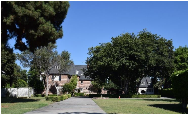
2232 California Avenue, Monrovia AIN: 8521004056
