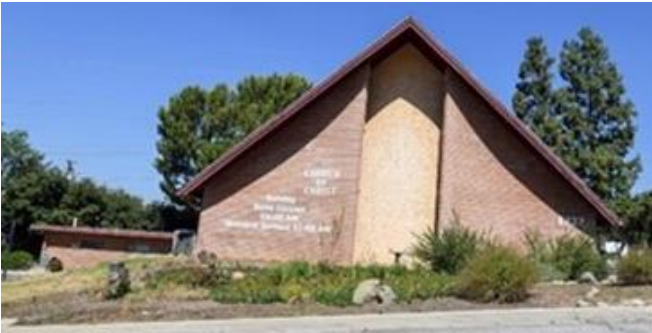
Unite Church 1727 Kinneloa Mesa Canyon Road AIN: 5860013012 Date of Construction: 1970
