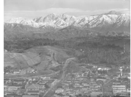
Construction of Pasadena Freeway, 1962 (Source: UCLA Libraries)
