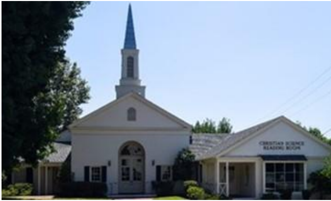
Christian Science Church and Reading Room 942 E. Altadena Drive AIN: 5845001001 Date of Construction: 1949
