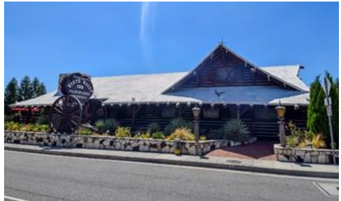
7247 Rosemead Blvd, East San Gabriel AIN: 5379006038 Date of Construction 1965
