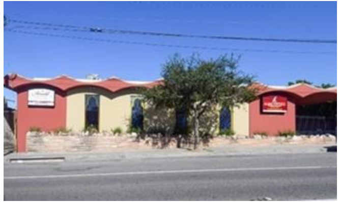
Hillside Tabernacle City of Faith Arnold Family Funeral Home 2561 N. Fair Oaks Avenue AIN: 58350110250 Date of Construction: 1963
