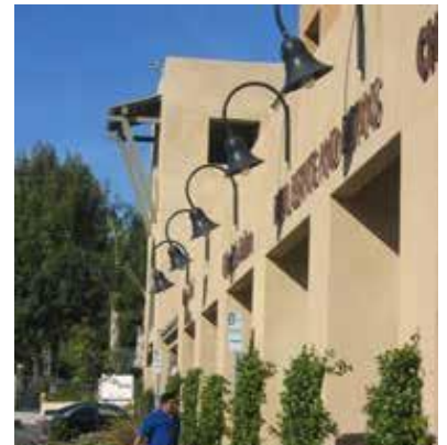
Example photo illustrating clearly defined and distinct building entrances.
