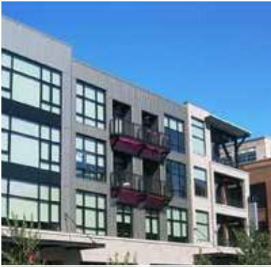
Example photo illustrating building façade with a distinct base and varying treatment to breakup building mass.
