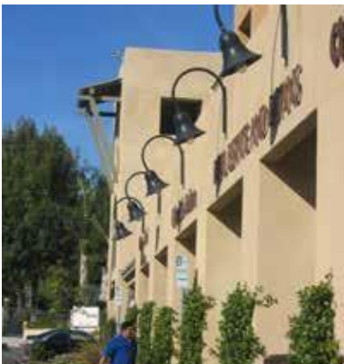
Example photo illustrating outdoor lighting located at all building entryways.
