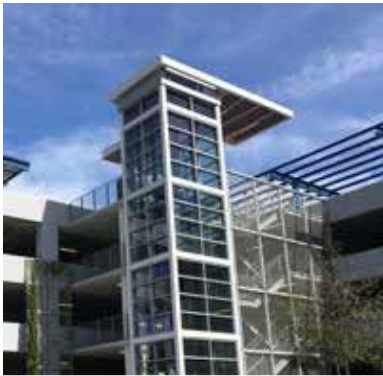
Example photo illustrating a parking structure with architectural and screening features.
