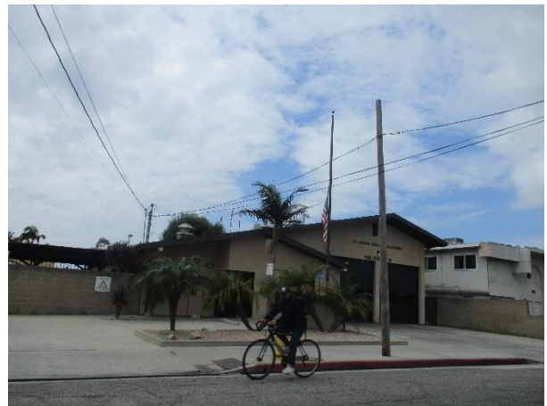
Fire Station 18 in Lennox
