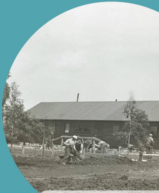
Alondra Park under construction, 1935
