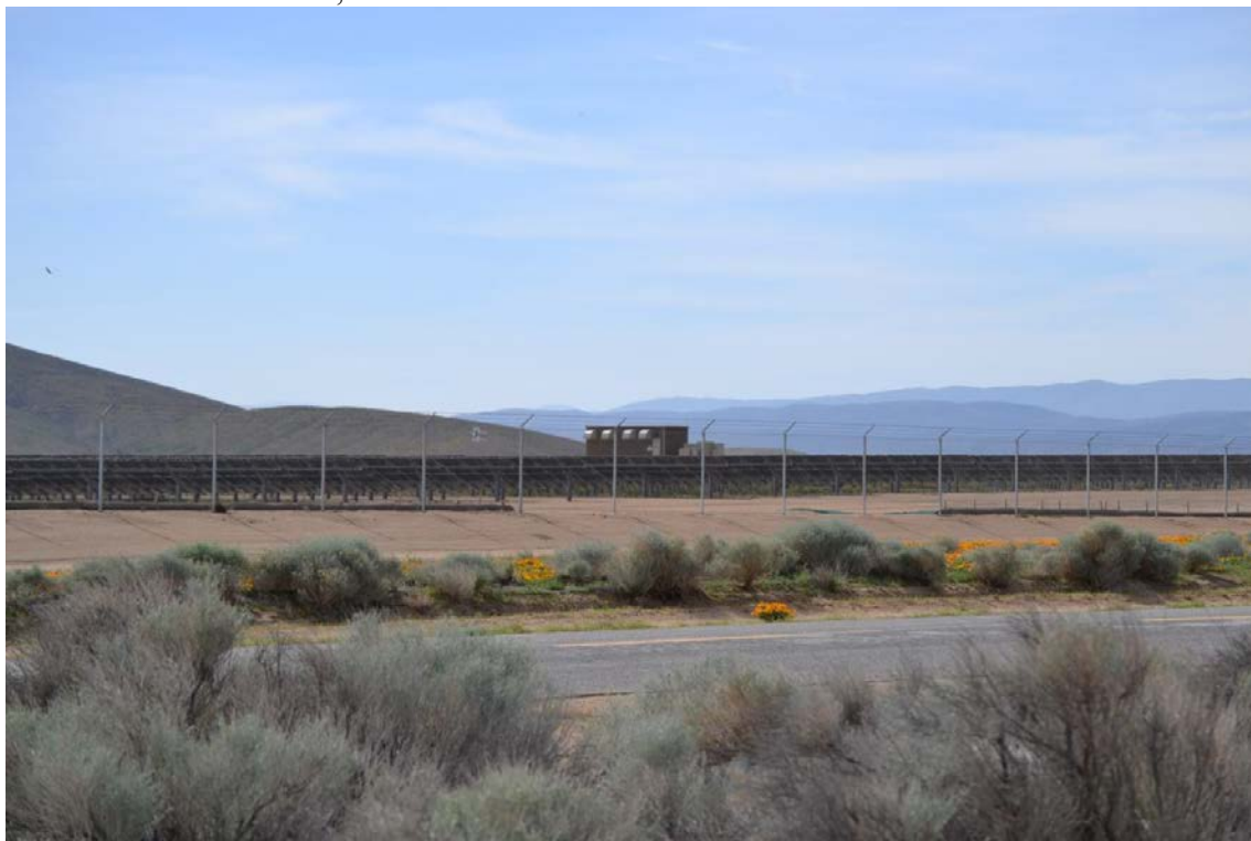
After the construction of AVSR 1, note the chainlink and barbed wire fencing, impermeable to ground dwelling wildlife.
