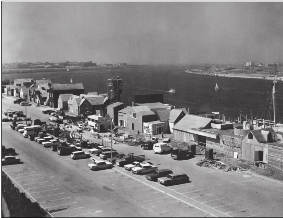
Fisherman's Village under construction 1969. Los Angeles Public Library
