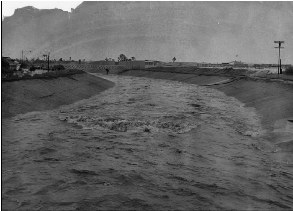
Ballona Creek Flood Control Channel 1958. Los Angeles Public Library
