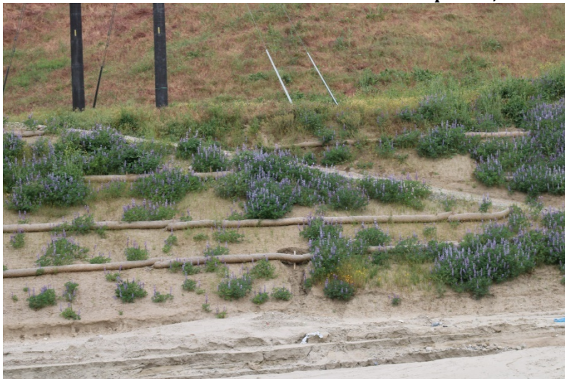
Photo 127: South Terminal and Catch Basins: April 25, 2023
