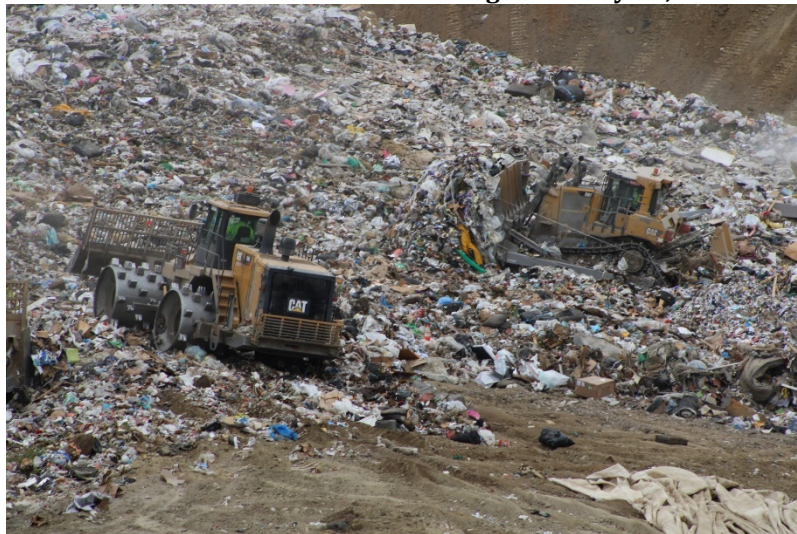
Photo 63: Cell 6 and Cell 8 Working Area: May 25, 2023
