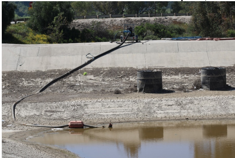
Photo 131: South Terminal and Catch Basins: April 25, 2023
