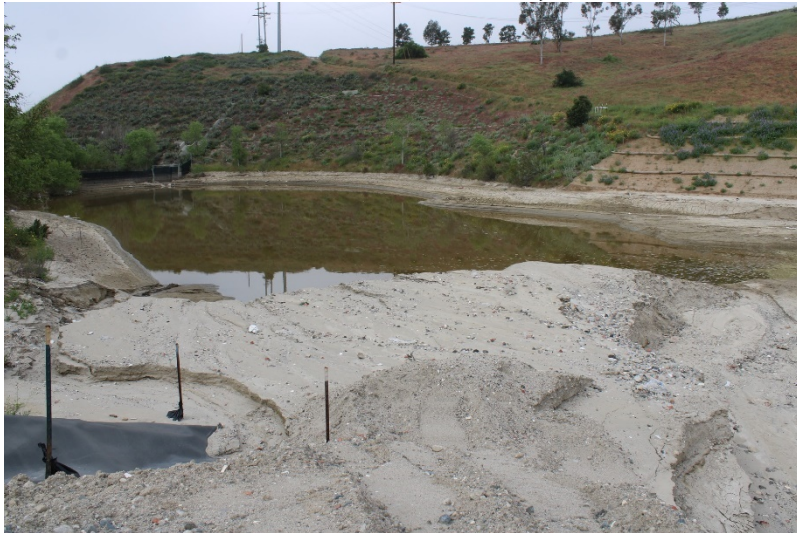
Photo 119: South Terminal and Catch Basins: April 25, 2023
