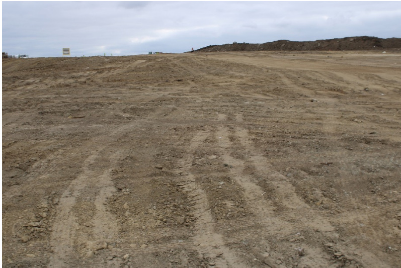
Photo 17: Top Deck Working Area: May 25, 2023
