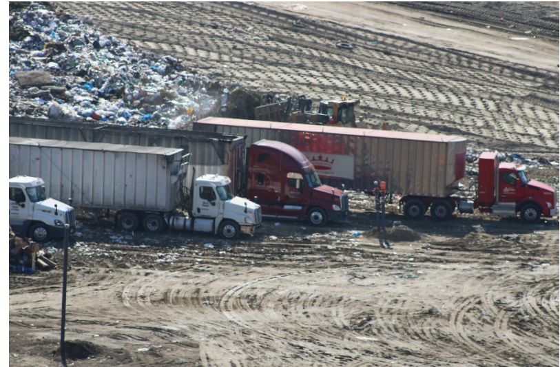
Photo 86: Cell 6 and Cell 8 Working Area: June 14, 2023
