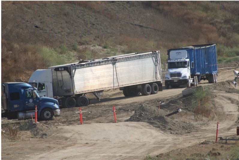
Photo 77: Cell 6 and Cell 8 Working Area: June 14, 2023
