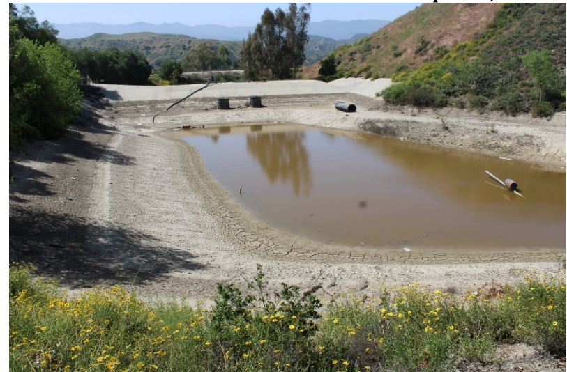
Photo 128: South Terminal and Catch Basins: April 25, 2023
