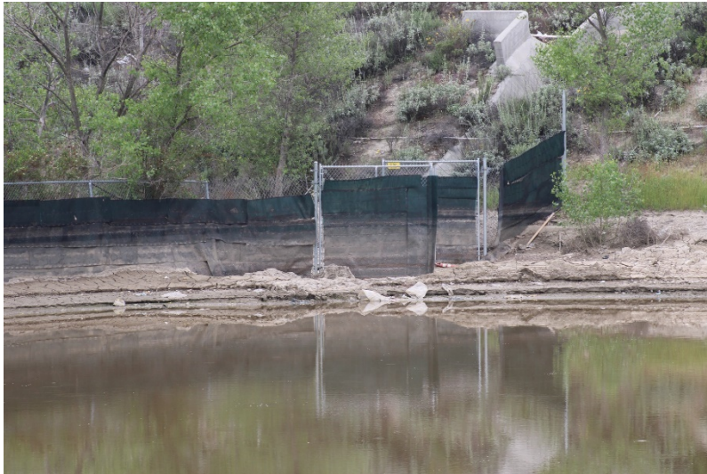
Photo 125: South Terminal and Catch Basins: April 25, 2023
