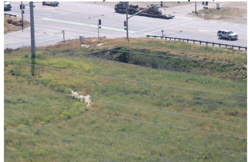
Photo 208: Wolcott Way Entrance Facilities: April 25, 2023
