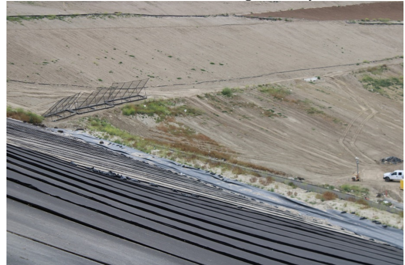
Photo 56: Cell 6 and Cell 8 Working Area: May 25, 2023
