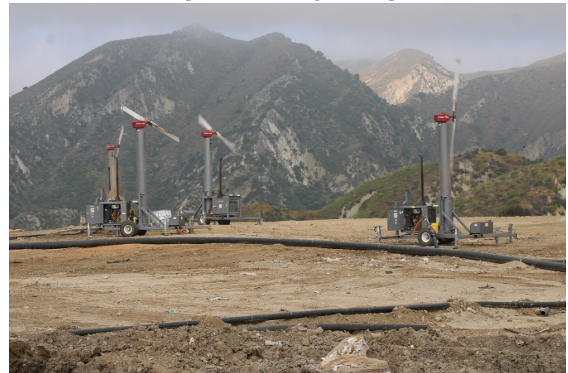
Photo 12: Top Deck Working Area: April 25, 2023
