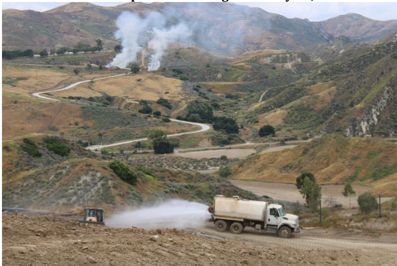
Photo 23: Top Deck Working Area: May 25, 2023
