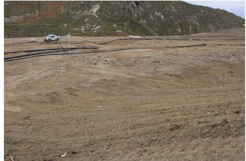
Photo 26: Top Deck Working Area: May 25, 2023
