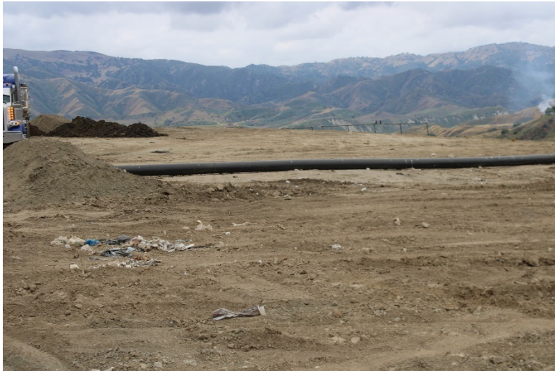
Photo 21: Top Deck Working Area: May 25, 2023
