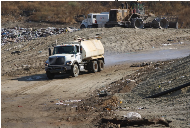
Photo 75: Cell 6 and Cell 8 Working Area: June 14, 2023
