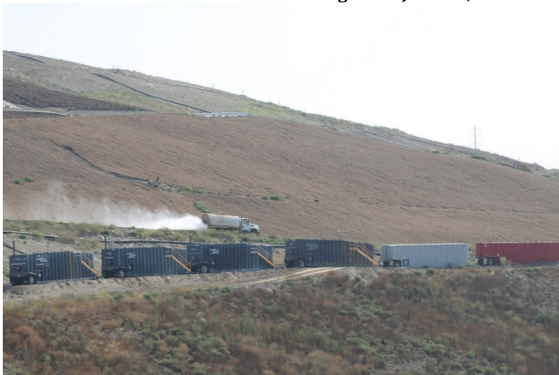
Photo 79: Cell 6 and Cell 8 Working Area: June 14, 2023
