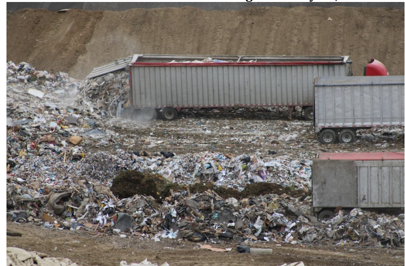
Photo 64: Cell 6 and Cell 8 Working Area: May 25, 2023
