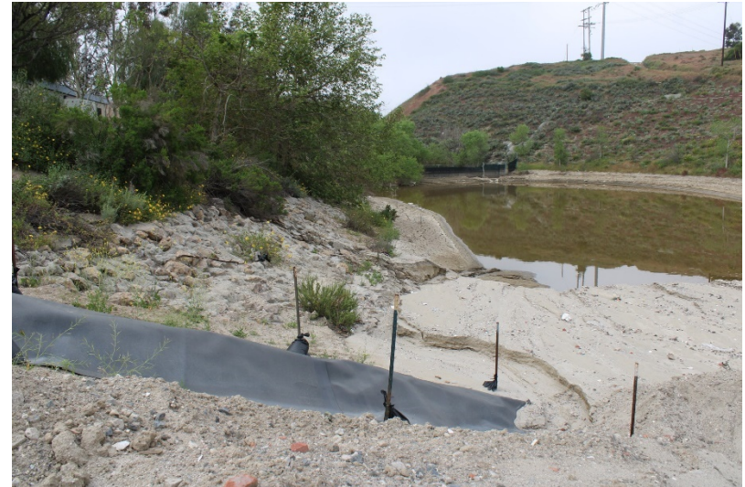
Photo 118: South Terminal and Catch Basins: April 25, 2023
