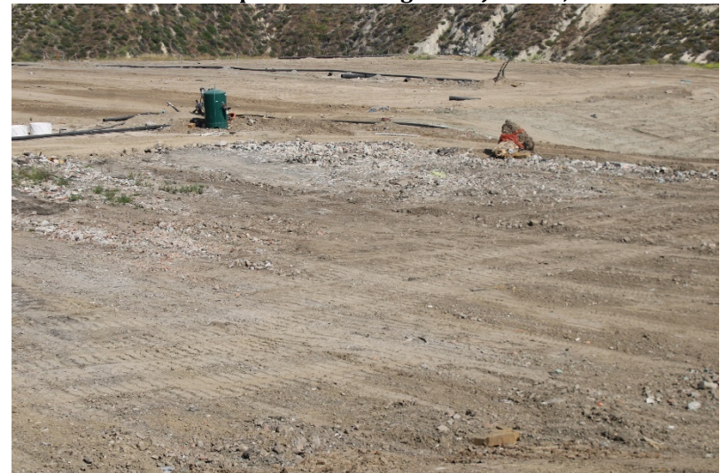
Photo 36: Top Deck Working Area: June 14, 2023
