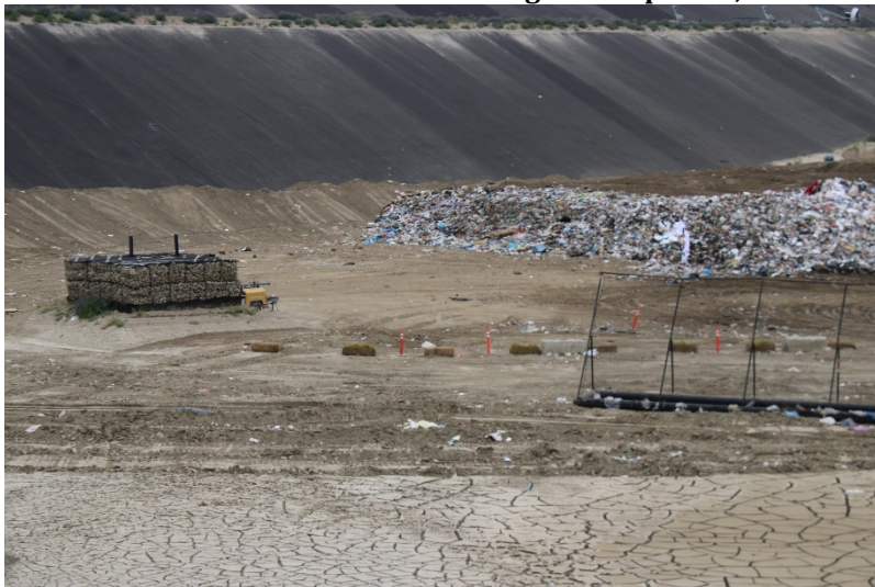
Photo 43: Cell 6 and Cell 8 Working Area: April 25, 2023
