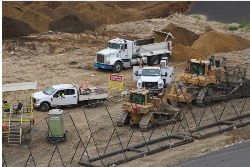
Photo 65: Cell 6 and Cell 8 Working Area: May 25, 2023
