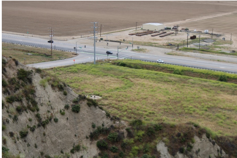
Photo 213: Wolcott Way Entrance Facilities: May 25, 2023
