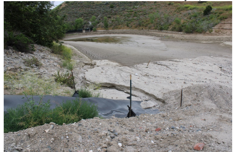
Photo 144: South Terminal and Catch Basins: May 25, 2023
