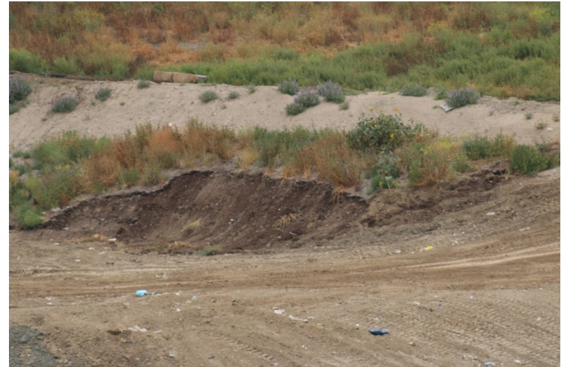
Photo 50: Cell 6 and Cell 8 Working Area: April 25, 2023
