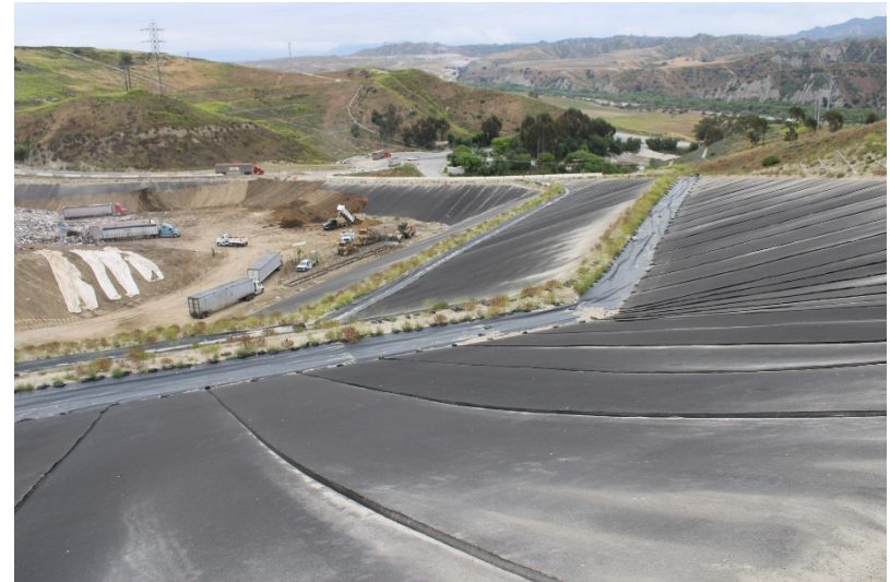
Photo 54: Cell 6 and Cell 8 Working Area: May 25, 2023
