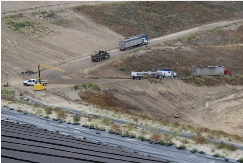
Photo 57: Cell 6 and Cell 8 Working Area: May 25, 2023
