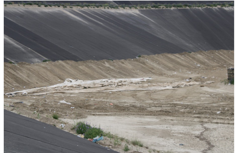
Photo 42: Cell 6 and Cell 8 Working Area: April 25, 2023
