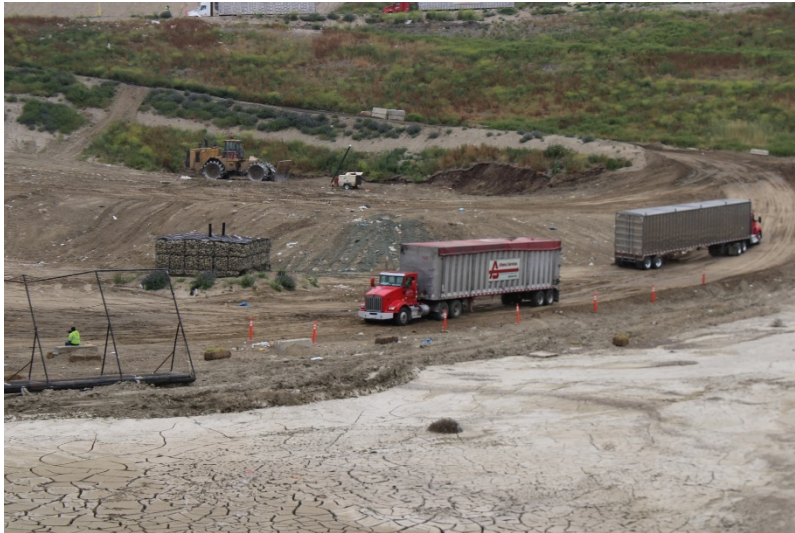
Photo 45: Cell 6 and Cell 8 Working Area: April 25, 2023
