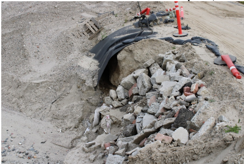
Photo 123: South Terminal and Catch Basins: April 25, 2023
