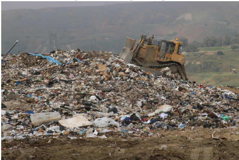
Photo 11: Top Deck Working Area: April 25, 2023
