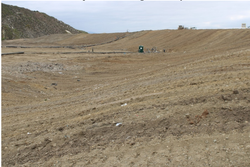
Photo 27: Top Deck Working Area: May 25, 2023
