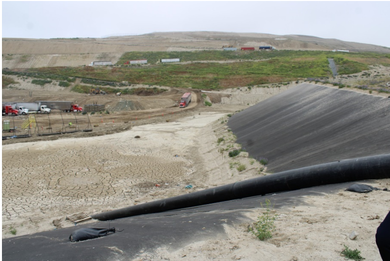
Photo 41: Cell 6 and Cell 8 Working Area: April 25, 2023
