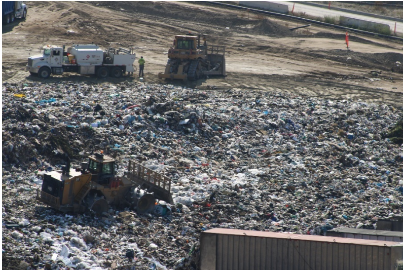
Photo 85: Cell 6 and Cell 8 Working Area: June 14, 2023
