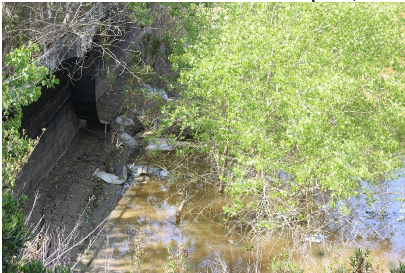
Photo 135: South Terminal and Catch Basins: April 25, 2023
