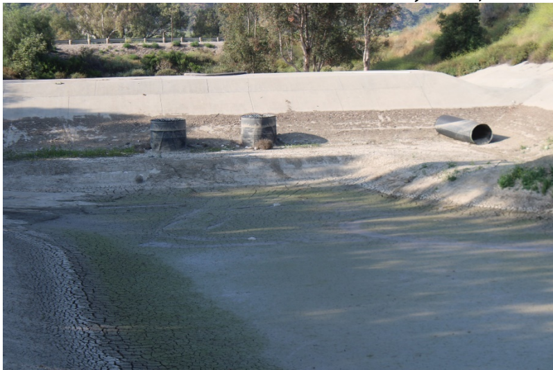
Photo 155: South Terminal and Catch Basins: June 14, 2023
