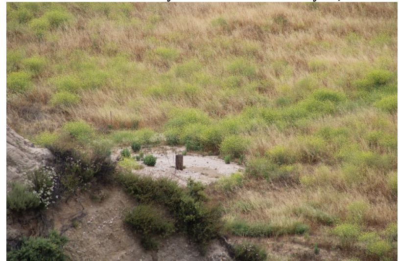
Photo 216: Wolcott Way Entrance Facilities: May 25, 2023
