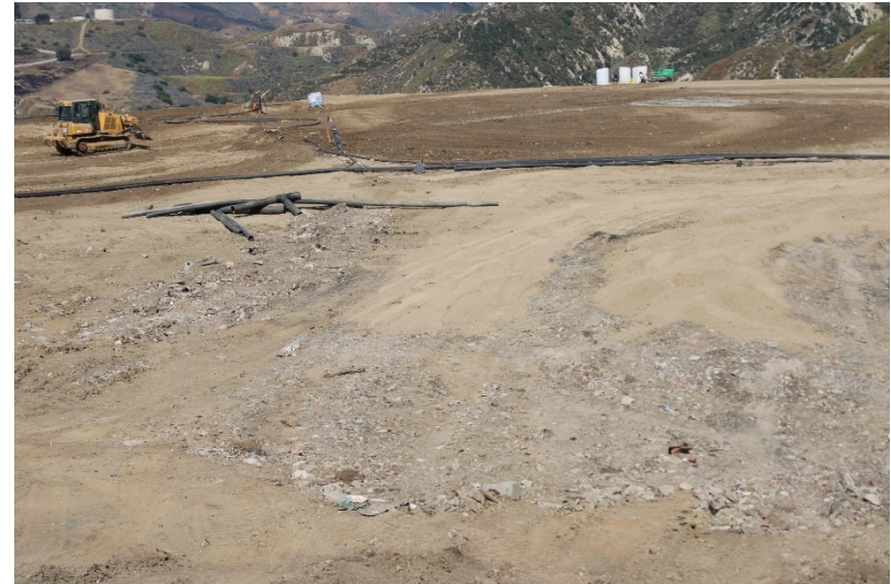
Photo 34: Top Deck Working Area: June 14, 2023
