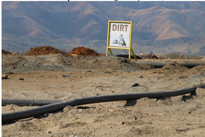
Photo 31: Top Deck Working Area: June 14, 2023
