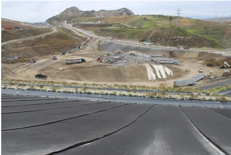
Photo 53: Cell 6 and Cell 8 Working Area: May 25, 2023
