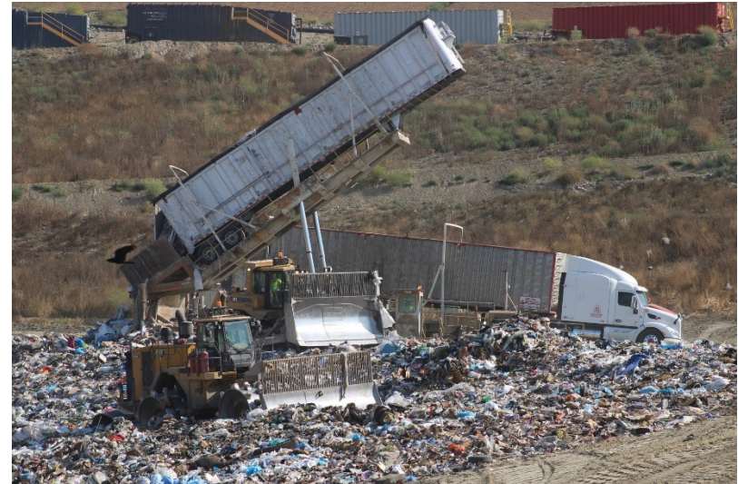
Photo 74: Cell 6 and Cell 8 Working Area: June 14, 2023
