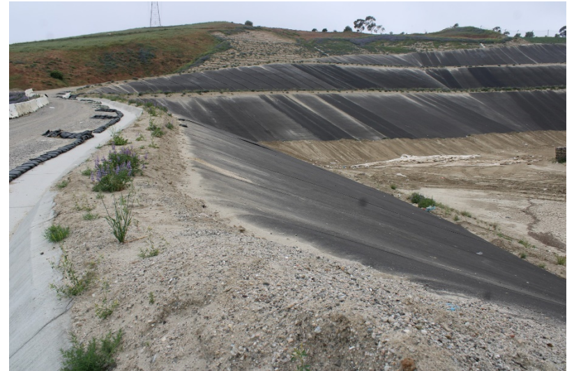
Photo 38: Cell 6 and Cell 8 Working Area: April 25, 2023
