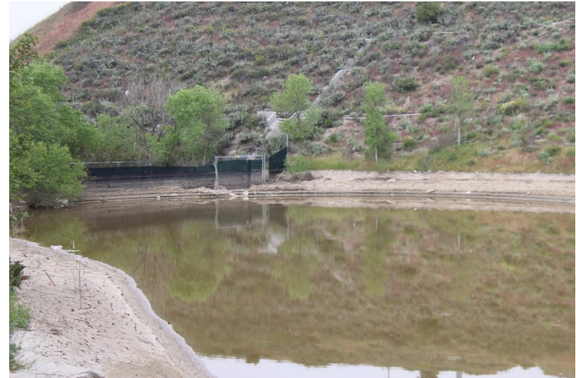
Photo 122: South Terminal and Catch Basins: April 25, 2023
