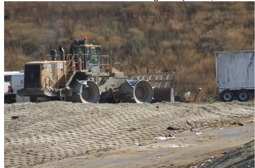
Photo 76: Cell 6 and Cell 8 Working Area: June 14, 2023
