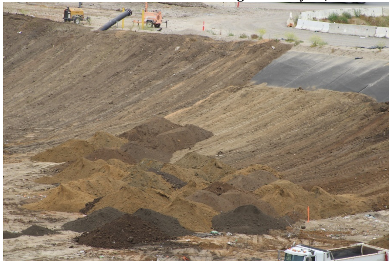
Photo 67: Cell 6 and Cell 8 Working Area: May 25, 2023
