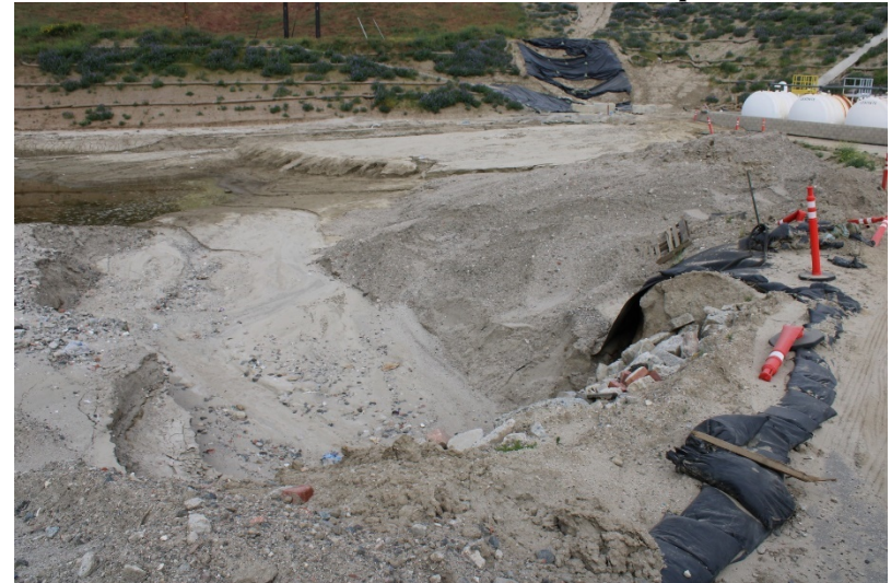
Photo 120: South Terminal and Catch Basins: April 25, 2023
