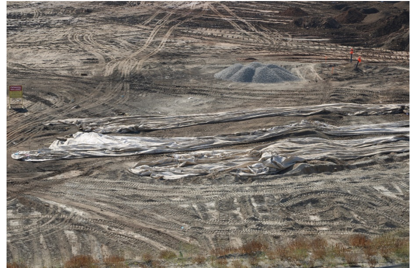
Photo 82: Cell 6 and Cell 8 Working Area: June 14, 2023
