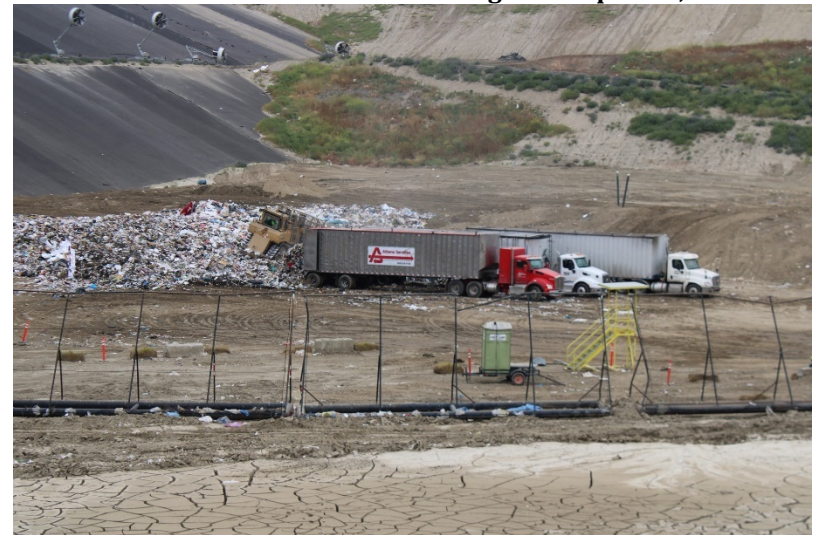
Photo 44: Cell 6 and Cell 8 Working Area: April 25, 2023
