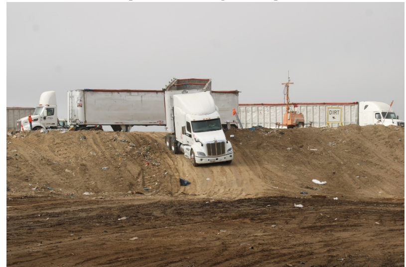
Photo 8: Top Deck Working Area: April 25, 2023
