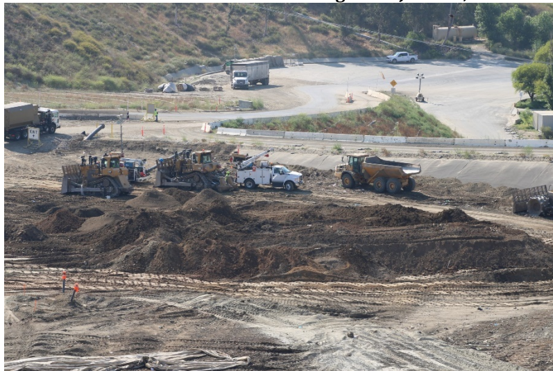
Photo 83: Cell 6 and Cell 8 Working Area: June 14, 2023
