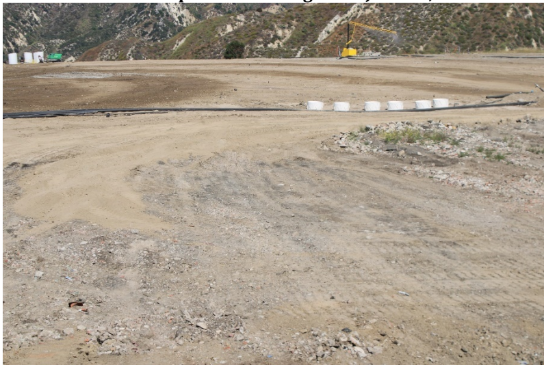
Photo 35: Top Deck Working Area: June 14, 2023
