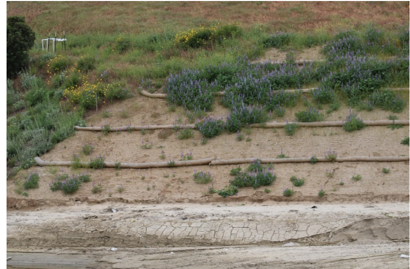
Photo 126: South Terminal and Catch Basins: April 25, 2023
