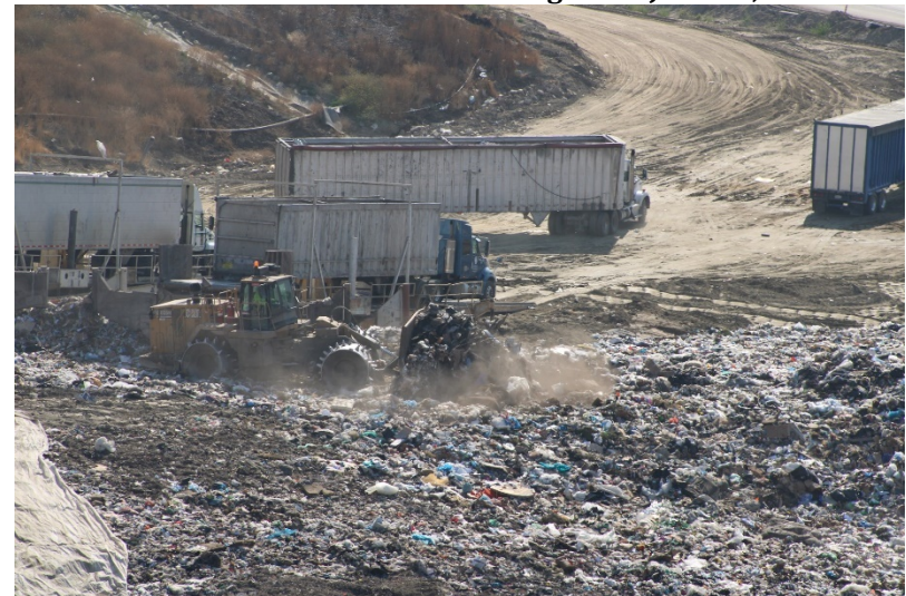
Photo 84: Cell 6 and Cell 8 Working Area: June 14, 2023
