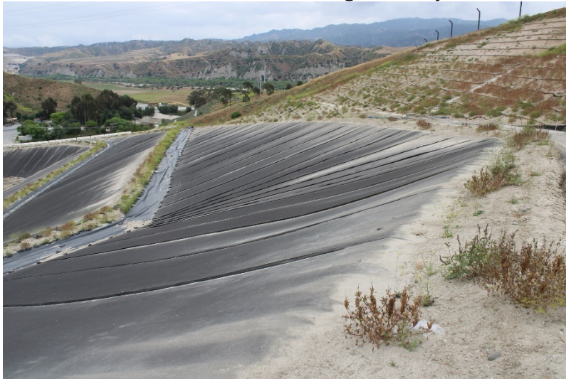
Photo 55: Cell 6 and Cell 8 Working Area: May 25, 2023
