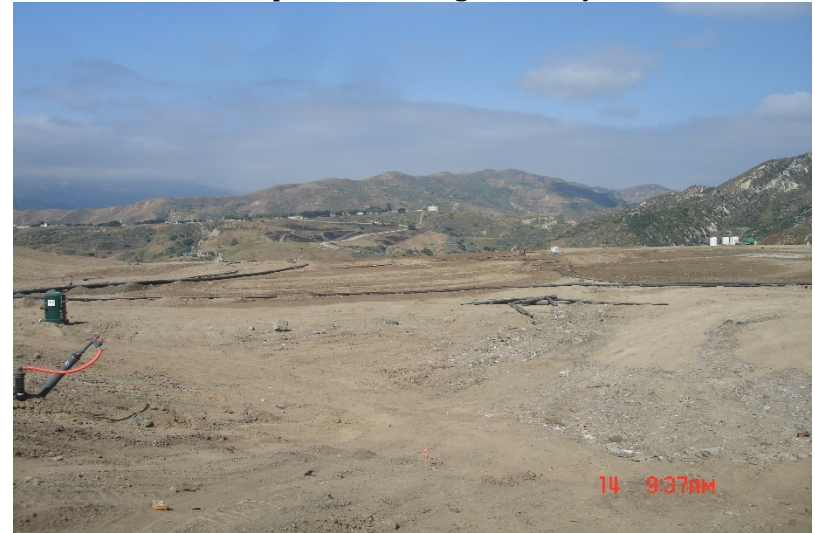
Photo 28: Top Deck Working Area: June 14, 2023
