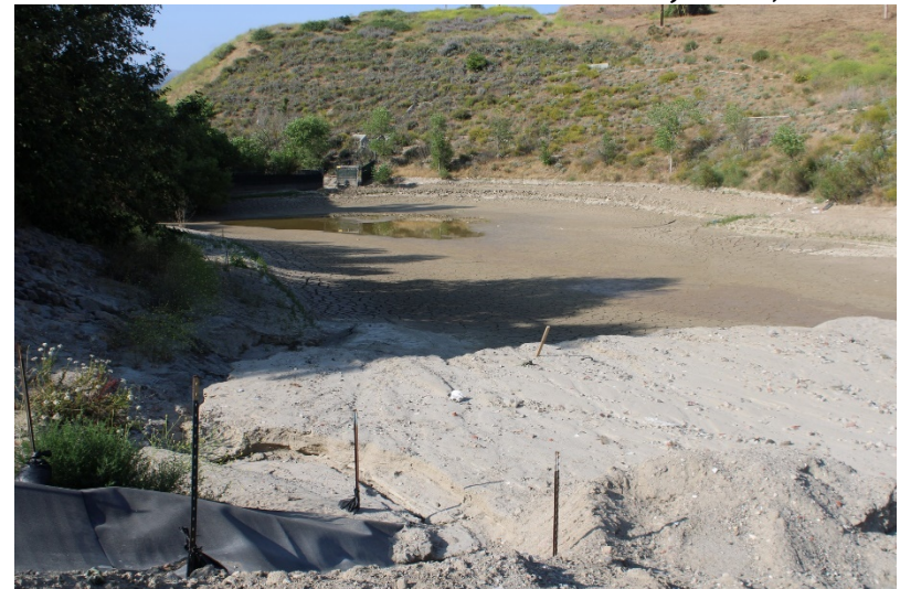
Photo 160: South Terminal and Catch Basins: June 14, 2023
