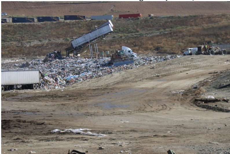
Photo 71: Cell 6 and Cell 8 Working Area: June 14, 2023
