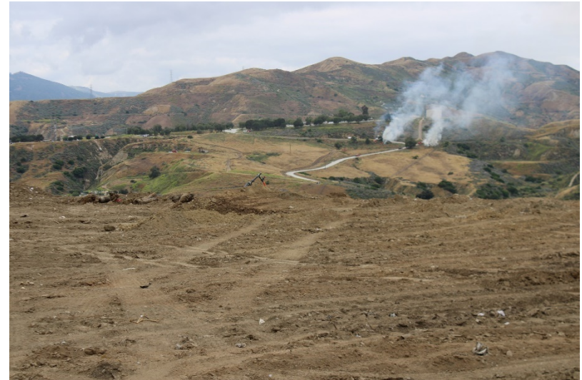
Photo 22: Top Deck Working Area: May 25, 2023
