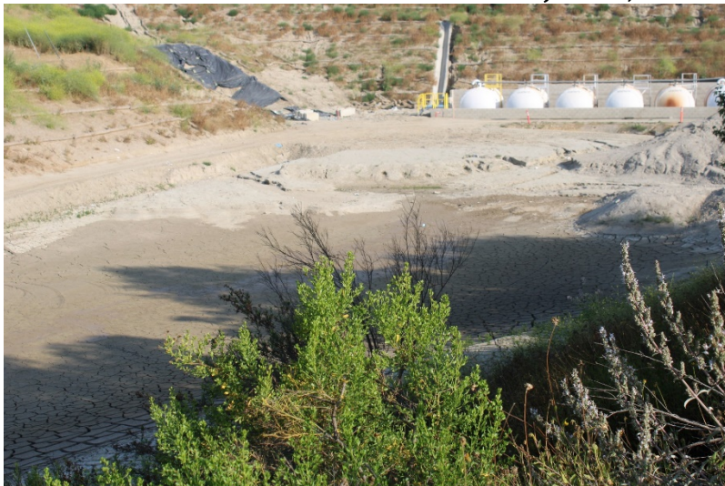
Photo 159: South Terminal and Catch Basins: June 14, 2023
