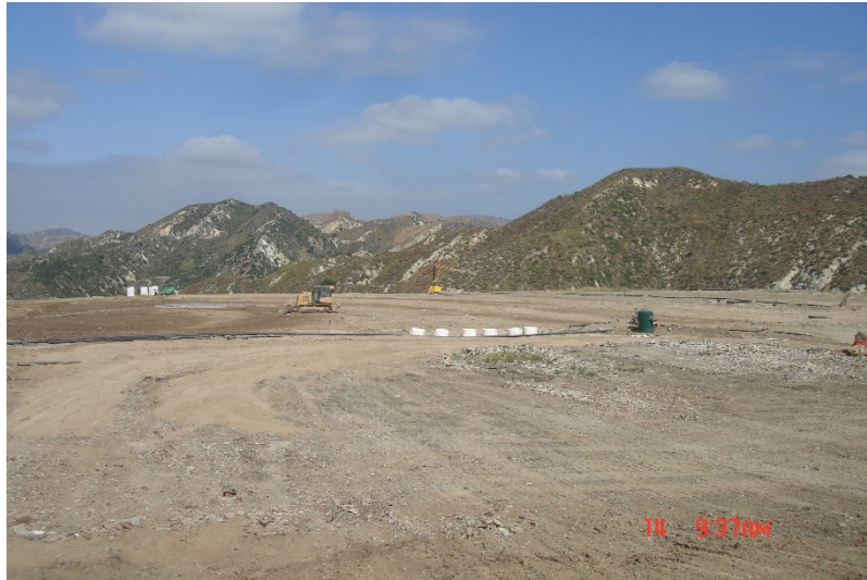
Photo 29: Top Deck Working Area: June 14, 2023
