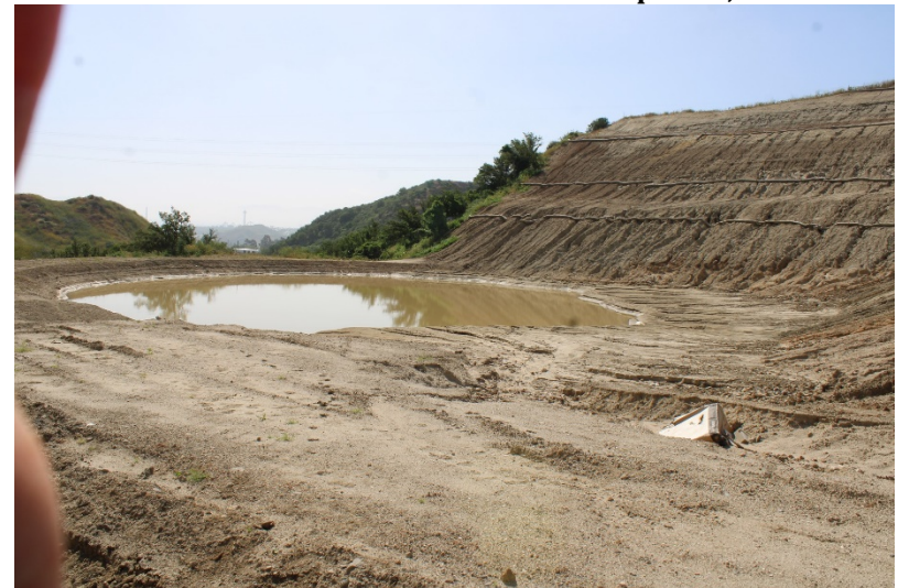
Photo 172: Northeast Sediment Basin: April 25, 2023
