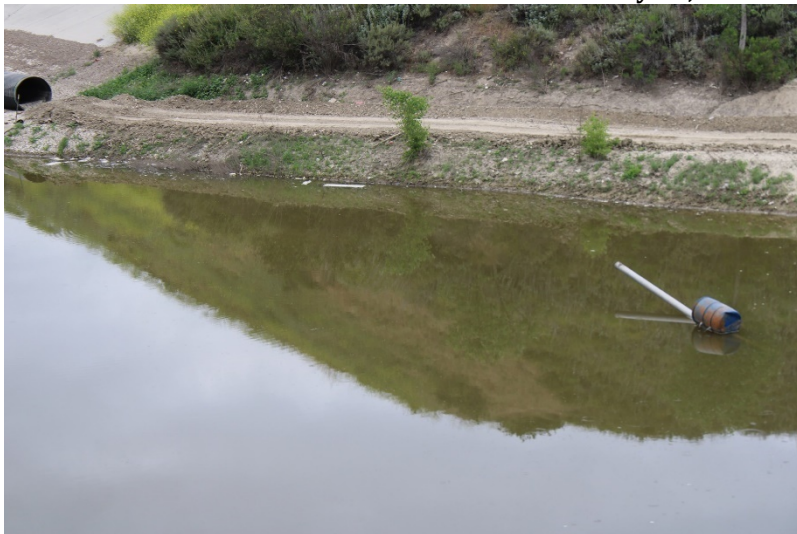
Photo 151: South Terminal and Catch Basins: May 25, 2023
