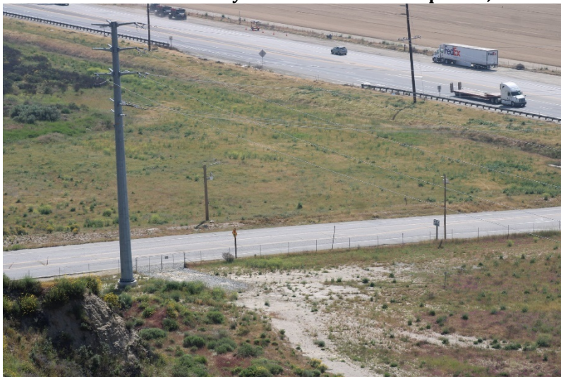
Photo 207: Wolcott Way Entrance Facilities: April 25, 2023
