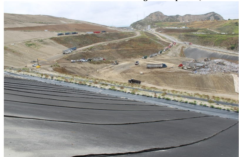
Photo 52: Cell 6 and Cell 8 Working Area: May 25, 2023
