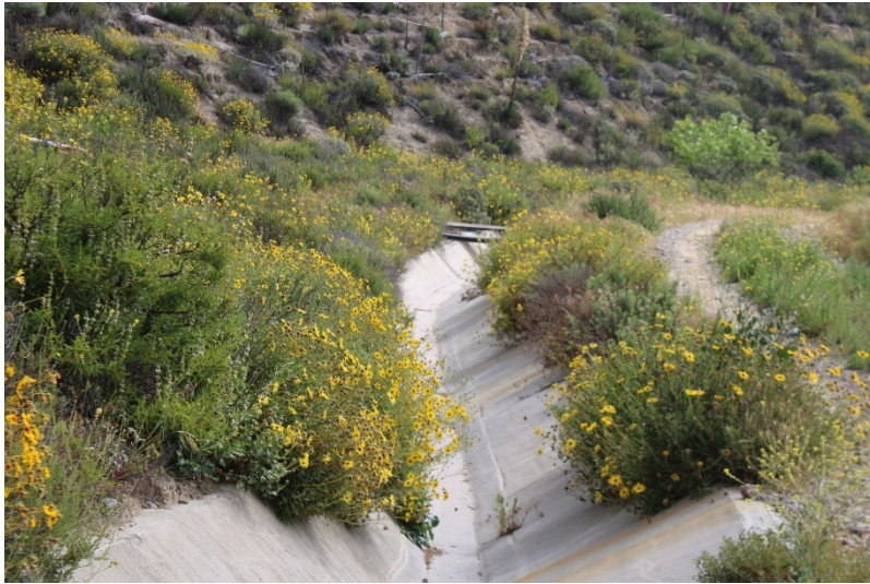
Photo 173: Landfill Perimeter Drainage Channel: April 25, 2023
