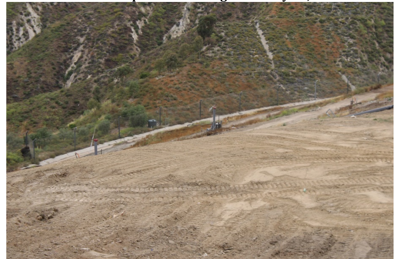
Photo 24: Top Deck Working Area: May 25, 2023
