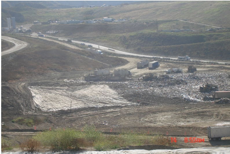
Photo 69: Cell 6 and Cell 8 Working Area: June 14, 2023
