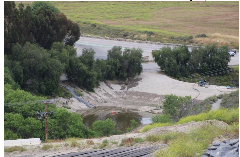
Photo 152: South Terminal and Catch Basins: May 25, 2023
