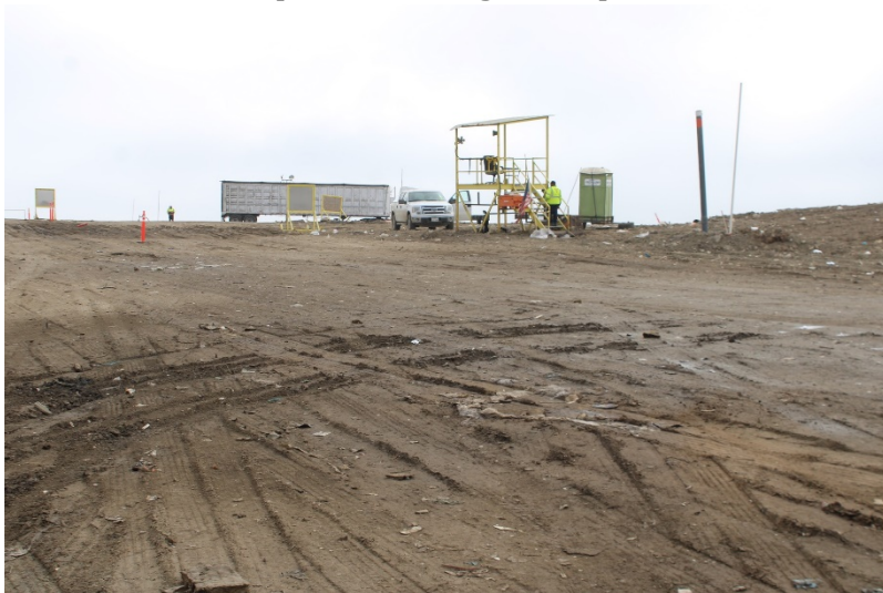
Photo 3: Top Deck Working Area: April 25, 2023
