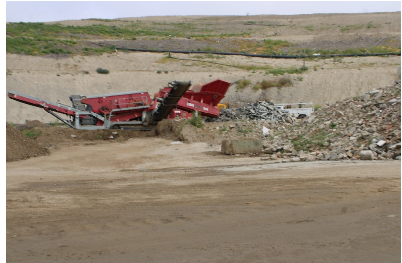
Photo 2: Top Deck Working Area: April 25, 2023
