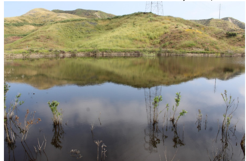
Photo 164: Northeast Sediment Basin: April 25, 2023
