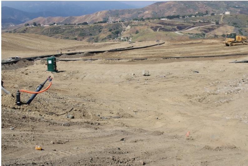
Photo 33: Top Deck Working Area: June 14, 2023
