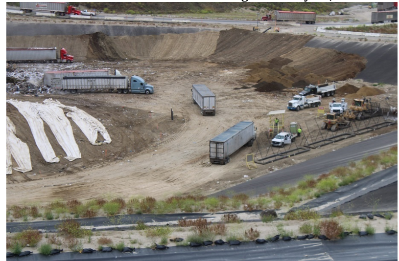
Photo 60: Cell 6 and Cell 8 Working Area: May 25, 2023
