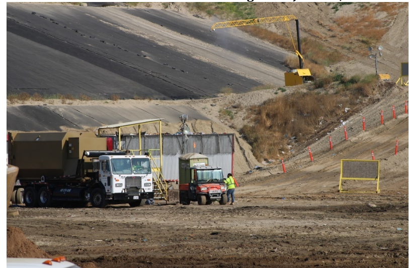
Photo 72: Cell 6 and Cell 8 Working Area: June 14, 2023
