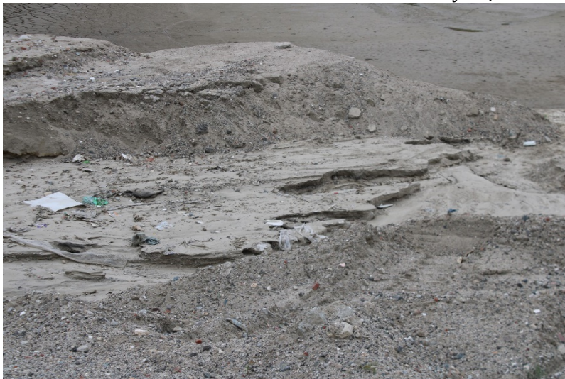
Photo 147: South Terminal and Catch Basins: May 25, 2023
