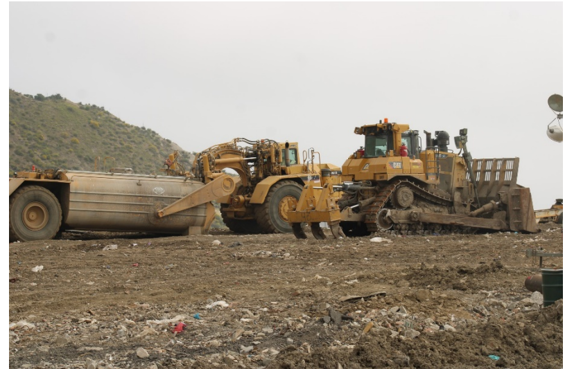
Photo 14: Top Deck Working Area: April 25, 2023
