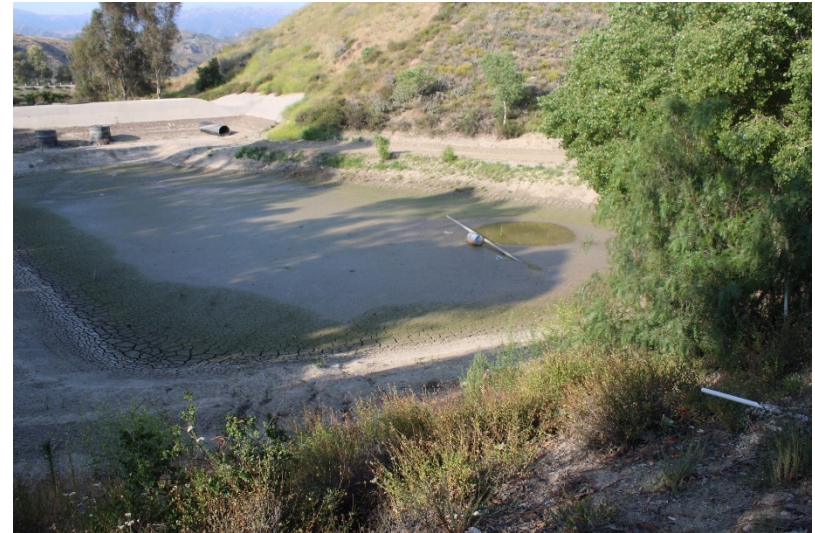
Photo 154: South Terminal and Catch Basins: June 14, 2023
