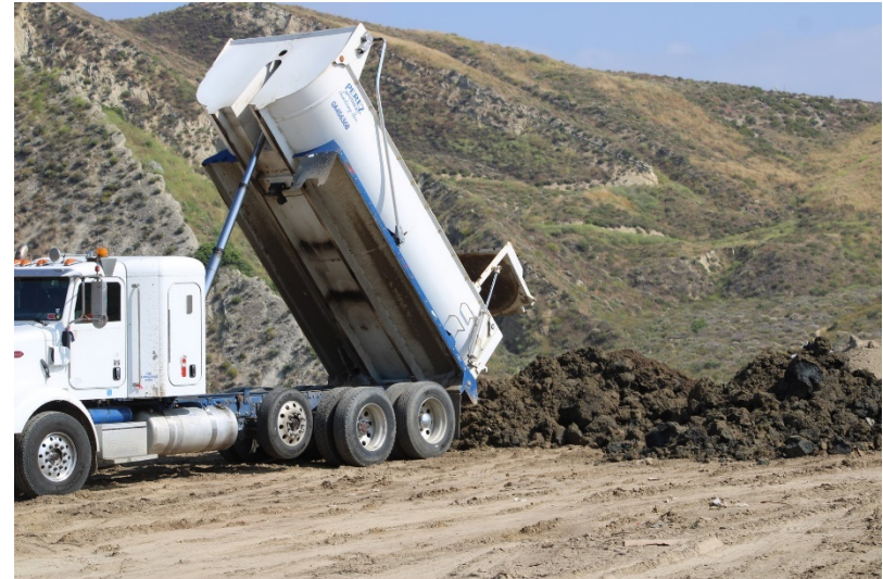
Photo 30: Top Deck Working Area: June 14, 2023
