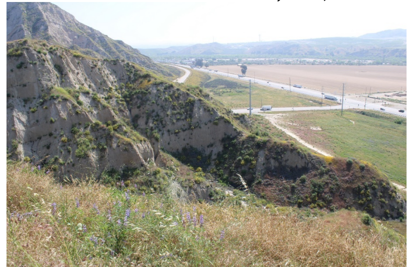
Photo 204: Wolcott Way Entrance Facilities: April 25, 2023
