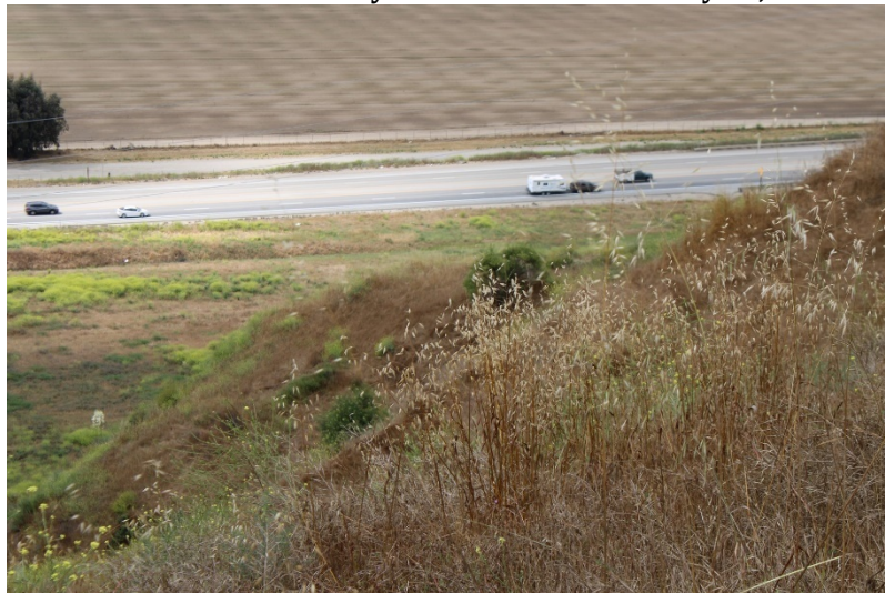
Photo 215: Wolcott Way Entrance Facilities: May 25, 2023
