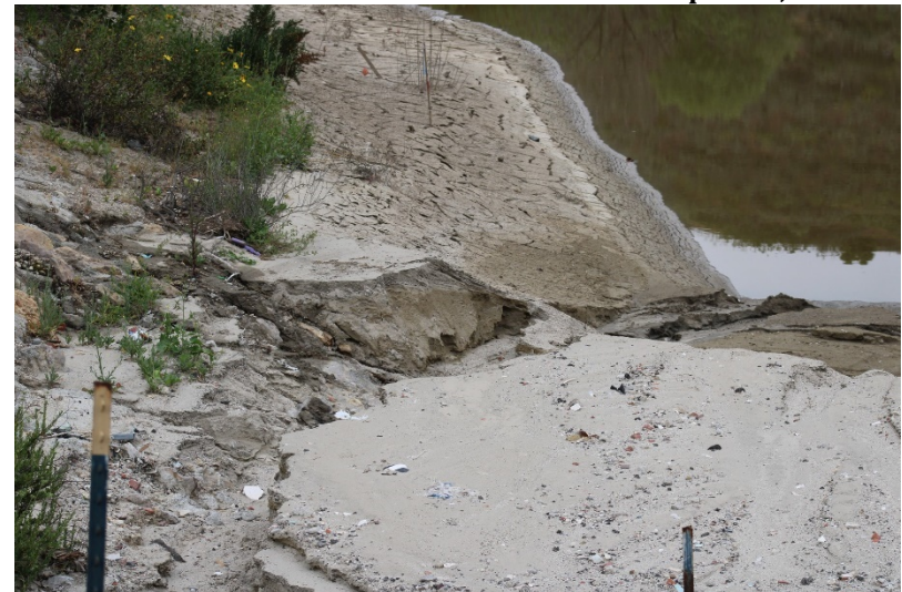
Photo 124: South Terminal and Catch Basins: April 25, 2023
