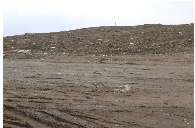
Photo 4: Top Deck Working Area: April 25, 2023
