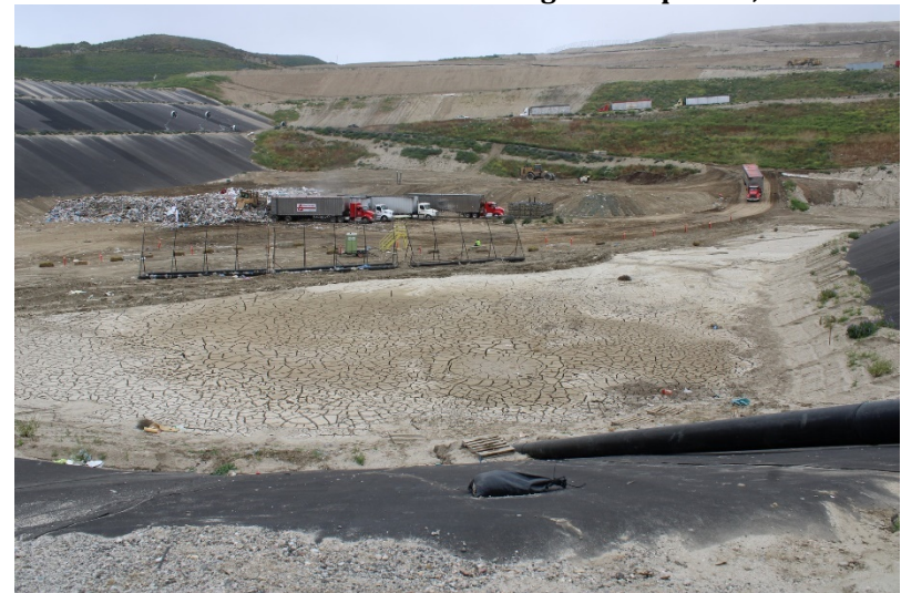
Photo 40: Cell 6 and Cell 8 Working Area: April 25, 2023
