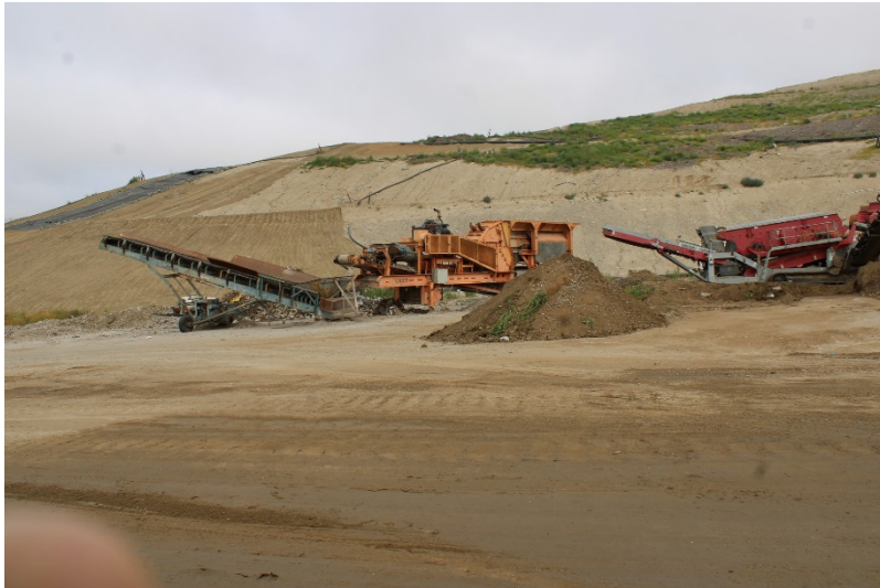
Photo 1: Top Deck Working Area: April 25, 2023
