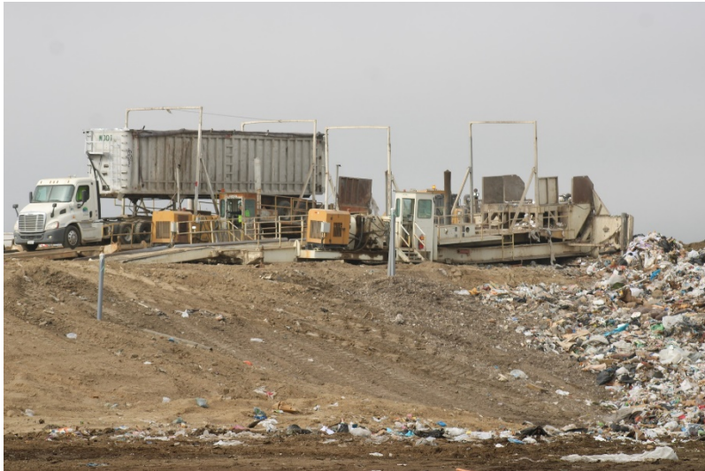
Photo 9: Top Deck Working Area: April 25, 2023
