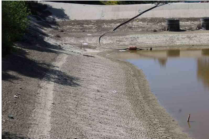
Photo 129: South Terminal and Catch Basins: April 25, 2023
