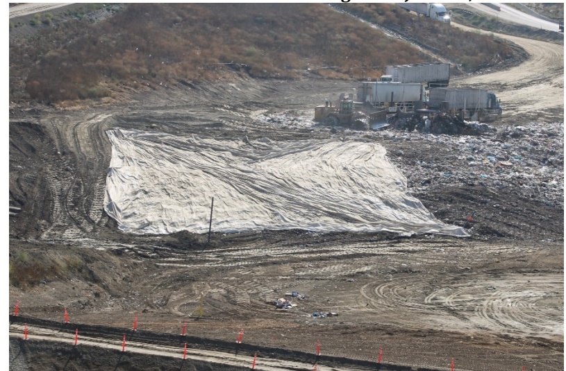
Photo 80: Cell 6 and Cell 8 Working Area: June 14, 2023
