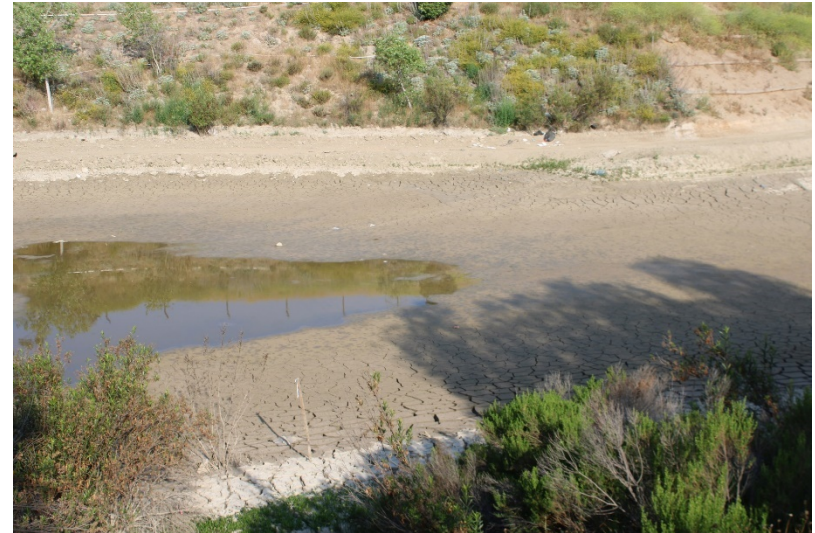
Photo 158: South Terminal and Catch Basins: June 14, 2023
