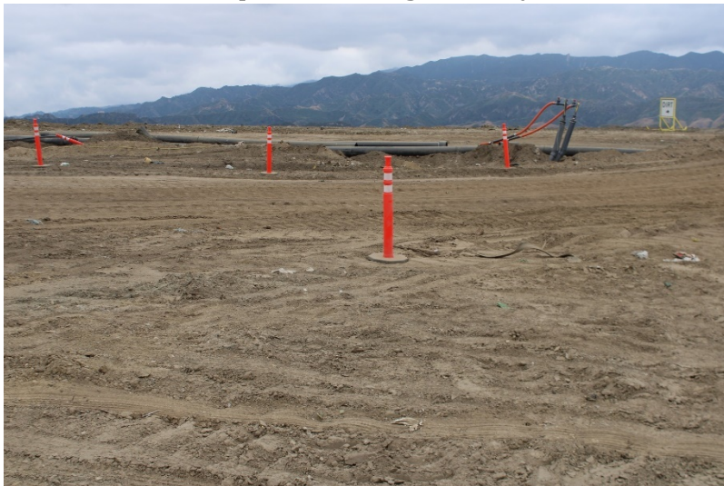
Photo 19: Top Deck Working Area: May 25, 2023
