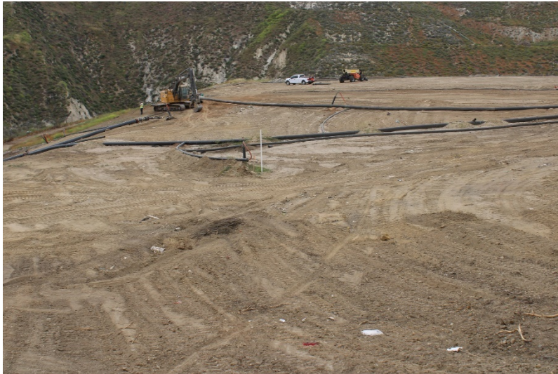
Photo 25: Top Deck Working Area: May 25, 2023
