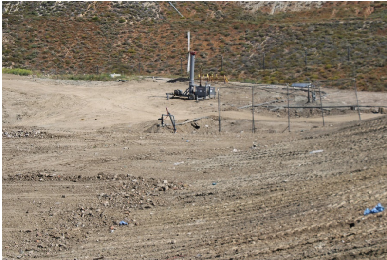
Photo 37: Top Deck Working Area: June 14, 2023
