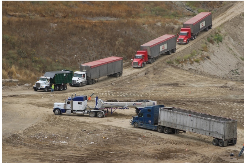
Photo 61: Cell 6 and Cell 8 Working Area: May 25, 2023
