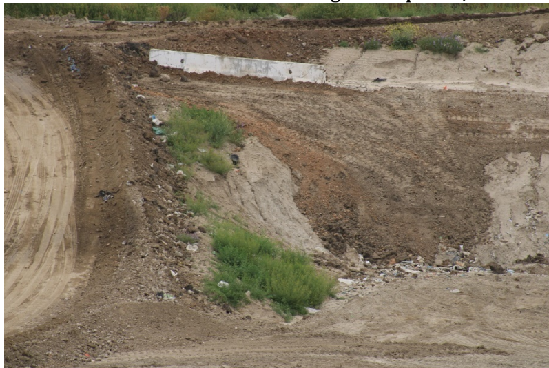
Photo 51: Cell 6 and Cell 8 Working Area: April 25, 2023
