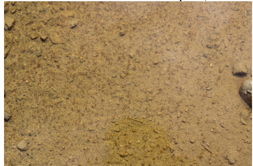
Photo 168: Northeast Sediment Basin: April 25, 2023
