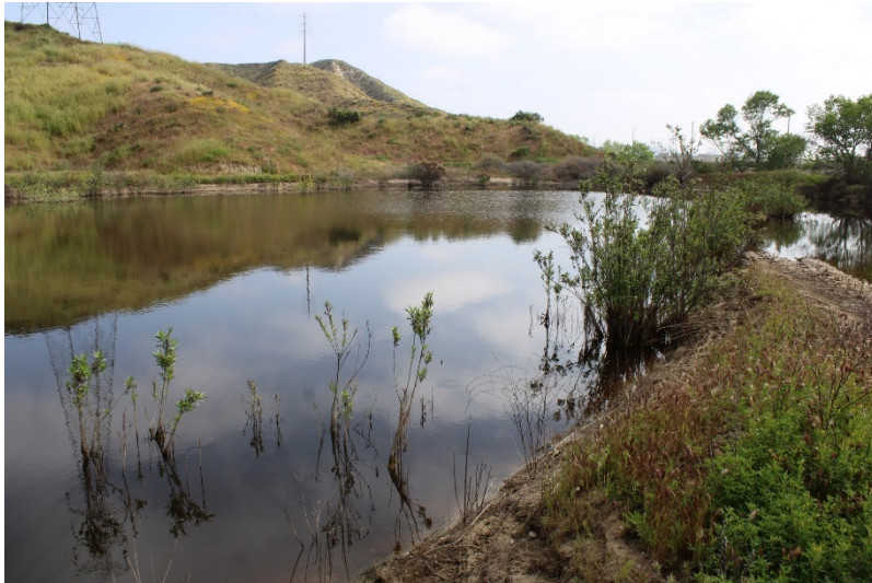
Photo 165: Northeast Sediment Basin: April 25, 2023
