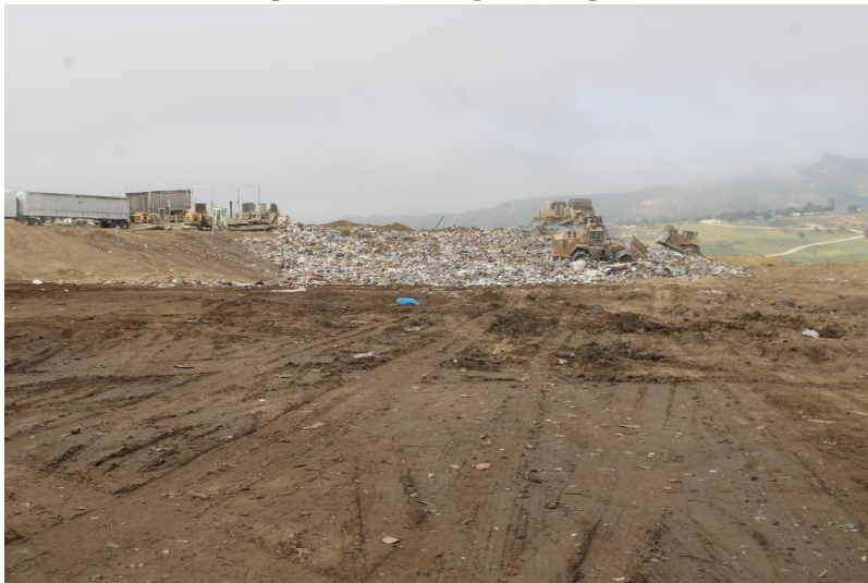
Photo 7: Top Deck Working Area: April 25, 2023
