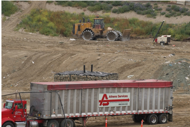
Photo 49: Cell 6 and Cell 8 Working Area: April 25, 2023
