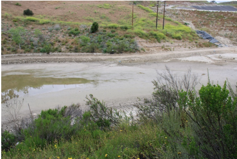
Photo 141: South Terminal and Catch Basins: May 25, 2023
