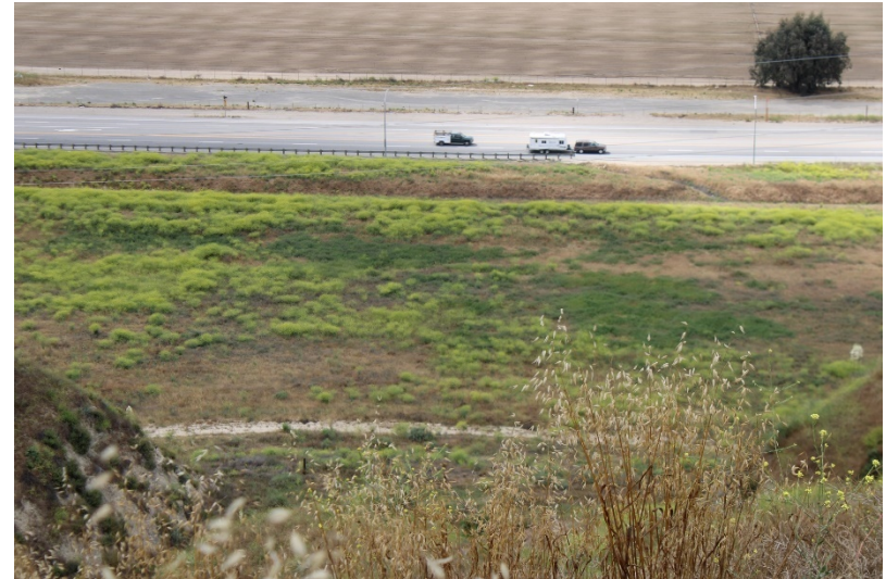
Photo 214: Wolcott Way Entrance Facilities: May 25, 2023
