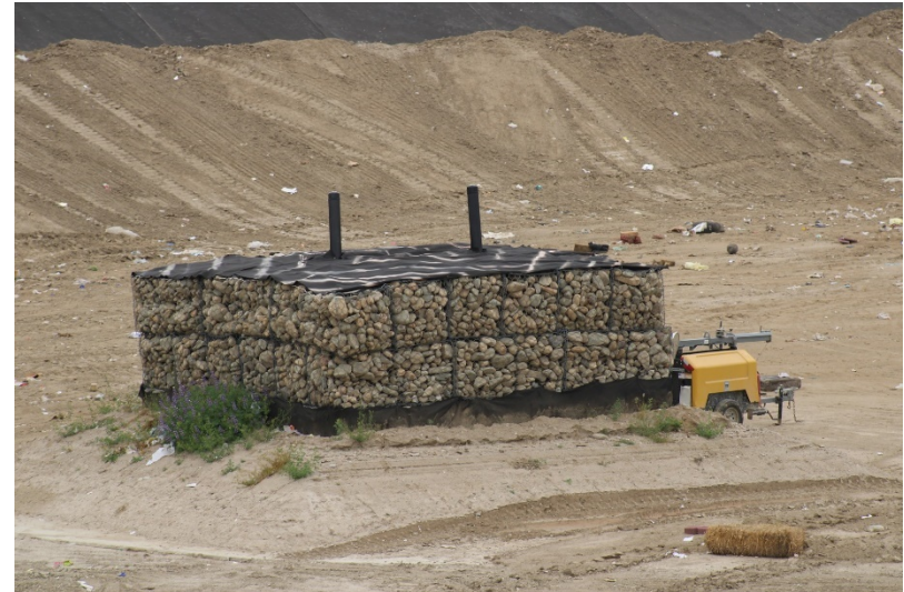
Photo 46: Cell 6 and Cell 8 Working Area: April 25, 2023
