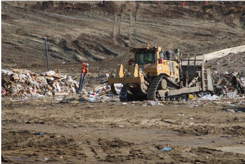
Photo 73: Cell 6 and Cell 8 Working Area: June 14, 2023
