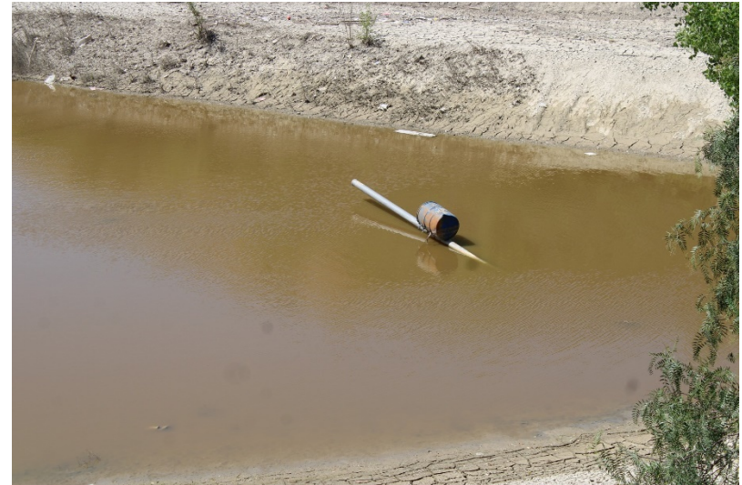
Photo 130: South Terminal and Catch Basins: April 25, 2023
