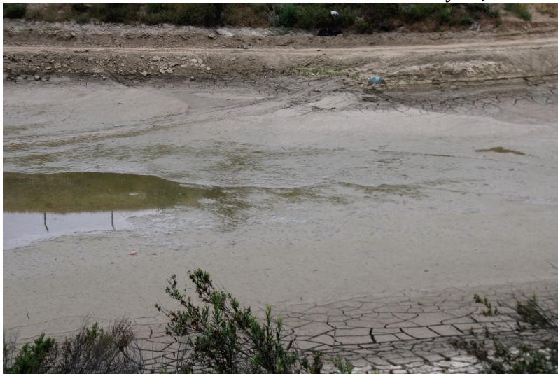
Photo 143: South Terminal and Catch Basins: May 25, 2023
