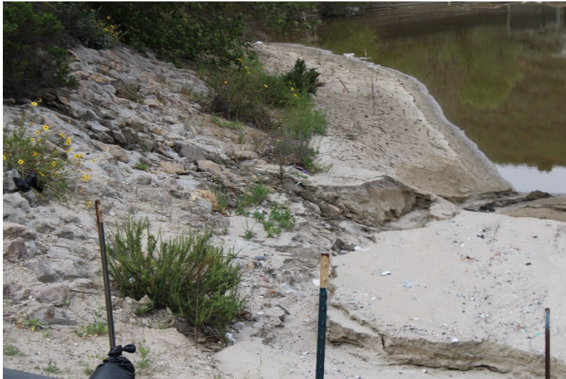
Photo 121: South Terminal and Catch Basins: April 25, 2023
