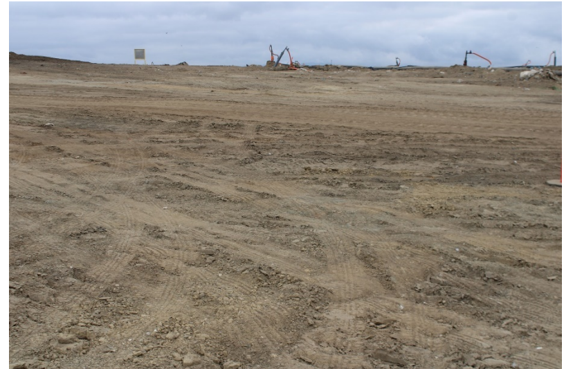
Photo 18: Top Deck Working Area: May 25, 2023
