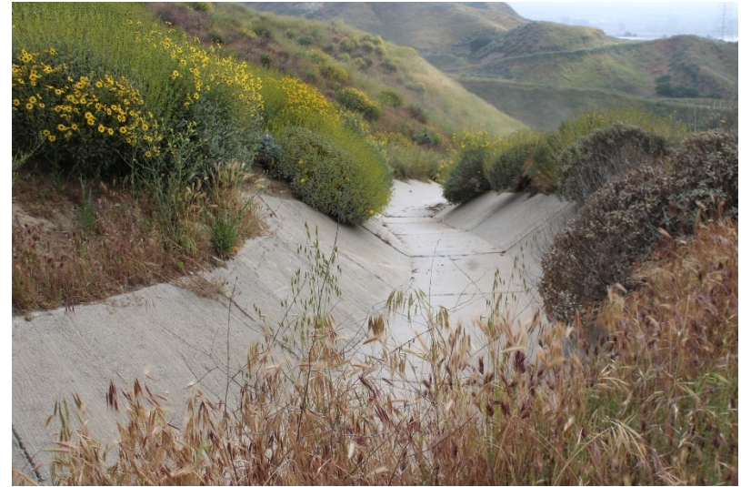
Photo 174: Landfill Perimeter Drainage Channel: April 25, 2023
