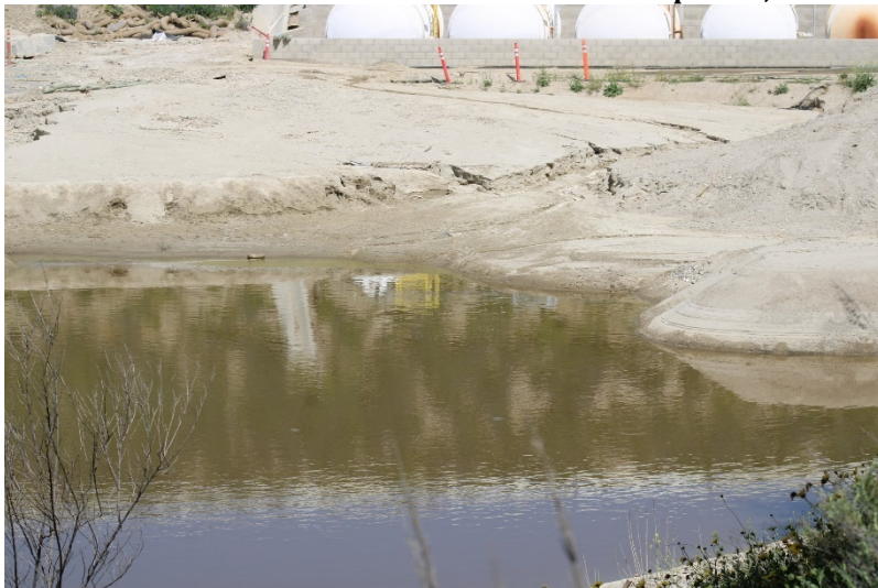
Photo 139: South Terminal and Catch Basins: April 25, 2023
