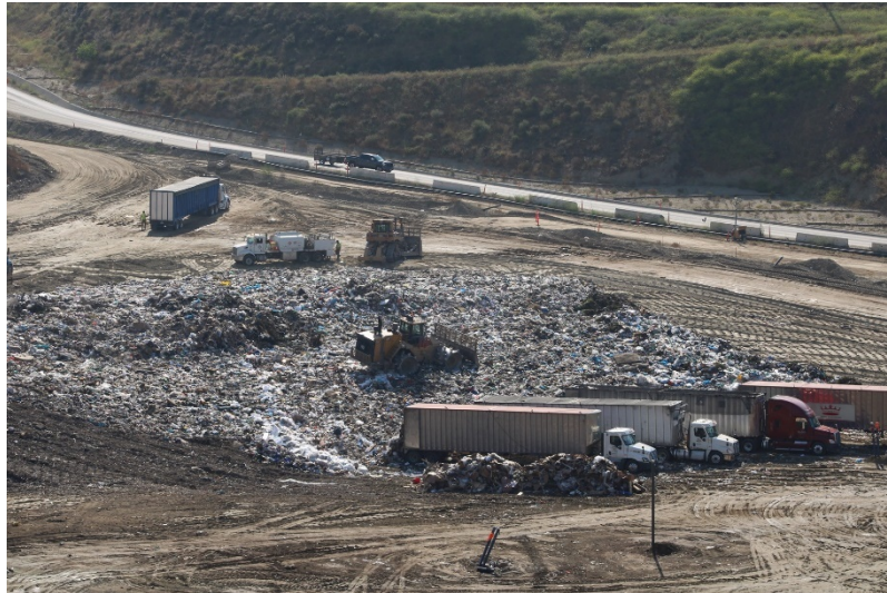
Photo 81: Cell 6 and Cell 8 Working Area: June 14, 2023
