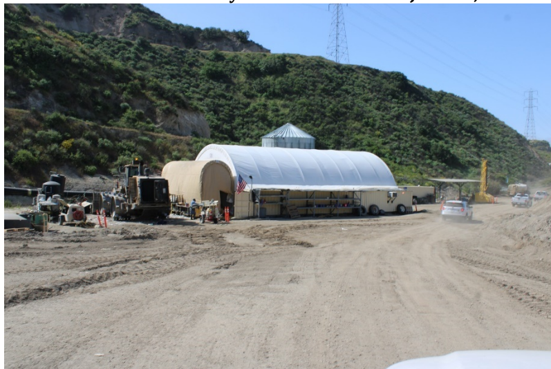
Photo 219: Maintenance and Admin Buildings: April 25, 2023
