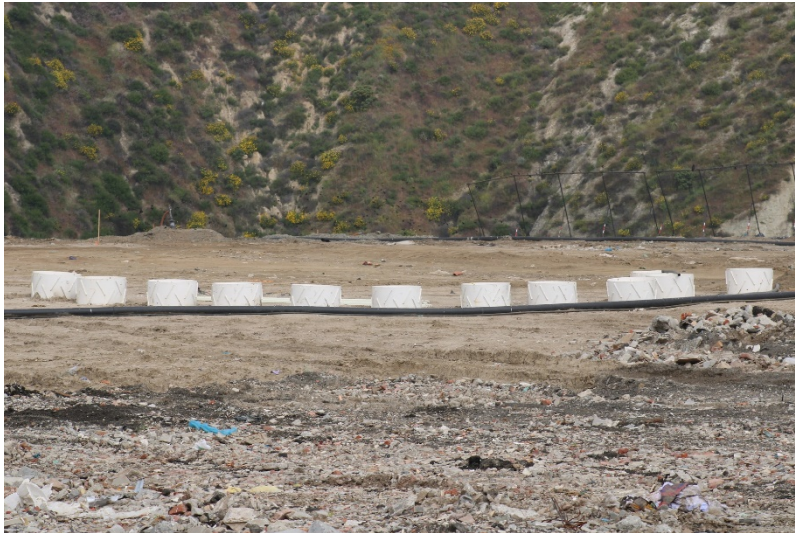
Photo 13: Top Deck Working Area: April 25, 2023
