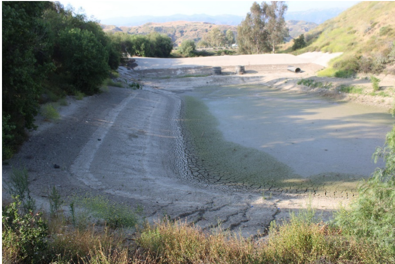
Photo 153: South Terminal and Catch Basins: June 14, 2023
