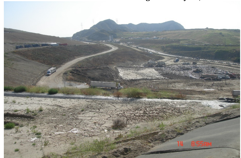
Photo 68: Cell 6 and Cell 8 Working Area: June 14, 2023
