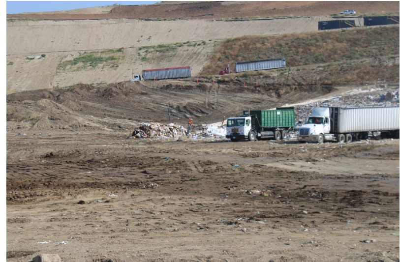
Photo 70: Cell 6 and Cell 8 Working Area: June 14, 2023
