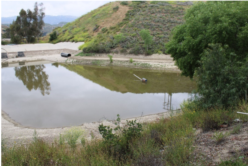
Photo 149: South Terminal and Catch Basins: May 25, 2023
