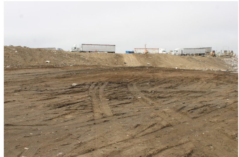
Photo 6: Top Deck Working Area: April 25, 2023
