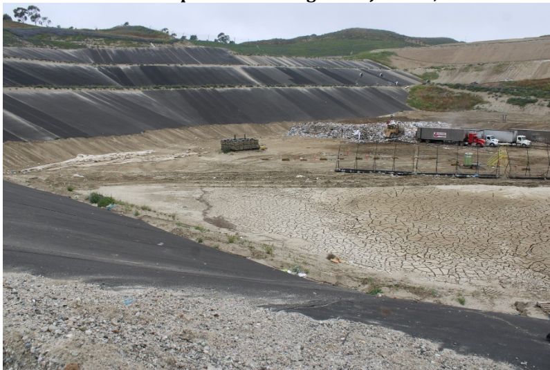
Photo 39: Cell 6 and Cell 8 Working Area: April 25, 2023
