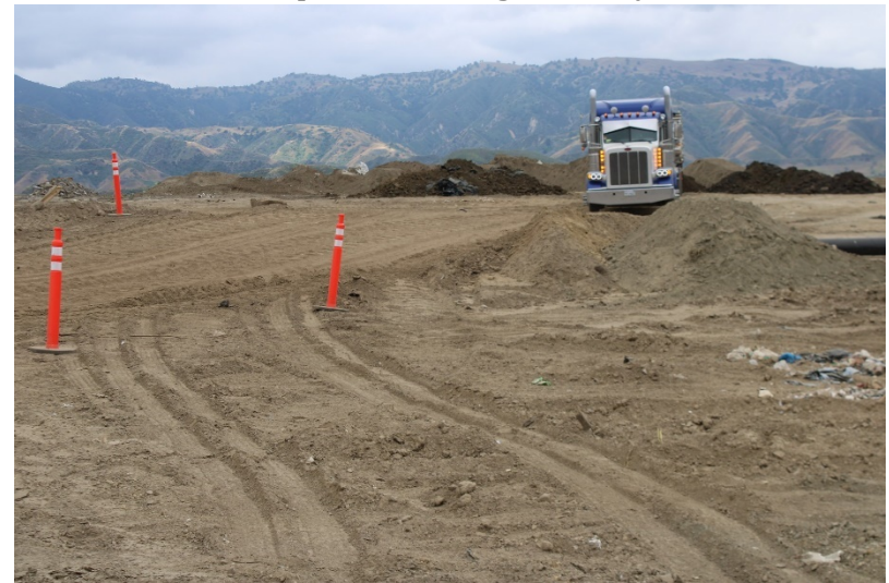
Photo 20: Top Deck Working Area: May 25, 2023
