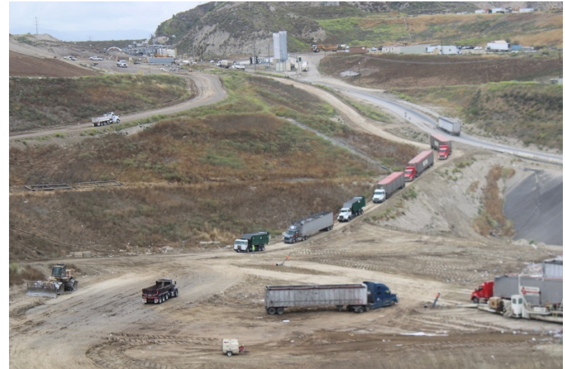
Photo 58: Cell 6 and Cell 8 Working Area: May 25, 2023
