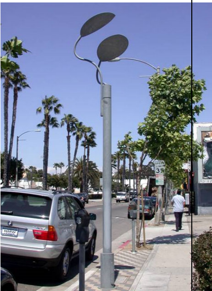
Example of pedestrian-scale Pedestrian street lighting example
