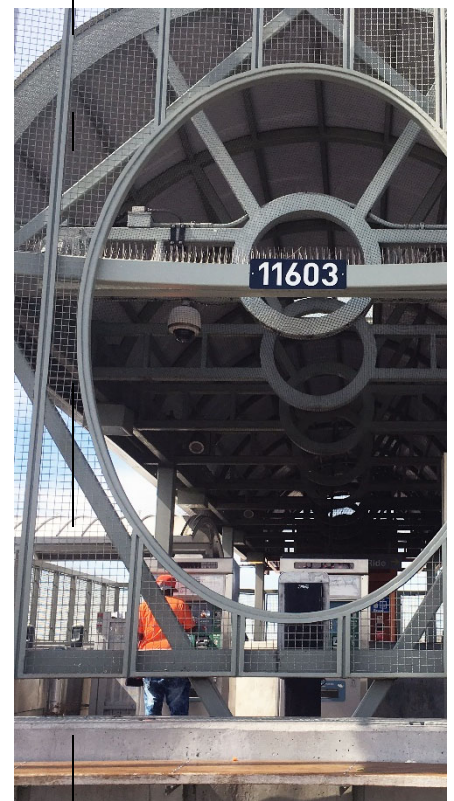
Existing entrance into the Vermont/Athens Station.
