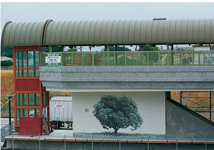
Existing view of station platform, transit station boarding area.
