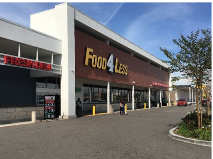
Existing Food4Less Supermarket facing Western Avenue.
