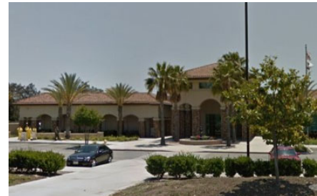
Existing Los Angeles County Sheriff's Department Southwest Station along Imperial highway.
