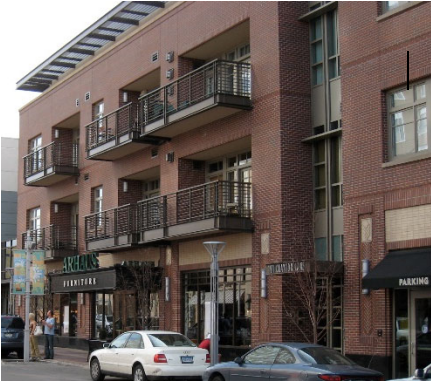
Example ground floor commercial with shopfront frontage and residential above.
