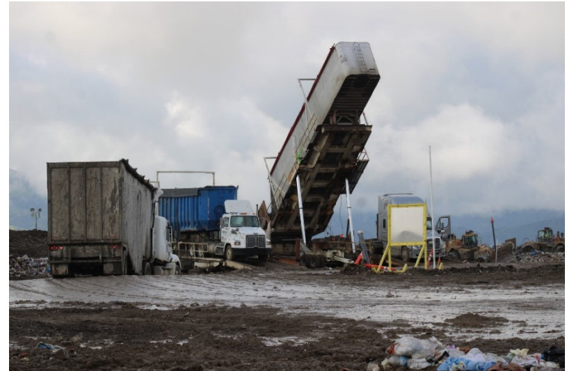
Photo 46: Top Deck Working Area: March 23, 2023
