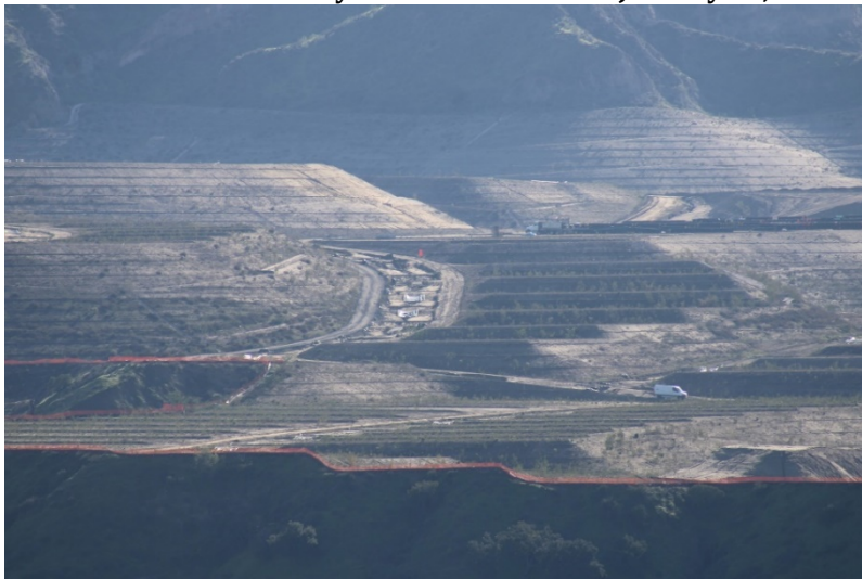
Photo 155: Wolcott Way Entrance Facilities: January 19, 2023
