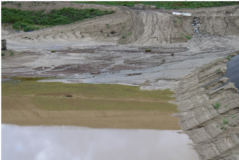
Photo 319: Cell 8 Construction: March 23, 2023
