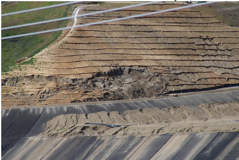
Photo 291: Cell 8 Construction: February 28, 2023
