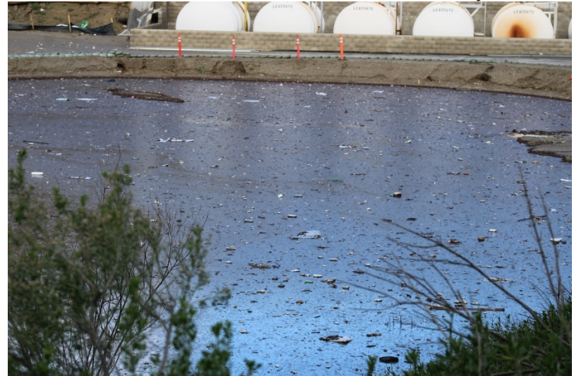
Photo 108: South Terminal and Catch Basins: February 28, 2023
