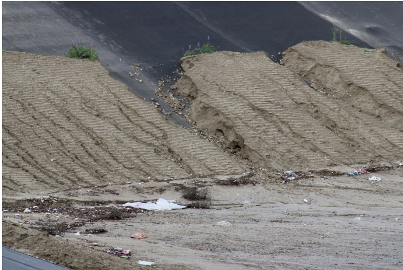
Photo 321: Cell 8 Construction: March 23, 2023
