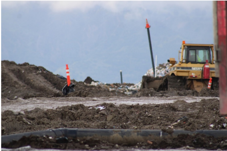
Photo 41: Top Deck Working Area: March 23, 2023
