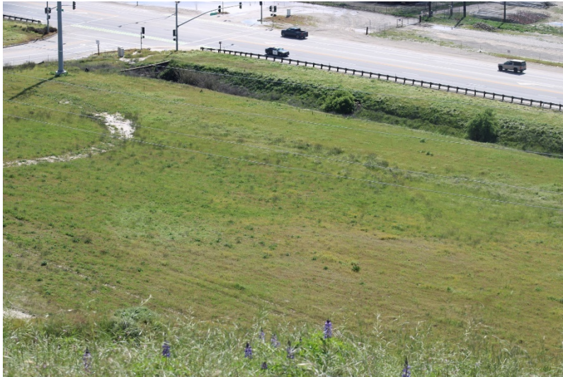
Photo 165: Wolcott Way Entrance Facilities: March 23, 2023
