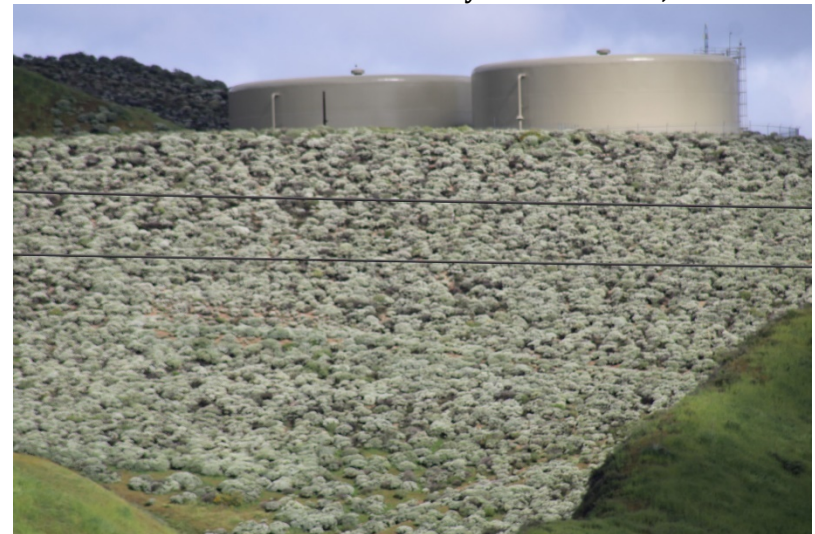
Photo 68: Closed Landfill - Canyon B: March 23, 2023
