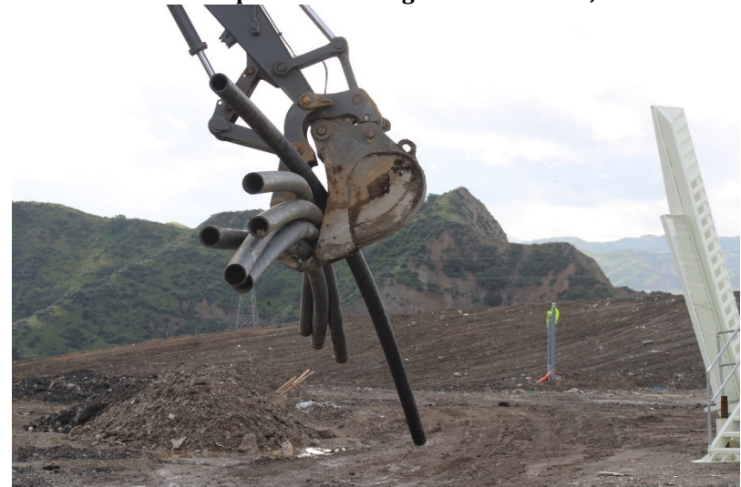
Photo 56: Top Deck Working Area: March 23, 2023
