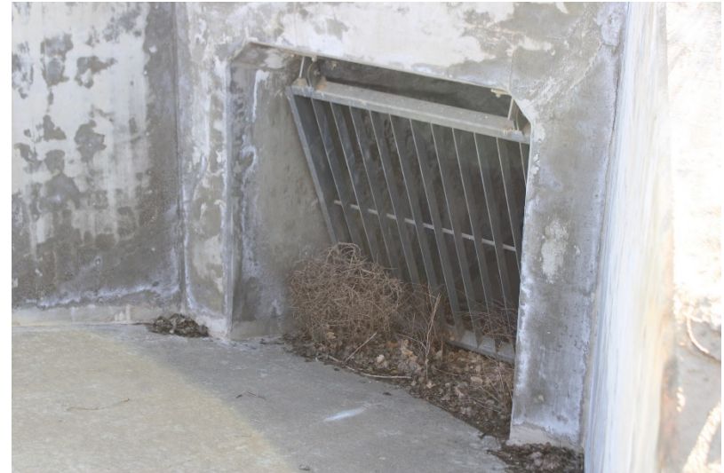
Photo 122: Northeast Sediment Basin: January 19, 2023
