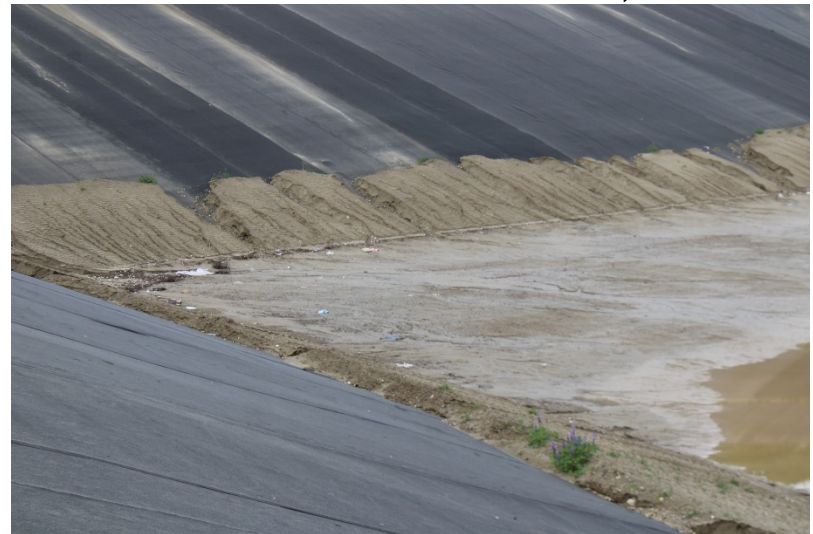
Photo 316: Cell 8 Construction: March 23, 2023
