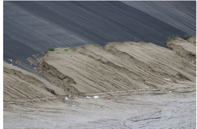
Photo 322: Cell 8 Construction: March 23, 2023
