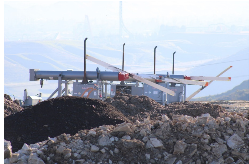
Photo 12: Top Deck Working Area: January 19, 2023
