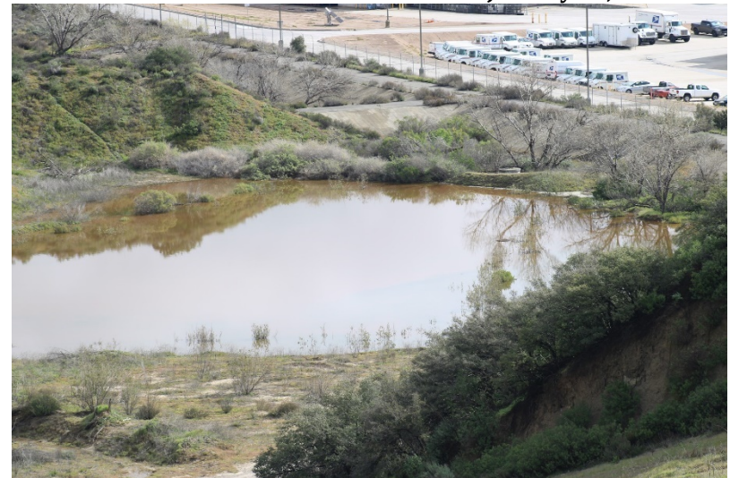
Photo 124: Northeast Sediment Basin: February 28, 2023
