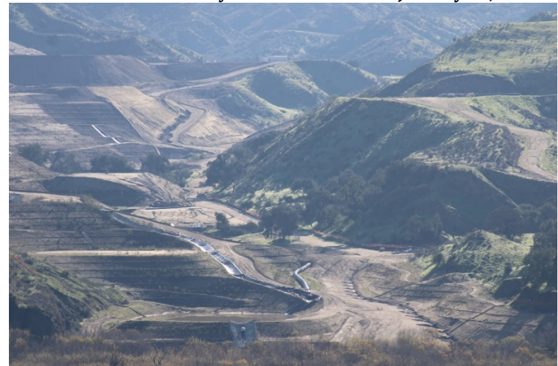
Photo 156: Wolcott Way Entrance Facilities: January 19, 2023
