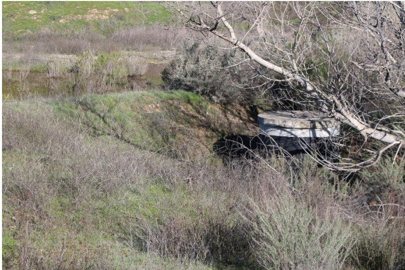
Photo 121: Northeast Sediment Basin: January 19, 2023
