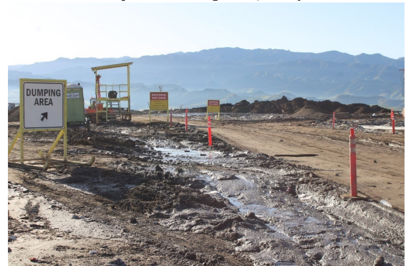
Photo 4: Top Deck Working Area: January 19, 2023
