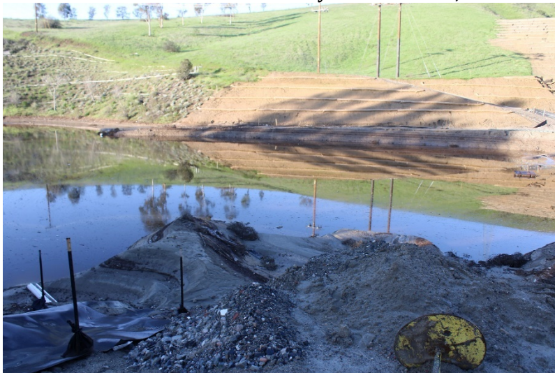
Photo 71: South Terminal and Catch Basins: January 19, 2023
