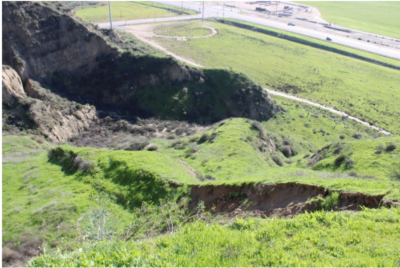
Photo 149: Wolcott Way Entrance Facilities: January 19, 2023
