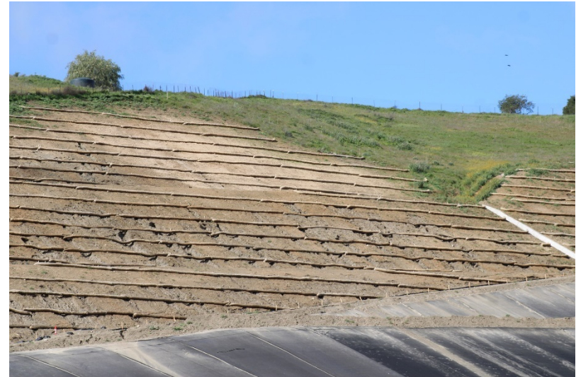
Photo 310: Cell 8 Construction: February 28, 2023
