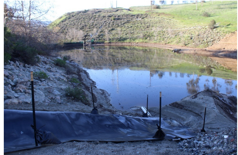
Photo 70: South Terminal and Catch Basins: January 19, 2023
