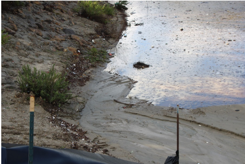
Photo 89: South Terminal and Catch Basins: February 28, 2023
