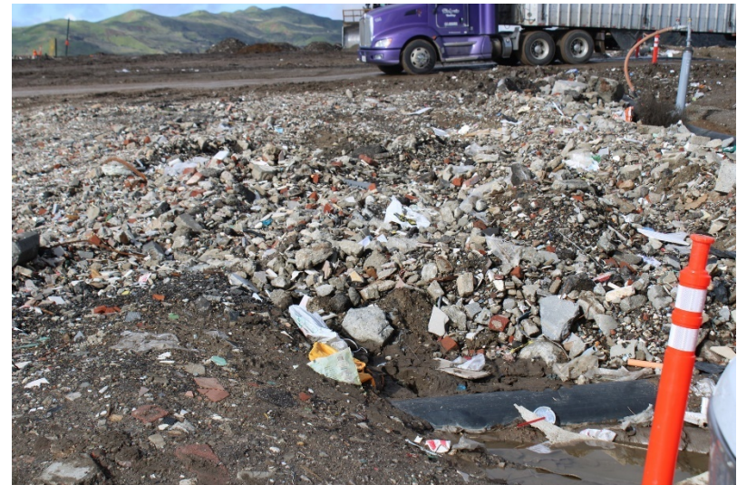
Photo 30: Top Deck Working Area: February 28, 2023
