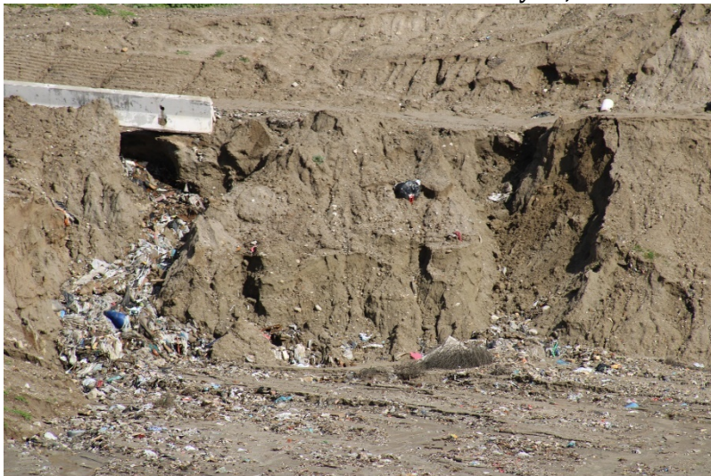
Photo 307: Cell 8 Construction: February 28, 2023
