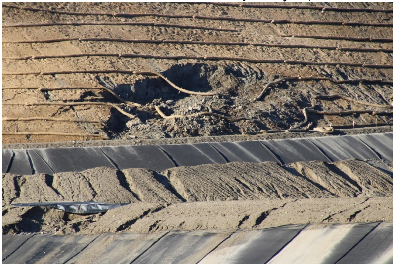
Photo 287: Cell 8 Construction: January 19, 2023
