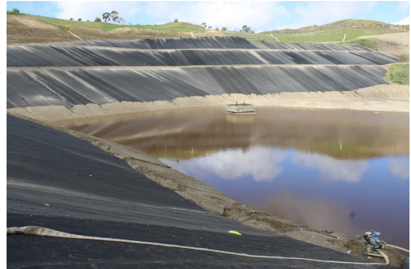
Photo 294: Cell 8 Construction: February 28, 2023
