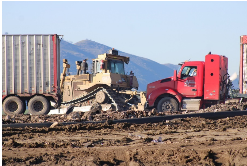
Photo 19: Top Deck Working Area: January 19, 2023
