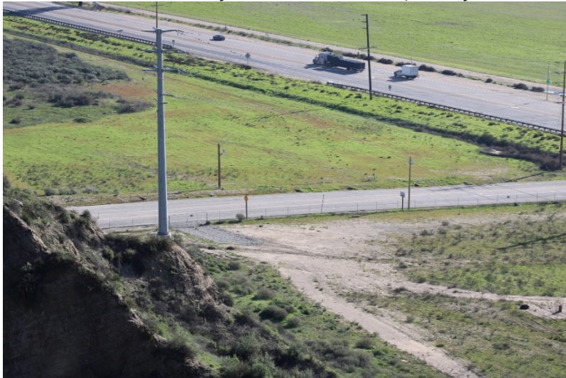
Photo 151: Wolcott Way Entrance Facilities: January 19, 2023
