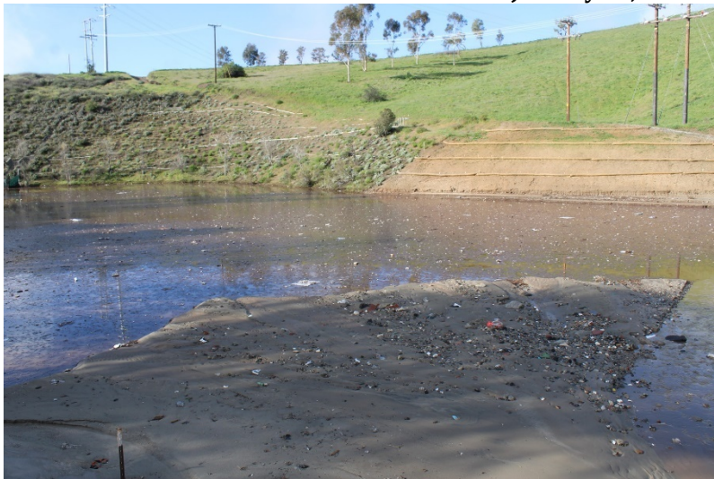
Photo 87: South Terminal and Catch Basins: February 28, 2023
