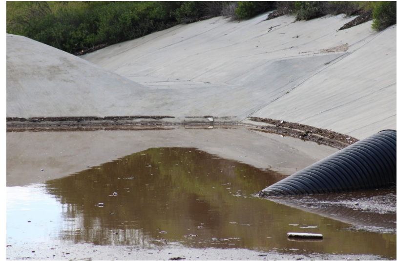
Photo 102: South Terminal and Catch Basins: February 28, 2023
