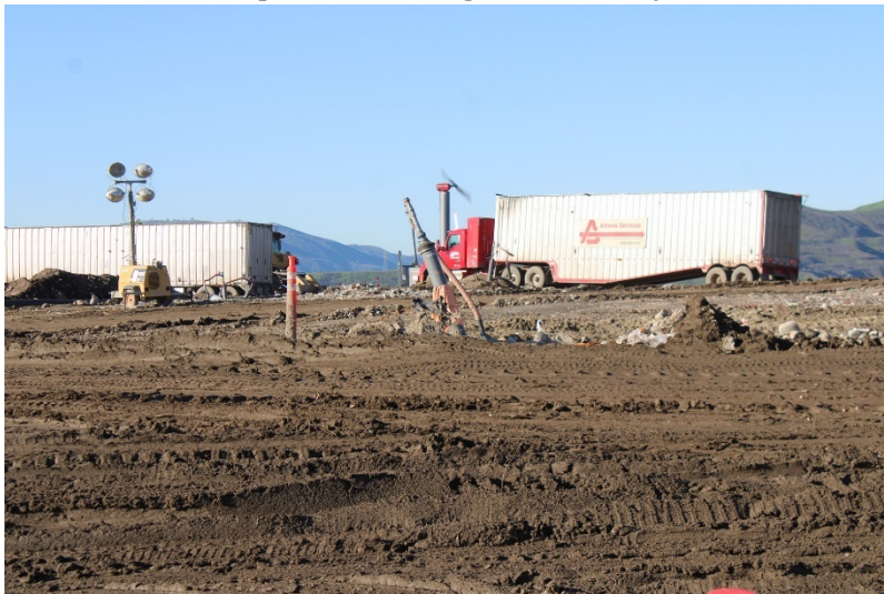
Photo 7: Top Deck Working Area: January 19, 2023
