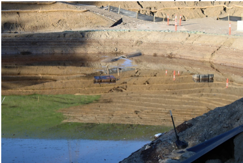
Photo 75: South Terminal and Catch Basins: January 19, 2023
