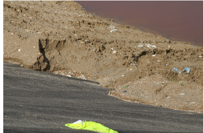
Photo 302: Cell 8 Construction: February 28, 2023
