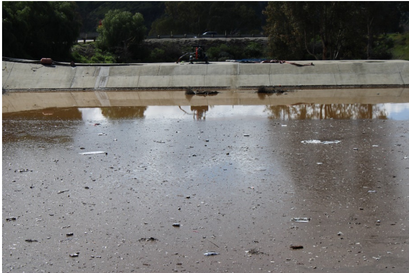
Photo 97: South Terminal and Catch Basins: February 28, 2023
