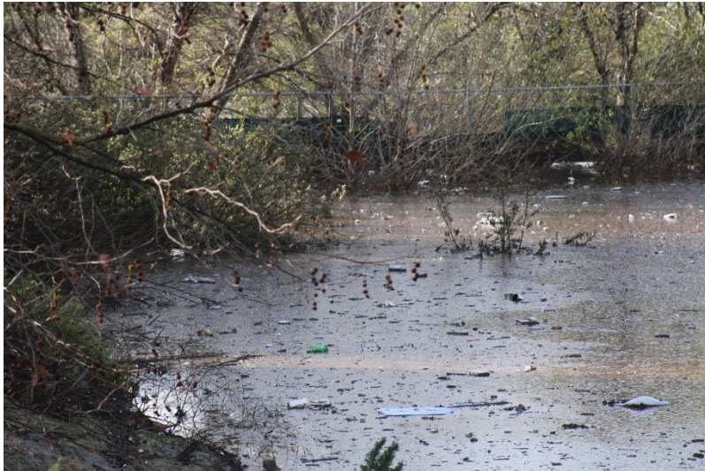
Photo 93: South Terminal and Catch Basins: February 28, 2023
