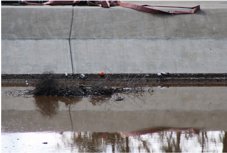
Photo 101: South Terminal and Catch Basins: February 28, 2023
