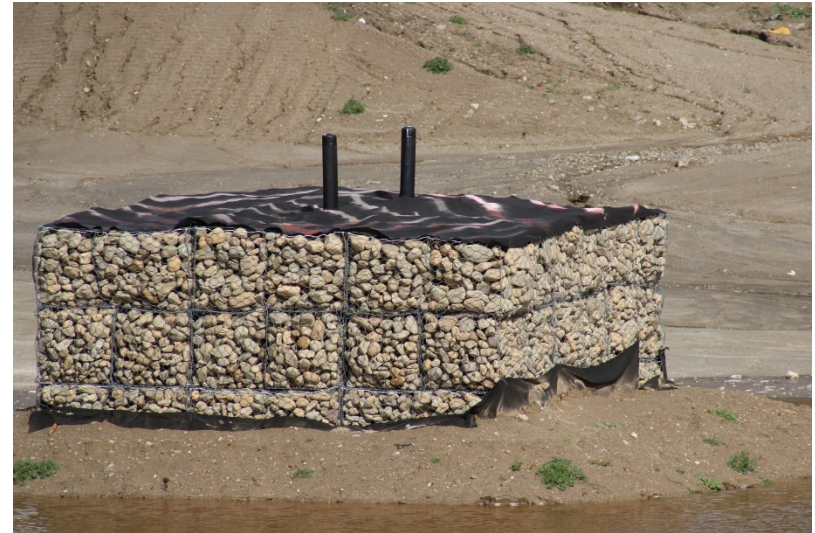
Photo 306: Cell 8 Construction: February 28, 2023
