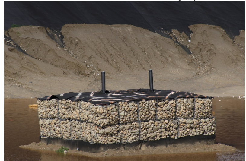
Photo 304: Cell 8 Construction: February 28, 2023
