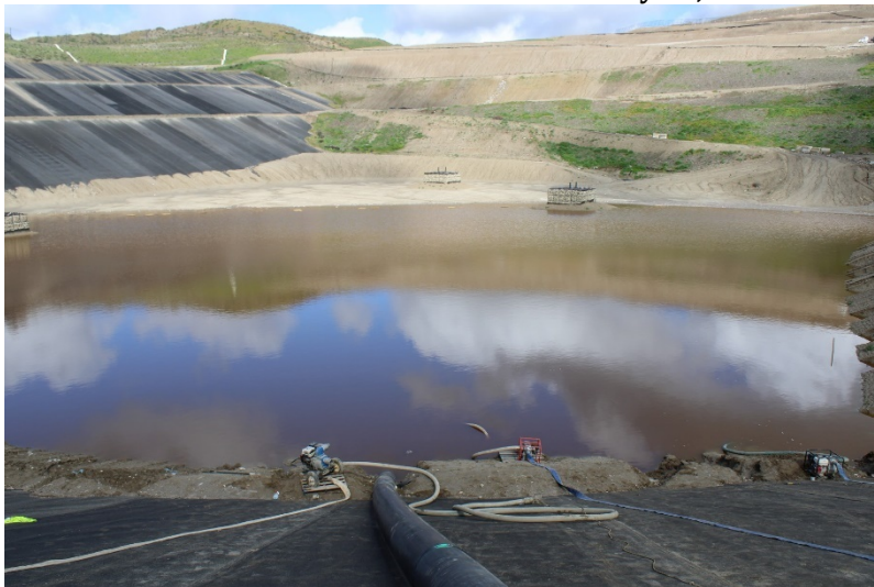
Photo 295: Cell 8 Construction: February 28, 2023
