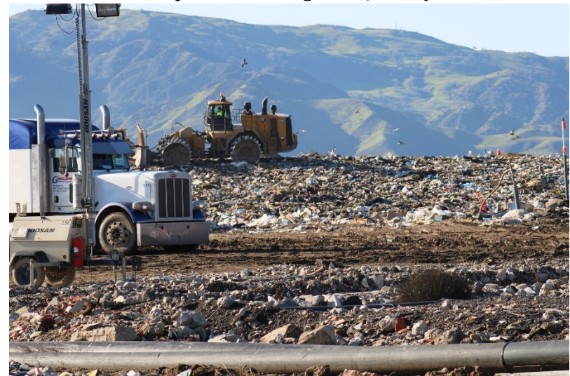
Photo 16: Top Deck Working Area: January 19, 2023
