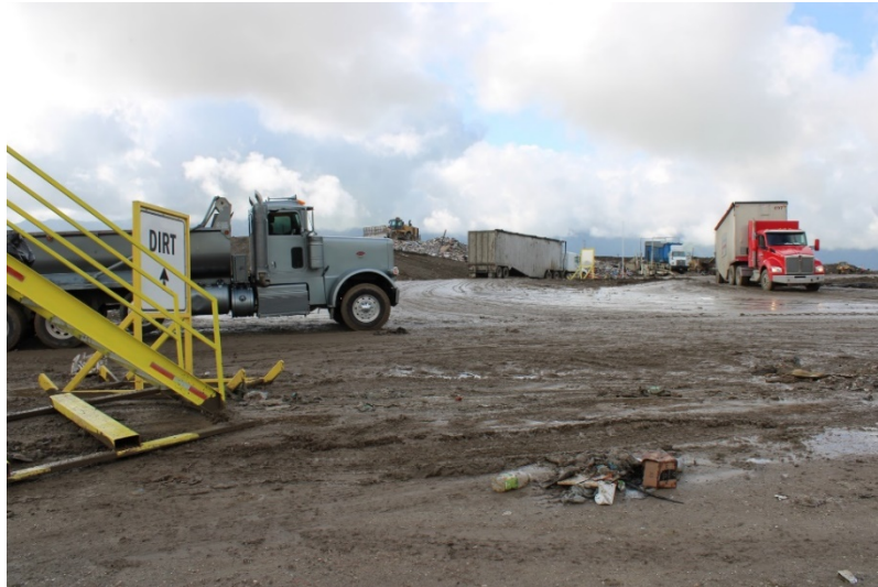
Photo 37: Top Deck Working Area: March 23, 2023
