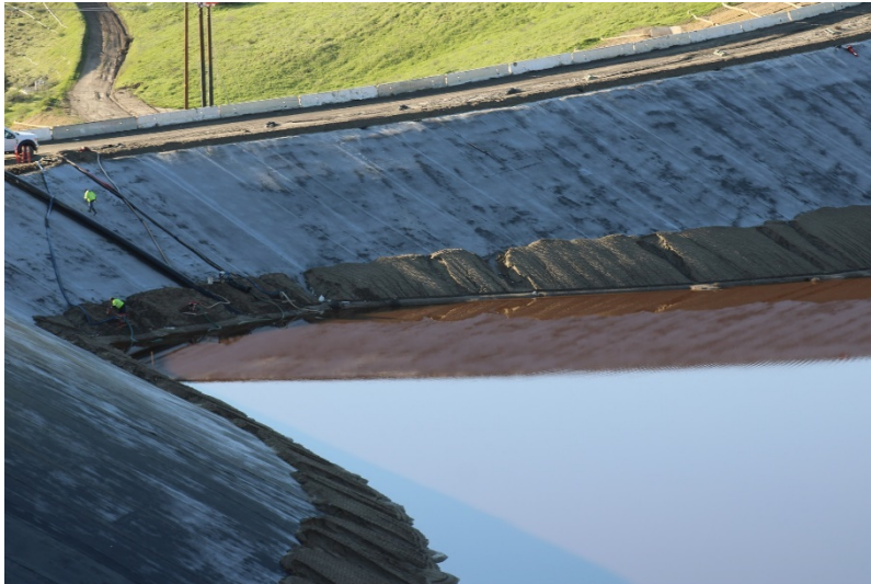
Photo 281: Cell 8 Construction: January 19, 2023
