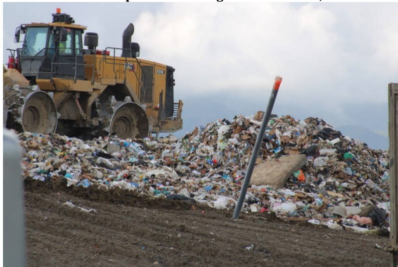
Photo 39: Top Deck Working Area: March 23, 2023
