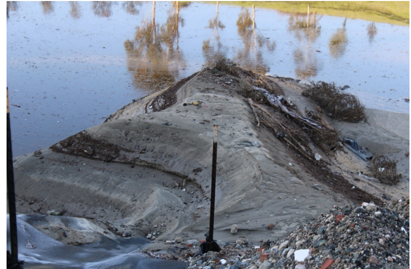
Photo 74: South Terminal and Catch Basins: January 19, 2023
