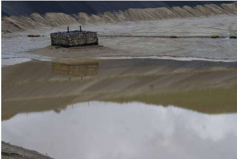
Photo 317: Cell 8 Construction: March 23, 2023
