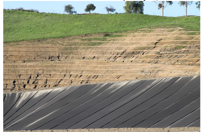
Photo 284: Cell 8 Construction: January 19, 2023
