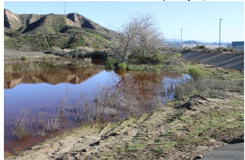
Photo 120: Northeast Sediment Basin: January 19, 2023
