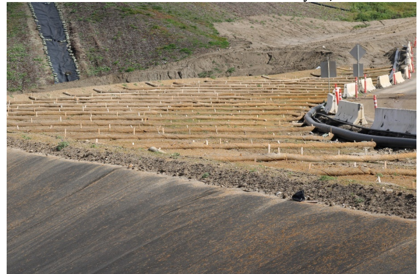
Photo 308: Cell 8 Construction: February 28, 2023
