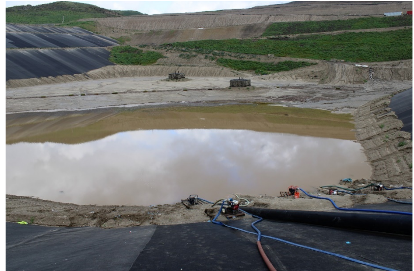
Photo 314: Cell 8 Construction: March 23, 2023
