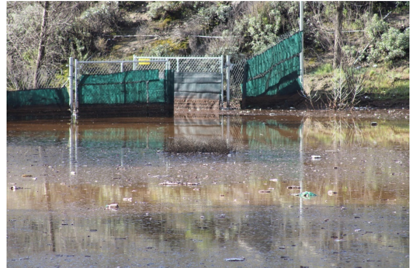
Photo 94: South Terminal and Catch Basins: February 28, 2023
