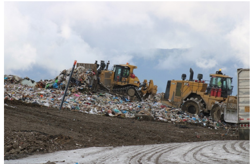
Photo 54: Top Deck Working Area: March 23, 2023
