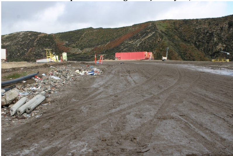
Photo 23: Top Deck Working Area: February 28, 2023
