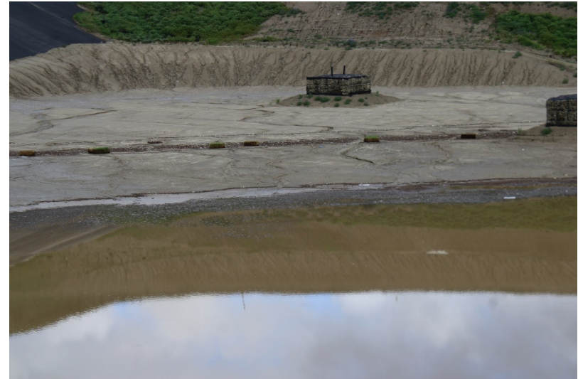
Photo 318: Cell 8 Construction: March 23, 2023
