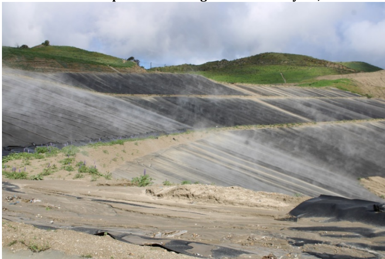
Photo 35: Top Deck Working Area: March 23, 2023
