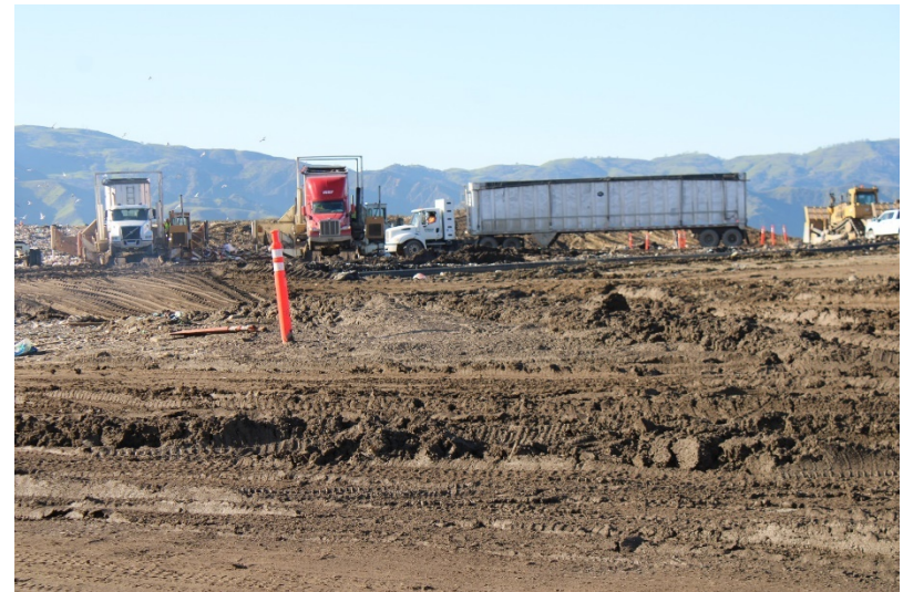
Photo 6: Top Deck Working Area: January 19, 2023
