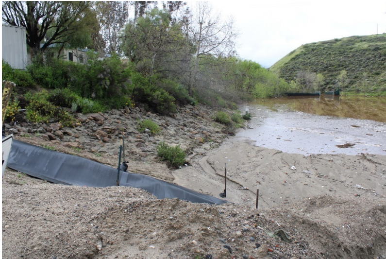
Photo 109: South Terminal and Catch Basins: March 23, 2023
