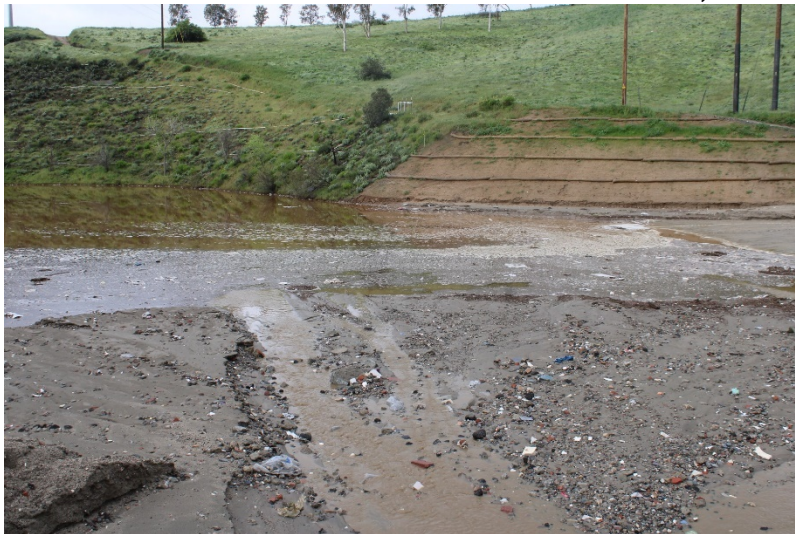
Photo 111: South Terminal and Catch Basins: March 23, 2023
