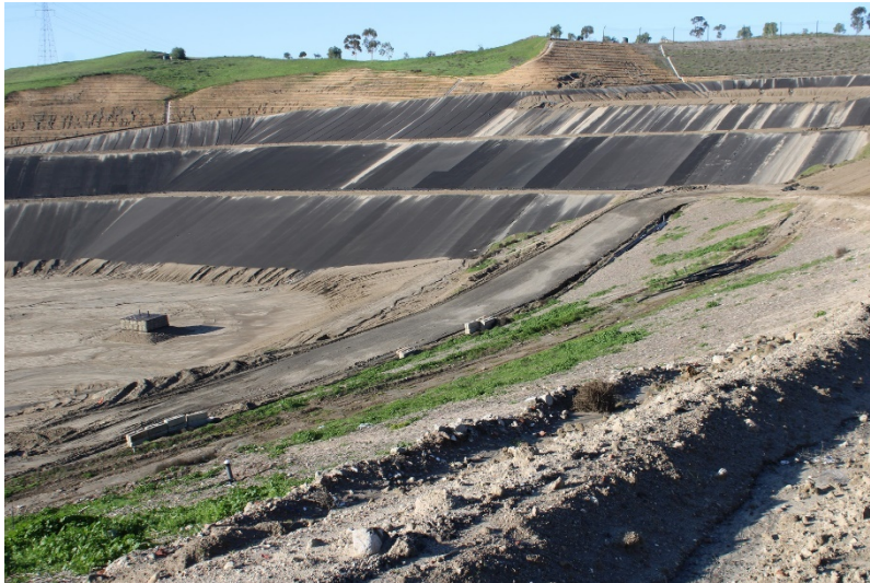
Photo 277: Cell 8 Construction: January 19, 2023
