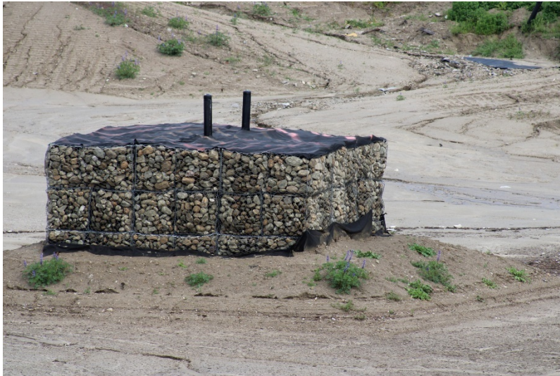
Photo 325: Cell 8 Construction: March 23, 2023
