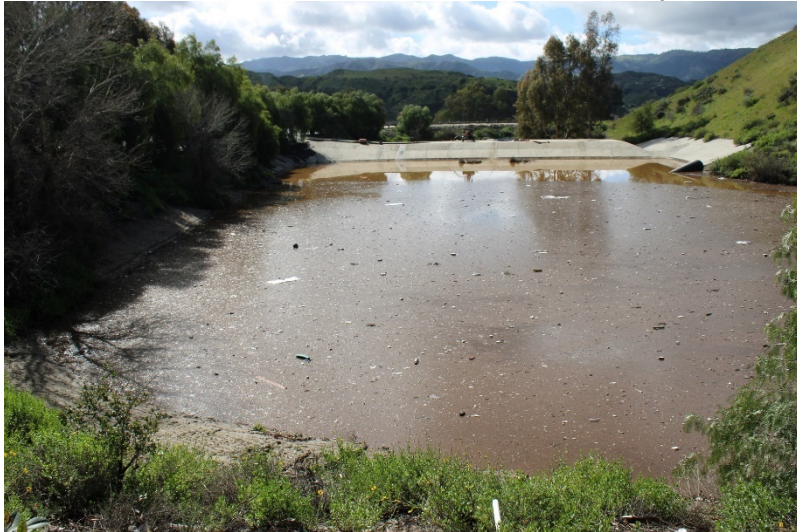
Photo 95: South Terminal and Catch Basins: February 28, 2023
