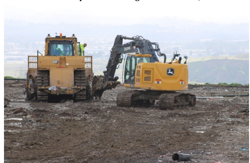
Photo 48: Top Deck Working Area: March 23, 2023
