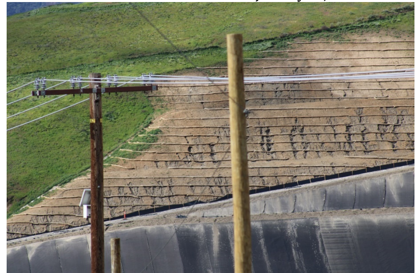
Photo 288: Cell 8 Construction: February 28, 2023
