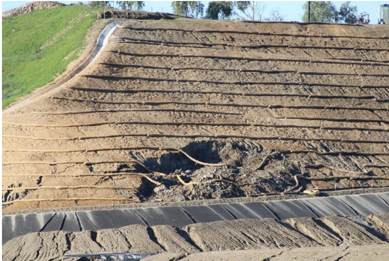
Photo 285: Cell 8 Construction: January 19, 2023
