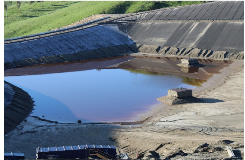
Photo 278: Cell 8 Construction: January 19, 2023
