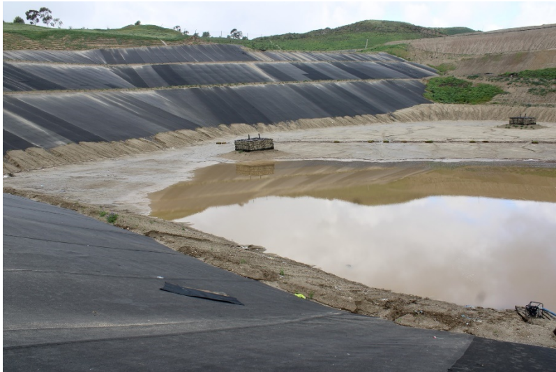
Photo 313: Cell 8 Construction: March 23, 2023
