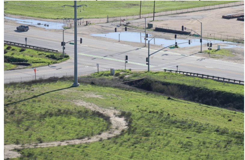
Photo 152: Wolcott Way Entrance Facilities: January 19, 2023
