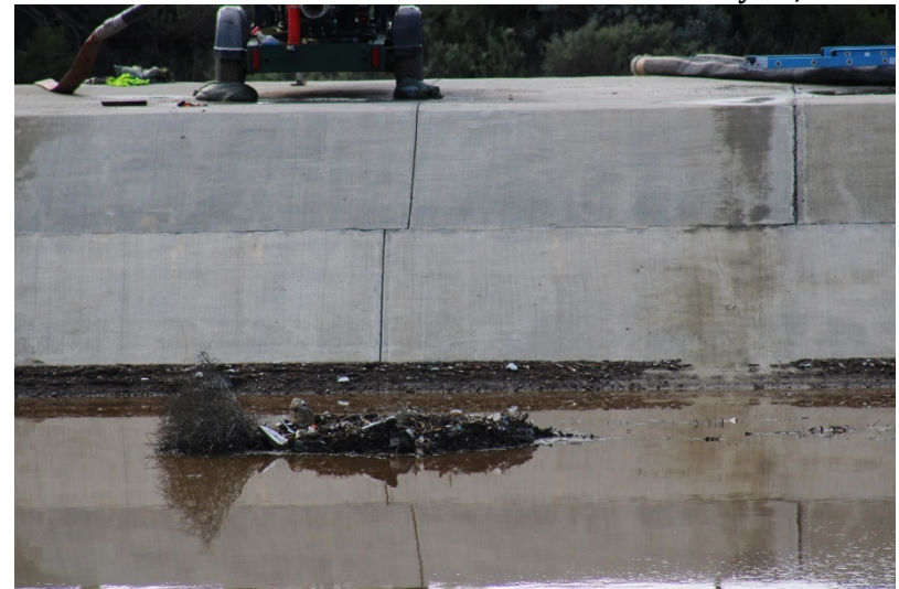
Photo 100: South Terminal and Catch Basins: February 28, 2023
