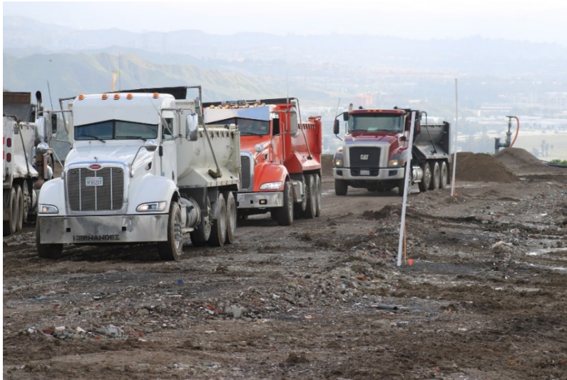
Photo 49: Top Deck Working Area: March 23, 2023
