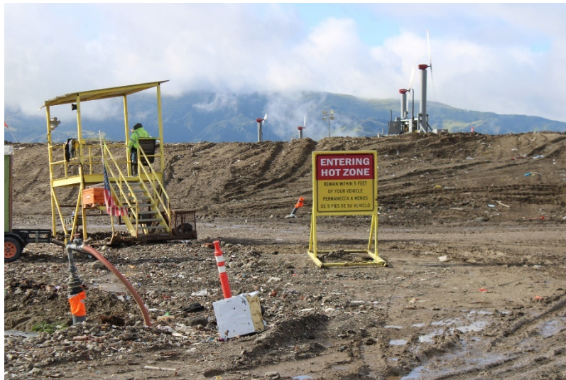
Photo 29: Top Deck Working Area: February 28, 2023
