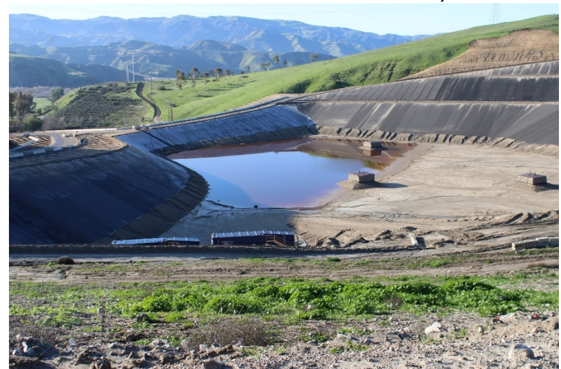
Photo 276: Cell 8 Construction: January 19, 2023
