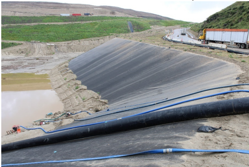
Photo 315: Cell 8 Construction: March 23, 2023
