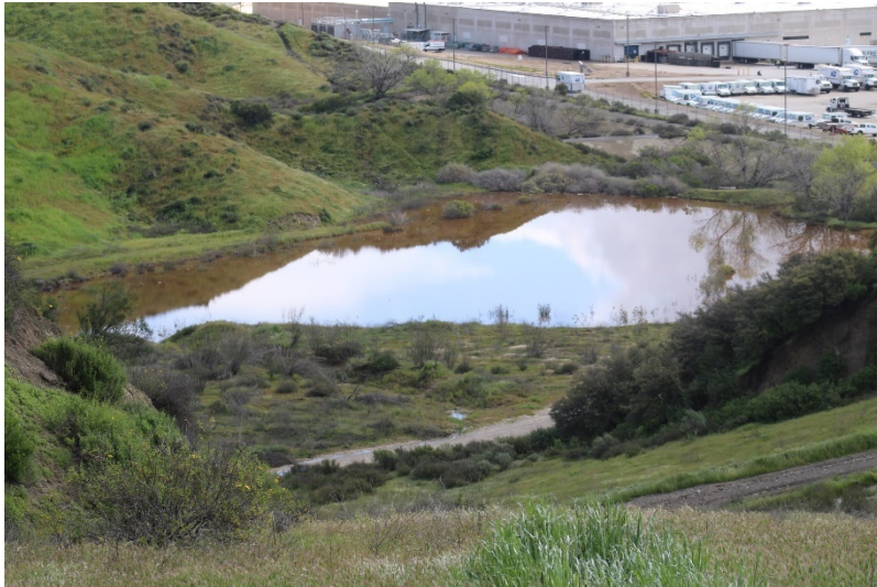
Photo 125: Northeast Sediment Basin: March 23, 2023
