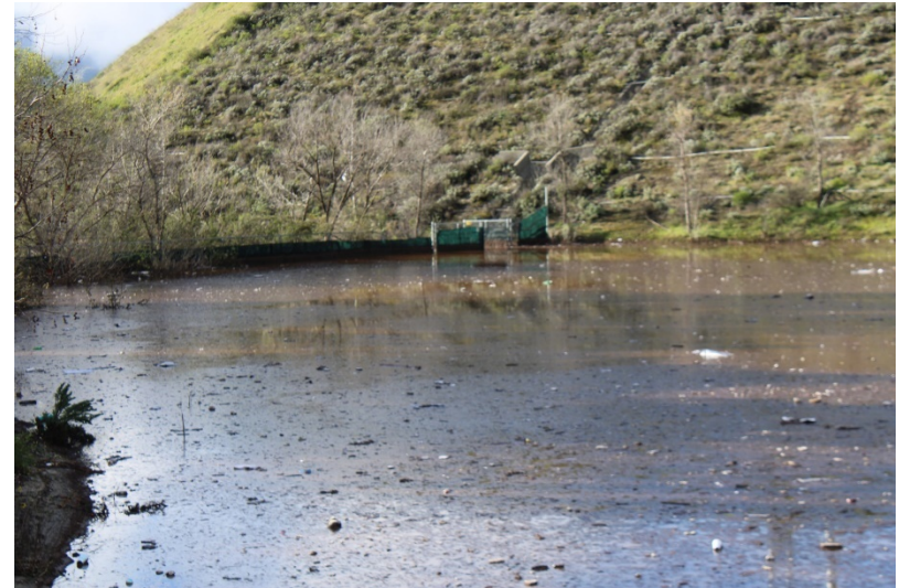
Photo 90: South Terminal and Catch Basins: February 28, 2023
