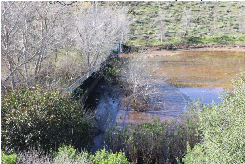
Photo 83: South Terminal and Catch Basins: January 19, 2023
