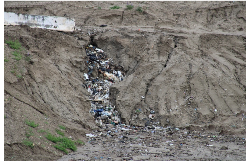
Photo 326: Cell 8 Construction: March 23, 2023
