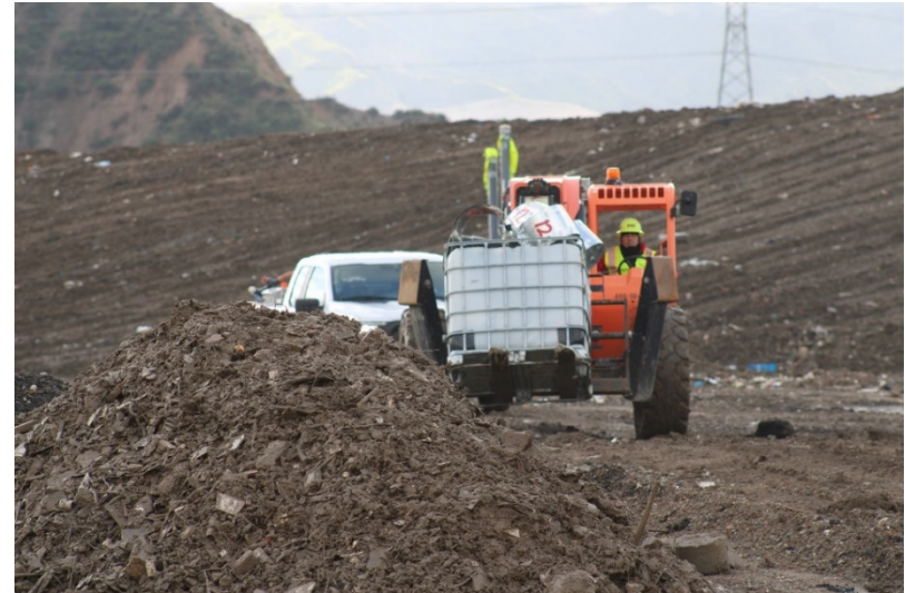
Photo 50: Top Deck Working Area: March 23, 2023
