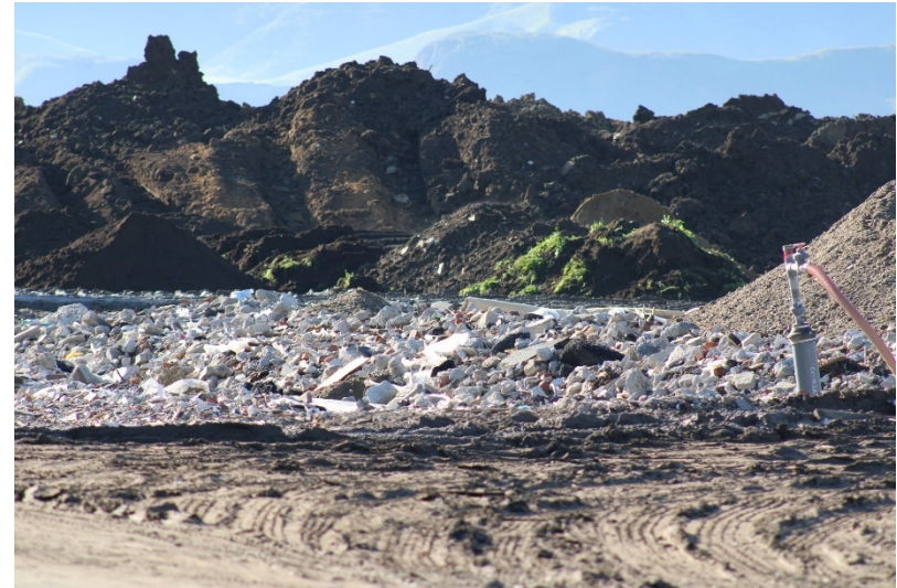
Photo 14: Top Deck Working Area: January 19, 2023
