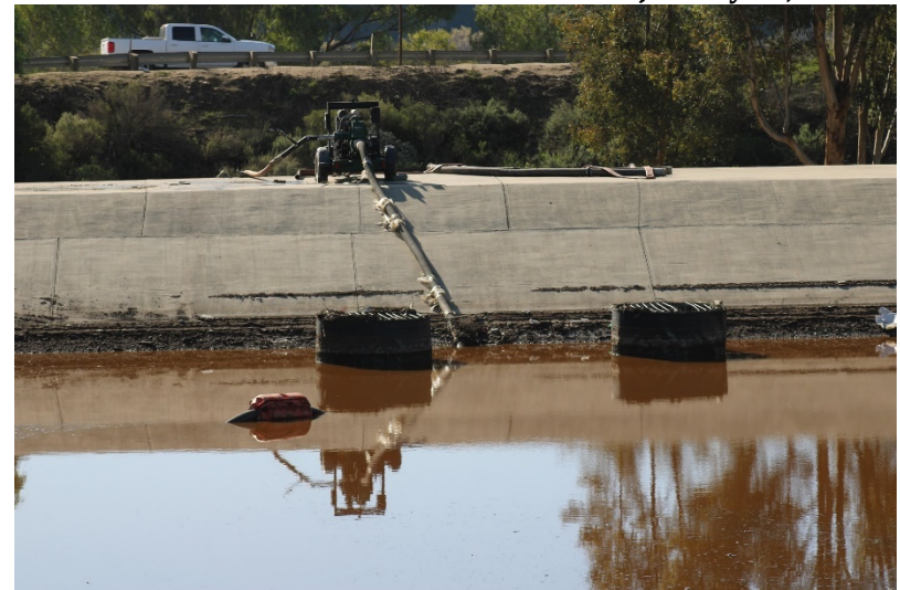
Photo 80: South Terminal and Catch Basins: January 19, 2023
