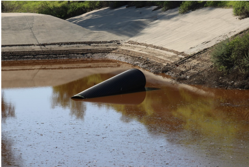
Photo 81: South Terminal and Catch Basins: January 19, 2023
