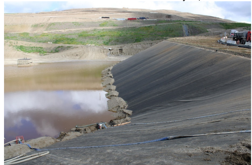
Photo 296: Cell 8 Construction: February 28, 2023
