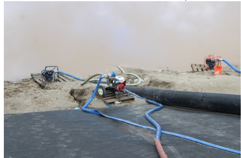
Photo 320: Cell 8 Construction: March 23, 2023
