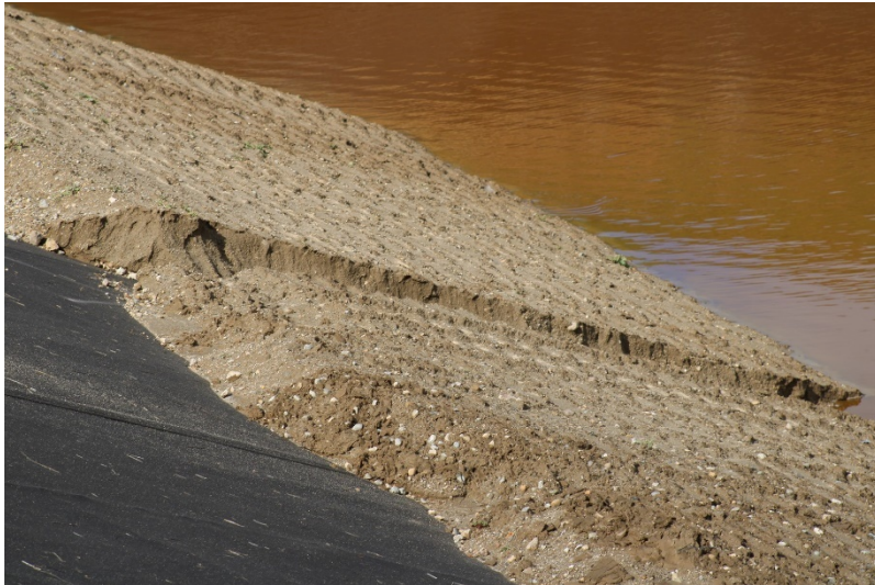
Photo 301: Cell 8 Construction: February 28, 2023
