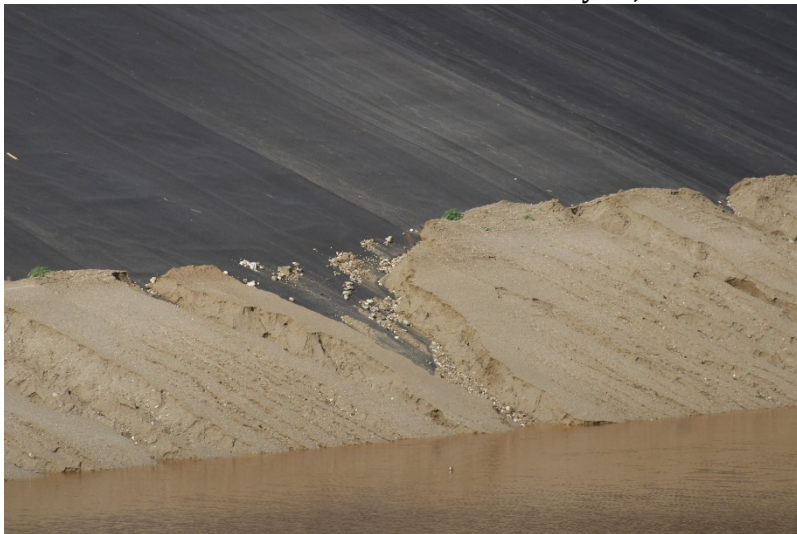
Photo 303: Cell 8 Construction: February 28, 2023
