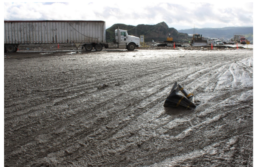
Photo 26: Top Deck Working Area: February 28, 2023
