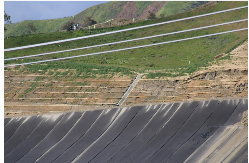
Photo 290: Cell 8 Construction: February 28, 2023
