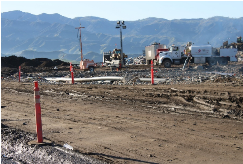
Photo 5: Top Deck Working Area: January 19, 2023
