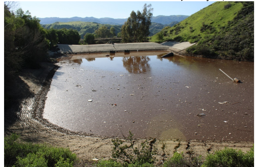
Photo 76: South Terminal and Catch Basins: January 19, 2023
