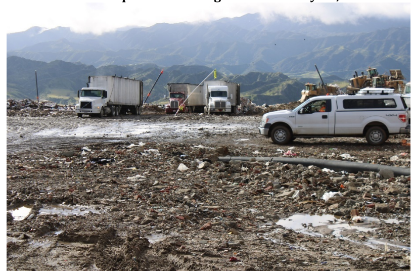
Photo 28: Top Deck Working Area: February 28, 2023
