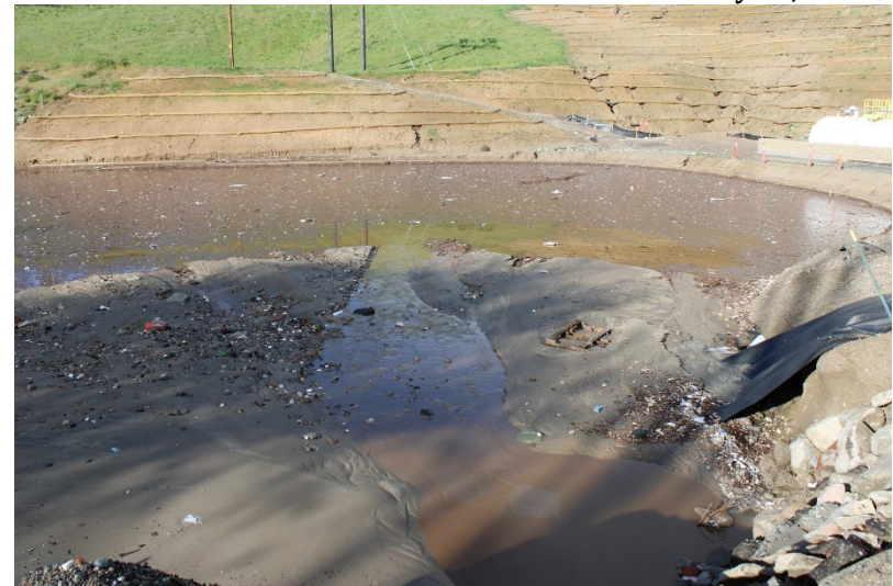
Photo 88: South Terminal and Catch Basins: February 28, 2023
