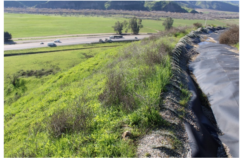
Photo 150: Wolcott Way Entrance Facilities: January 19, 2023
