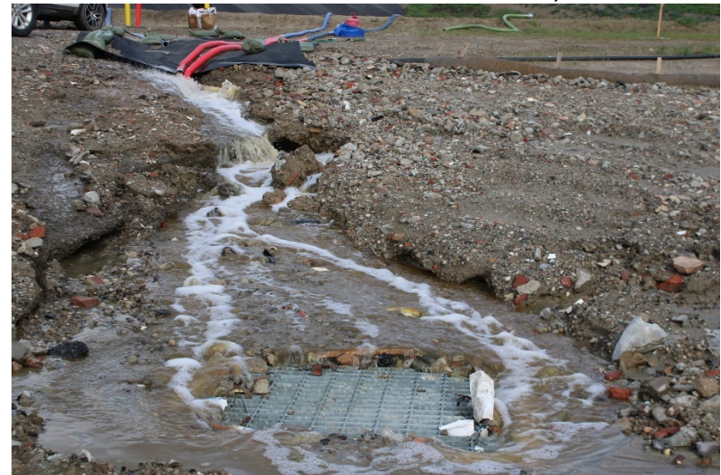
Photo 328: Cell 8 Construction: March 23, 2023
