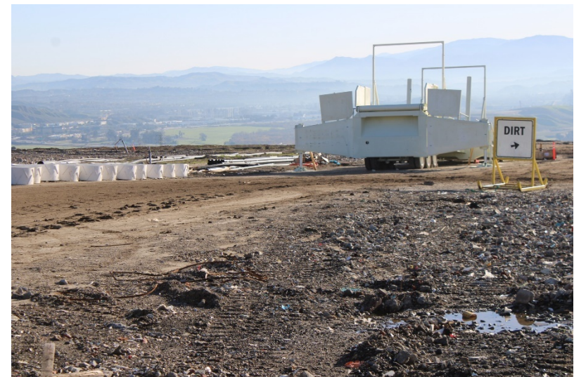
Photo 2: Top Deck Working Area: January 19, 2023
