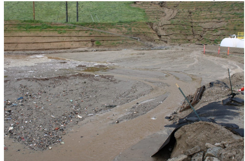
Photo 112: South Terminal and Catch Basins: March 23, 2023
