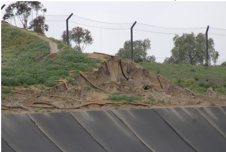
Photo 327: Cell 8 Construction: March 23, 2023
