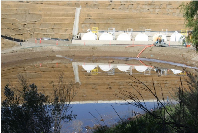
Photo 85: South Terminal and Catch Basins: January 19, 2023
