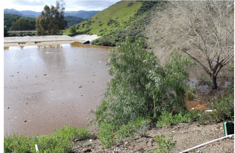
Photo 96: South Terminal and Catch Basins: February 28, 2023
