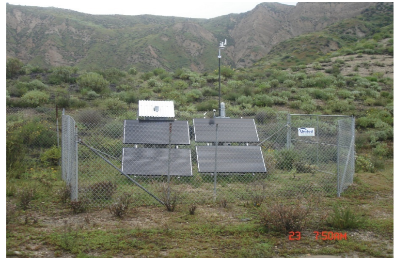
Photo 162: Wolcott Way Entrance Facilities: March 23, 2023
