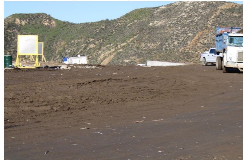
Photo 8: Top Deck Working Area: January 19, 2023
