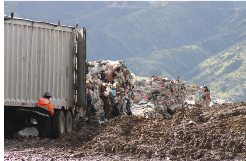
Photo 34: Top Deck Working Area: February 28, 2023
