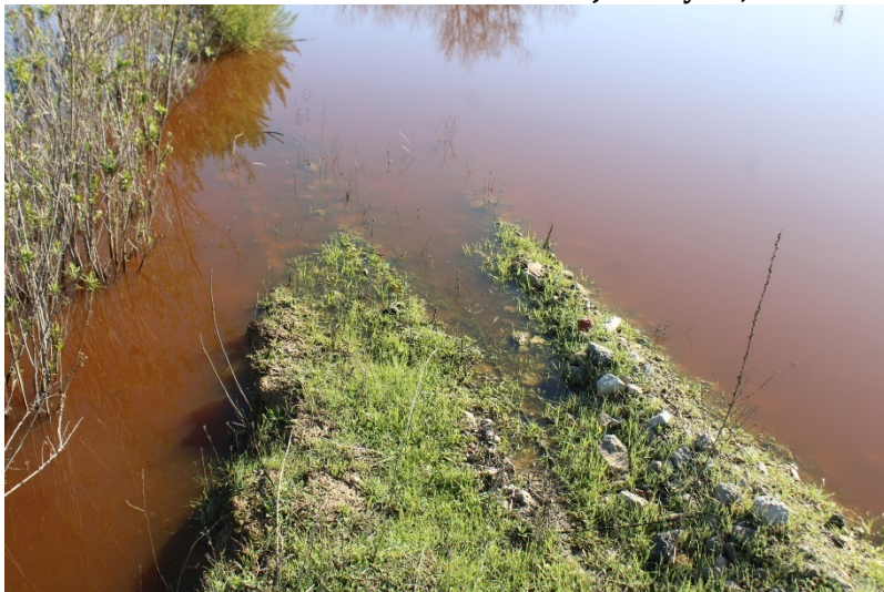
Photo 119: Northeast Sediment Basin: January 19, 2023
