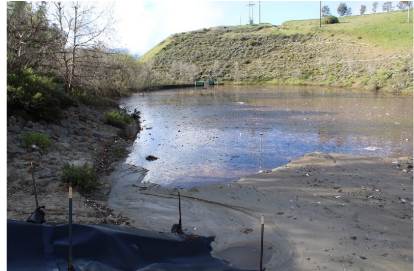
Photo 86: South Terminal and Catch Basins: February 28, 2023
