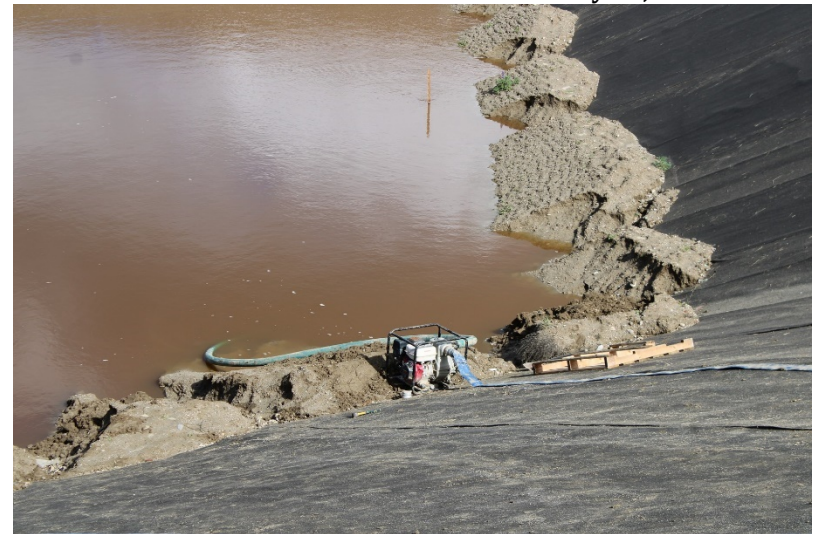
Photo 300: Cell 8 Construction: February 28, 2023
