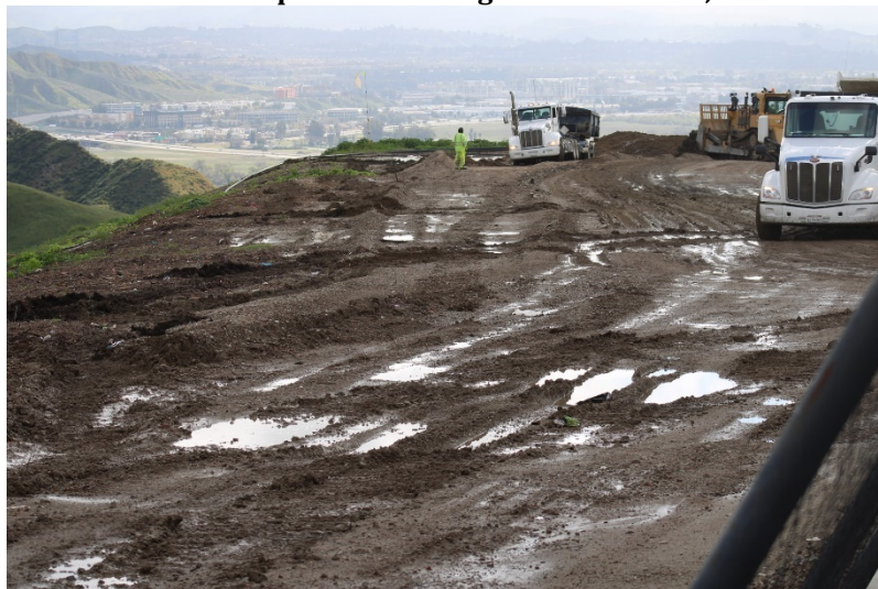
Photo 55: Top Deck Working Area: March 23, 2023
