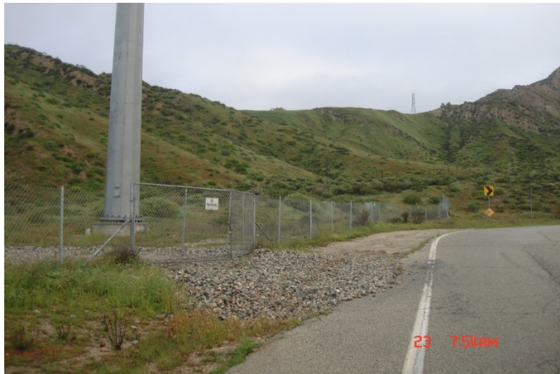
Photo 161: Wolcott Way Entrance Facilities: March 23, 2023
