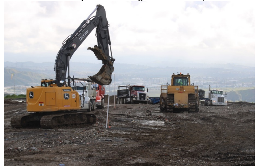
Photo 44: Top Deck Working Area: March 23, 2023
