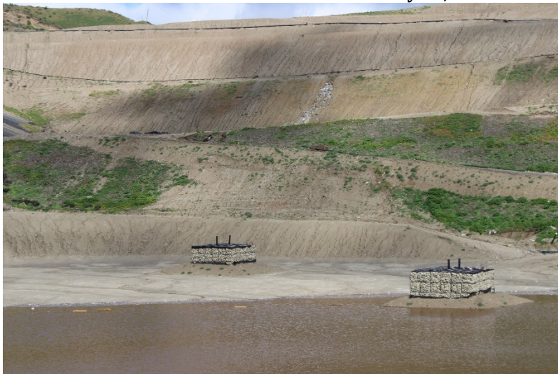
Photo 299: Cell 8 Construction: February 28, 2023
