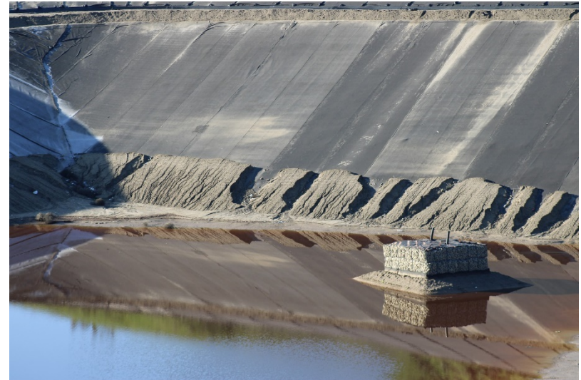
Photo 282: Cell 8 Construction: January 19, 2023
