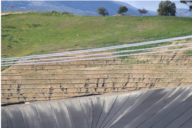
Photo 289: Cell 8 Construction: February 28, 2023
