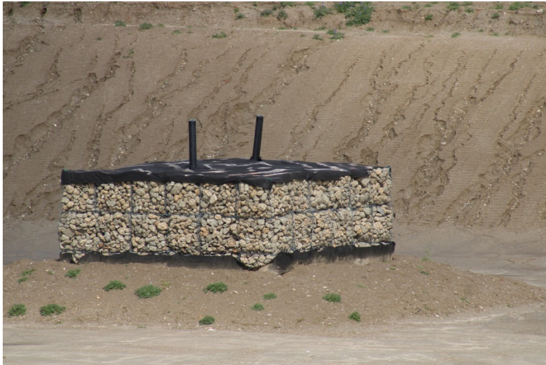
Photo 305: Cell 8 Construction: February 28, 2023
