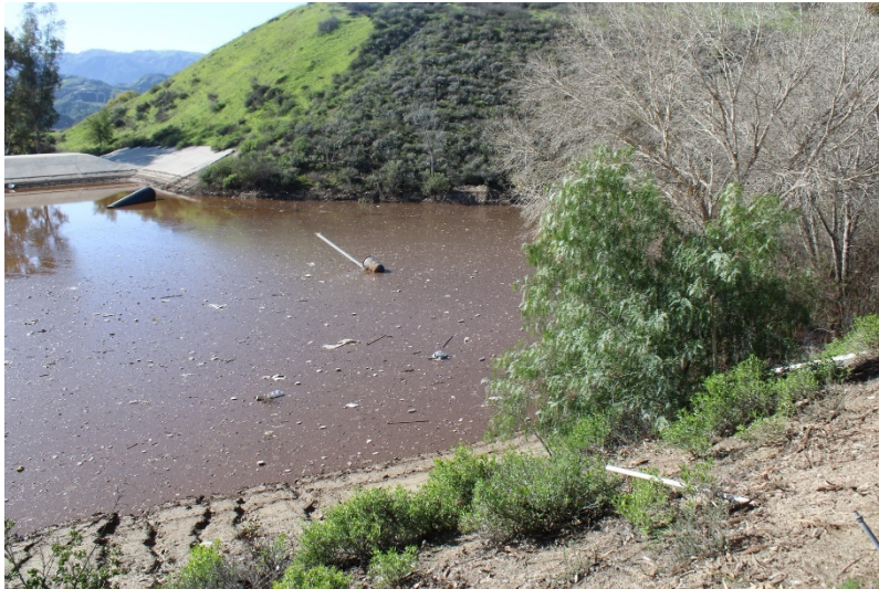
Photo 77: South Terminal and Catch Basins: January 19, 2023
