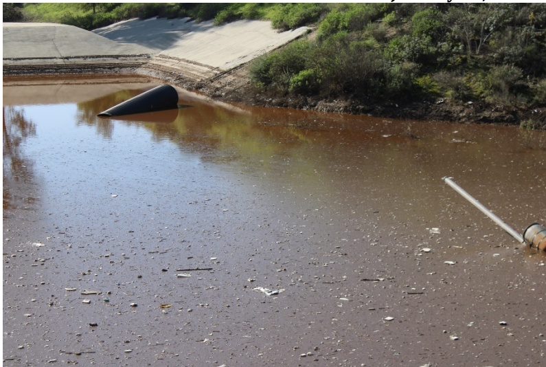
Photo 79: South Terminal and Catch Basins: January 19, 2023
