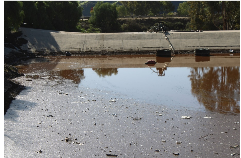
Photo 78: South Terminal and Catch Basins: January 19, 2023
