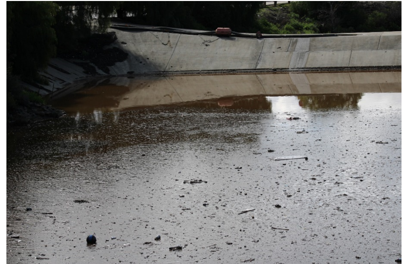
Photo 98: South Terminal and Catch Basins: February 28, 2023
