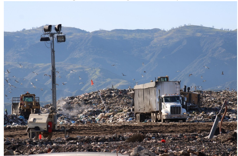
Photo 20: Top Deck Working Area: January 19, 2023
