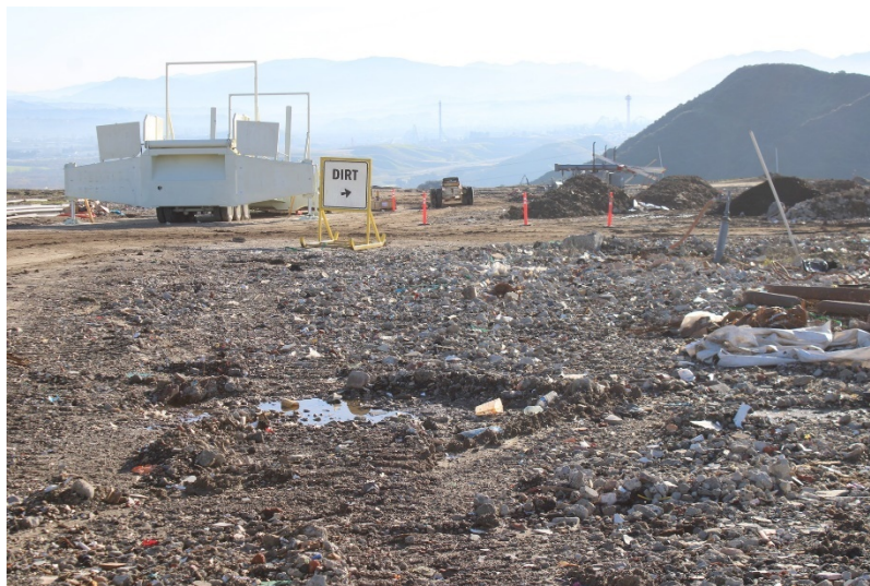
Photo 1: Top Deck Working Area: January 19, 2023
