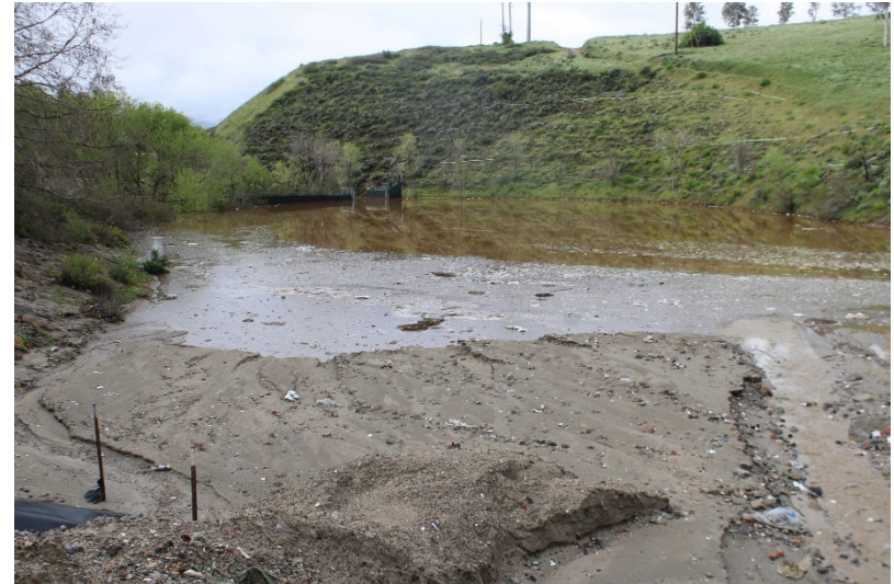
Photo 110: South Terminal and Catch Basins: March 23, 2023
