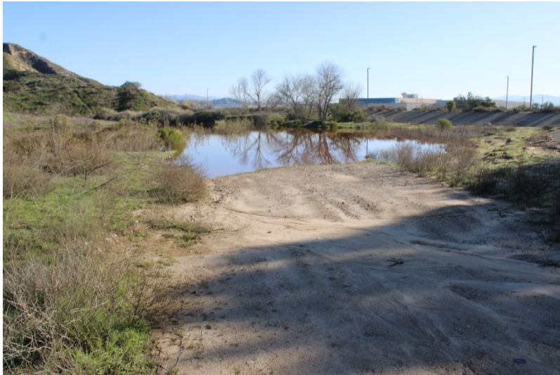
Photo 117: Northeast Sediment Basin: January 19, 2023
