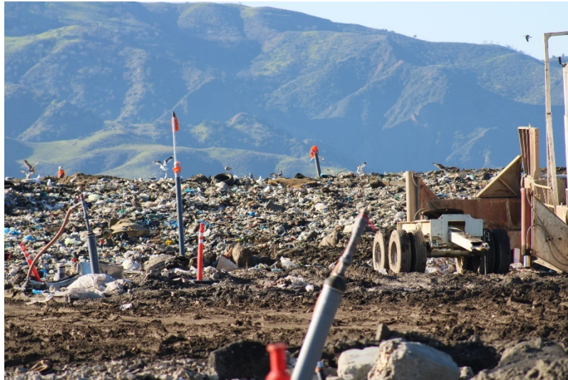
Photo 17: Top Deck Working Area: January 19, 2023
