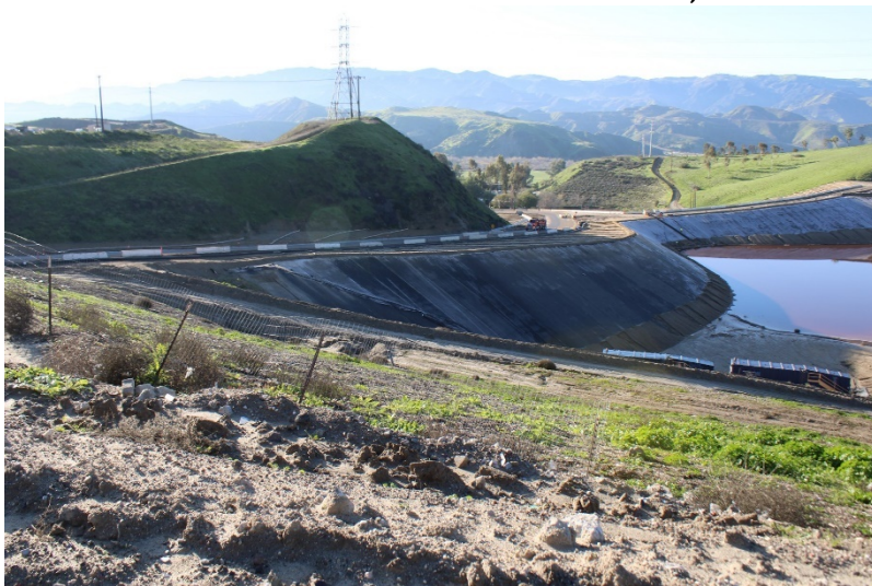
Photo 275: Cell 8 Construction: January 19, 2023
