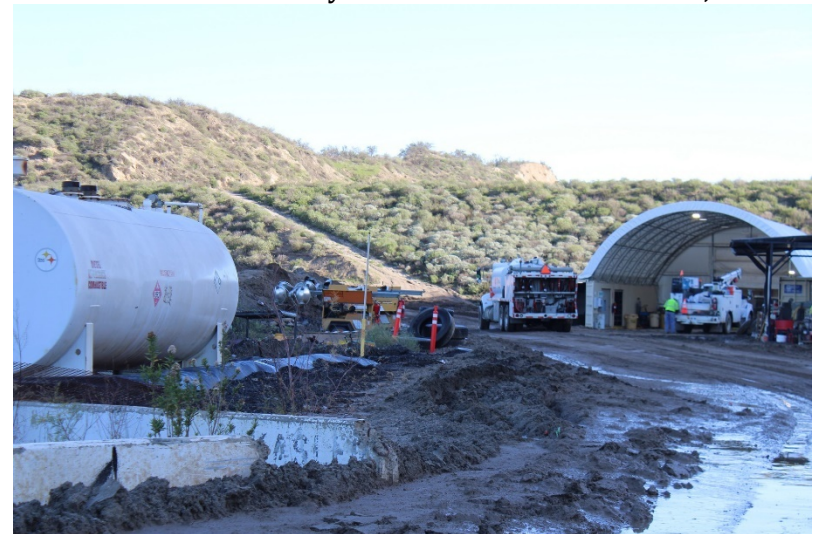
Photo 168: Maintenance and Admin Buildings: January 19, 2023
