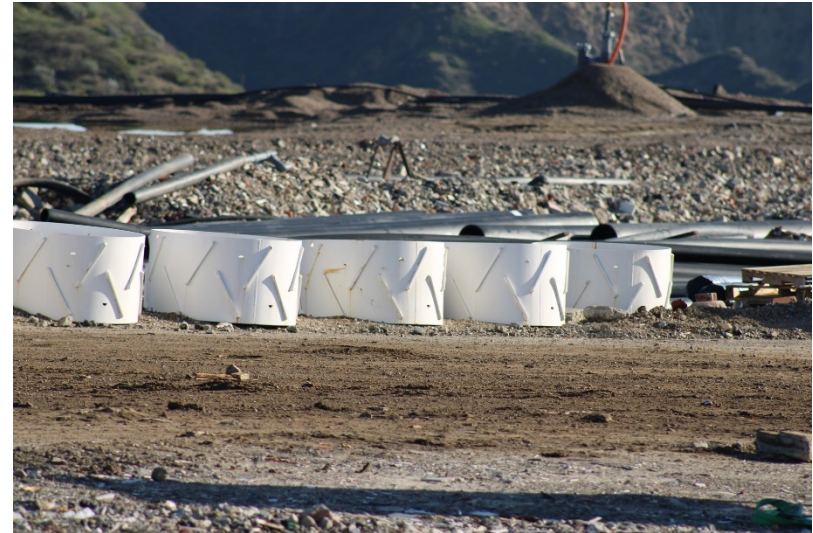
Photo 10: Top Deck Working Area: January 19, 2023
