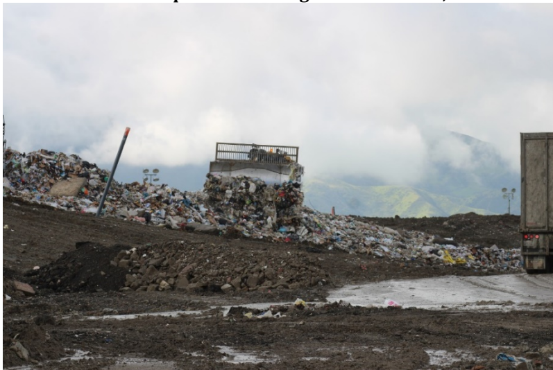
Photo 47: Top Deck Working Area: March 23, 2023
