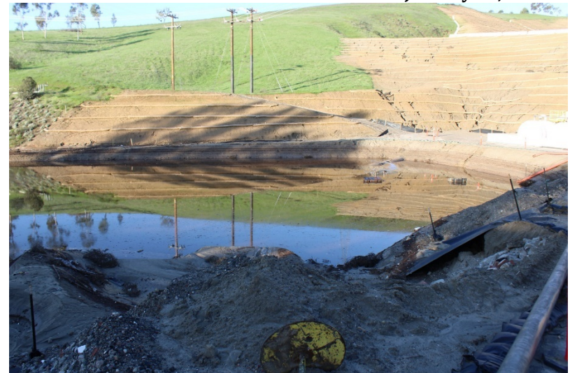
Photo 72: South Terminal and Catch Basins: January 19, 2023
