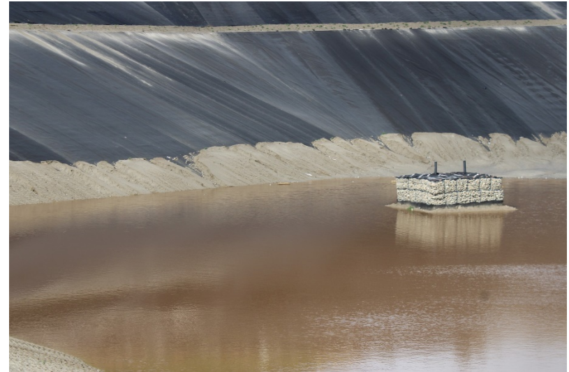
Photo 298: Cell 8 Construction: February 28, 2023
