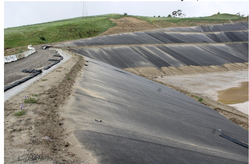
Photo 312: Cell 8 Construction: March 23, 2023
