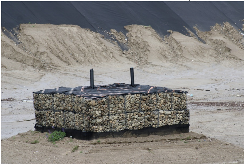
Photo 323: Cell 8 Construction: March 23, 2023
