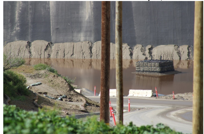
Photo 292: Cell 8 Construction: February 28, 2023
