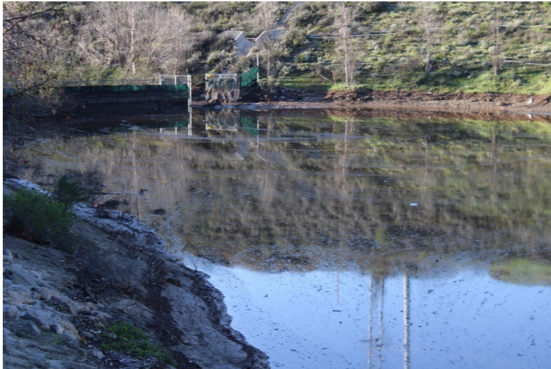
Photo 73: South Terminal and Catch Basins: January 19, 2023
