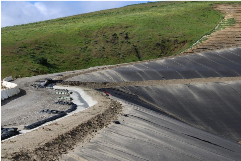
Photo 297: Cell 8 Construction: February 28, 2023
