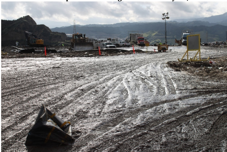
Photo 27: Top Deck Working Area: February 28, 2023
