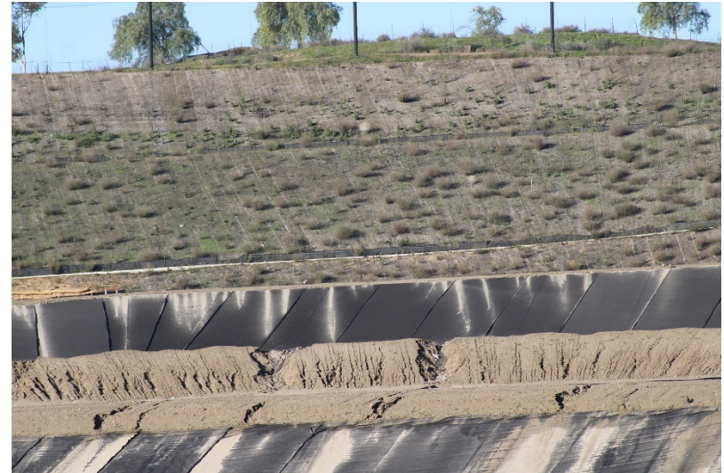
Photo 286: Cell 8 Construction: January 19, 2023
