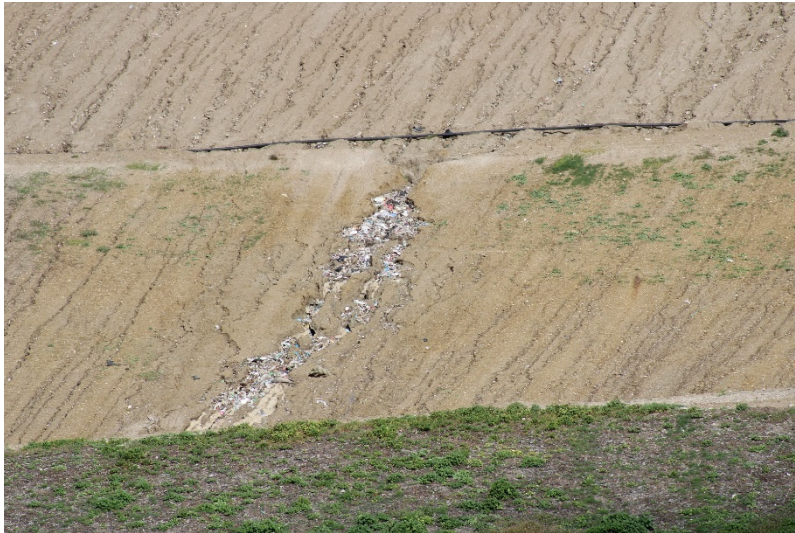
Photo 309: Cell 8 Construction: February 28, 2023
