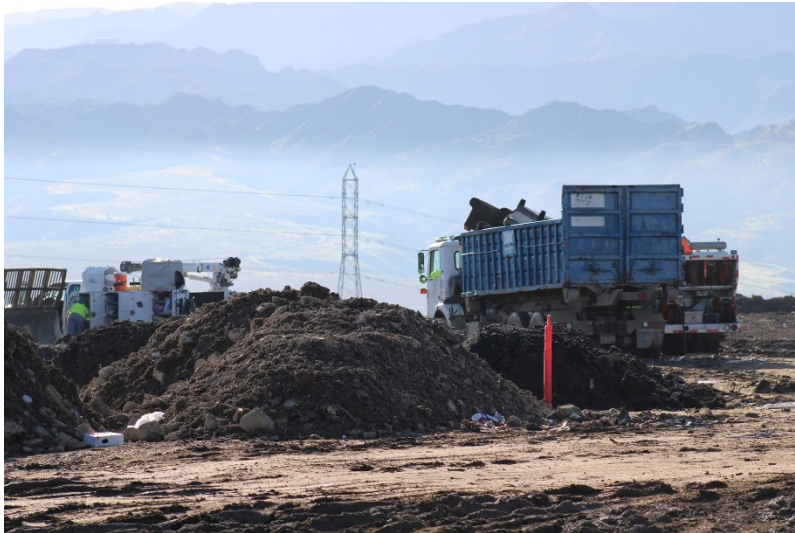
Photo 13: Top Deck Working Area: January 19, 2023
