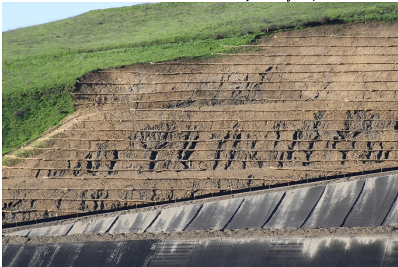
Photo 283: Cell 8 Construction: January 19, 2023
