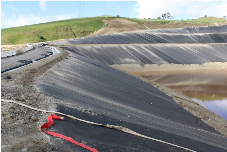
Photo 293: Cell 8 Construction: February 28, 2023
