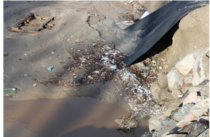
Photo 92: South Terminal and Catch Basins: February 28, 2023
