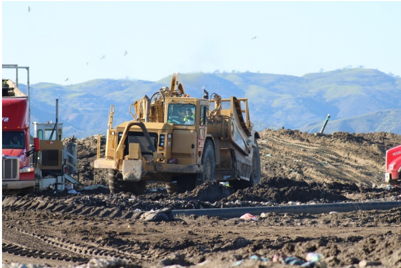
Photo 21: Top Deck Working Area: January 19, 2023
