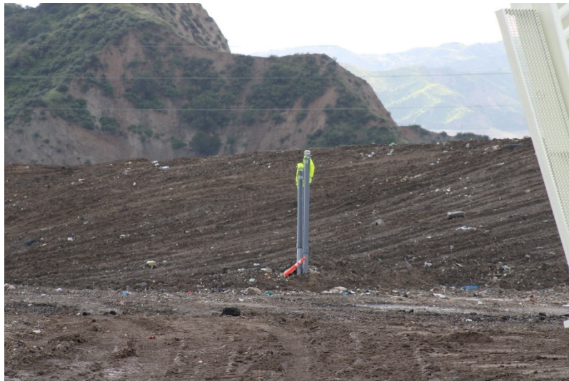
Photo 53: Top Deck Working Area: March 23, 2023
