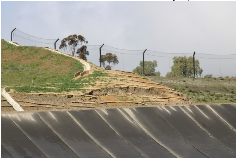
Photo 311: Cell 8 Construction: February 28, 2023
