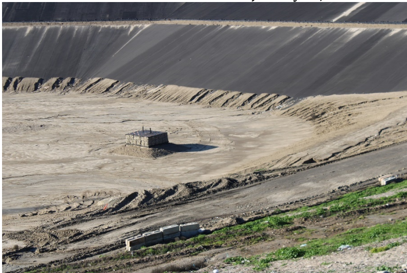
Photo 279: Cell 8 Construction: January 19, 2023
