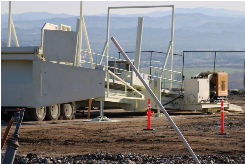
Photo 11: Top Deck Working Area: January 19, 2023
