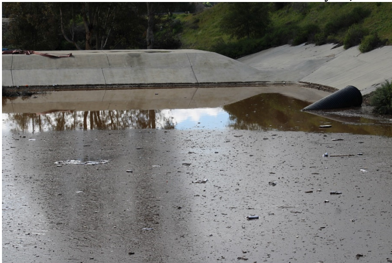
Photo 99: South Terminal and Catch Basins: February 28, 2023
