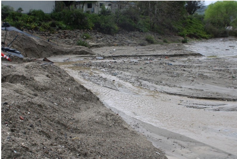
Photo 113: South Terminal and Catch Basins: March 23, 2023
