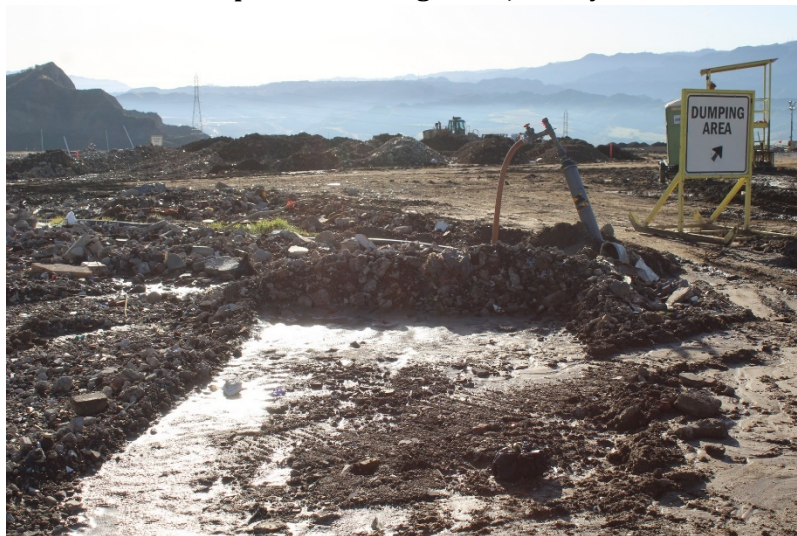
Photo 3: Top Deck Working Area: January 19, 2023
