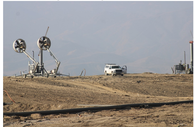
Photo 8: Top Deck Working Area: October 12, 2022
