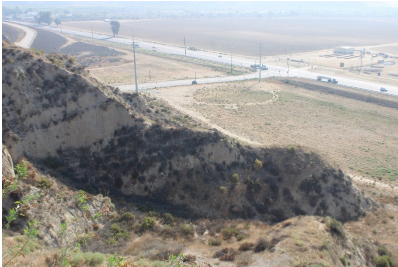
Photo 237: Wolcott Way Entrance Facilities: October 12, 2022
