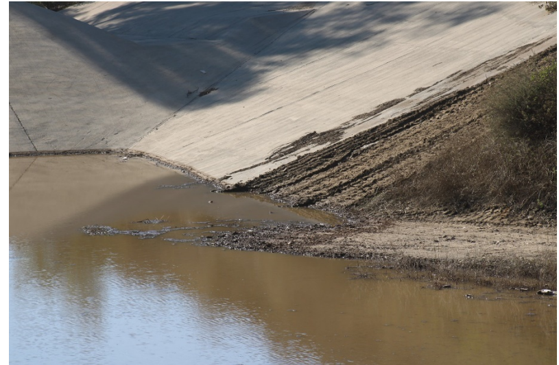
Photo 178: South Terminal and Catch Basins: December 14, 2022
