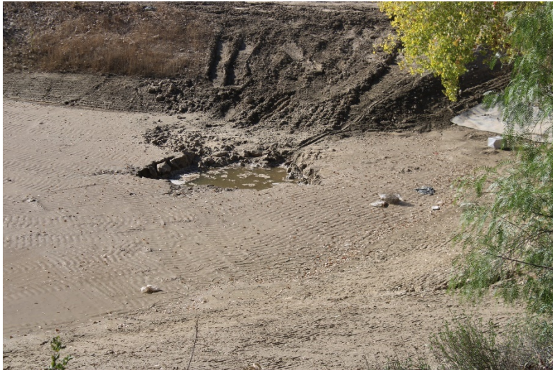
Photo 157: South Terminal and Catch Basins: November 30, 2022
