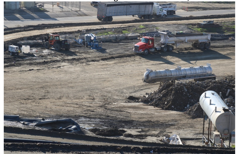
Photo 80: Cell 6 Working Area: December 14, 2022
