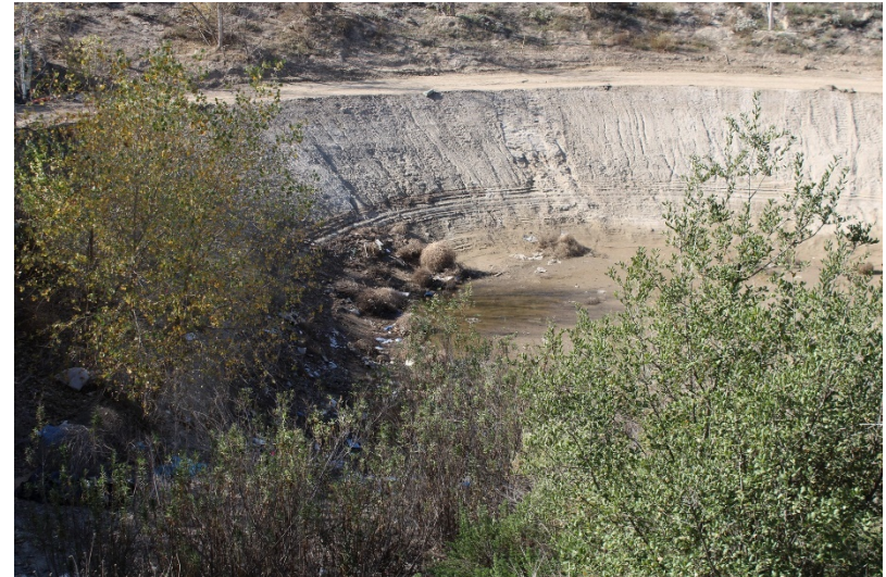
Photo 162: South Terminal and Catch Basins: November 30, 2022
