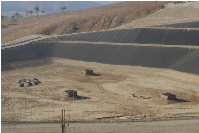
Photo 411: Cell 8 Construction: October 12, 2022
