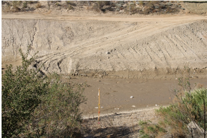
Photo 163: South Terminal and Catch Basins: November 30, 2022
