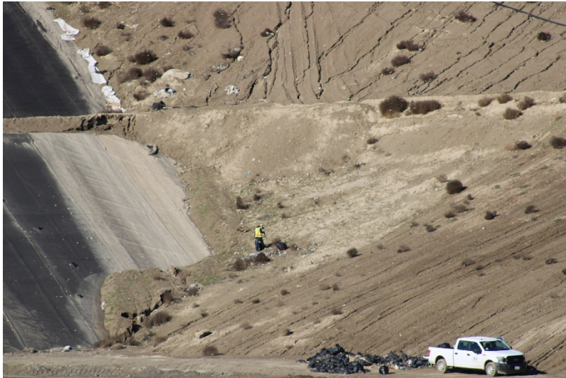
Photo 453: Cell Construction: December 12, 2022
