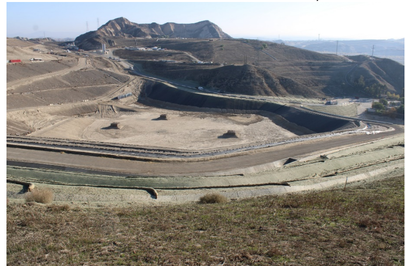
Photo 428: Cell 8 Construction: November 30, 2022
