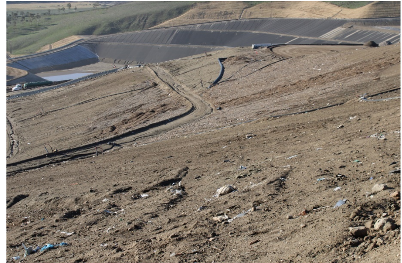
Photo 78: Cell 6 Working Area: December 14, 2022
