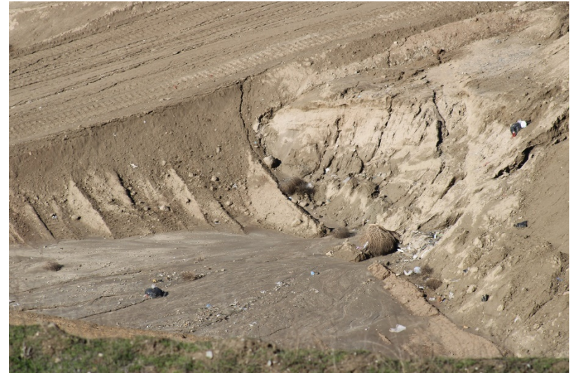
Photo 450: Cell Construction: December 12, 2022
