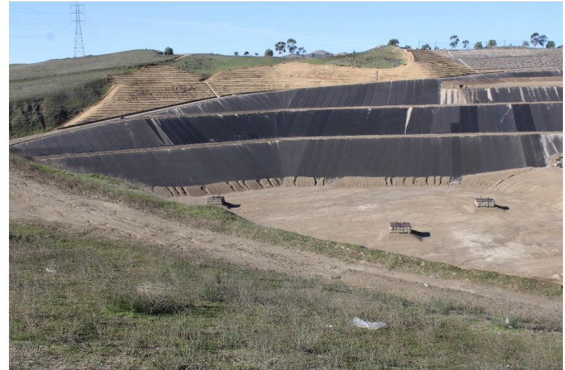
Photo 442: Cell Construction: December 12, 2022
