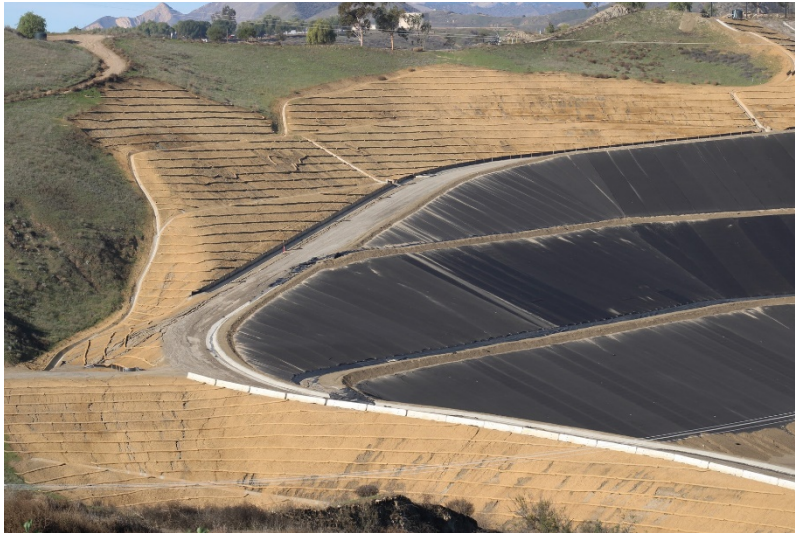
Photo 437: Cell Construction: December 12, 2022
