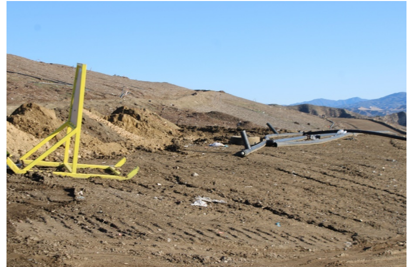
Photo 50: Top Deck Working Area: December 14, 2022
