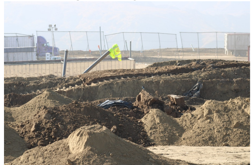
Photo 20: Top Deck Working Area: October 12, 2022
