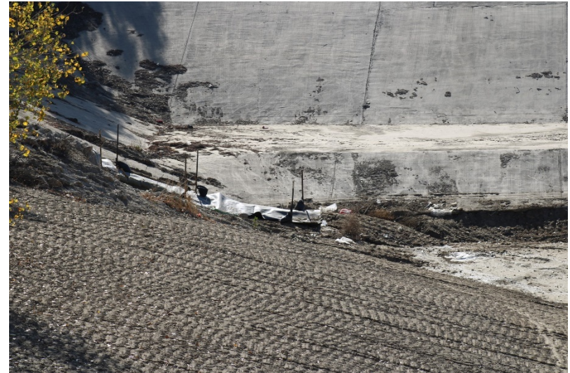
Photo 158: South Terminal and Catch Basins: November 30, 2022
