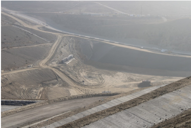
Photo 409: Cell 8 Construction: October 12, 2022
