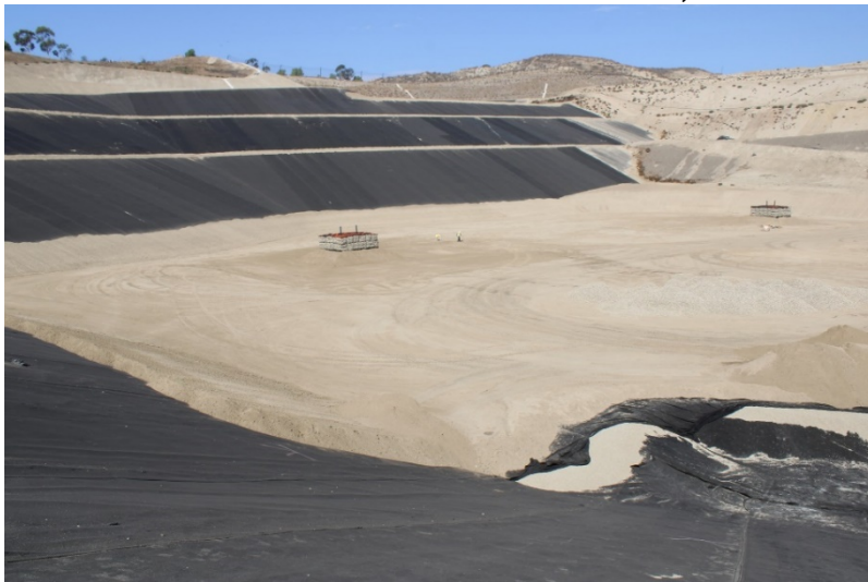
Photo 415: Cell 8 Construction: October 12, 2022
