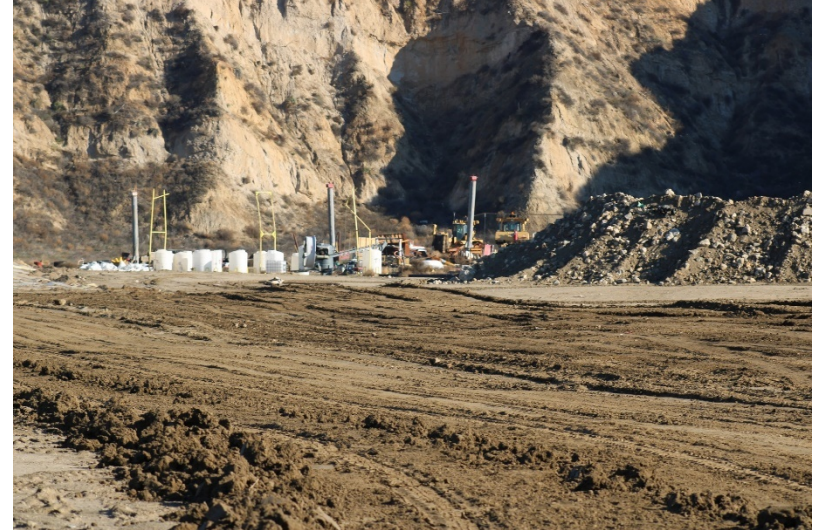
Photo 104: Closed Landfill - Primary Canyon: December 14, 2022
