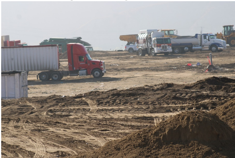
Photo 19: Top Deck Working Area: October 12, 2022
