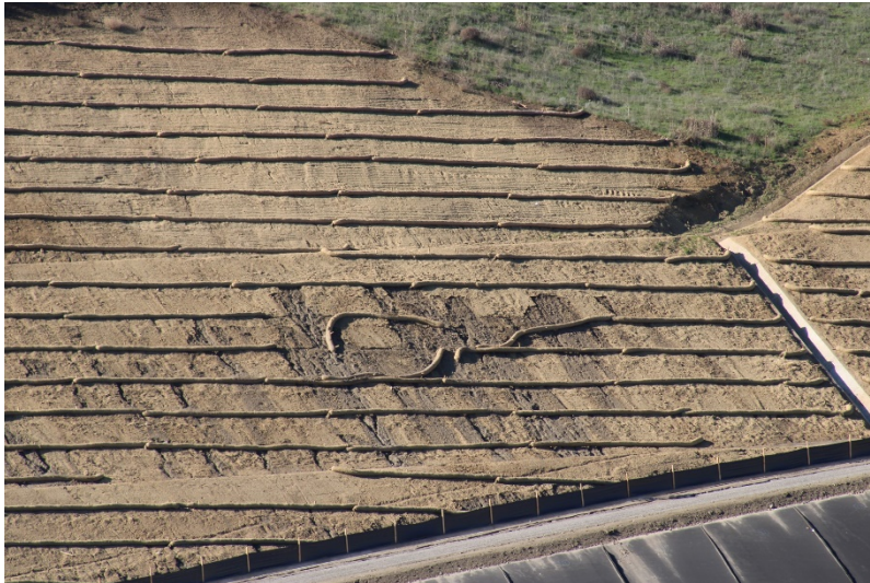
Photo 457: Cell Construction: December 12, 2022
