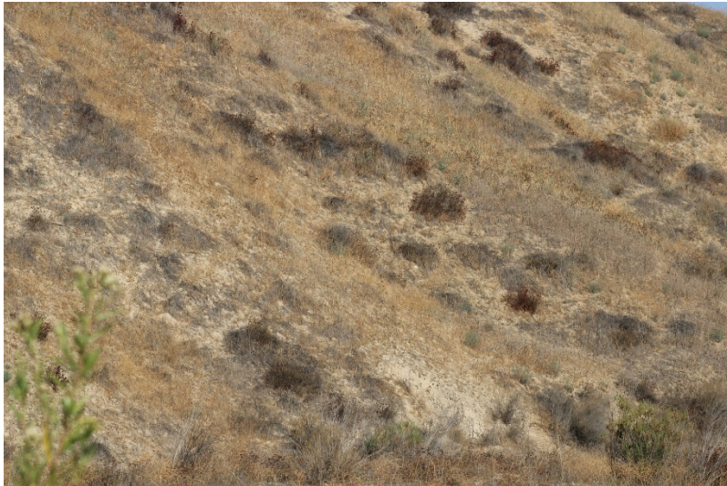
Photo 109: Closed Landfill – Canyon B: October 12, 2022
