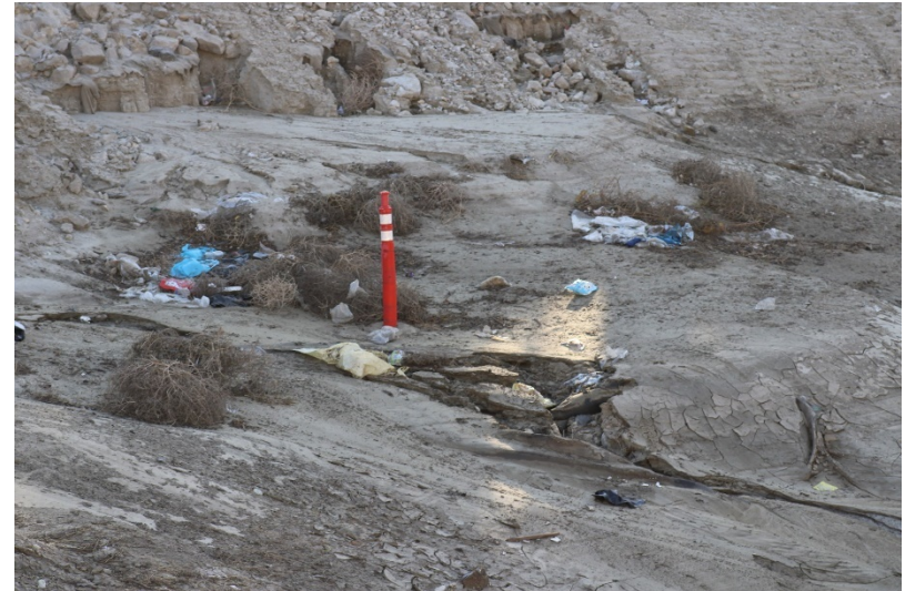
Photo 152: South Terminal and Catch Basins: November 30, 2022
