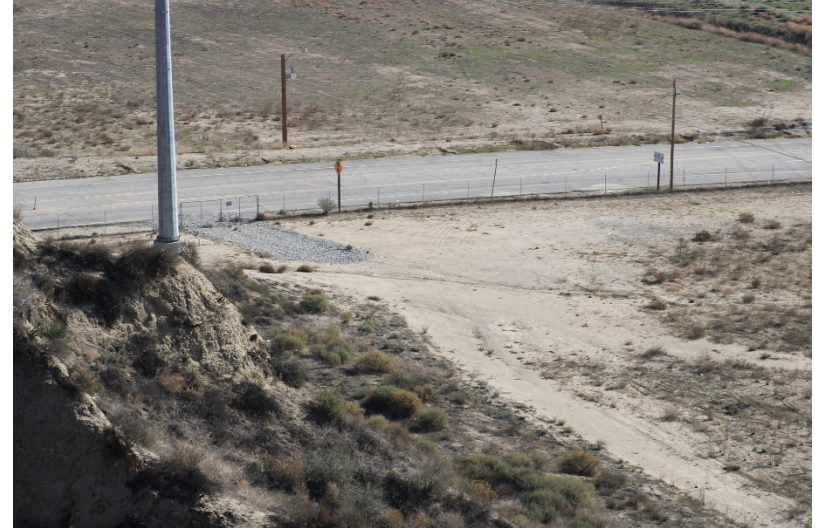
Photo 244: Wolcott Way Entrance Facilities: November 30, 2022
