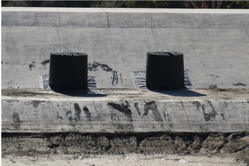
Photo 159: South Terminal and Catch Basins: November 30, 2022
