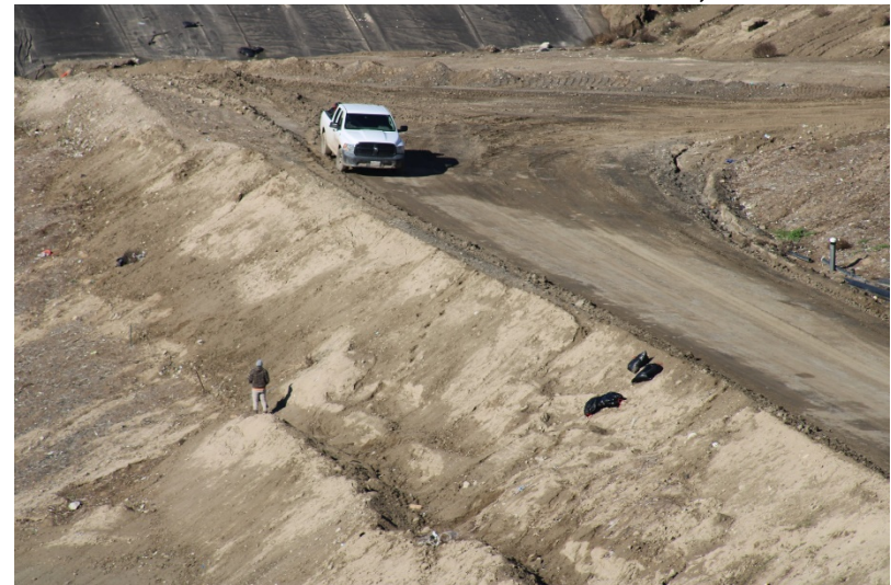
Photo 452: Cell Construction: December 12, 2022
