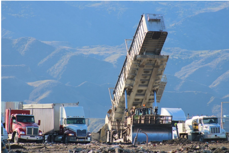
Photo 45: Top Deck Working Area: December 14, 2022
