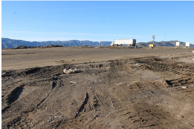
Photo 33: Top Deck Working Area: December 14, 2022
