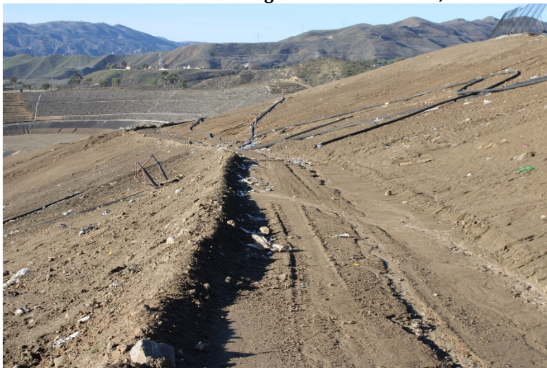
Photo 79: Cell 6 Working Area: December 14, 2022
