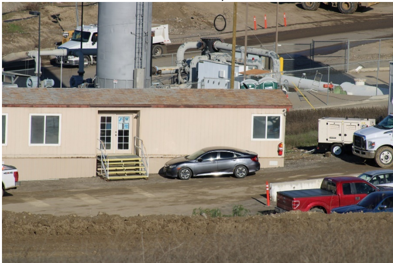
Photo 263: Maintenance and Admin Buildings: December 14, 2022
