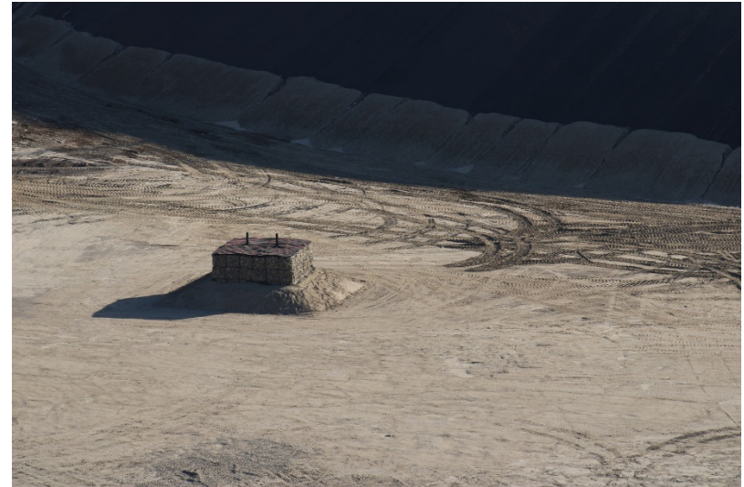
Photo 434: Cell 8 Construction: November 30, 2022
