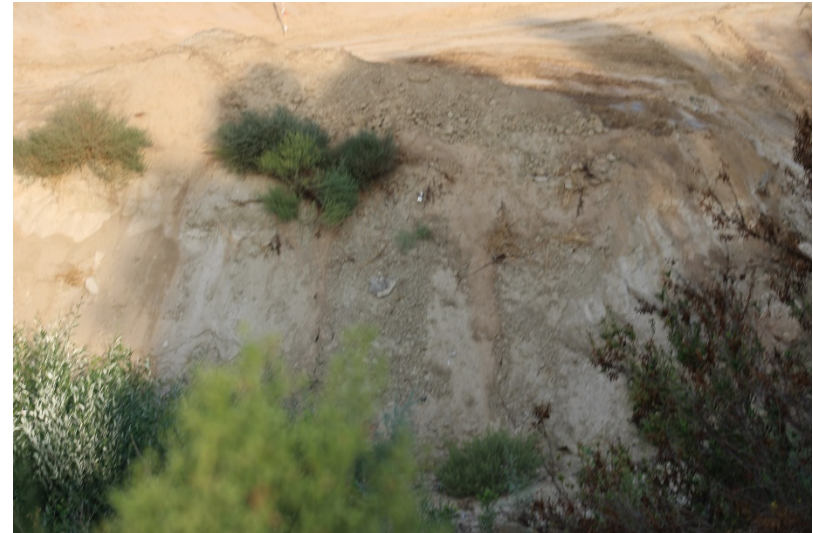
Photo 142: South Terminal and Catch Basins: October 12, 2022
