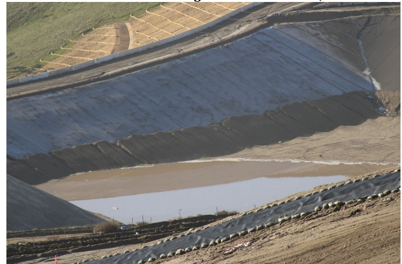
Photo 84: Cell 6 Working Area: December 14, 2022
