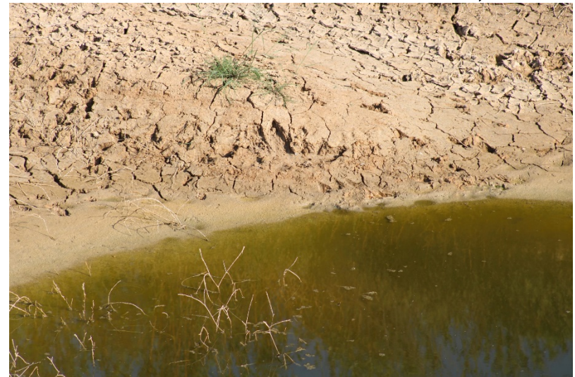
Photo 184: Northeast Sediment Basin: October 12, 2022
