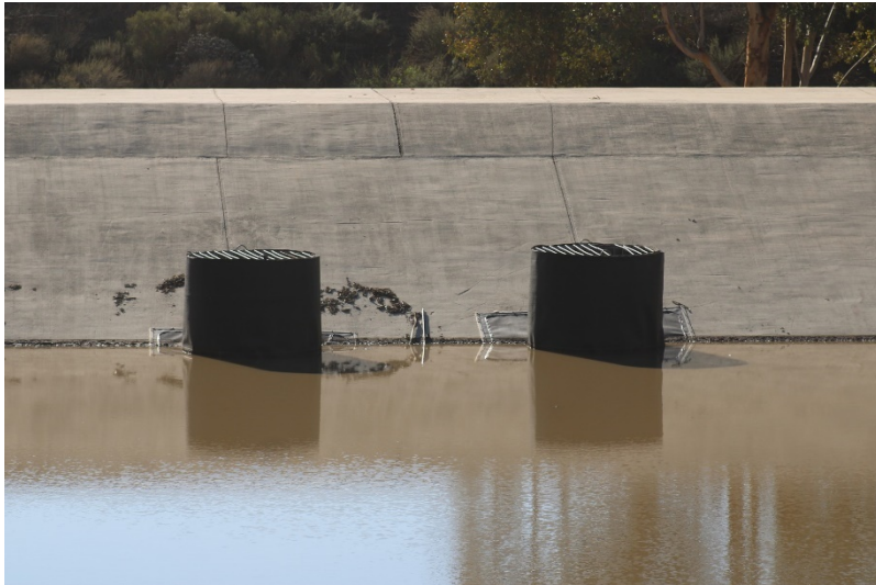
Photo 177: South Terminal and Catch Basins: December 14, 2022
