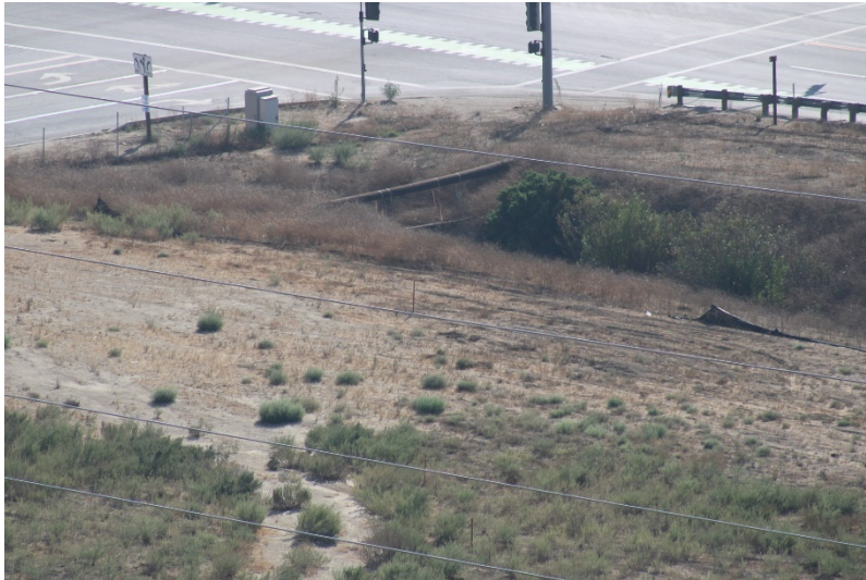
Photo 241: Wolcott Way Entrance Facilities: October 12, 2022
