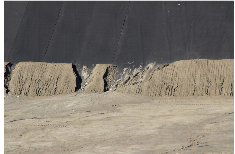
Photo 446: Cell Construction: December 12, 2022
