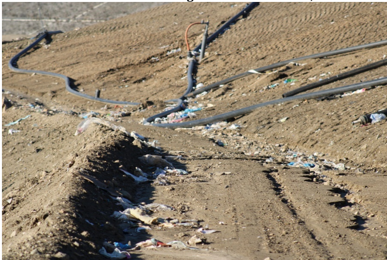
Photo 83: Cell 6 Working Area: December 14, 2022
