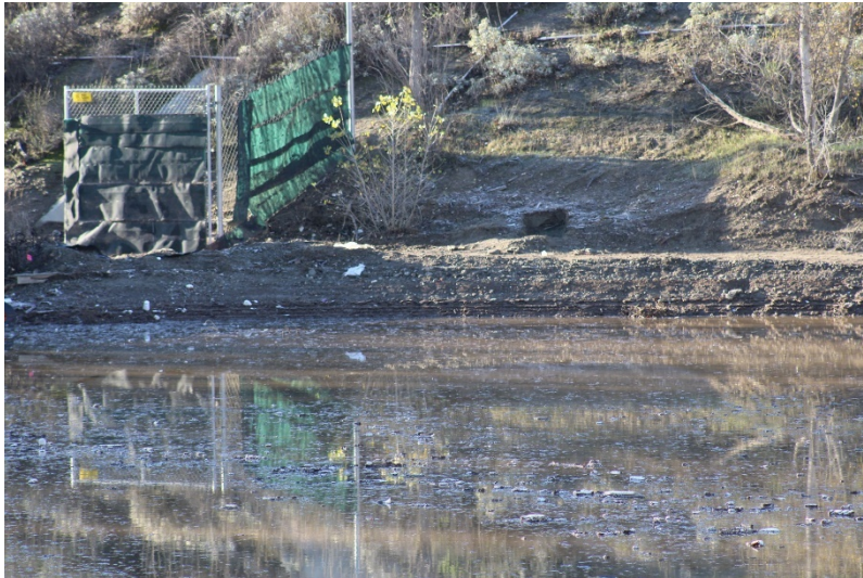
Photo 169: South Terminal and Catch Basins: December 14, 2022
