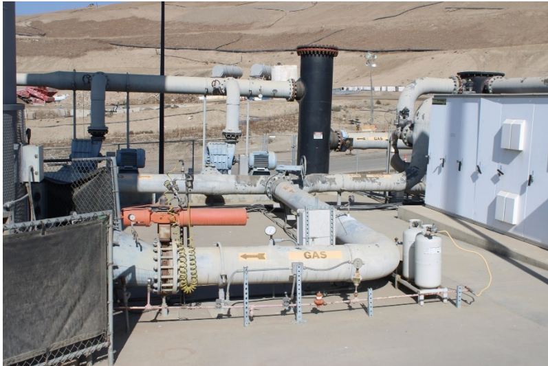
Photo 209: Flare 100 and Flare 150: October 12, 2022
