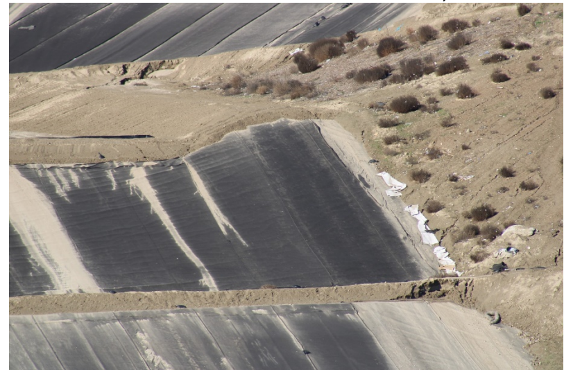
Photo 456: Cell Construction: December 12, 2022
