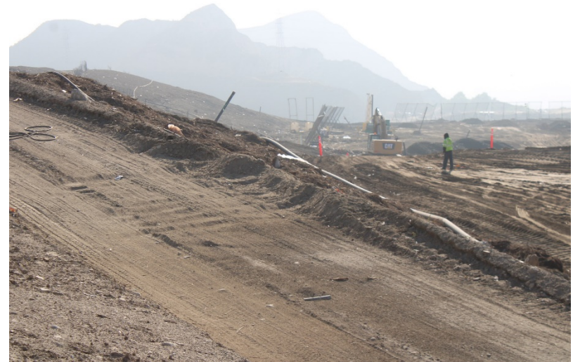
Photo 10: Top Deck Working Area: October 12, 2022
