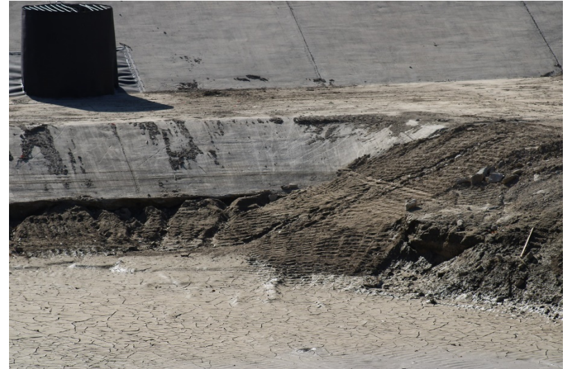
Photo 160: South Terminal and Catch Basins: November 30, 2022
