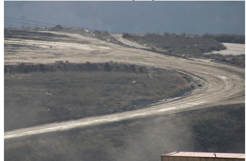
Photo 96: Closed Landfill – Primary Canyon: November 30, 2022
