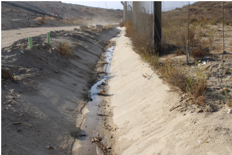
Photo 195: Landfill Perimeter Drainage Channel: October 12, 2022
