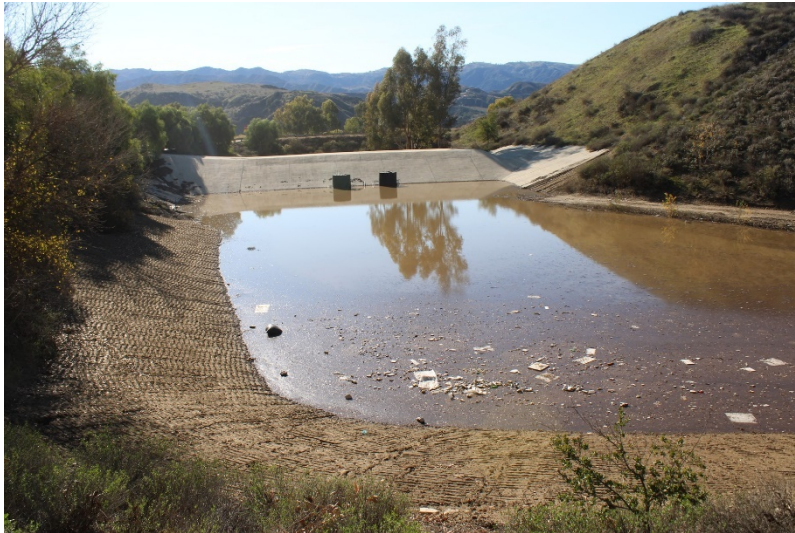
Photo 171: South Terminal and Catch Basins: December 14, 2022
