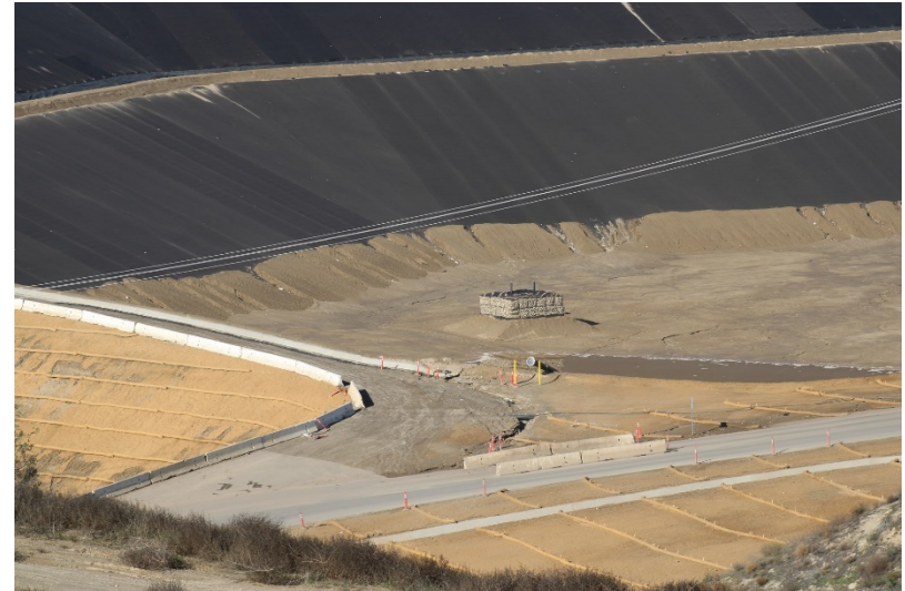
Photo 438: Cell Construction: December 12, 2022
