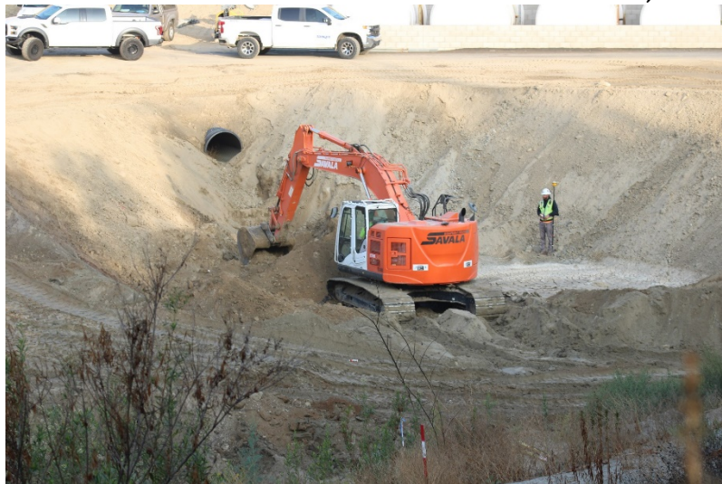
Photo 143: South Terminal and Catch Basins: October 12, 2022
