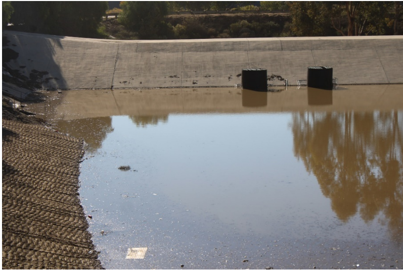
Photo 173: South Terminal and Catch Basins: December 14, 2022
