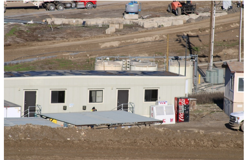
Photo 262: Maintenance and Admin Buildings: December 14, 2022
