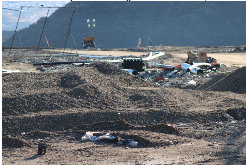
Photo 35: Top Deck Working Area: December 14, 2022
