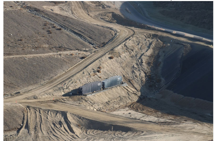
Photo 432: Cell 8 Construction: November 30, 2022
