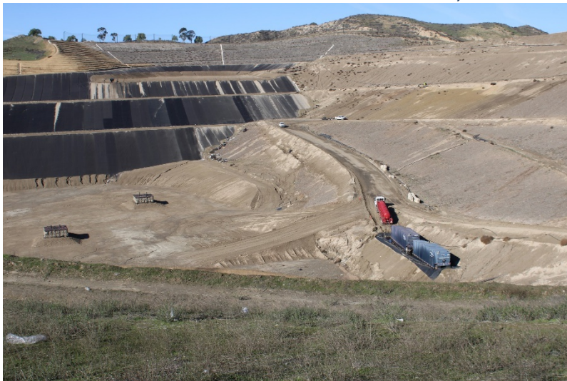
Photo 443: Cell Construction: December 12, 2022
