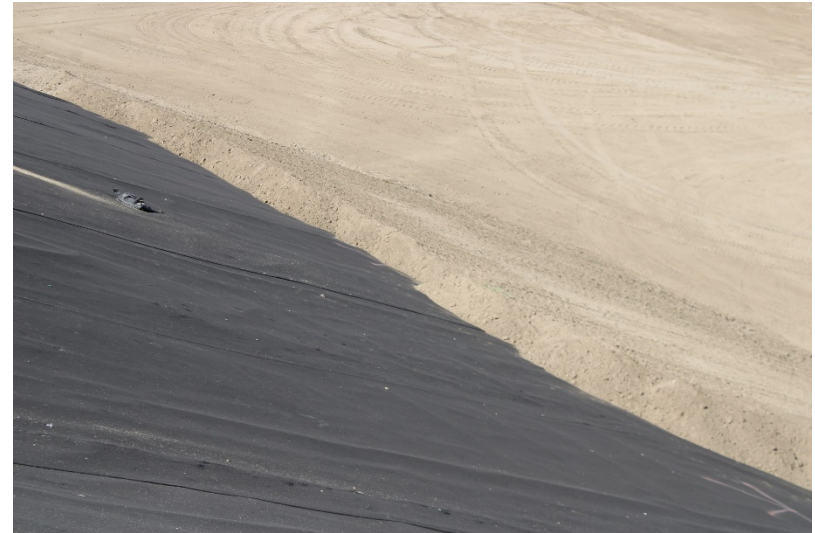
Photo 426: Cell 8 Construction: October 12, 2022
