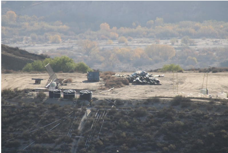
Photo 93: Closed Landfill – Primary Canyon: November 30, 2022
