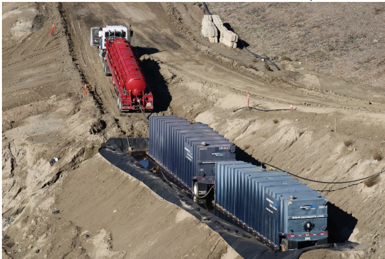
Photo 451: Cell Construction: December 12, 2022
