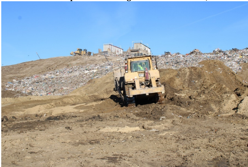
Photo 47: Top Deck Working Area: December 14, 2022
