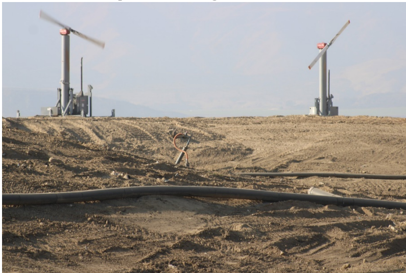
Photo 7: Top Deck Working Area: October 12, 2022
