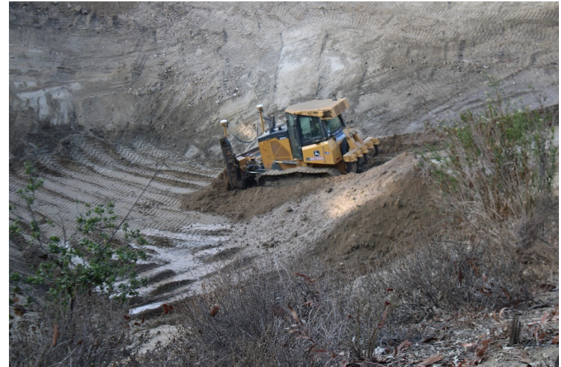
Photo 146: South Terminal and Catch Basins: October 12, 2022
