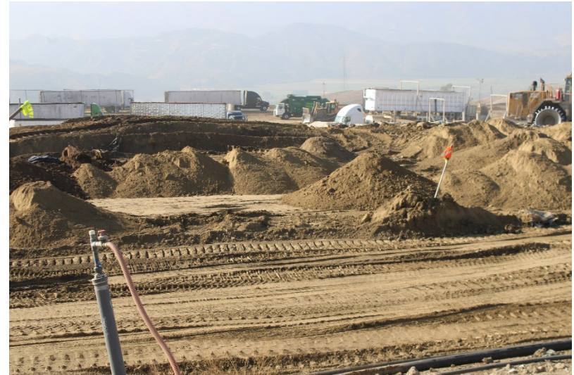
Photo 14: Top Deck Working Area: October 12, 2022
