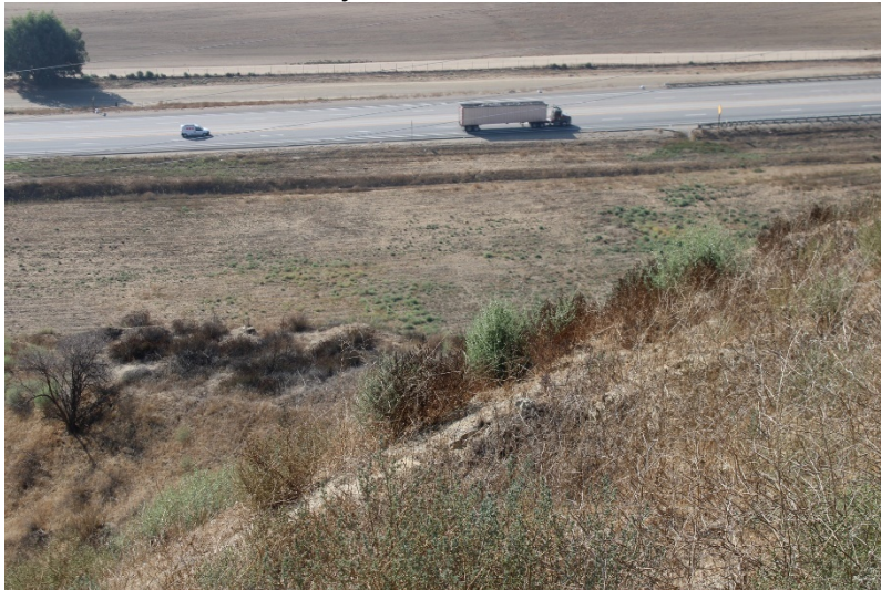
Photo 239: Wolcott Way Entrance Facilities: October 12, 2022
