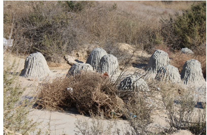
Photo 198: Landfill Perimeter Drainage Channel: November 30, 2022
