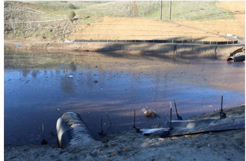
Photo 166: South Terminal and Catch Basins: December 14, 2022
