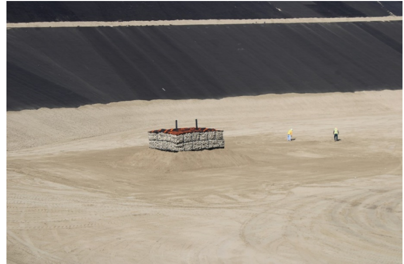
Photo 418: Cell 8 Construction: October 12, 2022
