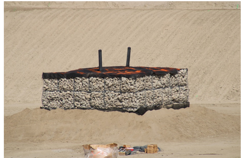
Photo 422: Cell 8 Construction: October 12, 2022
