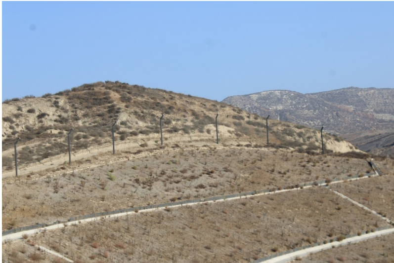
Photo 201: Westside Perimeter Ridge: October 12, 2022
