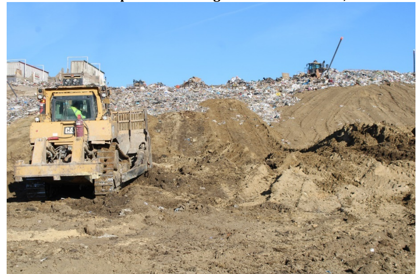
Photo 48: Top Deck Working Area: December 14, 2022
