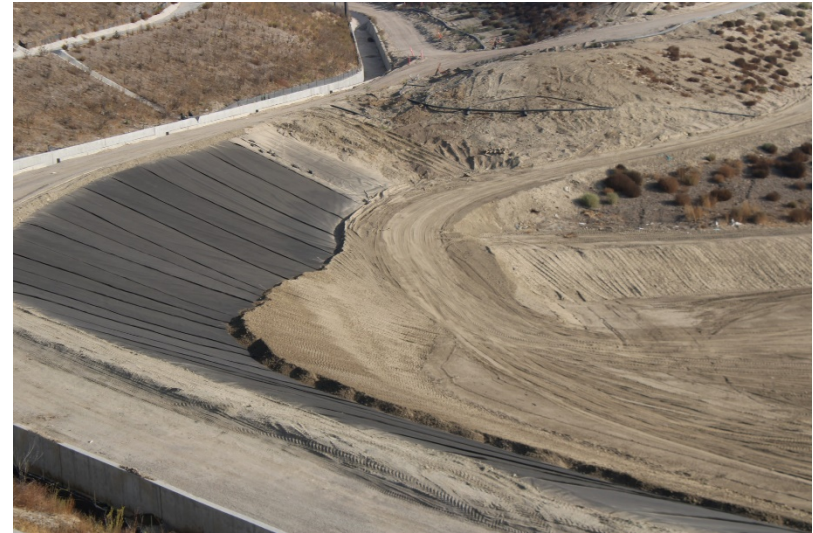
Photo 406: Cell 8 Construction: October 12, 2022
