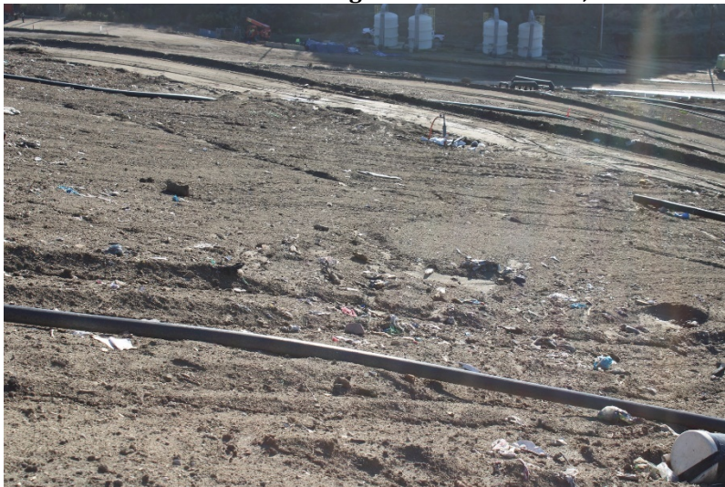
Photo 75: Cell 6 Working Area: December 14, 2022
