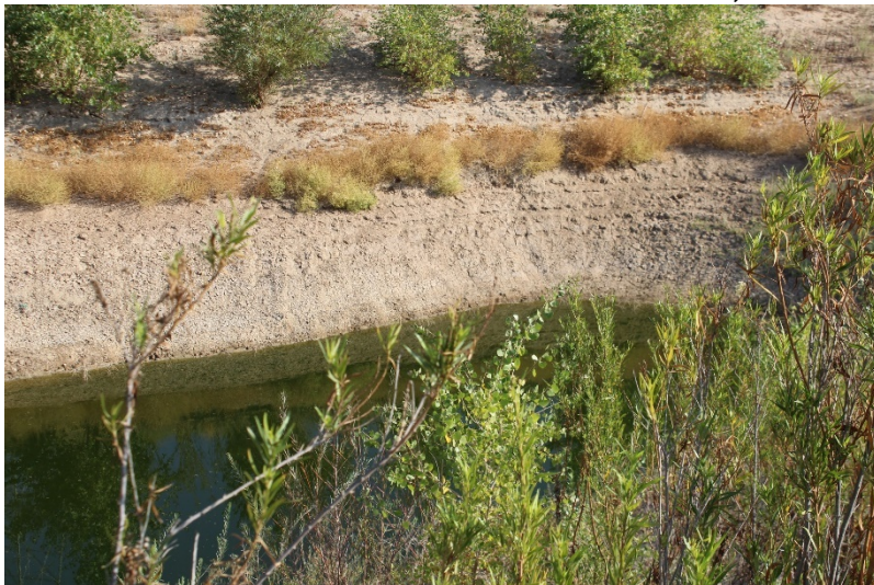
Photo 183: Northeast Sediment Basin: October 12, 2022
