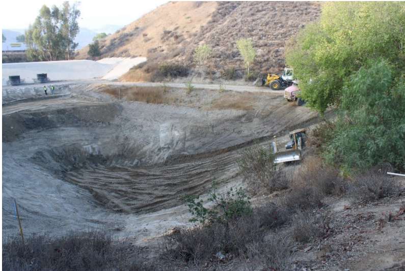
Photo 133: South Terminal and Catch Basins: October 12, 2022
