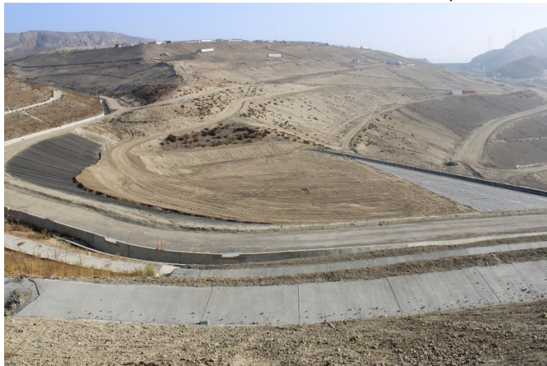
Photo 403: Cell 8 Construction: October 12, 2022
