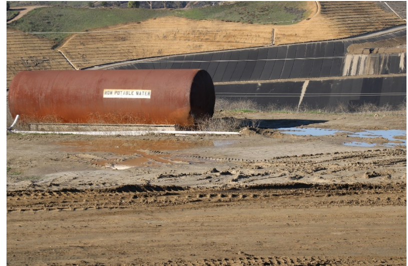
Photo 102: Closed Landfill - Primary Canyon: December 14, 2022
