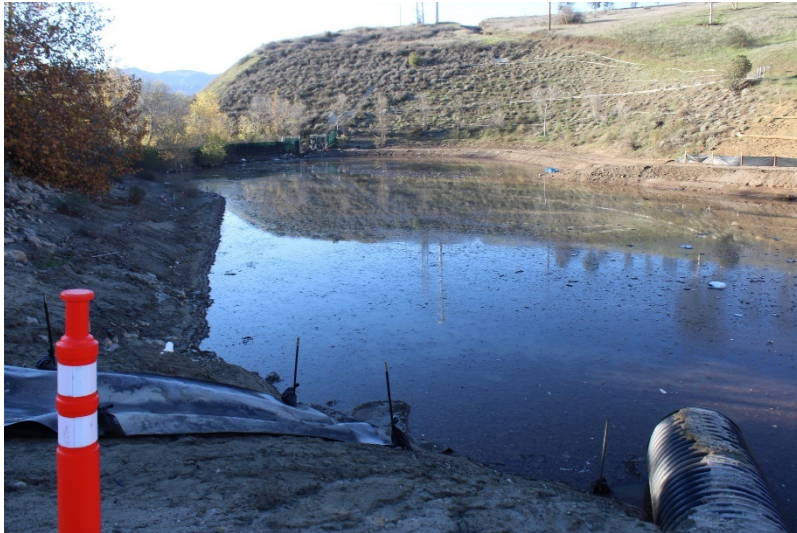
Photo 165: South Terminal and Catch Basins: December 14, 2022
