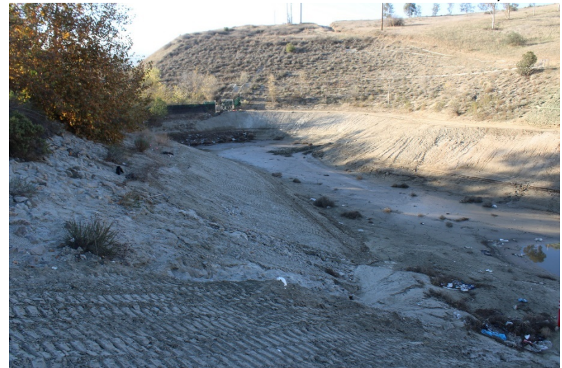
Photo 148: South Terminal and Catch Basins: November 30, 2022
