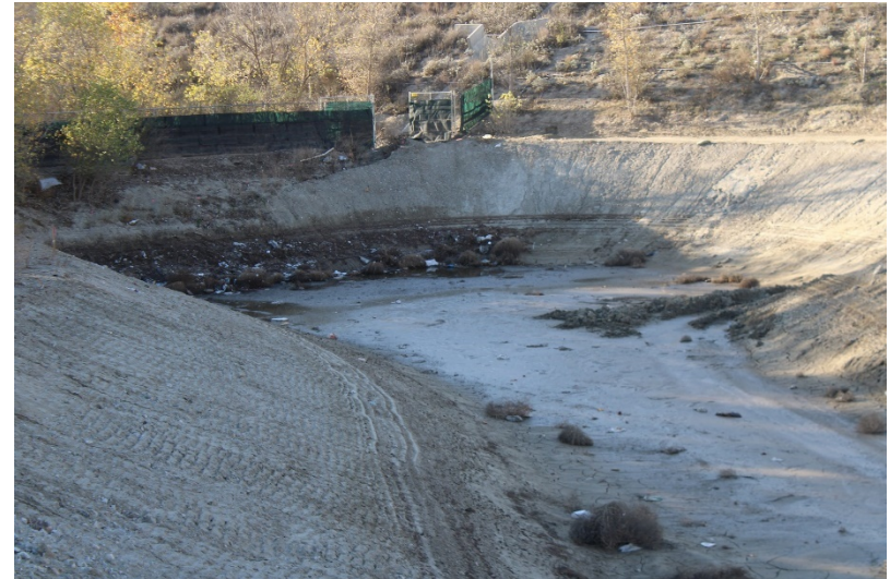
Photo 150: South Terminal and Catch Basins: November 30, 2022
