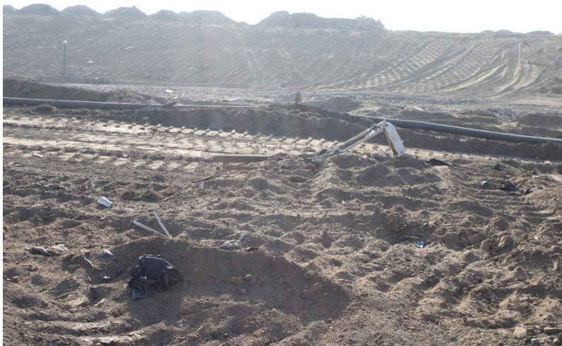
Photo 3: Top Deck Working Area: October 12, 2022
