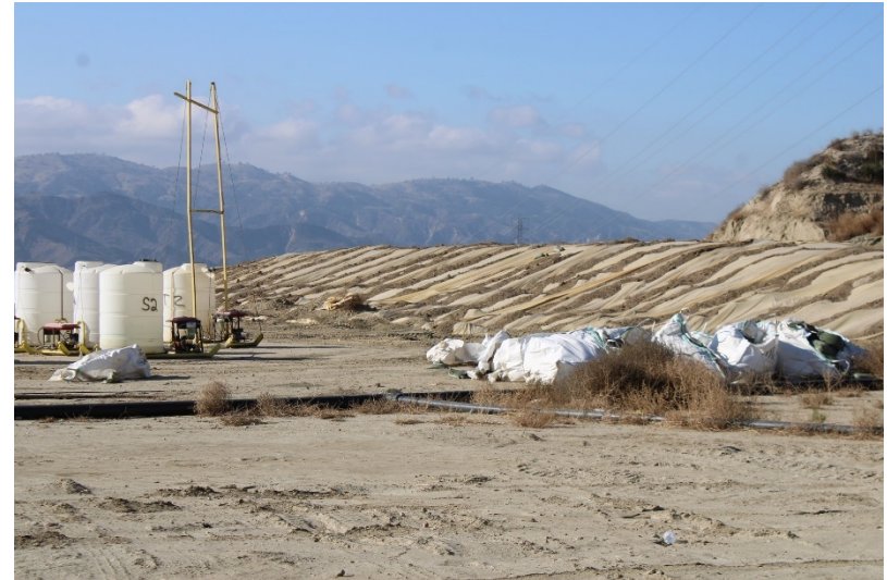
Photo 98: Closed Landfill – Primary Canyon: November 30, 2022
