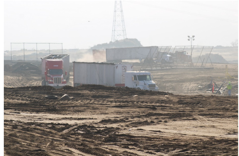
Photo 18: Top Deck Working Area: October 12, 2022
