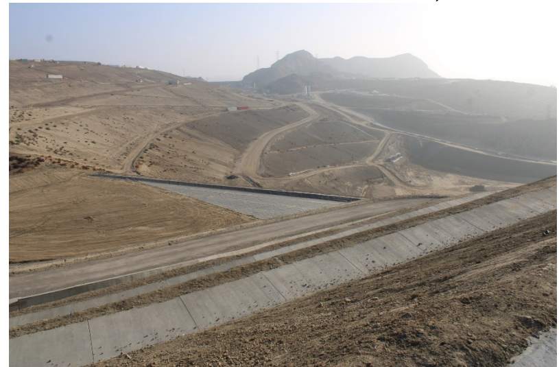
Photo 404: Cell 8 Construction: October 12, 2022
