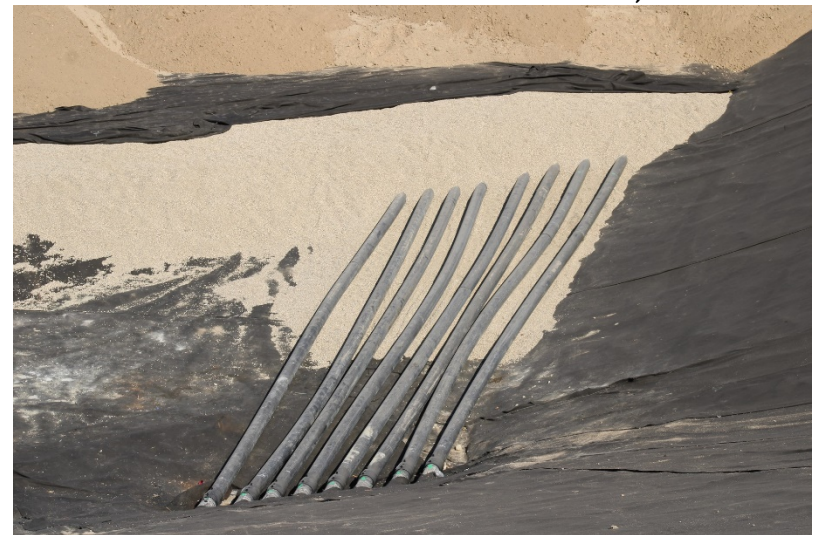
Photo 424: Cell 8 Construction: October 12, 2022
