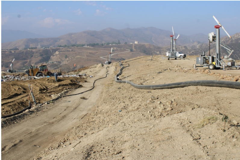
Photo 17: Top Deck Working Area: October 12, 2022
