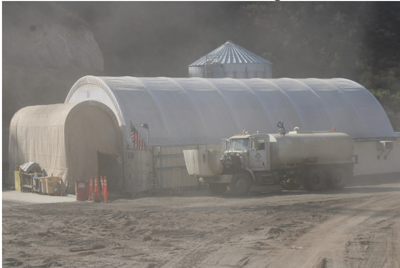
Photo 259: Maintenance and Admin Buildings: October 12, 2022
