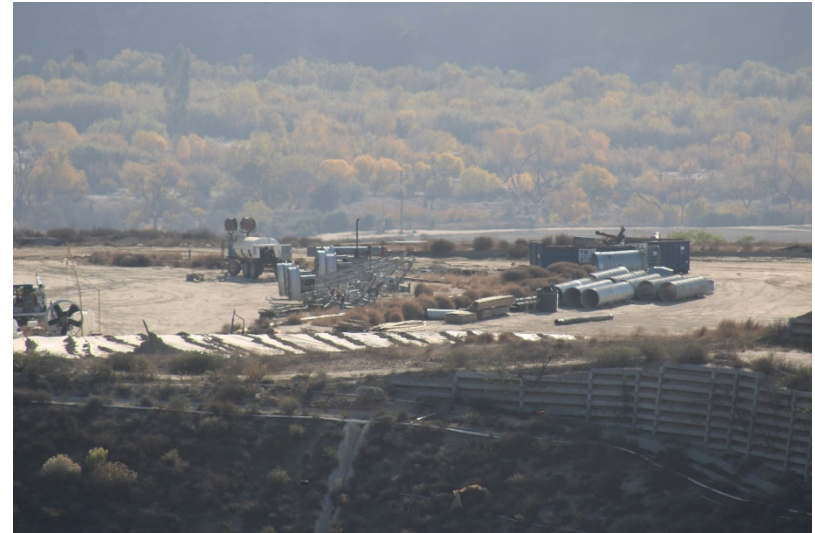
Photo 94: Closed Landfill – Primary Canyon: November 30, 2022
