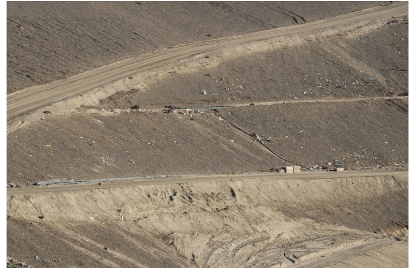
Photo 430: Cell 8 Construction: November 30, 2022
