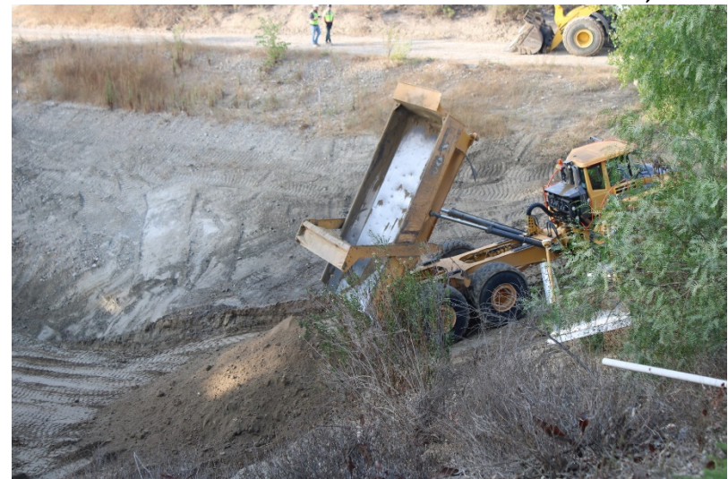
Photo 144: South Terminal and Catch Basins: October 12, 2022
