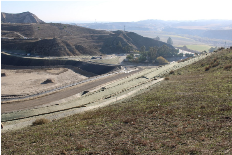
Photo 429: Cell 8 Construction: November 30, 2022
