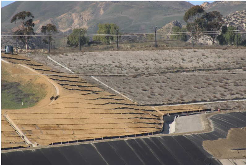
Photo 441: Cell Construction: December 12, 2022
