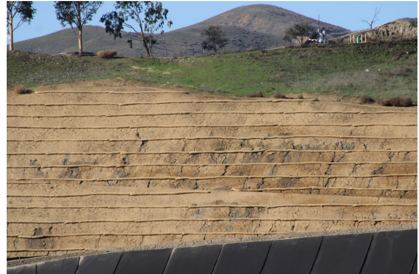
Photo 458: Cell Construction: December 12, 2022
