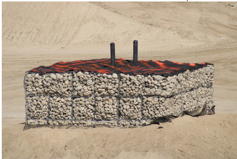
Photo 423: Cell 8 Construction: October 12, 2022
