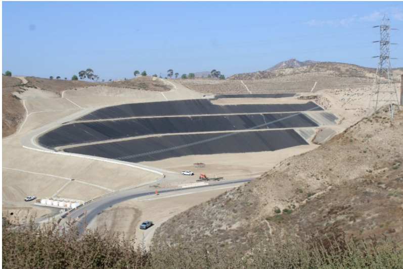
Photo 413: Cell 8 Construction: October 12, 2022
