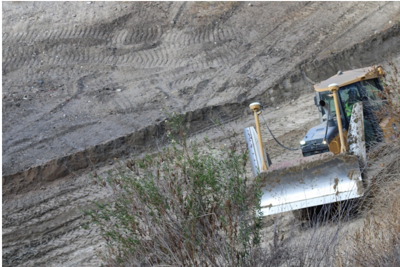
Photo 137: South Terminal and Catch Basins: October 12, 2022
