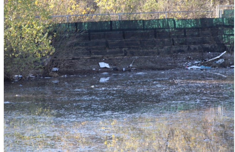
Photo 168: South Terminal and Catch Basins: December 14, 2022
