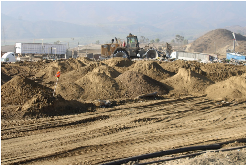
Photo 15: Top Deck Working Area: October 12, 2022
