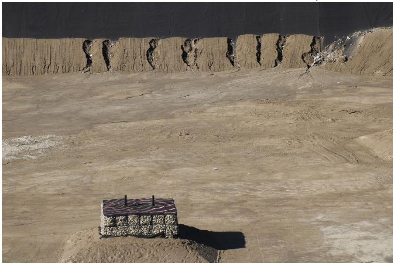
Photo 447: Cell Construction: December 12, 2022
