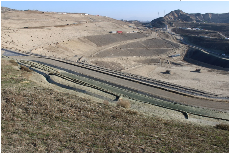
Photo 427: Cell 8 Construction: November 30, 2022
