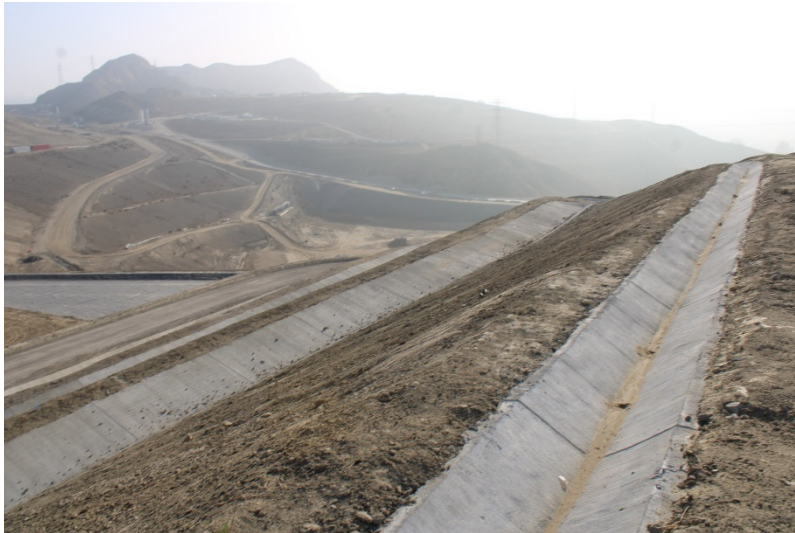
Photo 405: Cell 8 Construction: October 12, 2022
