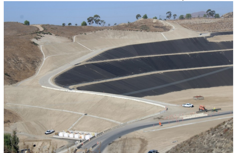
Photo 412: Cell 8 Construction: October 12, 2022
