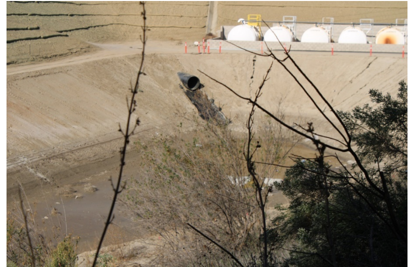
Photo 164: South Terminal and Catch Basins: November 30, 2022
