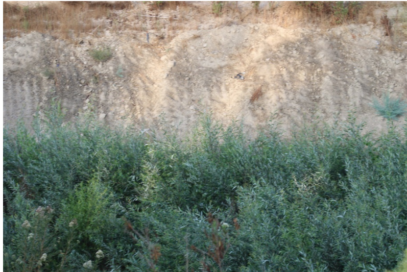
Photo 141: South Terminal and Catch Basins: October 12, 2022
