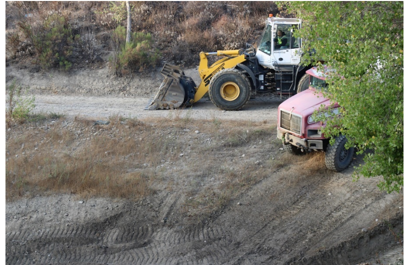
Photo 138: South Terminal and Catch Basins: October 12, 2022
