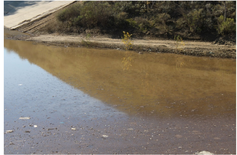
Photo 174: South Terminal and Catch Basins: December 14, 2022
