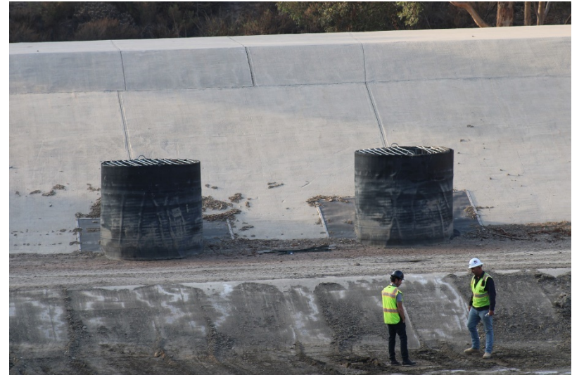
Photo 134: South Terminal and Catch Basins: October 12, 2022
