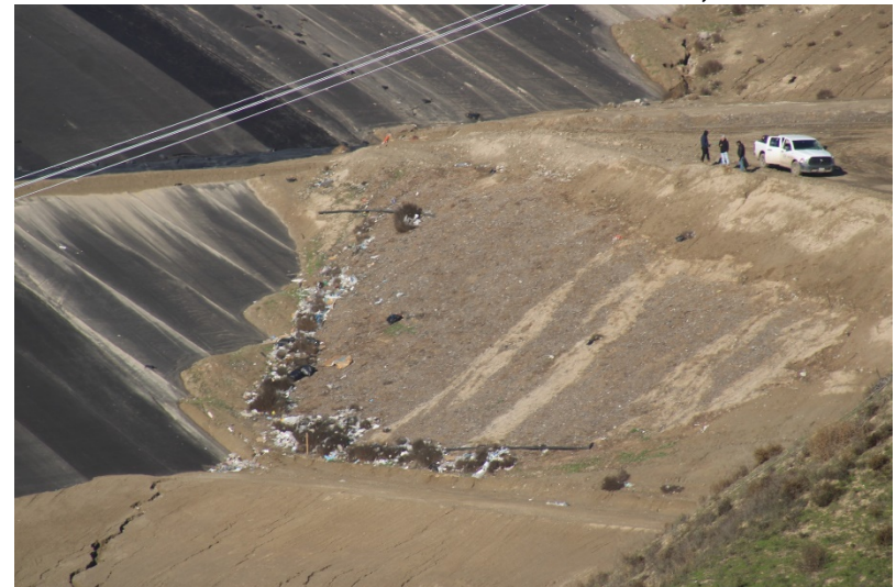
Photo 440: Cell Construction: December 12, 2022
