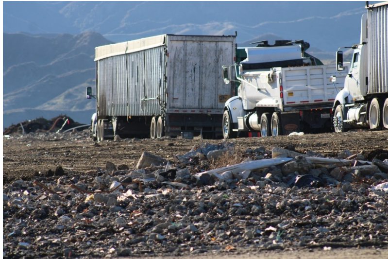
Photo 37: Top Deck Working Area: December 14, 2022
