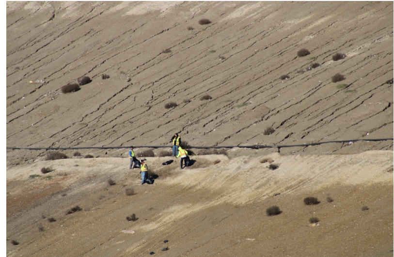
Photo 454: Cell Construction: December 12, 2022
