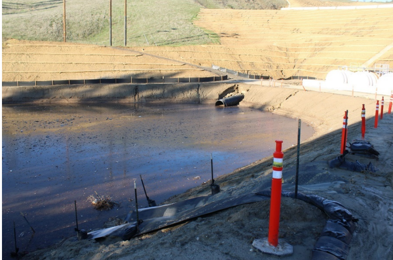
Photo 167: South Terminal and Catch Basins: December 14, 2022
