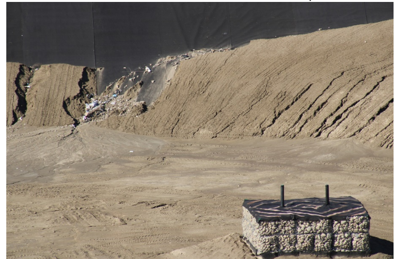
Photo 448: Cell Construction: December 12, 2022
