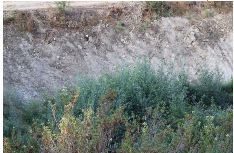
Photo 140: South Terminal and Catch Basins: October 12, 2022
