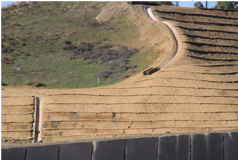
Photo 459: Cell Construction: December 12, 2022
