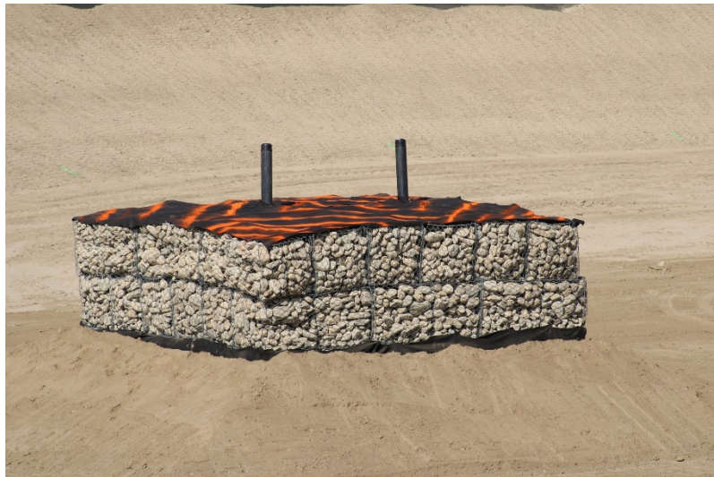
Photo 421: Cell 8 Construction: October 12, 2022
