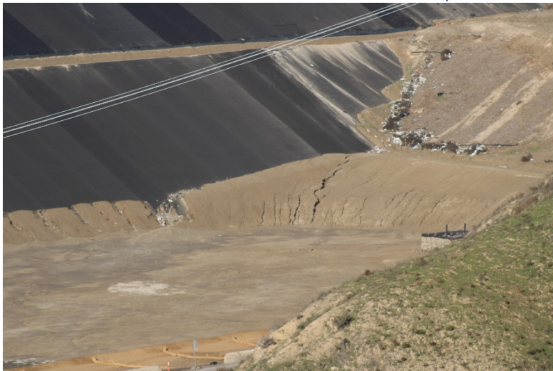
Photo 439: Cell Construction: December 12, 2022
