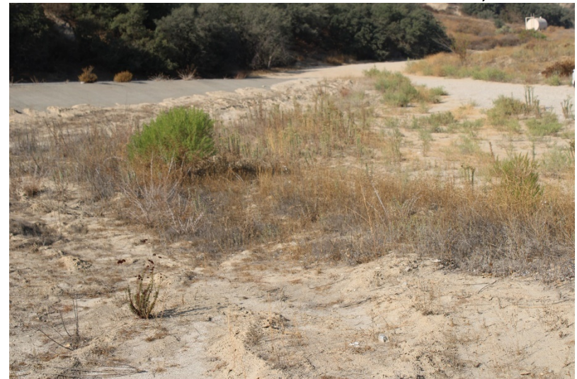
Photo 188: Northeast Sediment Basin: October 12, 2022
