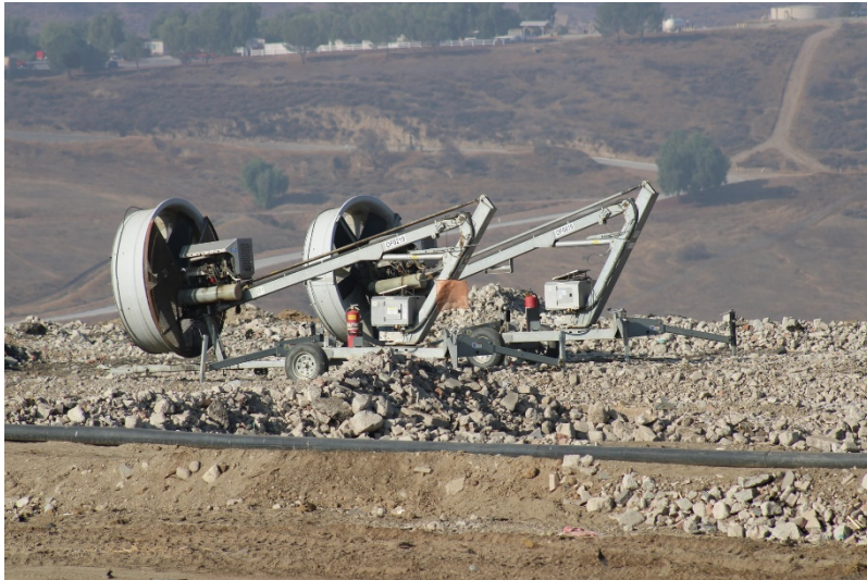
Photo 9: Top Deck Working Area: October 12, 2022
