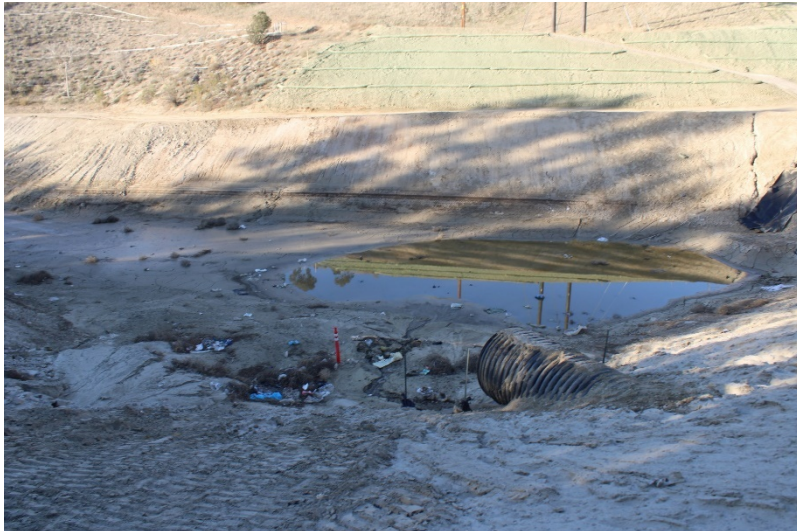
Photo 149: South Terminal and Catch Basins: November 30, 2022
