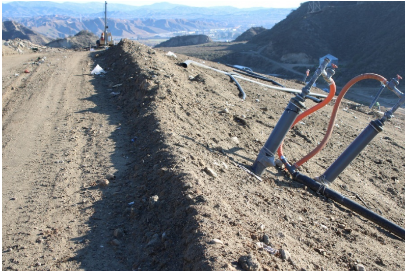
Photo 57: Top Deck Working Area: December 14, 2022
