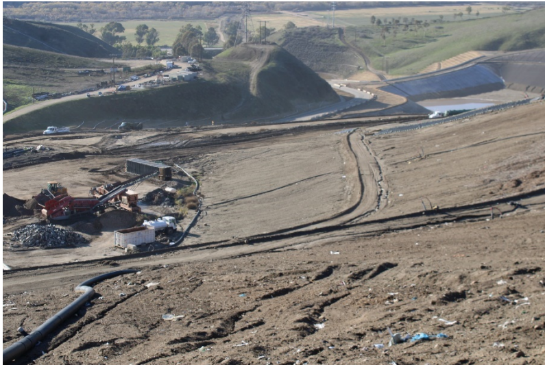
Photo 77: Cell 6 Working Area: December 14, 2022
