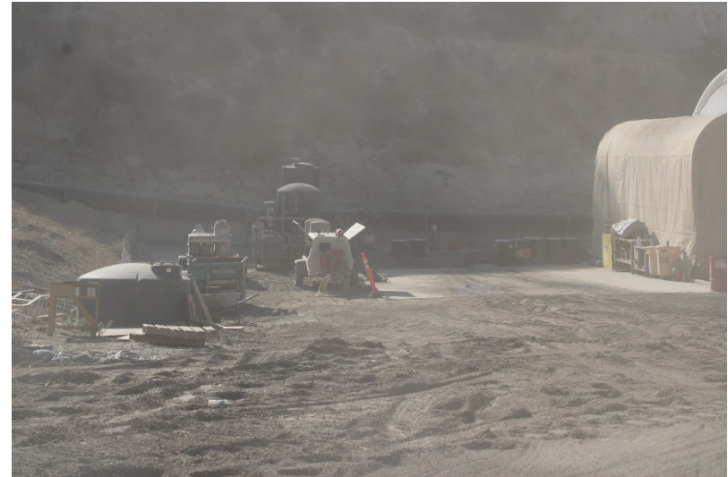
Photo 258: Maintenance and Admin Buildings: October 12, 2022
