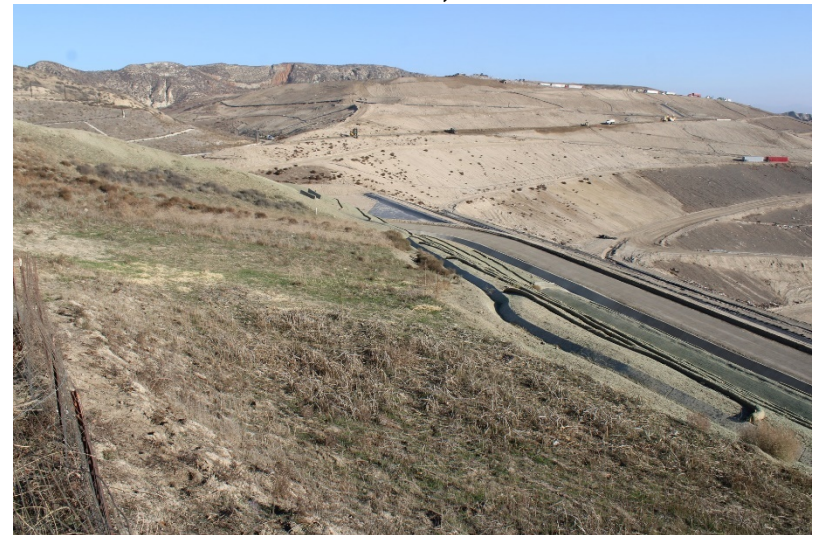
Photo 196: Landfill Perimeter Drainage Channel: November 30, 2022
