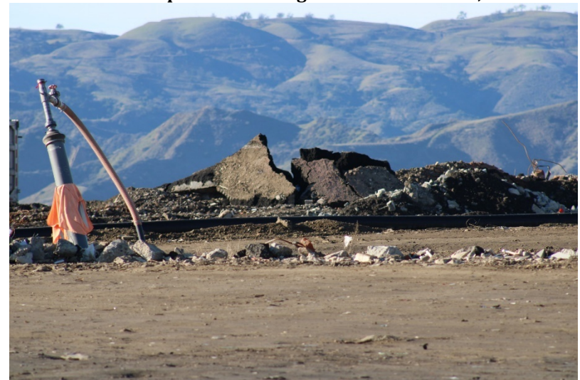
Photo 40: Top Deck Working Area: December 14, 2022
