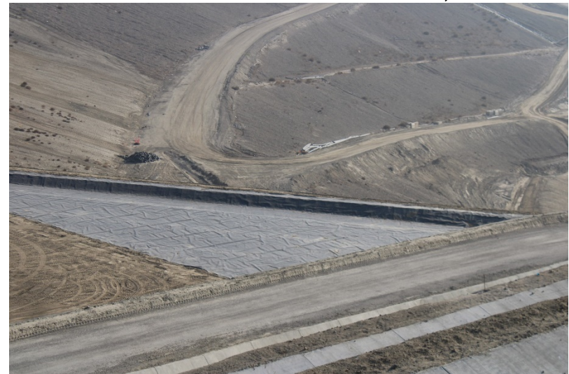
Photo 408: Cell 8 Construction: October 12, 2022
