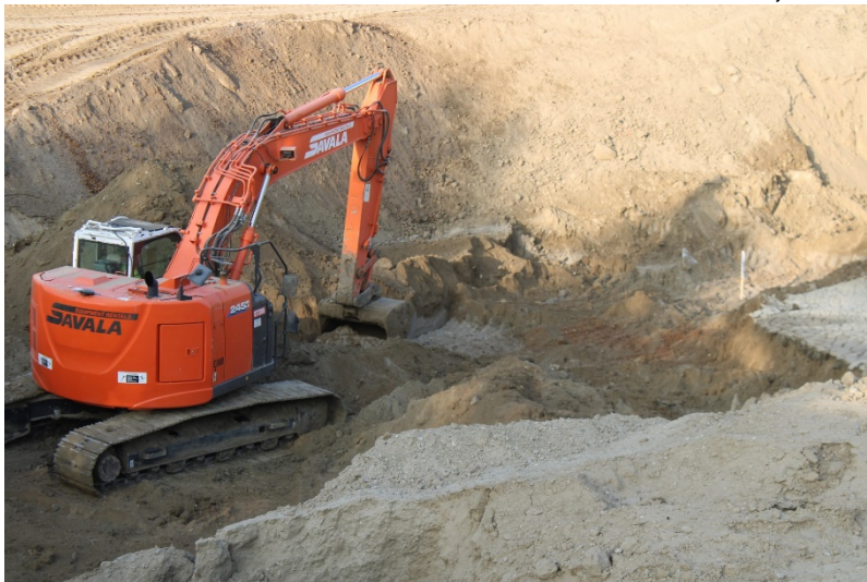
Photo 147: South Terminal and Catch Basins: October 12, 2022
