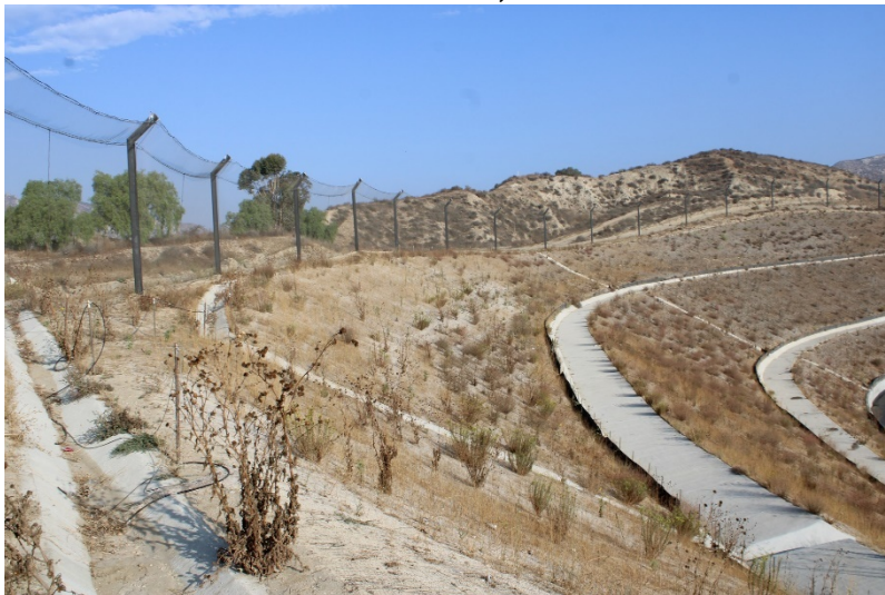
Photo 199: Westside Perimeter Ridge: October 12, 2022
