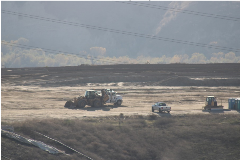
Photo 95: Closed Landfill – Primary Canyon: November 30, 2022
