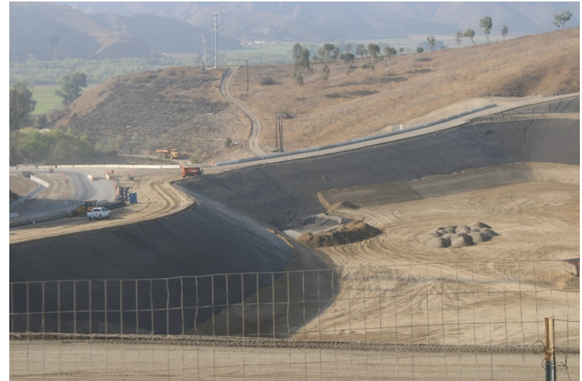
Photo 410: Cell 8 Construction: October 12, 2022
