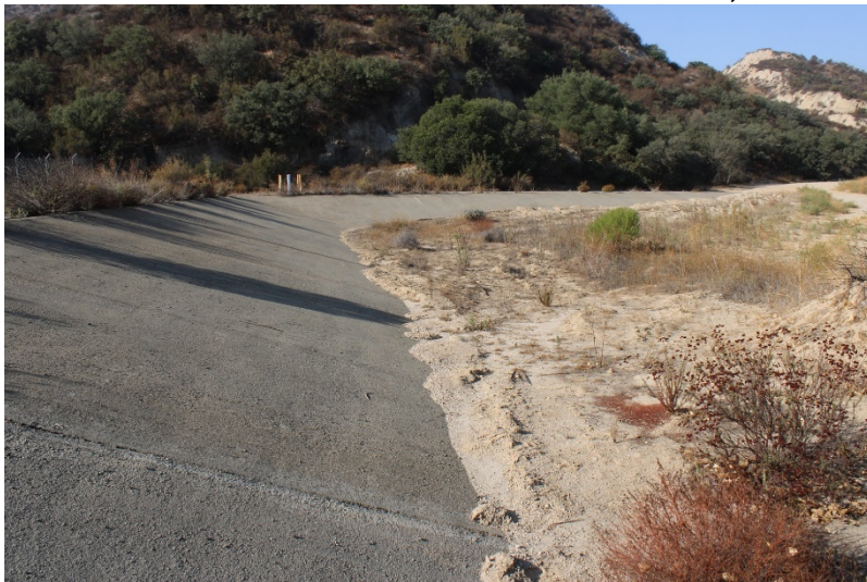
Photo 187: Northeast Sediment Basin: October 12, 2022
