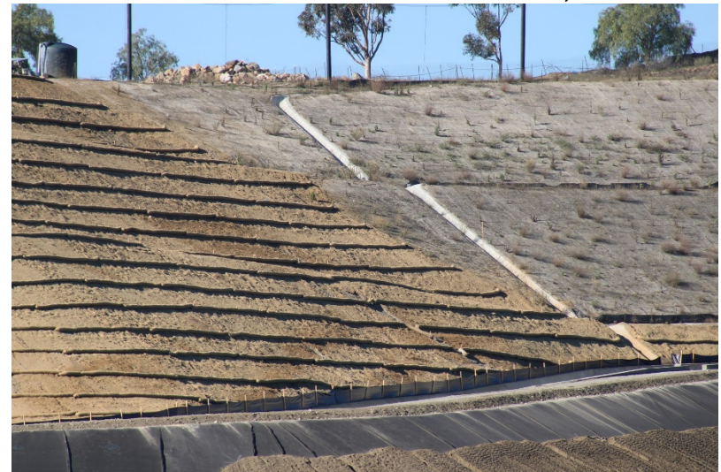
Photo 460: Cell Construction: December 12, 2022
