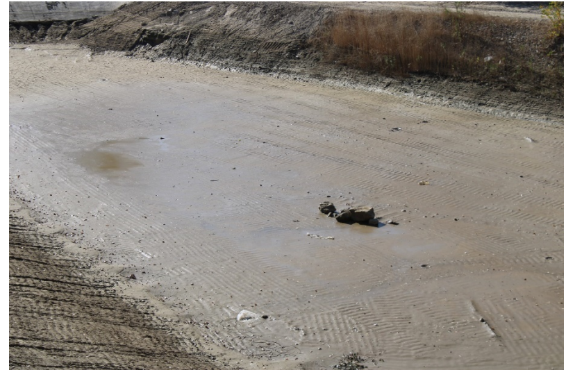
Photo 156: South Terminal and Catch Basins: November 30, 2022
