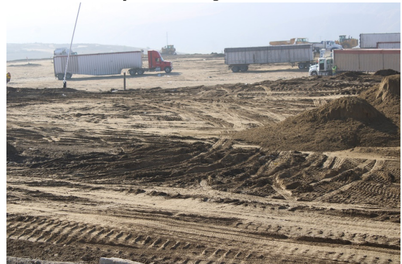
Photo 12: Top Deck Working Area: October 12, 2022
