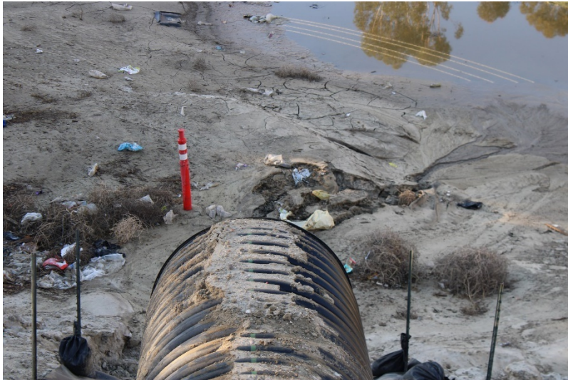
Photo 151: South Terminal and Catch Basins: November 30, 2022
