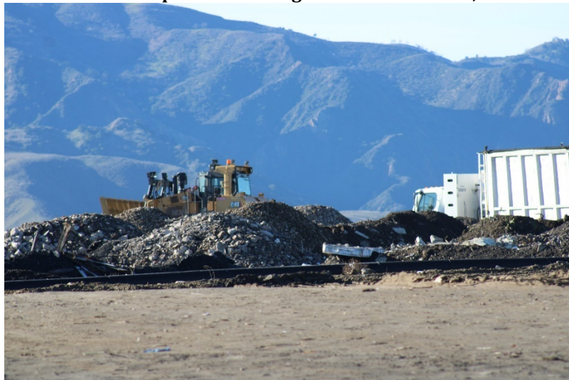
Photo 39: Top Deck Working Area: December 14, 2022
