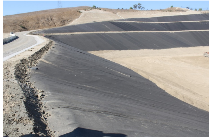
Photo 414: Cell 8 Construction: October 12, 2022
