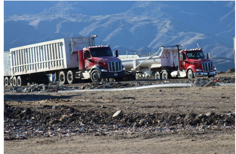
Photo 38: Top Deck Working Area: December 14, 2022
