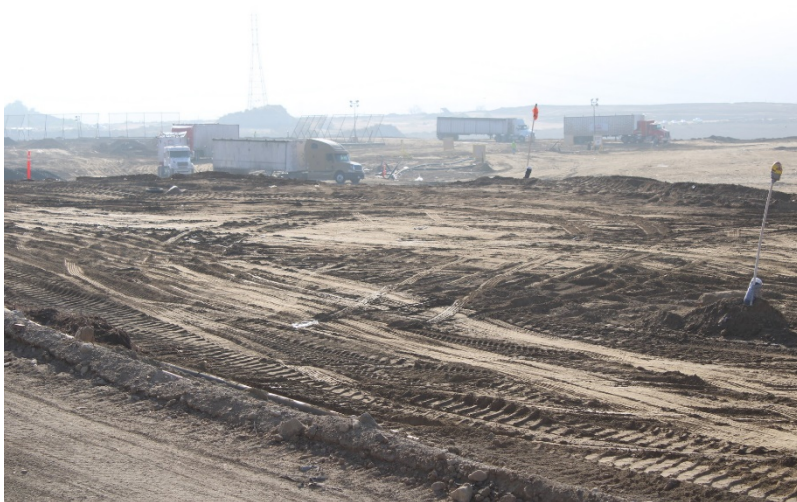
Photo 11: Top Deck Working Area: October 12, 2022
