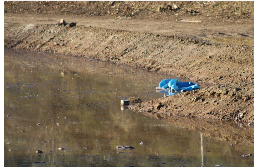
Photo 170: South Terminal and Catch Basins: December 14, 2022
