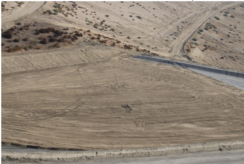
Photo 407: Cell 8 Construction: October 12, 2022
