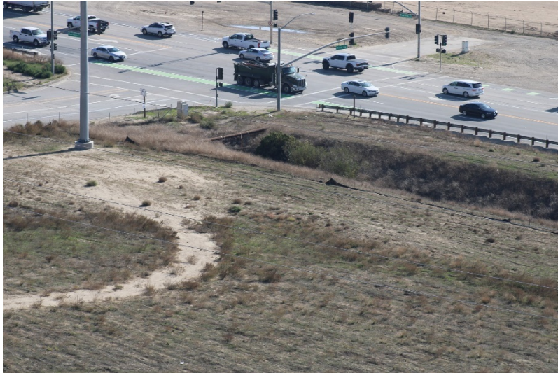
Photo 245: Wolcott Way Entrance Facilities: November 30, 2022
