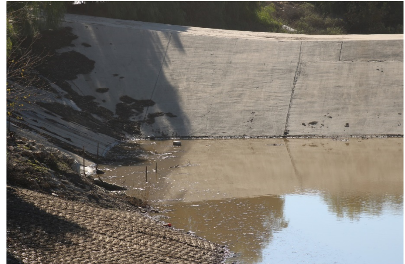
Photo 176: South Terminal and Catch Basins: December 14, 2022
