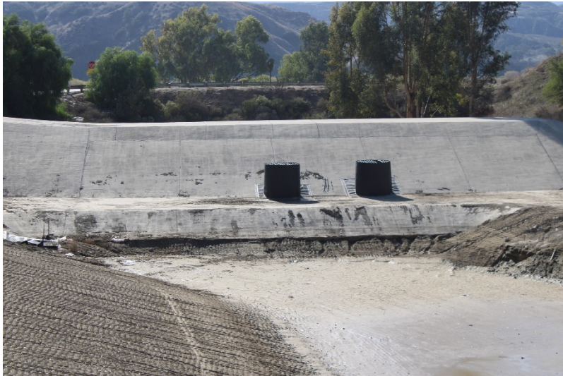
Photo 155: South Terminal and Catch Basins: November 30, 2022
