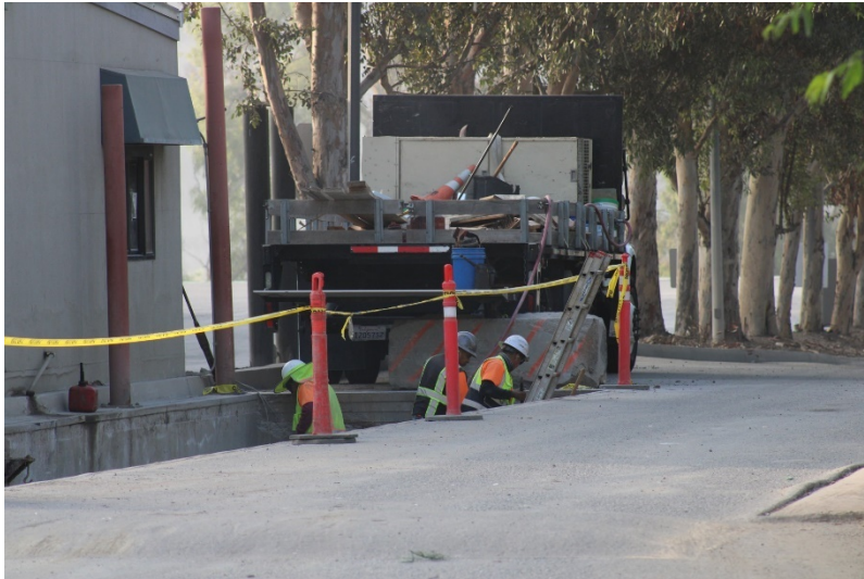
Photo 257: Maintenance and Admin Buildings: October 12, 2022
