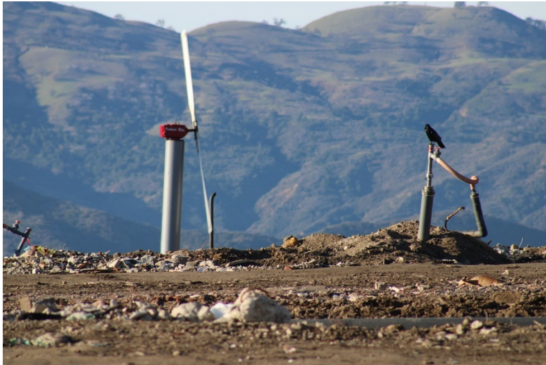
Photo 41: Top Deck Working Area: December 14, 2022
