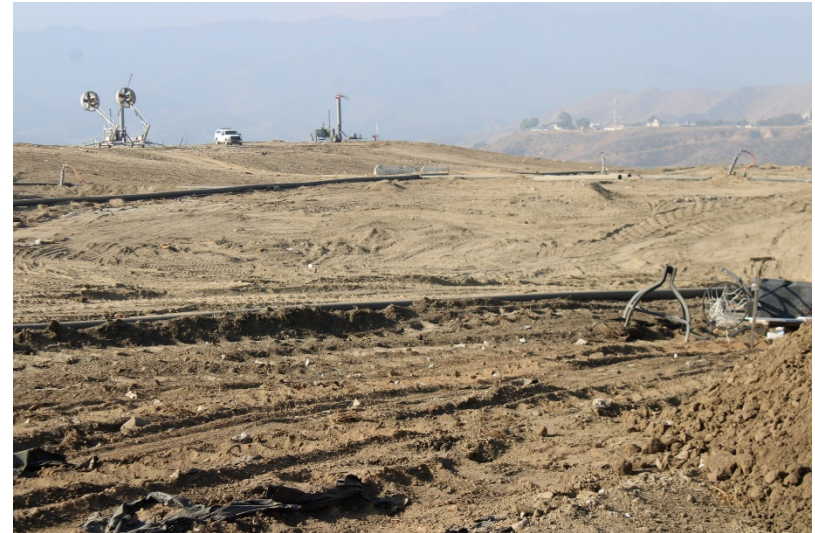
Photo 6: Top Deck Working Area: October 12, 2022
