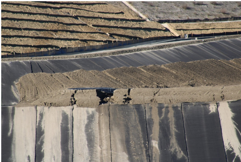
Photo 455: Cell Construction: December 12, 2022
