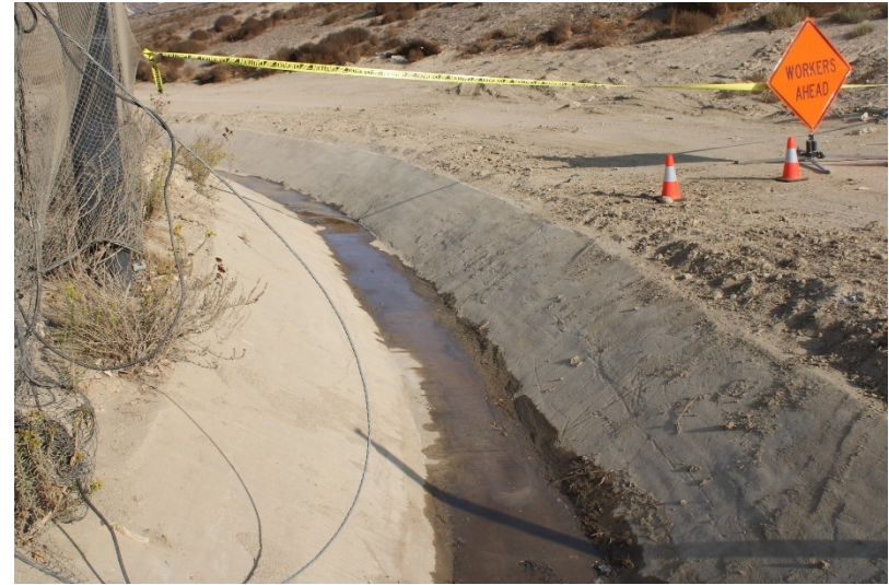
Photo 194: Landfill Perimeter Drainage Channel: October 12, 2022
