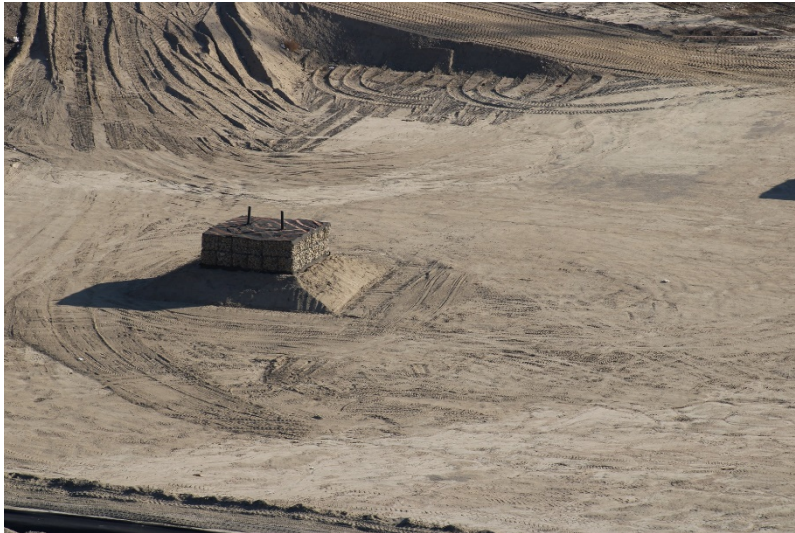
Photo 433: Cell 8 Construction: November 30, 2022
