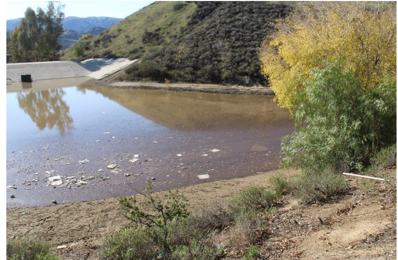
Photo 172: South Terminal and Catch Basins: December 14, 2022
