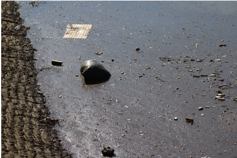
Photo 179: South Terminal and Catch Basins: December 14, 2022
