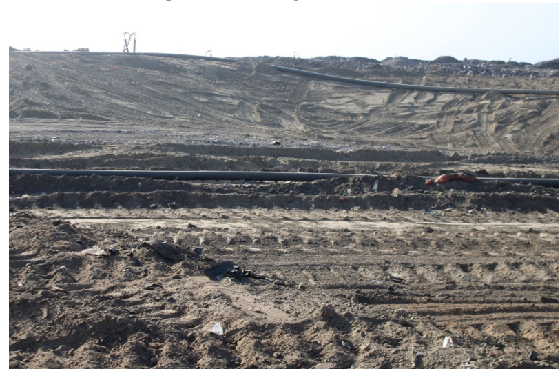
Photo 4: Top Deck Working Area: October 12, 2022
