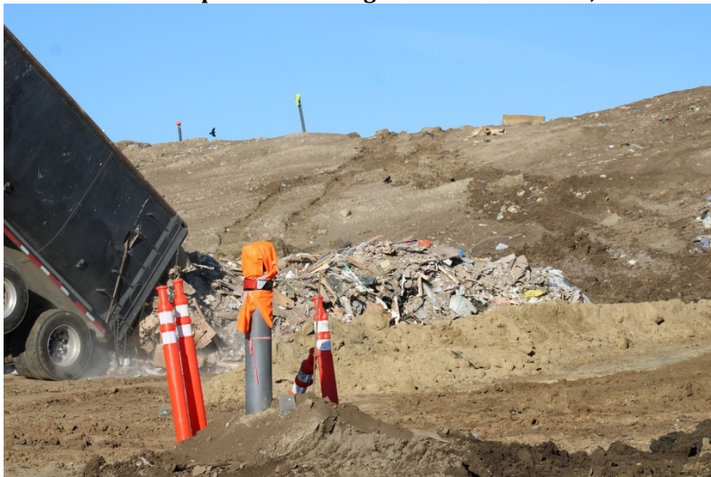
Photo 51: Top Deck Working Area: December 14, 2022
