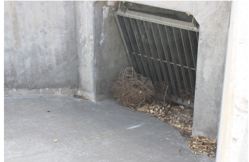
Photo 186: Northeast Sediment Basin: October 12, 2022
