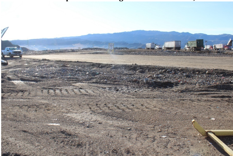
Photo 31: Top Deck Working Area: December 14, 2022
