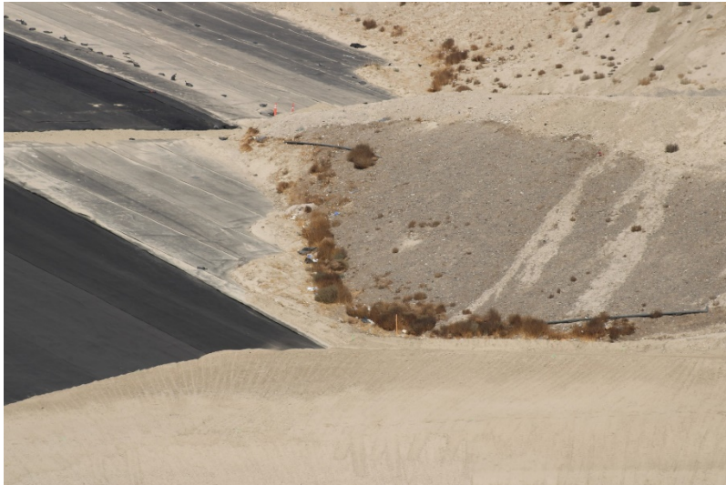
Photo 425: Cell 8 Construction: October 12, 2022
