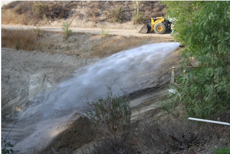
Photo 145: South Terminal and Catch Basins: October 12, 2022
