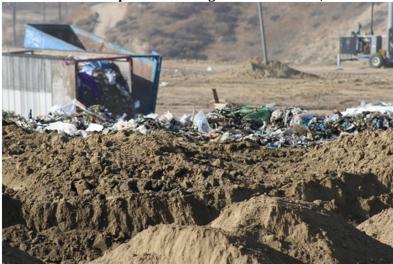
Photo 23: Top Deck Working Area: October 12, 2022
