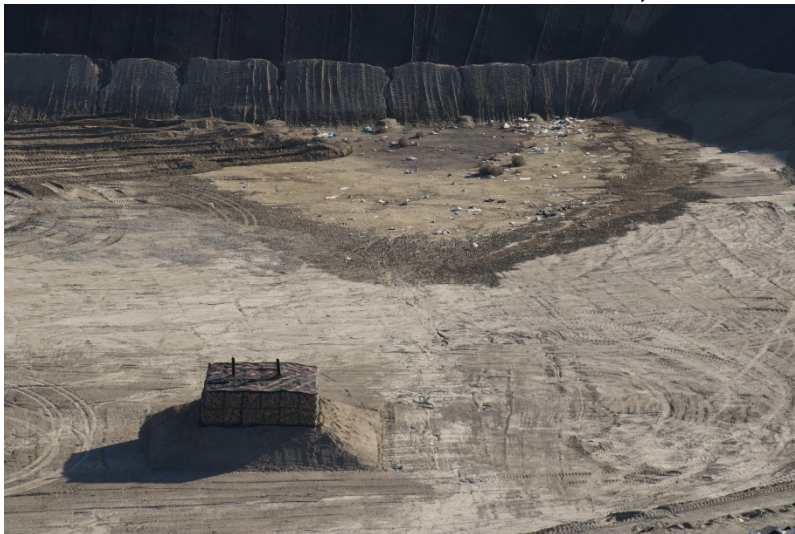
Photo 435: Cell 8 Construction: November 30, 2022
