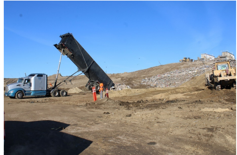
Photo 46: Top Deck Working Area: December 14, 2022
