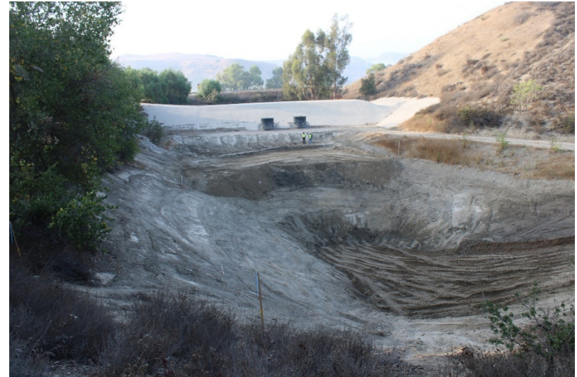
Photo 132: South Terminal and Catch Basins: October 12, 2022
