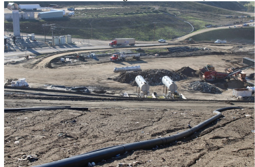
Photo 76: Cell 6 Working Area: December 14, 2022
