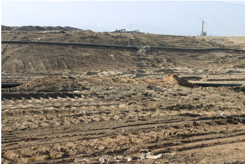
Photo 5: Top Deck Working Area: October 12, 2022
