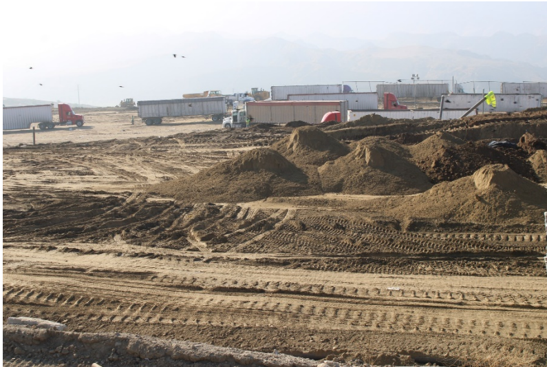
Photo 13: Top Deck Working Area: October 12, 2022
