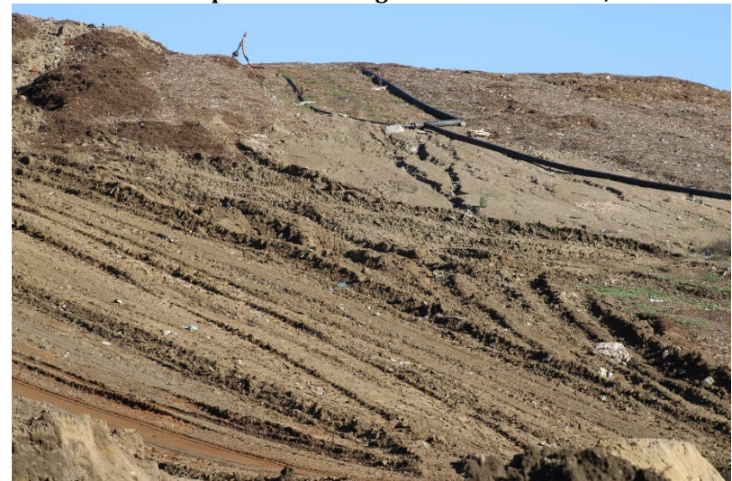
Photo 56: Top Deck Working Area: December 14, 2022
