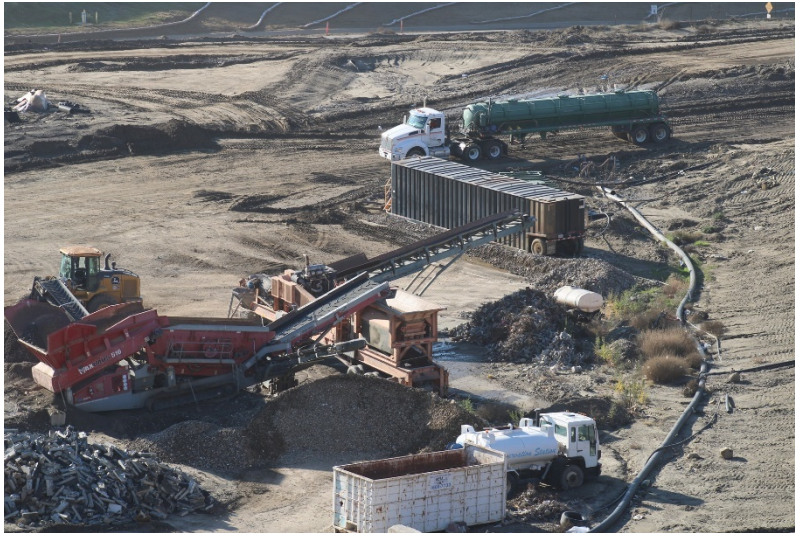
Photo 81: Cell 6 Working Area: December 14, 2022
