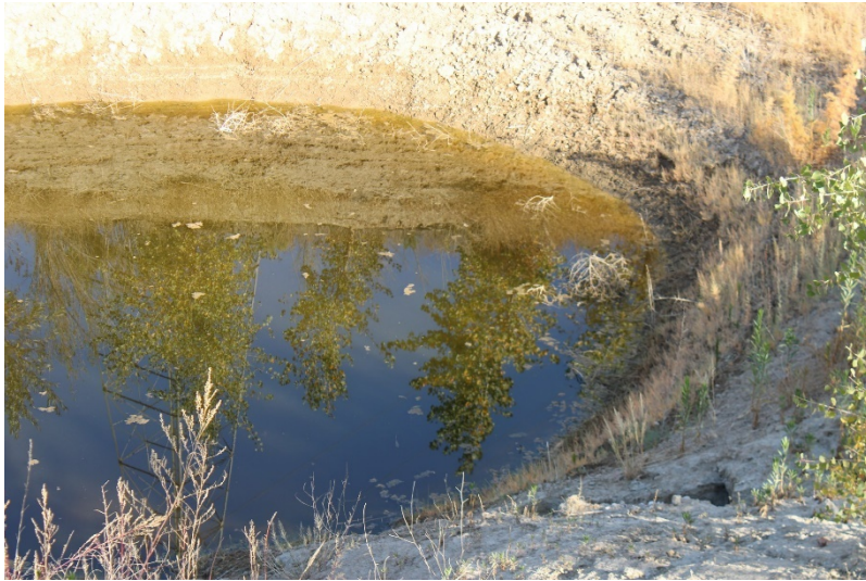
Photo 193: Northeast Sediment Basin: November 30, 2022
