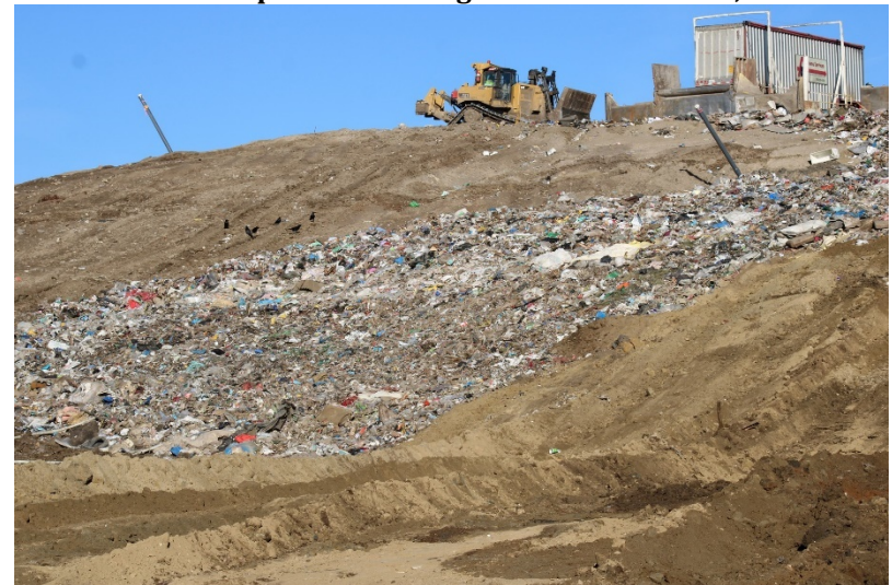
Photo 52: Top Deck Working Area: December 14, 2022
