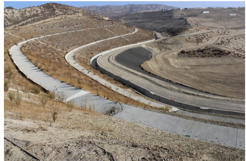
Photo 402: Cell 8 Construction: October 12, 2022
