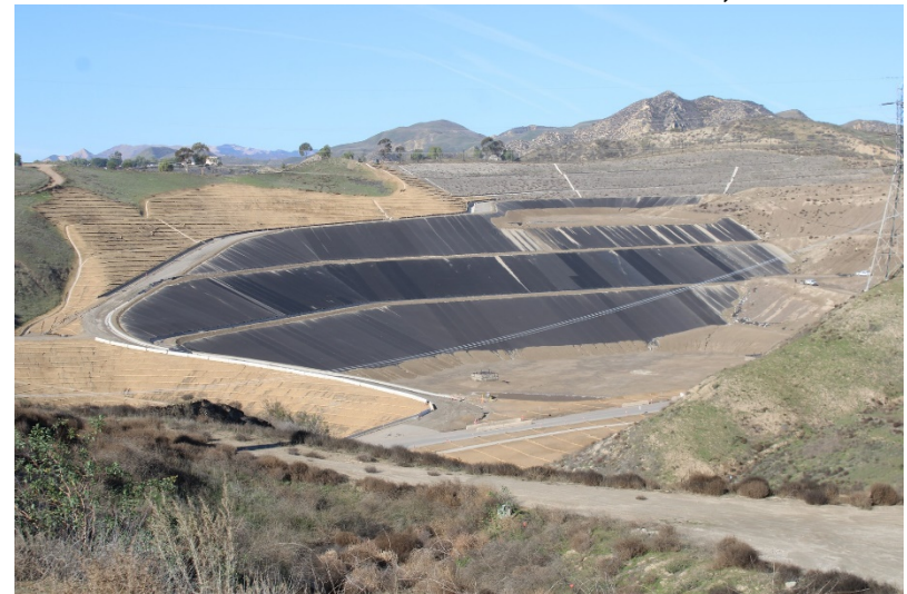
Photo 436: Cell 8 Construction: December 12, 2022
