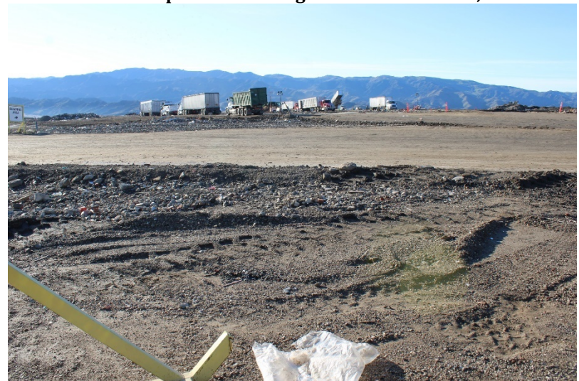
Photo 32: Top Deck Working Area: December 14, 2022
