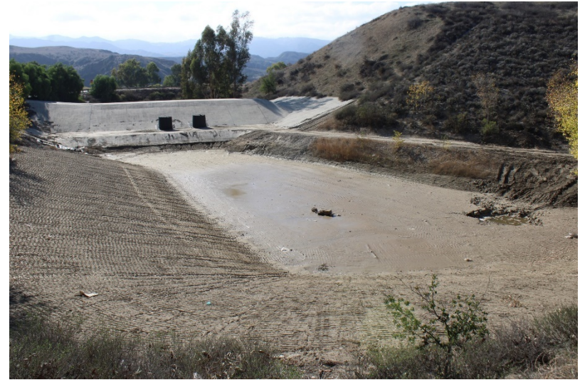
Photo 154: South Terminal and Catch Basins: November 30, 2022
