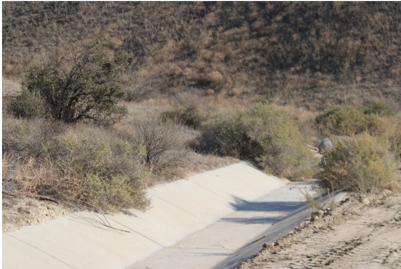
Photo 197: Landfill Perimeter Drainage Channel: November 30, 2022
