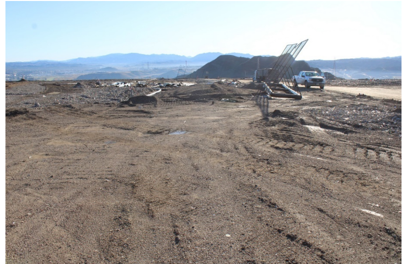
Photo 30: Top Deck Working Area: December 14, 2022
