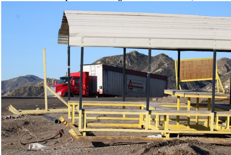
Photo 43: Top Deck Working Area: December 14, 2022
