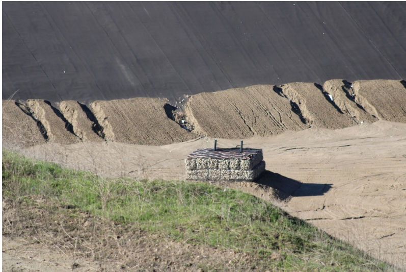
Photo 445: Cell Construction: December 12, 2022
