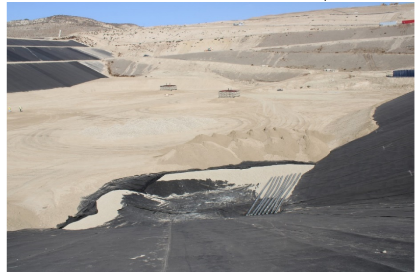
Photo 416: Cell 8 Construction: October 12, 2022
