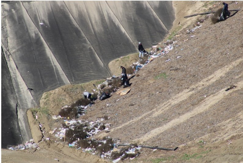
Photo 449: Cell Construction: December 12, 2022
