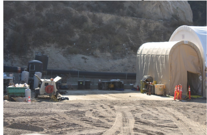
Photo 260: Maintenance and Admin Buildings: November 30, 2022
