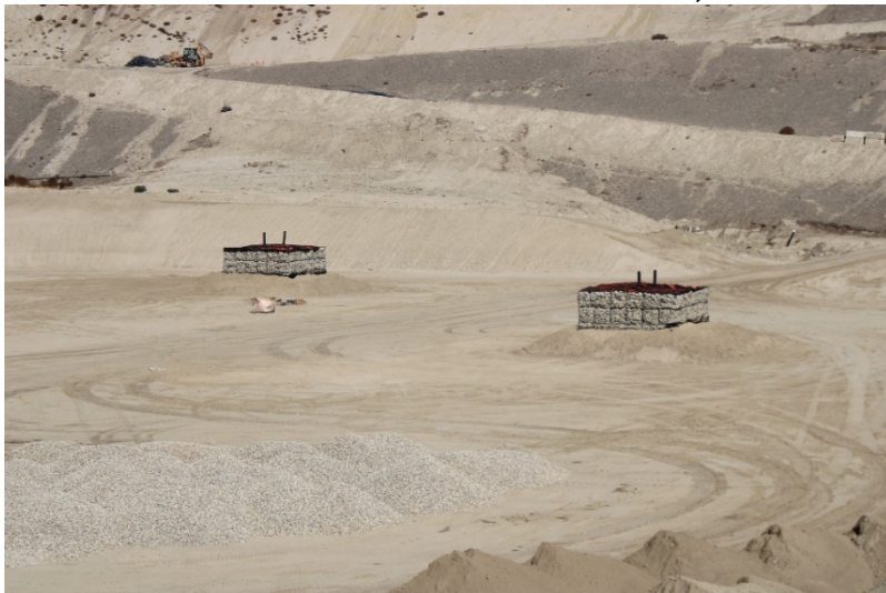
Photo 419: Cell 8 Construction: October 12, 2022
