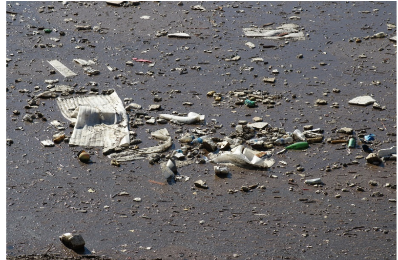
Photo 180: South Terminal and Catch Basins: December 14, 2022
