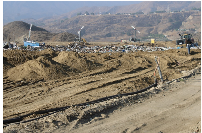
Photo 16: Top Deck Working Area: October 12, 2022
