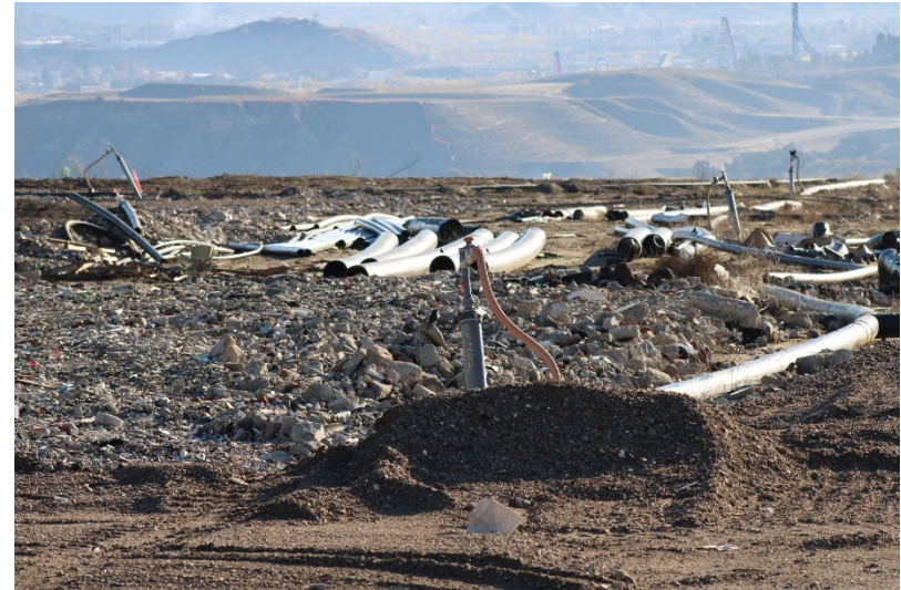
Photo 34: Top Deck Working Area: December 14, 2022
