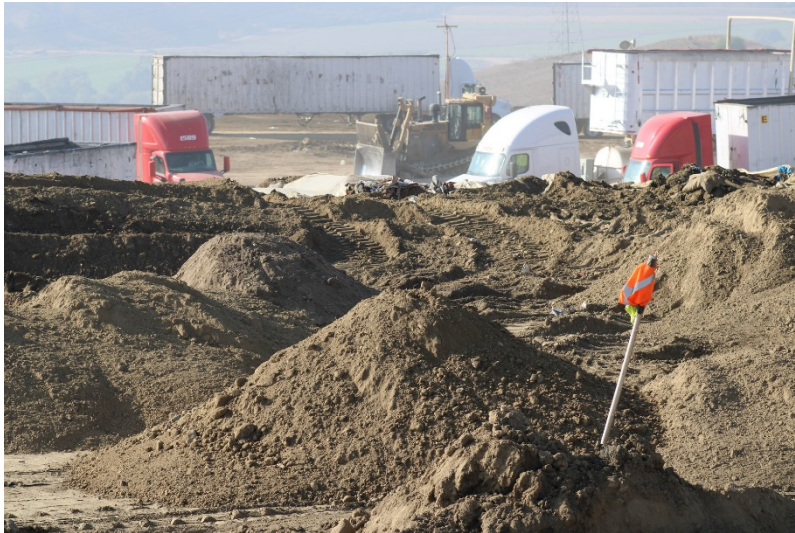
Photo 21: Top Deck Working Area: October 12, 2022
