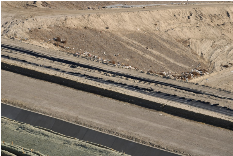
Photo 431: Cell 8 Construction: November 30, 2022
