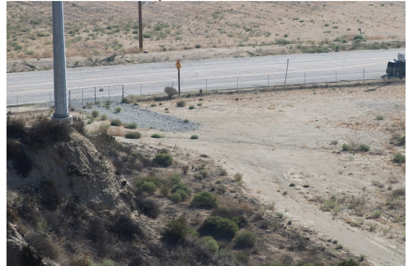
Photo 240: Wolcott Way Entrance Facilities: October 12, 2022
