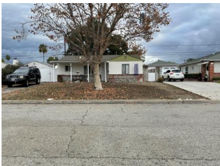
A one-story single-family home in Covina Islands. Note lack of sidewalk
