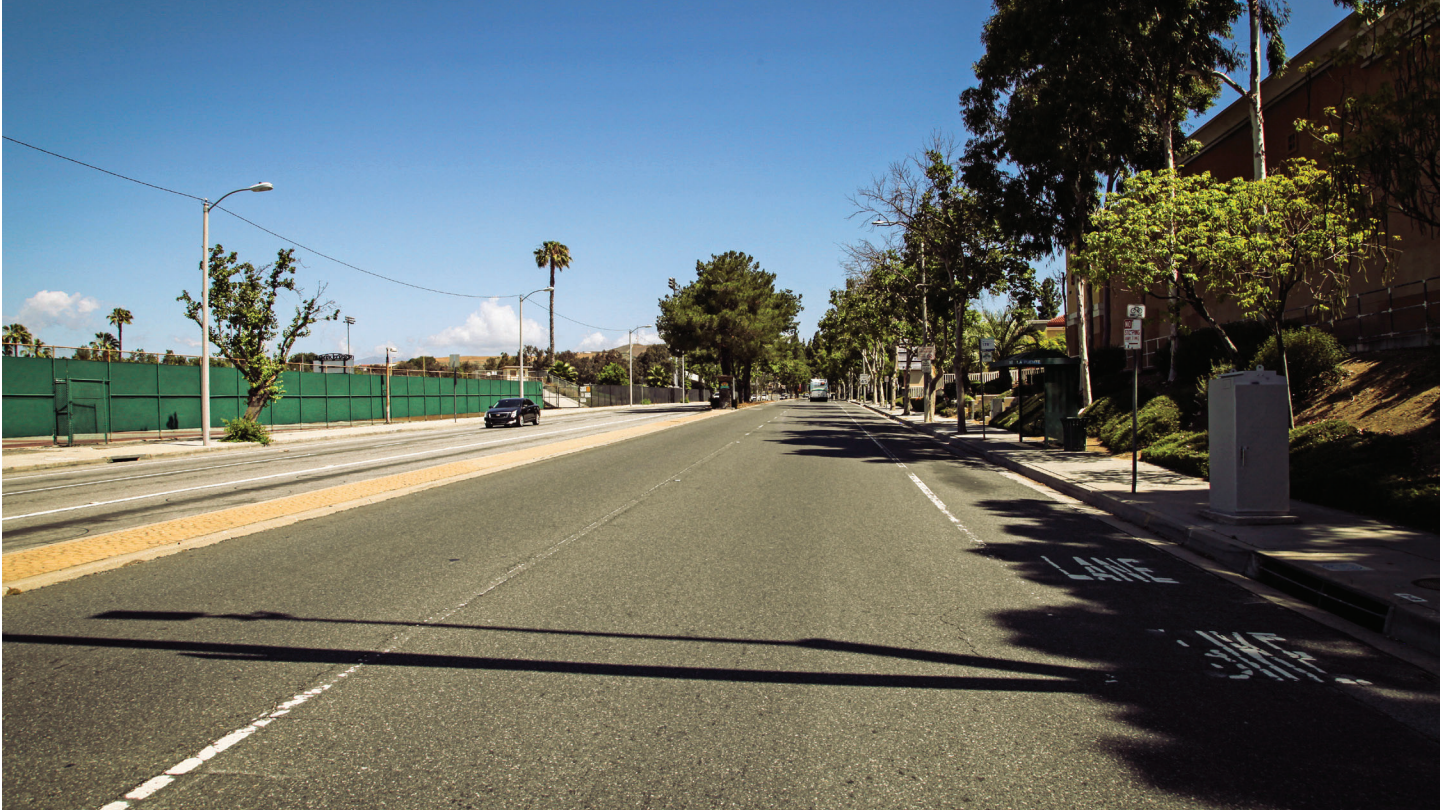
Typical Conditions (Before)
