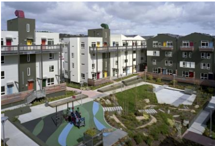
The open space area for this multifamily residential development incorporates both softscape areas and decorative hardscape.
