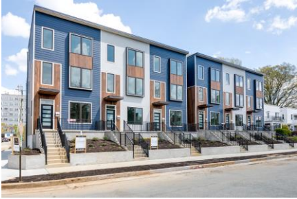
The above townhomes, in lieu of a landscaped parkway, have stoops that adjoin directly to the public sidewalk.
