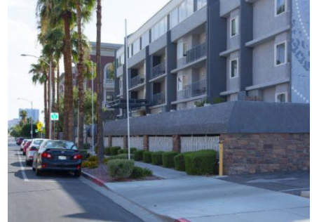
Decorative metal grills along the ground-level, sidewalk-facing façade help mask the podium parking.
