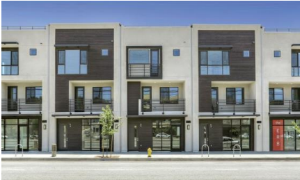
Balconies on the second level become overhangs at the ground level entrances of the above townhomes.
