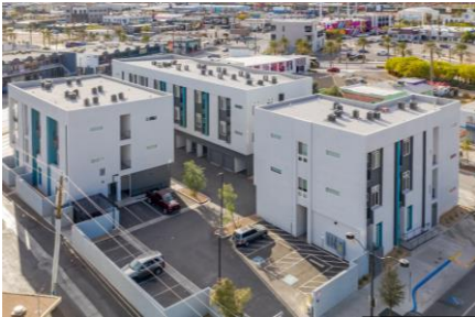
The surface parking behind the above multifamily development is located in the rear of the lot, set back from property lines, and incorporates landscaped islands in the design.
