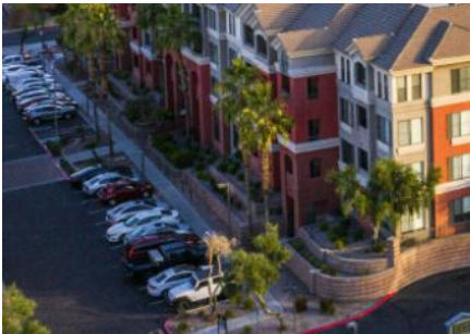
A walk path made from brick pavers creates a clearly visible and safer area for pedestrians to cut across the surface parking lot towards the multifamily development.
