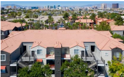
This multifamily development has a hipped roof with cross gables along the primary façade.
