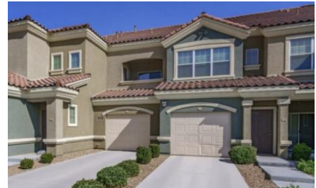
The townhomes above recess and project the entrances and garages to create a modulated front façade.
