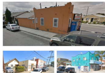
These are examples of Accessory Commercial Units that could be in your neighborhood.
