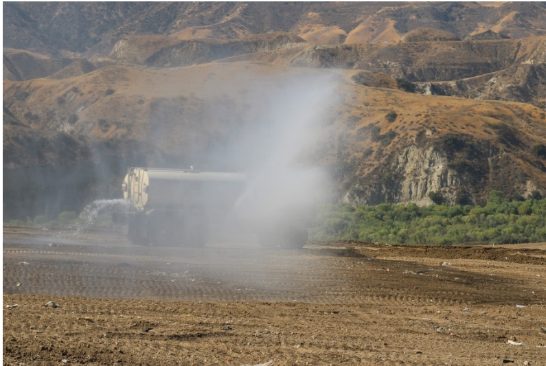
Photo 49: Cell 6 Working Area: July 21, 2022
