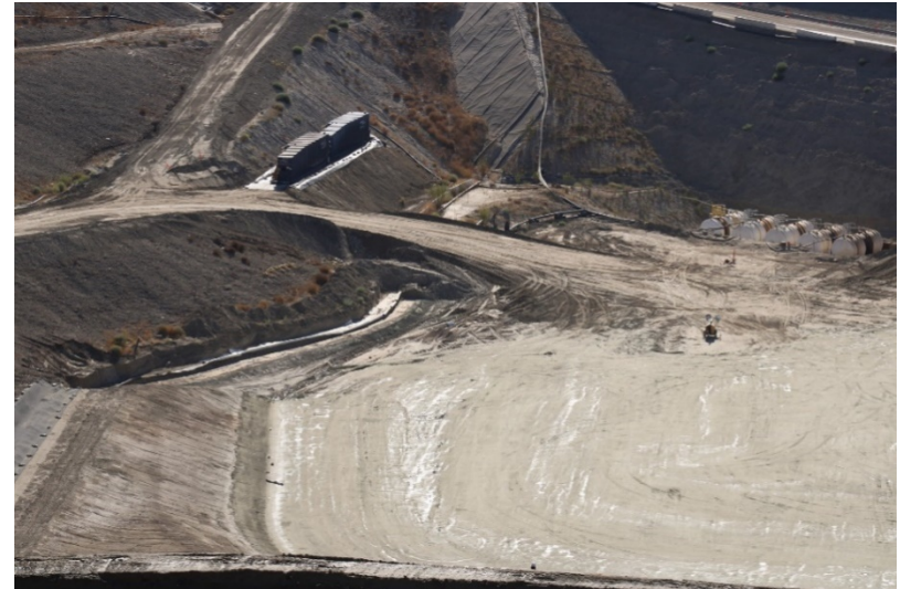
Photo 398: Cell 8 Construction: July 21, 2022
