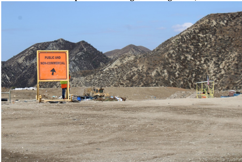
Photo 23: Top Deck Working Area: September 13, 2022
