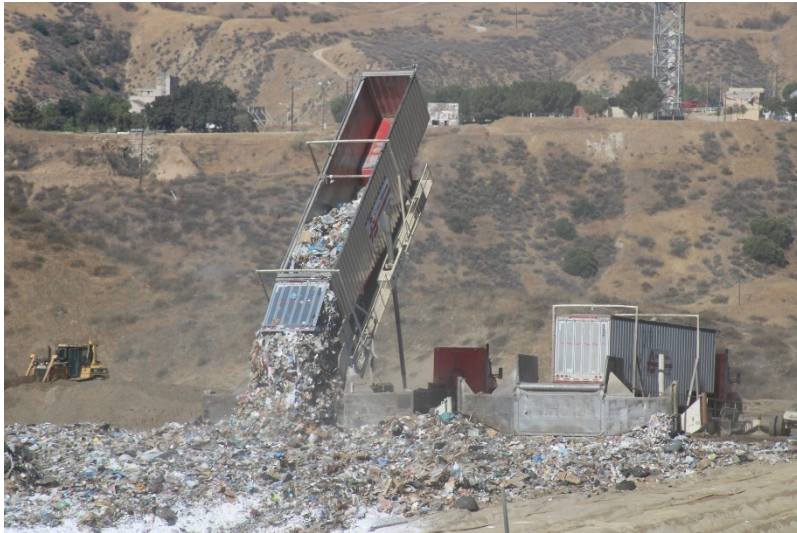
Photo 41: Cell 6 Working Area: July 21, 2022
