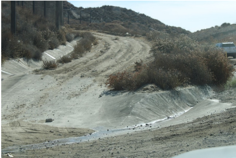
Photo 205: Landfill Perimeter Drainage Channel: July 21, 2022
