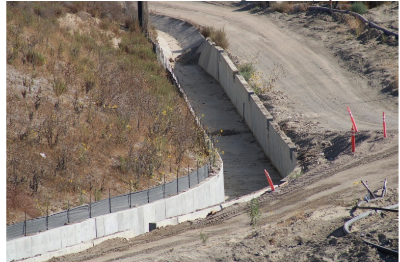
Photo 208: Landfill Perimeter Drainage Channel: August 23, 2022
