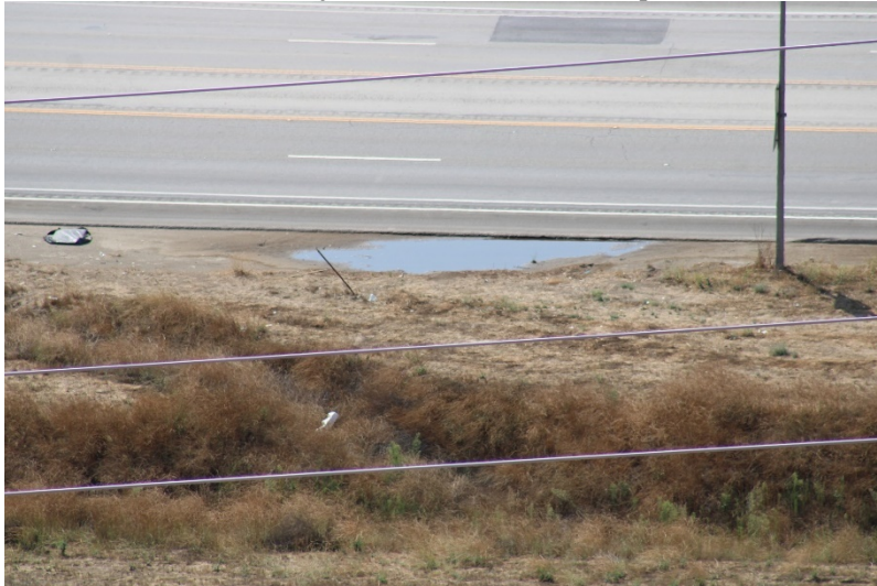
Photo 283: Wolcott Way Entrance Facilities: September 13, 2022
