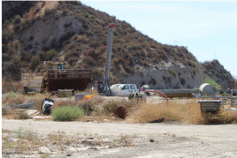
Photo 101: Closed Landfill - Primary Canyon: July 21, 2022
