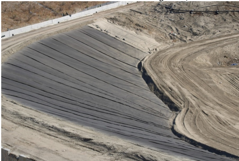
Photo 419: Cell 8 Construction: August 23, 2022
