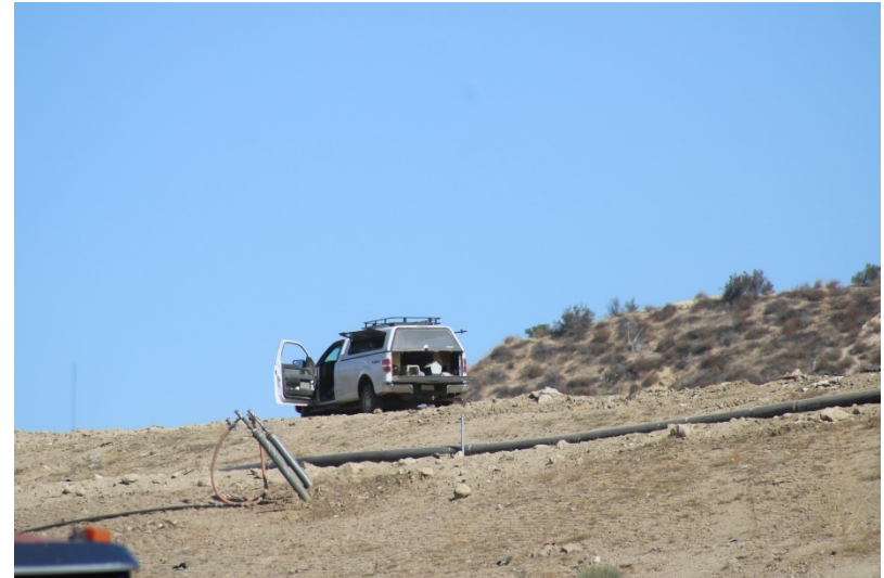
Photo 46: Cell 6 Working Area: July 21, 2022
