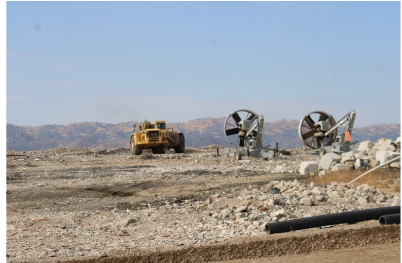
Photo 94: Cell 6 Working Area: September 13, 2022
