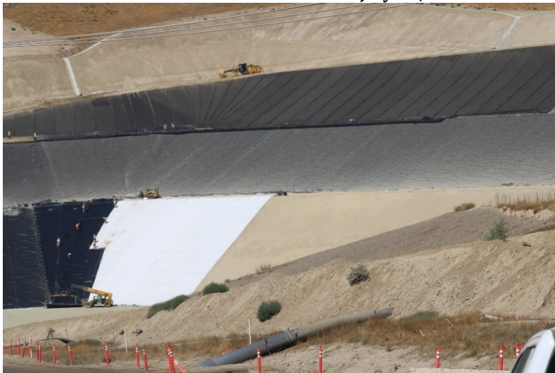
Photo 403: Cell 8 Construction: July 21, 2022
