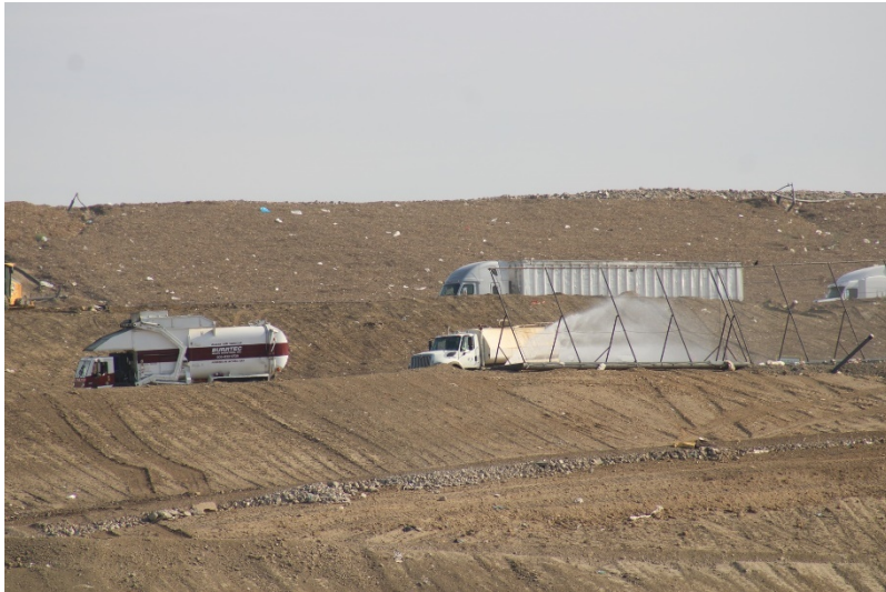
Photo 73: Cell 6 Working Area: September 13, 2022
