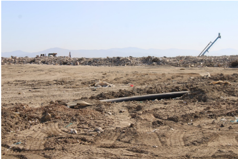
Photo 17: Top Deck Working Area: August 23, 2022
