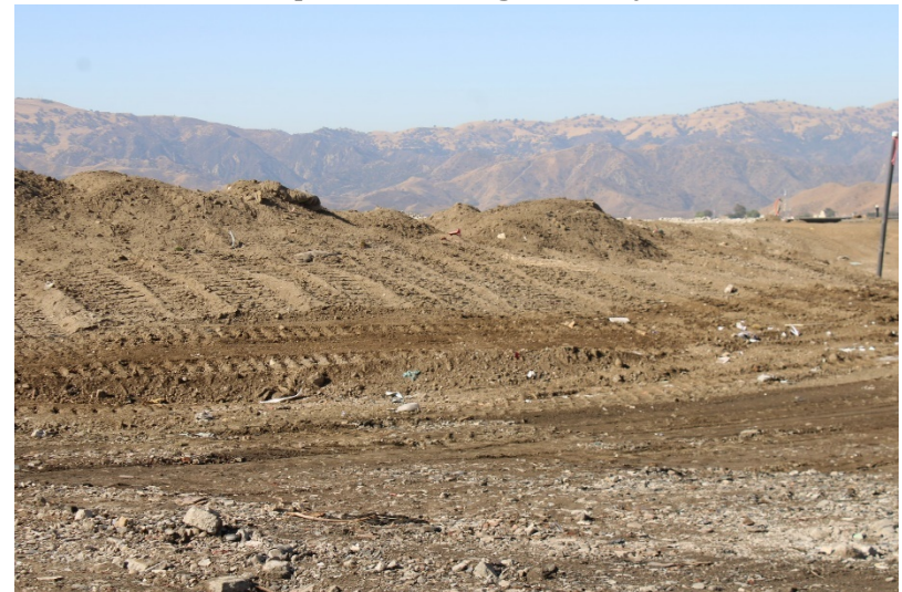
Photo 8: Top Deck Working Area: August 23, 2022
