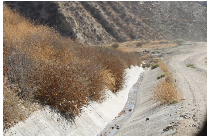
Photo 206: Landfill Perimeter Drainage Channel: July 21, 2022
