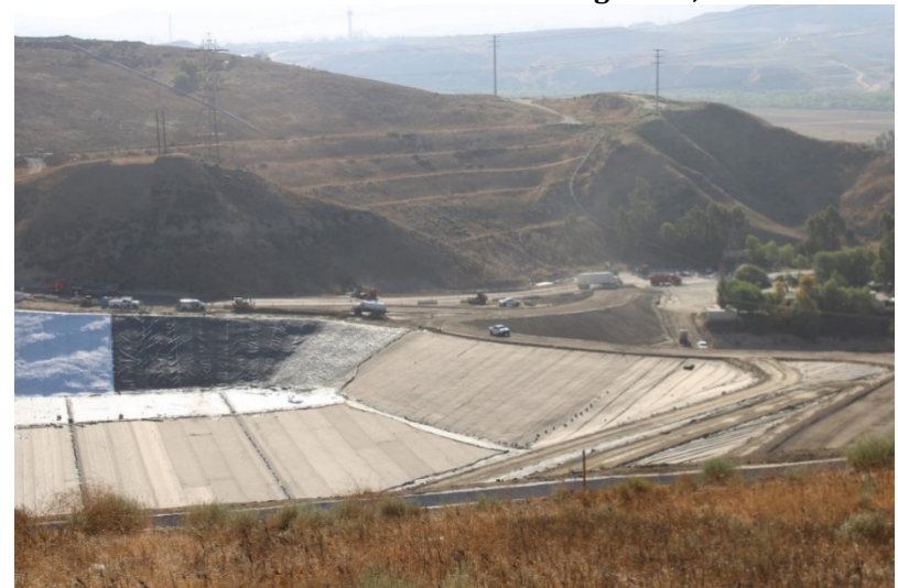
Photo 408: Cell 8 Construction: August 23, 2022
