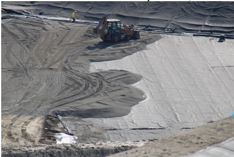
Photo 435: Cell 8 Construction: September 13, 2022
