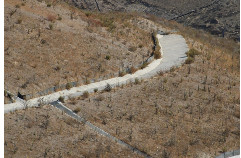
Photo 212: Landfill Perimeter Drainage Channel: August 23, 2022
