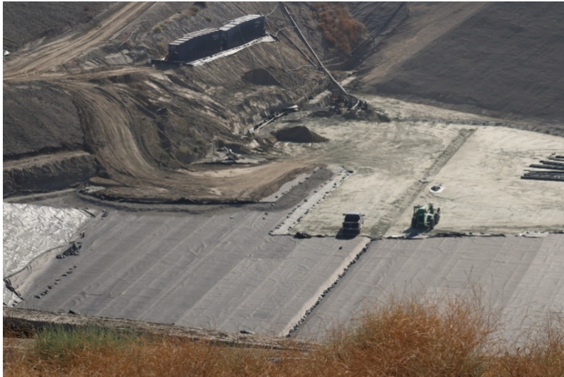
Photo 413: Cell 8 Construction: August 23, 2022
