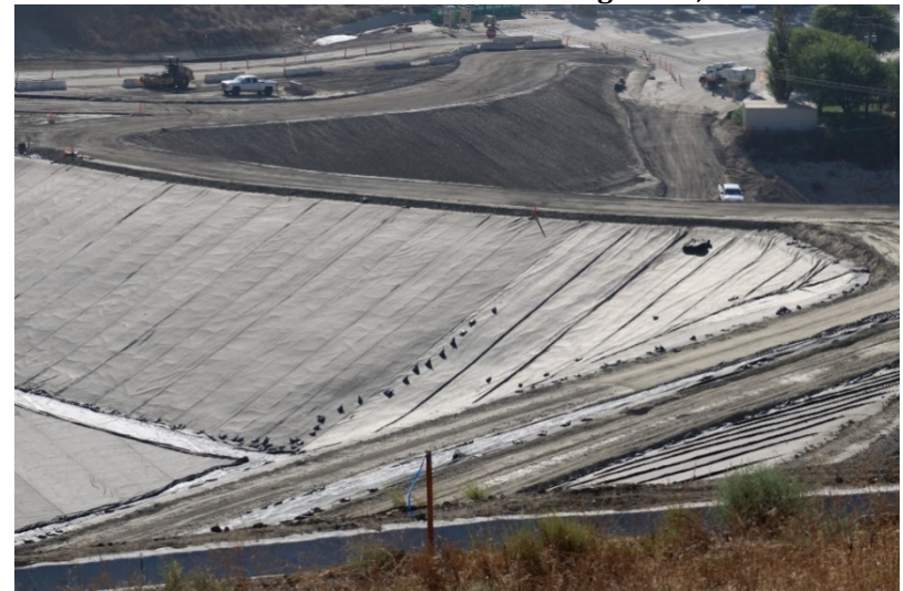
Photo 416: Cell 8 Construction: August 23, 2022
