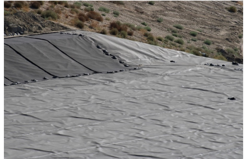
Photo 390: Cell 8 Construction: July 21, 2022
