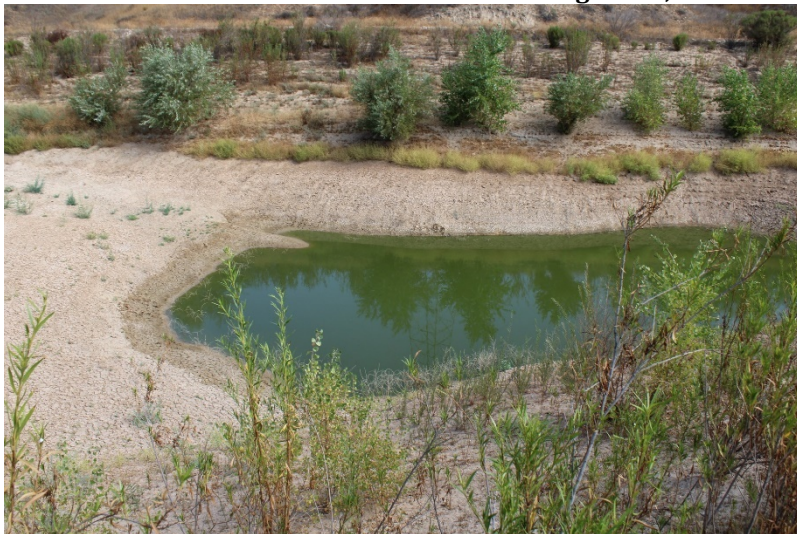
Photo 195: Northeast Sediment Basin: September 13, 2022
