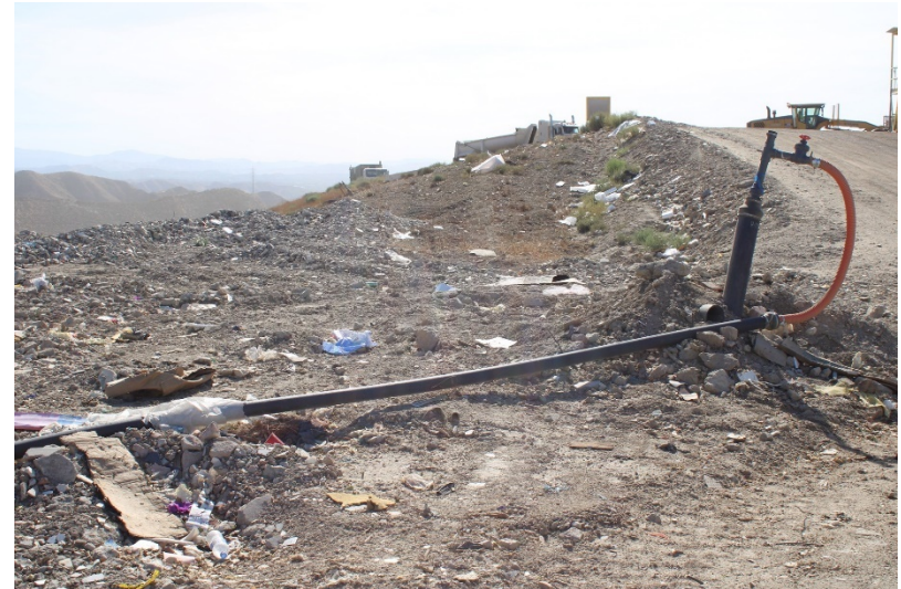
Photo 6: Top Deck Working Area: July 21, 2022
