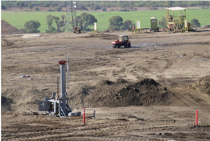
Photo 65: Cell 6 Working Area: August 23, 2022
