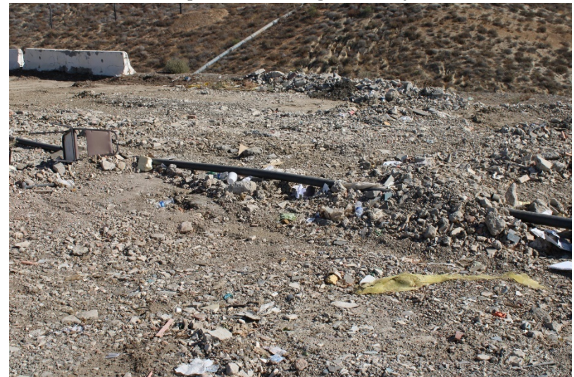
Photo 4: Top Deck Working Area: July 21, 2022
