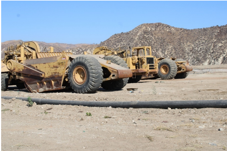
Photo 13: Top Deck Working Area: August 23, 2022
