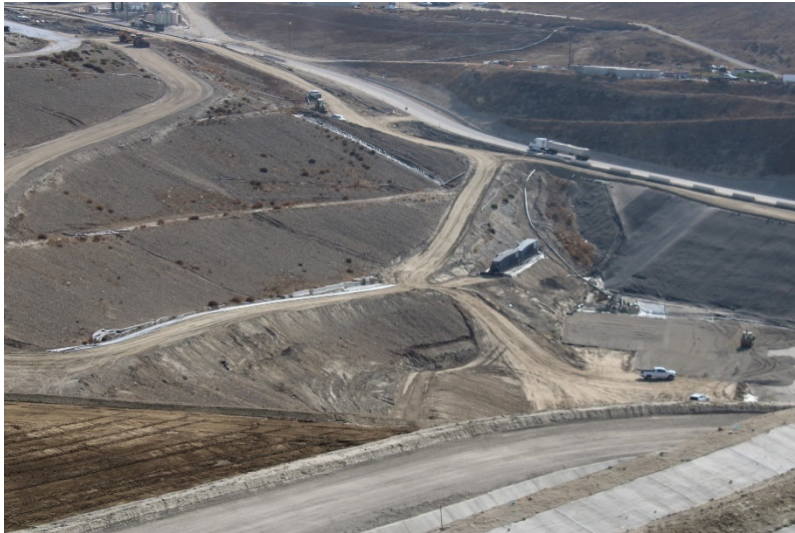
Photo 429: Cell 8 Construction: September 13, 2022
