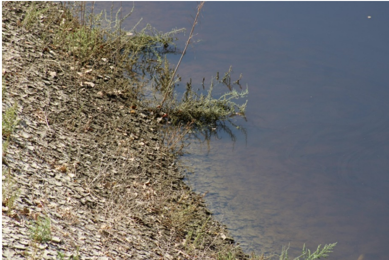
Photo 181: South Terminal and Catch Basins: September 13, 2022
