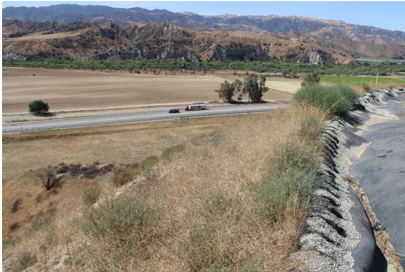
Photo 269: Wolcott Way Entrance Facilities: July 21, 2022
