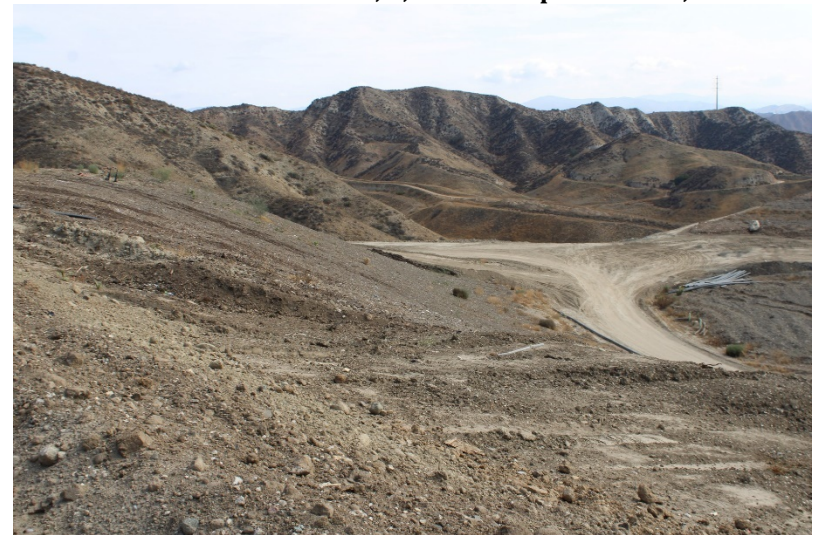
Photo 152: Future Cells 7, 9, and 10: September 13, 2022
