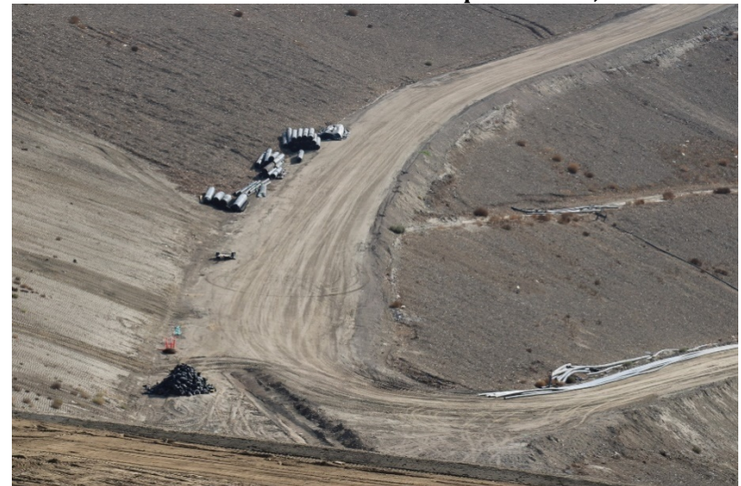
Photo 432: Cell 8 Construction: September 13, 2022
