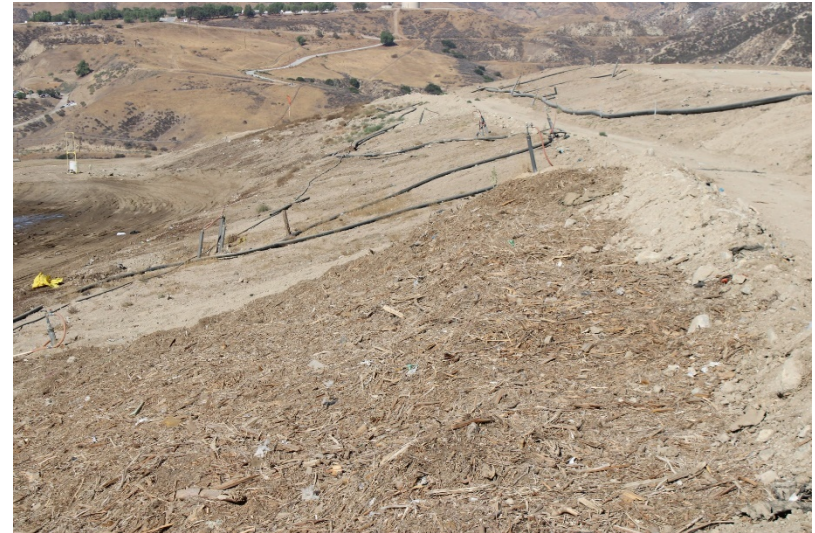
Photo 22: Top Deck Working Area: August 23, 2022
