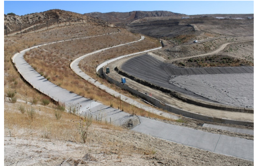
Photo 382: Cell 8 Construction: July 21, 2022
