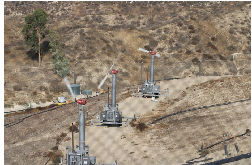
Photo 86: Cell 6 Working Area: September 13, 2022
