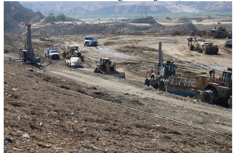
Photo 56: Cell 6 Working Area: August 23, 2022
