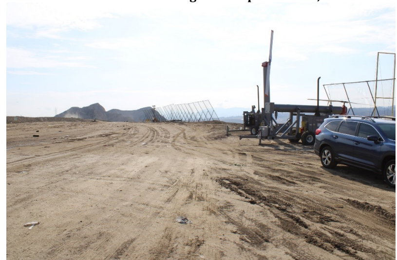
Photo 80: Cell 6 Working Area: September 13, 2022
