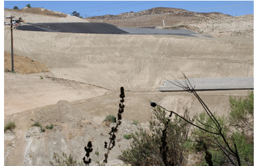
Photo 162: South Terminal and Catch Basins: July 21, 2022
