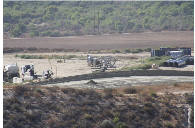
Photo 98: Closed Landfill - Primary Canyon: July 21, 2022
