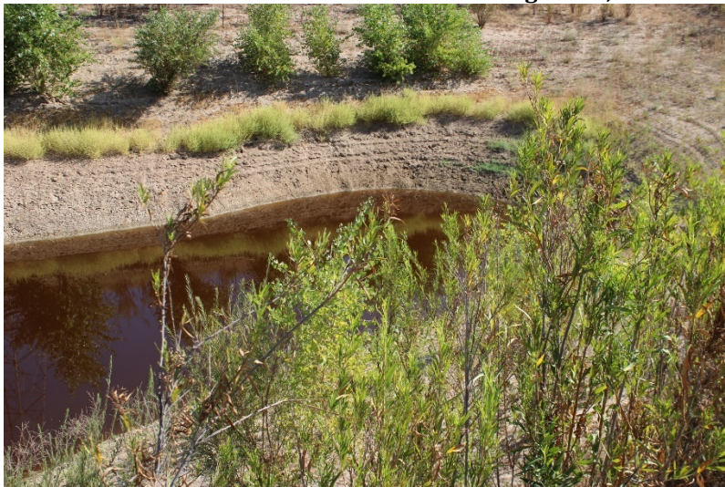
Photo 191: Northeast Sediment Basin: August 23, 2022
