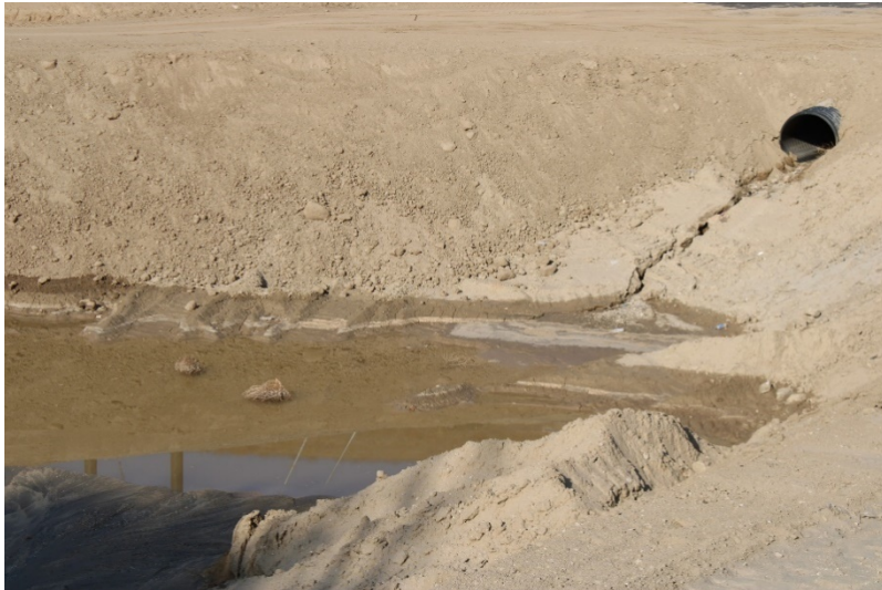
Photo 425: Cell 8 Construction: September 13, 2022
