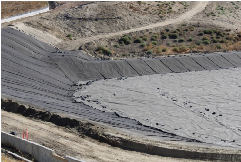
Photo 385: Cell 8 Construction: July 21, 2022
