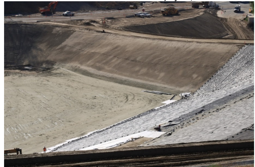
Photo 400: Cell 8 Construction: July 21, 2022
