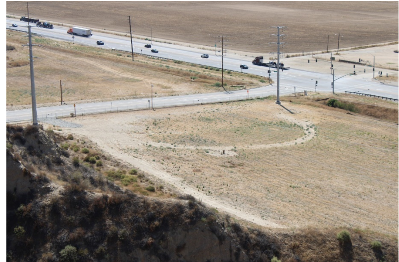
Photo 270: Wolcott Way Entrance Facilities: July 21, 2022
