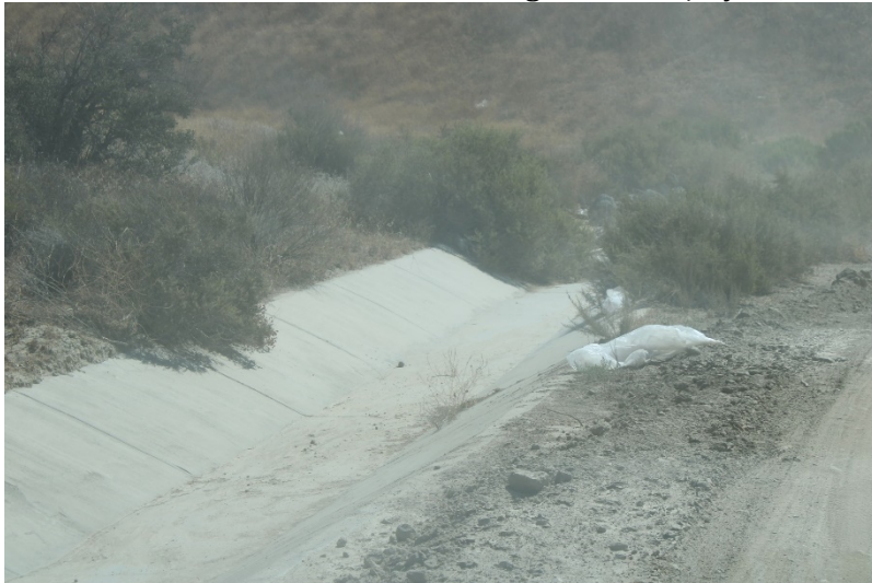
Photo 207: Landfill Perimeter Drainage Channel: July 21, 2022
