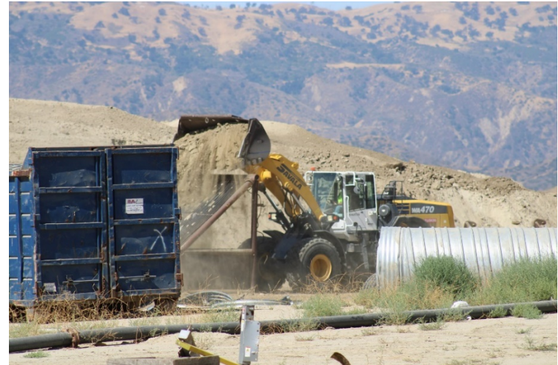
Photo 110: Closed Landfill - Primary Canyon: July 21, 2022
