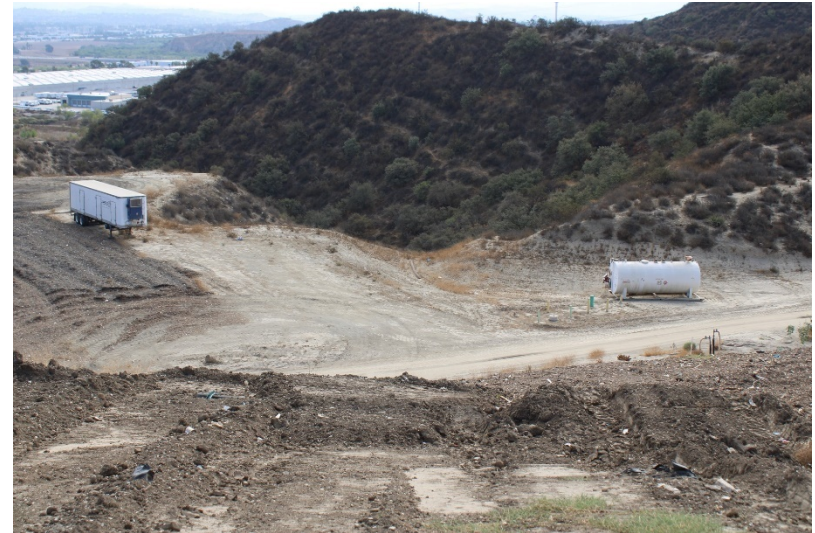
Photo 154: Future Cells 7, 9, and 10: September 13, 2022
