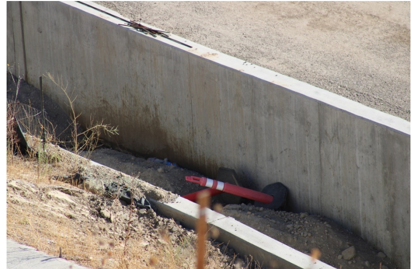
Photo 210: Landfill Perimeter Drainage Channel: August 23, 2022
