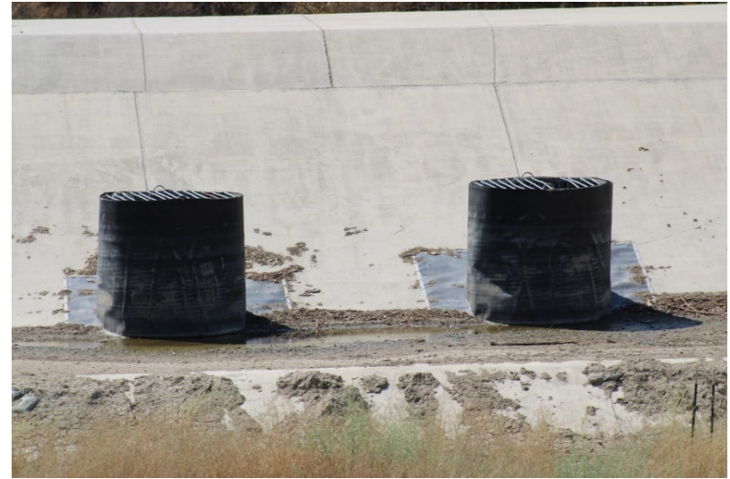
Photo 178: South Terminal and Catch Basins: September 13, 2022
