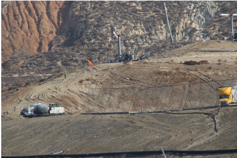
Photo 69: Cell 6 Working Area: September 13, 2022
