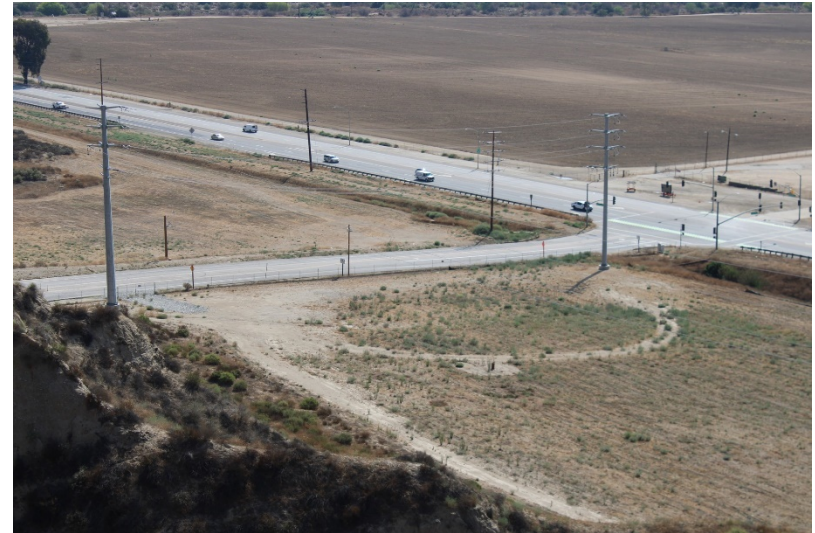
Photo 282: Wolcott Way Entrance Facilities: September 13, 2022
