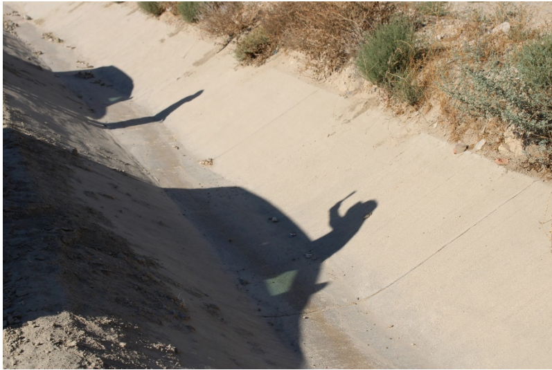
Photo 217: Landfill Perimeter Drainage Channel: August 23, 2022
