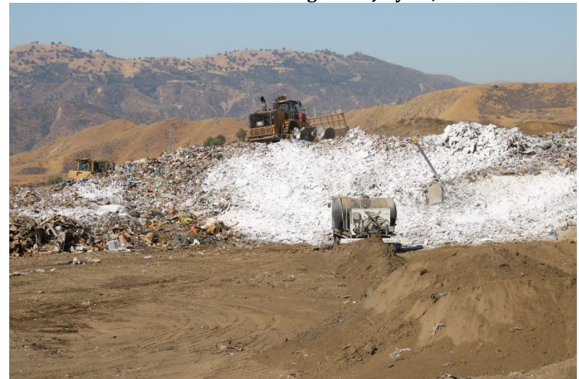
Photo 44: Cell 6 Working Area: July 21, 2022
