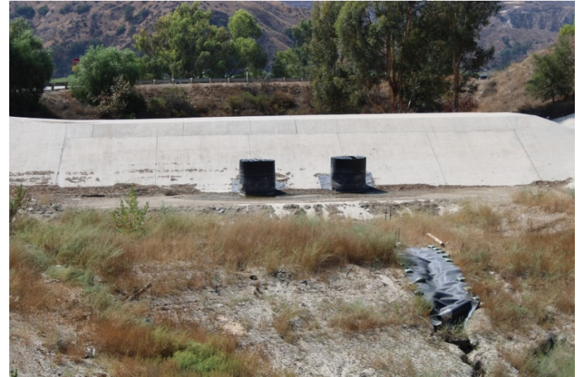
Photo 176: South Terminal and Catch Basins: September 13, 2022
