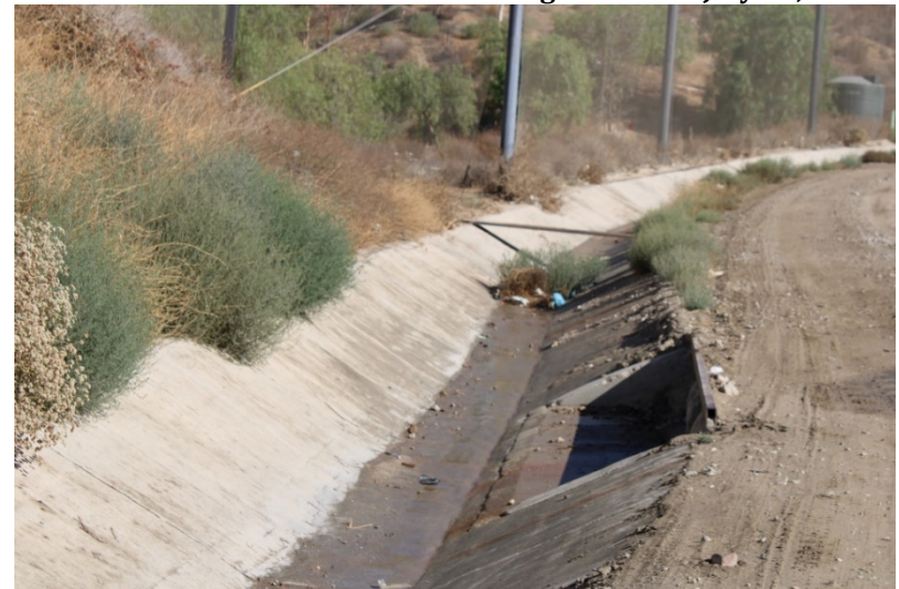
Photo 204: Landfill Perimeter Drainage Channel: July 21, 2022
