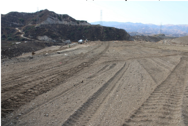
Photo 151: Future Cells 7, 9, and 10: September 13, 2022
