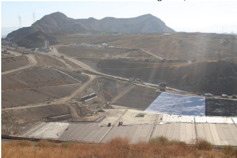
Photo 407: Cell 8 Construction: August 23, 2022
