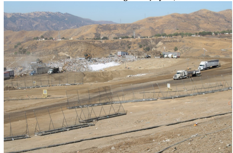
Photo 32: Cell 6 Working Area: July 21, 2022
