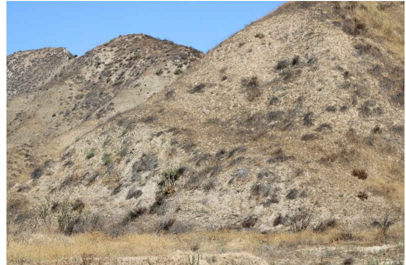
Photo 130: Closed Landfill - Canyon B: July 21, 2022
