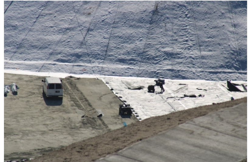
Photo 422: Cell 8 Construction: August 23, 2022
