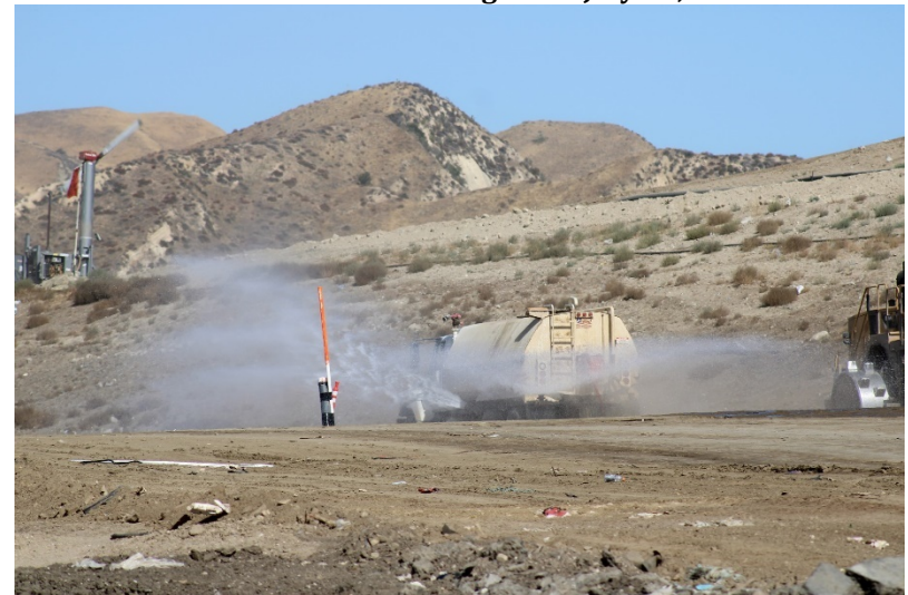
Photo 48: Cell 6 Working Area: July 21, 2022
