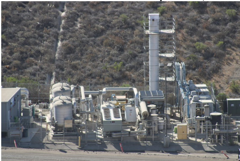
Photo 263: Gas-to-Energy Facility: July 21, 2022
