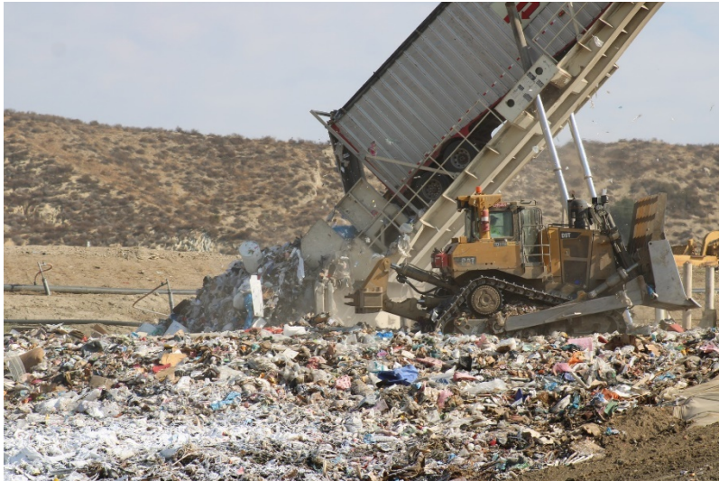
Photo 89: Cell 6 Working Area: September 13, 2022
