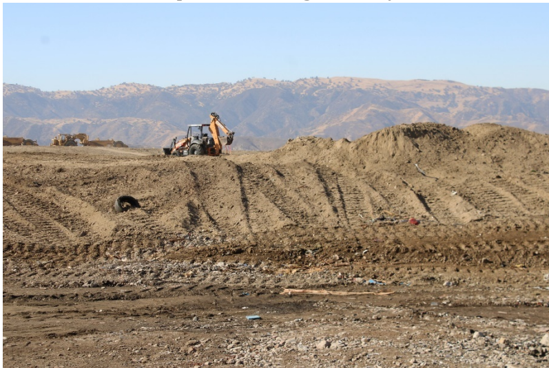
Photo 7: Top Deck Working Area: August 23, 2022
