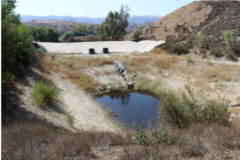
Photo 175: South Terminal and Catch Basins: September 13, 2022
