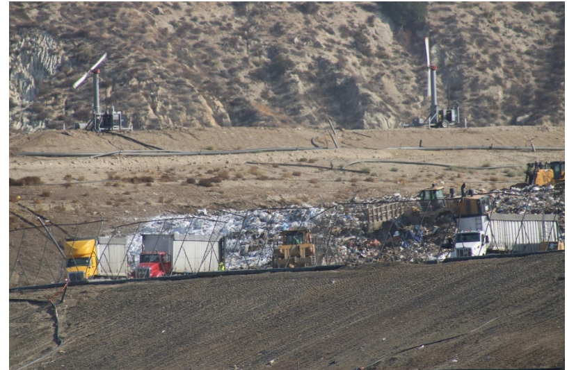
Photo 70: Cell 6 Working Area: September 13, 2022
