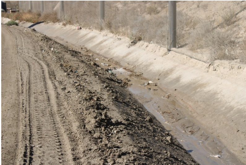
Photo 201: Landfill Perimeter Drainage Channel: July 21, 2022
