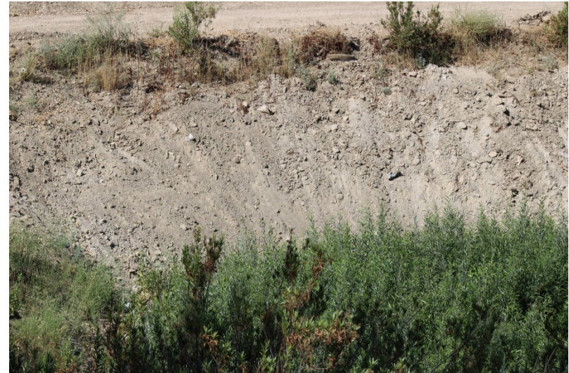
Photo 170: South Terminal and Catch Basins: August 23, 2022
