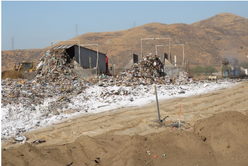
Photo 45: Cell 6 Working Area: July 21, 2022
