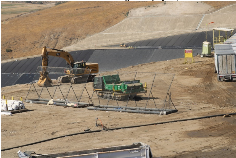
Photo 35: Cell 6 Working Area: July 21, 2022
