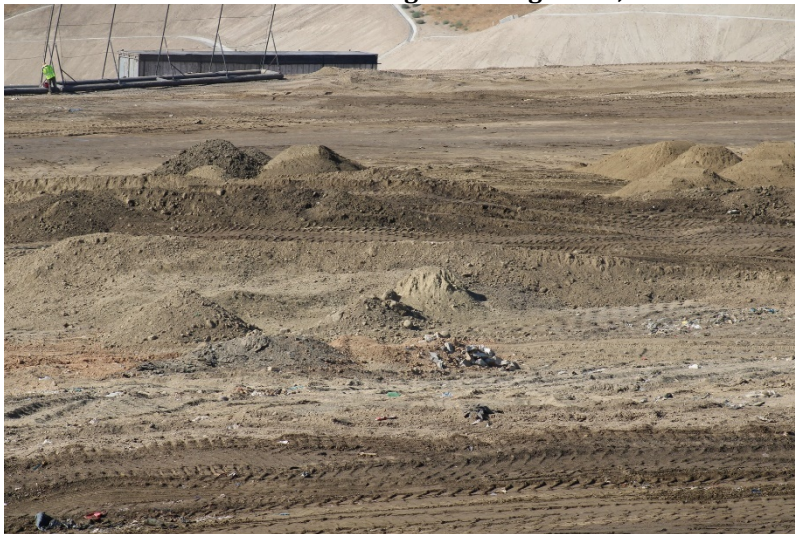
Photo 67: Cell 6 Working Area: August 23, 2022
