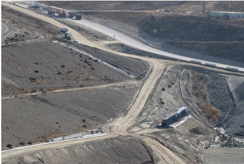
Photo 433: Cell 8 Construction: September 13, 2022
