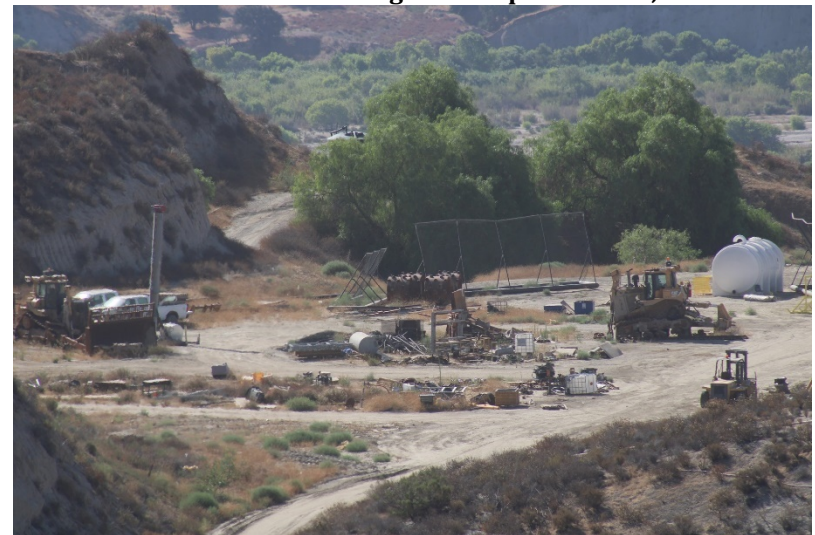
Photo 96: Closed Landfill - Primary Canyon: July 21, 2022
