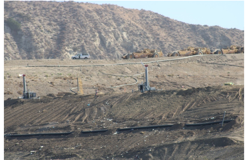
Photo 26: Cell 6 Working Area: July 21, 2022
