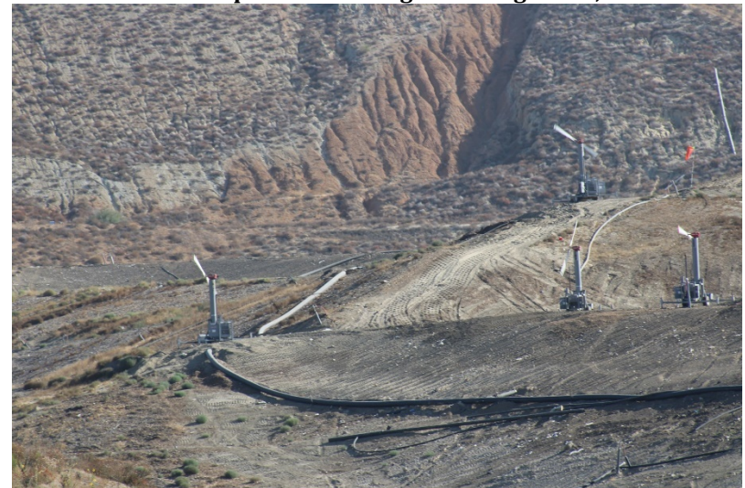
Photo 24: Cell 6 Working Area: July 21, 2022
