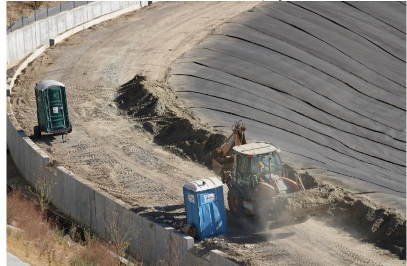
Photo 388: Cell 8 Construction: July 21, 2022
