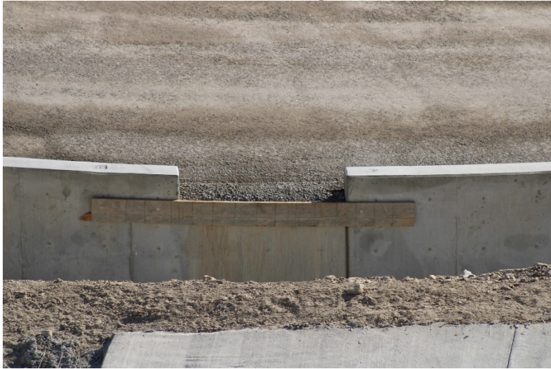
Photo 211: Landfill Perimeter Drainage Channel: August 23, 2022
