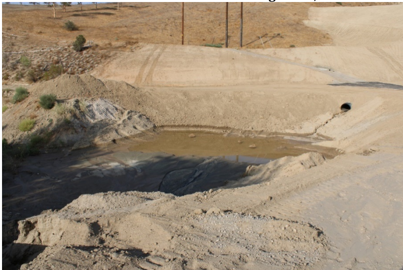
Photo 423: Cell 8 Construction: September 13, 2022
