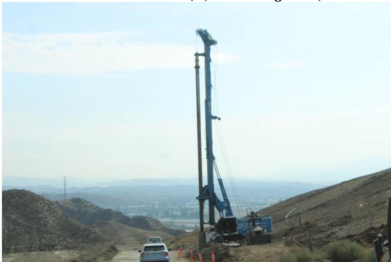
Photo 147: Future Cells 7, 9, and 10: September 13, 2022
