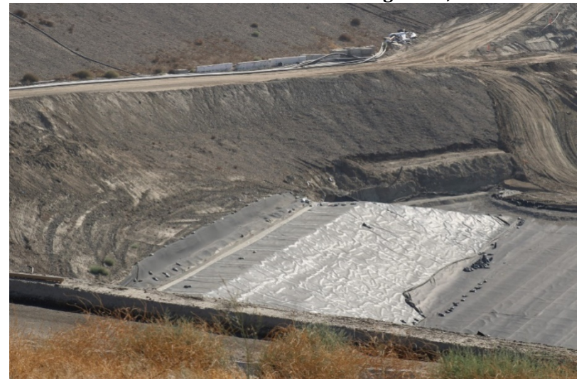
Photo 412: Cell 8 Construction: August 23, 2022
