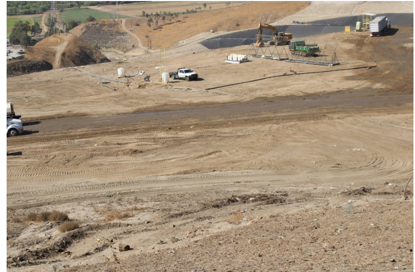
Photo 30: Cell 6 Working Area: July 21, 2022
