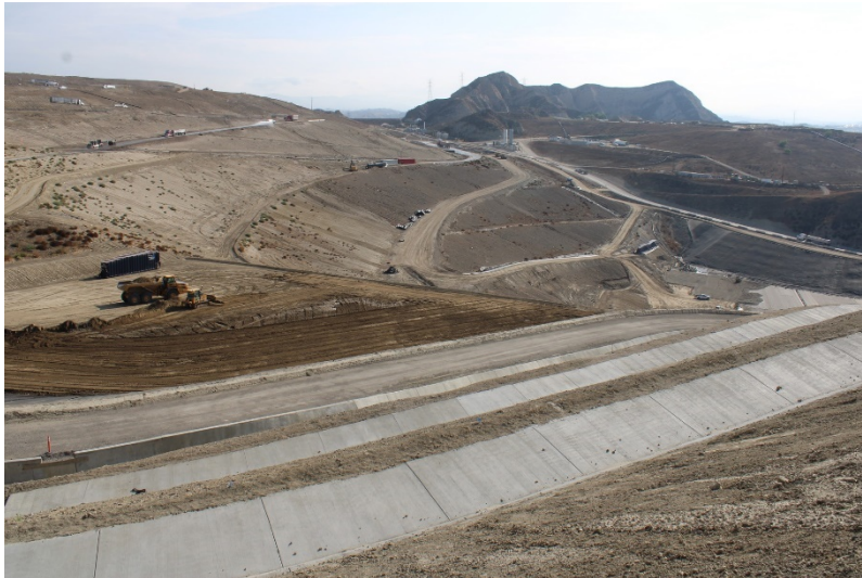
Photo 221: Landfill Perimeter Drainage Channel: September 13, 2022
