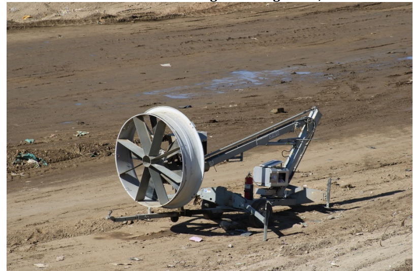
Photo 68: Cell 6 Working Area: August 23, 2022
