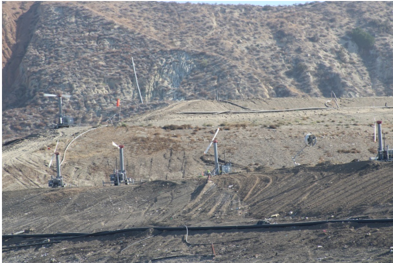
Photo 25: Cell 6 Working Area: July 21, 2022
