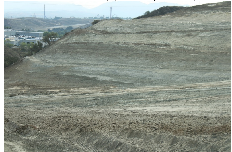
Photo 156: Future Cells 7, 9, and 10: September 13, 2022
