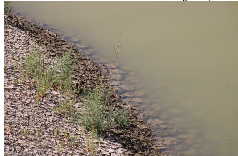
Photo 168: South Terminal and Catch Basins: August 23, 2022
