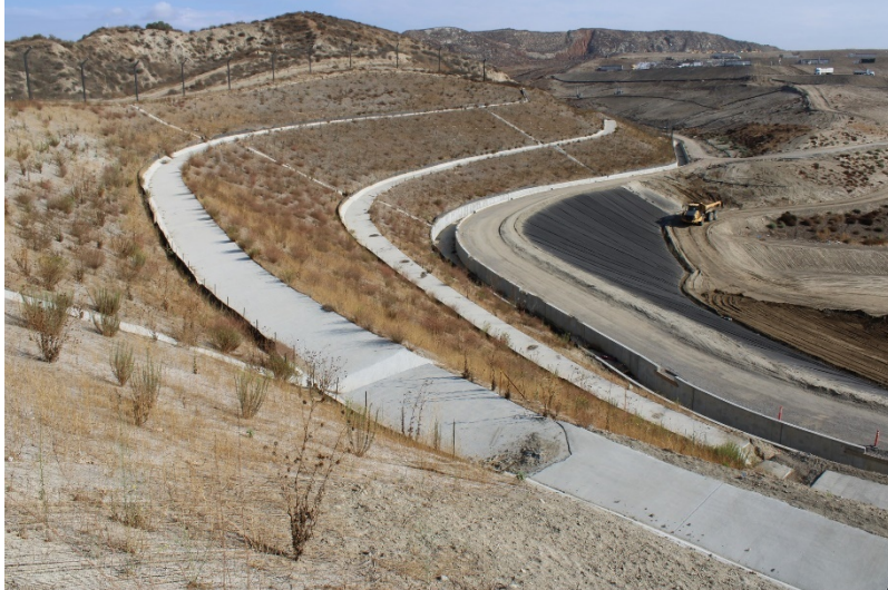
Photo 219: Landfill Perimeter Drainage Channel: September 13, 2022
