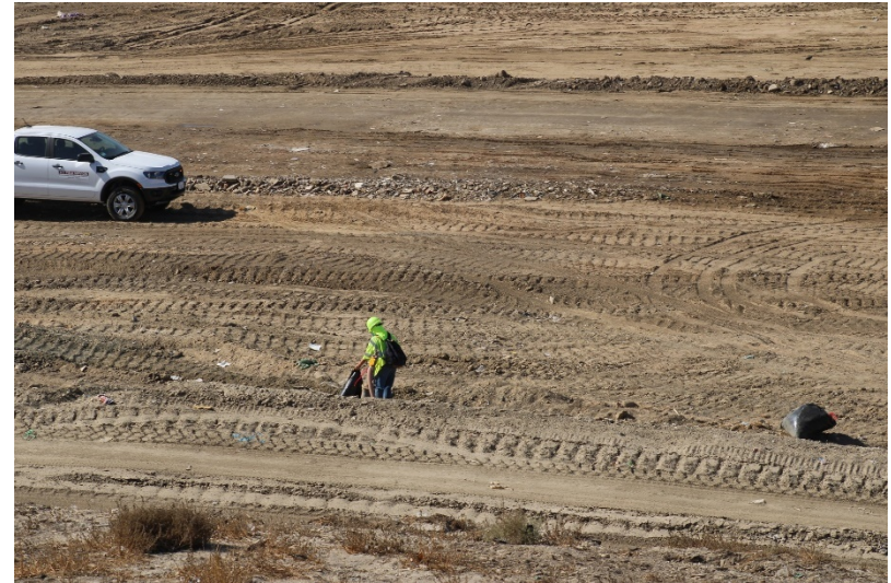
Photo 34: Cell 6 Working Area: July 21, 2022
