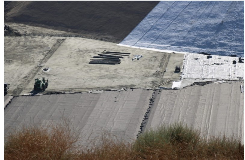
Photo 414: Cell 8 Construction: August 23, 2022
