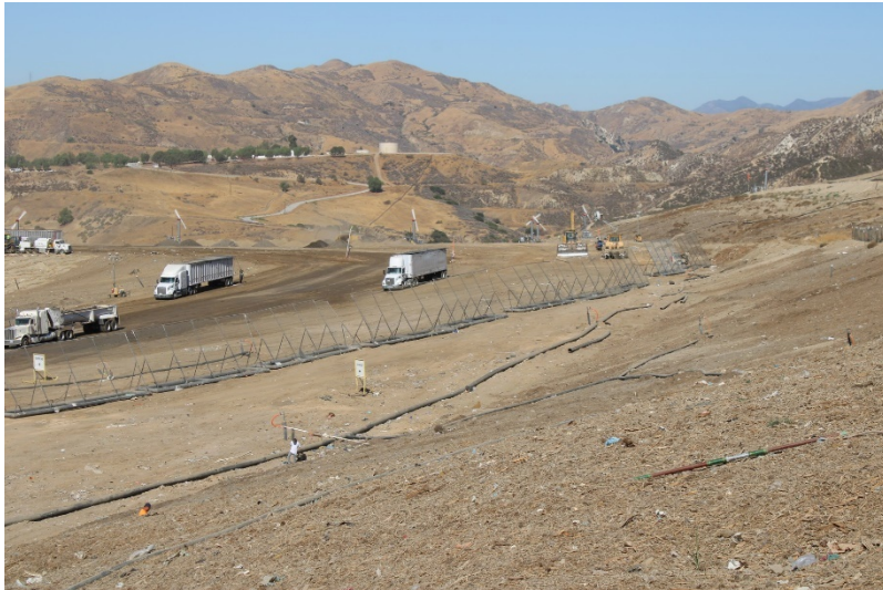
Photo 33: Cell 6 Working Area: July 21, 2022
