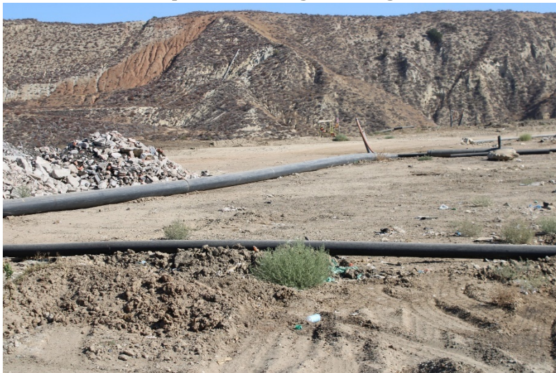
Photo 15: Top Deck Working Area: August 23, 2022
