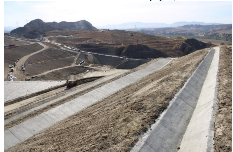
Photo 384: Cell 8 Construction: July 21, 2022
