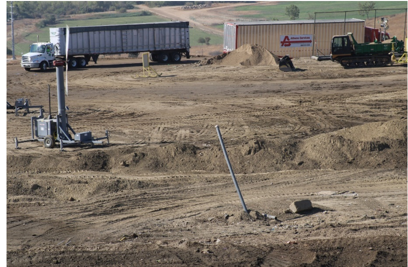
Photo 66: Cell 6 Working Area: August 23, 2022
