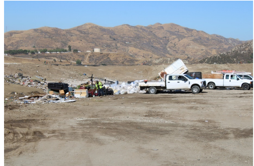
Photo 2: Top Deck Working Area: July 21, 2022
