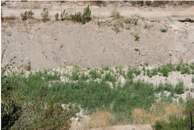
Photo 161: South Terminal and Catch Basins: July 21, 2022
