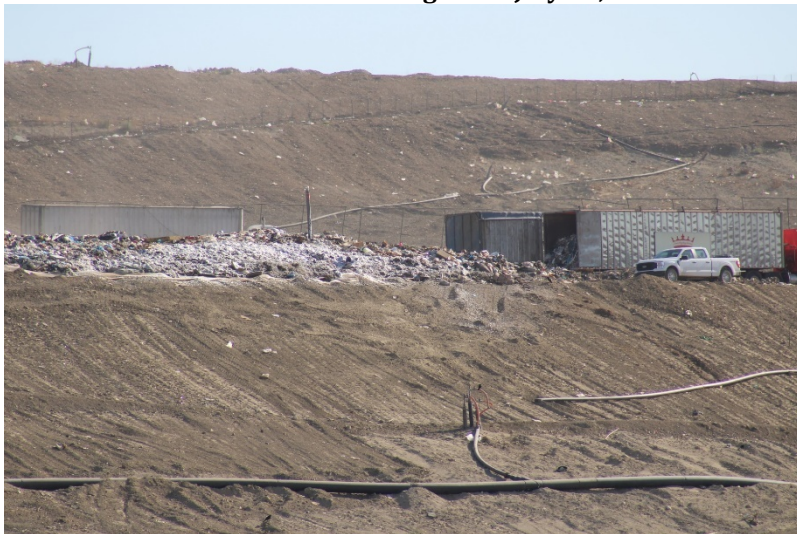
Photo 27: Cell 6 Working Area: July 21, 2022
