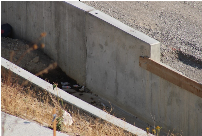
Photo 227: Landfill Perimeter Drainage Channel: September 13, 2022
