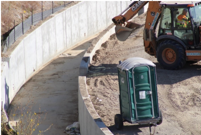
Photo 395: Cell 8 Construction: July 21, 2022
