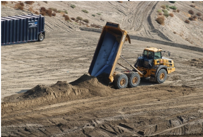
Photo 431: Cell 8 Construction: September 13, 2022
