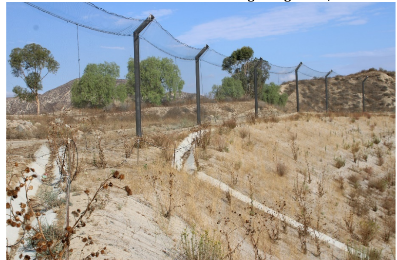
Photo 240: Westside Perimeter Ridge: September 13, 2022
