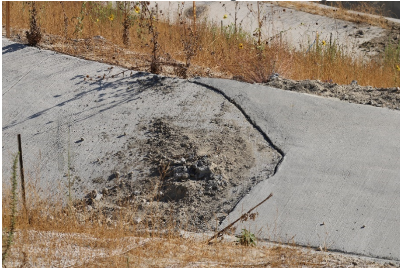
Photo 215: Landfill Perimeter Drainage Channel: August 23, 2022
