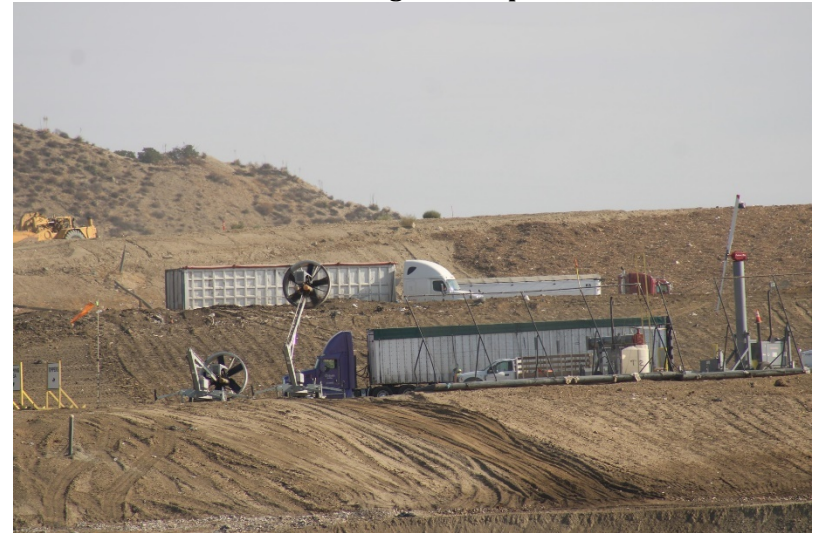
Photo 72: Cell 6 Working Area: September 13, 2022
