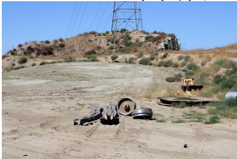
Photo 103: Closed Landfill - Primary Canyon: July 21, 2022
