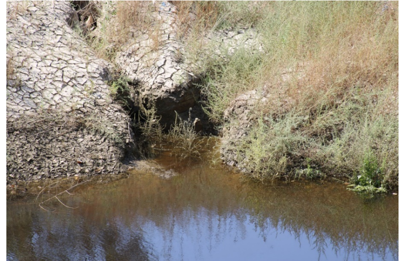
Photo 180: South Terminal and Catch Basins: September 13, 2022
