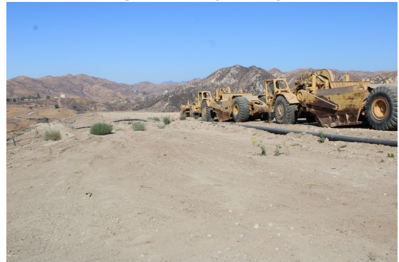
Photo 12: Top Deck Working Area: August 23, 2022
