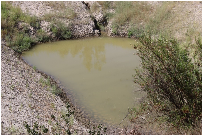
Photo 165: South Terminal and Catch Basins: August 23, 2022
