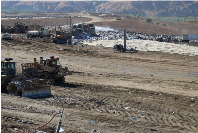
Photo 57: Cell 6 Working Area: August 23, 2022
