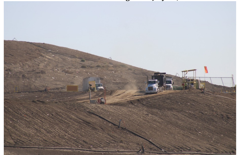
Photo 28: Cell 6 Working Area: July 21, 2022
