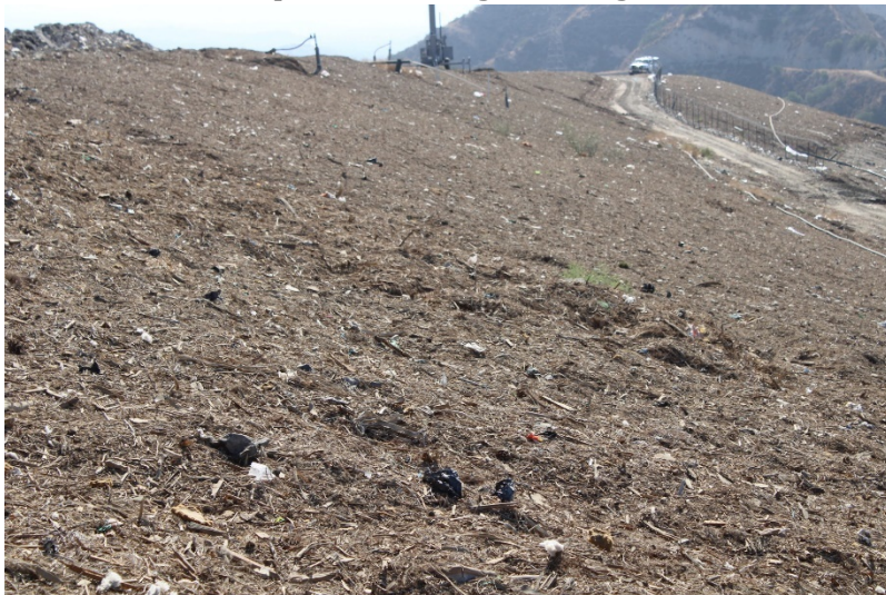
Photo 19: Top Deck Working Area: August 23, 2022
