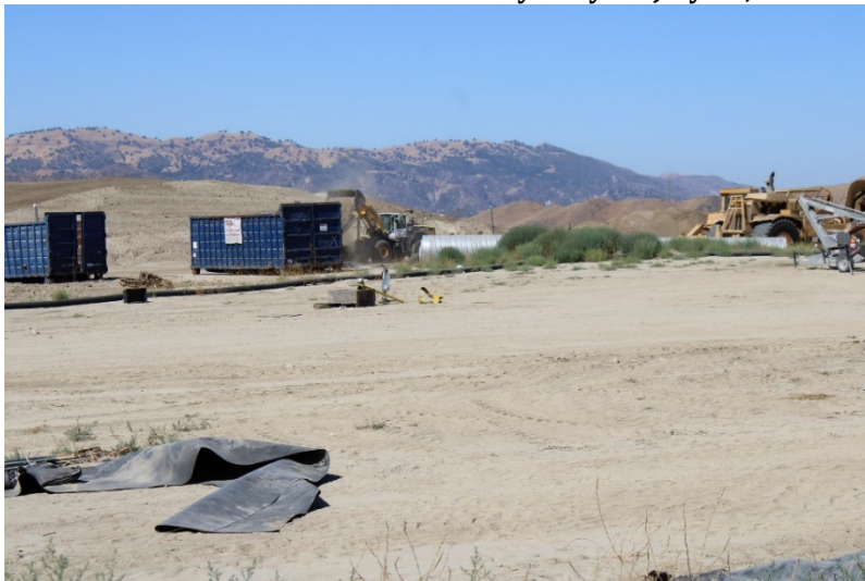
Photo 107: Closed Landfill - Primary Canyon: July 21, 2022
