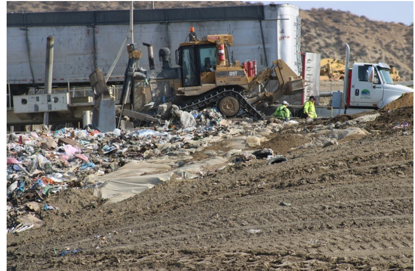
Photo 90: Cell 6 Working Area: September 13, 2022
