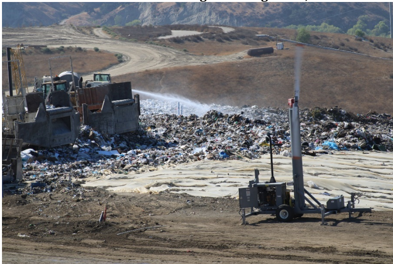
Photo 63: Cell 6 Working Area: August 23, 2022
