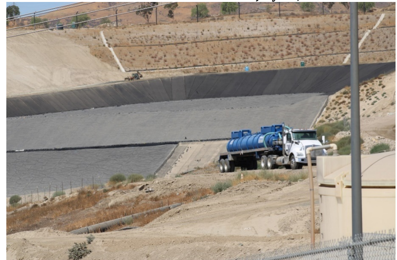
Photo 404: Cell 8 Construction: July 21, 2022
