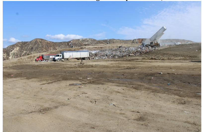
Photo 76: Cell 6 Working Area: September 13, 2022
