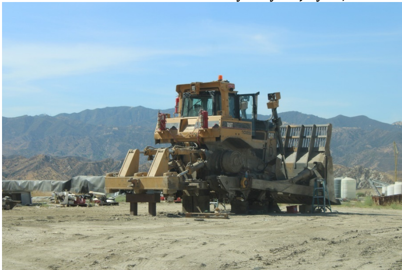
Photo 99: Closed Landfill - Primary Canyon: July 21, 2022
