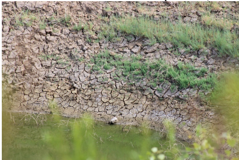
Photo 199: Northeast Sediment Basin: September 13, 2022
