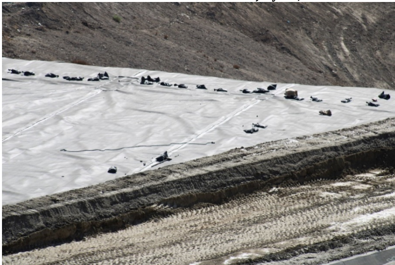
Photo 391: Cell 8 Construction: July 21, 2022
