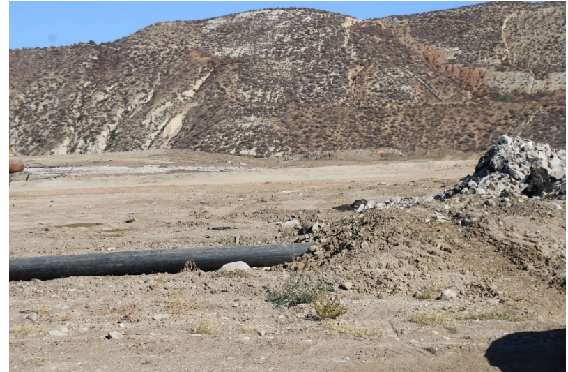
Photo 14: Top Deck Working Area: August 23, 2022
