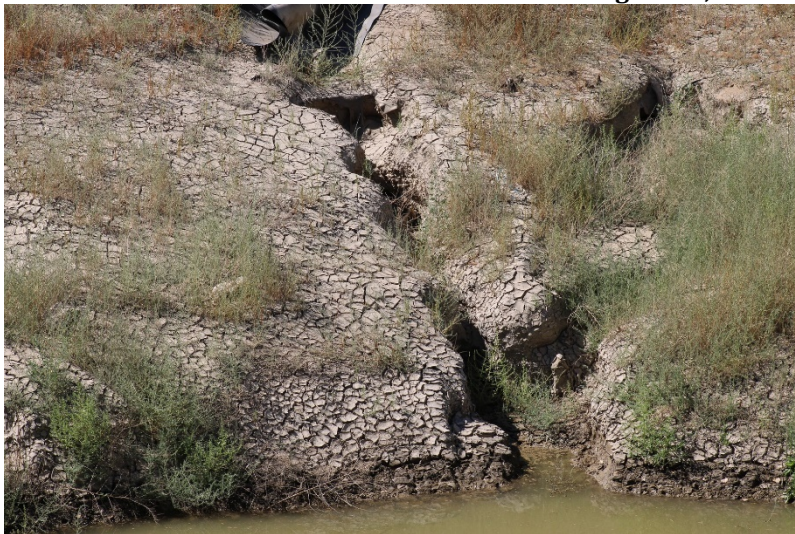
Photo 167: South Terminal and Catch Basins: August 23, 2022
