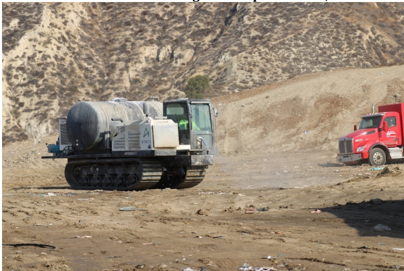
Photo 87: Cell 6 Working Area: September 13, 2022
