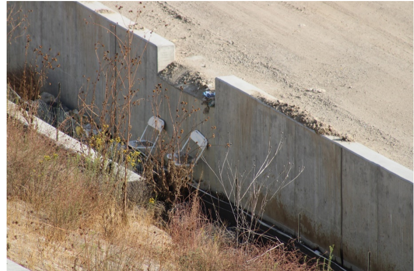
Photo 226: Landfill Perimeter Drainage Channel: September 13, 2022
