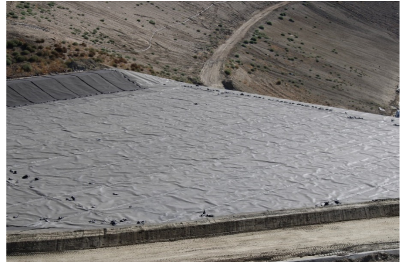
Photo 386: Cell 8 Construction: July 21, 2022
