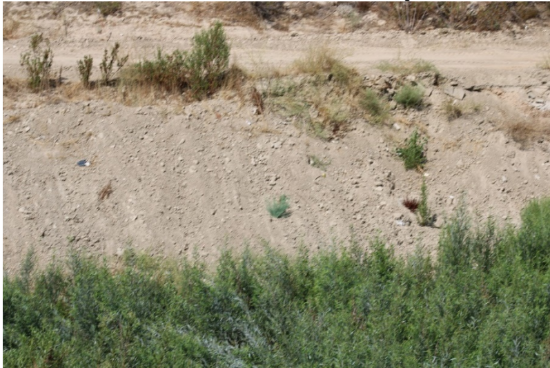
Photo 183: South Terminal and Catch Basins: September 13, 2022
