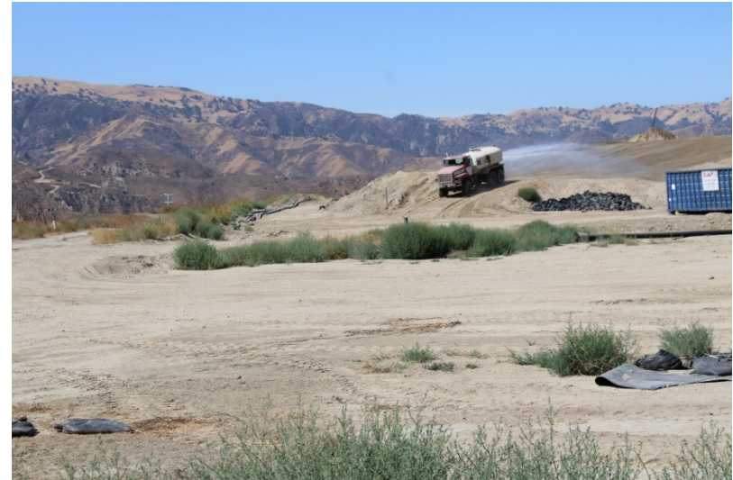
Photo 106: Closed Landfill - Primary Canyon: July 21, 2022
