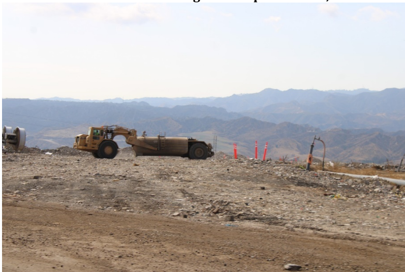
Photo 95: Cell 6 Working Area: September 13, 2022
