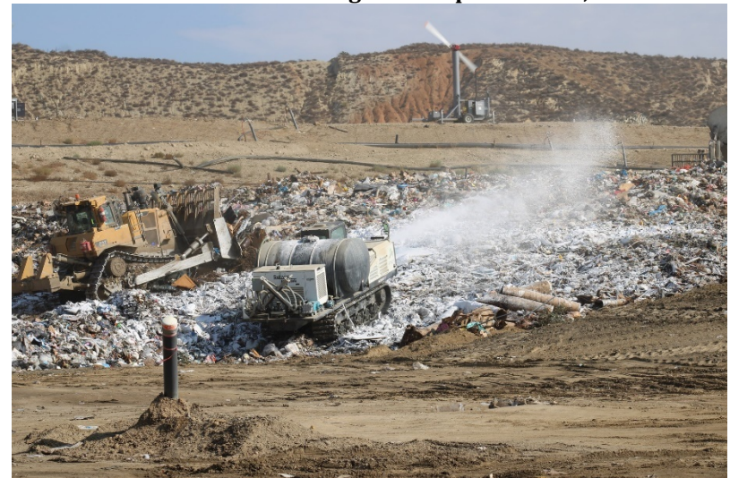
Photo 88: Cell 6 Working Area: September 13, 2022
