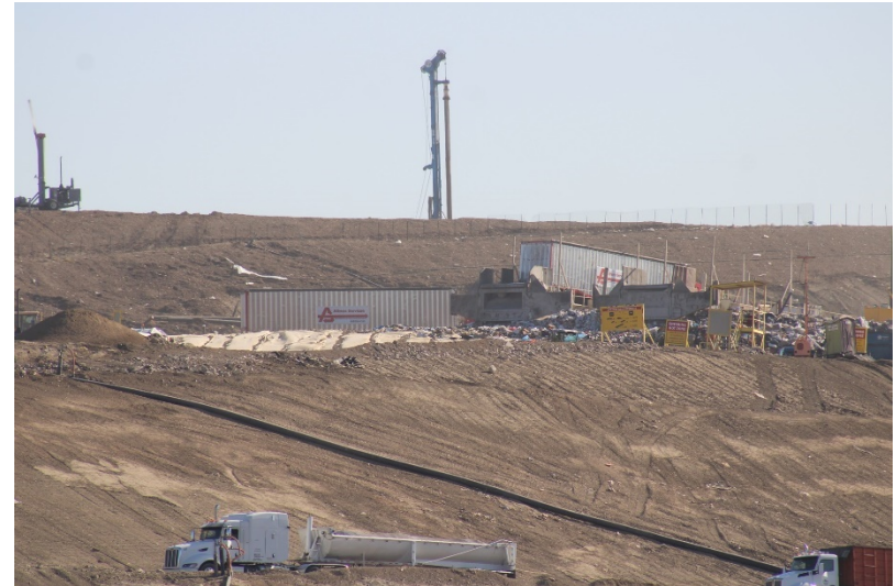
Photo 54: Cell 6 Working Area: August 23, 2022
