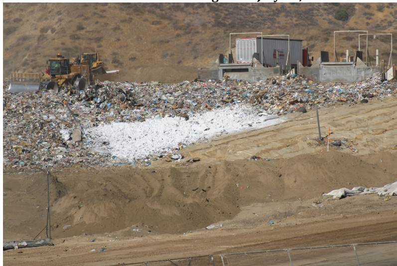
Photo 39: Cell 6 Working Area: July 21, 2022
