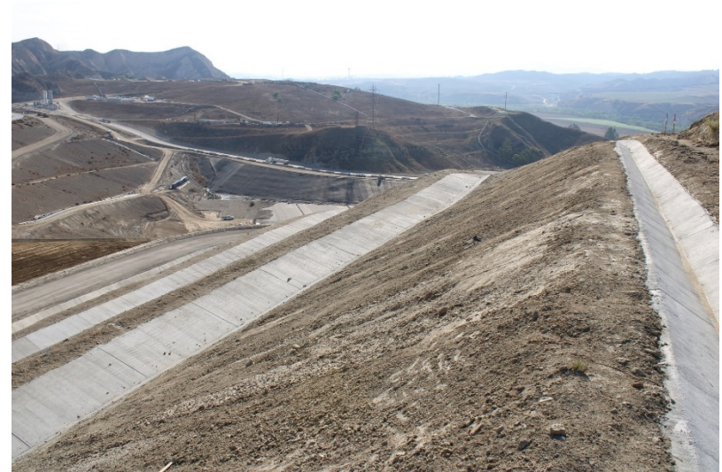
Photo 222: Landfill Perimeter Drainage Channel: September 13, 2022
