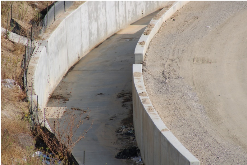
Photo 225: Landfill Perimeter Drainage Channel: September 13, 2022
