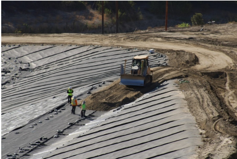
Photo 401: Cell 8 Construction: July 21, 2022
