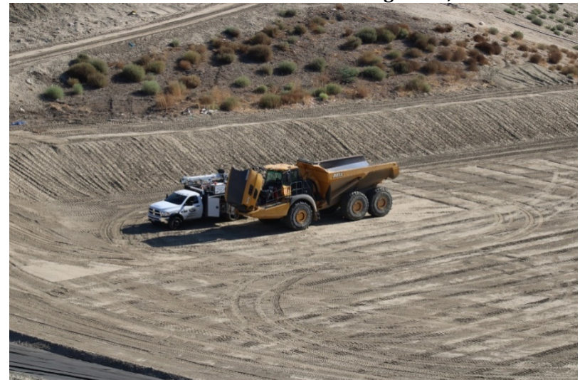
Photo 420: Cell 8 Construction: August 23, 2022
