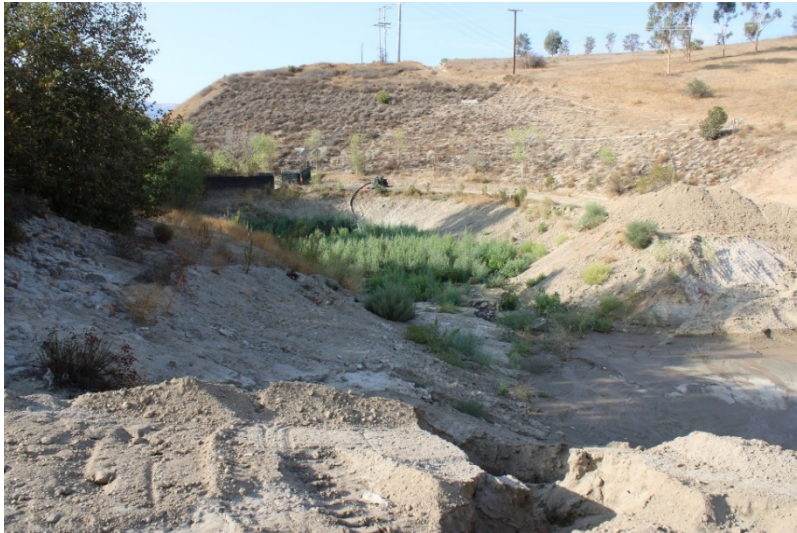
Photo 173: South Terminal and Catch Basins: September 13, 2022
