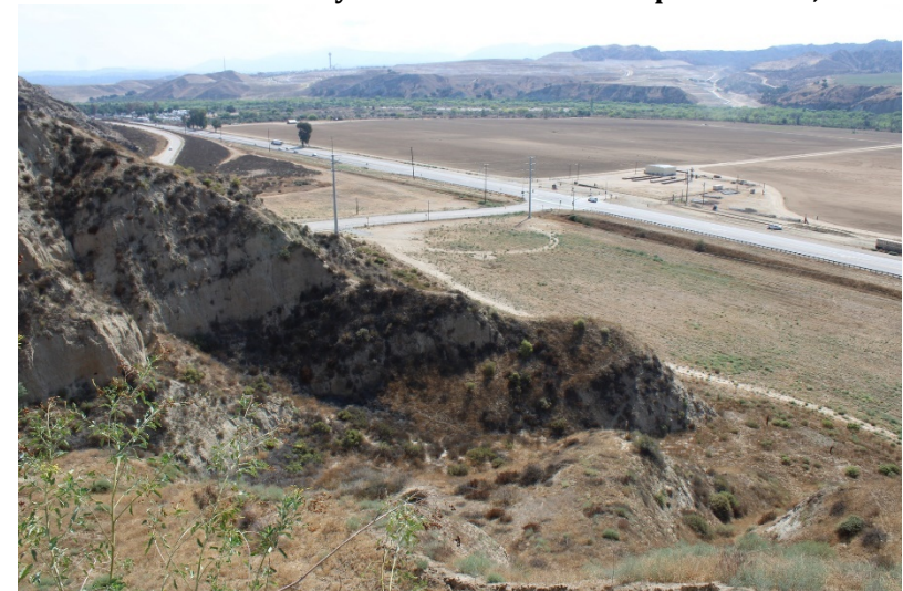
Photo 280: Wolcott Way Entrance Facilities: September 13, 2022
