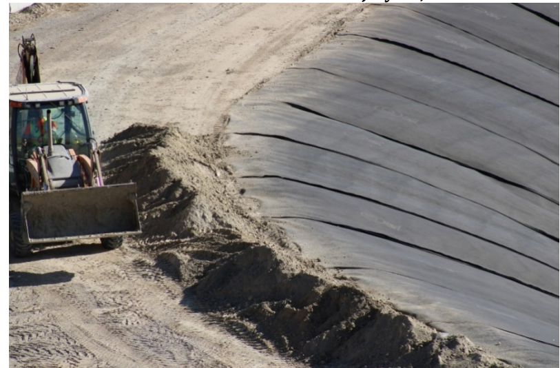
Photo 396: Cell 8 Construction: July 21, 2022
