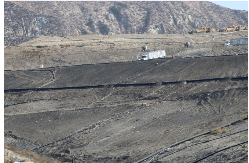
Photo 50: Cell 6 Working Area: August 23, 2022
