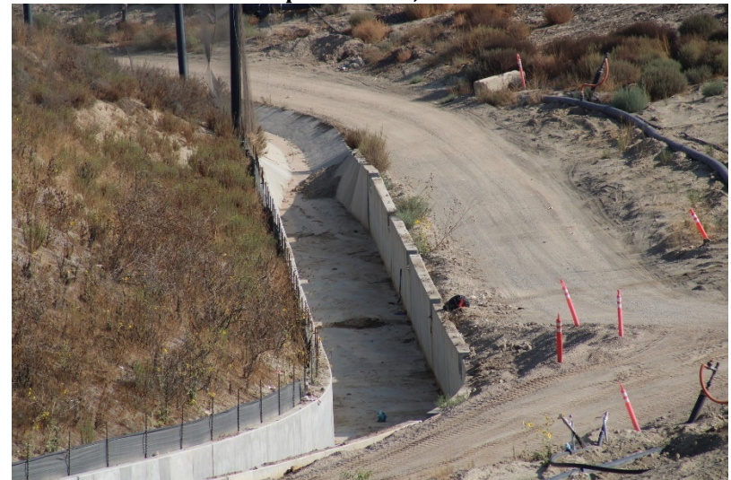
Photo 224: Landfill Perimeter Drainage Channel: September 13, 2022
