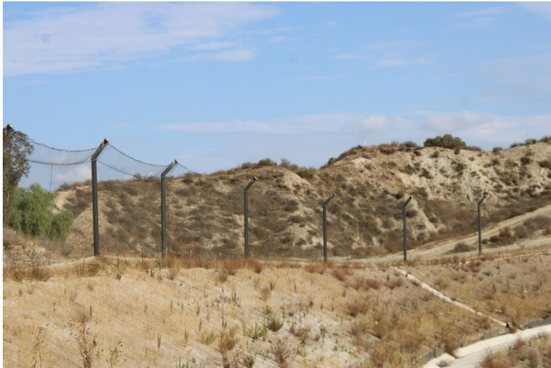
Photo 241: Westside Perimeter Ridge: September 13, 2022
