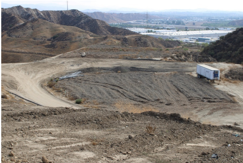
Photo 153: Future Cells 7, 9, and 10: September 13, 2022
