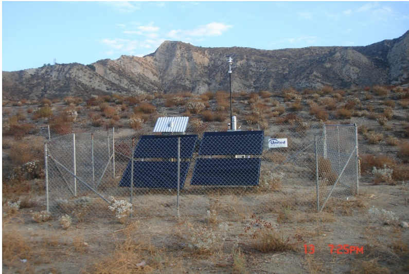
Photo 277: Wolcott Way Entrance Facilities: September 13, 2022
