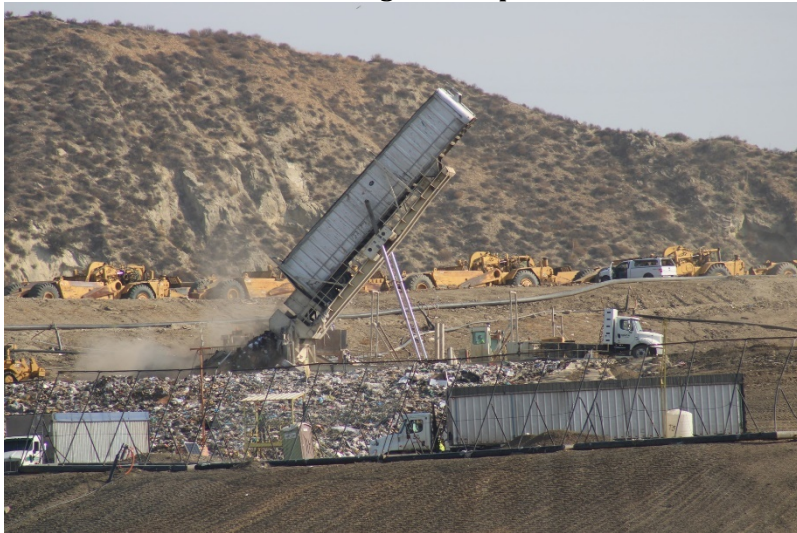
Photo 71: Cell 6 Working Area: September 13, 2022
