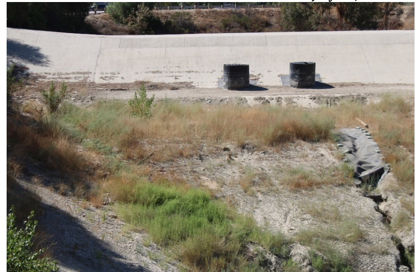
Photo 164: South Terminal and Catch Basins: August 23, 2022
