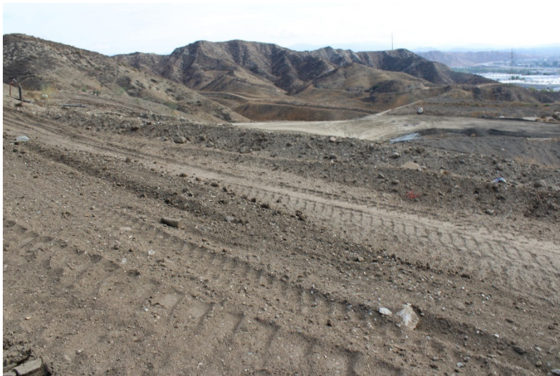
Photo 149: Future Cells 7, 9, and 10: September 13, 2022
