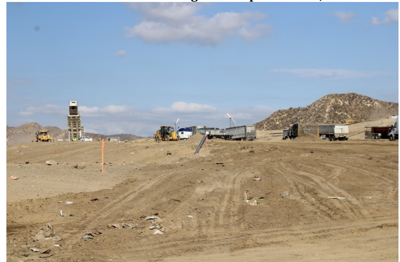
Photo 92: Cell 6 Working Area: September 13, 2022
