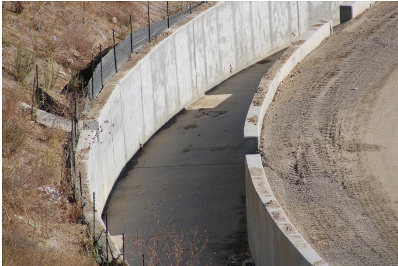
Photo 209: Landfill Perimeter Drainage Channel: August 23, 2022
