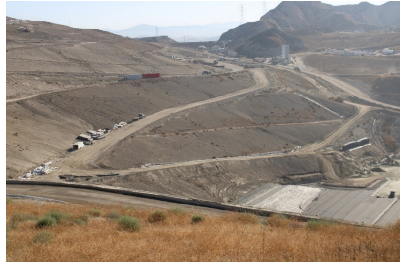
Photo 406: Cell 8 Construction: August 23, 2022
