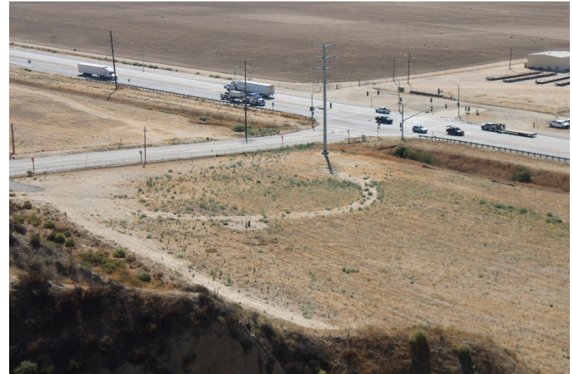
Photo 274: Wolcott Way Entrance Facilities: August 23, 2022
