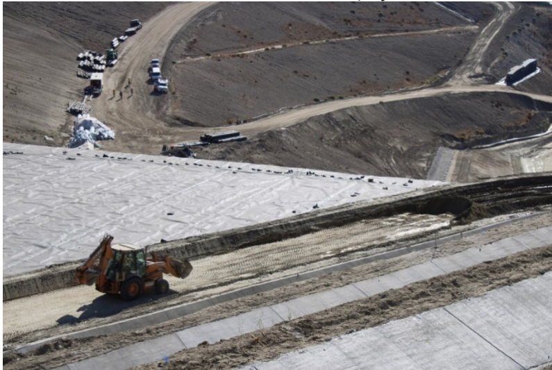
Photo 387: Cell 8 Construction: July 21, 2022
