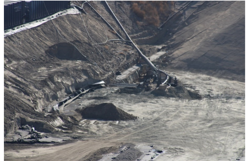
Photo 418: Cell 8 Construction: August 23, 2022
