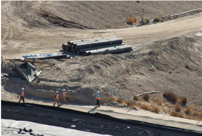
Photo 397: Cell 8 Construction: July 21, 2022
