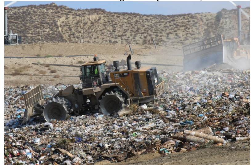
Photo 84: Cell 6 Working Area: September 13, 2022
