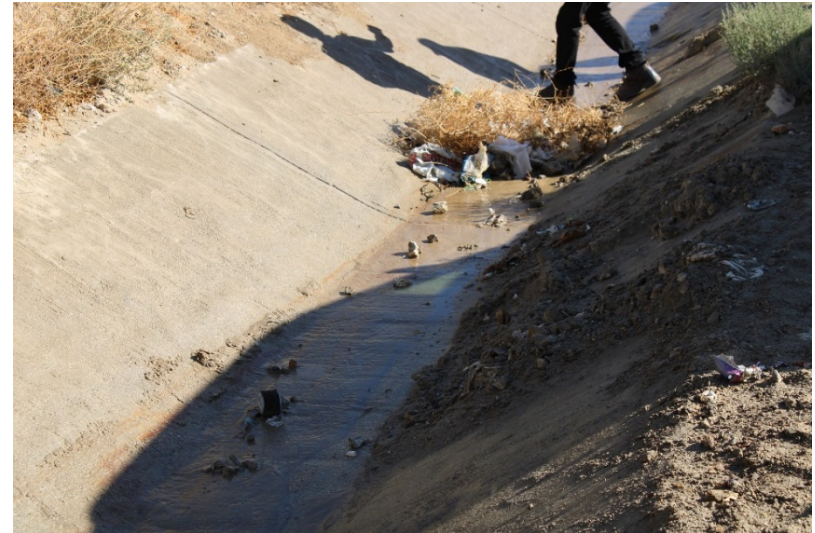
Photo 202: Landfill Perimeter Drainage Channel: July 21, 2022
