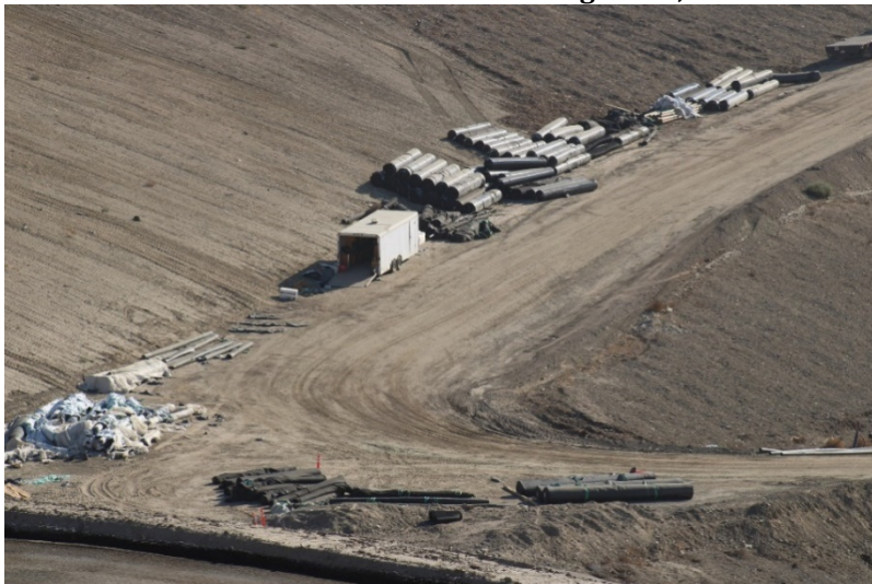
Photo 411: Cell 8 Construction: August 23, 2022
