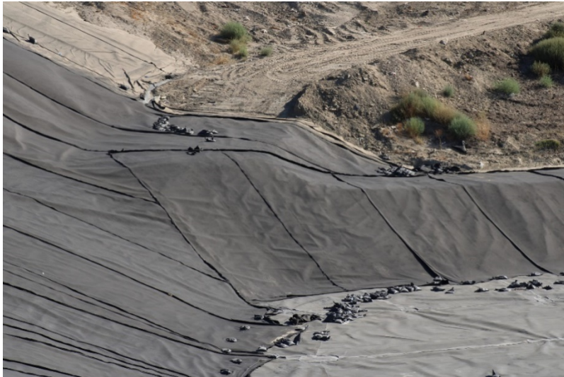
Photo 389: Cell 8 Construction: July 21, 2022
