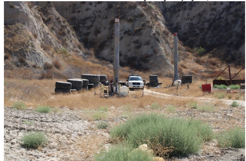
Photo 100: Closed Landfill - Primary Canyon: July 21, 2022
