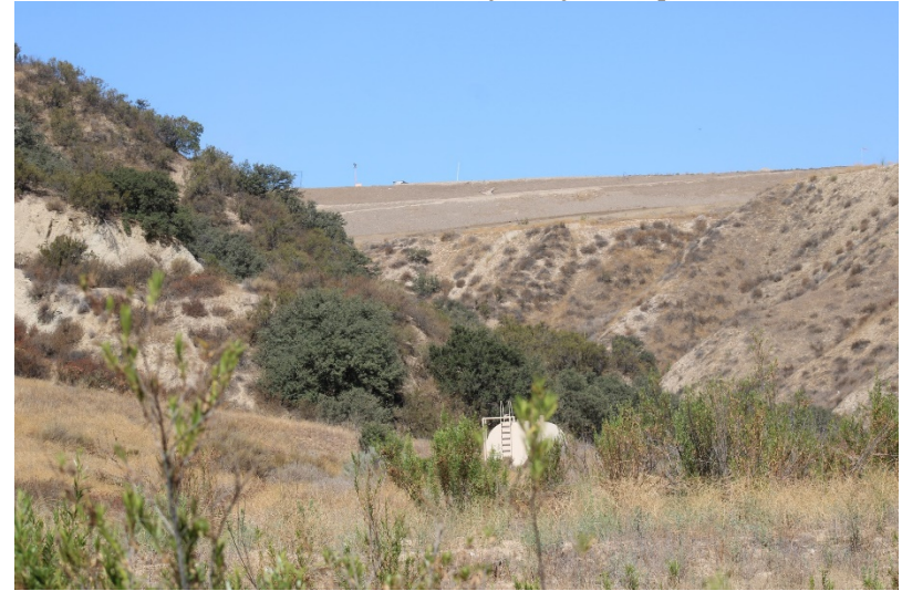
Photo 128: Closed Landfill - Canyon B: July 21, 2022
