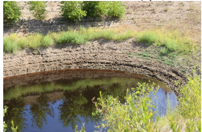
Photo 188: Northeast Sediment Basin: July 21, 2022
