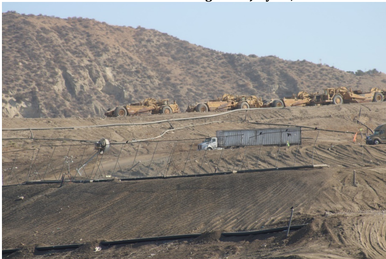
Photo 51: Cell 6 Working Area: August 23, 2022
