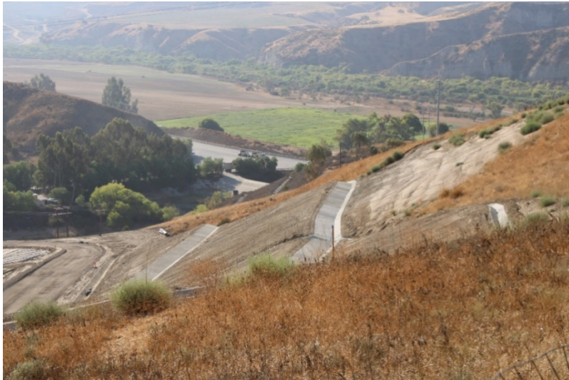
Photo 409: Cell 8 Construction: August 23, 2022
