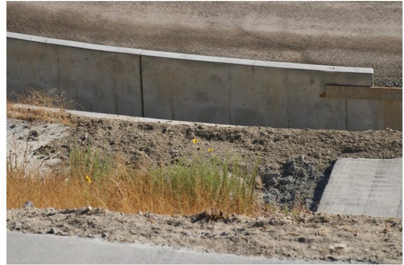
Photo 214: Landfill Perimeter Drainage Channel: August 23, 2022
