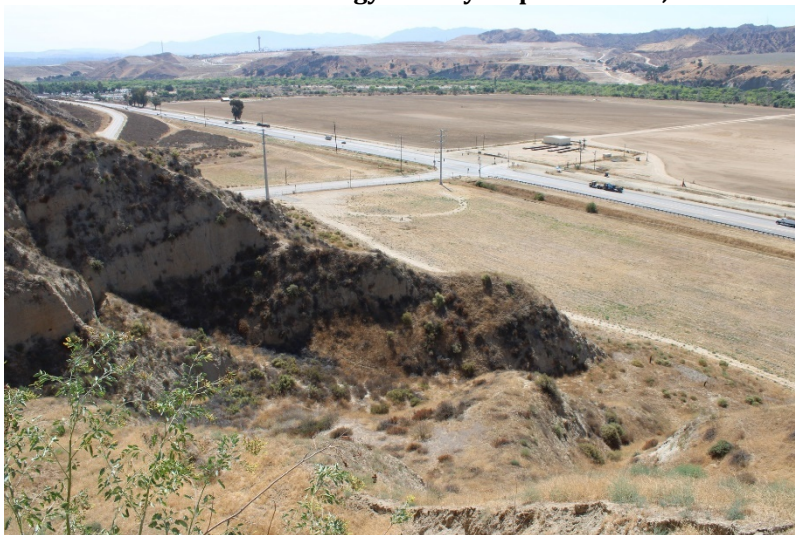
Photo 267: Wolcott Way Entrance Facilities: July 21, 2022
