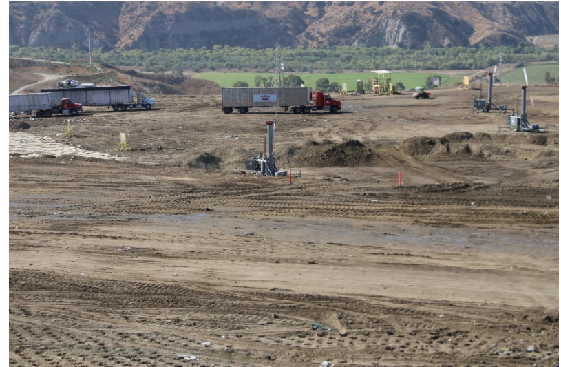
Photo 58: Cell 6 Working Area: August 23, 2022
