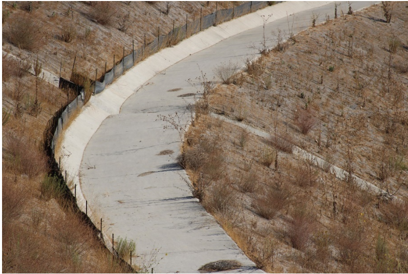
Photo 213: Landfill Perimeter Drainage Channel: August 23, 2022
