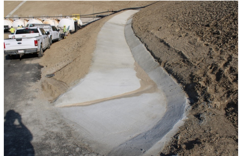
Photo 426: Cell 8 Construction: September 13, 2022
