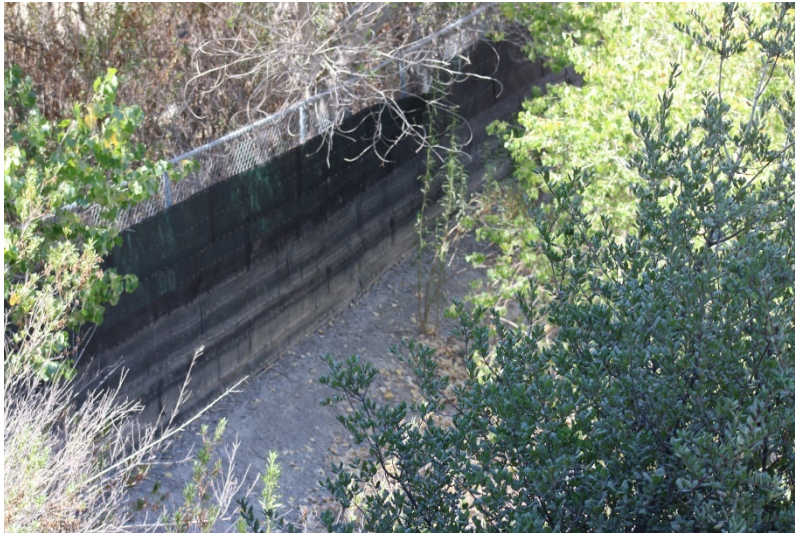
Photo 169: South Terminal and Catch Basins: August 23, 2022
