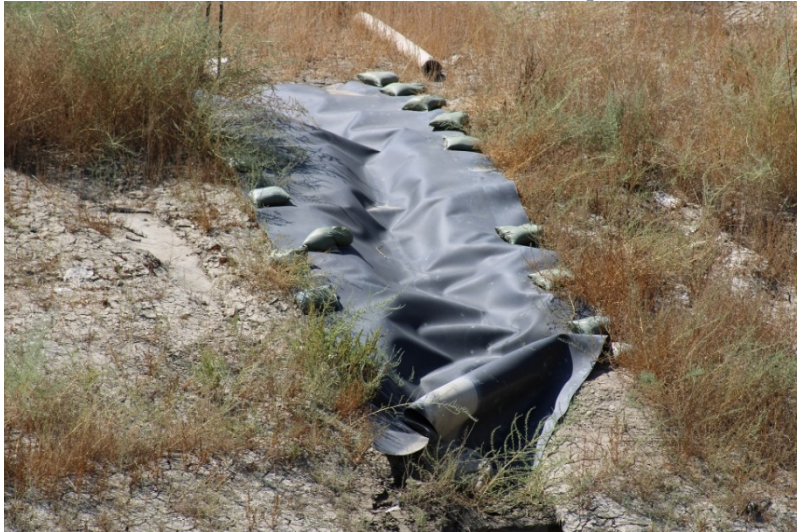
Photo 179: South Terminal and Catch Basins: September 13, 2022
