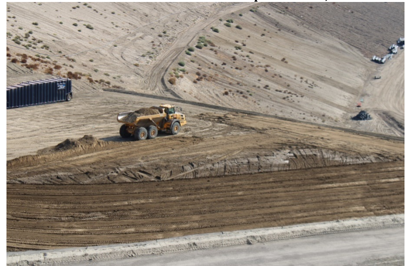
Photo 428: Cell 8 Construction: September 13, 2022
