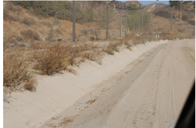
Photo 216: Landfill Perimeter Drainage Channel: August 23, 2022
