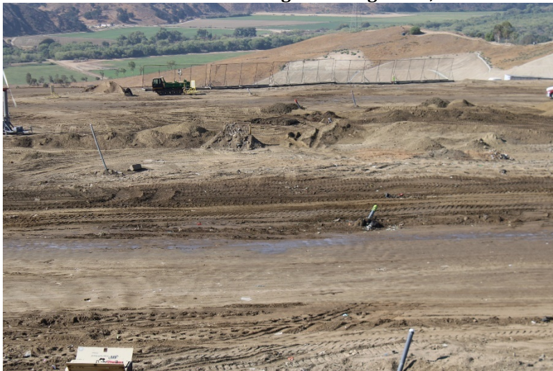
Photo 59: Cell 6 Working Area: August 23, 2022
