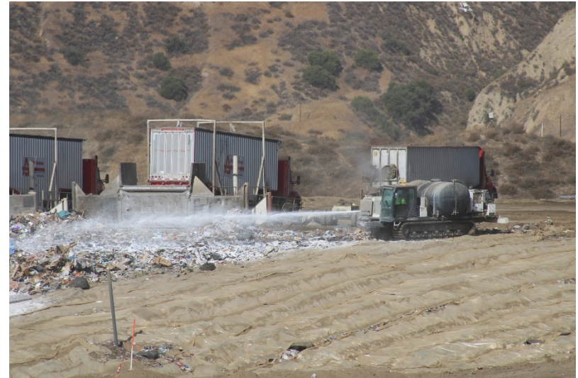
Photo 42: Cell 6 Working Area: July 21, 2022
