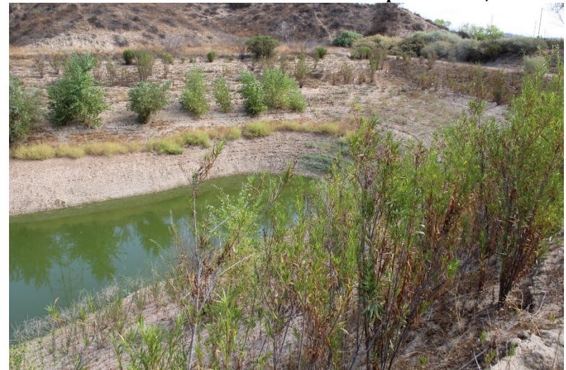
Photo 196: Northeast Sediment Basin: September 13, 2022
