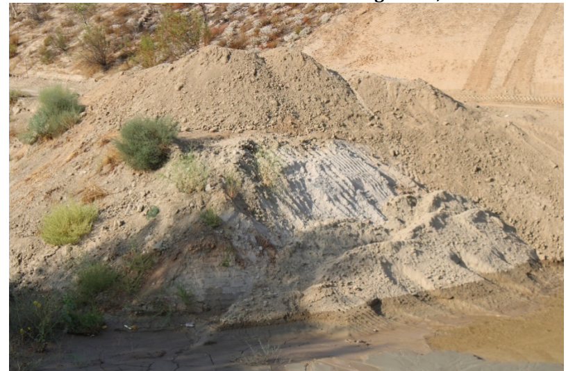
Photo 424: Cell 8 Construction: September 13, 2022
