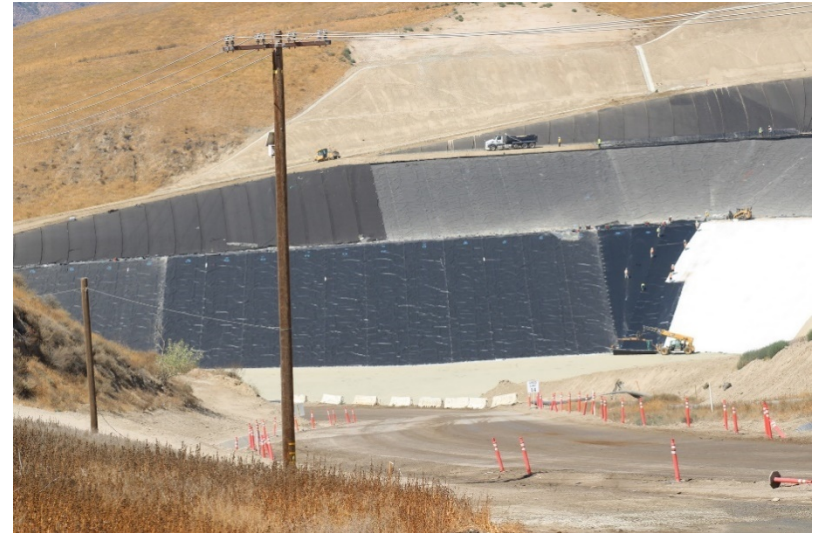
Photo 402: Cell 8 Construction: July 21, 2022
