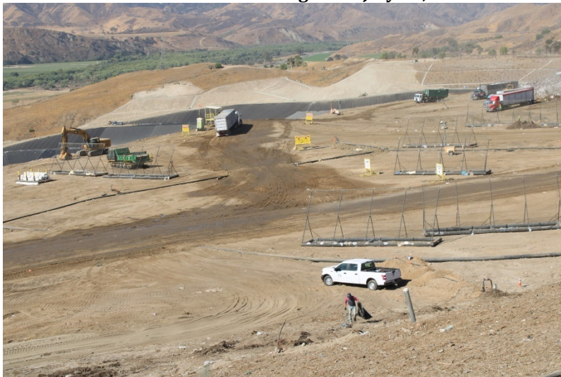
Photo 31: Cell 6 Working Area: July 21, 2022
