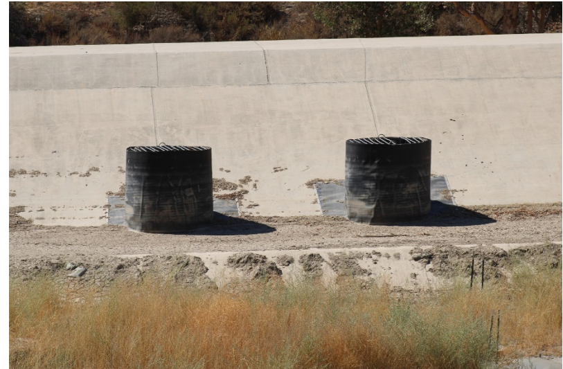
Photo 166: South Terminal and Catch Basins: August 23, 2022
