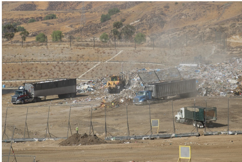
Photo 37: Cell 6 Working Area: July 21, 2022
