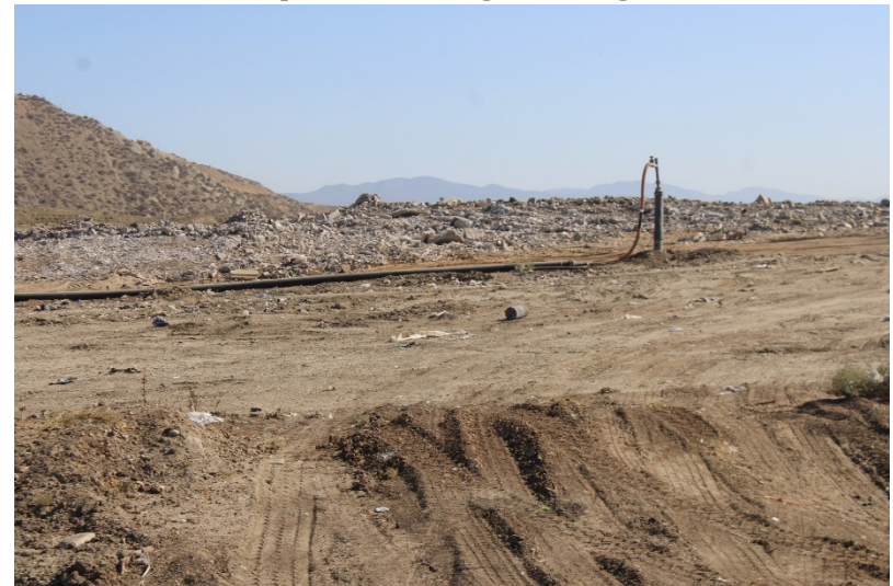
Photo 16: Top Deck Working Area: August 23, 2022
