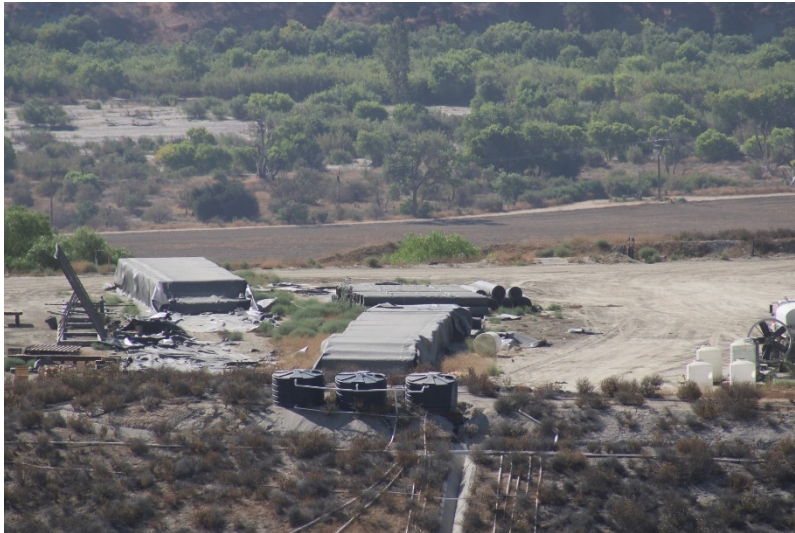
Photo 97: Closed Landfill - Primary Canyon: July 21, 2022
