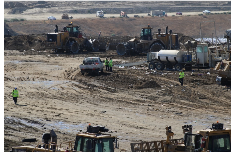
Photo 62: Cell 6 Working Area: August 23, 2022
