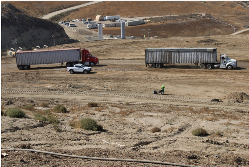
Photo 29: Cell 6 Working Area: July 21, 2022
