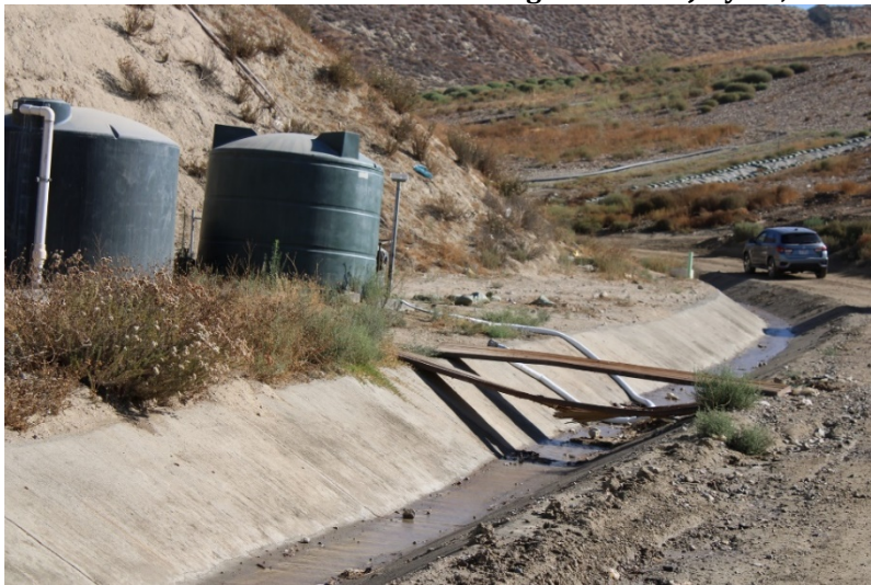
Photo 203: Landfill Perimeter Drainage Channel: July 21, 2022
