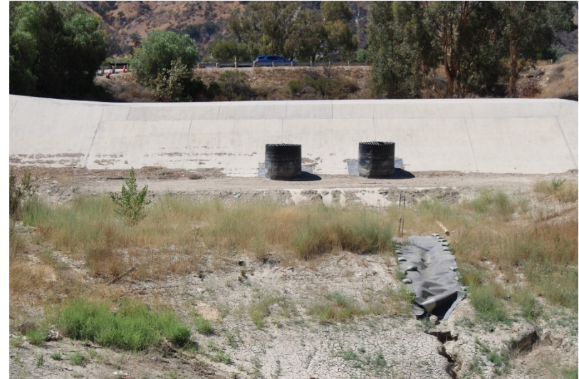
Photo 158: South Terminal and Catch Basins: July 21, 2022
