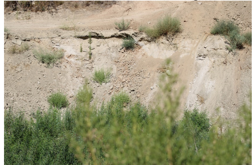
Photo 172: South Terminal and Catch Basins: August 23, 2022
