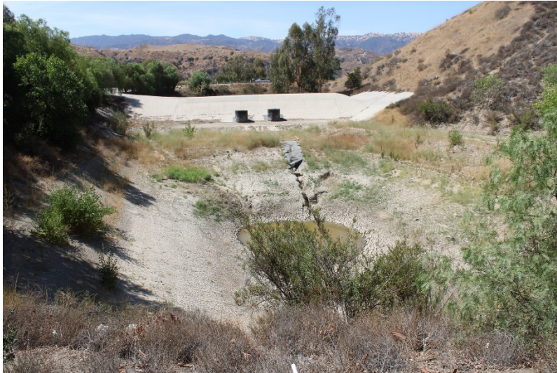
Photo 157: South Terminal and Catch Basins: July 21, 2022
