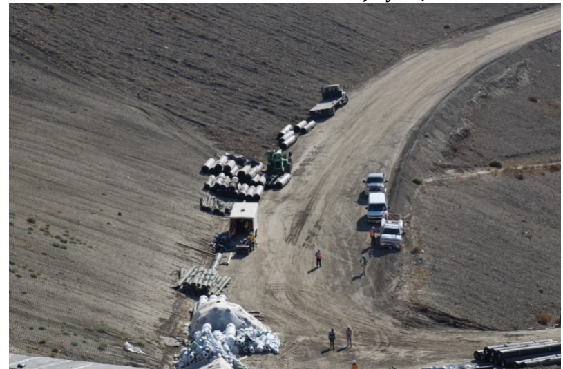
Photo 392: Cell 8 Construction: July 21, 2022
