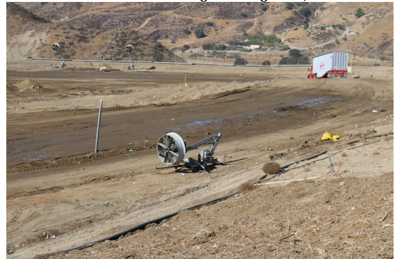
Photo 60: Cell 6 Working Area: August 23, 2022
