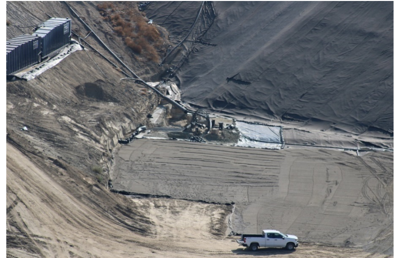
Photo 434: Cell 8 Construction: September 13, 2022
