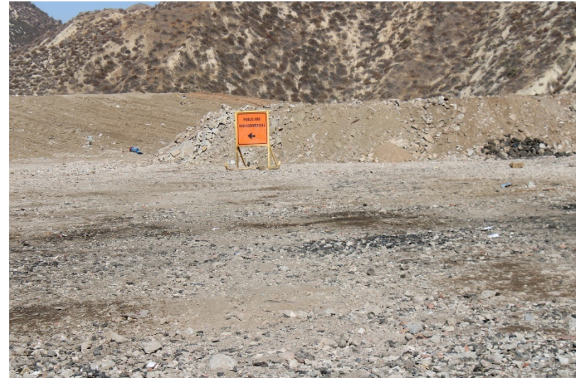
Photo 10: Top Deck Working Area: August 23, 2022
