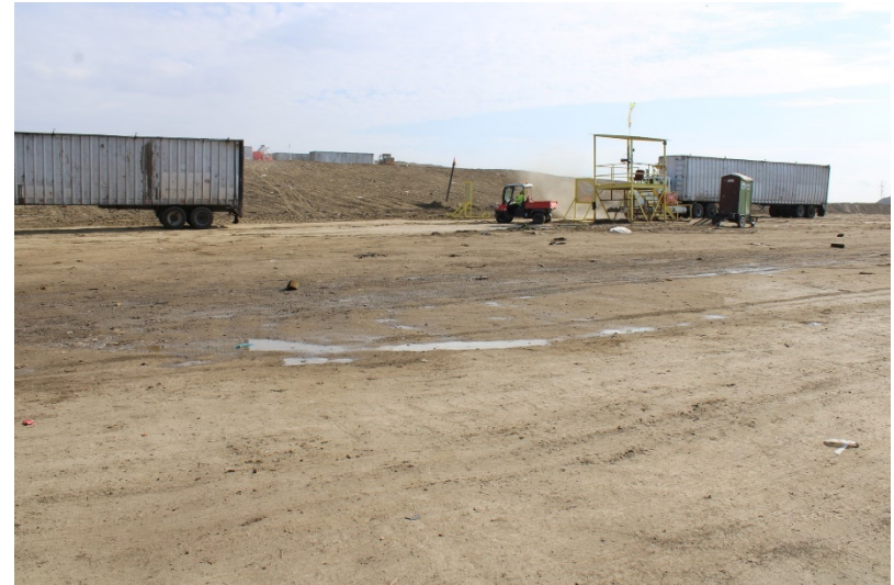
Photo 78: Cell 6 Working Area: September 13, 2022
