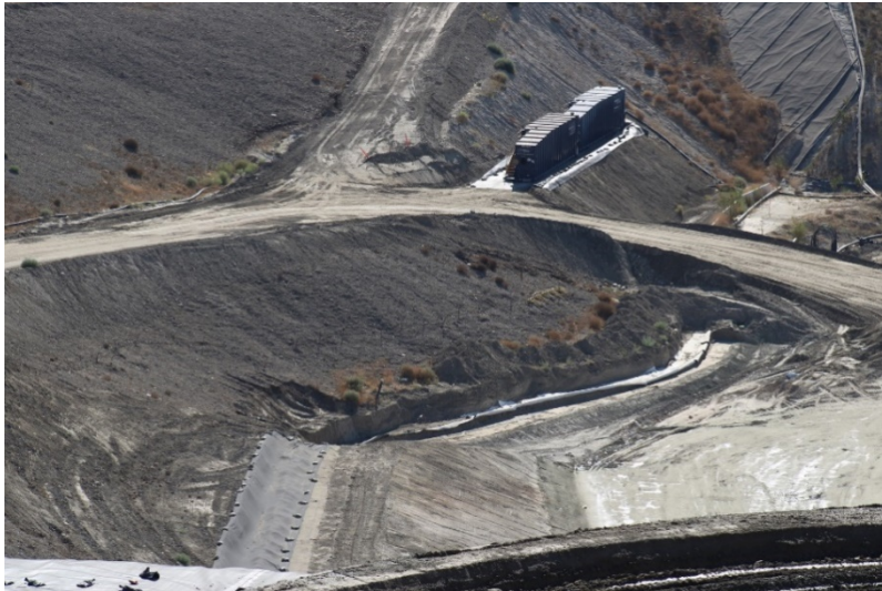
Photo 393: Cell 8 Construction: July 21, 2022
