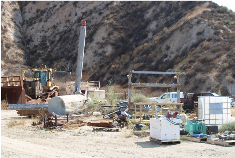
Photo 125: Closed Landfill - Primary Canyon: September 13, 2022
