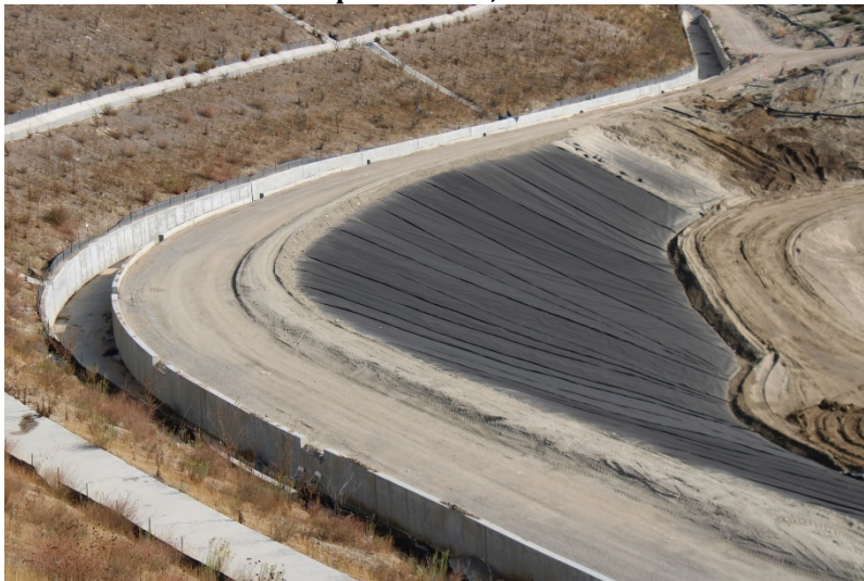
Photo 223: Landfill Perimeter Drainage Channel: September 13, 2022
