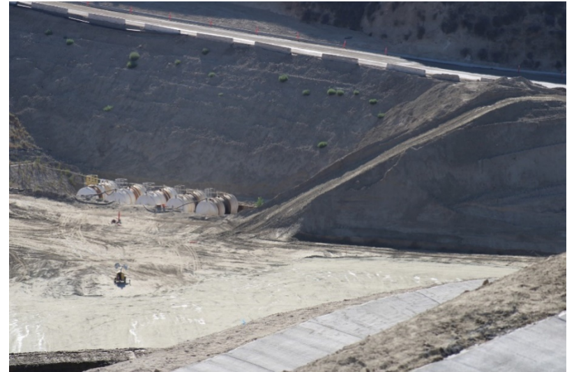
Photo 394: Cell 8 Construction: July 21, 2022
