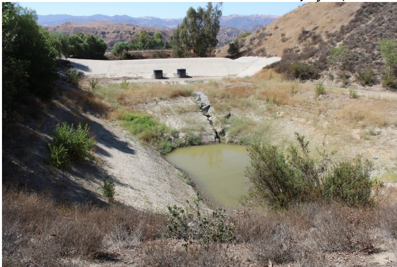
Photo 163: South Terminal and Catch Basins: August 23, 2022
