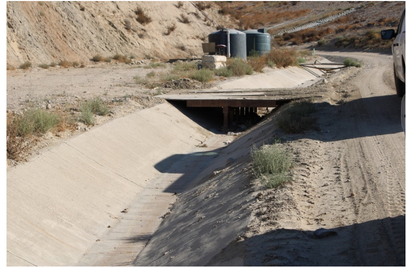
Photo 218: Landfill Perimeter Drainage Channel: August 23, 2022
