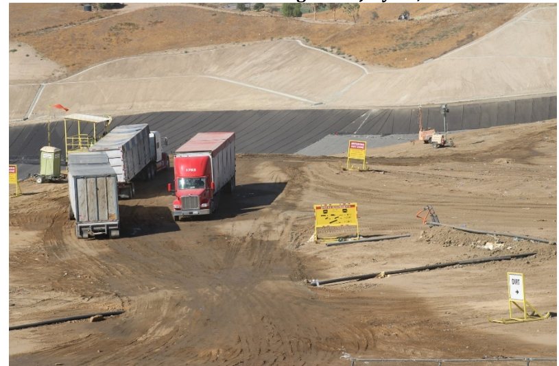
Photo 36: Cell 6 Working Area: July 21, 2022
