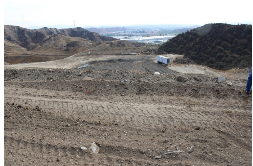
Photo 150: Future Cells 7, 9, and 10: September 13, 2022
