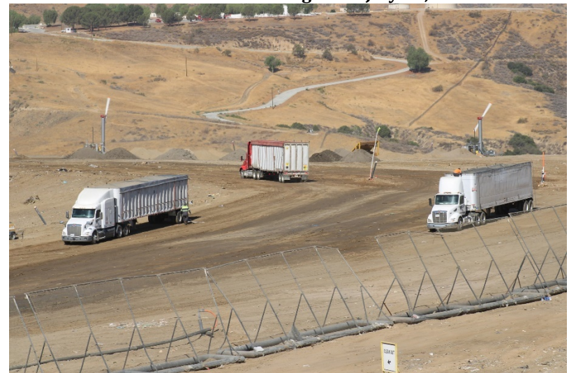
Photo 40: Cell 6 Working Area: July 21, 2022
