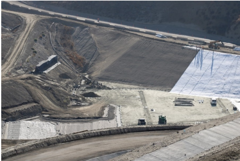
Photo 421: Cell 8 Construction: August 23, 2022
