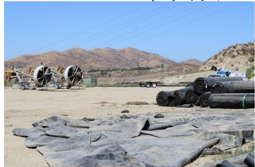
Photo 108: Closed Landfill - Primary Canyon: July 21, 2022
