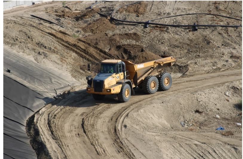
Photo 74: Cell 6 Working Area: September 13, 2022
