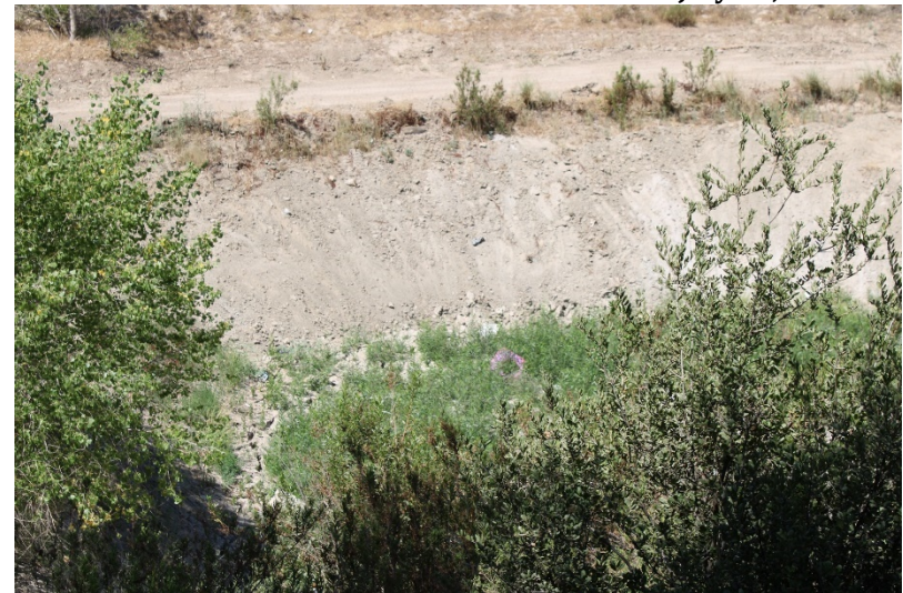
Photo 160: South Terminal and Catch Basins: July 21, 2022
