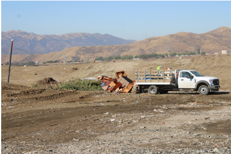
Photo 9: Top Deck Working Area: August 23, 2022
