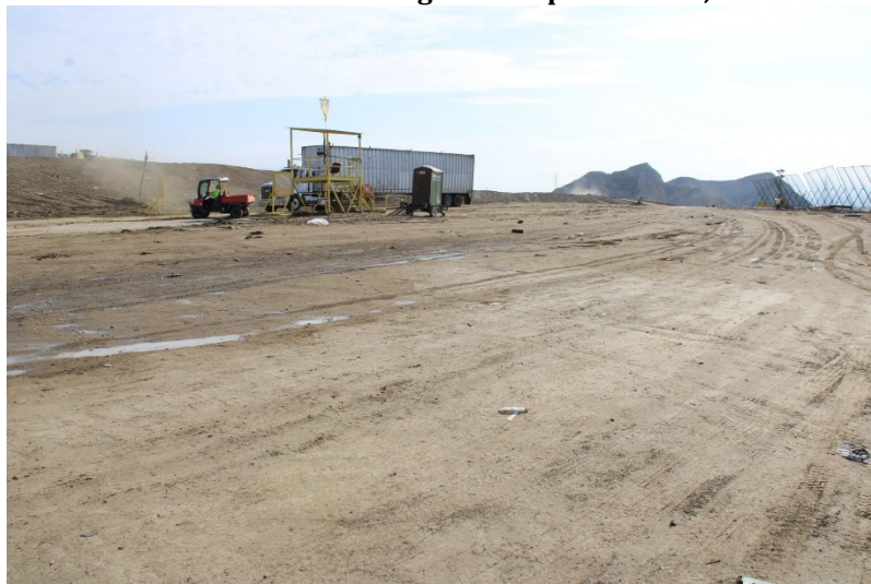
Photo 79: Cell 6 Working Area: September 13, 2022
