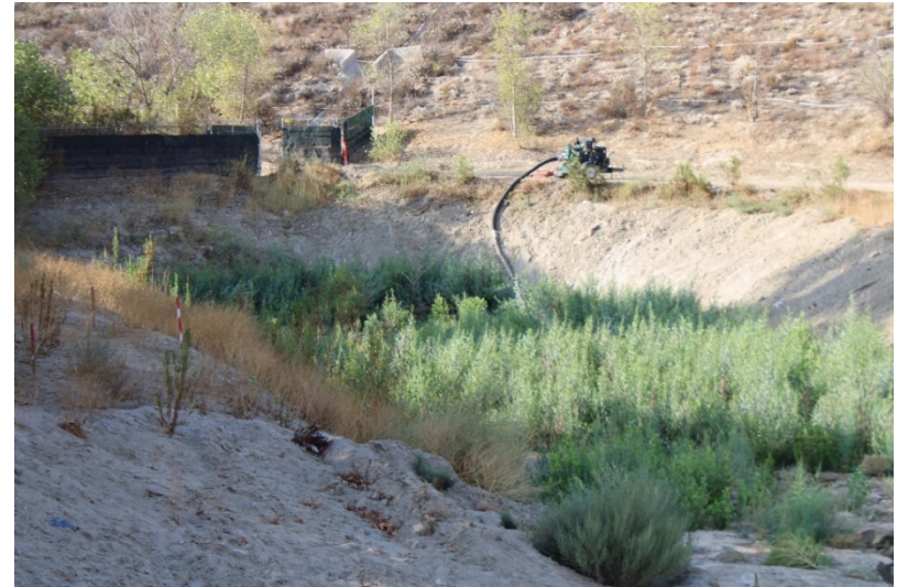
Photo 174: South Terminal and Catch Basins: September 13, 2022
