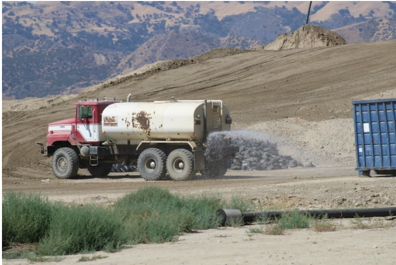
Photo 109: Closed Landfill - Primary Canyon: July 21, 2022
