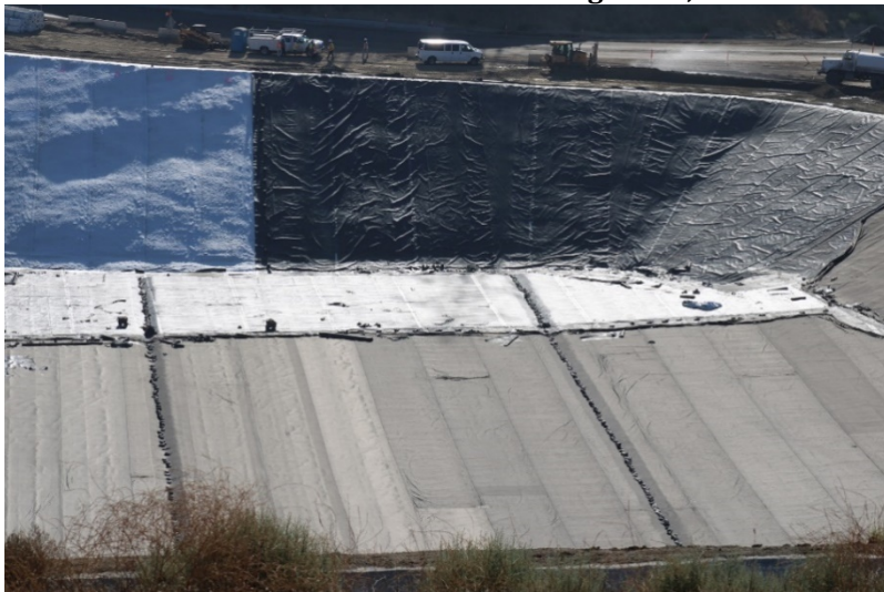
Photo 415: Cell 8 Construction: August 23, 2022
