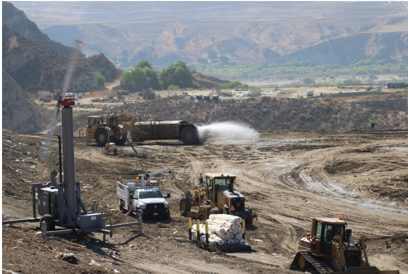
Photo 61: Cell 6 Working Area: August 23, 2022
