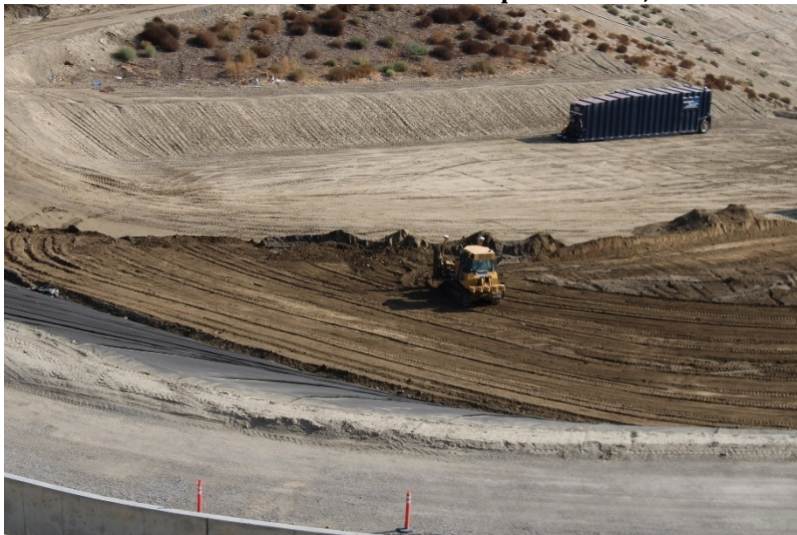
Photo 427: Cell 8 Construction: September 13, 2022
