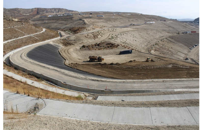
Photo 220: Landfill Perimeter Drainage Channel: September 13, 2022
