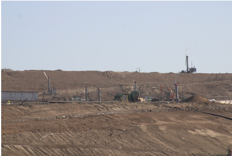
Photo 53: Cell 6 Working Area: August 23, 2022
