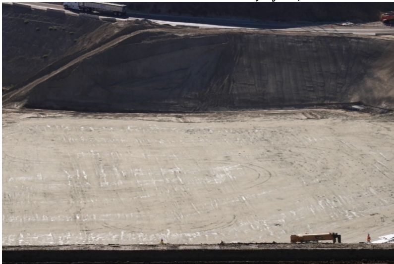
Photo 399: Cell 8 Construction: July 21, 2022
