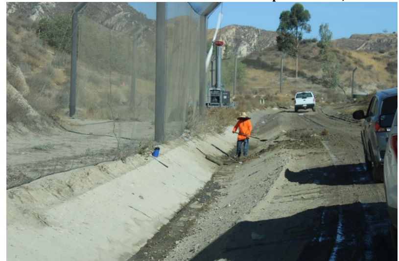
Photo 200: Landfill Perimeter Drainage Channel: July 21, 2022
