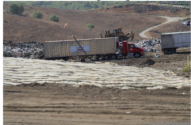
Photo 64: Cell 6 Working Area: August 23, 2022
