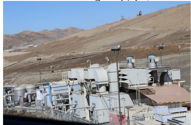
Photo 264: Gas-to-Energy Facility: July 21, 2022
