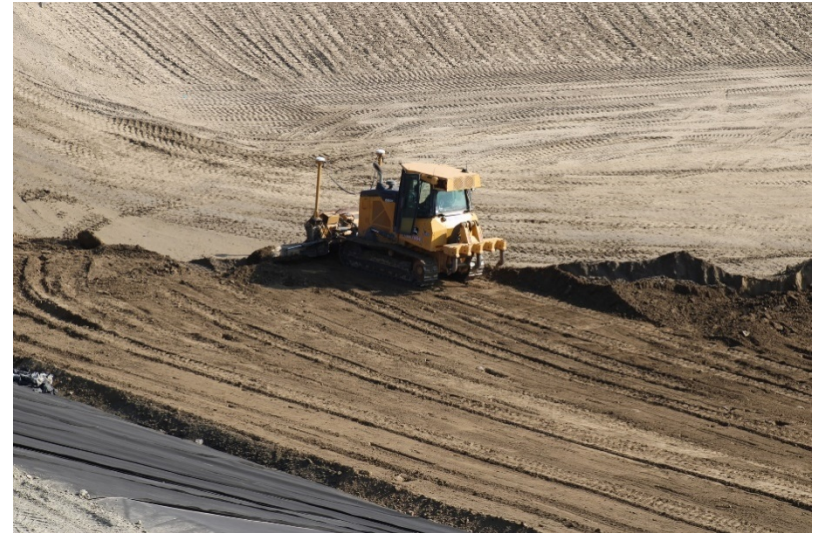
Photo 430: Cell 8 Construction: September 13, 2022
