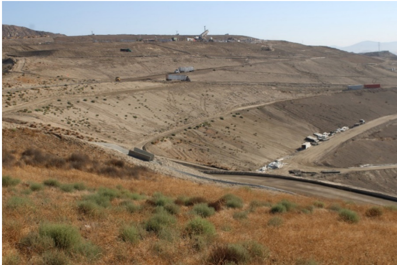
Photo 405: Cell 8 Construction: August 23, 2022
