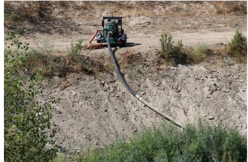
Photo 182: South Terminal and Catch Basins: September 13, 2022
