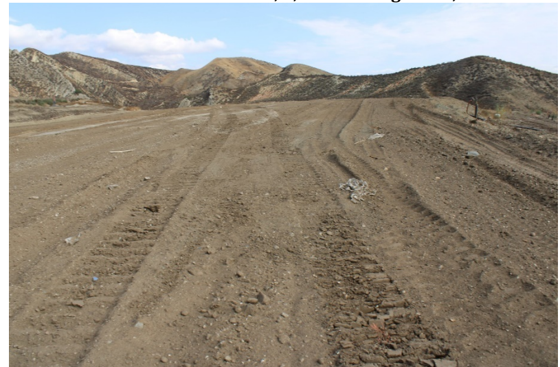
Photo 148: Future Cells 7, 9, and 10: September 13, 2022
