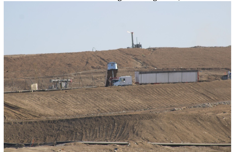
Photo 52: Cell 6 Working Area: August 23, 2022
