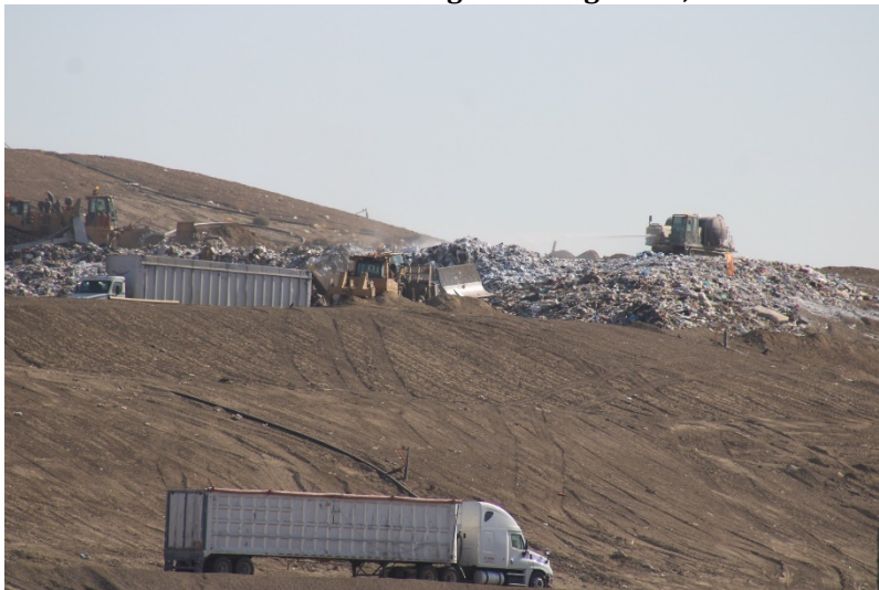
Photo 55: Cell 6 Working Area: August 23, 2022
