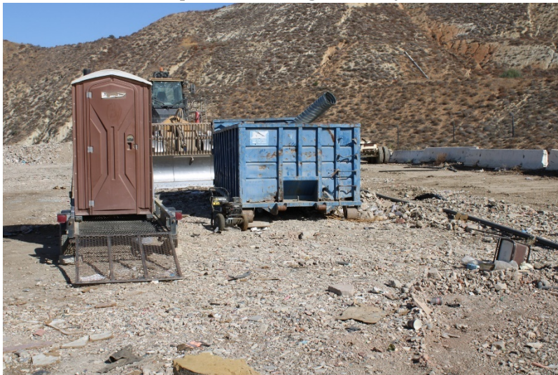
Photo 3: Top Deck Working Area: July 21, 2022
