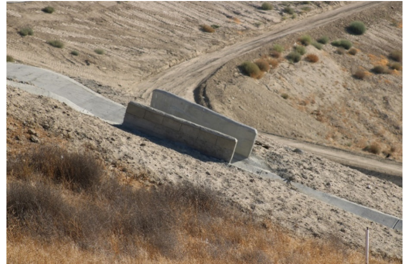
Photo 410: Cell 8 Construction: August 23, 2022
