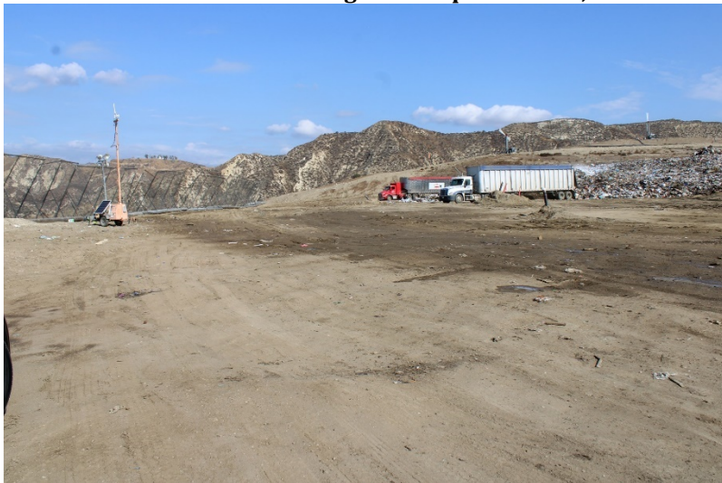
Photo 75: Cell 6 Working Area: September 13, 2022
