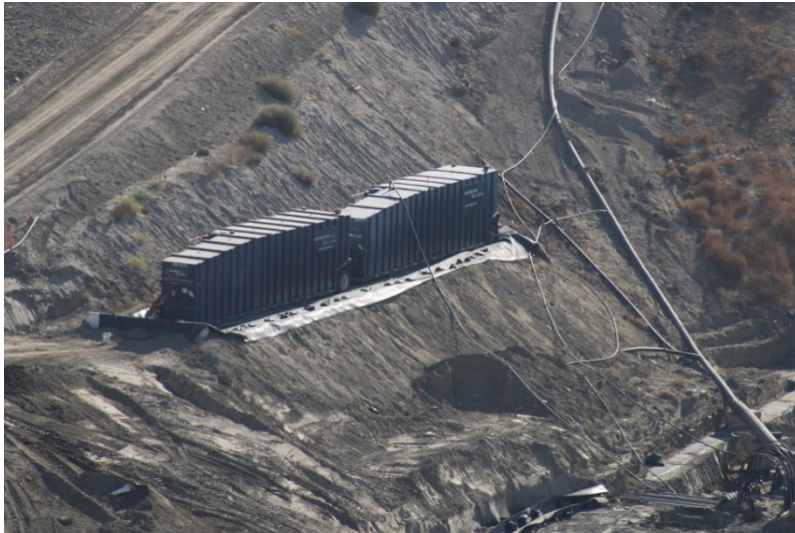
Photo 417: Cell 8 Construction: August 23, 2022
