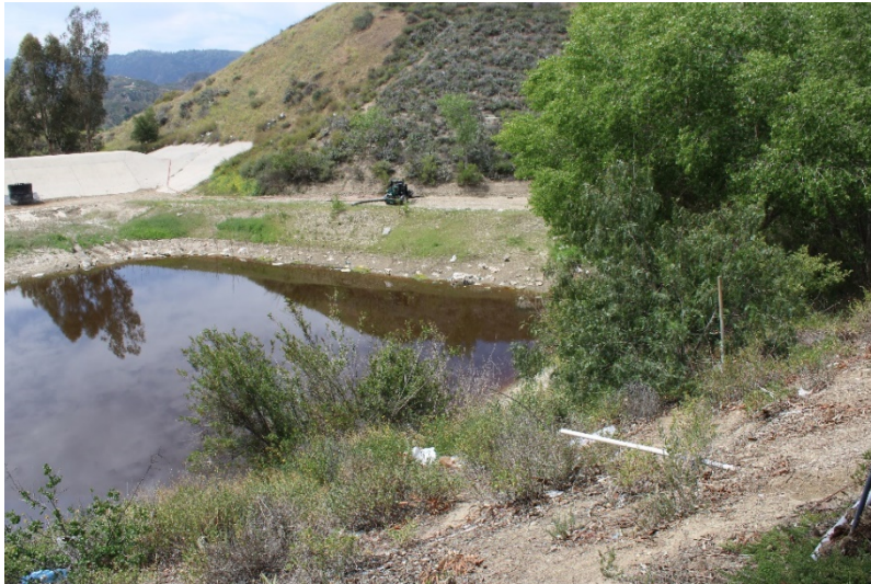
Photo 169: South Terminal and Catch Basins: April 26, 2022
