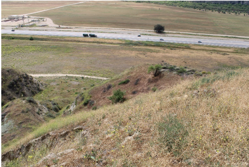
Photo 265: Wolcott Way Entrance Facilities: April 26, 2022
