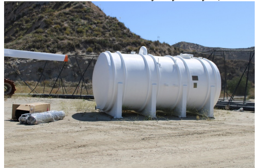
Photo 132: Closed Landfill - Primary Canyon: May 24, 2022
