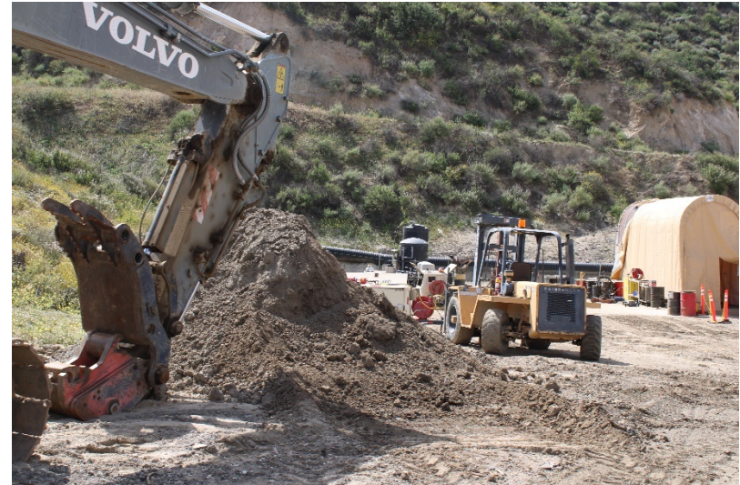
Photo 286: Maintenance and Admin Buildings: April 26, 2022
