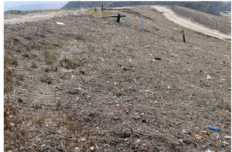
Photo 12: Top Deck Working Area: May 24, 2022
