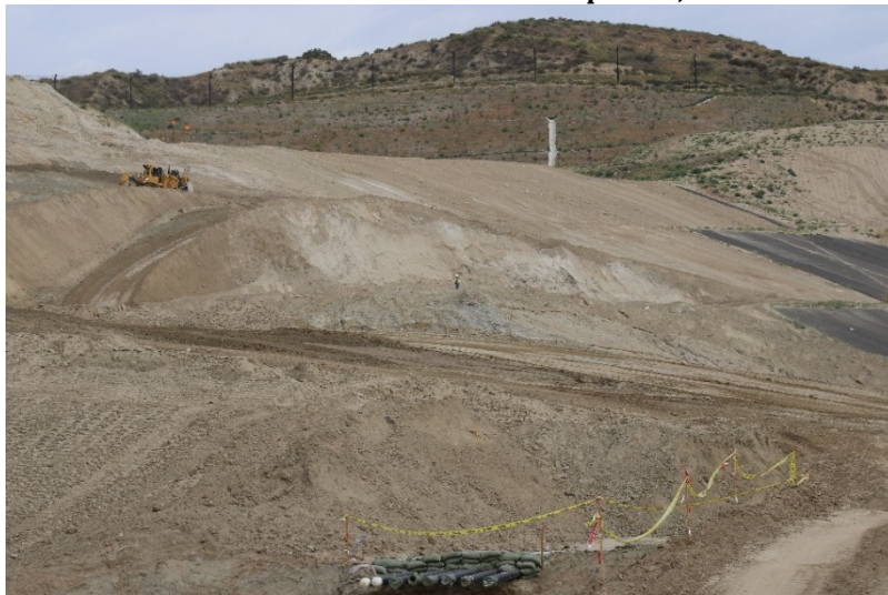
Photo 407: Cell 8 Construction: April 26, 2022
