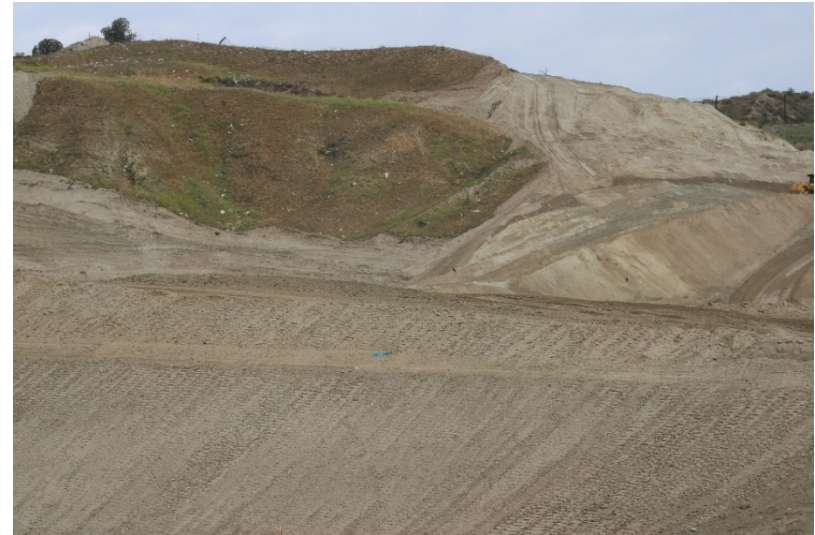
Photo 406: Cell 8 Construction: April 26, 2022
