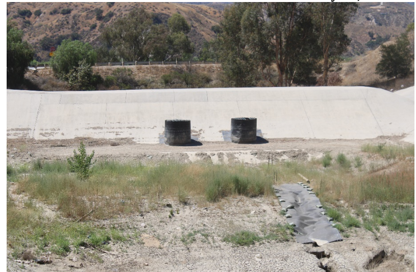
Photo 188: South Terminal and Catch Basins: June 21, 2022
