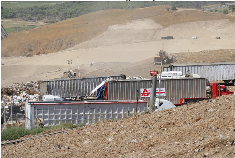
Photo 111: Cell 6 Working Area: June 21, 2022
