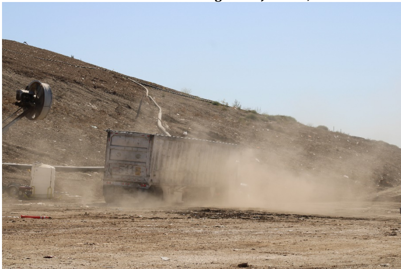
Photo 103: Cell 6 Working Area: June 21, 2022
