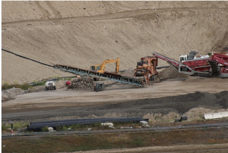
Photo 421: Cell 8 Construction: April 26, 2022
