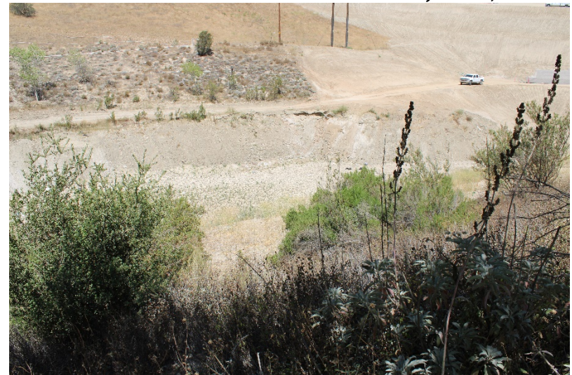
Photo 192: South Terminal and Catch Basins: June 21, 2022
