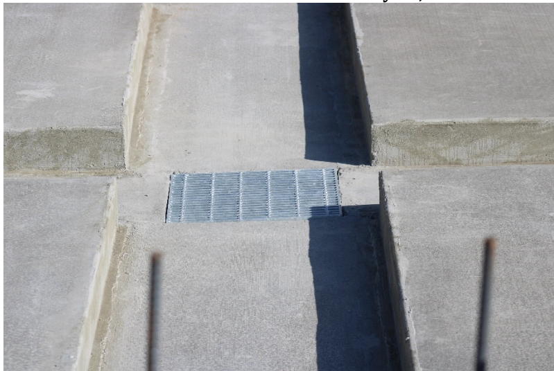
Photo 443: Cell 8 Construction: May 24, 2022
