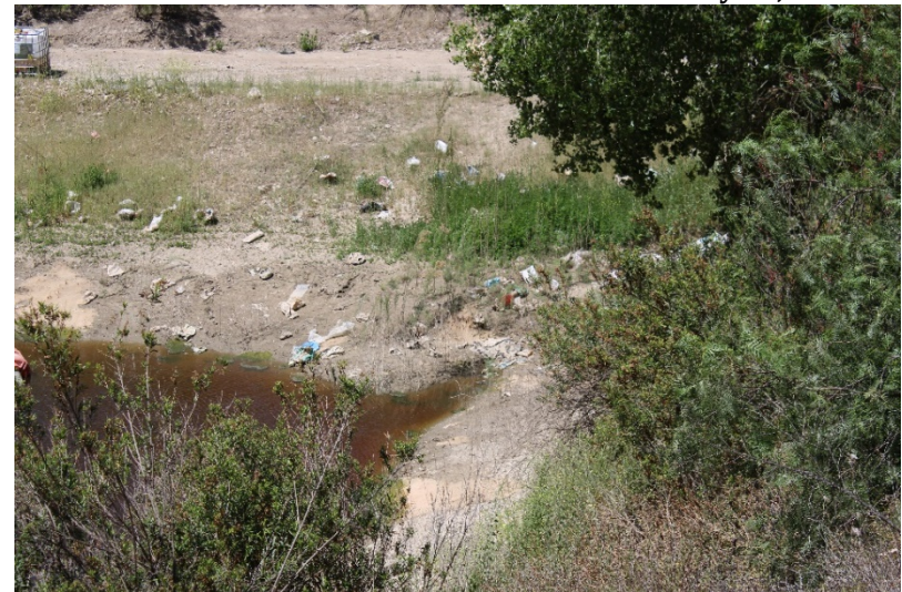
Photo 184: South Terminal and Catch Basins: May 24, 2022
