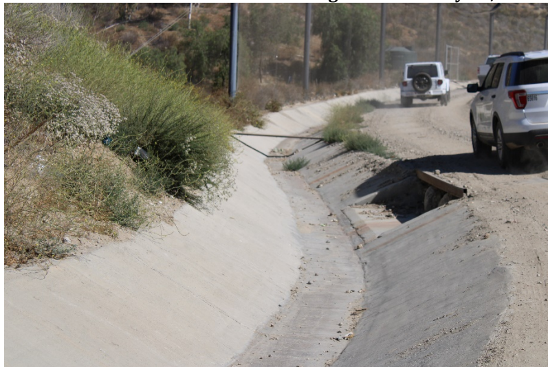
Photo 227: Landfill Perimeter Drainage Channel: May 24, 2022
