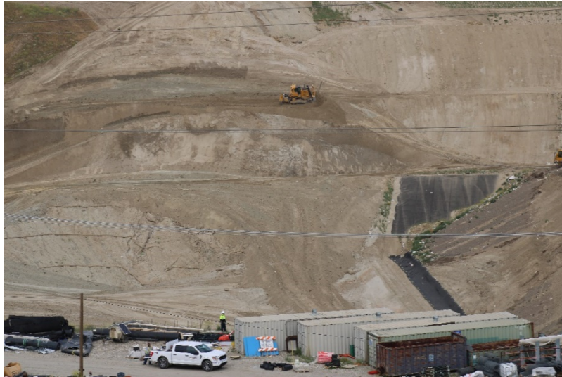
Photo 417: Cell 8 Construction: April 26, 2022
