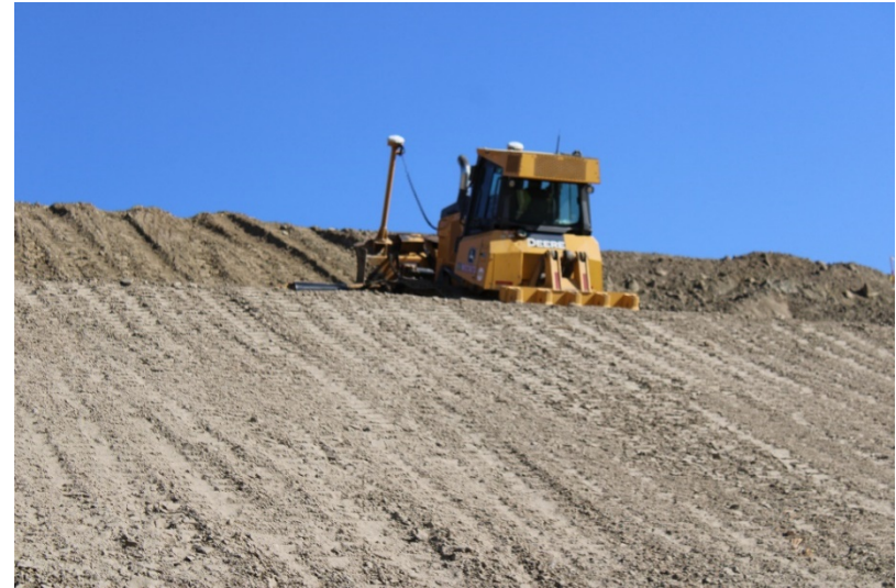
Photo 438: Cell 8 Construction: May 24, 2022
