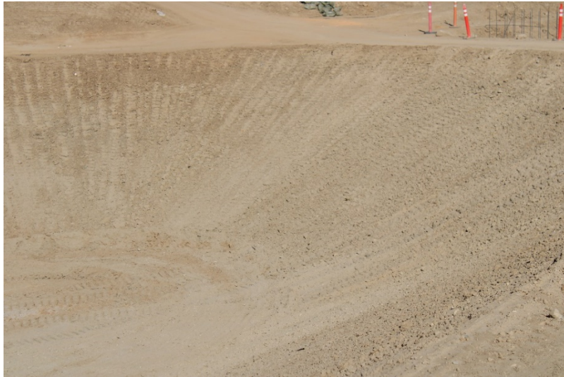
Photo 429: Cell 8 Construction: May 24, 2022
