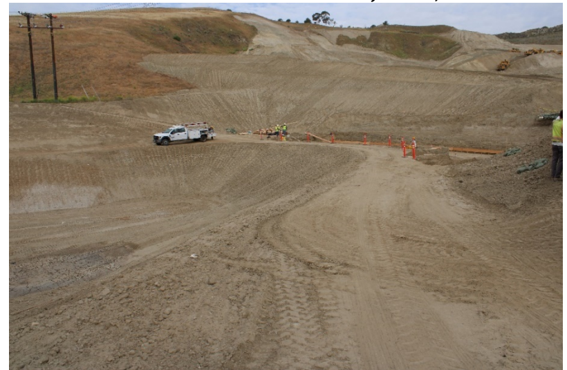
Photo 400: Cell 8 Construction: April 26, 2022
