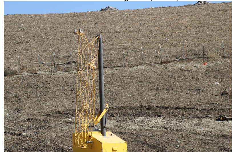
Photo 108: Cell 6 Working Area: June 21, 2022
