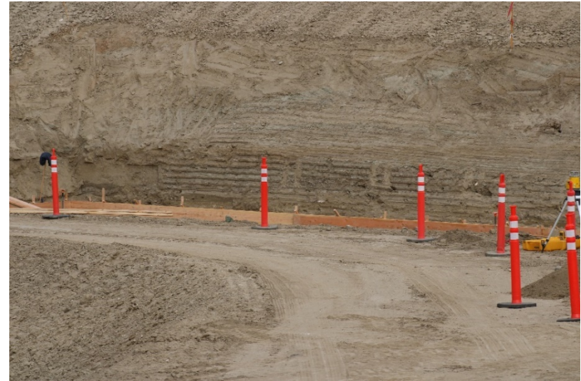
Photo 402: Cell 8 Construction: April 26, 2022
