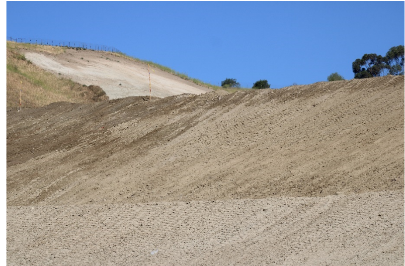
Photo 446: Cell 8 Construction: May 24, 2022
