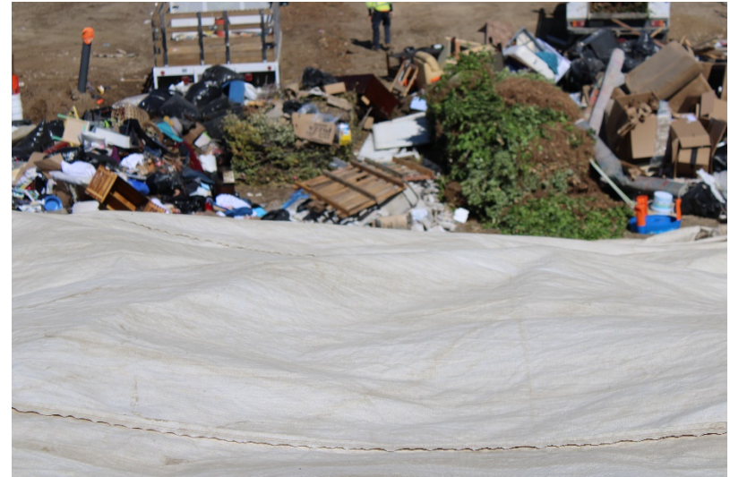
Photo 10: Top Deck Working Area: May 24, 2022
