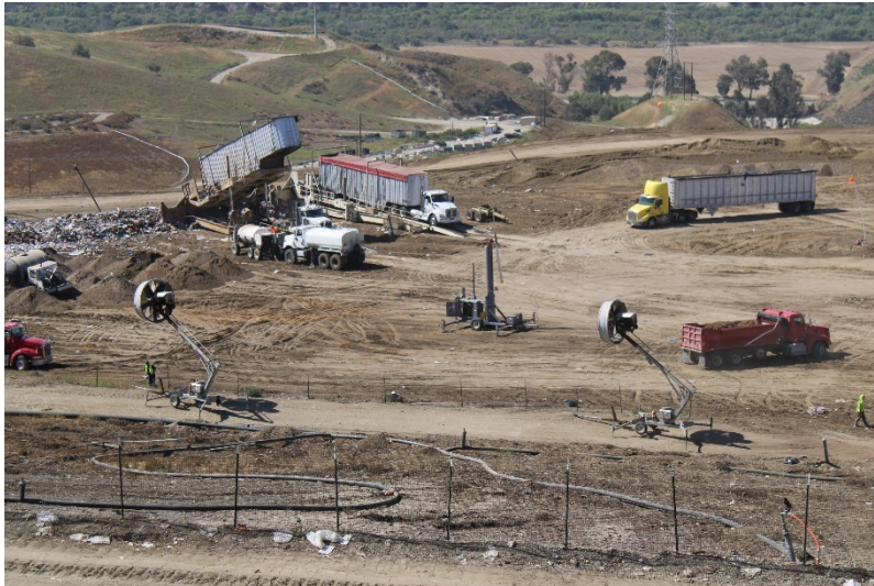
Photo 53: Cell 6 Working Area: May 24, 2022
