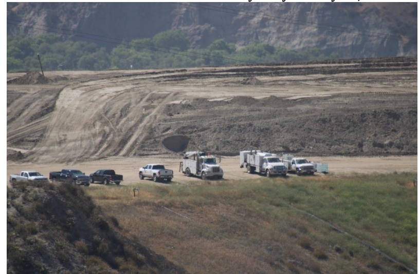
Photo 124: Closed Landfill - Primary Canyon: May 24, 2022
