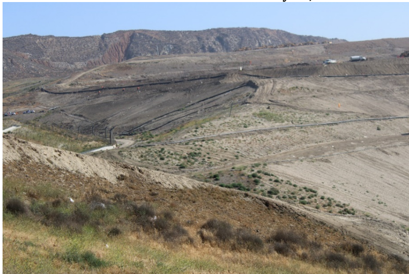
Photo 455: Cell 8 Construction: May 24, 2022
