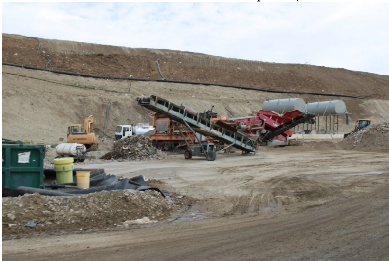
Photo 415: Cell 8 Construction: April 26, 2022
