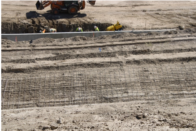
Photo 493: Cell 8 Construction: June 21, 2022
