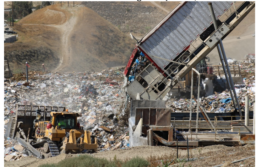
Photo 112: Cell 6 Working Area: June 21, 2022
