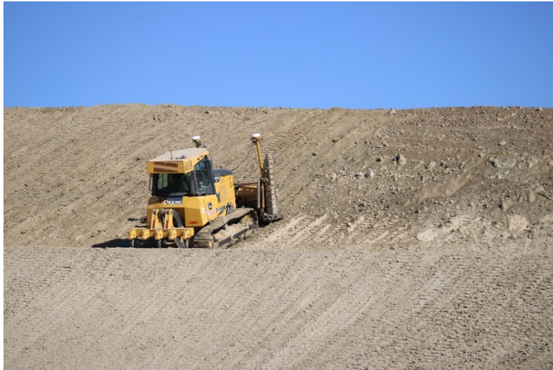
Photo 441: Cell 8 Construction: May 24, 2022
