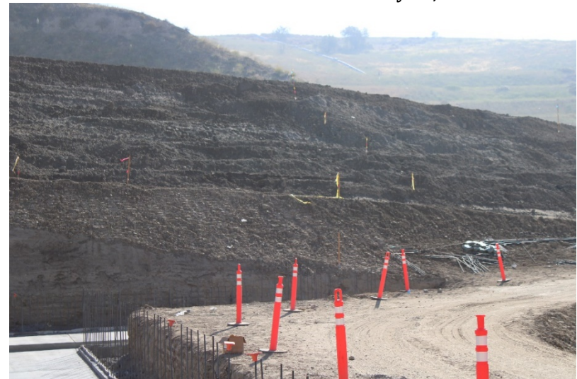
Photo 440: Cell 8 Construction: May 24, 2022
