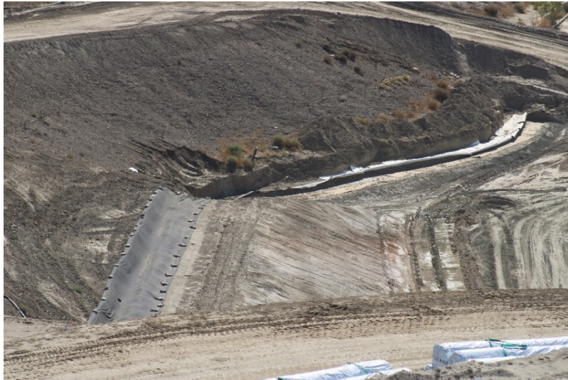
Photo 501: Cell 8 Construction: June 21, 2022
