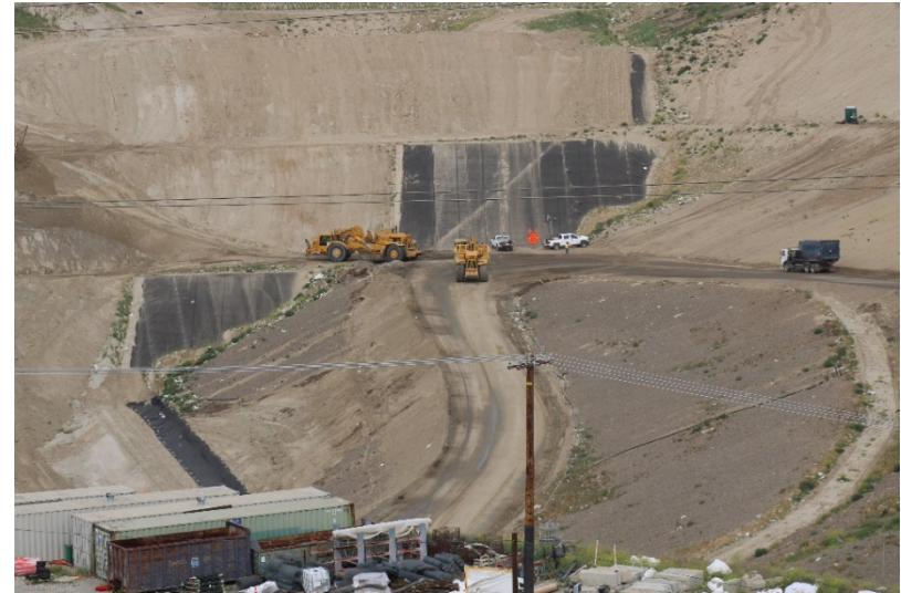
Photo 418: Cell 8 Construction: April 26, 2022
