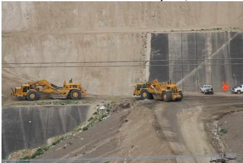
Photo 419: Cell 8 Construction: April 26, 2022
