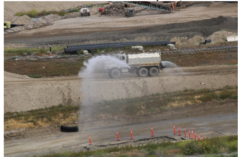
Photo 420: Cell 8 Construction: April 26, 2022
