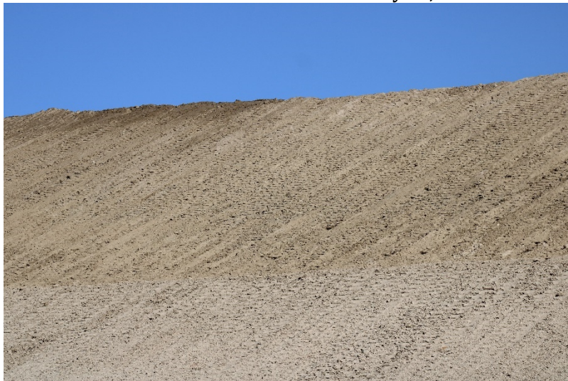
Photo 447: Cell 8 Construction: May 24, 2022
