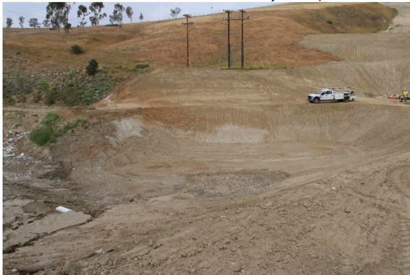
Photo 399: Cell 8 Construction: April 26, 2022
