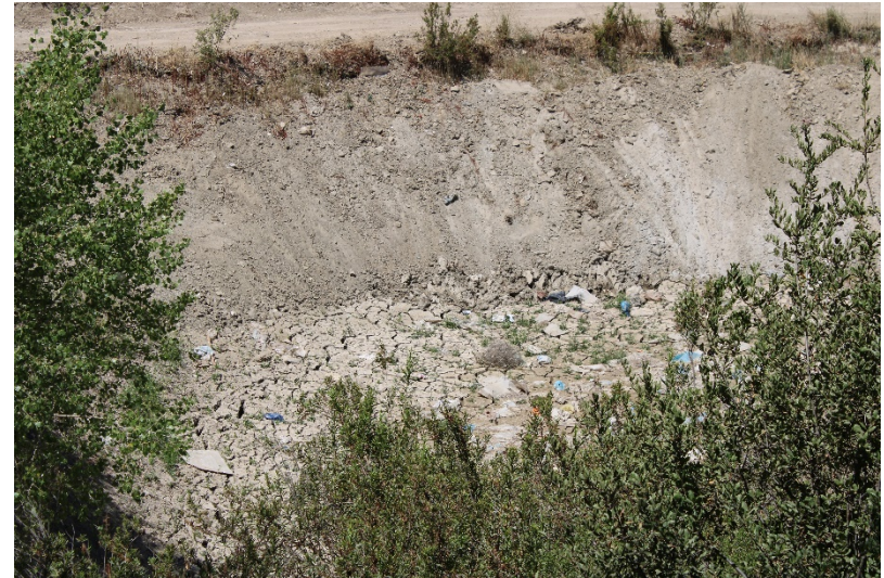
Photo 194: South Terminal and Catch Basins: June 21, 2022
