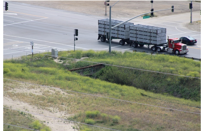
Photo 270: Wolcott Way Entrance Facilities: April 26, 2022
