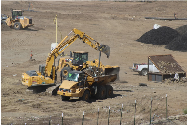
Photo 73: Cell 6 Working Area: May 24, 2022
