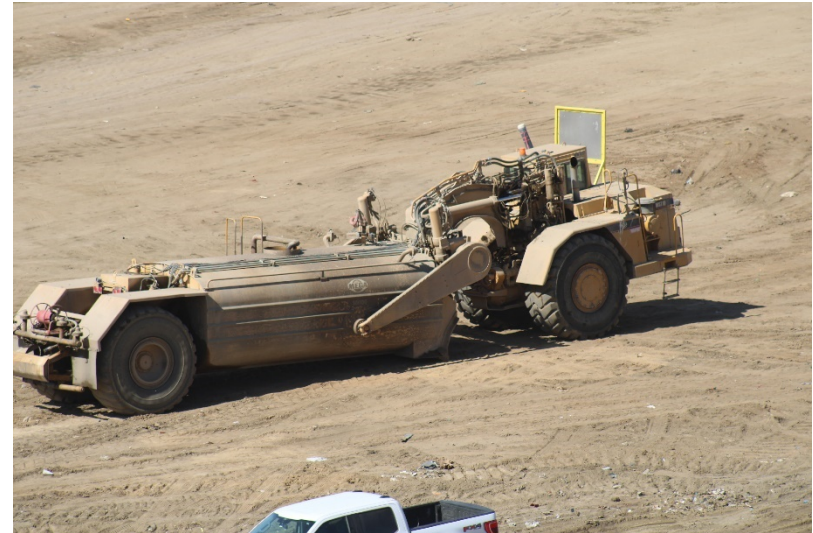
Photo 66: Cell 6 Working Area: May 24, 2022
