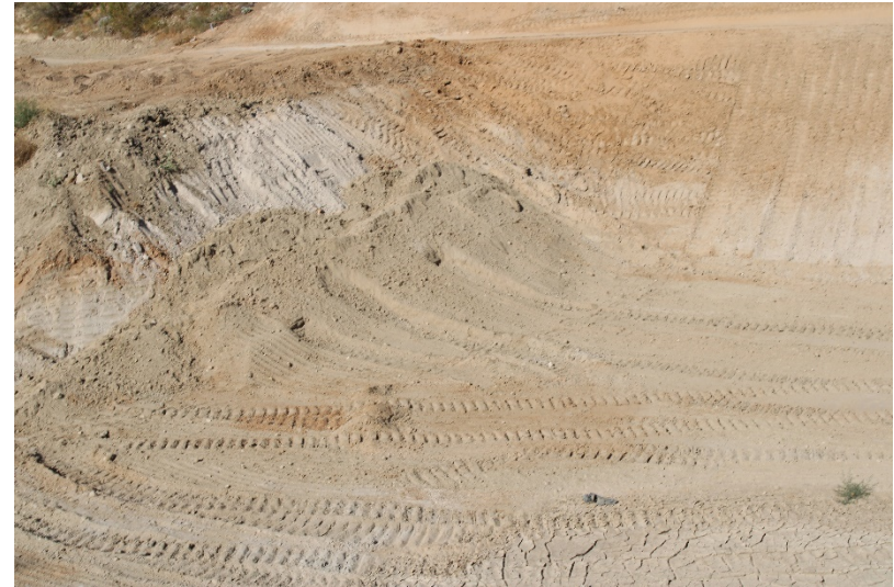
Photo 482: Cell 8 Construction: June 21, 2022
