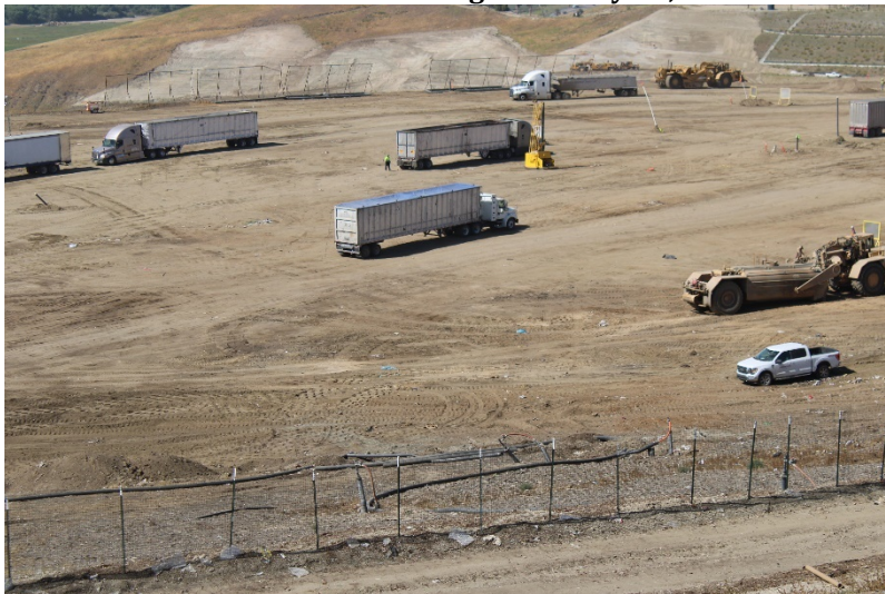
Photo 55: Cell 6 Working Area: May 24, 2022
