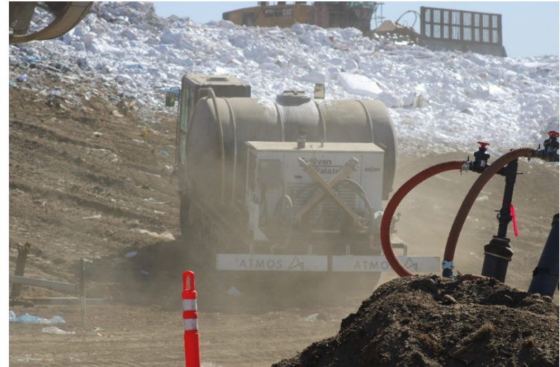
Photo 90: Cell 6 Working Area: June 21, 2022
