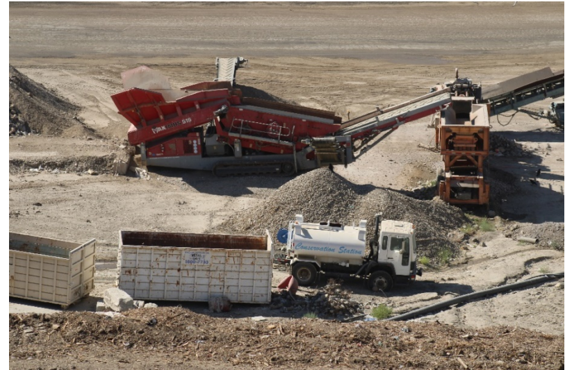
Photo 98: Cell 6 Working Area: June 21, 2022
