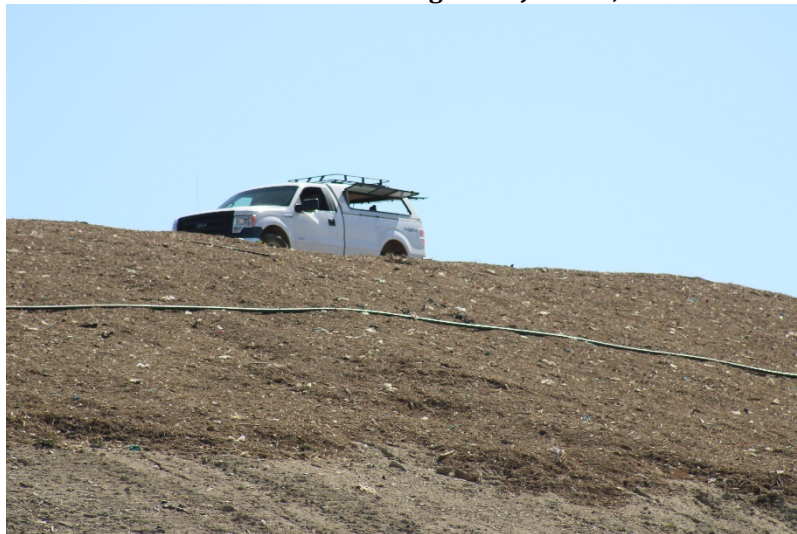
Photo 107: Cell 6 Working Area: June 21, 2022
