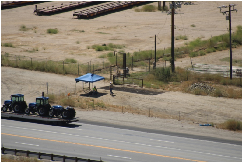
Photo 285: Wolcott Way Entrance Facilities: June 21, 2022
