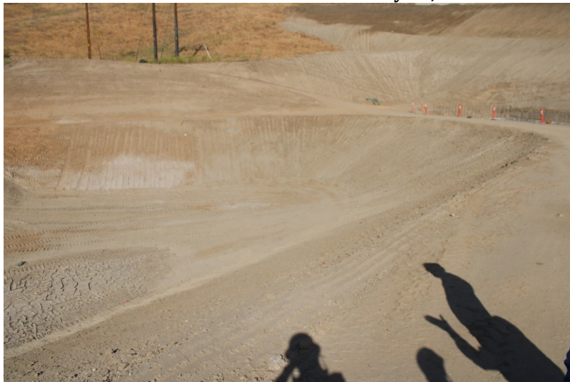
Photo 427: Cell 8 Construction: May 24, 2022
