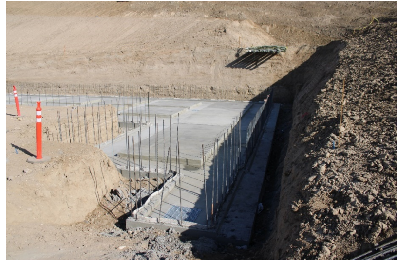
Photo 430: Cell 8 Construction: May 24, 2022
