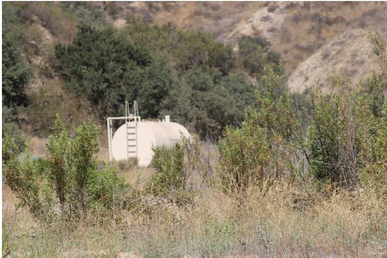
Photo 153: Closed Landfill - Canyon B: June 21, 2022
