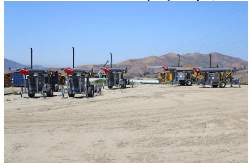
Photo 136: Closed Landfill - Primary Canyon: May 24, 2022
