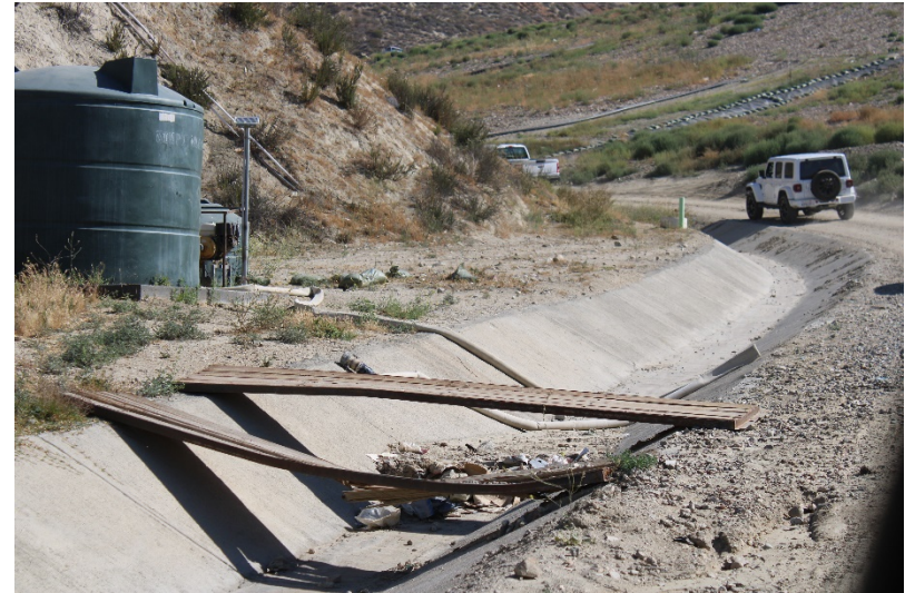
Photo 226: Landfill Perimeter Drainage Channel: May 24, 2022
