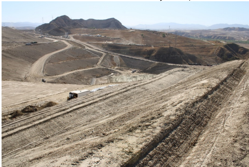
Photo 491: Cell 8 Construction: June 21, 2022
