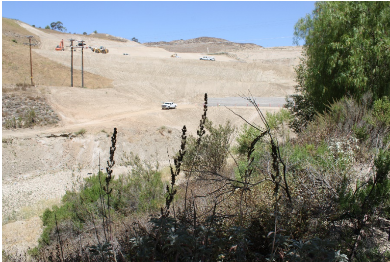
Photo 193: South Terminal and Catch Basins: June 21, 2022
