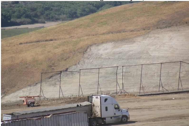
Photo 75: Cell 6 Working Area: May 24, 2022
