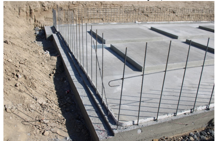
Photo 436: Cell 8 Construction: May 24, 2022
