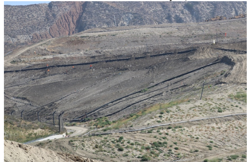
Photo 460: Cell 8 Construction: May 24, 2022
