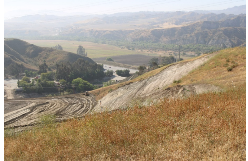
Photo 454: Cell 8 Construction: May 24, 2022
