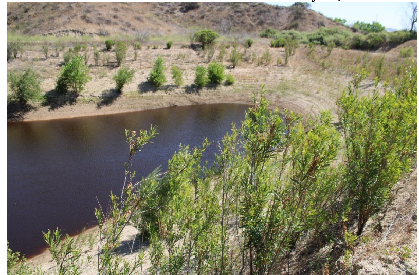
Photo 204: Northeast Sediment Basin: May 24, 2022
