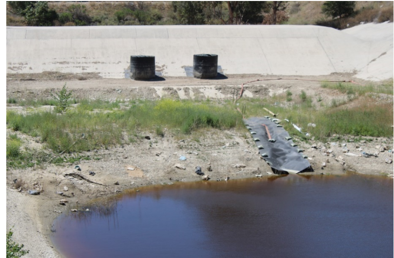
Photo 182: South Terminal and Catch Basins: May 24, 2022
