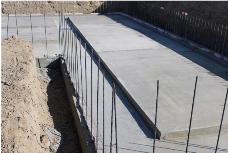
Photo 433: Cell 8 Construction: May 24, 2022
