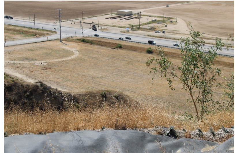
Photo 282: Wolcott Way Entrance Facilities: June 21, 2022
