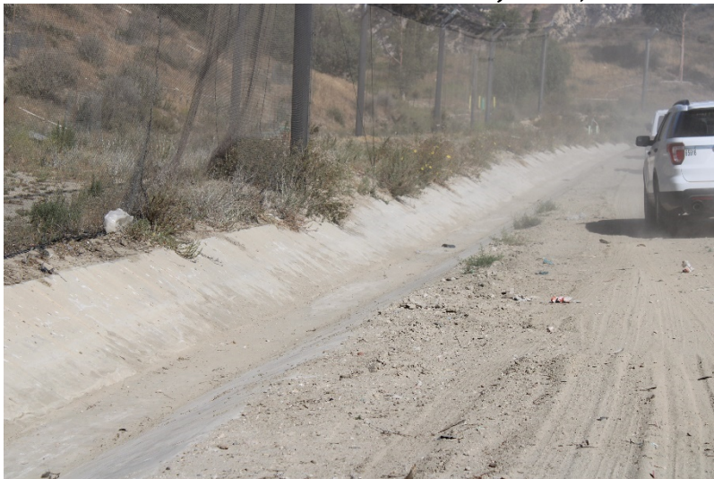
Photo 223: Landfill Perimeter Drainage Channel: May 24, 2022
