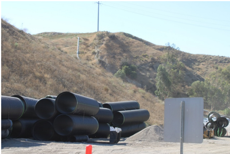
Photo 81: Cell 6 Working Area: June 21, 2022
