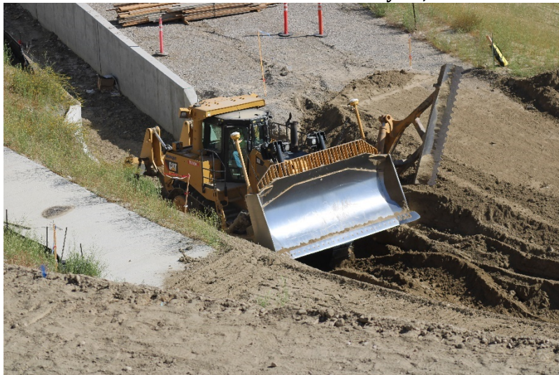
Photo 479: Cell 8 Construction: May 24, 2022
