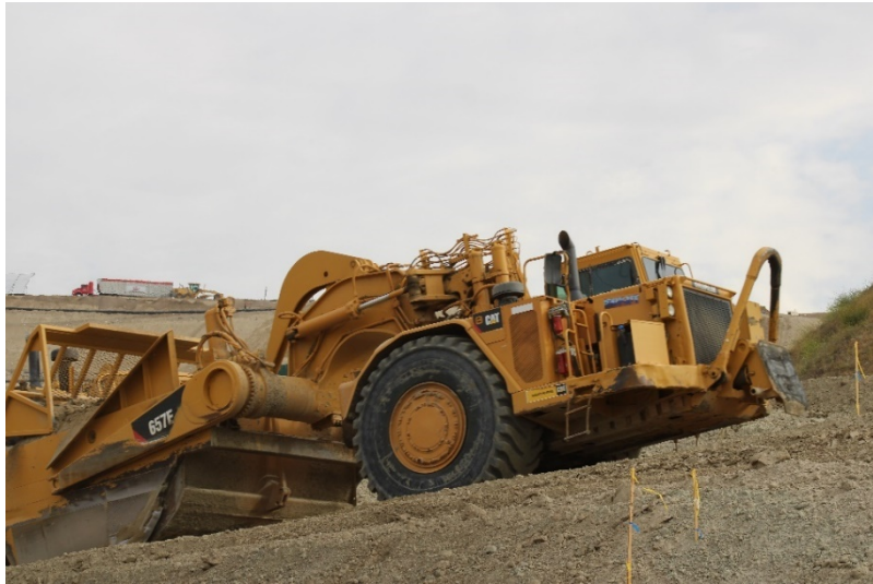
Photo 409: Cell 8 Construction: April 26, 2022
