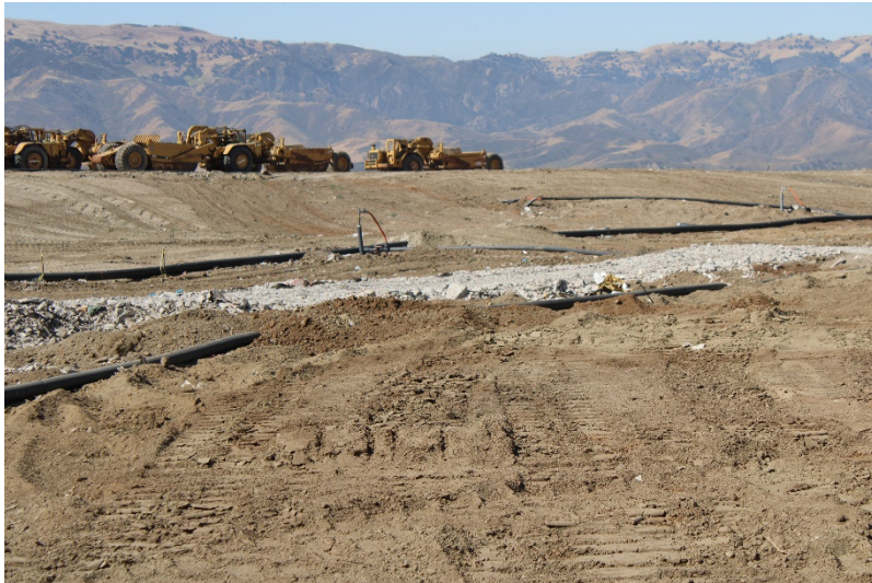
Photo 5: Top Deck Working Area: May 24, 2022
