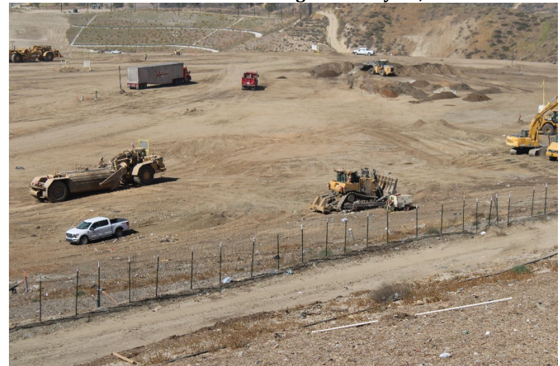
Photo 56: Cell 6 Working Area: May 24, 2022
