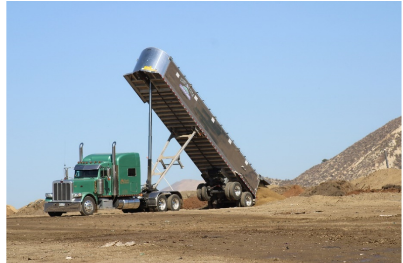
Photo 94: Cell 6 Working Area: June 21, 2022
