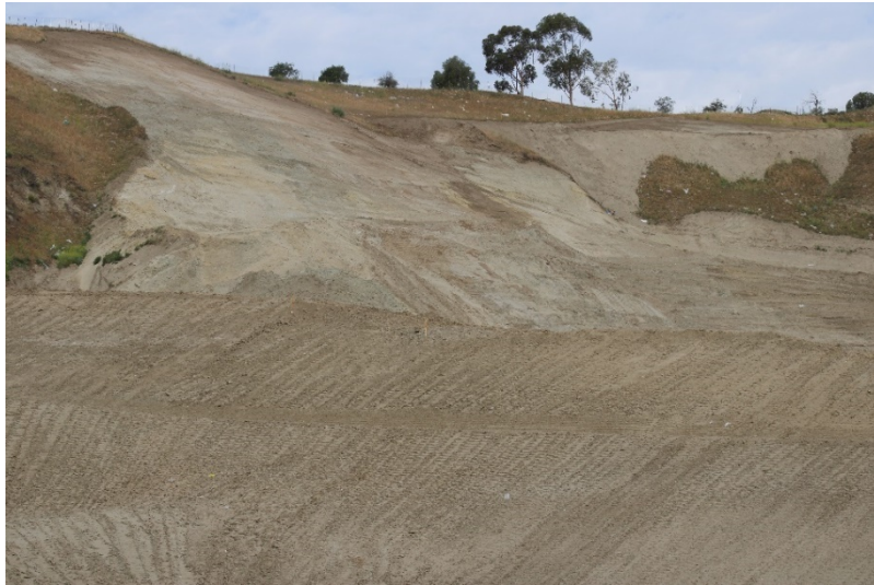
Photo 405: Cell 8 Construction: April 26, 2022
