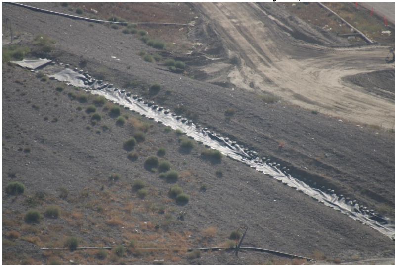
Photo 467: Cell 8 Construction: May 24, 2022
