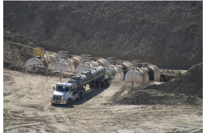
Photo 502: Cell 8 Construction: June 21, 2022
