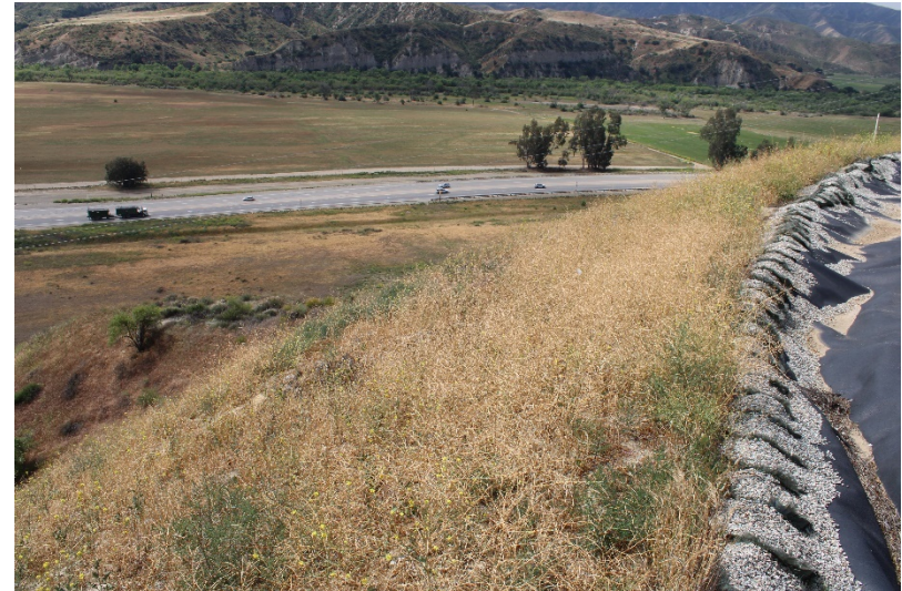
Photo 266: Wolcott Way Entrance Facilities: April 26, 2022
