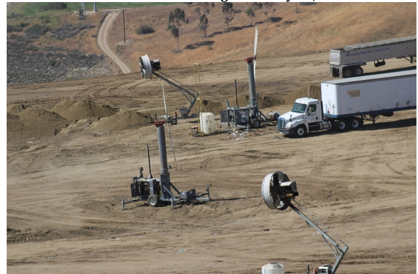
Photo 64: Cell 6 Working Area: May 24, 2022
