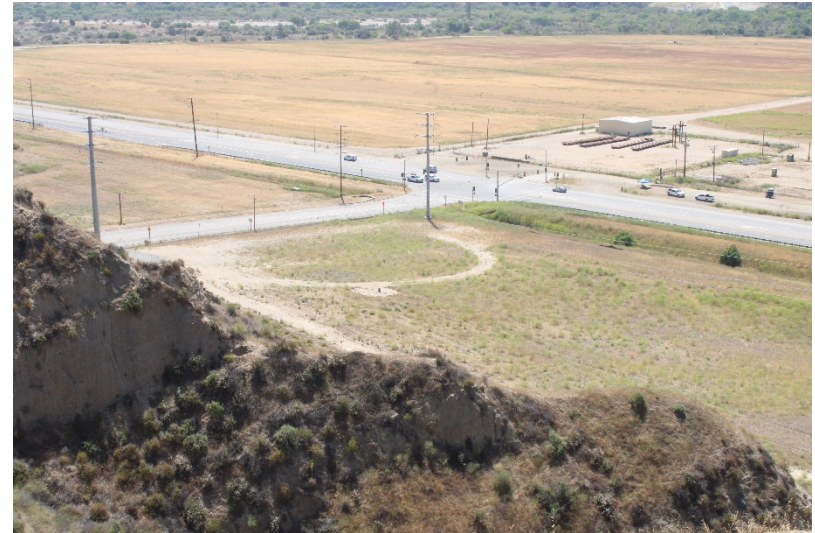
Photo 274: Wolcott Way Entrance Facilities: May 24, 2022
