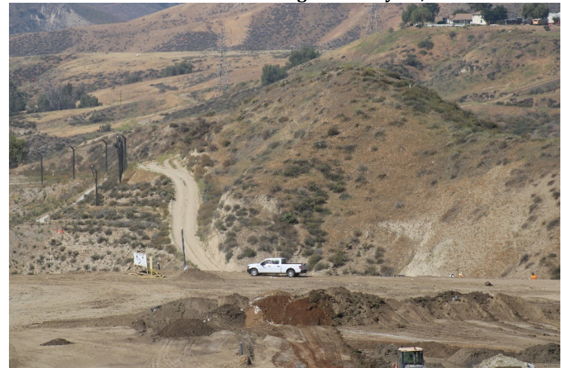
Photo 80: Cell 6 Working Area: May 24, 2022
