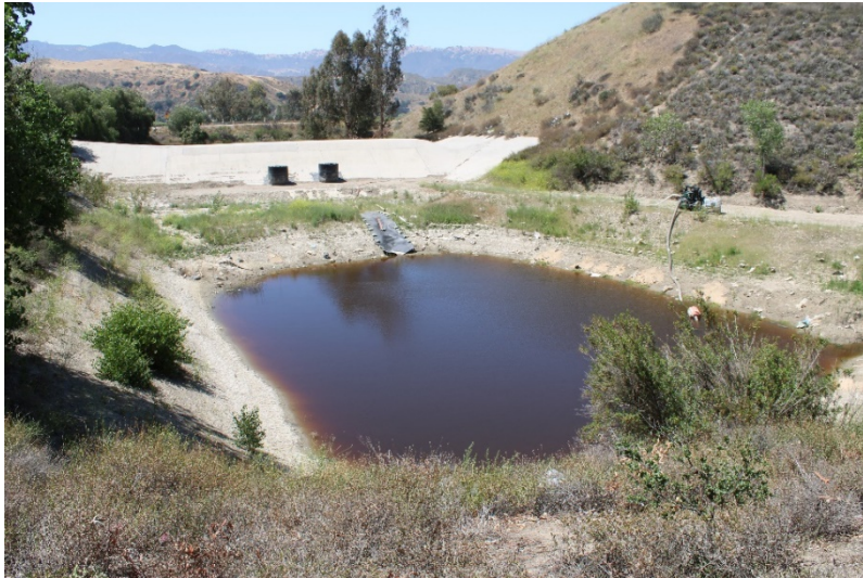
Photo 181: South Terminal and Catch Basins: May 24, 2022
