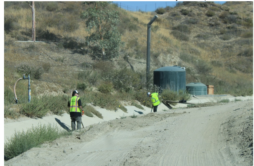
Photo 224: Landfill Perimeter Drainage Channel: May 24, 2022
