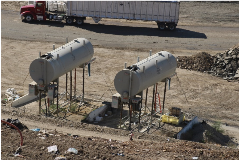
Photo 97: Cell 6 Working Area: June 21, 2022
