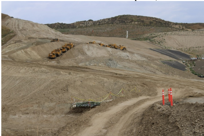
Photo 411: Cell 8 Construction: April 26, 2022
