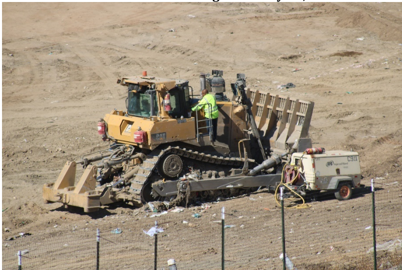
Photo 67: Cell 6 Working Area: May 24, 2022
