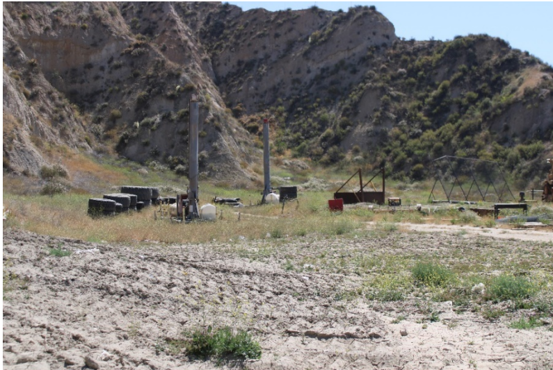
Photo 125: Closed Landfill - Primary Canyon: May 24, 2022
