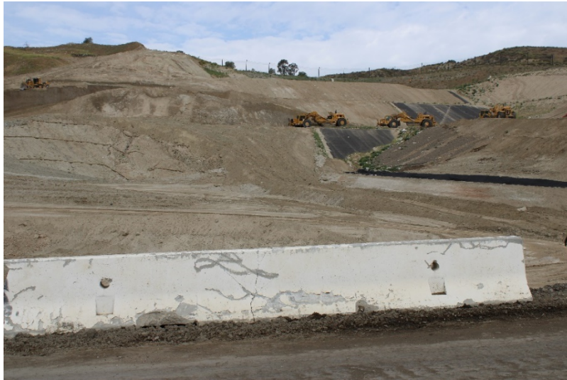
Photo 413: Cell 8 Construction: April 26, 2022
