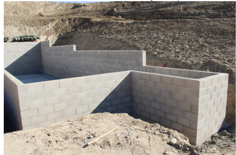
Photo 484: Cell 8 Construction: June 21, 2022
