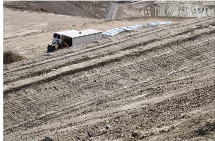
Photo 494: Cell 8 Construction: June 21, 2022
