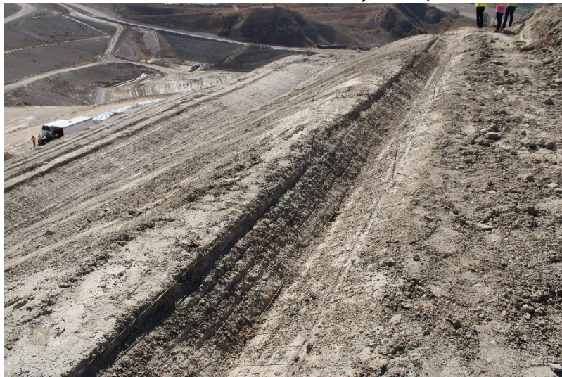
Photo 487: Cell 8 Construction: June 21, 2022
