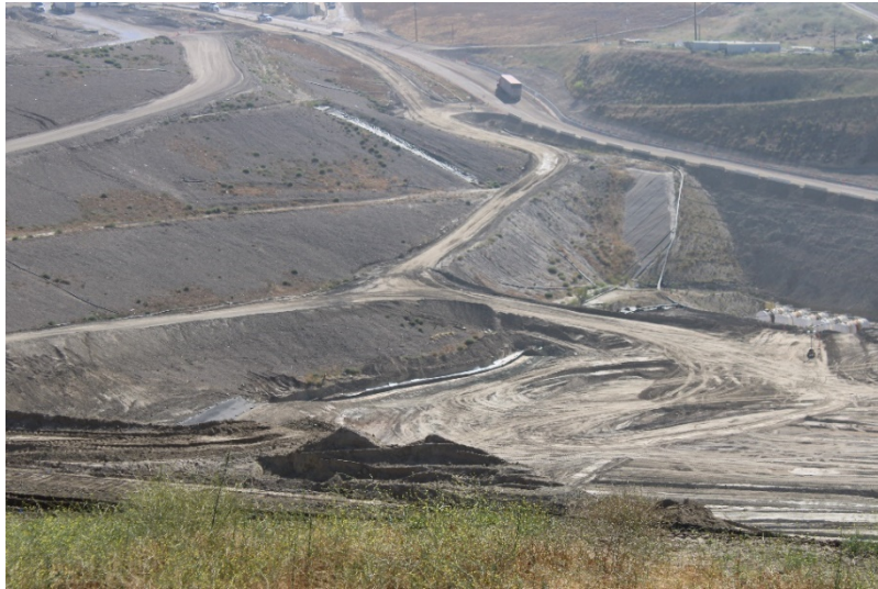
Photo 457: Cell 8 Construction: May 24, 2022
