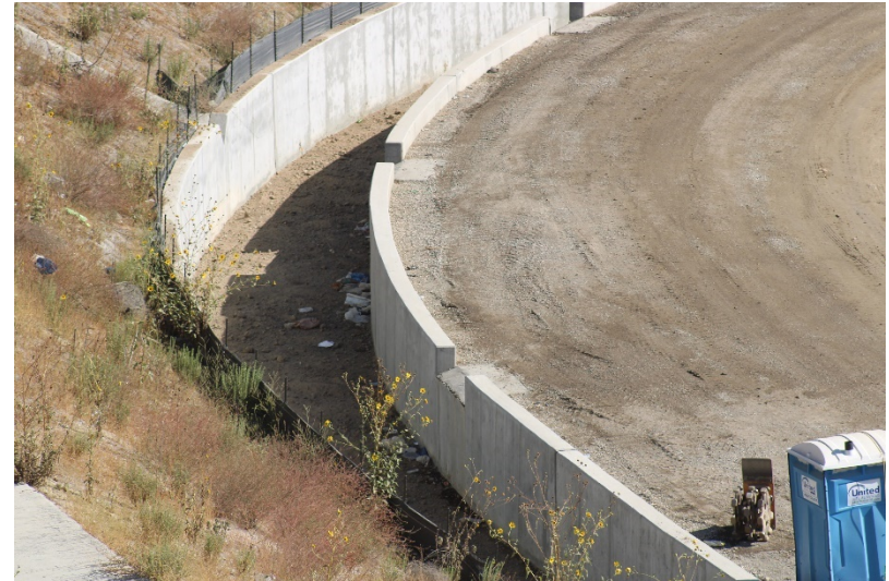
Photo 230: Landfill Perimeter Drainage Channel: June 21, 2022
