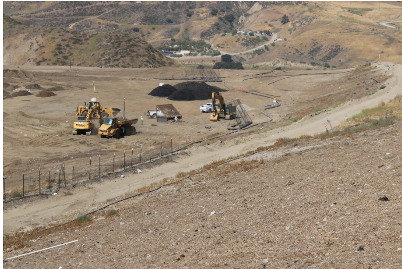
Photo 57: Cell 6 Working Area: May 24, 2022
