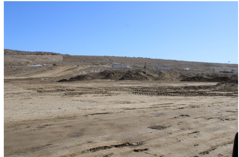
Photo 82: Cell 6 Working Area: June 21, 2022
