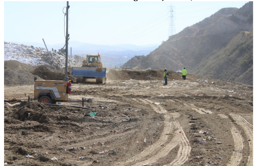
Photo 88: Cell 6 Working Area: June 21, 2022
