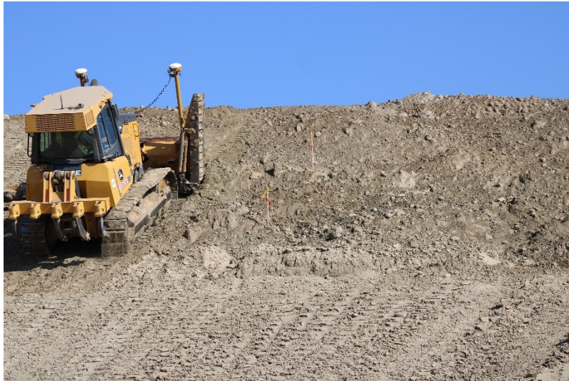
Photo 449: Cell 8 Construction: May 24, 2022
