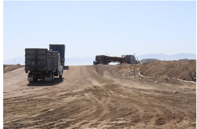
Photo 2: Top Deck Working Area: May 24, 2022
