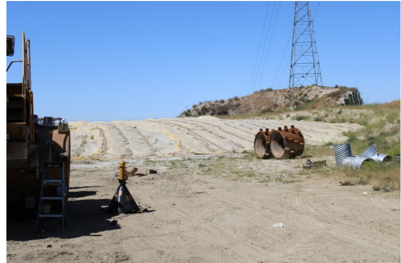
Photo 126: Closed Landfill - Primary Canyon: May 24, 2022
