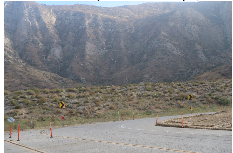
Photo 280: Wolcott Way Entrance Facilities: May 24, 2022
