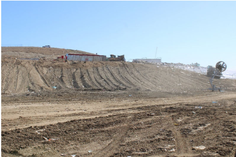
Photo 85: Cell 6 Working Area: June 21, 2022
