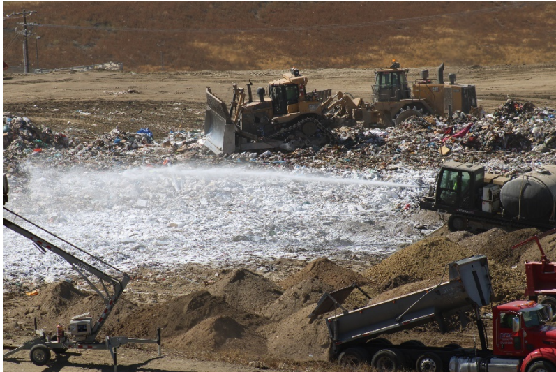
Photo 61: Cell 6 Working Area: May 24, 2022
