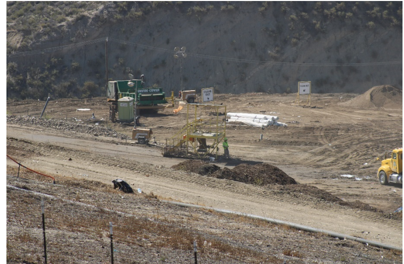
Photo 58: Cell 6 Working Area: May 24, 2022
