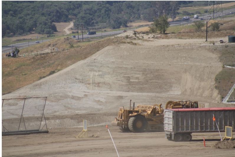
Photo 77: Cell 6 Working Area: May 24, 2022
