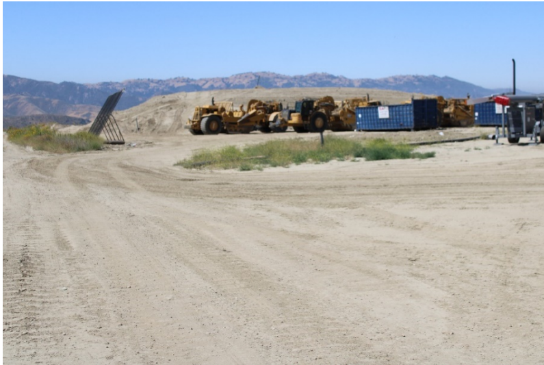
Photo 133: Closed Landfill - Primary Canyon: May 24, 2022
