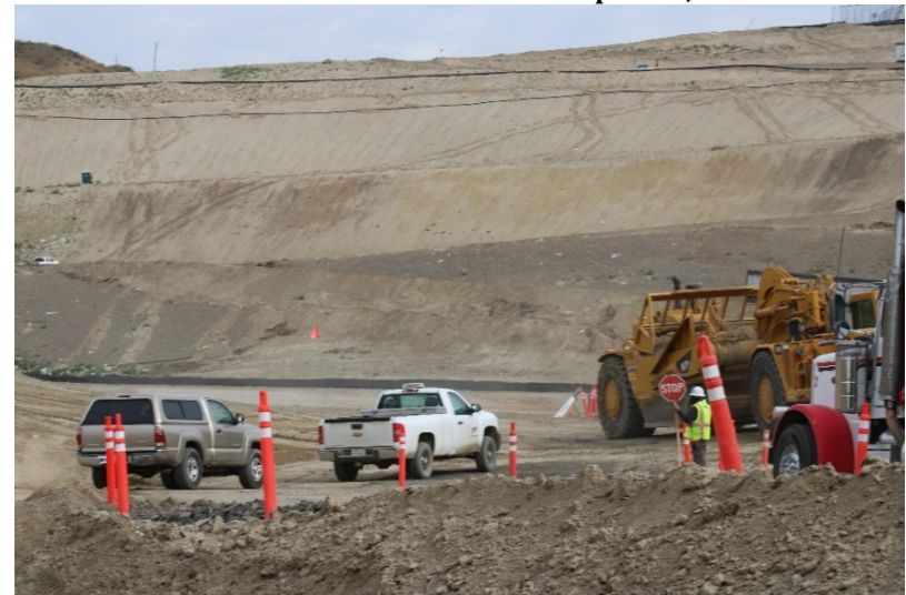
Photo 408: Cell 8 Construction: April 26, 2022
