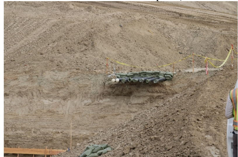
Photo 404 Cell 8 Construction: April 26, 2022
