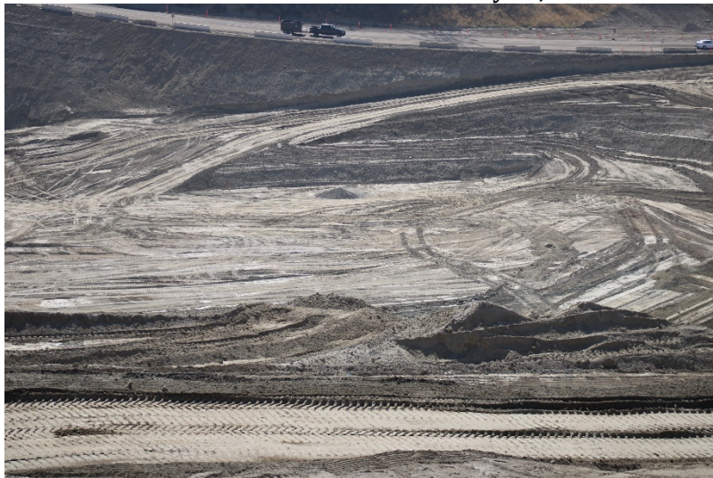
Photo 475: Cell 8 Construction: May 24, 2022
