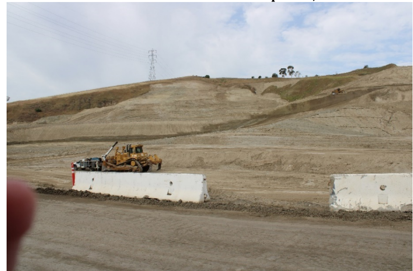
Photo 412: Cell 8 Construction: April 26, 2022
