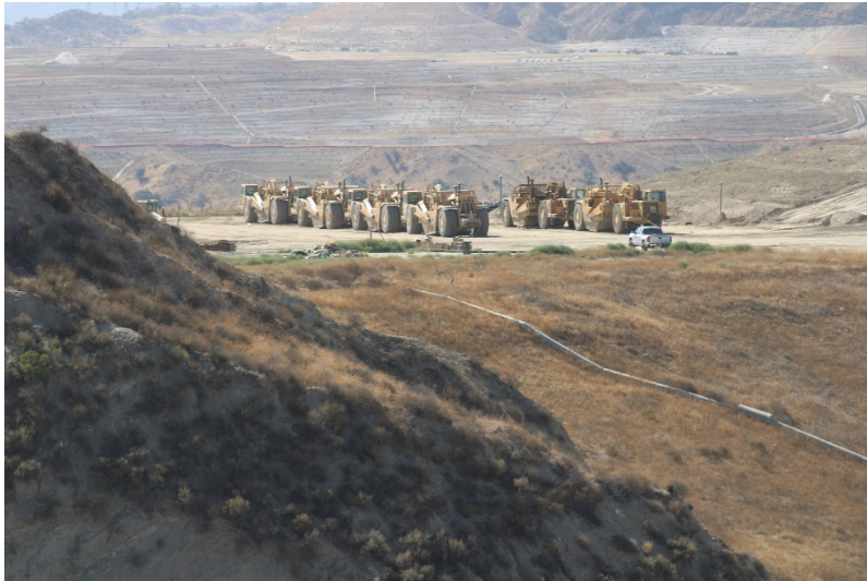
Photo 137: Closed Landfill - Primary Canyon: June 21, 2022
