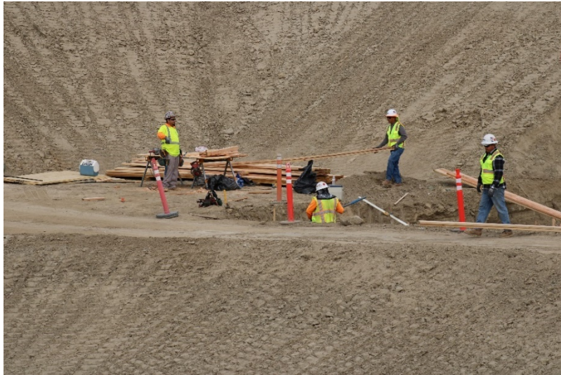
Photo 401: Cell 8 Construction: April 26, 2022
