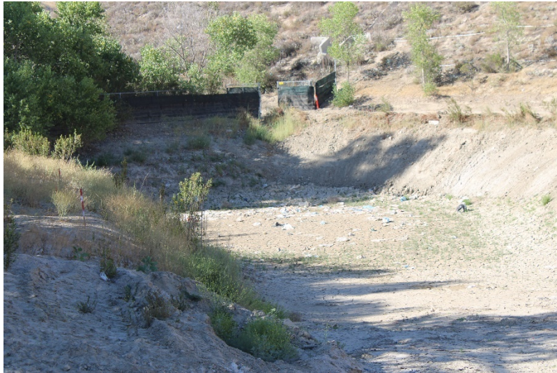
Photo 481: Cell 8 Construction: June 21, 2022
