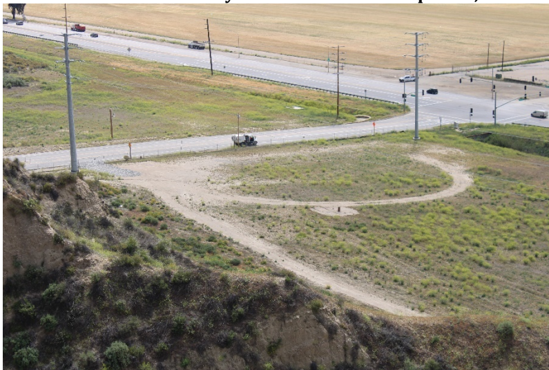
Photo 267: Wolcott Way Entrance Facilities: April 26, 2022
