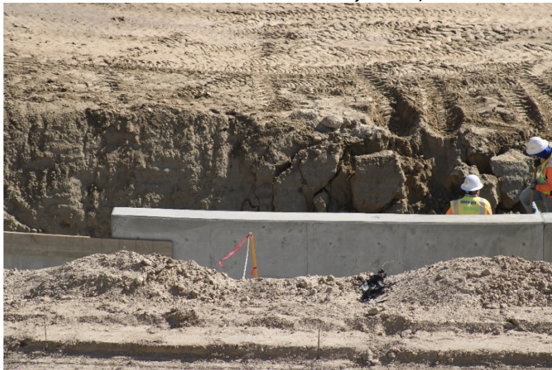
Photo 495: Cell 8 Construction: June 21, 2022
