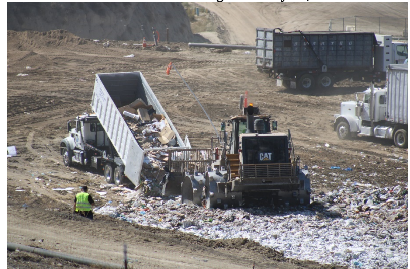
Photo 72: Cell 6 Working Area: May 24, 2022
