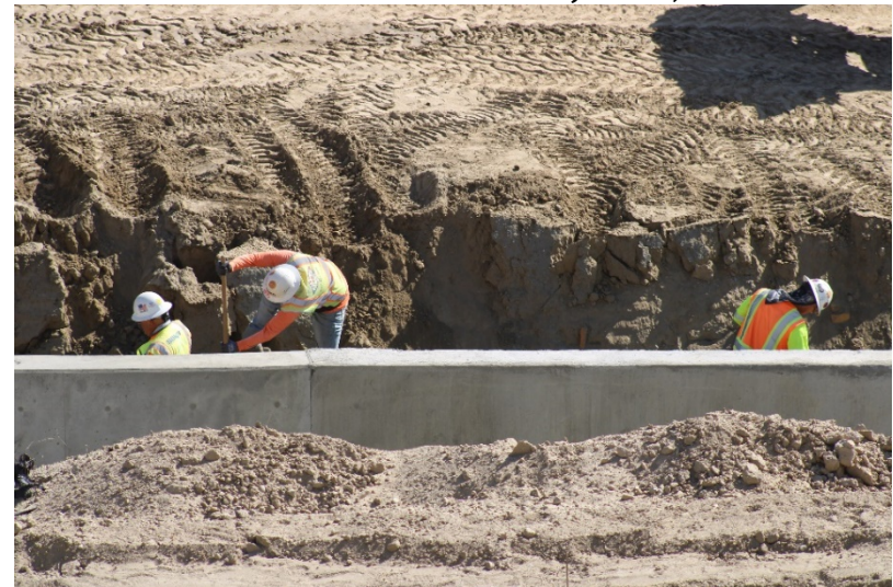
Photo 496: Cell 8 Construction: June 21, 2022
