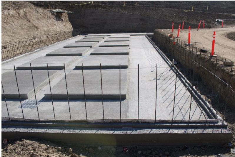
Photo 437: Cell 8 Construction: May 24, 2022
