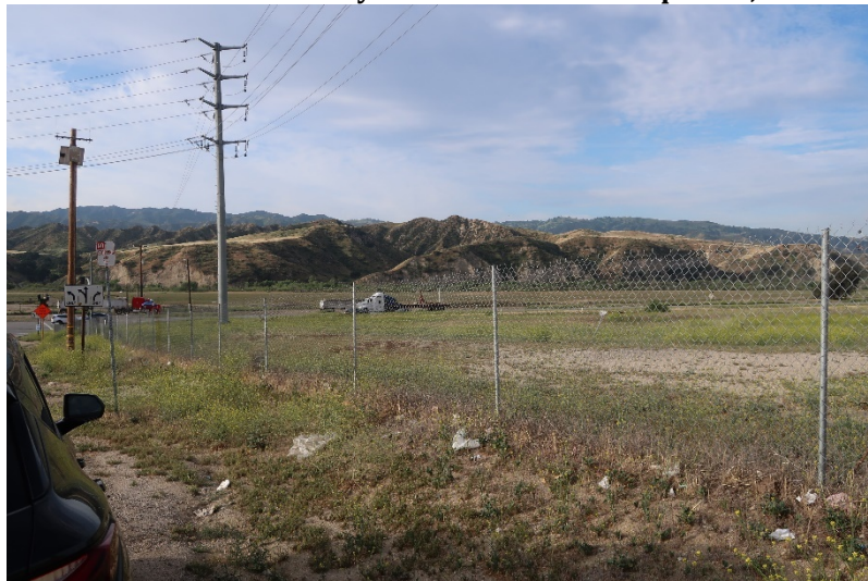
Photo 271: Wolcott Way Entrance Facilities: April 26, 2022
