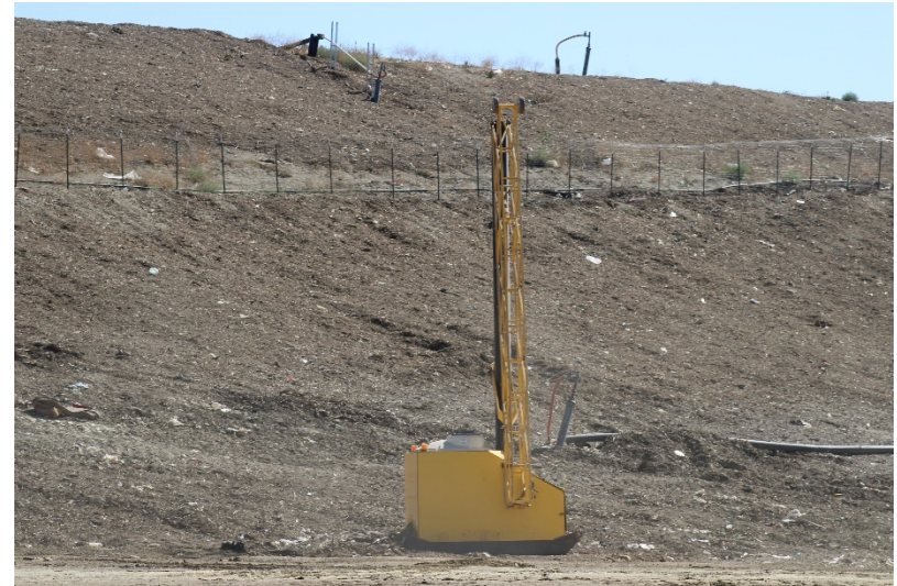
Photo 102: Cell 6 Working Area: June 21, 2022
