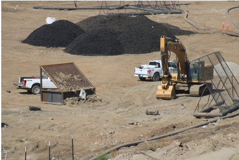
Photo 69: Cell 6 Working Area: May 24, 2022
