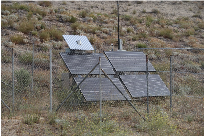
Photo 277: Wolcott Way Entrance Facilities: May 24, 2022
