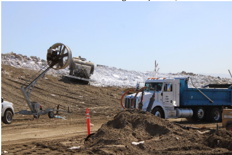
Photo 87: Cell 6 Working Area: June 21, 2022
