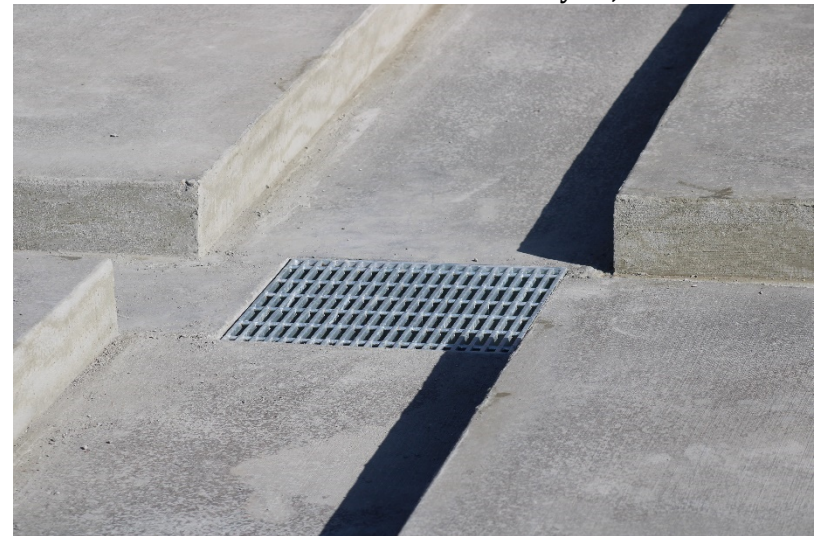
Photo 444: Cell 8 Construction: May 24, 2022
