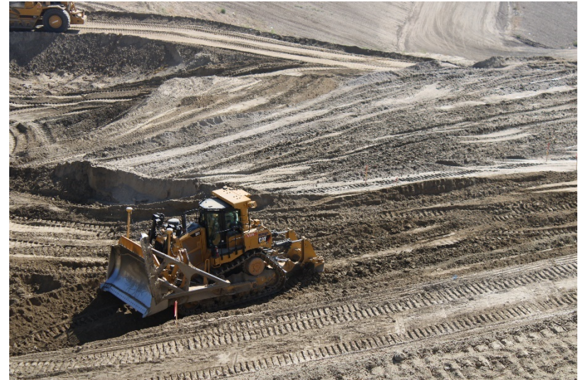
Photo 474: Cell 8 Construction: May 24, 2022
