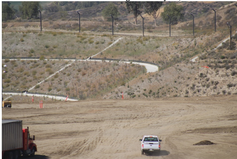
Photo 79: Cell 6 Working Area: May 24, 2022
