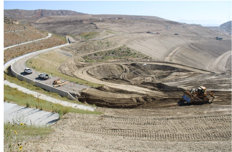
Photo 470: Cell 8 Construction: May 24, 2022
