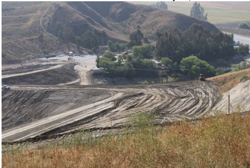
Photo 459: Cell 8 Construction: May 24, 2022
