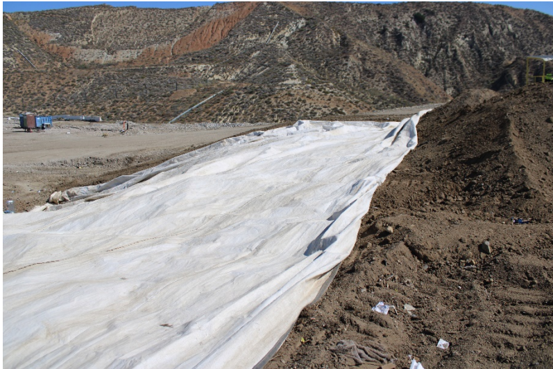
Photo 9: Top Deck Working Area: May 24, 2022
