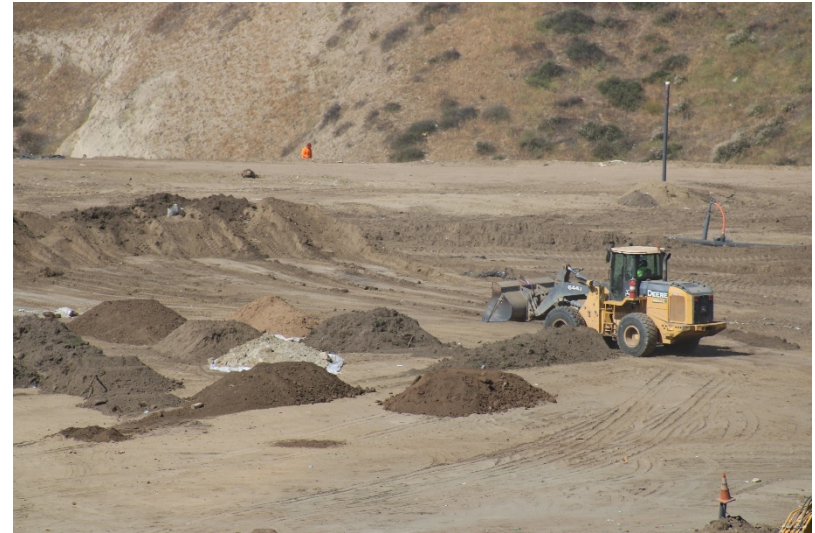
Photo 70: Cell 6 Working Area: May 24, 2022
