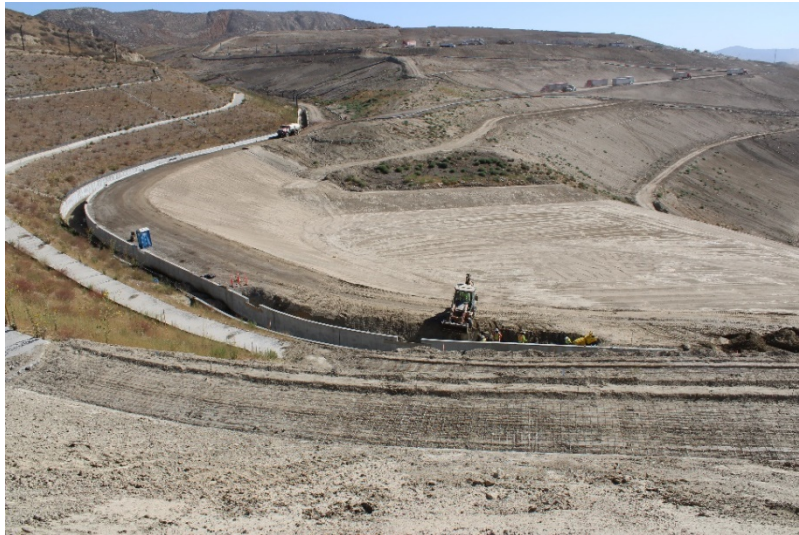
Photo 489: Cell 8 Construction: June 21, 2022
