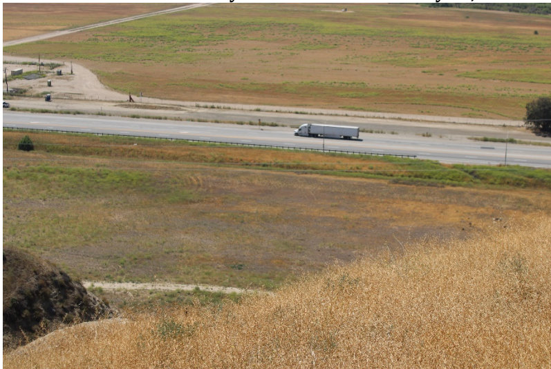
Photo 275: Wolcott Way Entrance Facilities: May 24, 2022
