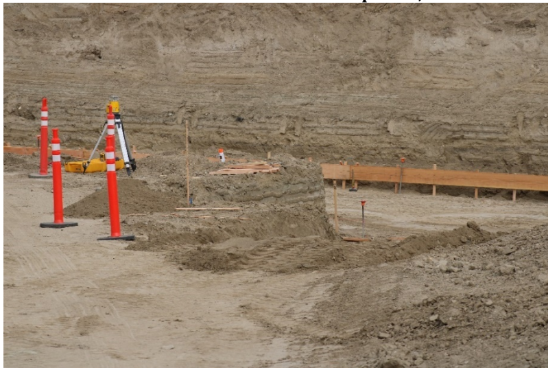
Photo 403: Cell 8 Construction: April 26, 2022
