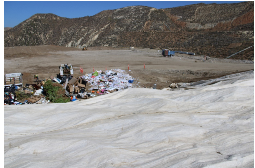
Photo 8: Top Deck Working Area: May 24, 2022
