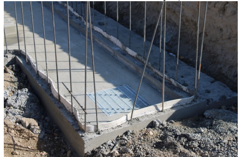
Photo 432: Cell 8 Construction: May 24, 2022
