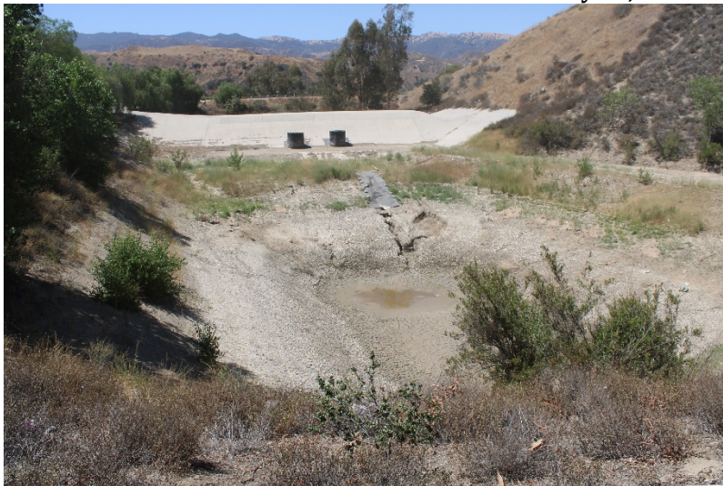
Photo 187: South Terminal and Catch Basins: June 21, 2022
