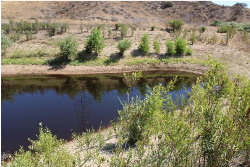
Photo 217: Northeast Sediment Basin: June 21, 2022
