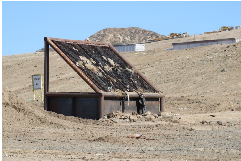
Photo 89: Cell 6 Working Area: June 21, 2022
