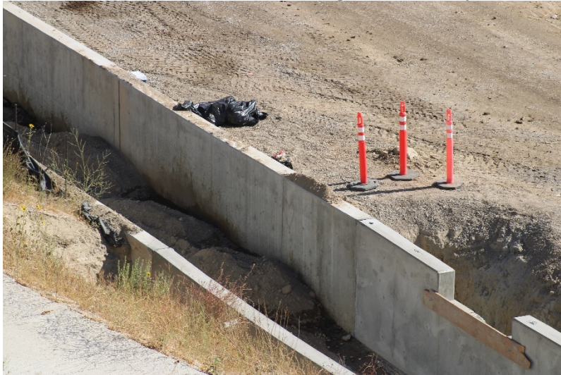
Photo 231: Landfill Perimeter Drainage Channel: June 21, 2022
