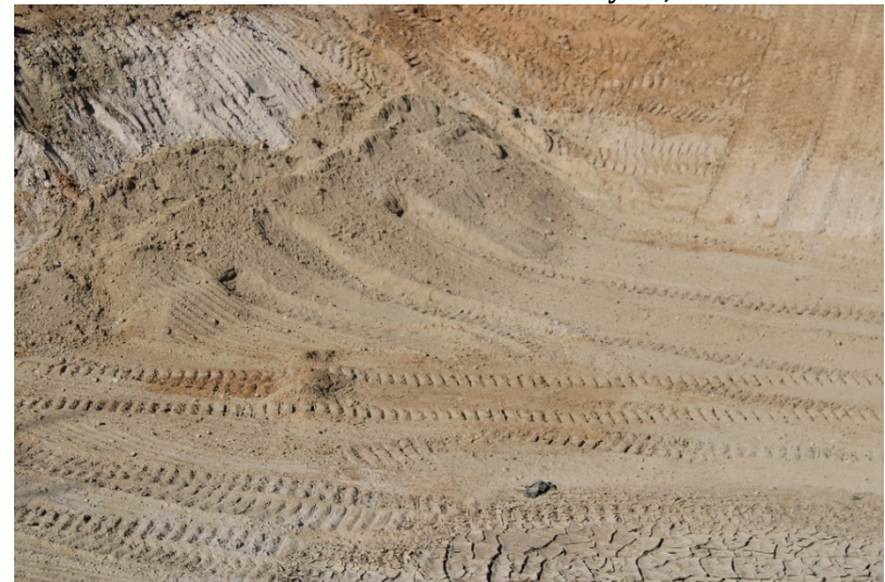
Photo 428: Cell 8 Construction: May 24, 2022
