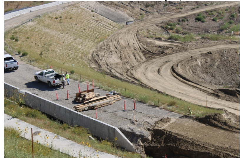
Photo 472: Cell 8 Construction: May 24, 2022
