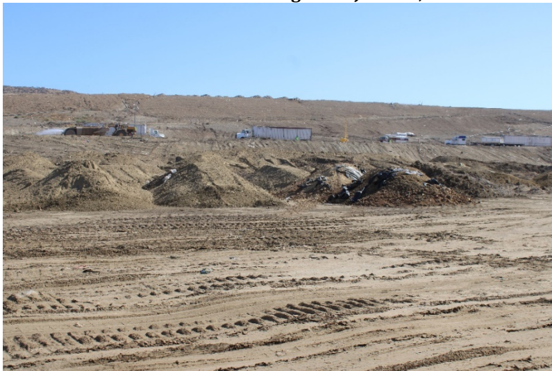
Photo 83: Cell 6 Working Area: June 21, 2022
