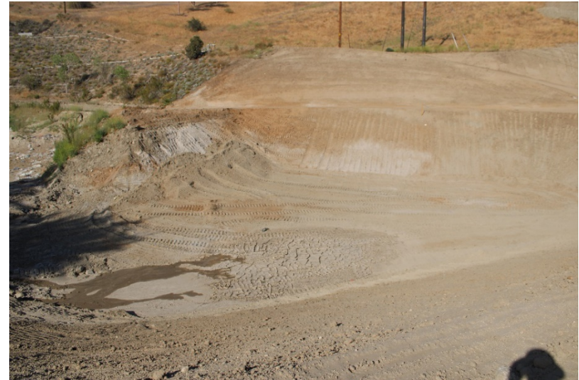
Photo 426: Cell 8 Construction: May 24, 2022
