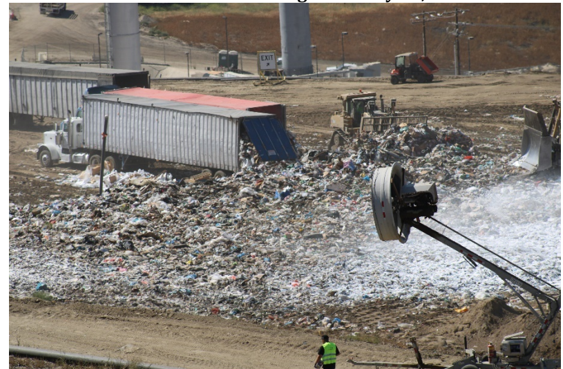
Photo 60: Cell 6 Working Area: May 24, 2022
