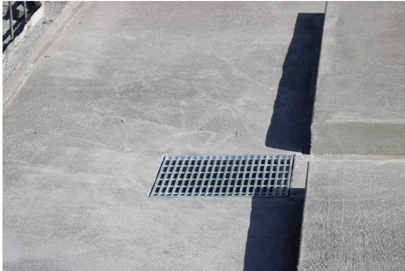
Photo 445: Cell 8 Construction: May 24, 2022
