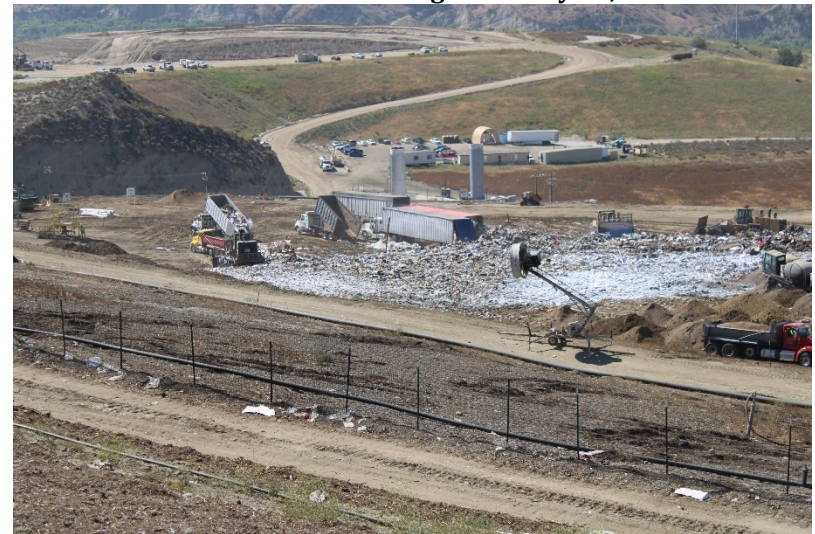
Photo 52: Cell 6 Working Area: May 24, 2022
