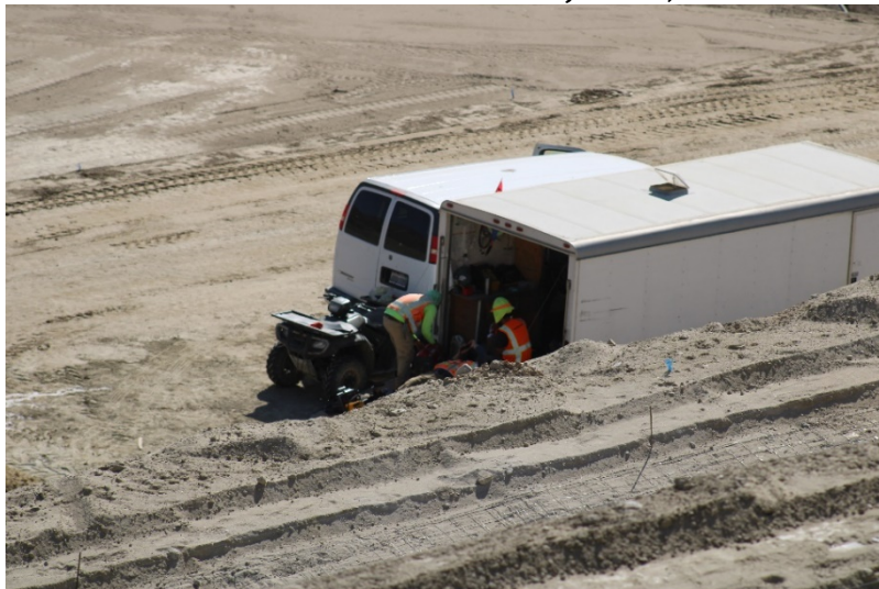
Photo 499: Cell 8 Construction: June 21, 2022
