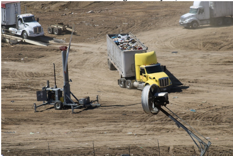
Photo 63: Cell 6 Working Area: May 24, 2022
