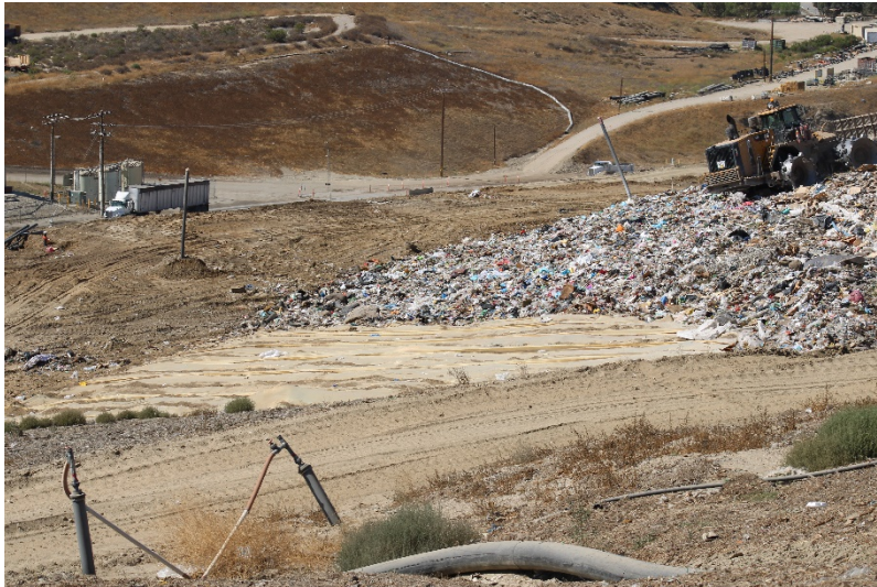
Photo 109: Cell 6 Working Area: June 21, 2022
