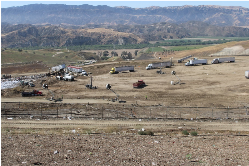
Photo 49: Cell 6 Working Area: May 24, 2022
