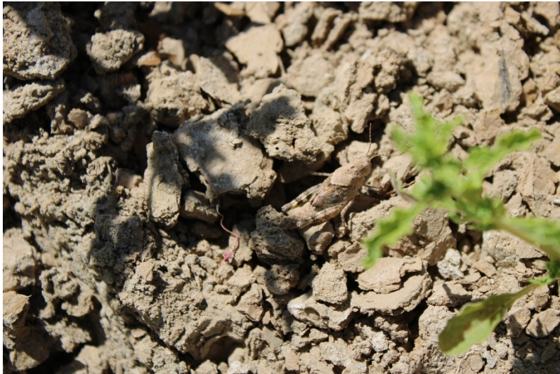
Photo 221: Northeast Sediment Basin: June 21, 2022
