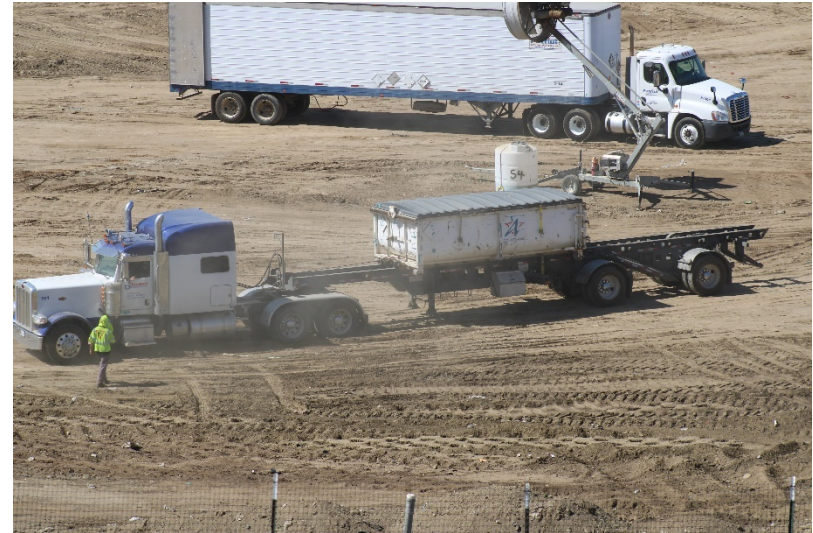
Photo 74: Cell 6 Working Area: May 24, 2022
