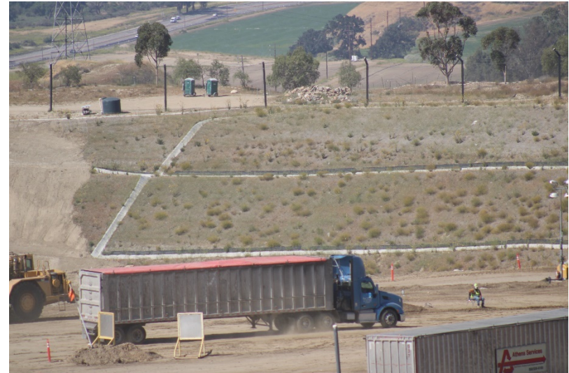
Photo 78: Cell 6 Working Area: May 24, 2022
