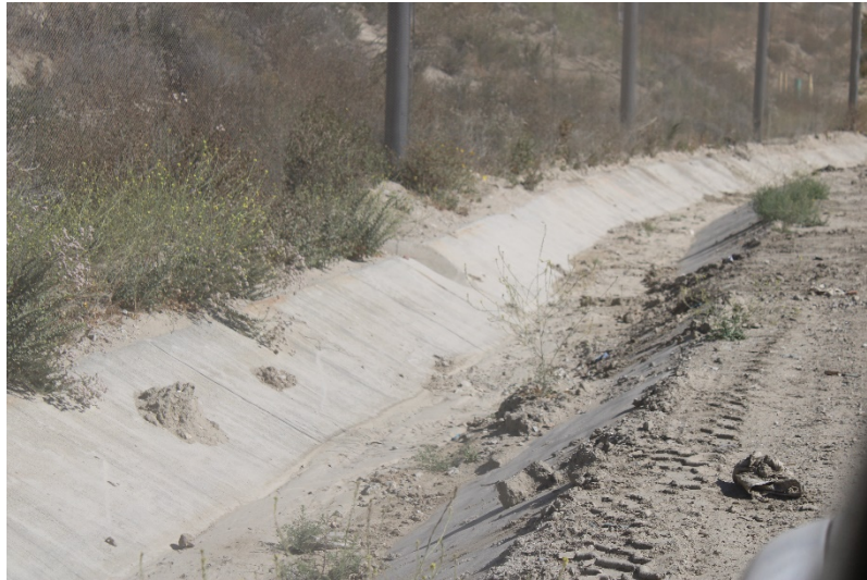
Photo 225: Landfill Perimeter Drainage Channel: May 24, 2022
