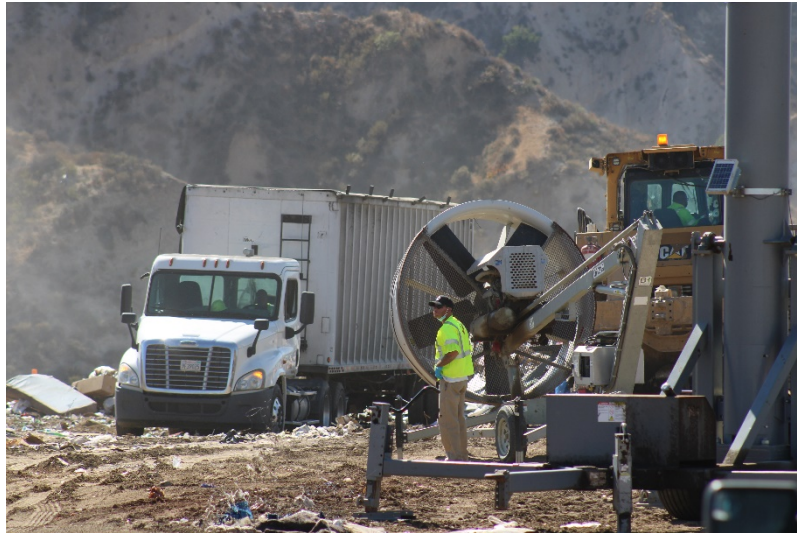
Photo 105: Cell 6 Working Area: June 21, 2022
