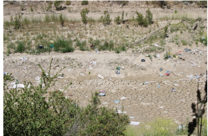
Photo 186: South Terminal and Catch Basins: May 24, 2022
