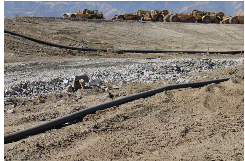
Photo 4: Top Deck Working Area: May 24, 2022
