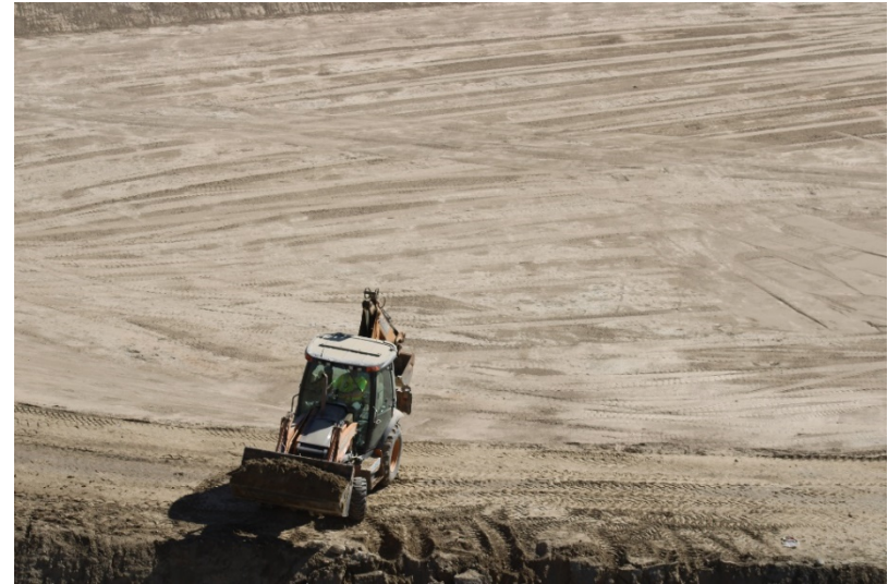
Photo 498: Cell 8 Construction: June 21, 2022
