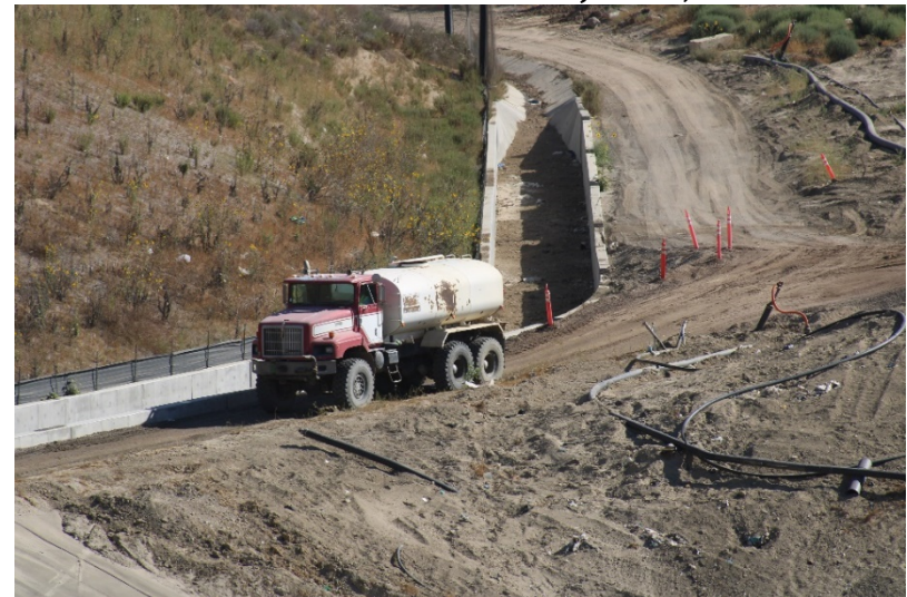
Photo 500: Cell 8 Construction: June 21, 2022
