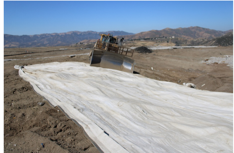
Photo 6: Top Deck Working Area: May 24, 2022
