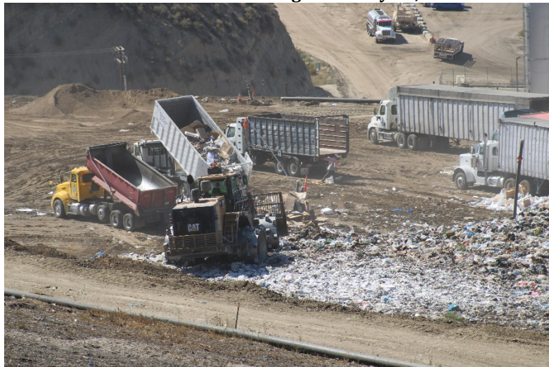
Photo 59: Cell 6 Working Area: May 24, 2022
