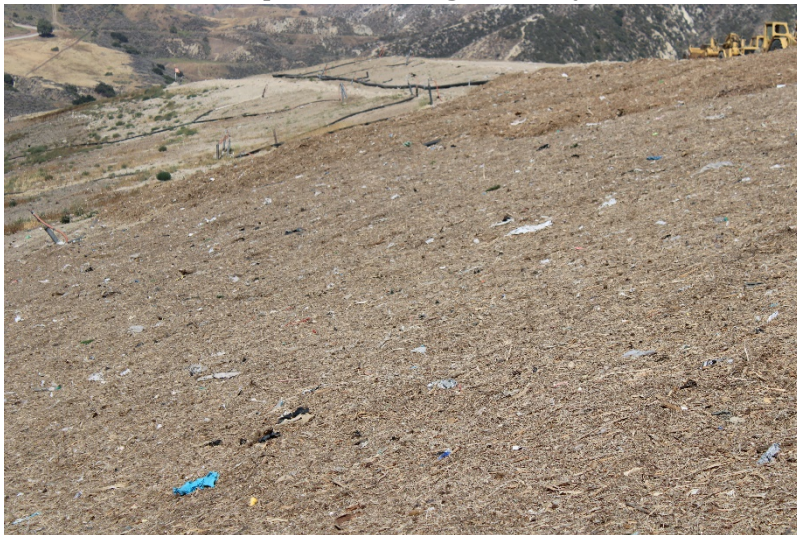
Photo 15: Top Deck Working Area: May 24, 2022
