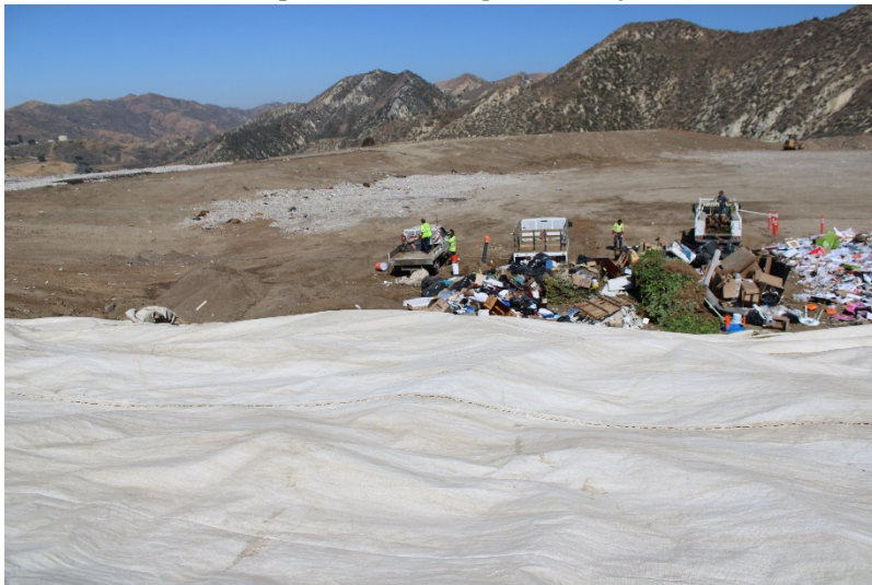
Photo 7: Top Deck Working Area: May 24, 2022
