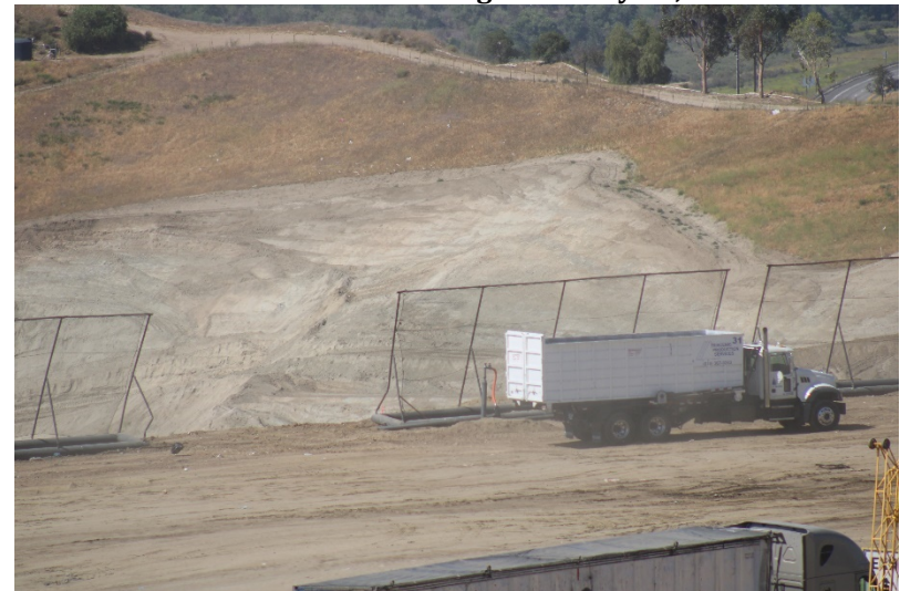
Photo 76: Cell 6 Working Area: May 24, 2022
