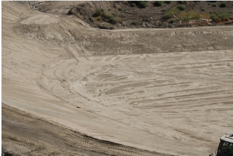
Photo 497: Cell 8 Construction: June 21, 2022
