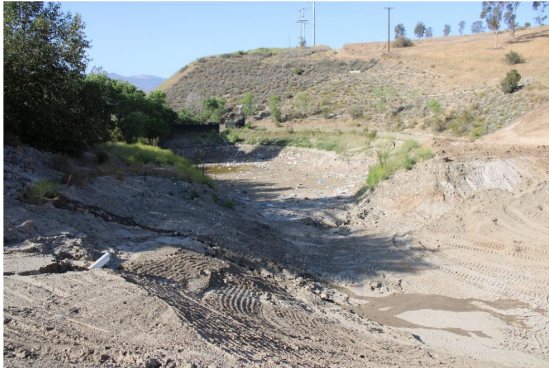
Photo 425: Cell 8 Construction: May 24, 2022
