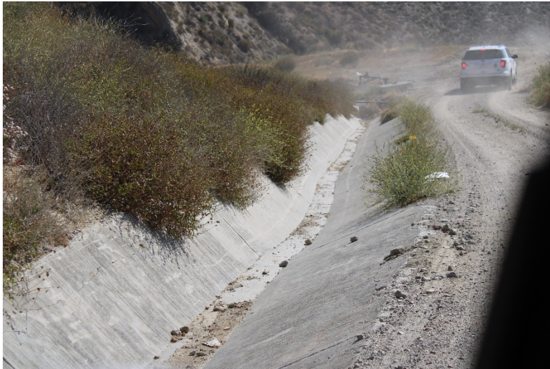
Photo 229: Landfill Perimeter Drainage Channel: May 24, 2022
