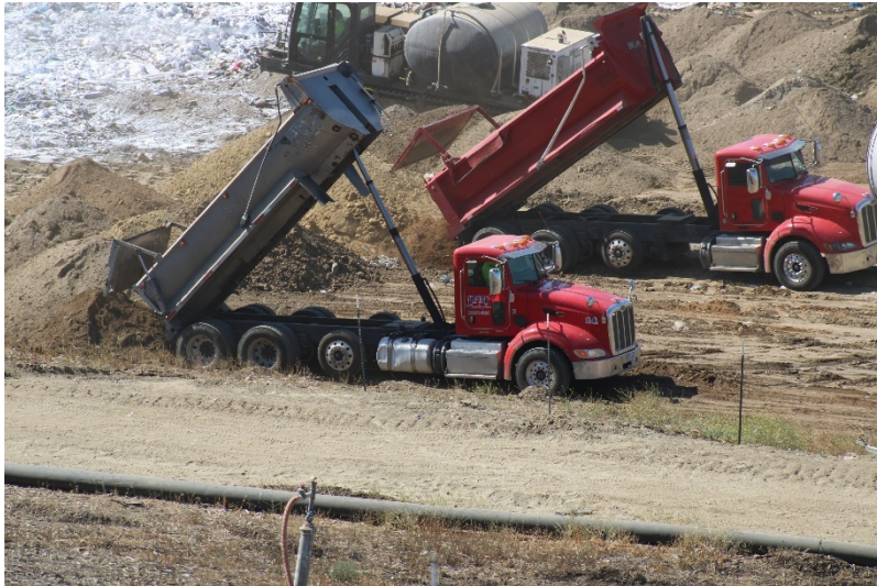
Photo 65: Cell 6 Working Area: May 24, 2022
