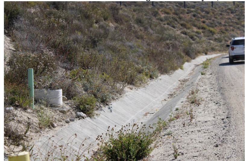
Photo 228: Landfill Perimeter Drainage Channel: May 24, 2022
