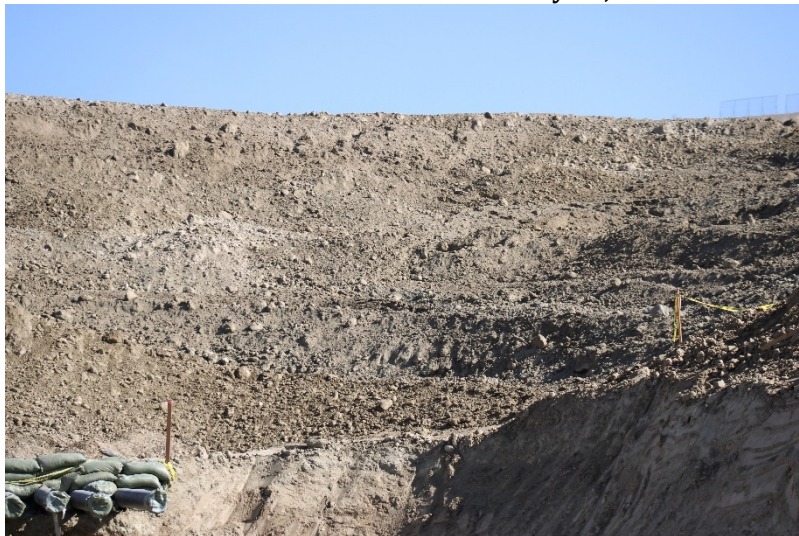
Photo 451: Cell 8 Construction: May 24, 2022
