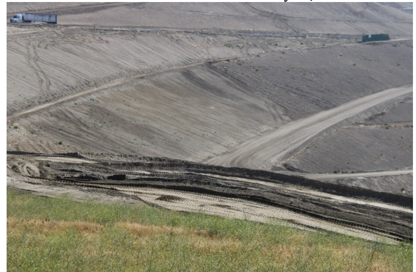
Photo 456: Cell 8 Construction: May 24, 2022
