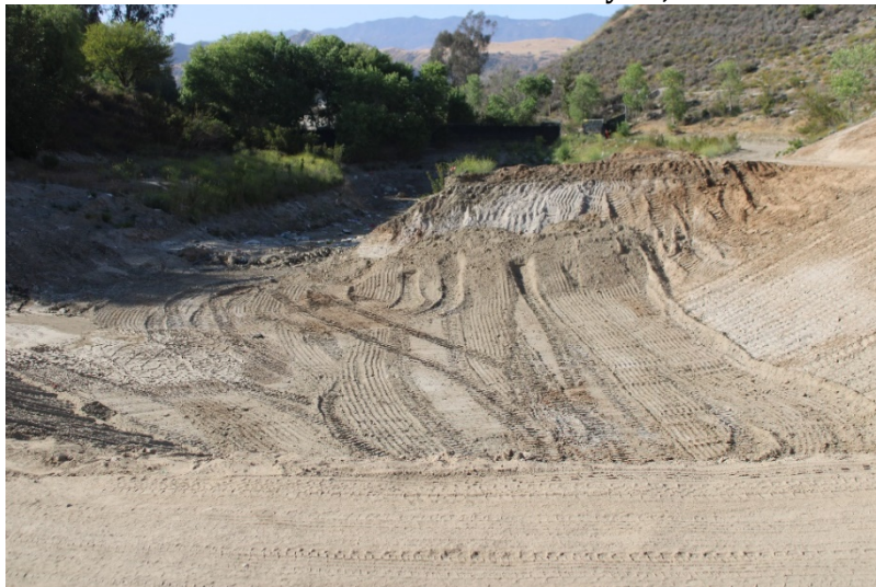
Photo 435: Cell 8 Construction: May 24, 2022
