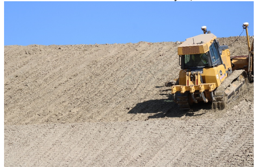
Photo 448: Cell 8 Construction: May 24, 2022
