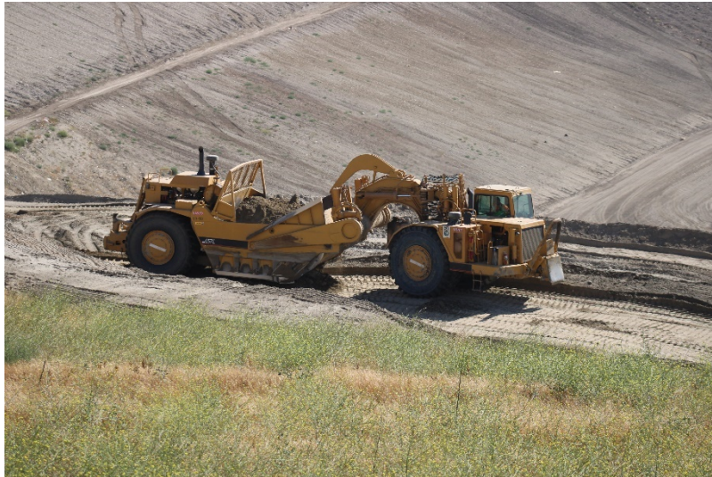
Photo 461: Cell 8 Construction: May 24, 2022
