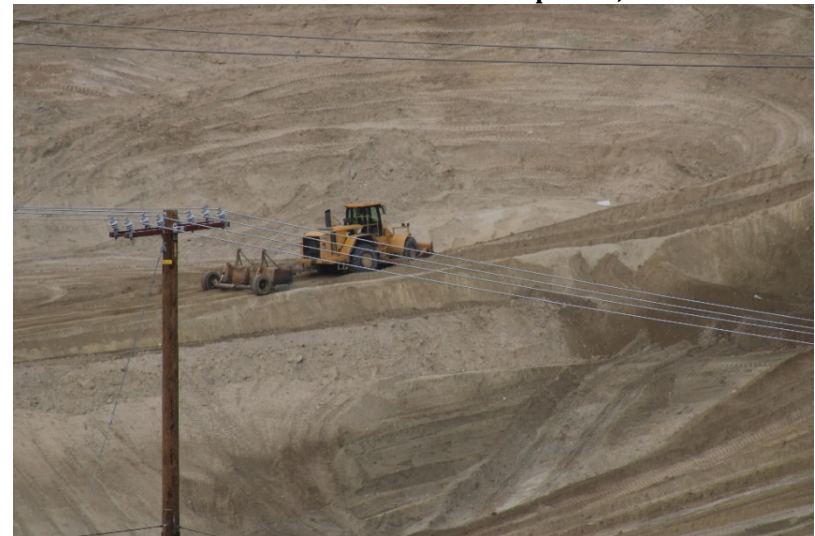
Photo 424: Cell 8 Construction: April 26, 2022
