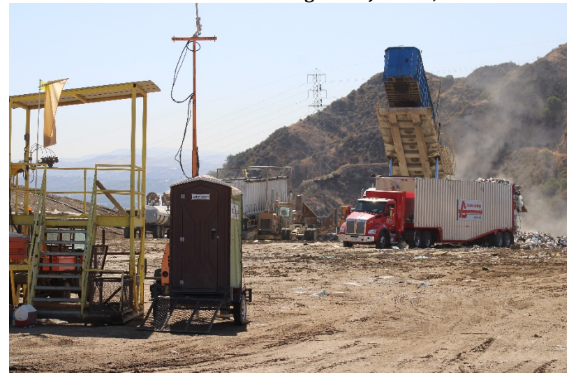
Photo 104: Cell 6 Working Area: June 21, 2022
