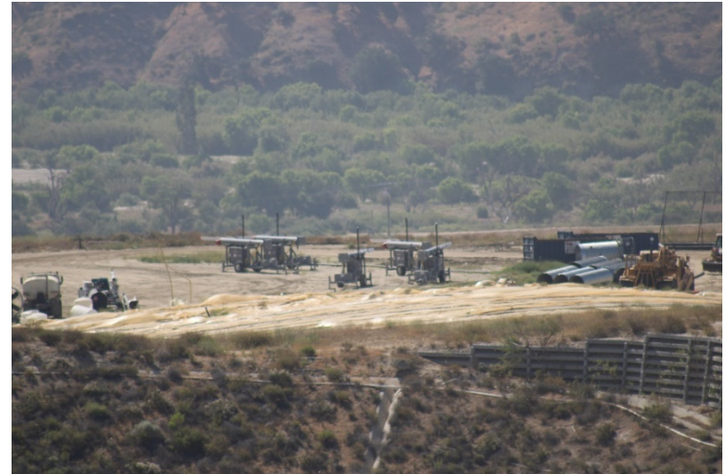
Photo 122: Closed Landfill - Primary Canyon: May 24, 2022
