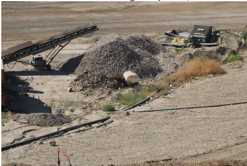
Photo 99: Cell 6 Working Area: June 21, 2022
