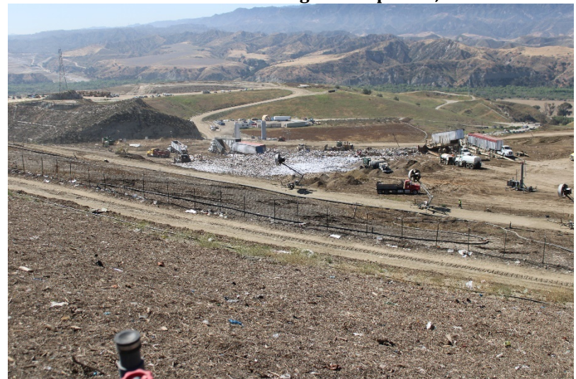
Photo 48: Cell 6 Working Area: May 24, 2022
