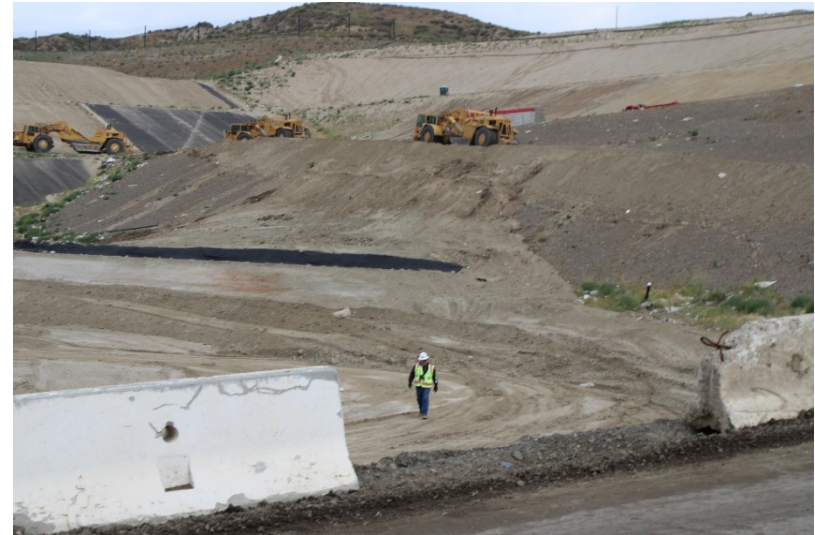
Photo 414: Cell 8 Construction: April 26, 2022
