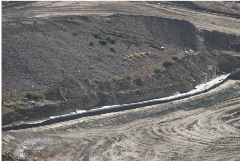
Photo 465: Cell 8 Construction: May 24, 2022
