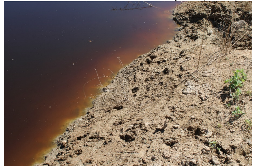
Photo 220: Northeast Sediment Basin: June 21, 2022
