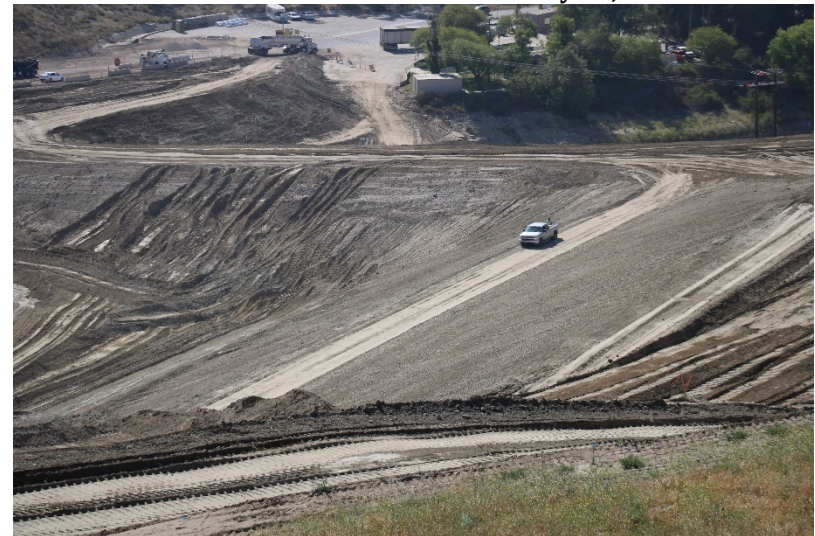
Photo 476: Cell 8 Construction: May 24, 2022
