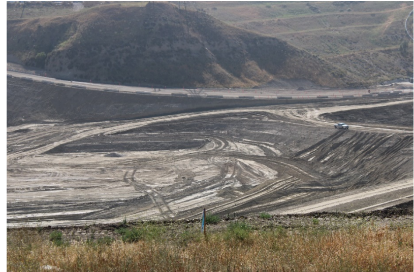
Photo 458: Cell 8 Construction: May 24, 2022
