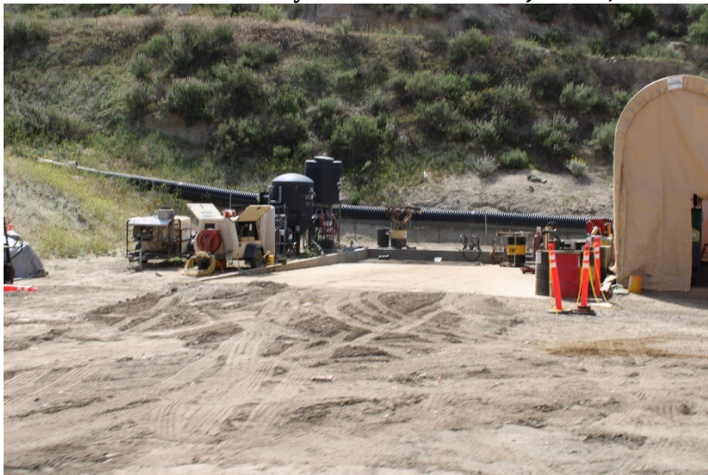
Photo 287: Maintenance and Admin Buildings: April 26, 2022
