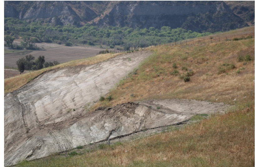
Photo 478: Cell 8 Construction: May 24, 2022
