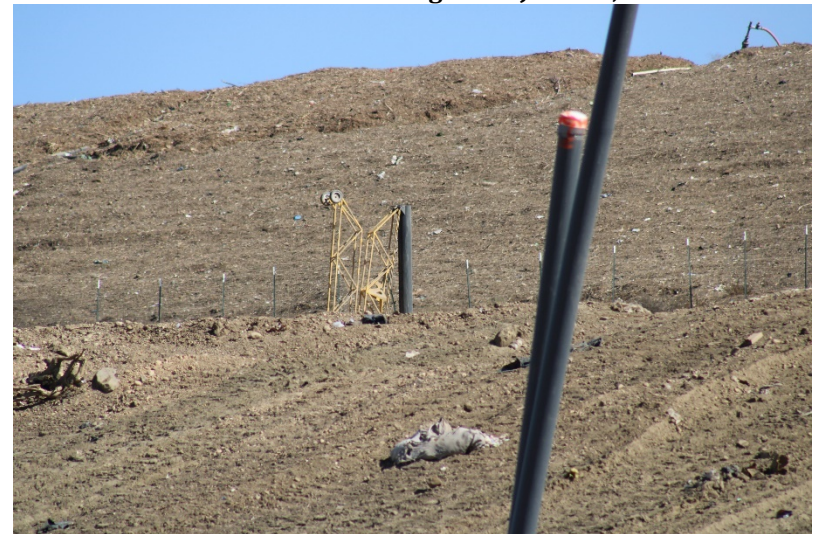
Photo 100: Cell 6 Working Area: June 21, 2022
