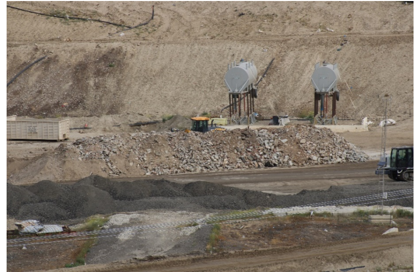
Photo 422: Cell 8 Construction: April 26, 2022
