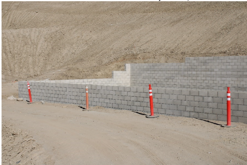
Photo 483: Cell 8 Construction: June 21, 2022
