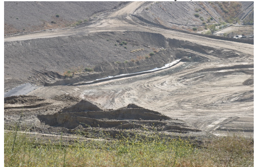
Photo 464: Cell 8 Construction: May 24, 2022
