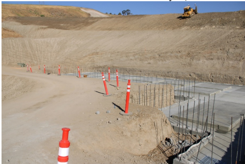
Photo 431: Cell 8 Construction: May 24, 2022
