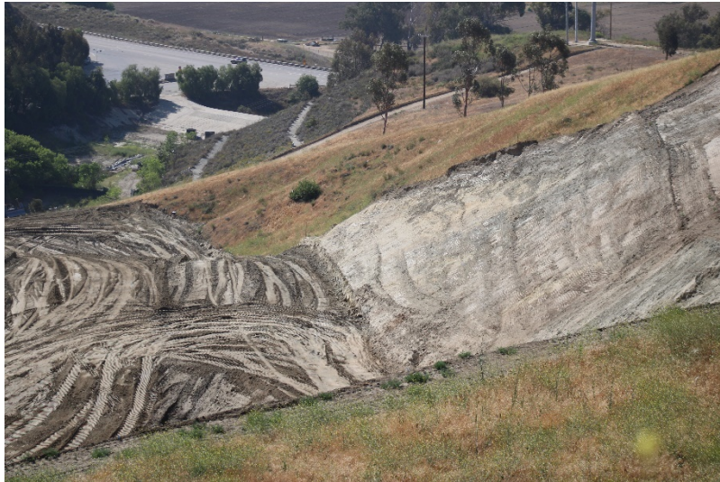
Photo 477: Cell 8 Construction: May 24, 2022
