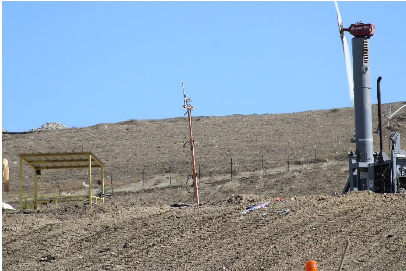
Photo 101: Cell 6 Working Area: June 21, 2022
