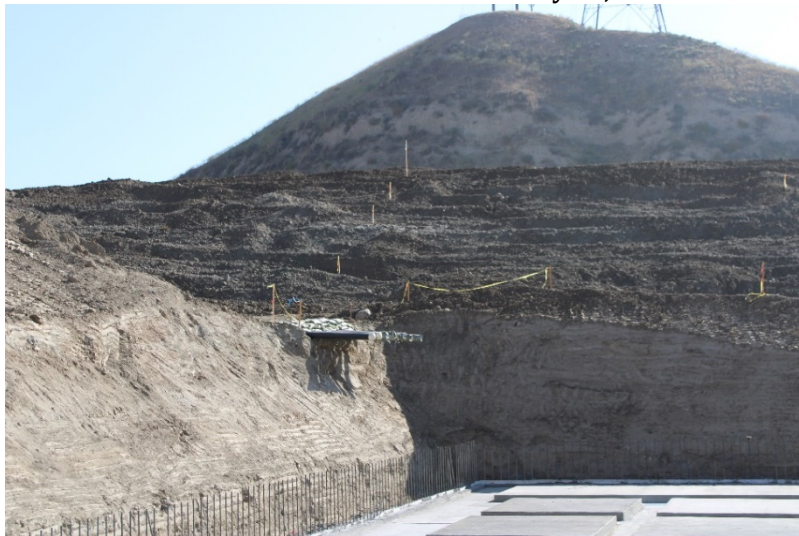
Photo 439: Cell 8 Construction: May 24, 2022
