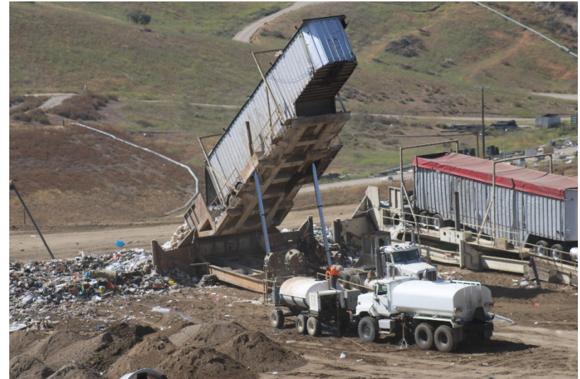
Photo 62: Cell 6 Working Area: May 24, 2022
