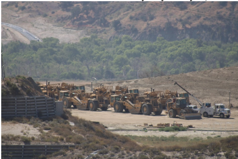
Photo 123: Closed Landfill - Primary Canyon: May 24, 2022
