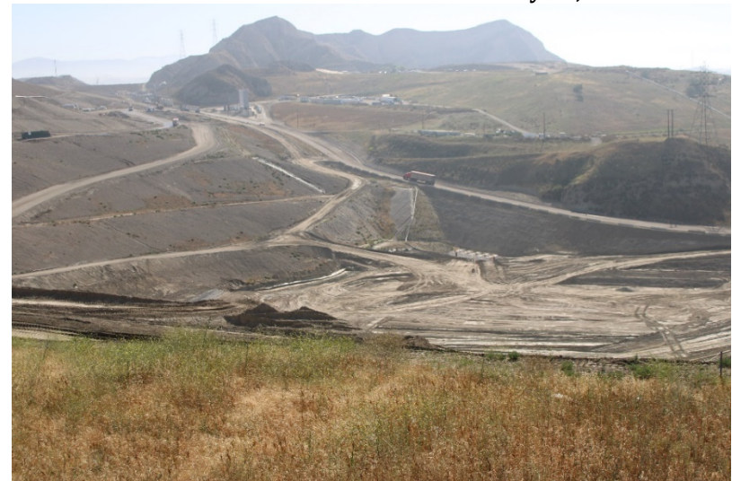
Photo 452: Cell 8 Construction: May 24, 2022
