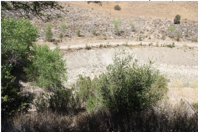
Photo 191: South Terminal and Catch Basins: June 21, 2022
