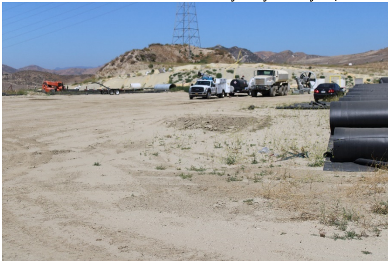
Photo 135: Closed Landfill - Primary Canyon: May 24, 2022
