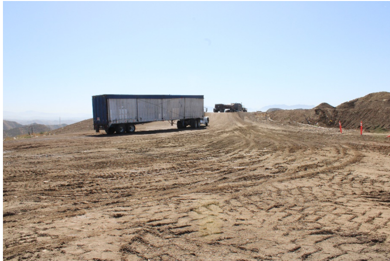
Photo 1: Top Deck Working Area: May 24, 2022
