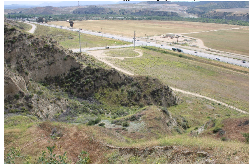
Photo 264: Wolcott Way Entrance Facilities: April 26, 2022
