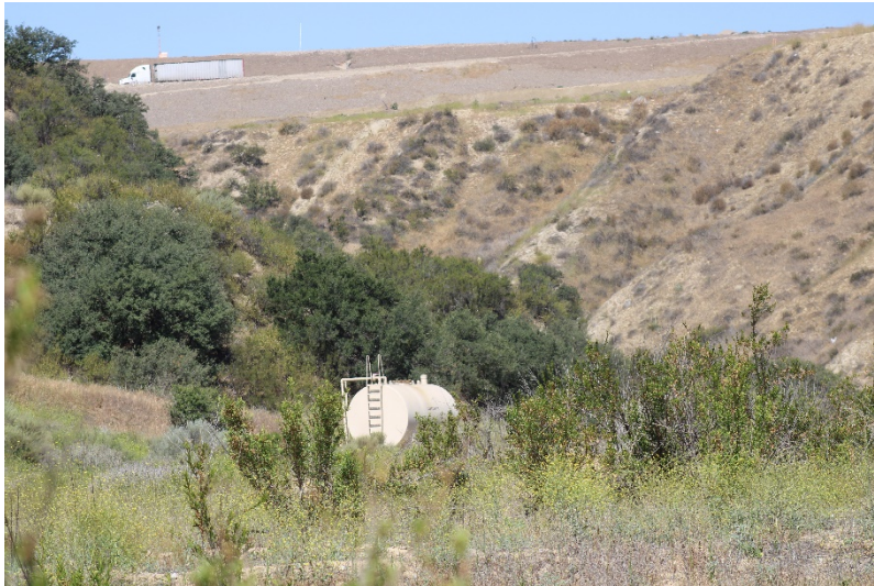
Photo 149: Closed Landfill - Canyon B: May 24, 2022
