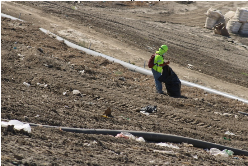
Photo 95: Cell 6 Working Area: June 21, 2022
