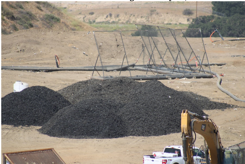
Photo 71: Cell 6 Working Area: May 24, 2022
