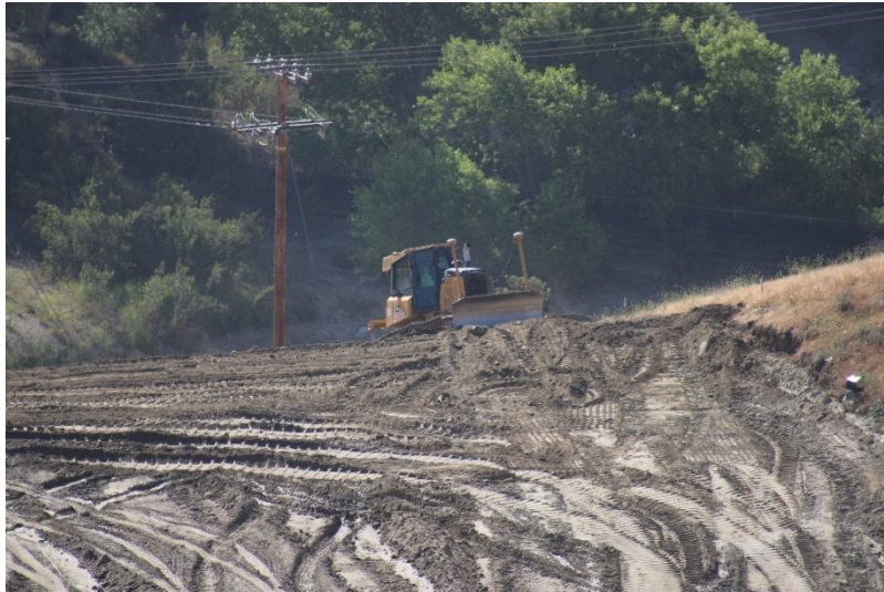
Photo 469: Cell 8 Construction: May 24, 2022
