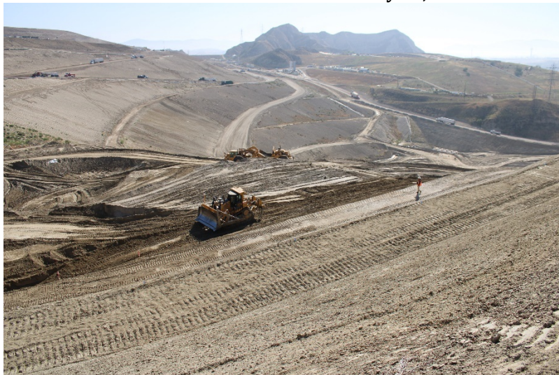
Photo 471: Cell 8 Construction: May 24, 2022
