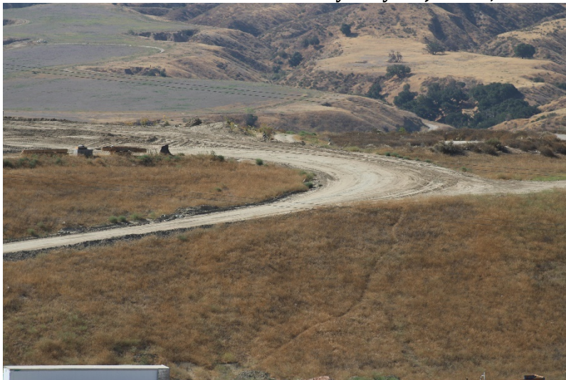
Photo 139: Closed Landfill - Primary Canyon: June 21, 2022
