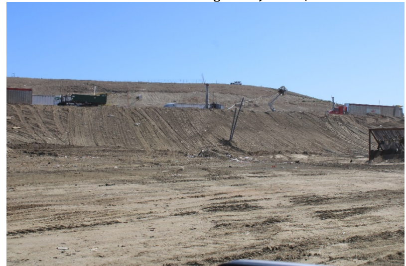
Photo 84: Cell 6 Working Area: June 21, 2022
