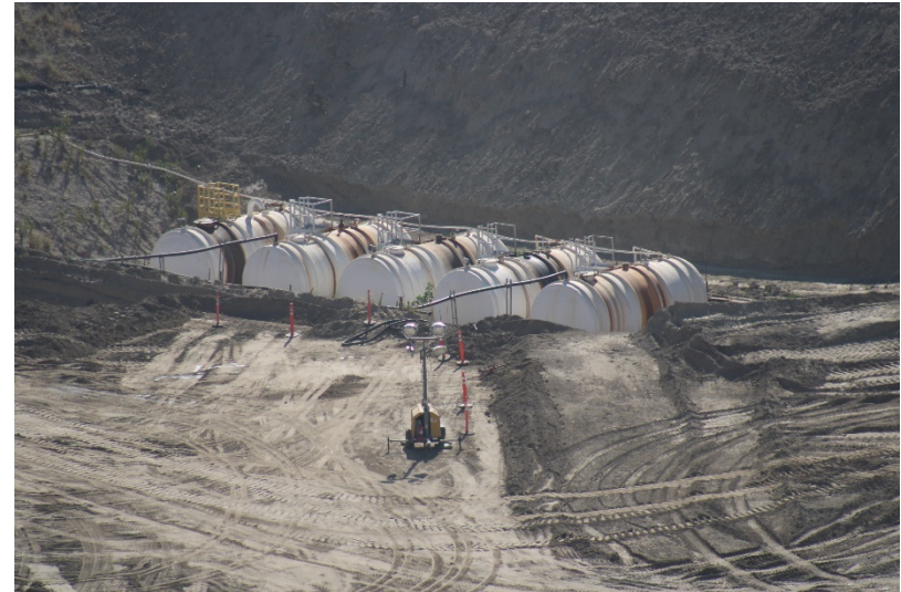
Photo 466: Cell 8 Construction: May 24, 2022
