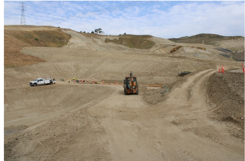
Photo 410: Cell 8 Construction: April 26, 2022
