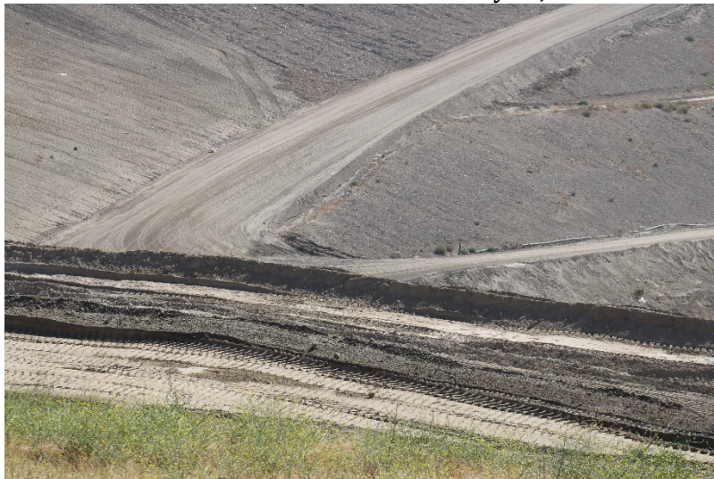
Photo 463: Cell 8 Construction: May 24, 2022
