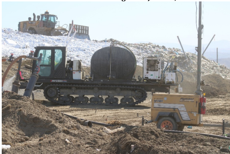
Photo 91: Cell 6 Working Area: June 21, 2022
