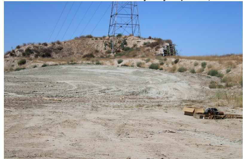
Photo 140: Closed Landfill - Primary Canyon: June 21, 2022
