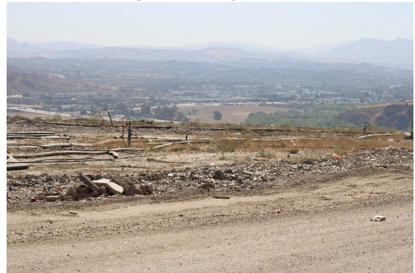
Photo 20: Top Deck Working Area: June 21, 2022
