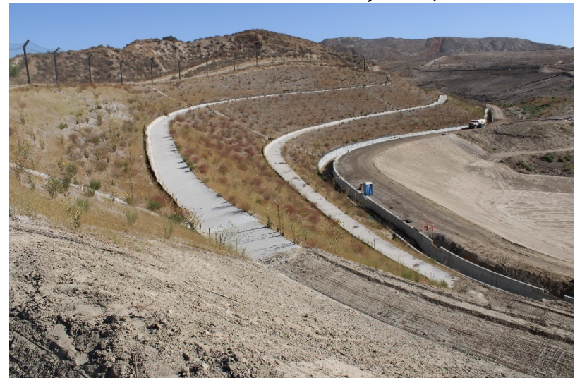
Photo 488: Cell 8 Construction: June 21, 2022
