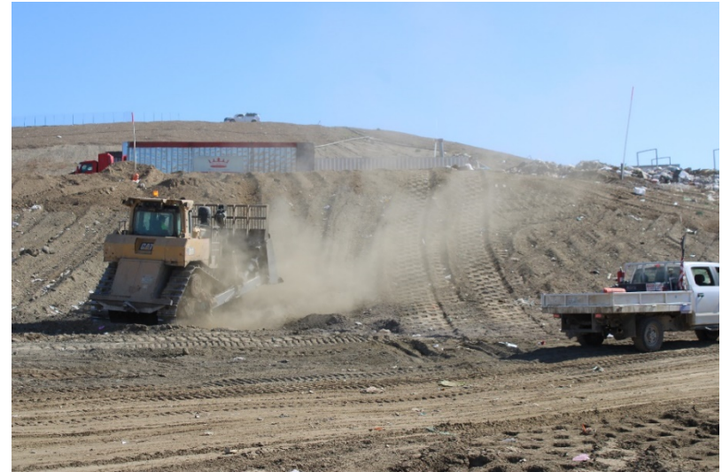
Photo 86: Cell 6 Working Area: June 21, 2022
