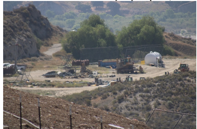
Photo 120: Closed Landfill - Primary Canyon: May 24, 2022
