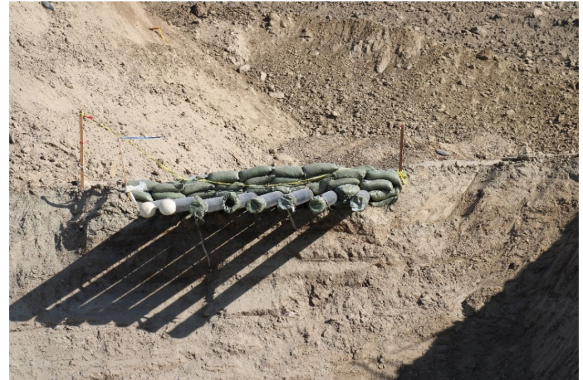
Photo 442: Cell 8 Construction: May 24, 2022
