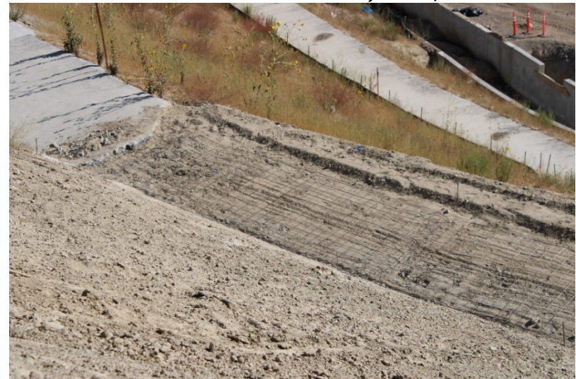
Photo 492: Cell 8 Construction: June 21, 2022
