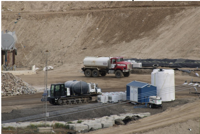
Photo 423: Cell 8 Construction: April 26, 2022
