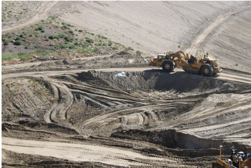
Photo 473: Cell 8 Construction: May 24, 2022
