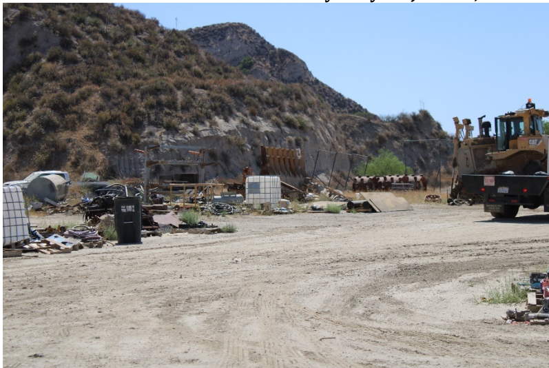
Photo 143: Closed Landfill - Primary Canyon: June 21, 2022
