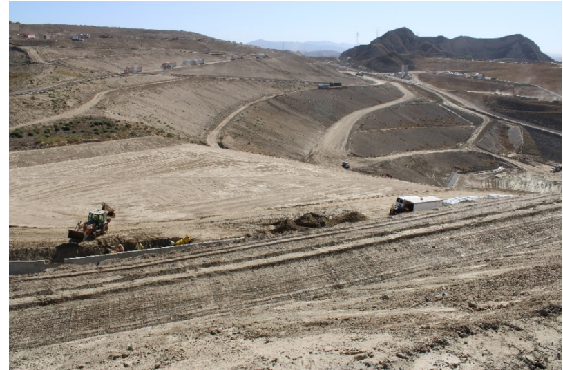
Photo 490: Cell 8 Construction: June 21, 2022
