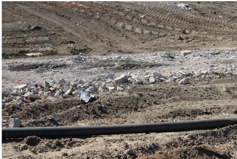
Photo 3: Top Deck Working Area: May 24, 2022
