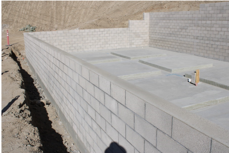
Photo 485: Cell 8 Construction: June 21, 2022
