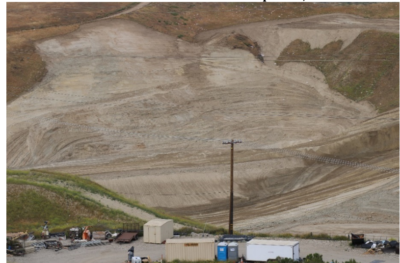
Photo 416: Cell 8 Construction: April 26, 2022
