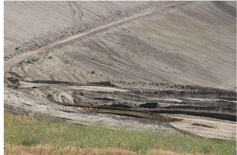
Photo 462: Cell 8 Construction: May 24, 2022
