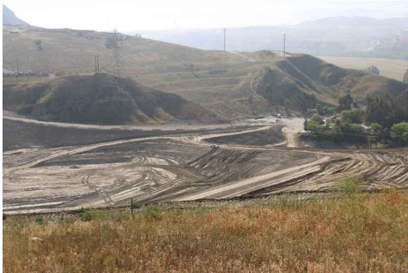
Photo 453: Cell 8 Construction: May 24, 2022
