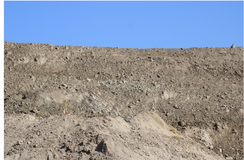
Photo 450: Site: Cell 8 Construction: May 24, 2022
