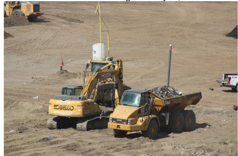
Photo 68: Cell 6 Working Area: May 24, 2022
