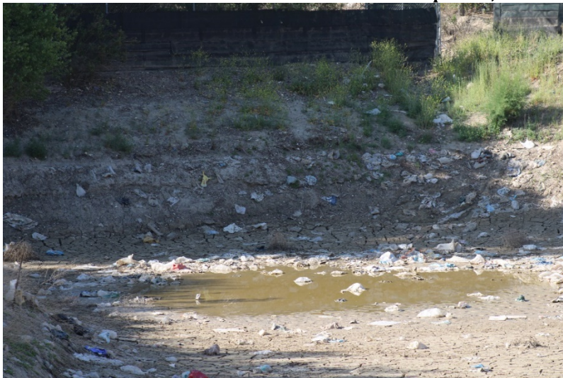
Photo 179: South Terminal and Catch Basins: May 24, 2022
