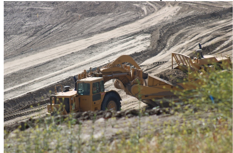
Photo 468: Cell 8 Construction: May 24, 2022
