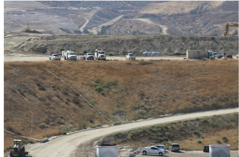
Photo 138: Closed Landfill - Primary Canyon: June 21, 2022
