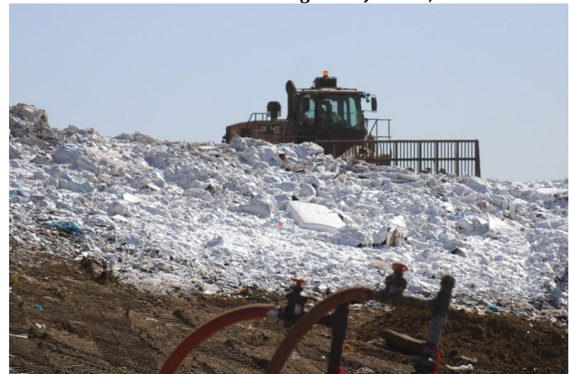
Photo 92: Cell 6 Working Area: June 21, 2022
