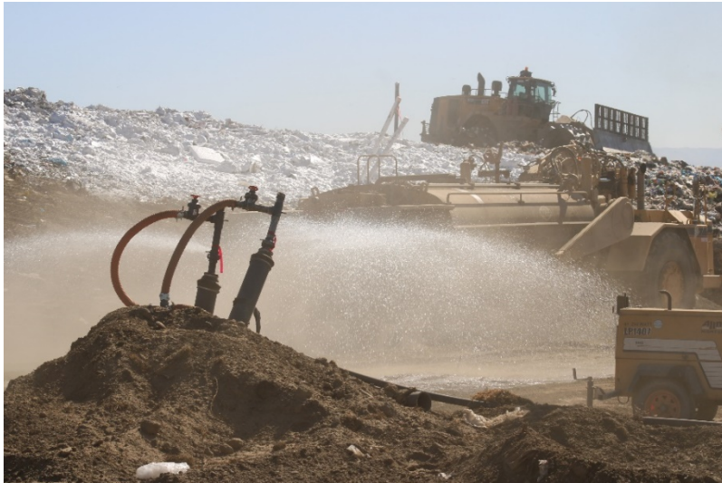
Photo 93: Cell 6 Working Area: June 21, 2022
