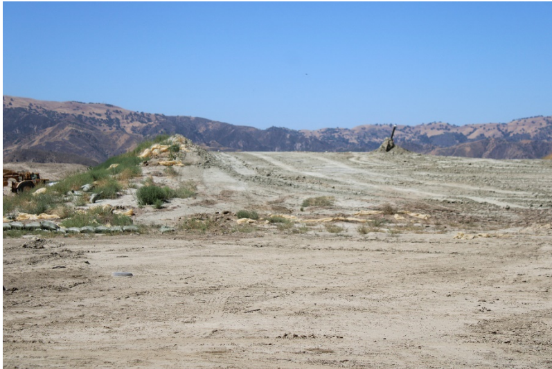
Photo 141: Closed Landfill - Primary Canyon: June 21, 2022
