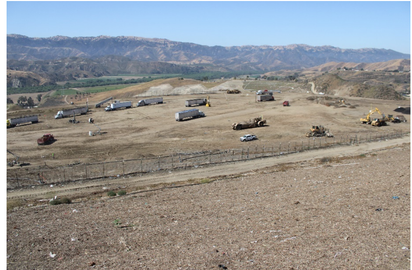
Photo 50: Cell 6 Working Area: May 24, 2022
