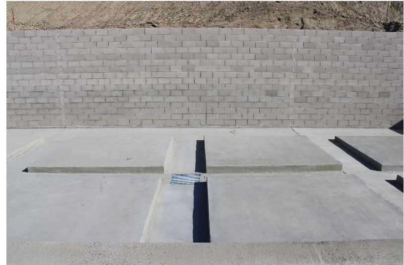
Photo 486: Cell 8 Construction: June 21, 2022
