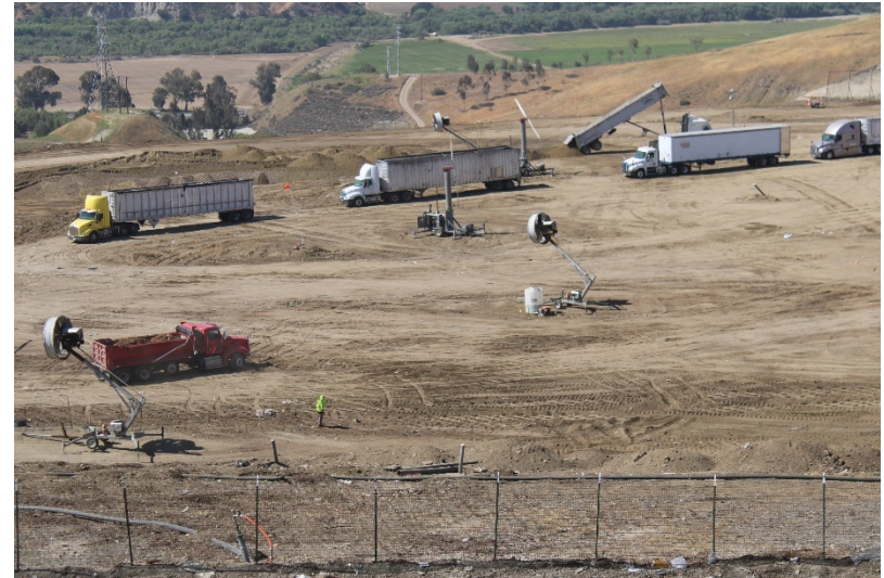
Photo 54: Cell 6 Working Area: May 24, 2022
