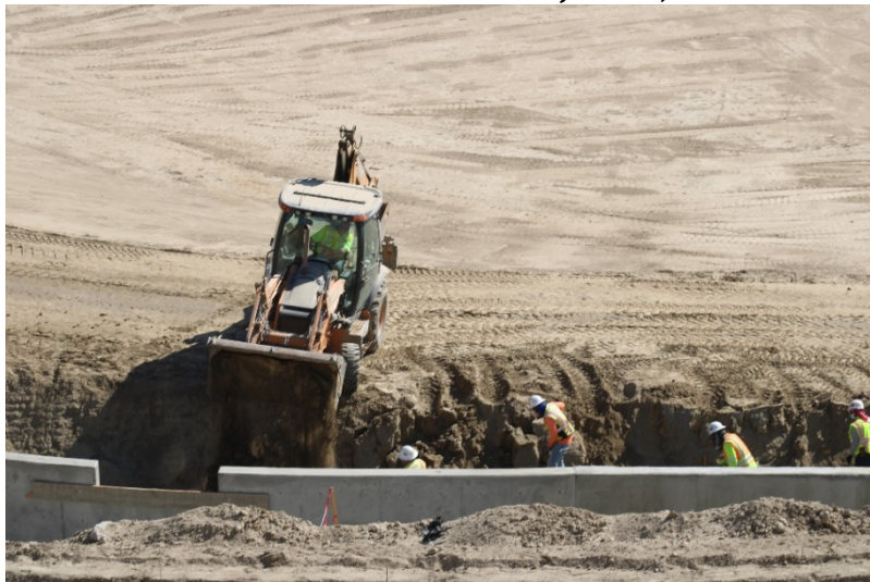
Photo 503: Cell 8 Construction: June 21, 2022
