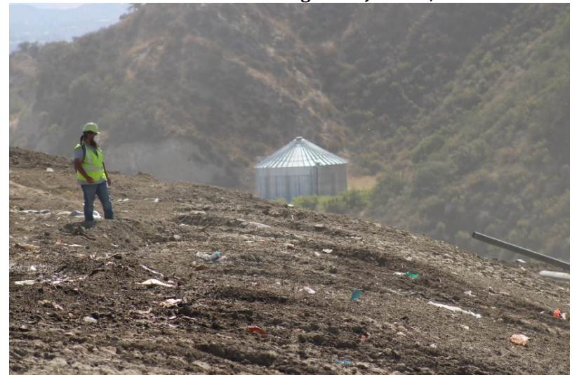
Photo 96: Cell 6 Working Area: June 21, 2022
