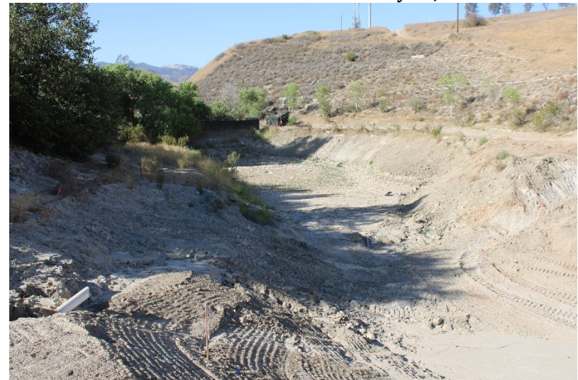
Photo 480: Cell 8 Construction: June 21, 2022
