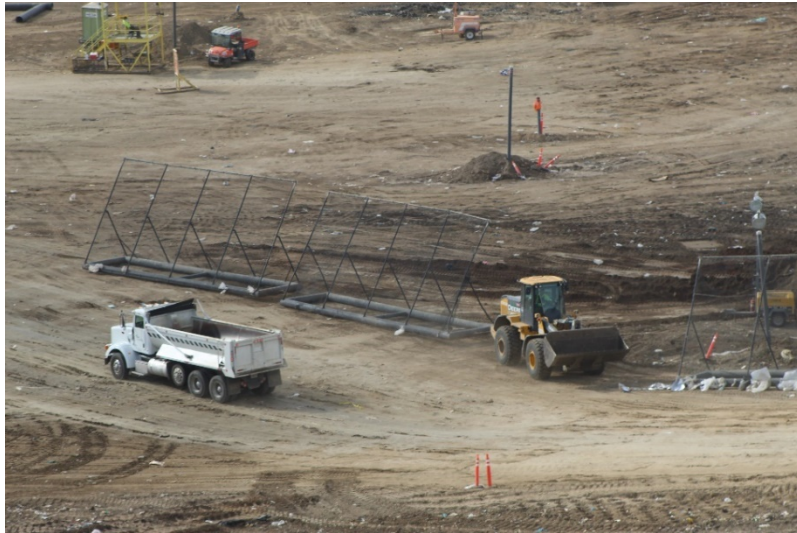
Photo 29: Cell 6 Working Area: February 22, 2022
