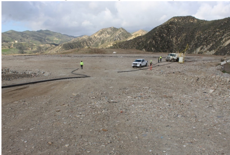
Photo 7: Top Deck Working Area: February 22, 2022
