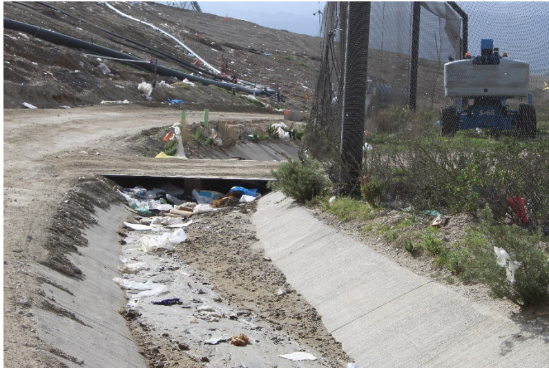
Photo 157: Site: February 22, 2022 February 22, 2022
