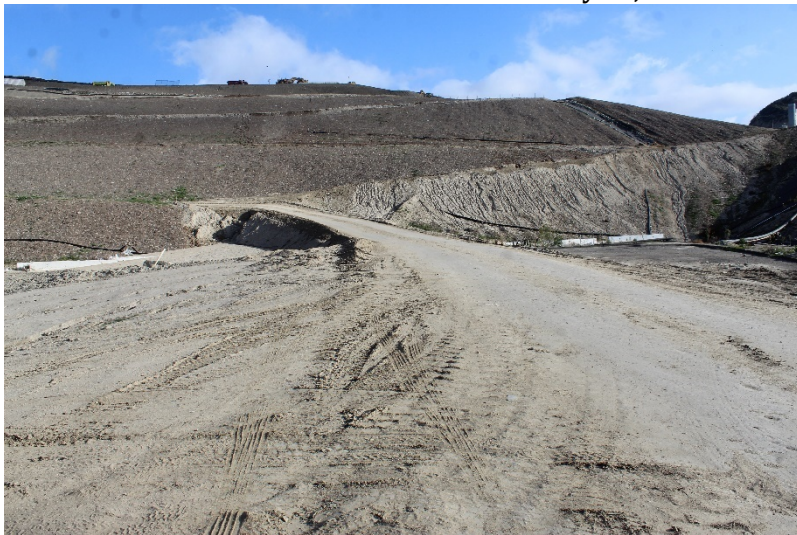
Photo 295: Cell 8 Construction: February 22, 2022
