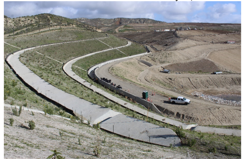
Photo 308: Cell 8 Construction: February 22, 2022
