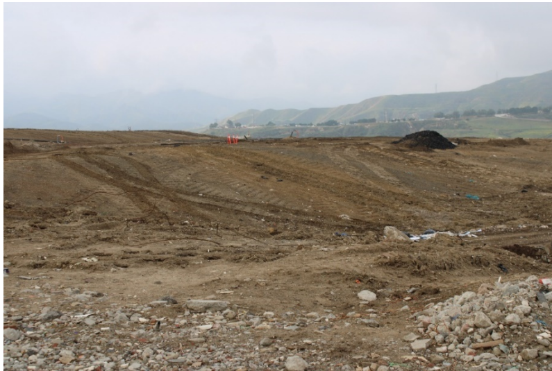
Photo 21: Top Deck Working Area: March 31, 2022
