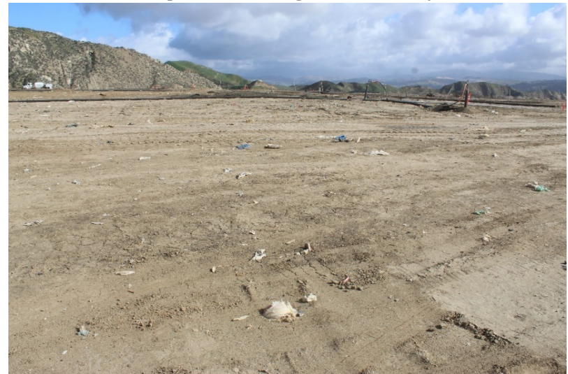
Photo 12: Top Deck Working Area: February 22, 2022
