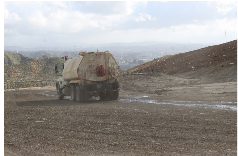
Photo 8: Top Deck Working Area: February 22, 2022
