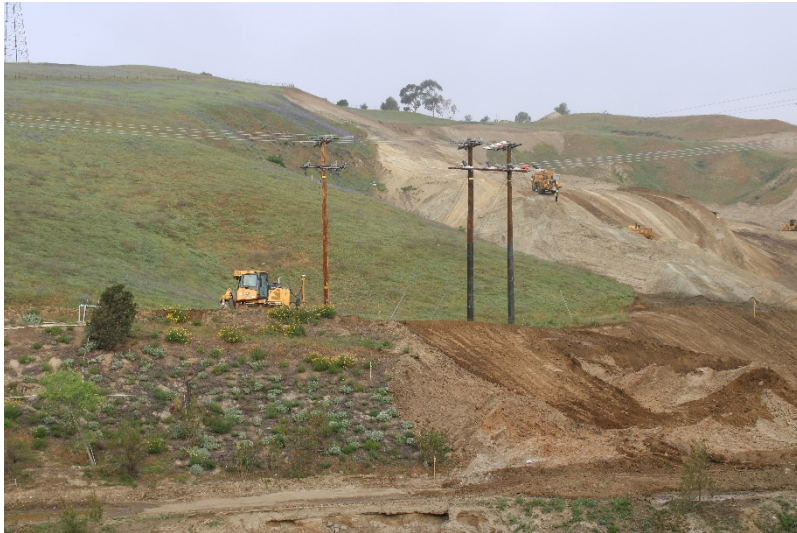
Photo 313: Cell 8 Construction: March 31, 2022
