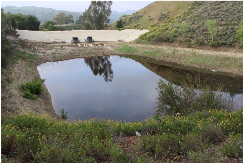
Photo 145: South Terminal and Catch Basins: March 31, 2022
