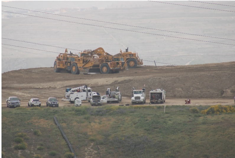
Photo 77: Closed Landfill - Primary Canyon: March 31, 2022
