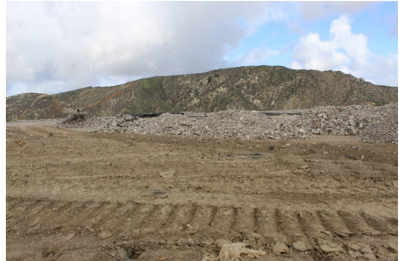
Photo 34: Cell 6 Working Area: February 22, 2022
