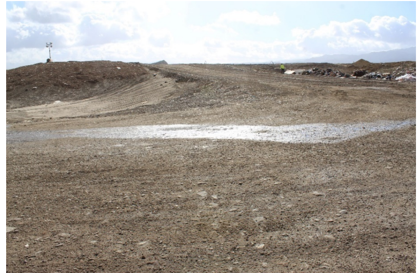
Photo 2: Top Deck Working Area: February 22, 2022
