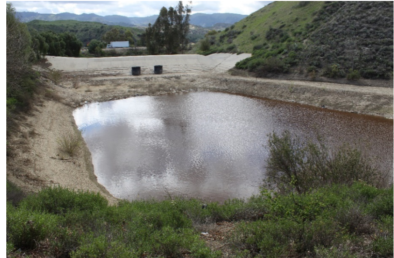
Photo 130: South Terminal and Catch Basins: February 22, 2022
