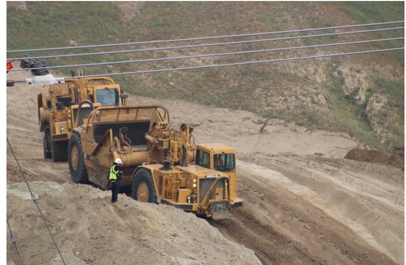
Photo 322: Cell 8 Construction: March 31, 2022
