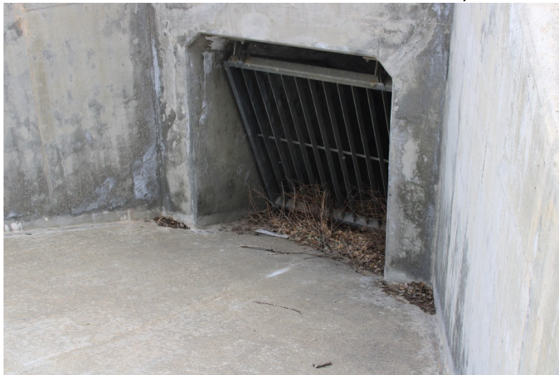
Photo 155: Northeast Sediment Basin: March 31, 2022
