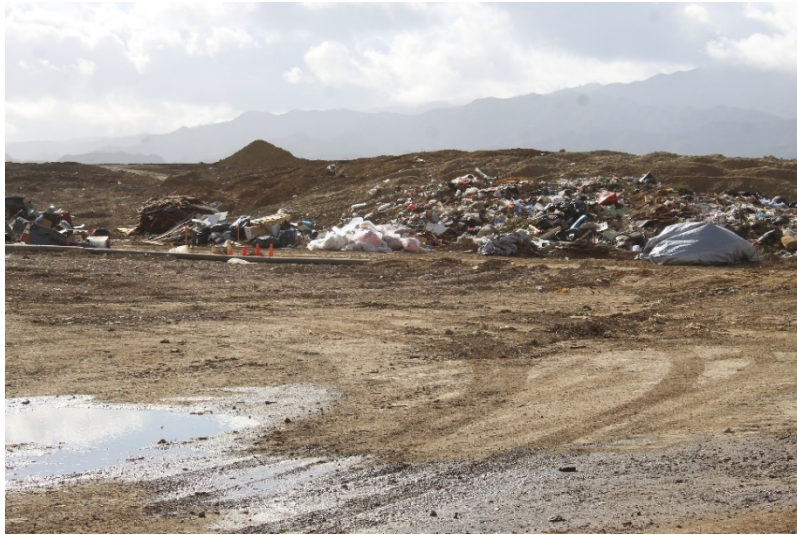
Photo 9: Top Deck Working Area: February 22, 2022
