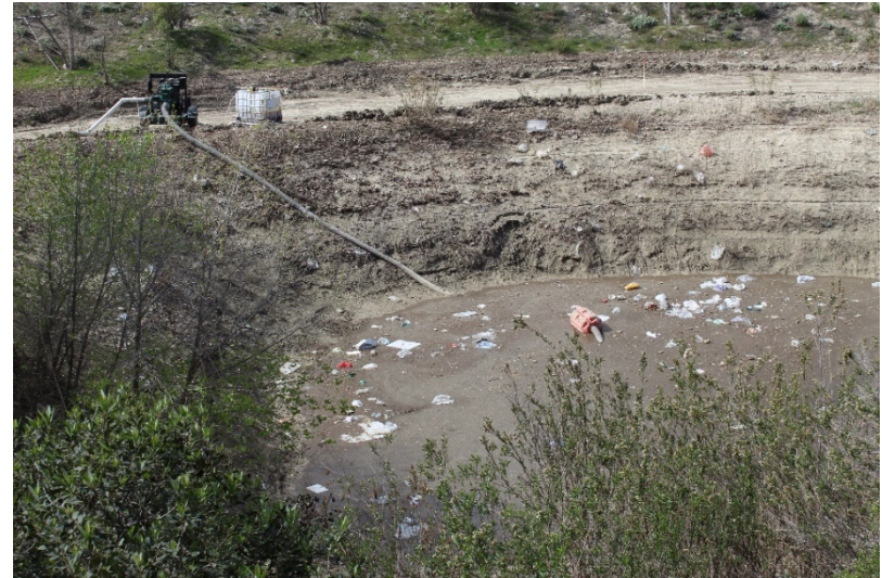
Photo 134: South Terminal and Catch Basins: February 22, 2022
