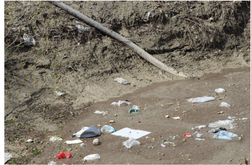
Photo 138: South Terminal and Catch Basins: February 22, 2022
