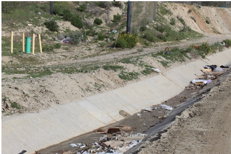
Photo 159: Site: February 22, 2022 February 22, 2022
