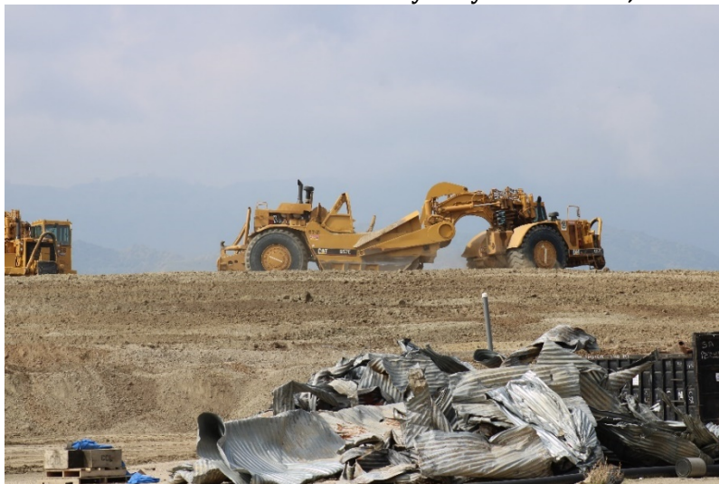
Photo 91: Closed Landfill – Primary Canyon: March 31, 2022
