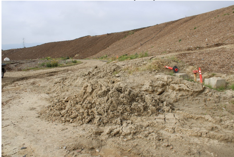
Photo 79: Closed Landfill - Primary Canyon: March 31, 2022
