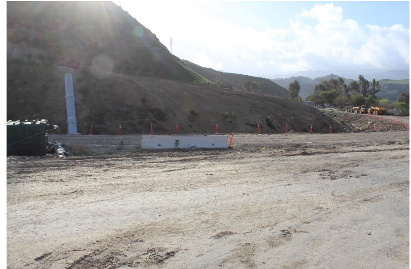
Photo 298: Cell 8 Construction: February 22, 2022
