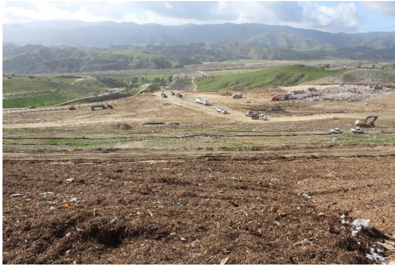
Photo 17: Top Deck Working Area: February 22, 2022
