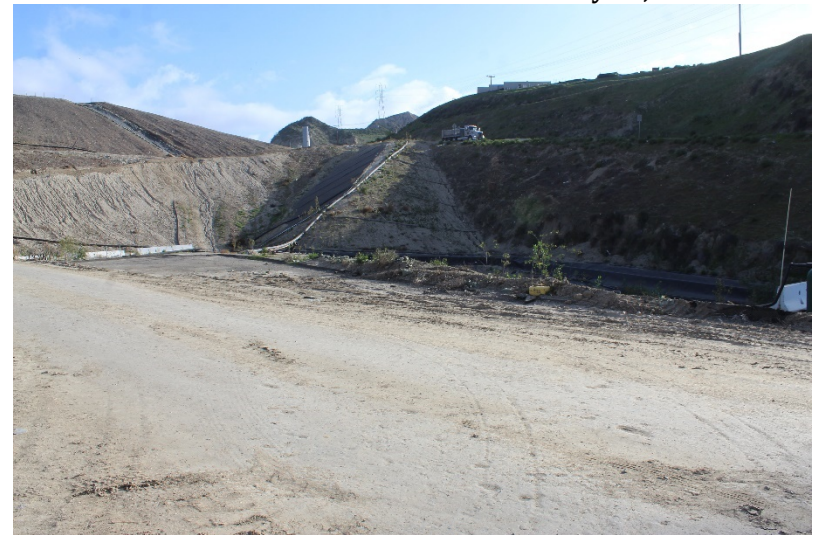
Photo 296: Cell 8 Construction: February 22, 2022
