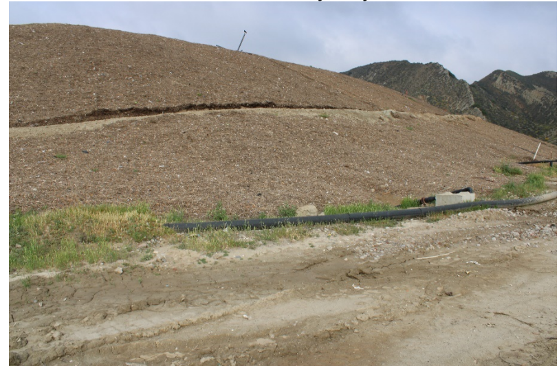
Photo 80: Closed Landfill - Primary Canyon: March 31, 2022
