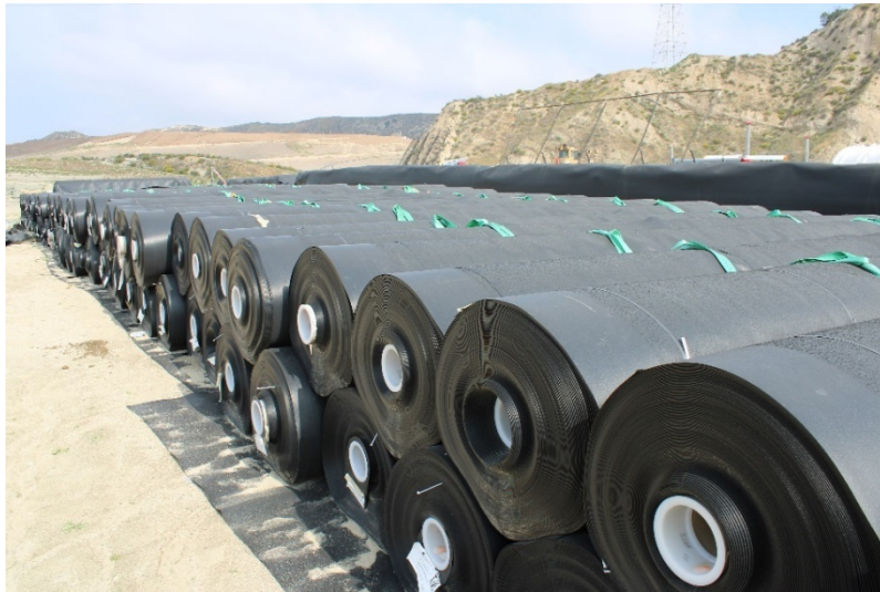
Photo 89: Closed Landfill – Primary Canyon: March 31, 2022
