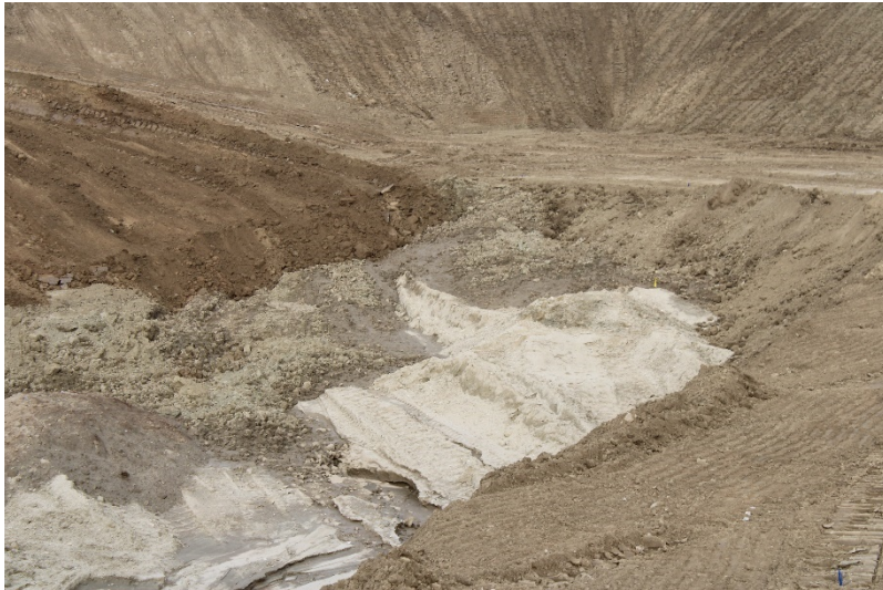
Photo 333: Cell 8 Construction: March 31, 2022
