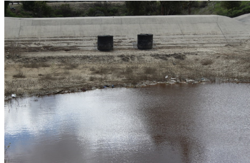
Photo 132: South Terminal and Catch Basins: February 22, 2022
