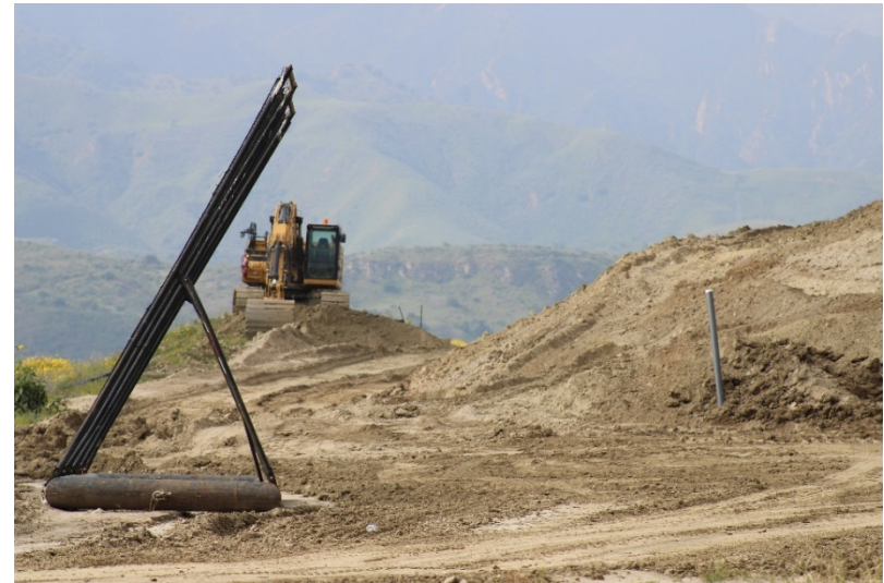
Photo 86: Closed Landfill – Primary Canyon: March 31, 2022
