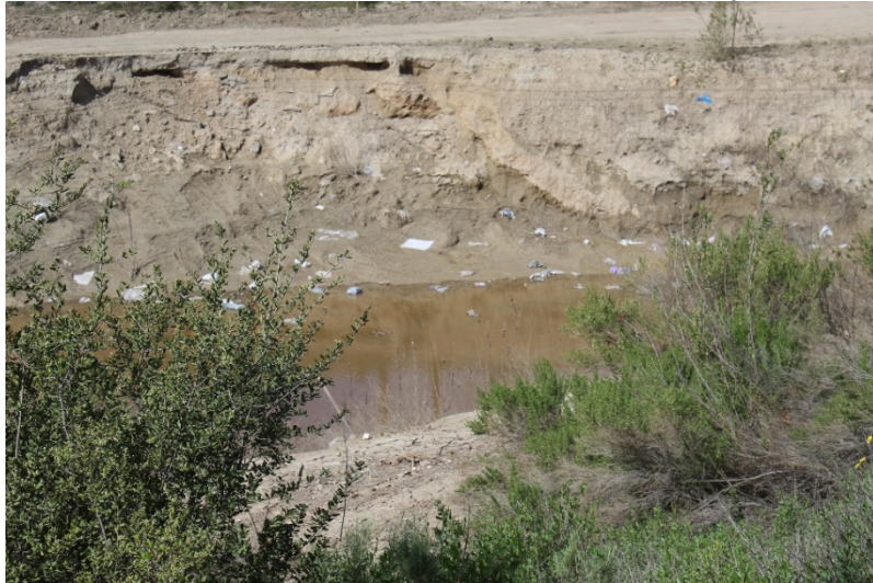
Photo 135: South Terminal and Catch Basins: February 22, 2022
