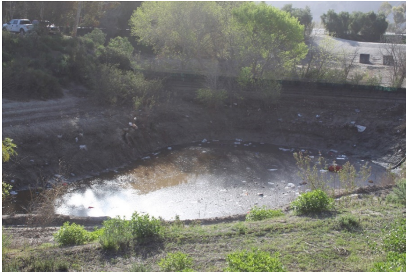
Photo 121: South Terminal and Catch Basins: February 22, 2022
