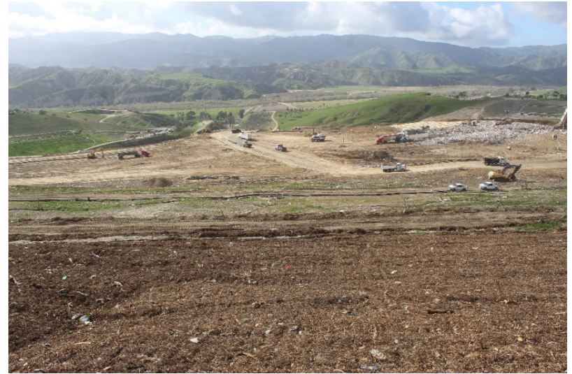
Photo 18: Top Deck Working Area: February 22, 2022
