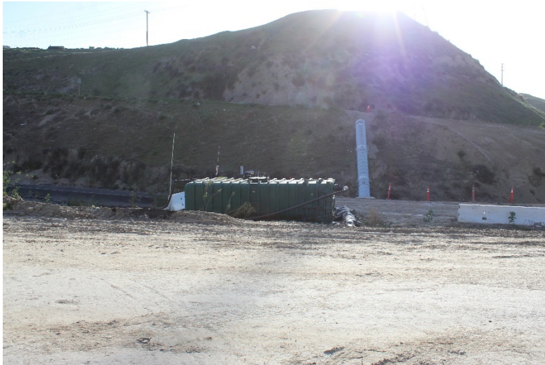
Photo 297: Cell 8 Construction: February 22, 2022
