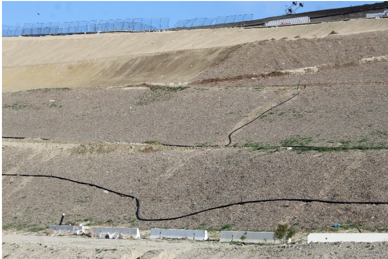
Photo 301: Cell 8 Construction: February 22, 2022
