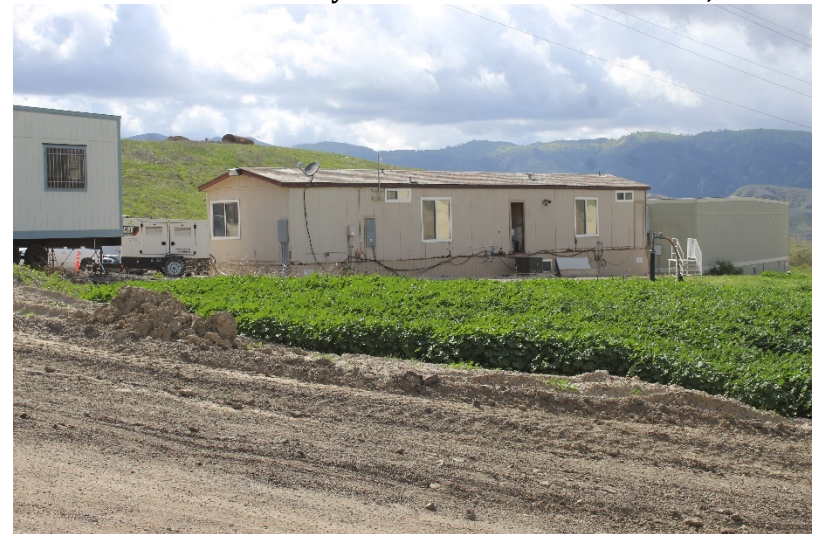
Photo 200: Maintenance and Admin Buildings: February 22, 2022
