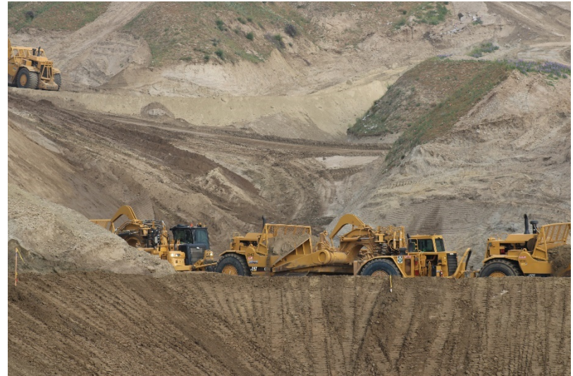
Photo 318: Cell 8 Construction: March 31, 2022
