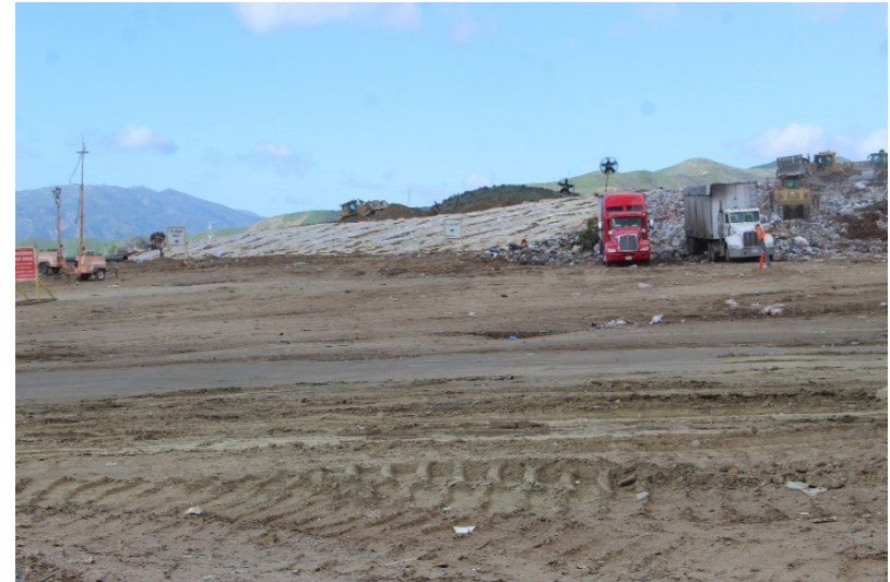
Photo 38: Cell 6 Working Area: February 22, 2022
