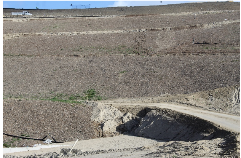
Photo 302: Cell 8 Construction: February 22, 2022
