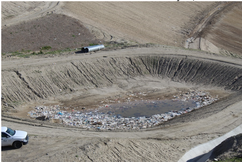
Photo 311: Cell 8 Construction: February 22, 2022
