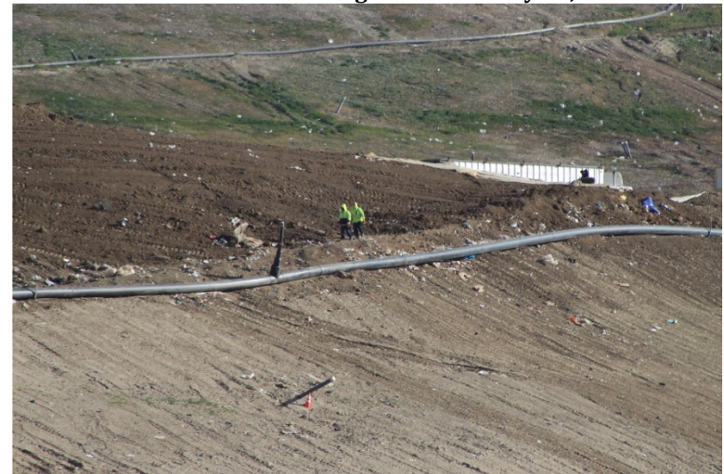
Photo 28: Cell 6 Working Area: February 22, 2022
