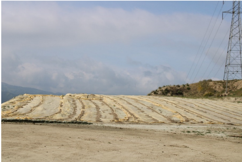
Photo 81: Closed Landfill – Primary Canyon: March 31, 2022
