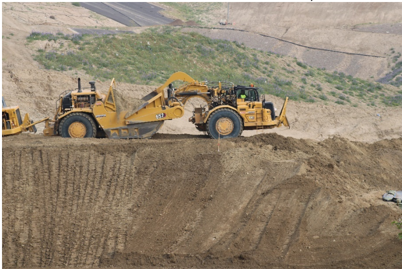
Photo 319: Cell 8 Construction: March 31, 2022
