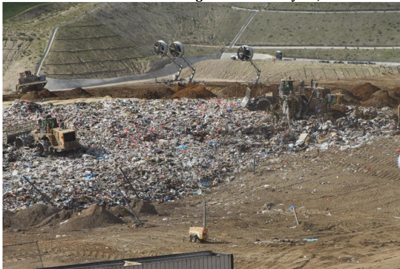
Photo 31: Cell 6 Working Area: February 22, 2022
