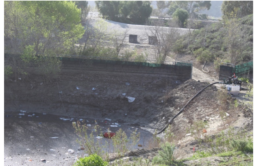
Photo 122: South Terminal and Catch Basins: February 22, 2022
