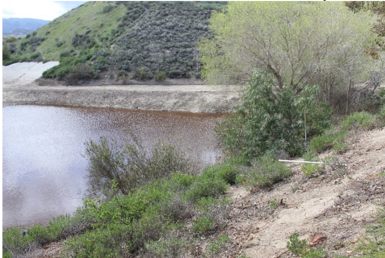
Photo 131: South Terminal and Catch Basins: February 22, 2022
