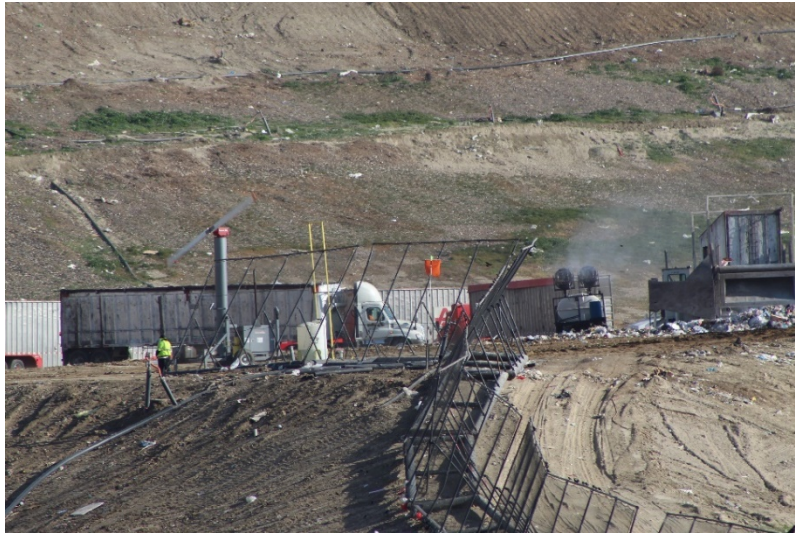
Photo 25: Cell 6 Working Area: February 22, 2022
