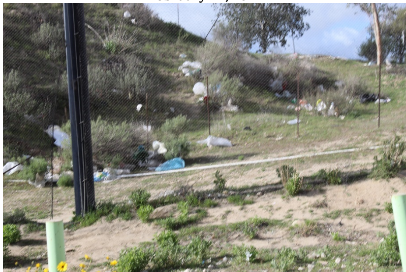
Photo 163: Westside Perimeter Drainage: February 22, 2022
