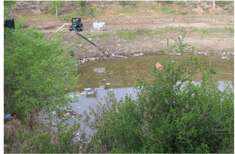
Photo 142: South Terminal and Catch Basins: March 31, 2022
