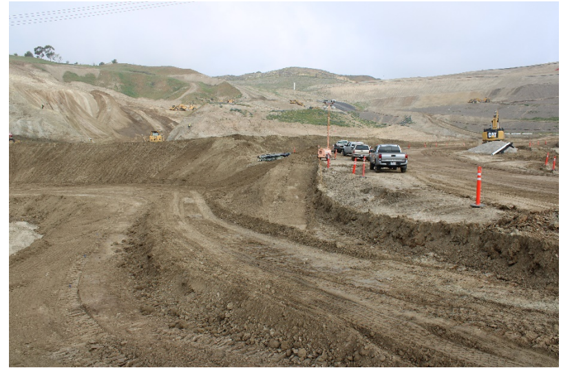
Photo 330: Cell 8 Construction: March 31, 2022
