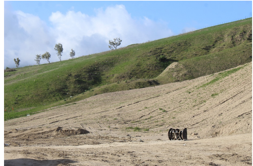
Photo 306: Cell 8 Construction: February 22, 2022
