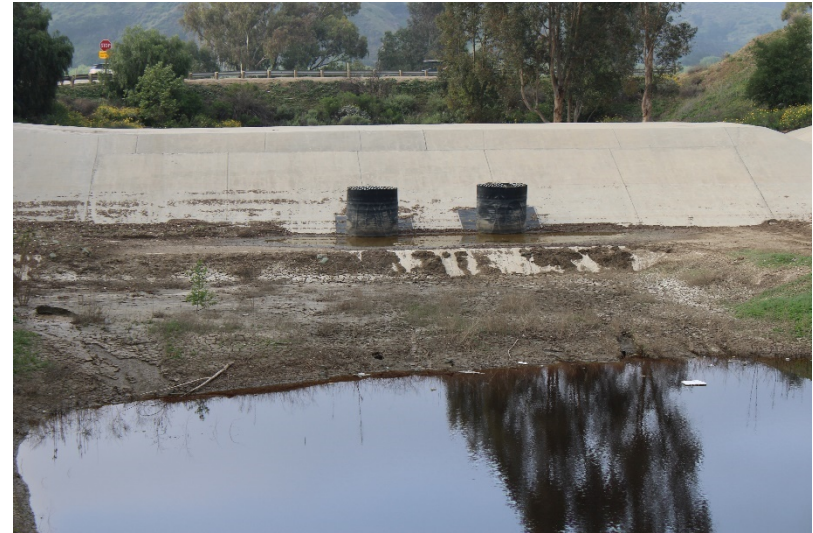
Photo 146: South Terminal and Catch Basins: March 31, 2022
