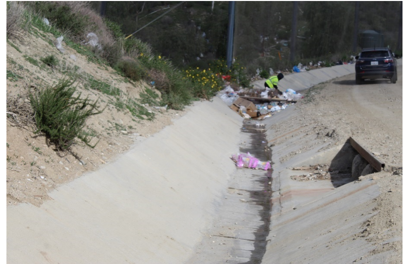
Photo 162: Site: February 22, 2022 February 22, 2022
