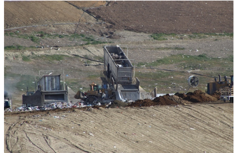
Photo 26: Cell 6 Working Area: February 22, 2022
