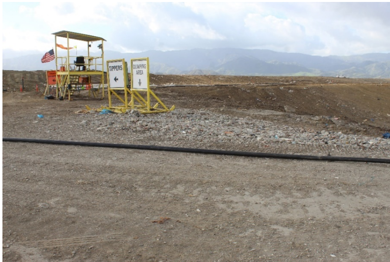
Photo 5: Top Deck Working Area: February 22, 2022
