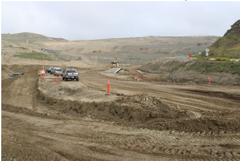
Photo 331: Cell 8 Construction: March 31, 2022
