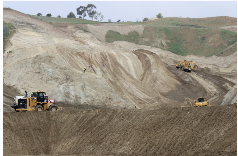
Photo 334: Cell 8 Construction: March 31, 2022
