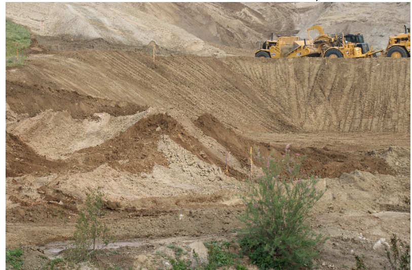
Photo 320: Cell 8 Construction: March 31, 2022
