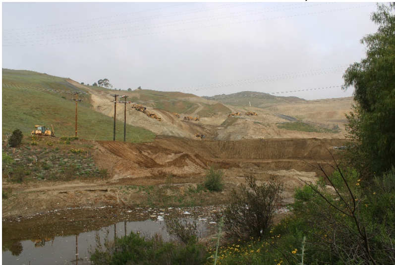
Photo 315: Cell 8 Construction: March 31, 2022
