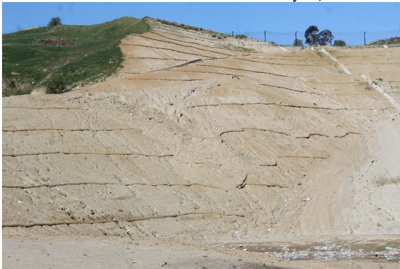
Photo 299: Cell 8 Construction: February 22, 2022
