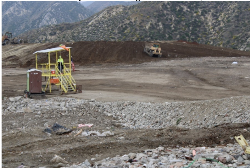
Photo 23: Top Deck Working Area: March 31, 2022
