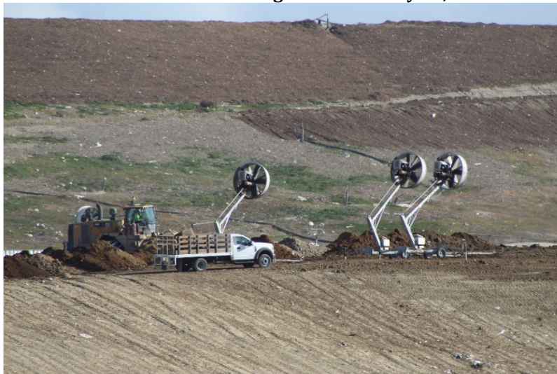
Photo 27: Cell 6 Working Area: February 22, 2022
