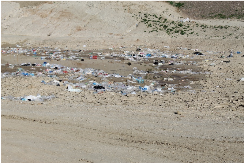
Photo 305: Cell 8 Construction: February 22, 2022
