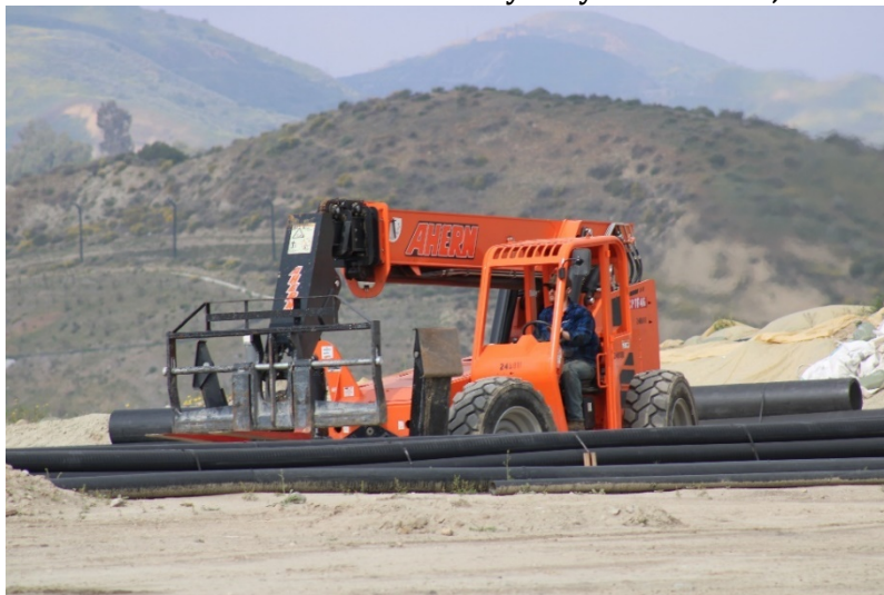
Photo 87: Closed Landfill – Primary Canyon: March 31, 2022
