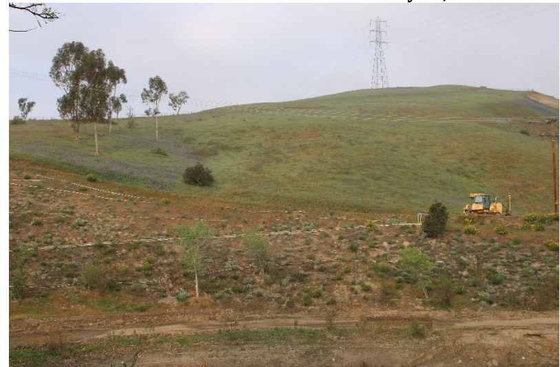
Photo 312: Cell 8 Construction: March 31, 2022
