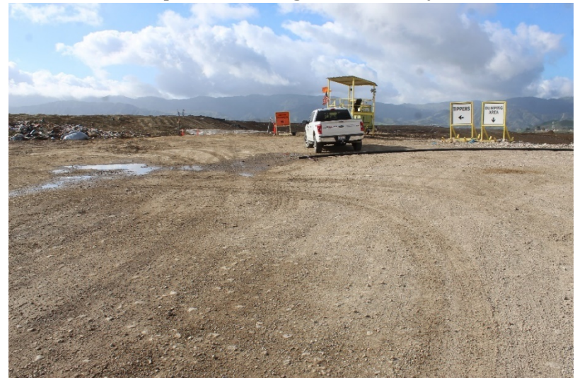
Photo 4: Top Deck Working Area: February 22, 2022
