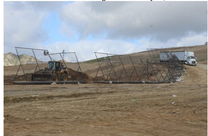
Photo 40: Cell 6 Working Area: February 22, 2022
