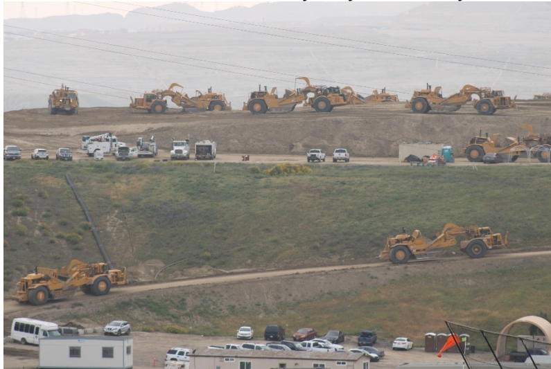
Photo 75: Closed Landfill - Primary Canyon: March 31, 2022
