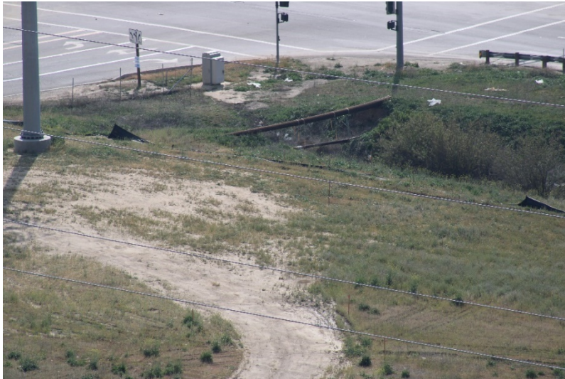
Photo 193: Wolcott Way Entrance Facilities: March 31, 2022
