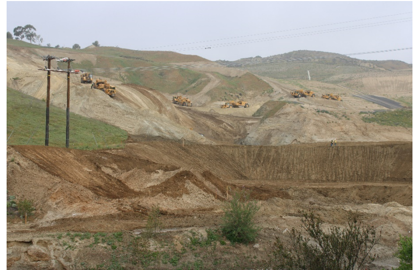
Photo 314: Cell 8 Construction: March 31, 2022
