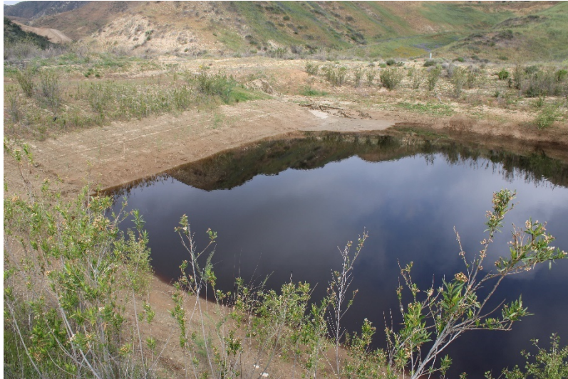
Photo 149: Northeast Sediment Basin: March 31, 2022
