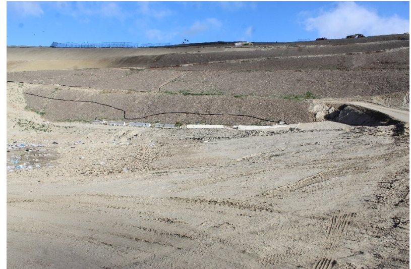
Photo 294: Cell 8 Construction: February 22, 2022
