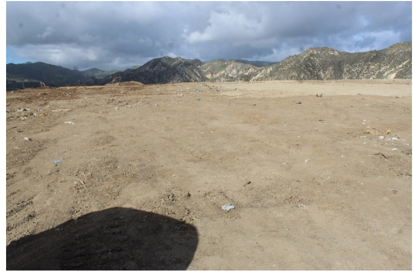
Photo 10: Top Deck Working Area: February 22, 2022
