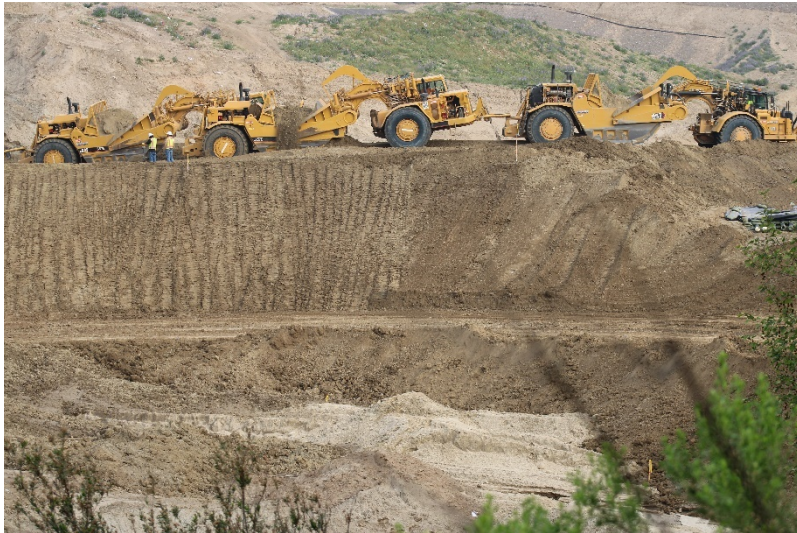
Photo 321: Cell 8 Construction: March 31, 2022
