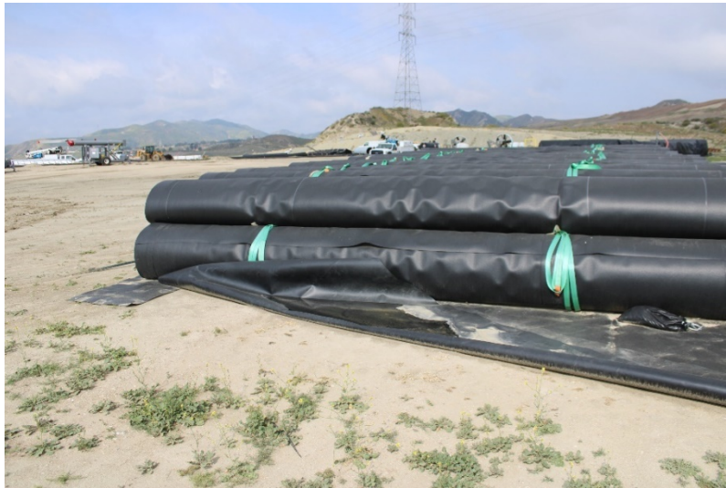
Photo 85: Closed Landfill – Primary Canyon: March 31, 2022
