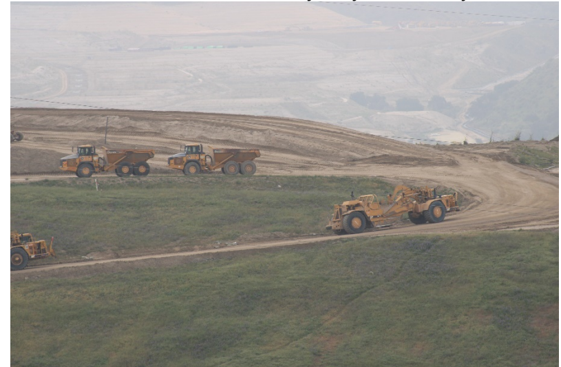
Photo 76: Closed Landfill - Primary Canyon: March 31, 2022
