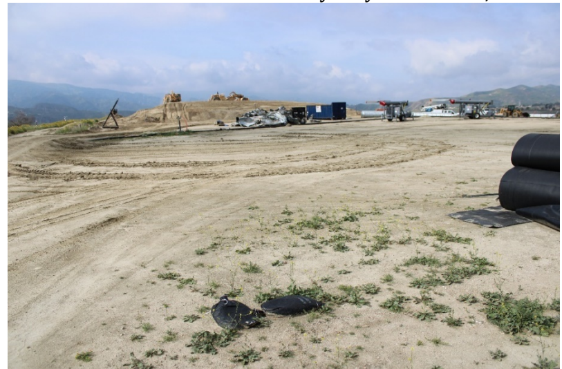
Photo 84: Closed Landfill – Primary Canyon: March 31, 2022
