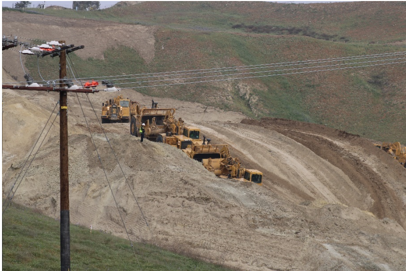
Photo 317: Cell 8 Construction: March 31, 2022
