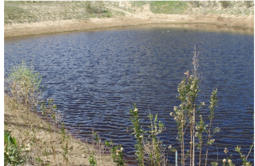
Photo 126: South Terminal and Catch Basins: February 22, 2022
