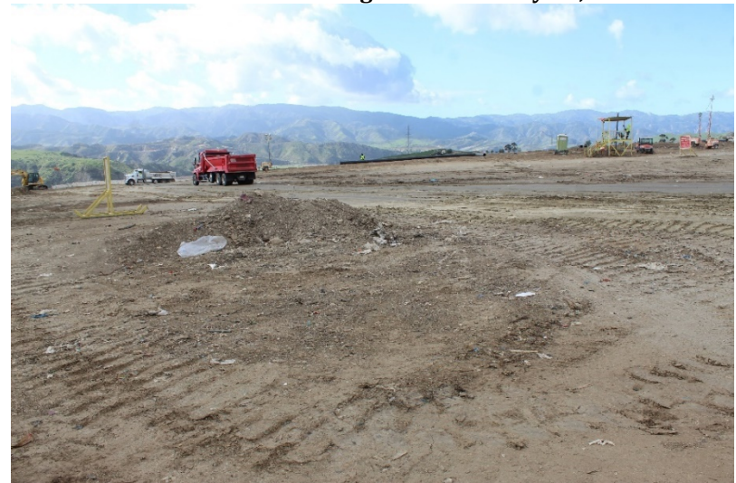
Photo 36: Cell 6 Working Area: February 22, 2022
