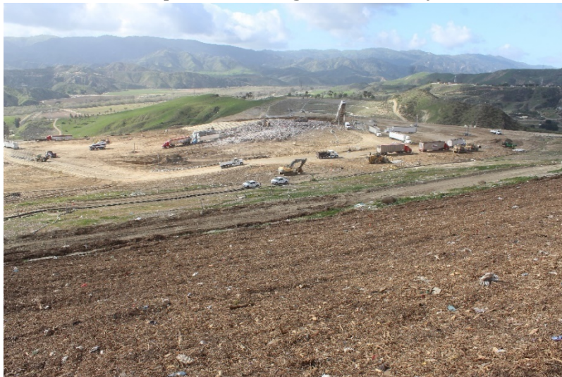
Photo 19: Top Deck Working Area: February 22, 2022
