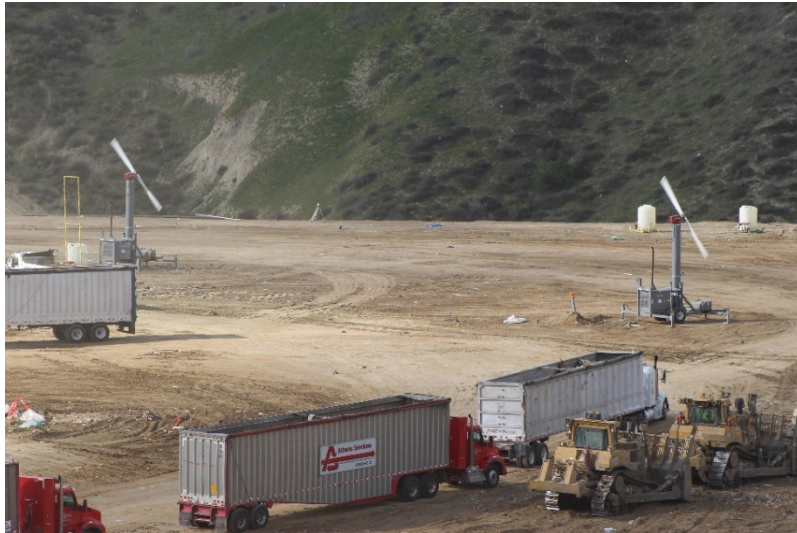
Photo 33: Cell 6 Working Area: February 22, 2022
