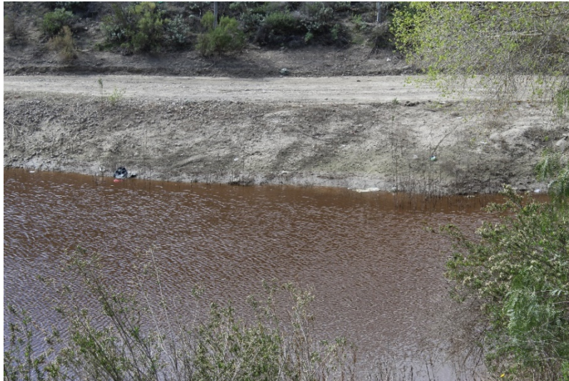
Photo 133: South Terminal and Catch Basins: February 22, 2022
