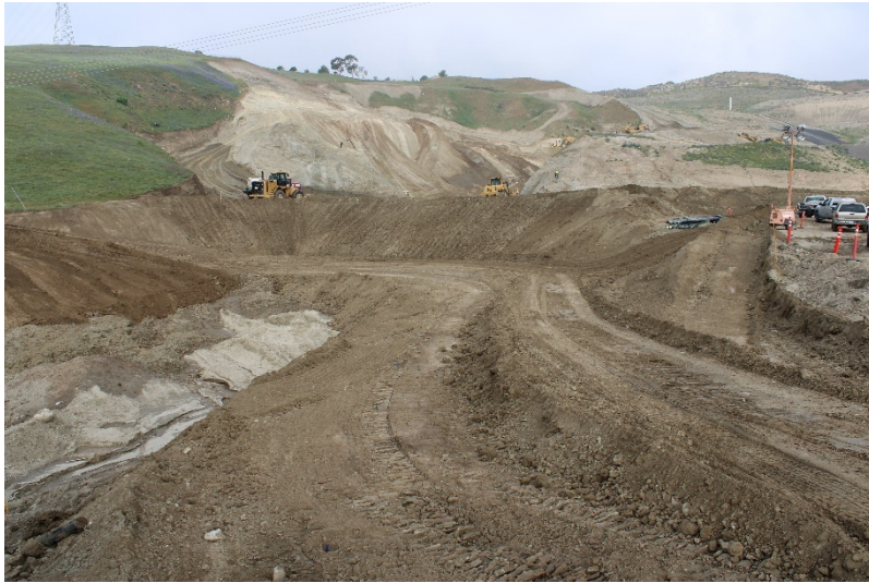
Photo 329: Cell 8 Construction: March 31, 2022
