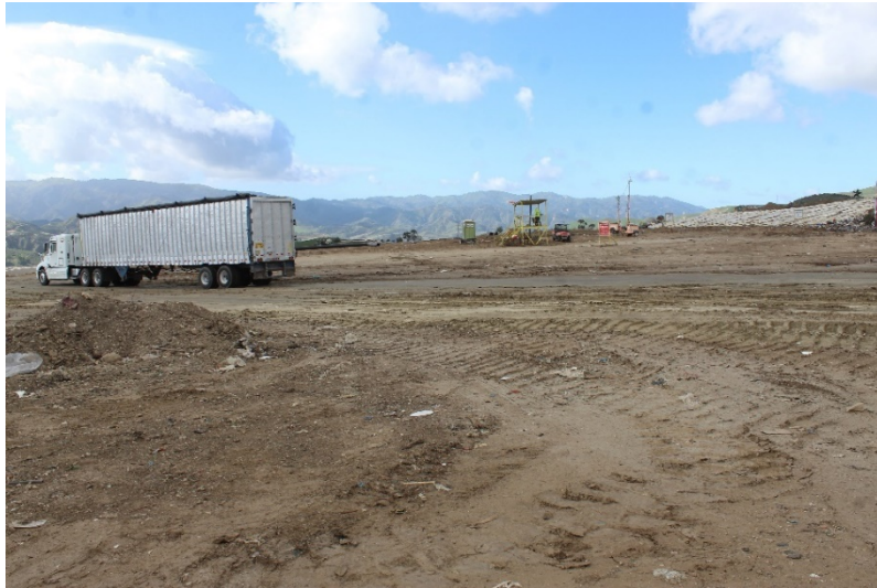
Photo 37: Cell 6 Working Area: February 22, 2022
