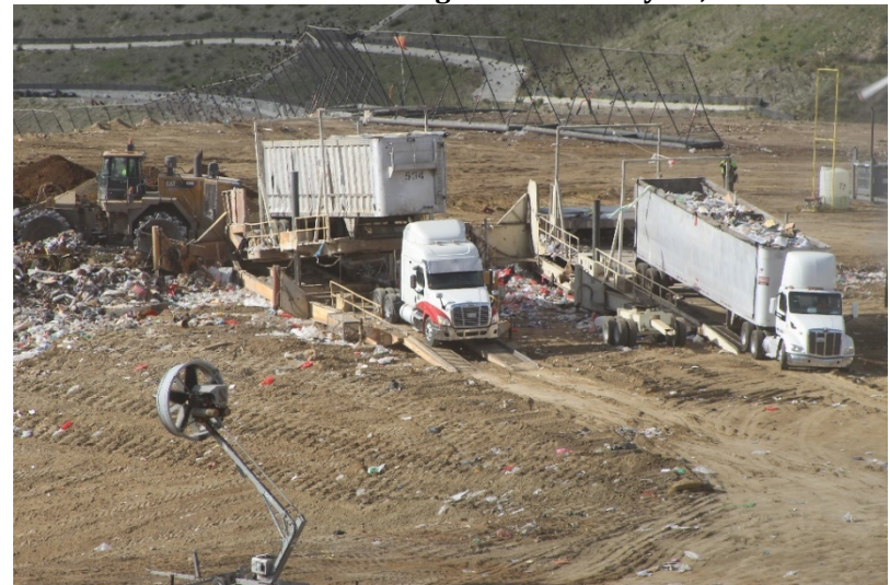
Photo 32: Cell 6 Working Area: February 22, 2022
