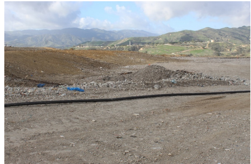
Photo 6: Top Deck Working Area: February 22, 2022
