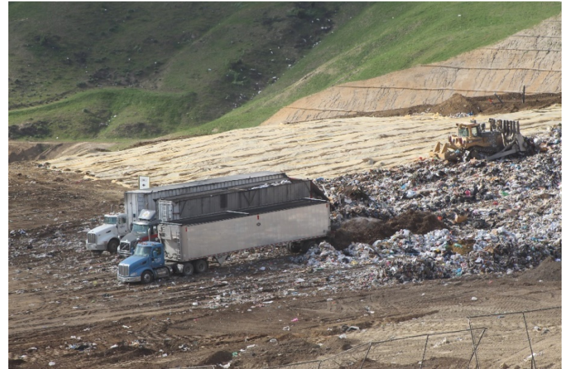
Photo 30: Cell 6 Working Area: February 22, 2022
