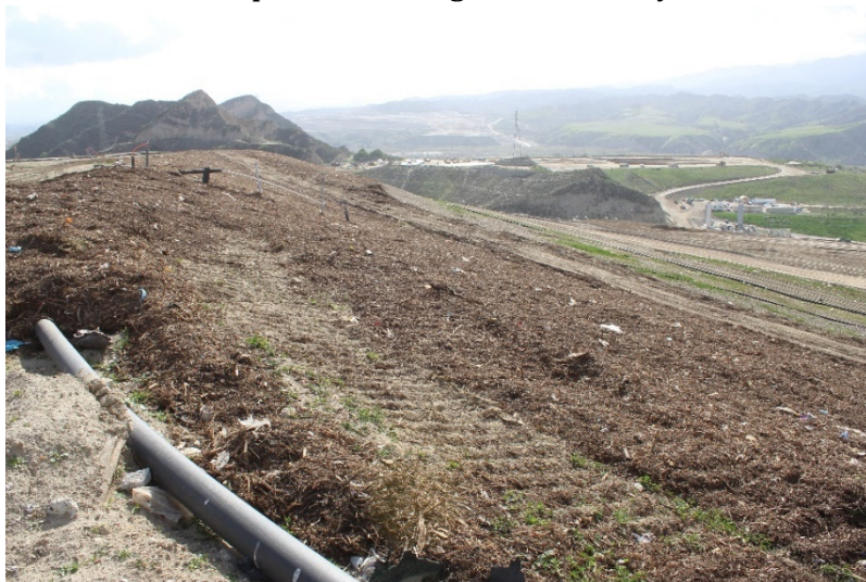
Photo 15: Top Deck Working Area: February 22, 2022
