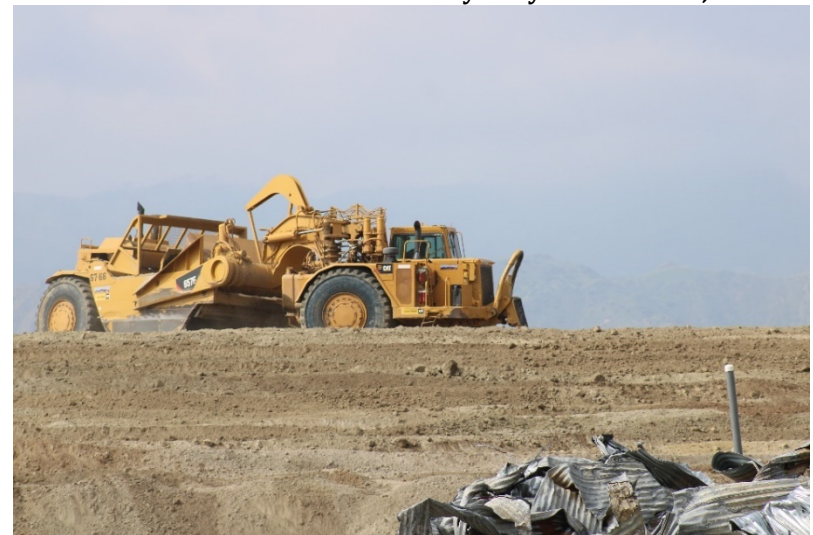
Photo 92: Closed Landfill – Primary Canyon: March 31, 2022
