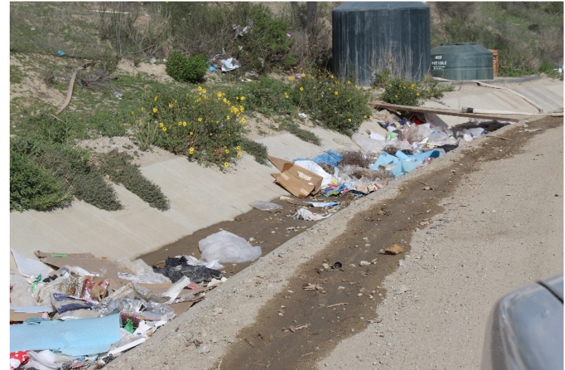
Photo 158: Landfill Perimeter Drainage Channel: February 22, 2022
