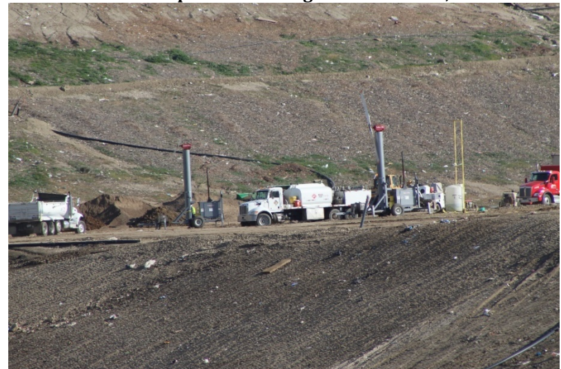
Photo 24: Cell 6 Working Area: February 22, 2022
