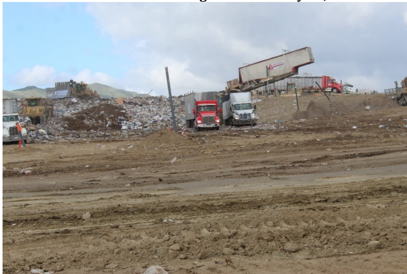
Photo 39: Cell 6 Working Area: February 22, 2022
