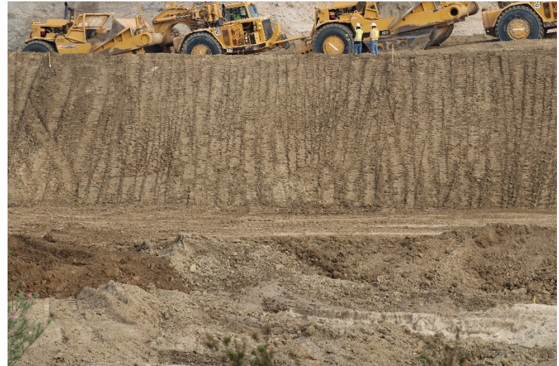
Photo 326: Cell 8 Construction: March 31, 2022
