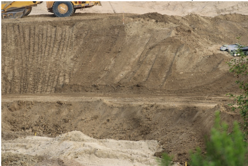
Photo 327: Cell 8 Construction: March 31, 2022
