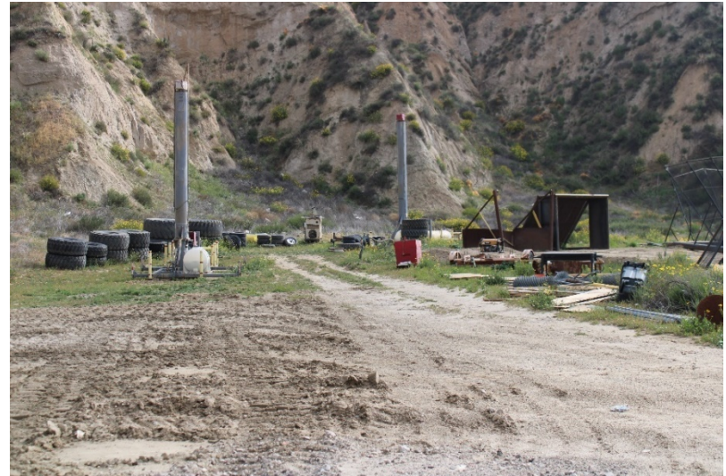
Photo 82: Closed Landfill – Primary Canyon: March 31, 2022
