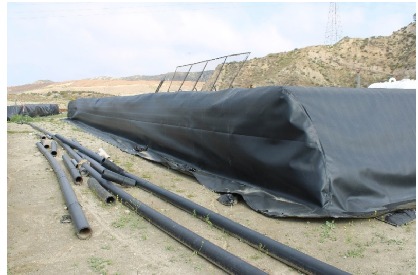
Photo 90: Closed Landfill – Primary Canyon: March 31, 2022
