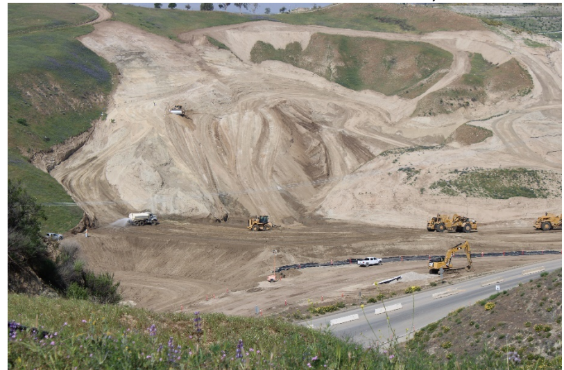
Photo 336: Cell 8 Construction: March 31, 2022
