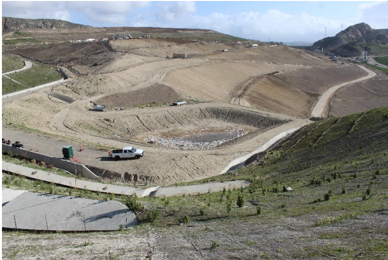
Photo 309: Cell 8 Construction: February 22, 2022
