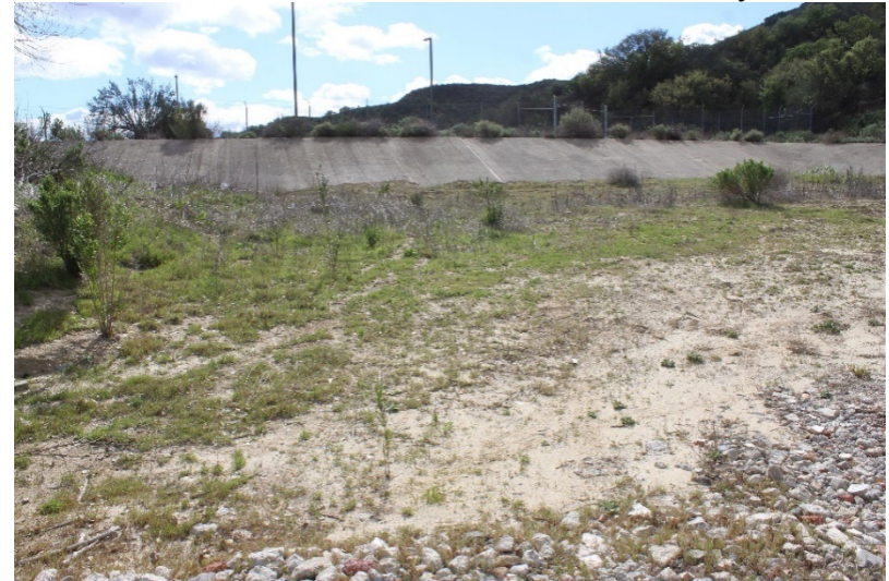
Photo 128: South Terminal and Catch Basins: February 22, 2022
