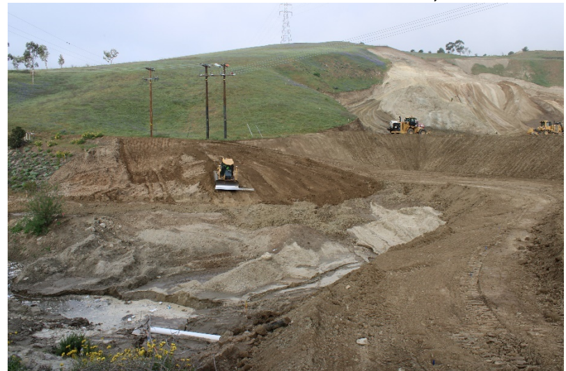
Photo 328: Cell 8 Construction: March 31, 2022
