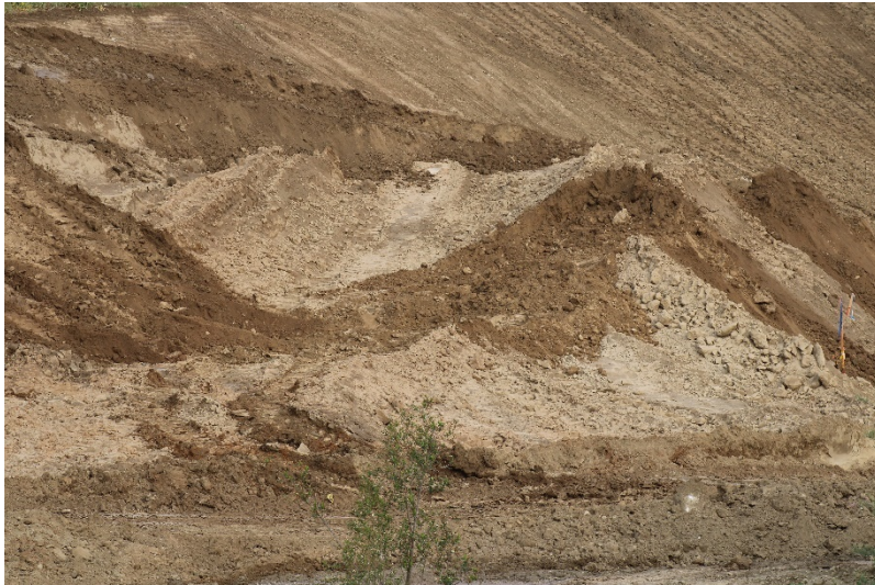
Photo 325: Cell 8 Construction: March 31, 2022
