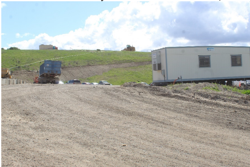
Photo 199: Maintenance and Admin Buildings: February 22, 2022
