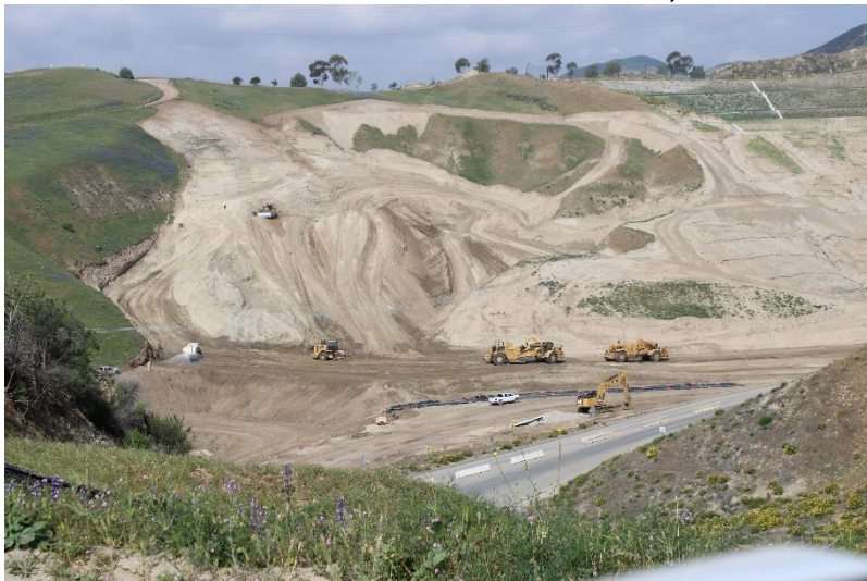
Photo 335: Cell 8 Construction: March 31, 2022
