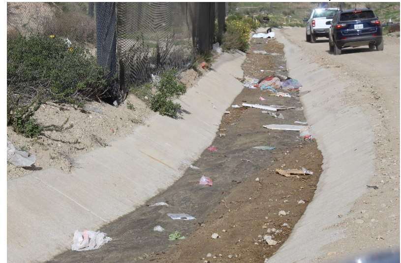
Photo 156: Site: February 22, 2022 February 22, 2022
