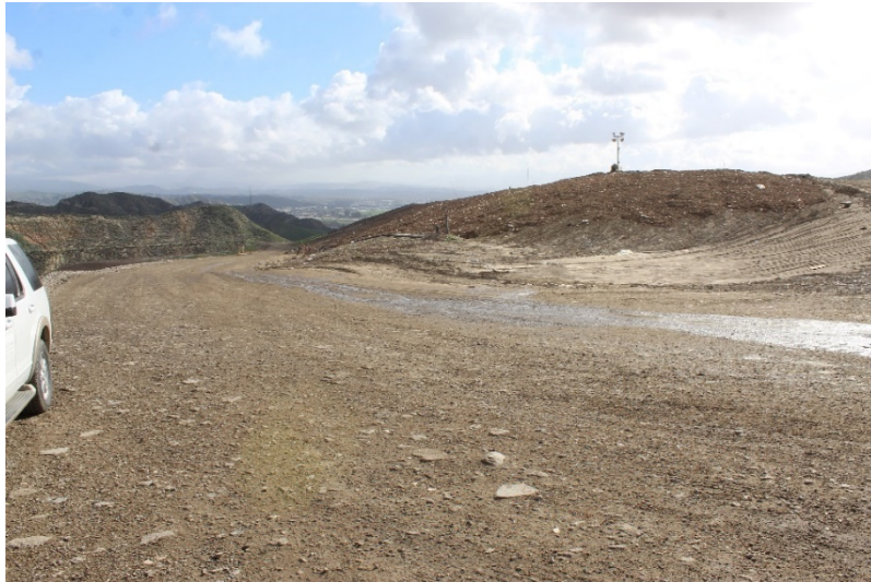
Photo 1: Top Deck Working Area: February 22, 2022
