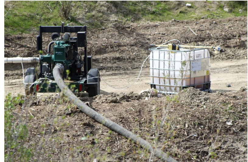
Photo 140: South Terminal and Catch Basins: February 22, 2022
