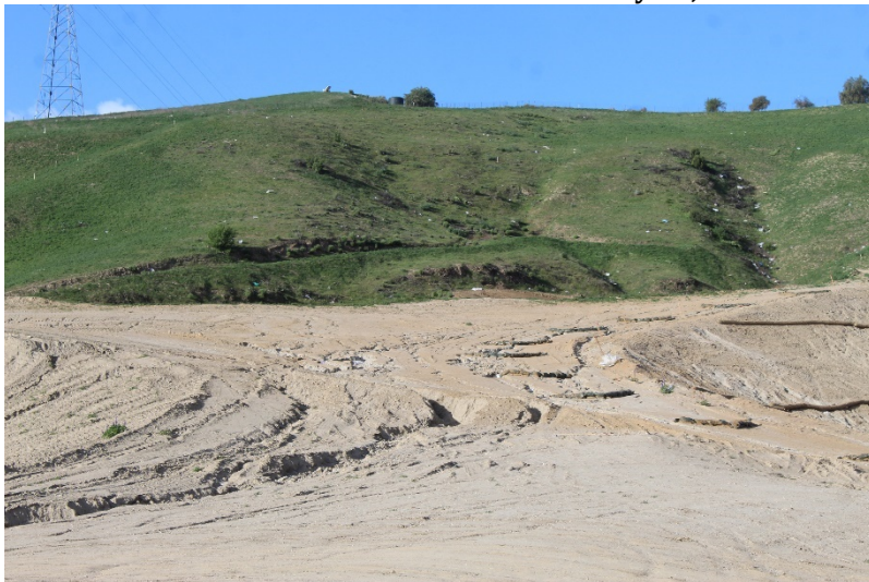
Photo 307: Cell 8 Construction: February 22, 2022
