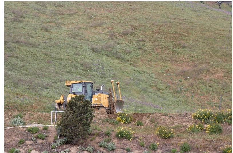
Photo 316: Cell 8 Construction: March 31, 2022
