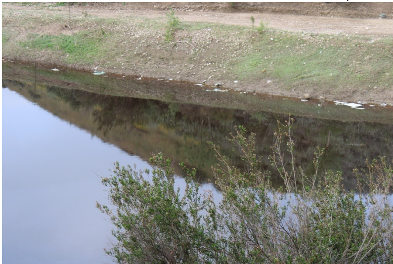
Photo 147: South Terminal and Catch Basins: March 31, 2022
