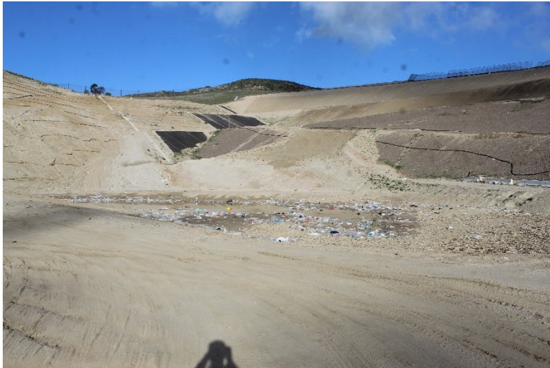
Photo 293: Cell 8 Construction: February 22, 2022
