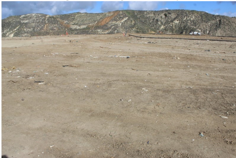
Photo 11: Top Deck Working Area: February 22, 2022
