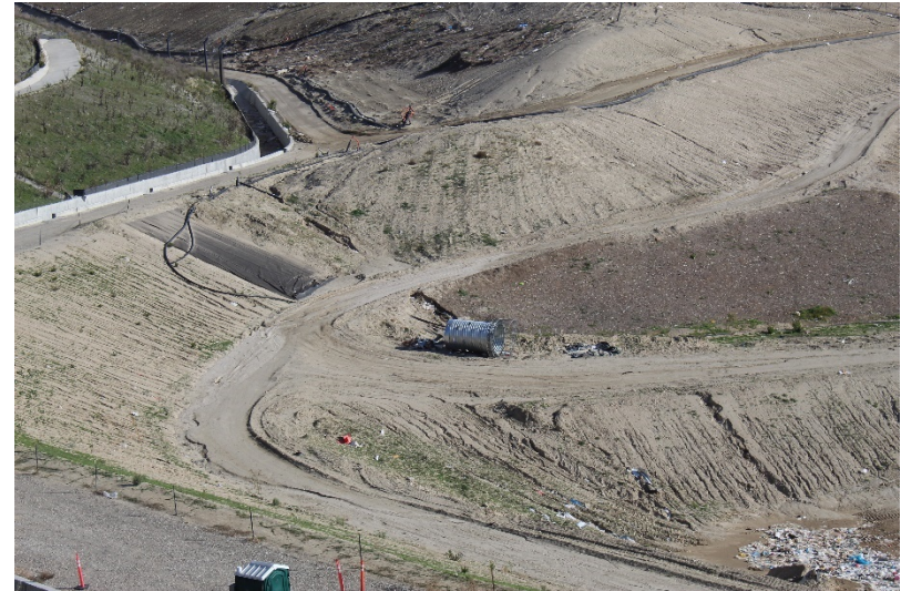
Photo 310: Cell 8 Construction: February 22, 2022
