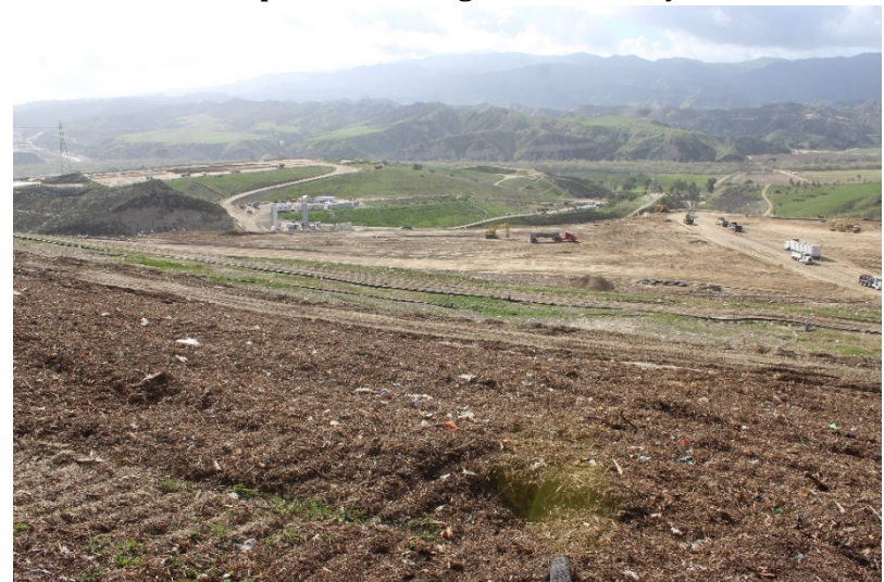
Photo 16: Top Deck Working Area: February 22, 2022
