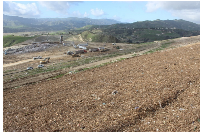
Photo 20: Top Deck Working Area: February 22, 2022
