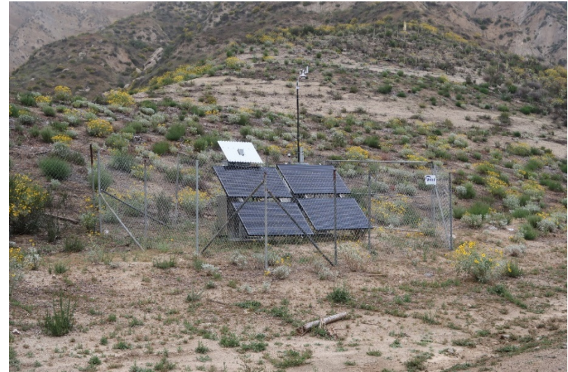
Photo 198: Wolcott Way Entrance Facilities: March 31, 2022
