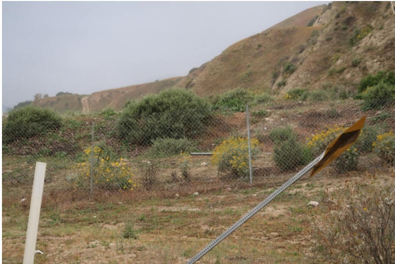
Photo 197: Wolcott Way Entrance Facilities: March 31, 2022
