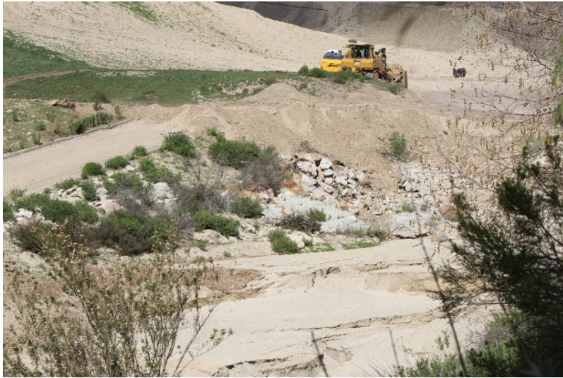
Photo 141: South Terminal and Catch Basins: February 22, 2022
