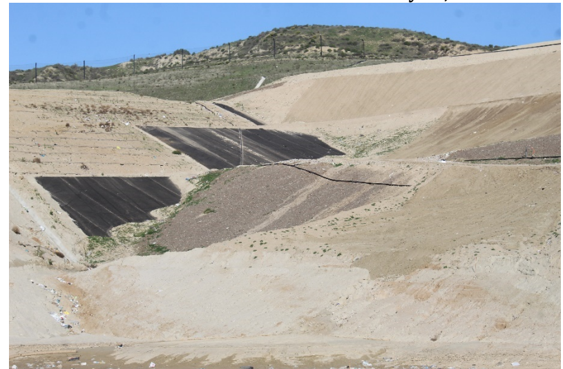
Photo 300: Cell 8 Construction: February 22, 2022
