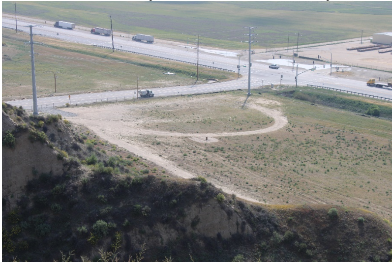
Photo 191: Wolcott Way Entrance Facilities: March 31, 2022
