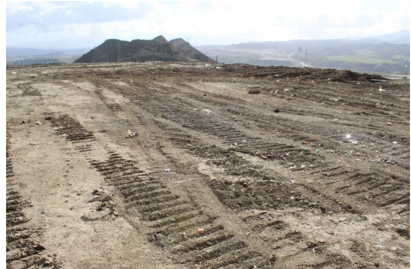
Photo 14: Top Deck Working Area: February 22, 2022
