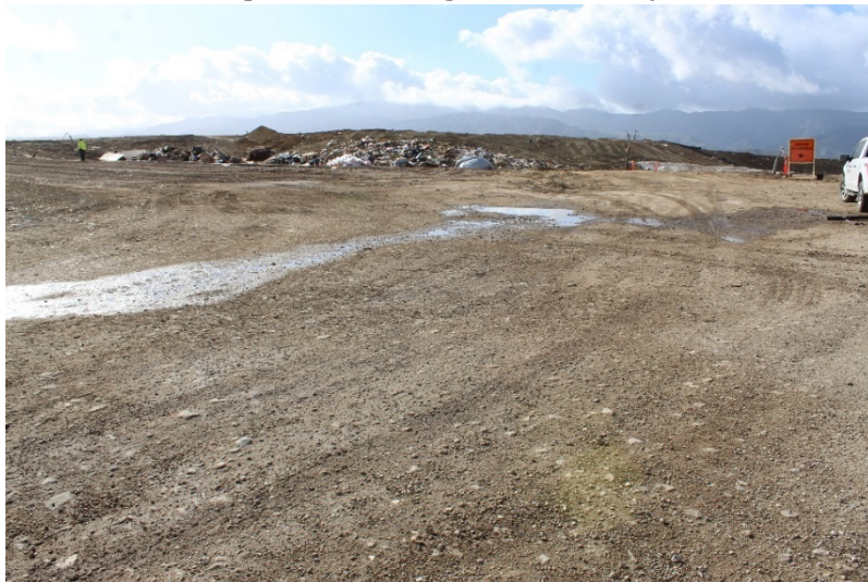
Photo 3: Top Deck Working Area: February 22, 2022
