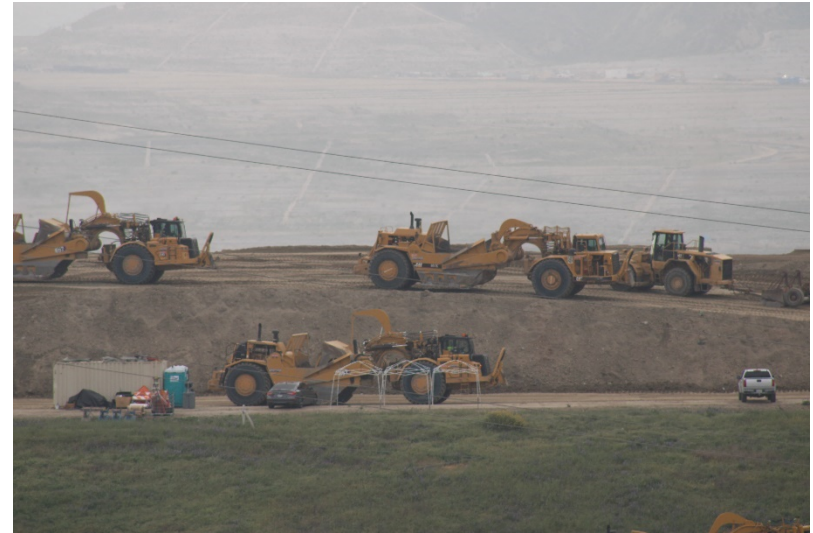
Photo 78: Closed Landfill - Primary Canyon: March 31, 2022
