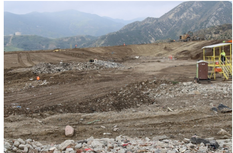
Photo 22: Top Deck Working Area: March 31, 2022
