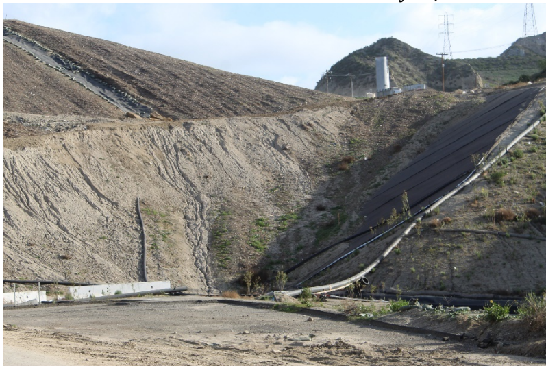
Photo 303: Cell 8 Construction: February 22, 2022
