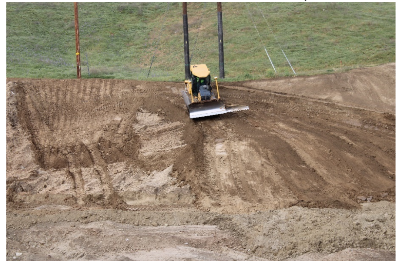
Photo 332: Cell 8 Construction: March 31, 2022
