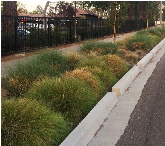
Figure 2-119 Bioswale with native grasses. Thousand Oaks, CA. Source: Gruen Associates
