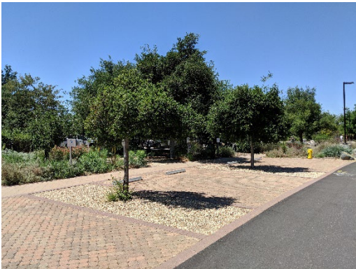
Figure 2-123 High solar reflectance pavers mitigating heat island effect. Governors Island, NY. Source: Gruen Associates
