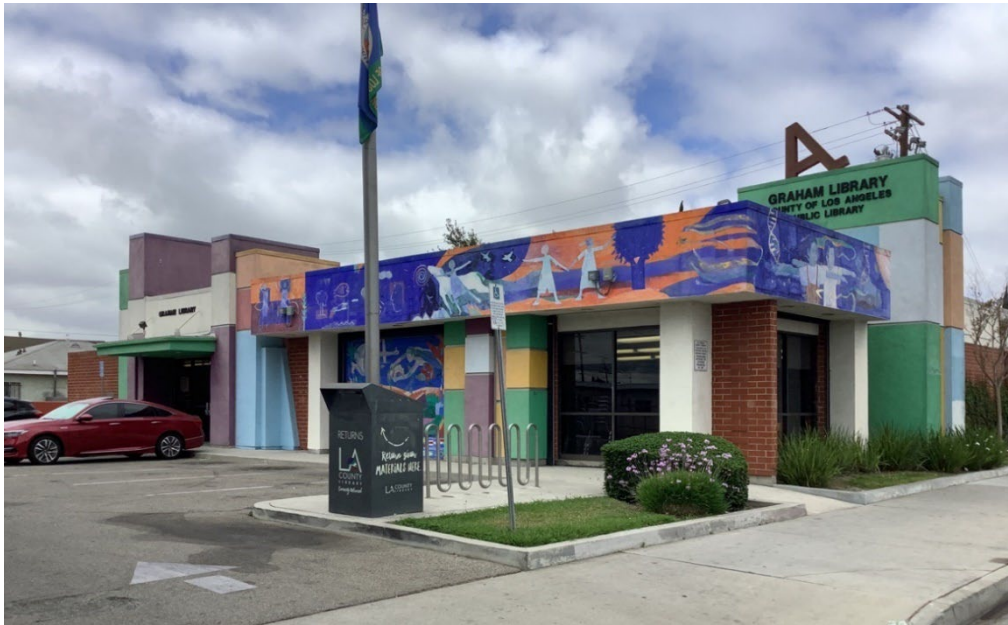
Firestone Library, 1900 Firestone Boulevard, Florence-Firestone
