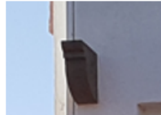
Decorative Exposed Rafter Tails
