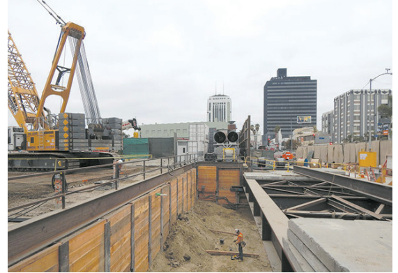
Coordination of underground utilities is critical to safely and efficiently operate Metro service.
