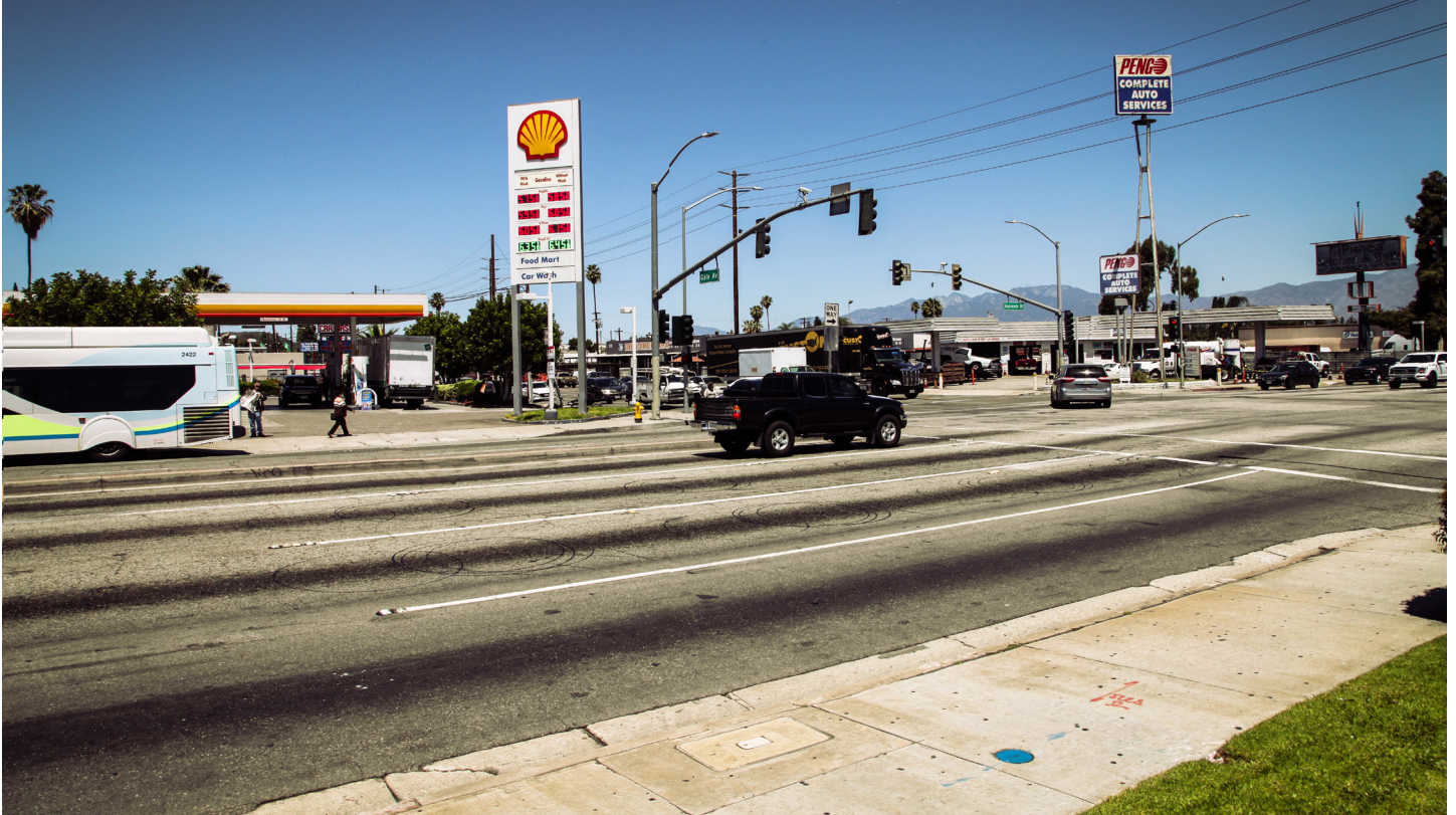
Typical Conditions (Before)
