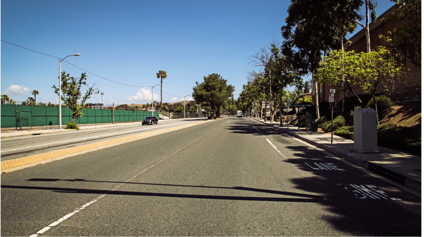
Typical Conditions (Before)
