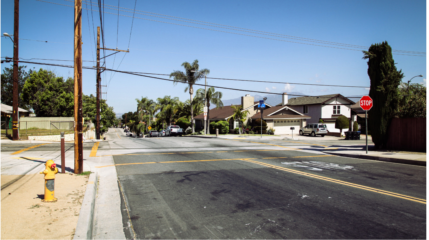
Typical Conditions (Before)
