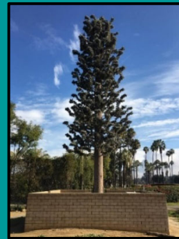
SBA Monarch Towers I, LLC/T-mobile
