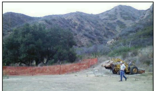
Preservation during grading C. Cuba
