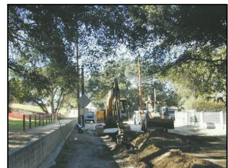
Utility upgrades T. Garrison
