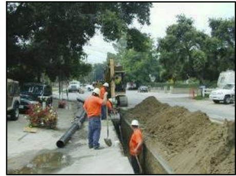
Utility line replacement C. Cuba
