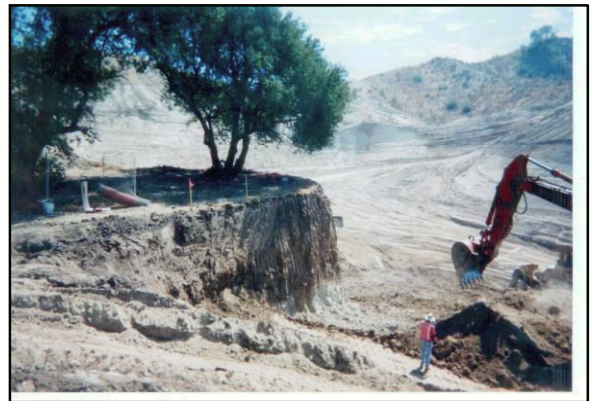
Construction monitoring C. Cuba
