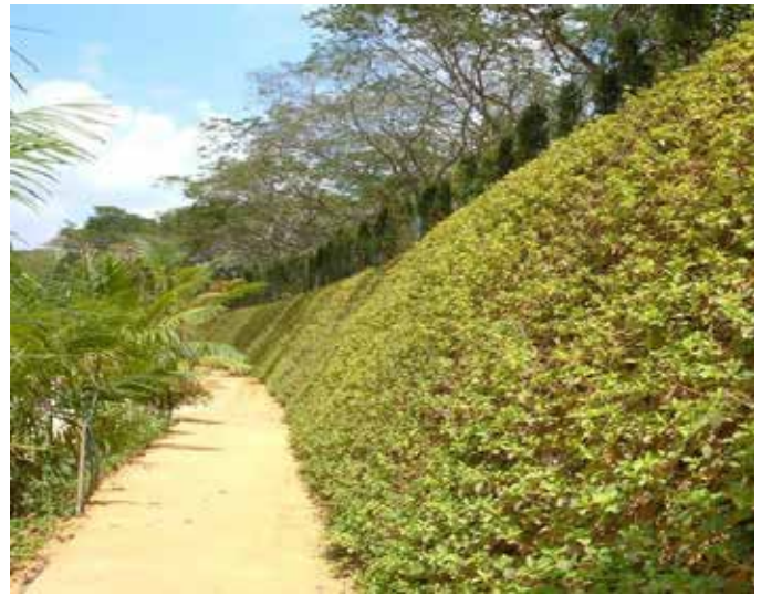
Vegetated Retaining Walls
