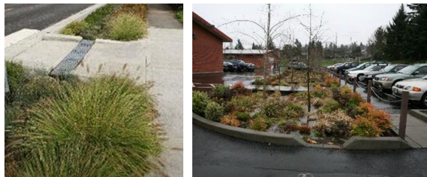
Vegetated infiltration and retention basins can serve as effective stormwater management tools as well as provide attractive naturalized open spaces for project residents.
