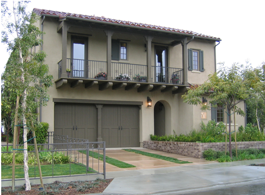
Architectural forms of classic mission and Monterey structures, such as arches and balconies, are incorporated in contemporary buildings to reflect early California heritage.
