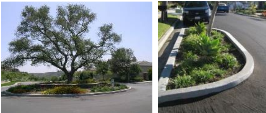
Roundabouts and chokers are one of many effective traffic-calming design measures that can be incorporated into Centennial's roadway network.
