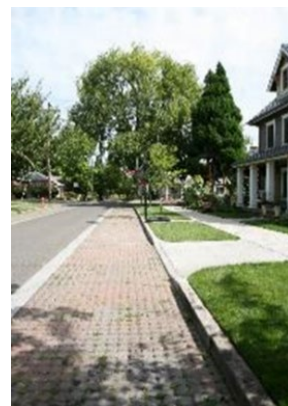
Green infrastructure can include features such as swales, vegetated buffers, sand filters, and artificial wetlands, which can be used to manage stormwater runoff and improve stormwater quality. Permeable paving reduces stormwater runoff and produces smaller increases in ambient air temperature than more energy-absorptive traditional paving materials
