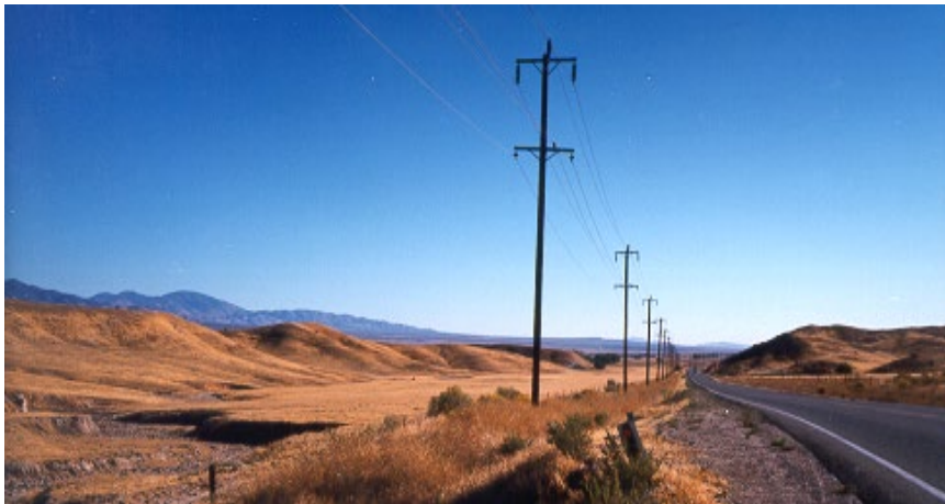
Existing utility lines that will serve Centennial follow SR-138.
