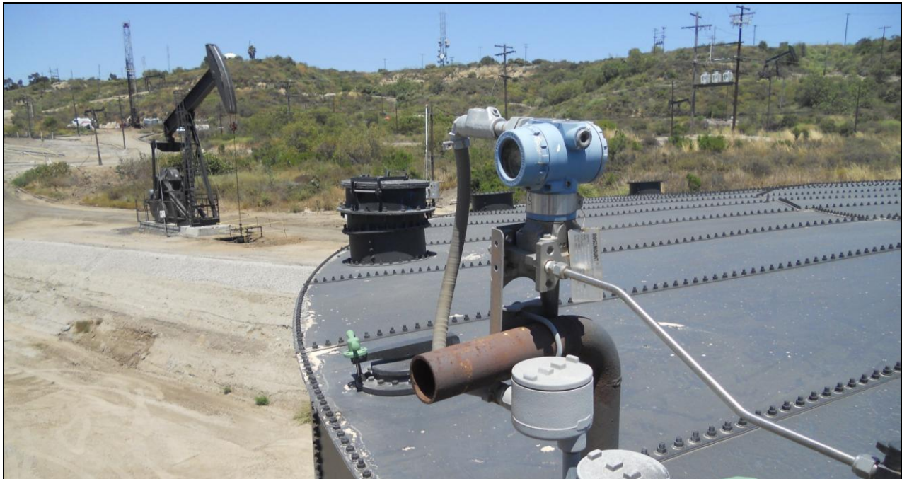
Tank Vapor Vent on Tank 2
