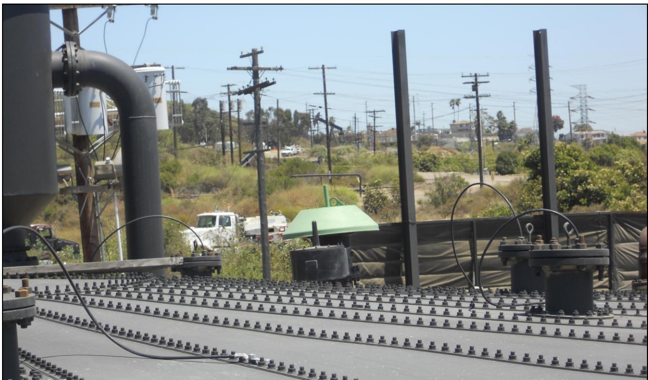
Tank Vapor Vent on Tank 2
