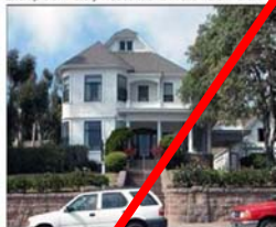
Example of a 2-1/2-story House with a raised Front Yard and wrap-around Porch.
