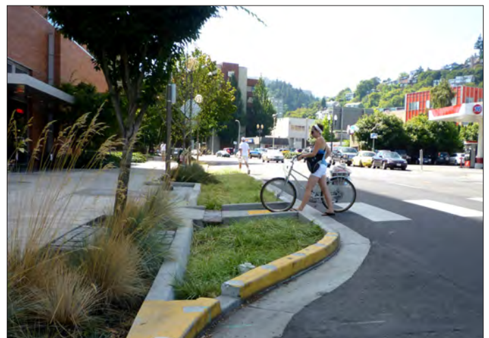
A curb extension with infiltration planters and enhanced crosswalk.
