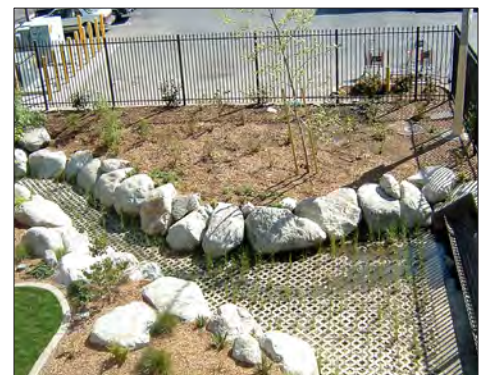
Storm water treatment
