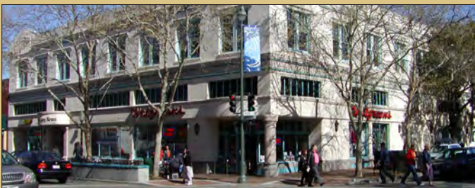
Housing over stores and offices
