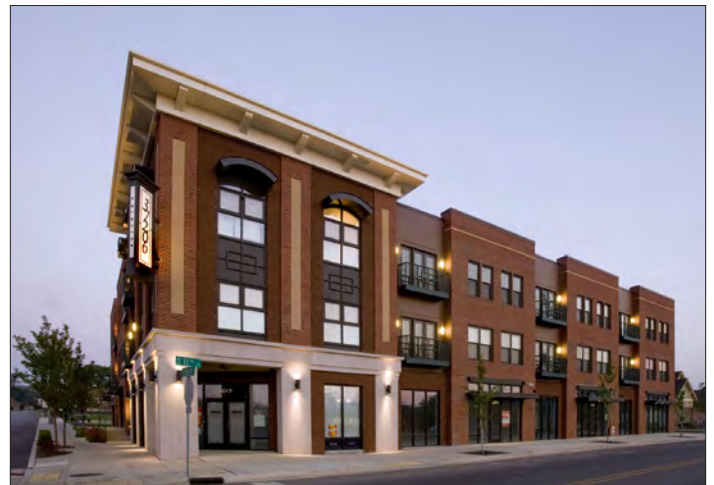
Mixed-use three story building example
