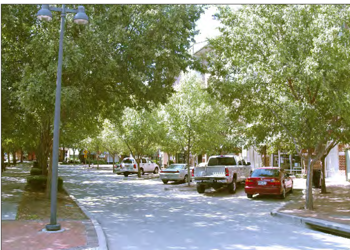
A V-gutter allows storm water to flow between the parking and the street.
