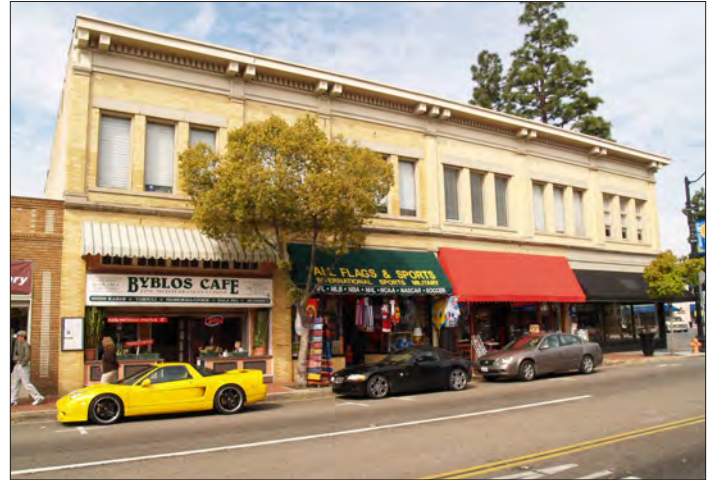
Two-story mixed-use building with offices or housing above
