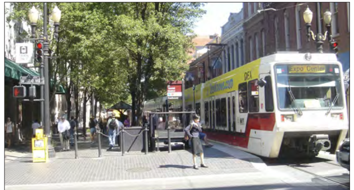
A pedestrian-oriented light rail station
