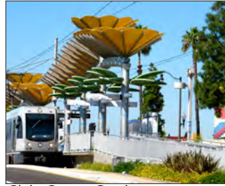
Civic Center Station
