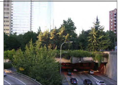
Freeway Park, Seattle
