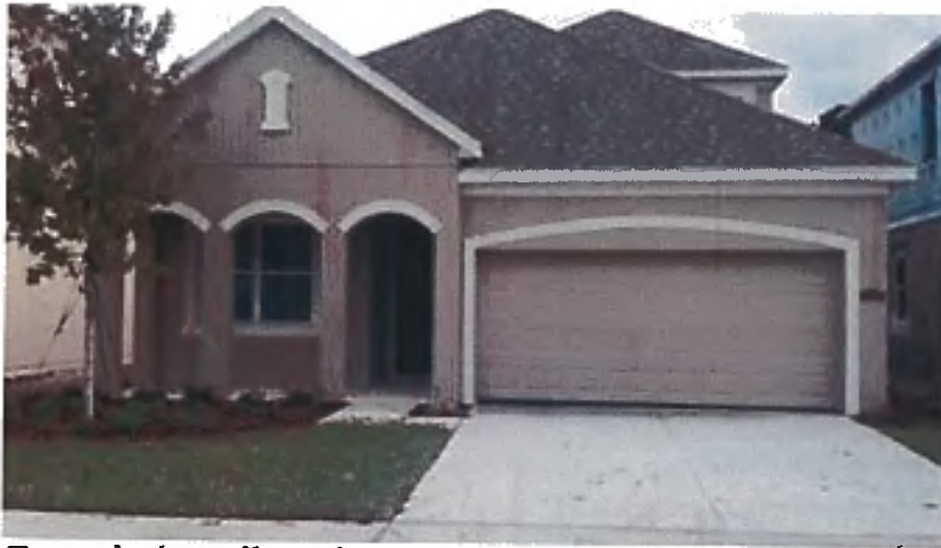
Example (not allowed): Double-loading garage door for two-car garage facing the street.
