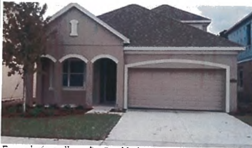
Example (not allowed): Double-loading garage door for two-car garage facing the street.
