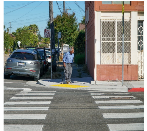
Example of a curb ramp and truncated dome
