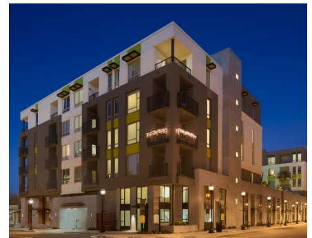
Illustrative photo of architecturally compatible lighting.
