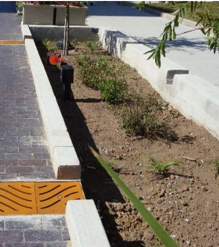
Illustrative photo of stormwater infiltration planter and drainage grate.
