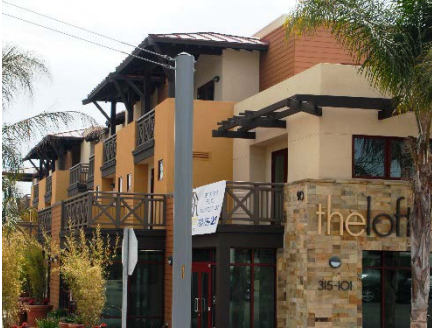
Illustrative photo of building modulation and articulation.
