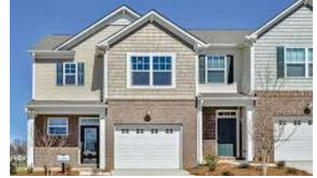
Example of attached housing that may be allowed in the CSLA R-2 Zone.
