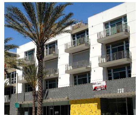
Example of balconies facing the sidewalk, which provide "eyes on the street."
