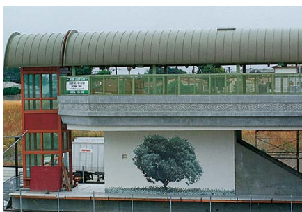
Existing view of transit station boarding area.
