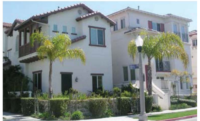
Example of multi-family residential development.
