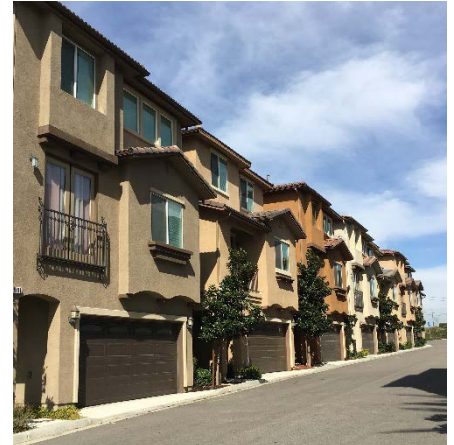
Existing Residential homes in the Specific Plan area.
