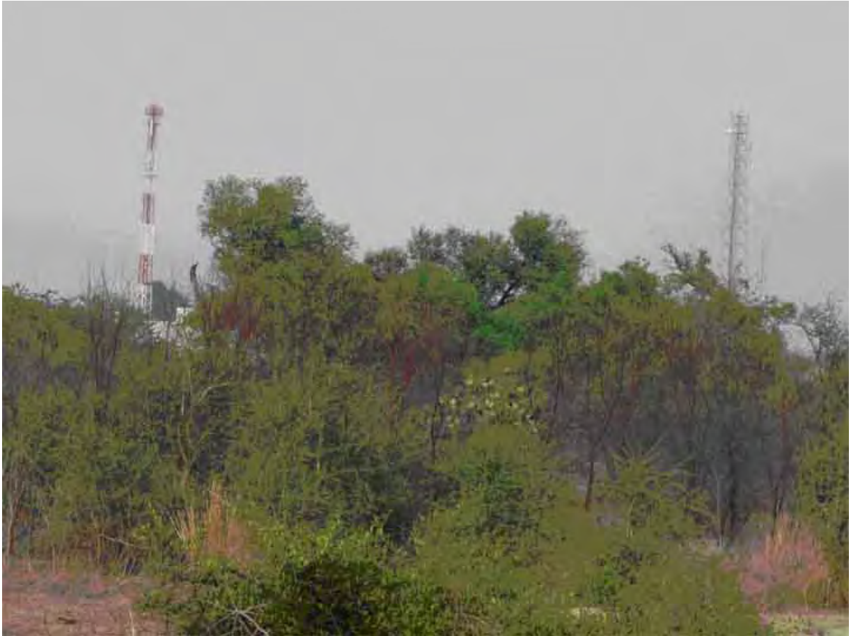
Cell Phone towers near Keoladeo National Park, Bharatpur, Rajasthan
